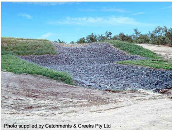
Basin spillway with two 90-degree bends
