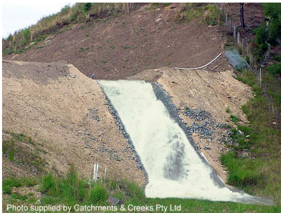
Supercritical flow down a spillway (NSW)
