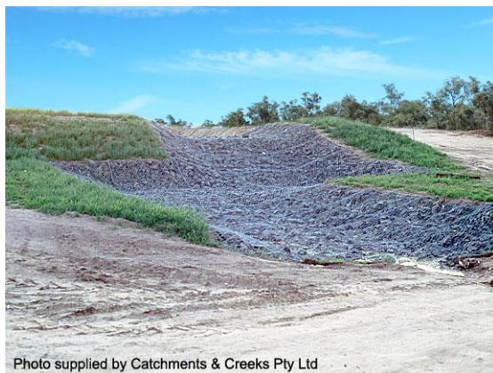
Basin spillway with two 90-degree bends
