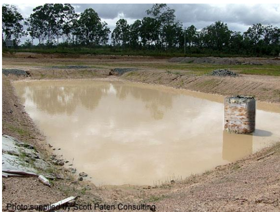
Type C basin with riser pipe outlet
