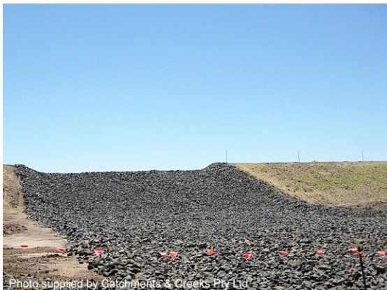
Rock-lined spillway (Qld)
