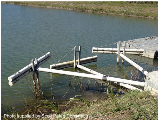
Multiple outlet system (Qld)
