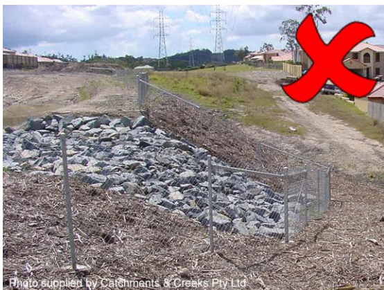
Sediment basin spillway
