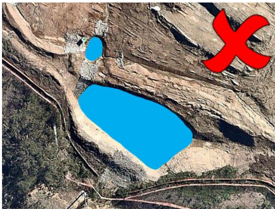
Forebay not aligned with basin
