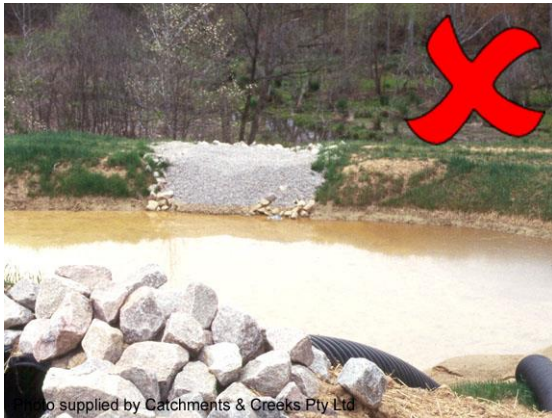
Insufficient freeboard
