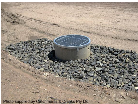
Riser pipe with aggregate filter (Qld)
