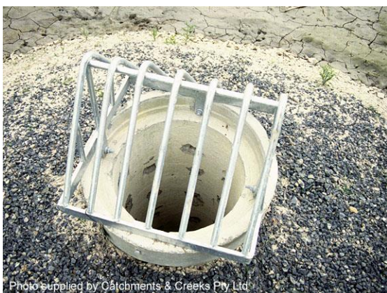
Riser pipe with aggregate filter (NSW)
