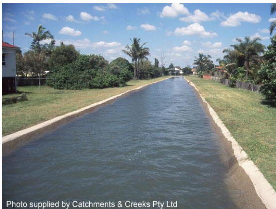
High tide backing-up into a coastal drain
