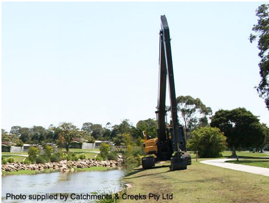
Basin de-silting (Qld)
