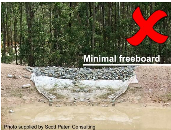
Insufficient freeboard
