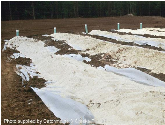
Sand filter under construction (USA)
