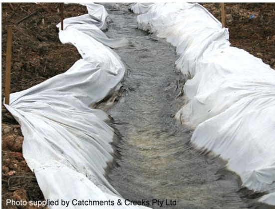
Geotextile-lined drain (NSW)
