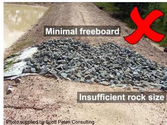
Insufficient freeboard
