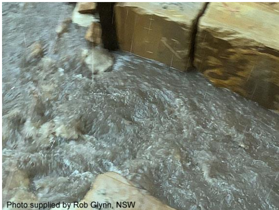
90-degree bend in a constructed channel
