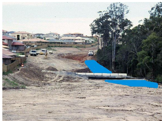
Road construction over stormwater pipe
