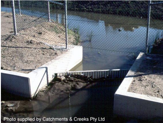
Litter screen at basin inlet (Qld)
