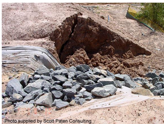
Embankment failure
