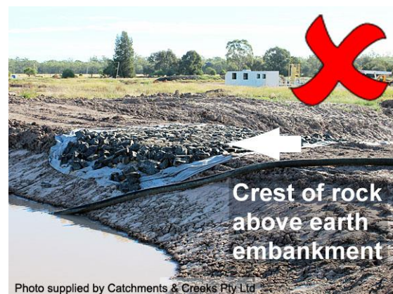
Insufficient freeboard
