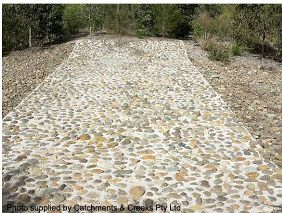
Concrete spillway crest (Qld)
