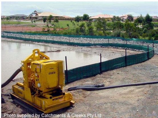
Pumped decant system (Qld)
