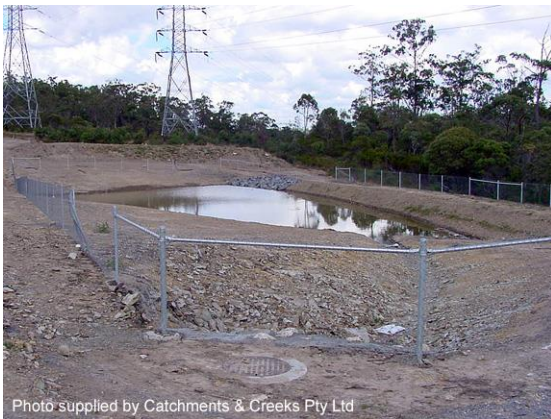
Fenced sediment basin adjacent to a creek
