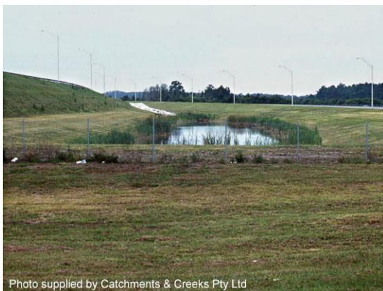
Pollution containment pond (USA)
