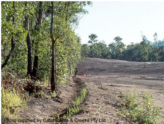
Catch drain diverting 'clean' bush runoff
