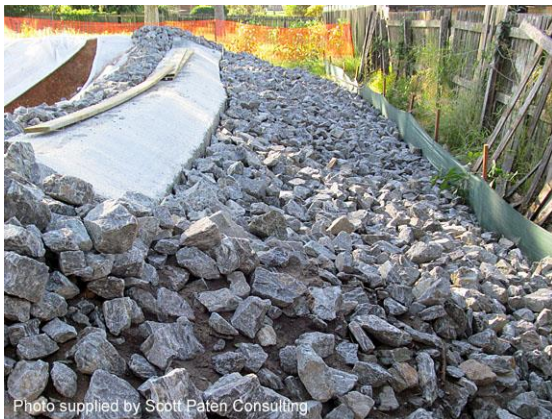
Flow must turn 90-degrees at base of spillway
