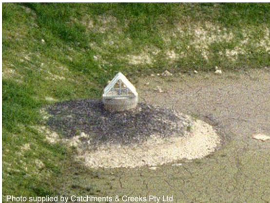
Riser pipe with aggregate filter (NSW)
