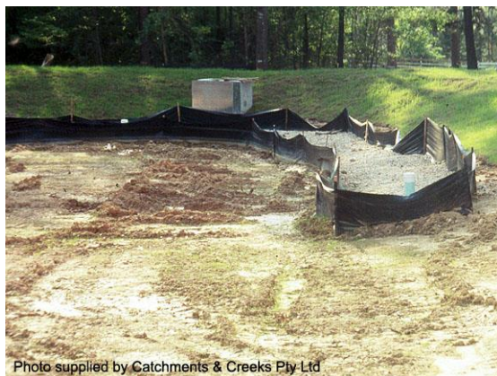
Sand filter surrounded by sed-fence (USA)
