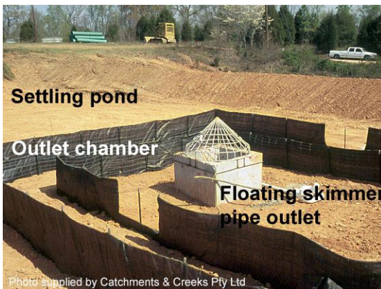
Skimmer pipe inside an outlet chamber
