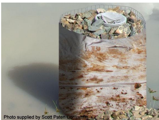
Gabion riser wrapped in filter cloth
