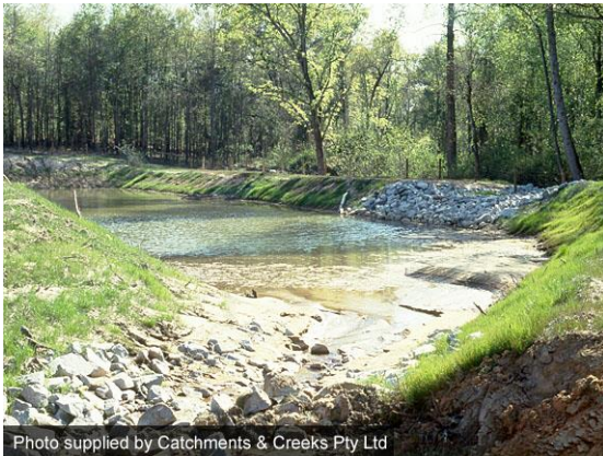
Rock filter dam outlet system (USA)
