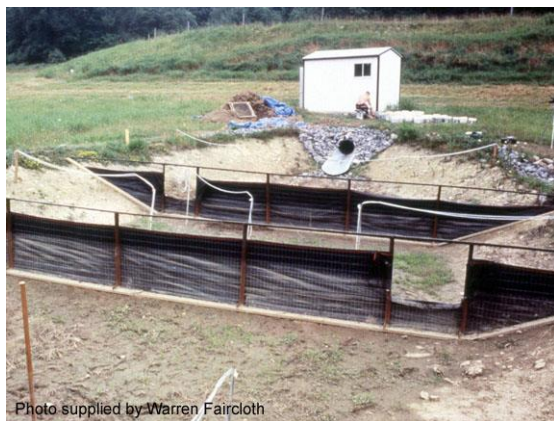
Permeable internal baffles (not ideal)
