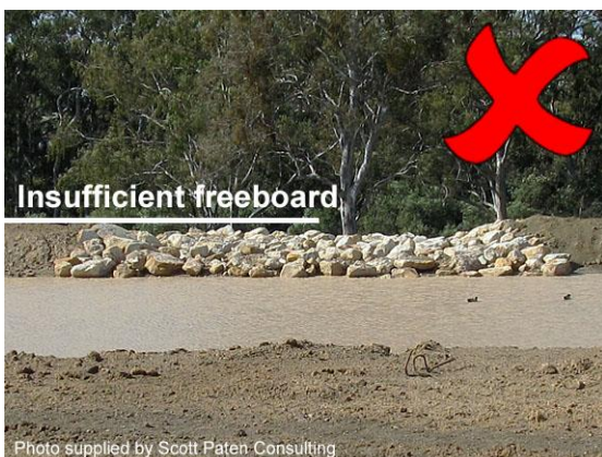
Insufficient freeboard
