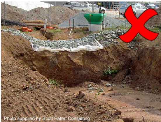
Step downstream face of forebay
