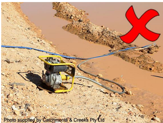
Intake pipe resting on the basin floor
