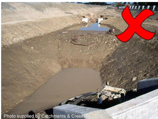
Intake pipe resting on the basin floor
