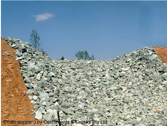
Crest of a rock-lined chute (USA)
