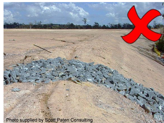
Insufficient freeboard
