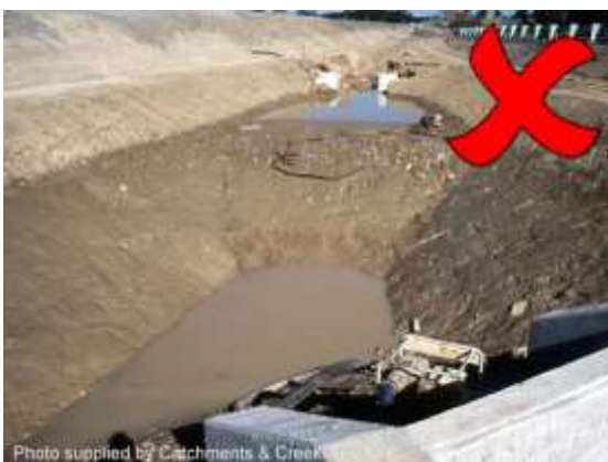
Intake pipe resting on the basin floor
