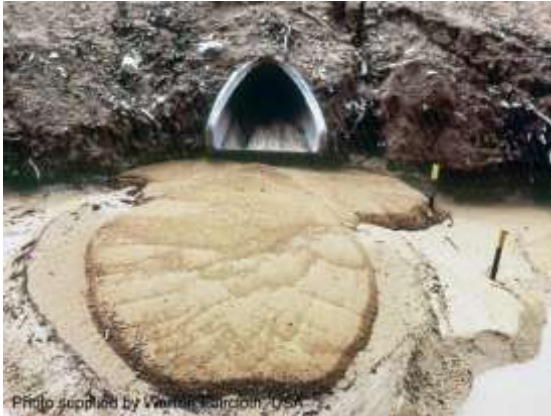
Deposition of coarse sediment (USA)
