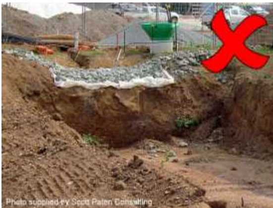
Steep downstream face of forebay
