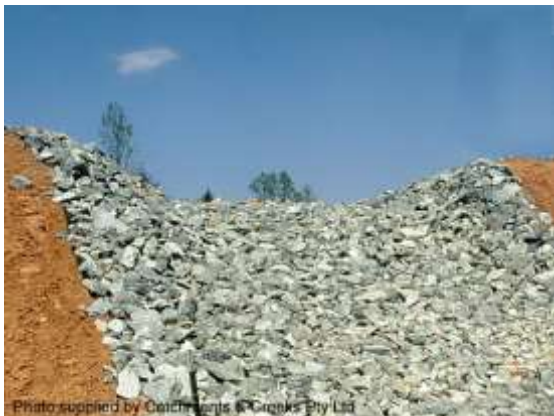
Crest of a rock-lined chute (USA)
