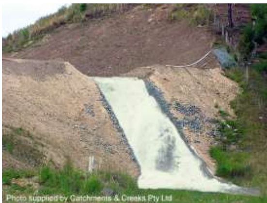
Supercritical flow down a spillway (NSW)
