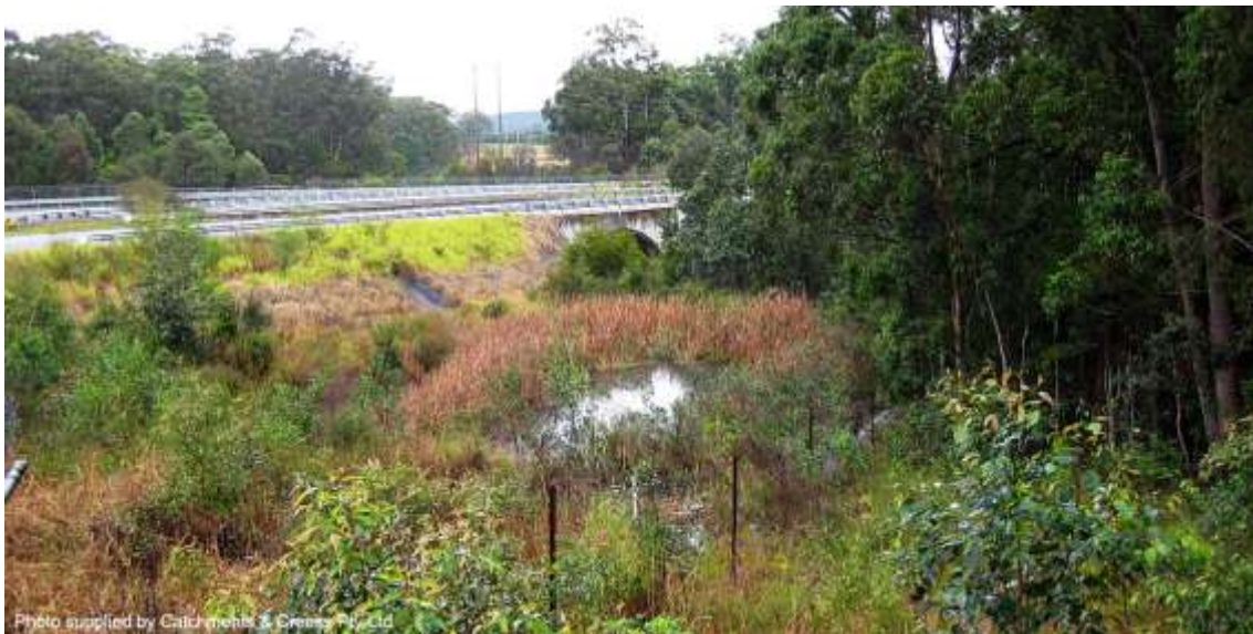
Sediment basins in the above site converted into wetlands (NSW)
