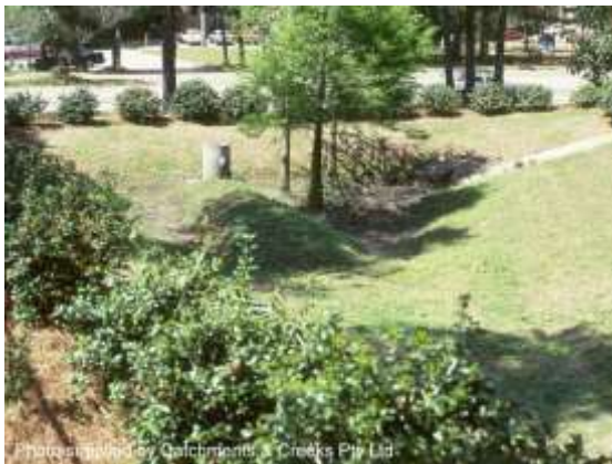
Sediment basin converted to OSD (USA)
