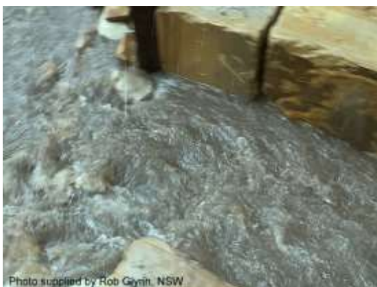
90-degree bend in a constructed channel
