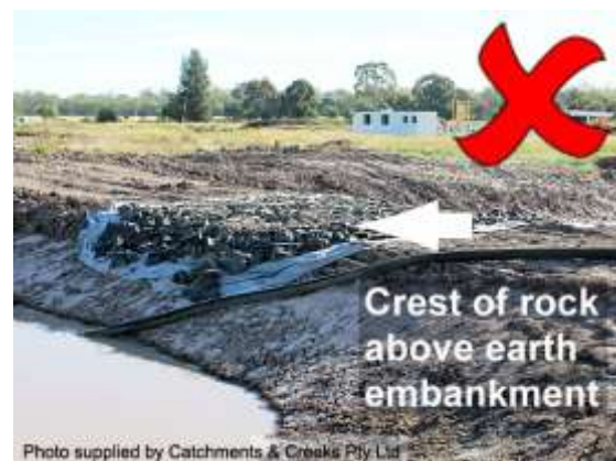
Insufficient freeboard
