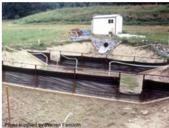
Permeable internal baffles (not ideal)
