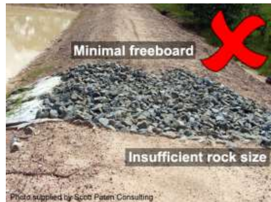
Insufficient freeboard
