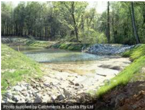
Rock filter dam outlet system (USA)
