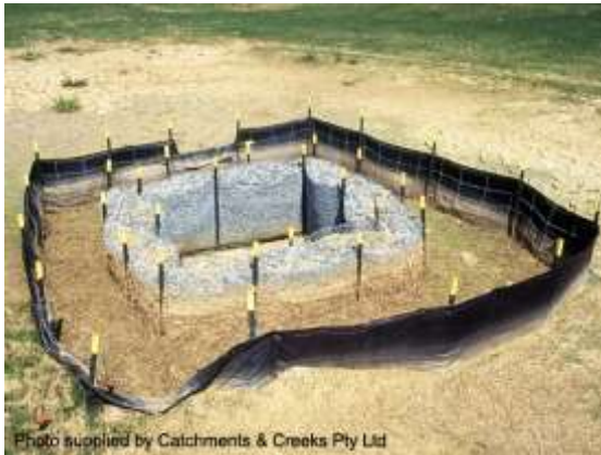
Sediment weir outlet system (USA)
