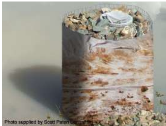
Gabion riser wrapped in filter cloth
