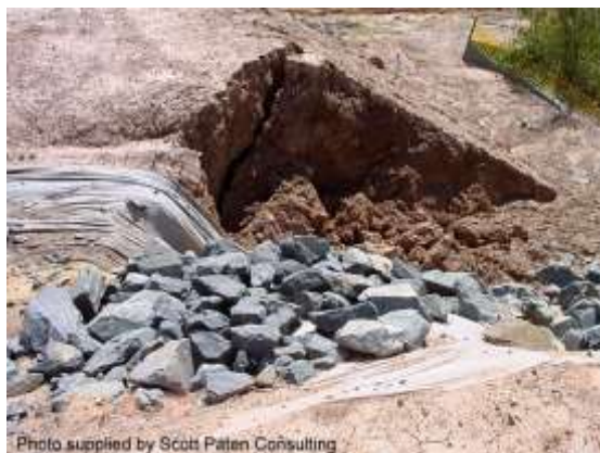
Embankment failure
