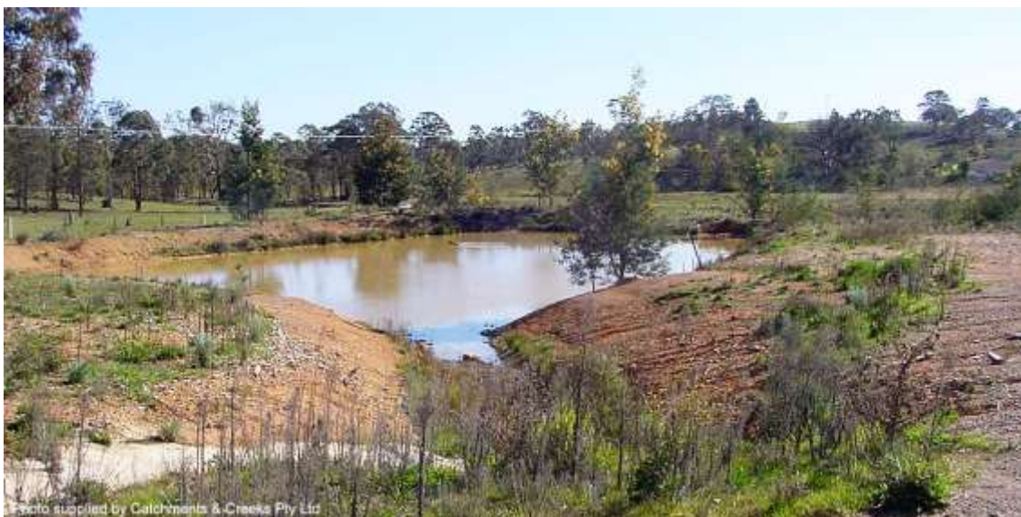
Sediment basin (associated with adjacent road works) retained as a farm dam (NSW)
