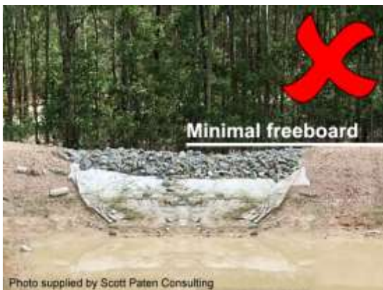
Insufficient freeboard
