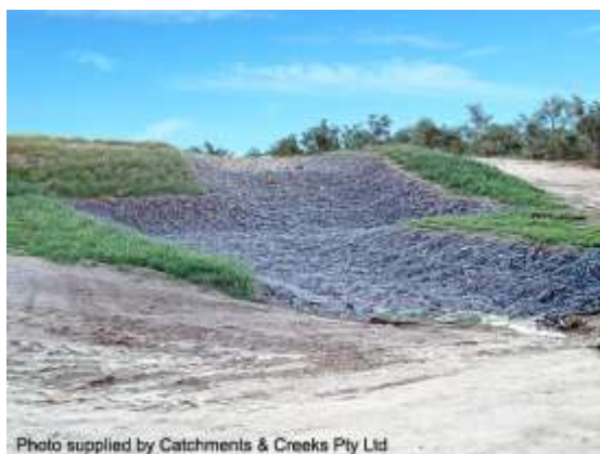
Basin spillway with two 90-degree bends
