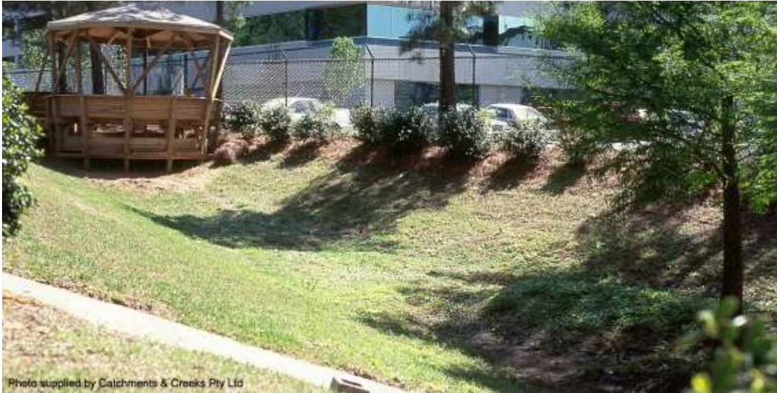
Basin converted to a detention basin, garden and area for factory works to lunch (USA)
