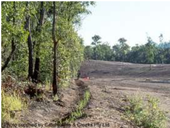
Catch drain diverting 'clean' bush runoff
