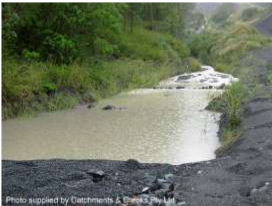
Constructed drain flowing into a basin
