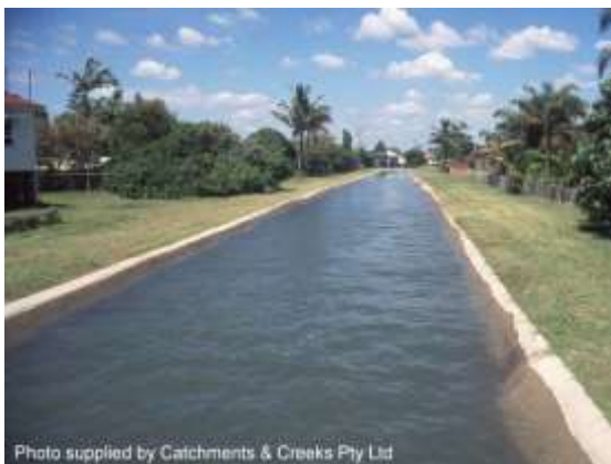
High tide backing-up into a coastal drain
