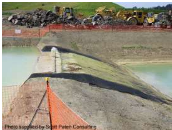
Bank slope downstream of level spreader
