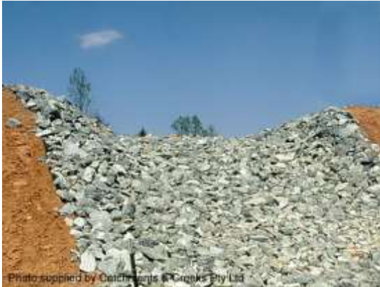
Crest of a rock-lined chute (USA)
