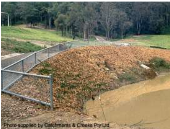
Partially fenced sediment basin (NSW)
