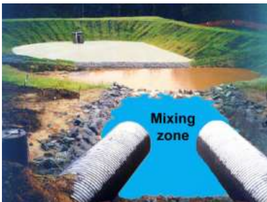
Energy dissipation and further mixing
