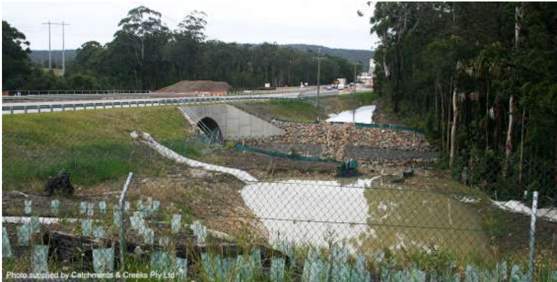
Sediment basins in operation during road construction works (NSW)
