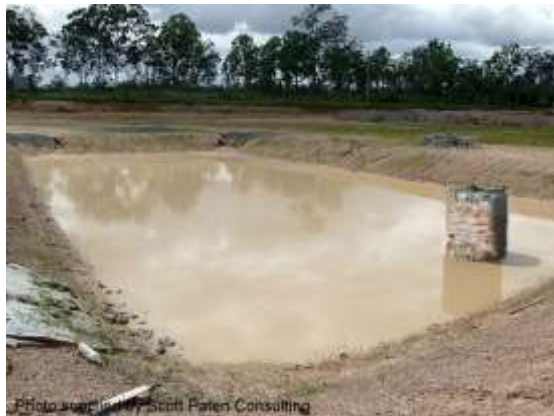
Type C basin with riser pipe outlet
