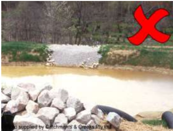
Insufficient freeboard
