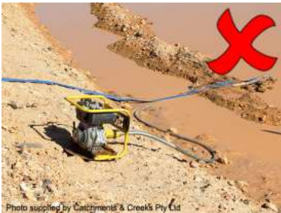
Intake pipe resting on the basin floor
