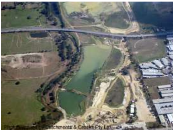
Several basins operating in 'series'
