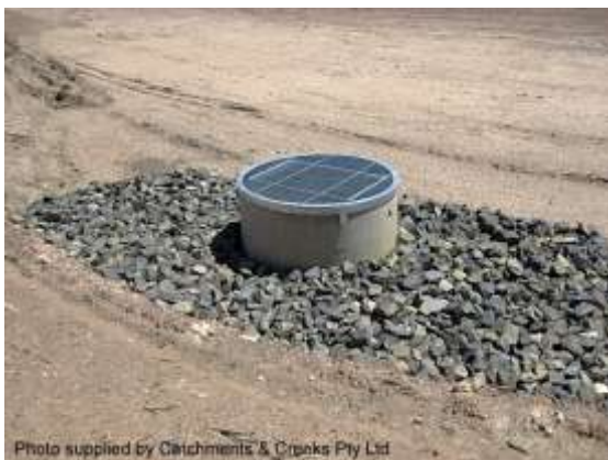
Riser pipe with aggregate filter (Qld)
