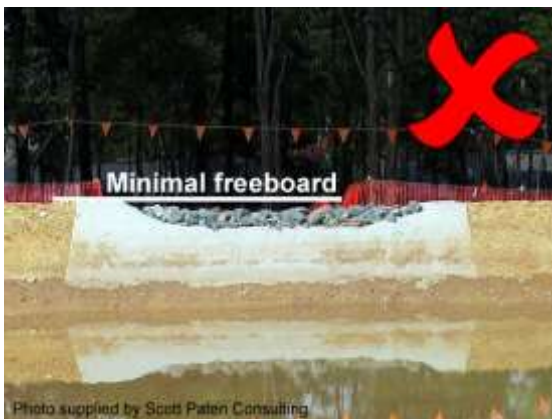
Insufficient freeboard
