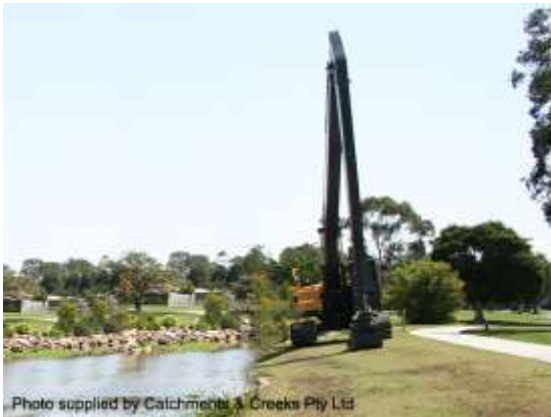
Basin de-silting (Qld)
