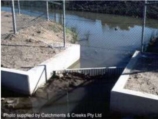
Litter screen at basin inlet (Qld)
