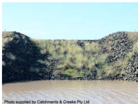
Energy dissipation pond (Qld)
