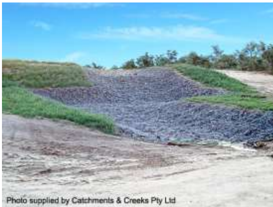
Basin spillway with two 90-degree bends
