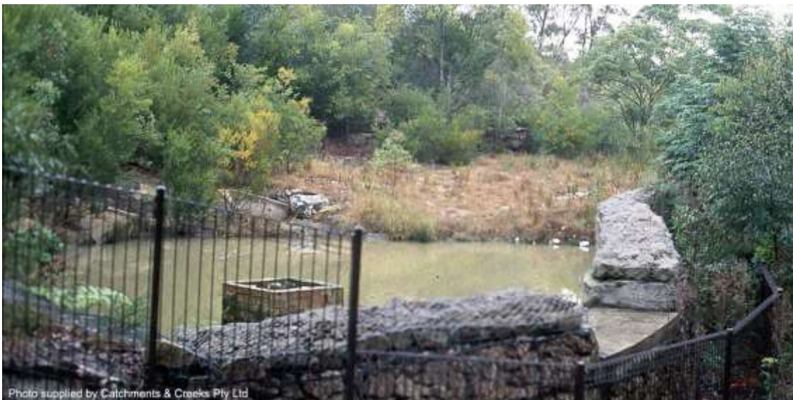
Sediment basin converted to a bio-retention basin (NSW)
