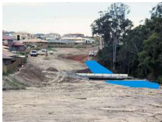
Road construction over stormwater pipe
