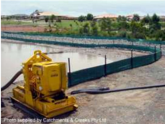
Pumped decant system (Qld)
