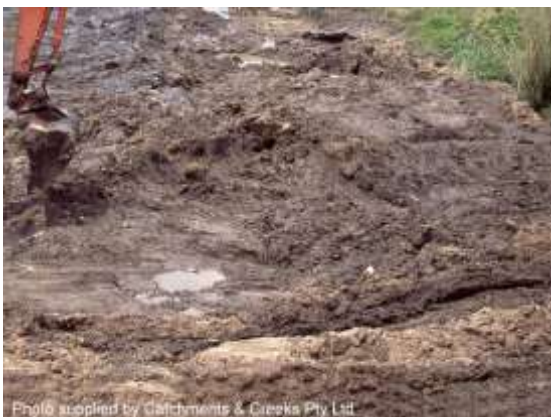
De-watering sediment (Qld)
