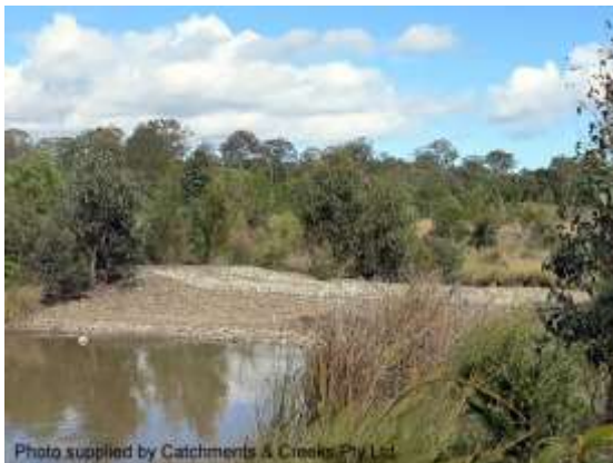
Basin spillway (Qld)
