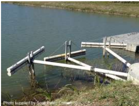
Multiple outlet system (Qld)
