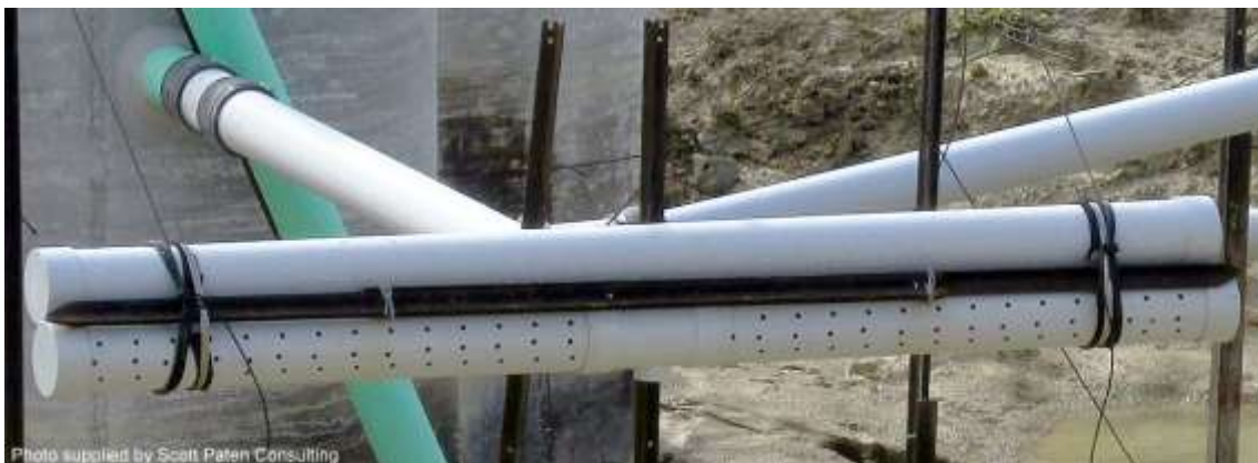
Auckland style floating (T-bar) de-watering system with two steel star-picket weights
