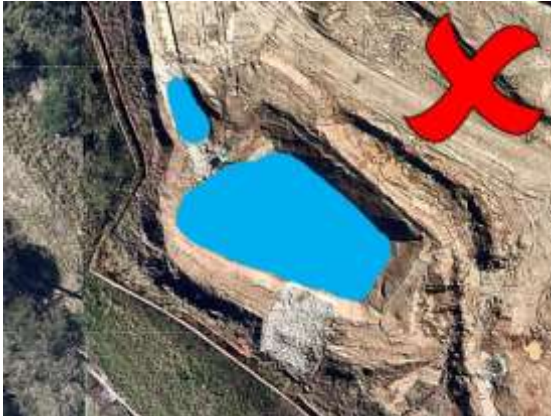
Inadequate forebay width
