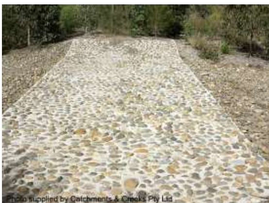
Concrete spillway crest (Qld)
