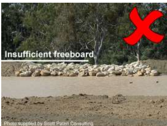
Insufficient freeboard
