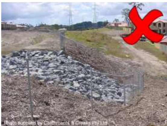
Sediment basin spillway
