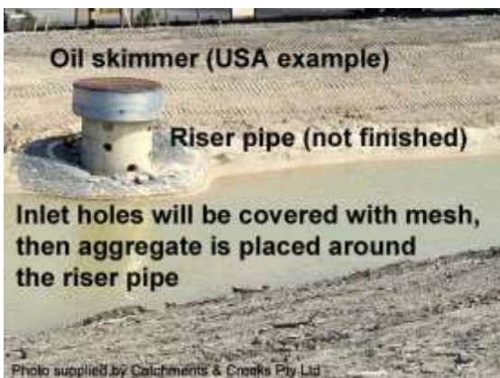
Riser pipe with aggregate filter (USA)
