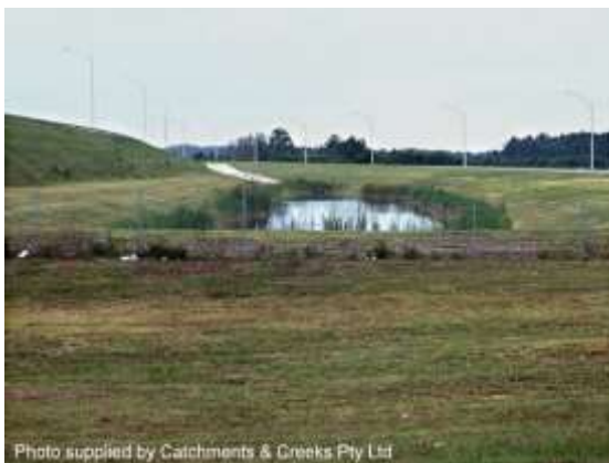
Pollution containment pond (USA)
