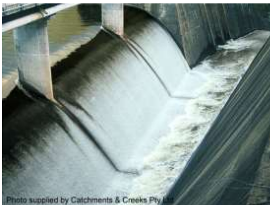
Lateral inflow spilling into a channel (Qld)
