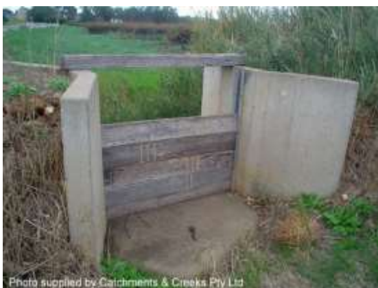
'Stop-board' outlet control system (SA)
