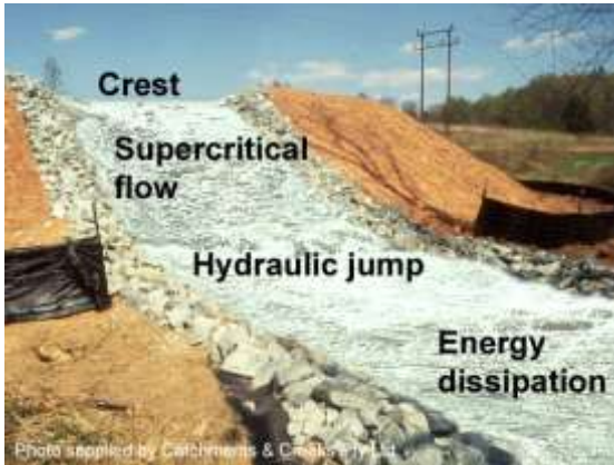
Flow conditions on a basin spillway (USA)
