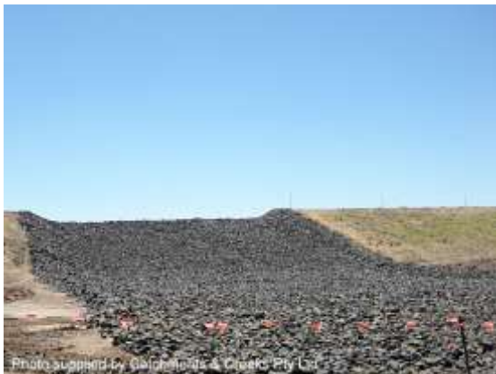
Rock-lined spillway (Qld)
