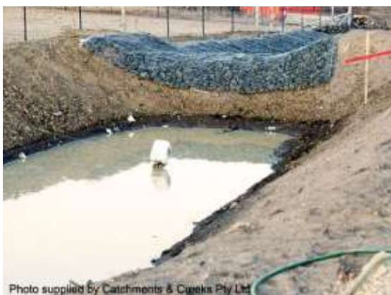
Rock mattress spillway (NSW)
