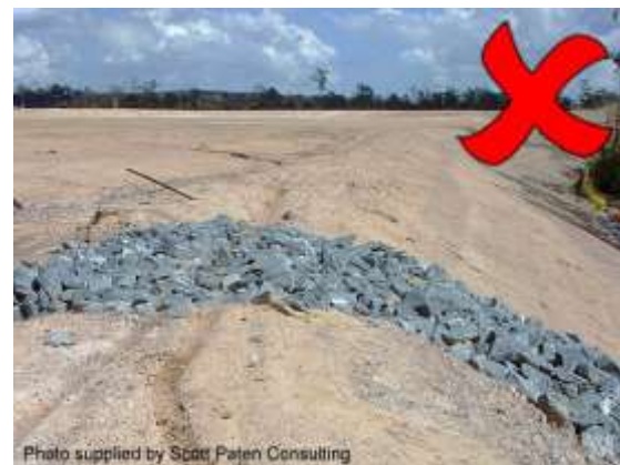
Insufficient freeboard
