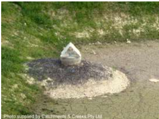
Riser pipe with aggregate filter (NSW)
