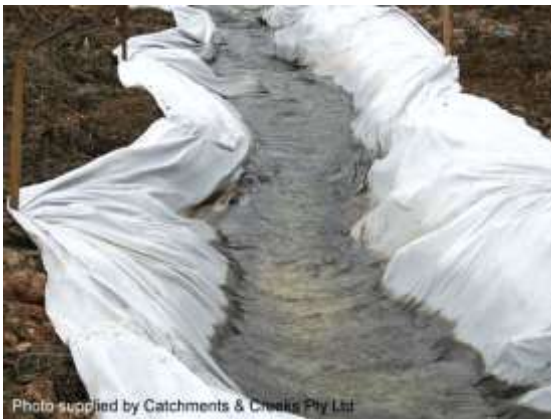
Geotextile-lined drain (NSW)
