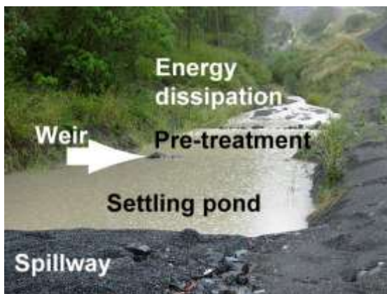
Multi-stage sediment basin (Qld)
