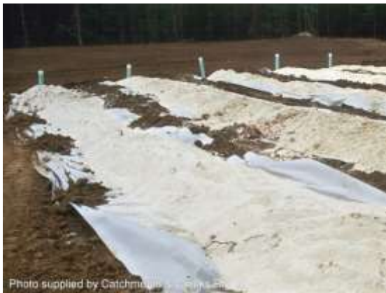
Sand filter under construction (USA)
