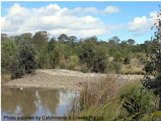
Type B basin overflow spillway
