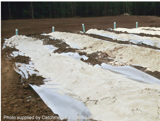
Sand filter under construction
