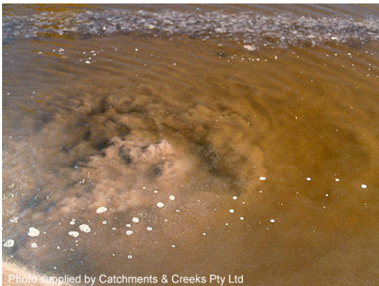
Sludge blanket disturbed by tank inflow
