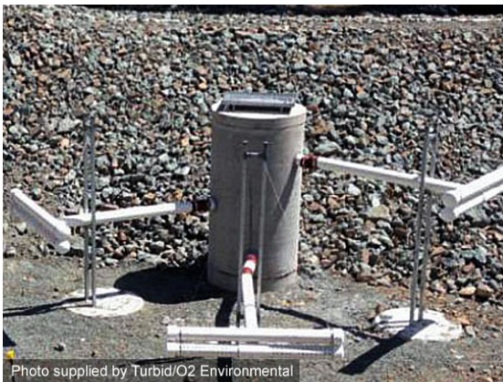
Auckland-type floating decant system
