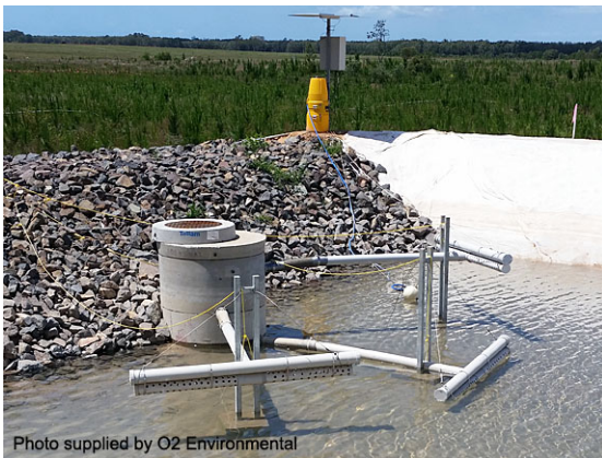
Type A basin decant system
