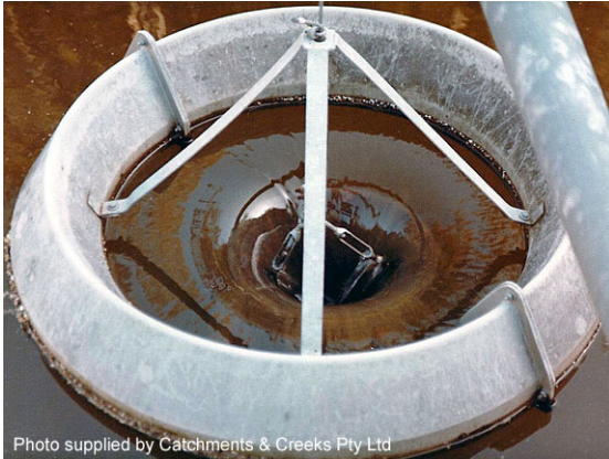
Circular, 'Morning Glory' decant weir
