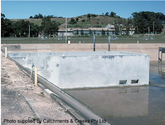
Inflow mixing box (fully drained tank)
