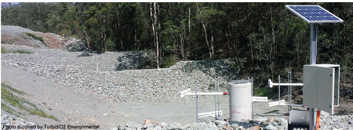
Auckland-type floating decant system (photo sourced from Turbid/O2 Environmental)
