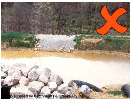
Photo 7 – Spillways must have a well-defined profile to fully contain the flow
