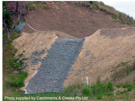
Photo 2 – Rock mattress-lined sediment basin emergency spillway
