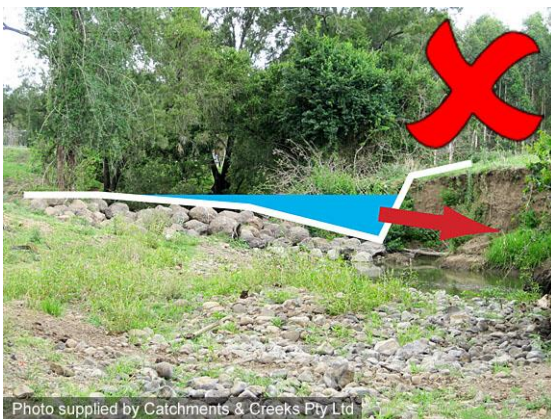
Flows spill unevenly over the rock weir
