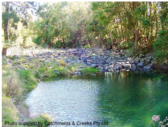
Pool downstream of a rock ramp (NSW)
