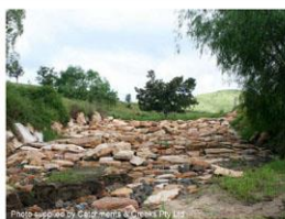
Photo 2 – Rock-lined gully chute
