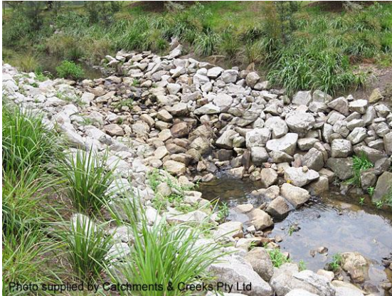
Rocks placed on a steep surface (Qld)
