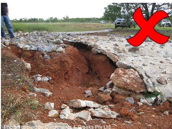
Grouted rock placed on dispersive soil
