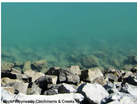
Open voids below permanent waterline
