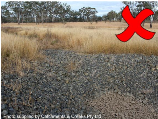
Gully chute formed from small rocks
