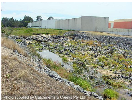
Energy dissipation basin for a chute
