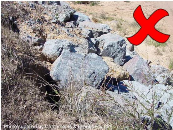
Erosion under rocks on a dispersive soil
