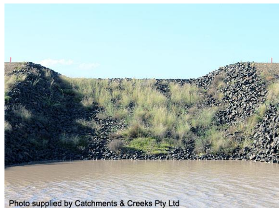
Dam spillway with flat, straight weir crest
