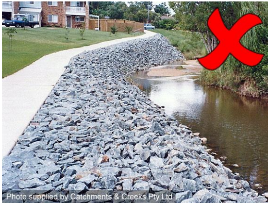
Rock placement without planting
