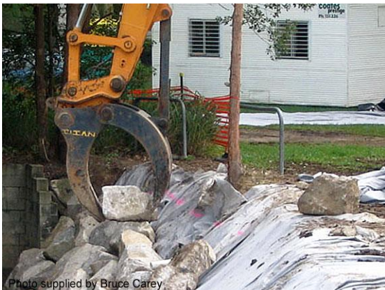
Rocks placed over a geotextile filter (Qld)
