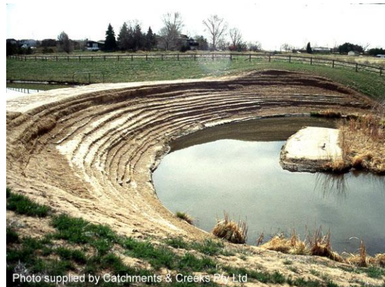
Grade control structure with curved crest
