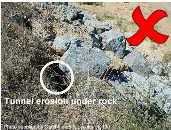
Tunnel erosion under rocks
