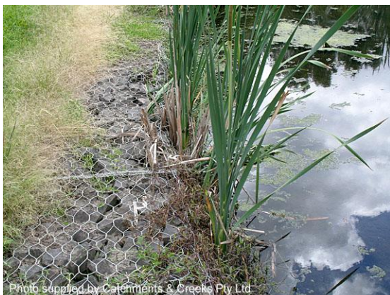
Gabion-lined waterway bank (NSW)
