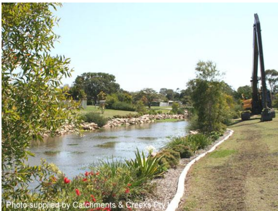
Waterway maintenance (Qld)
