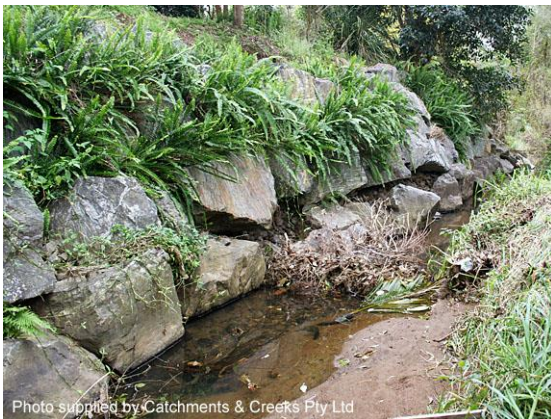
Stacked boulder wall (Qld)
