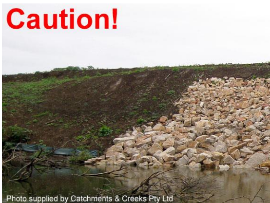
Rock downstream of a 'smooth' bank
