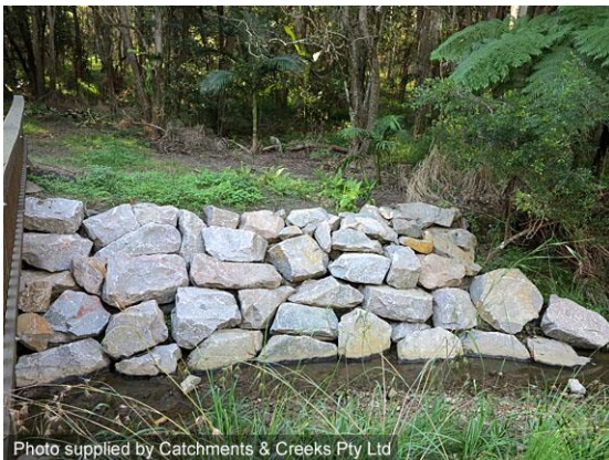
Stacked boulder wall adjacent a footbridge
