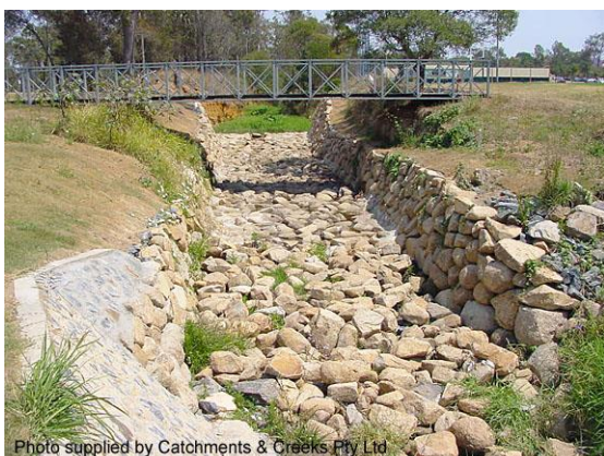
Grouted rock gully chute (Qld)
