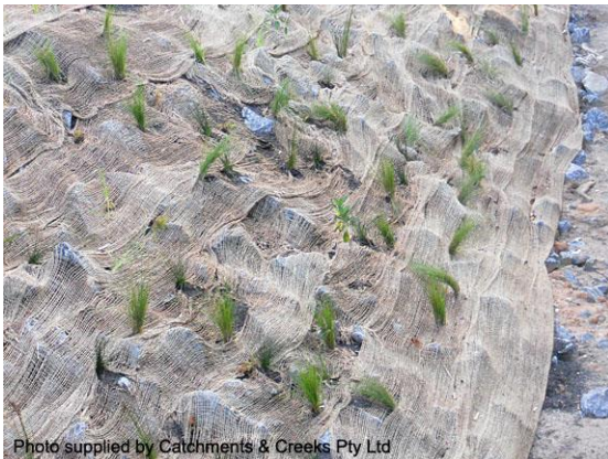
Planted rock covered with jute mesh
