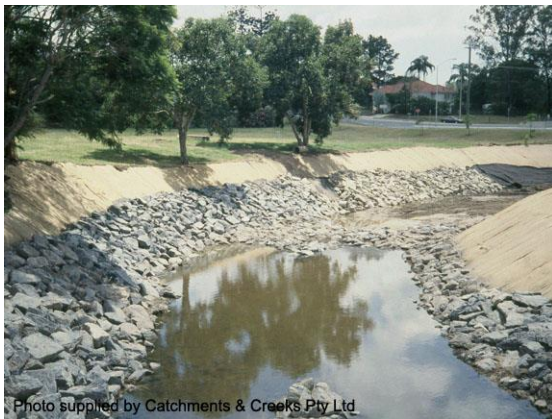
Rock stabilisation on channel bend (Qld)
