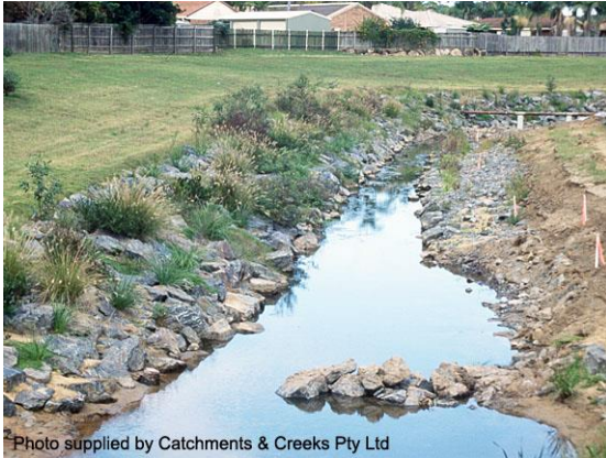
Vegetated rock stabilisation works
