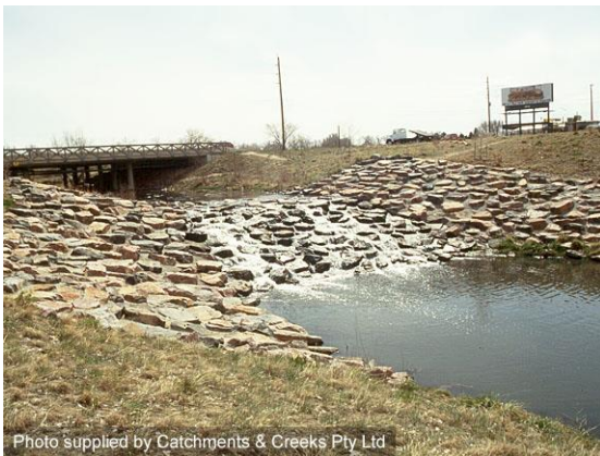
Curved weir crest on a drop structure
