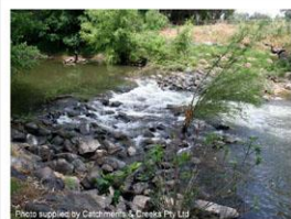
Photo 1 – Rock-lined waterway chute
