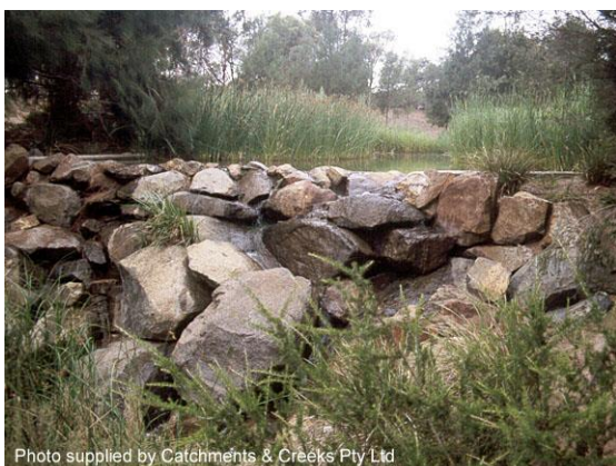
Grouted rock wetland outflow weir (Qld)
