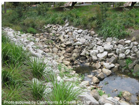
Pool-riffle in a narrow channel (Qld)
