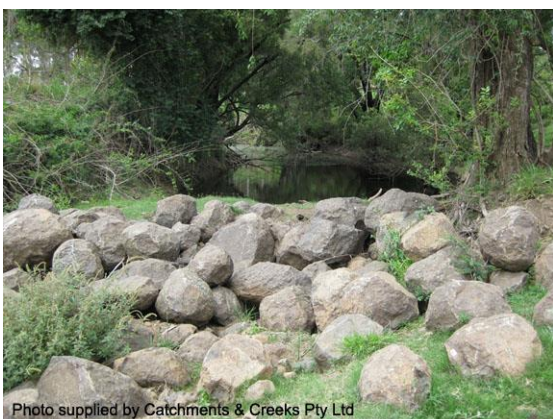
Gully chute formed from round rocks
