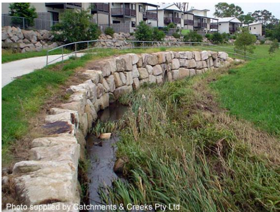
Stacked boulder wall (Qld)
