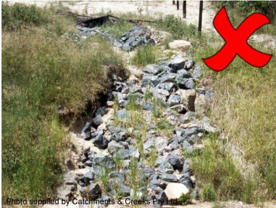
Batter chute placed on a dispersive soil
