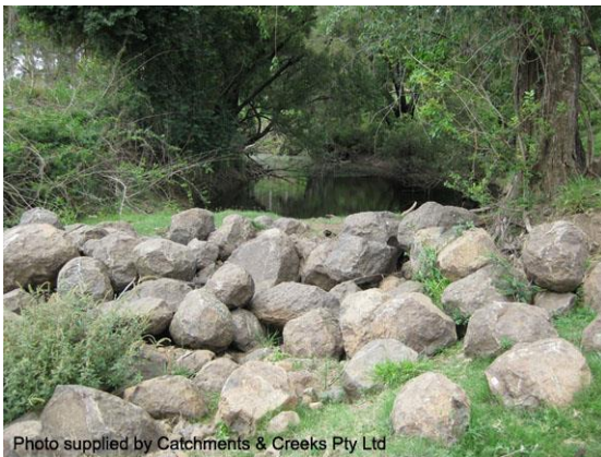
Rock weir made from round natural stone
