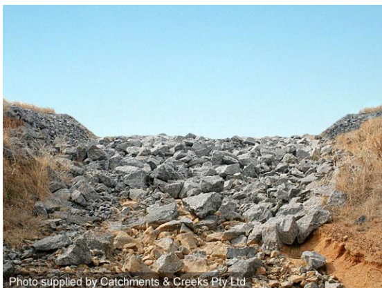
Looking upstream to crest of rock chute
