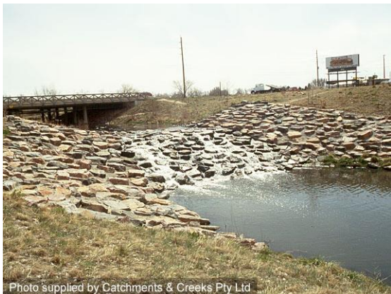
Grouted rock drop structure (USA)
