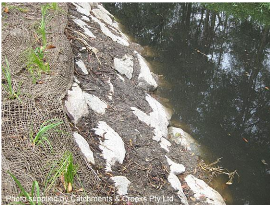
Voids filled with soil ready for planting
