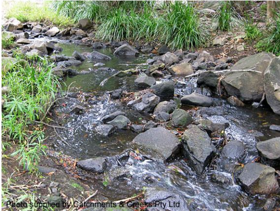
Constructed riffle in a clay-based creek
