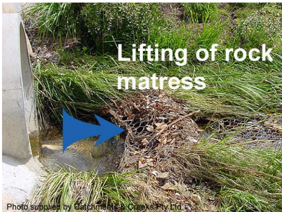
Lifting of rock mattress (Qld)
