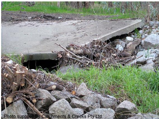
Rock displaced at end of concrete channel
