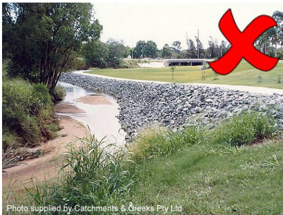
Rock placement without planting
