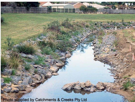
Vegetated rock stabilisation (Qld)
