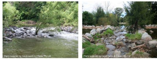
Photo 1 – Constructed riffle
