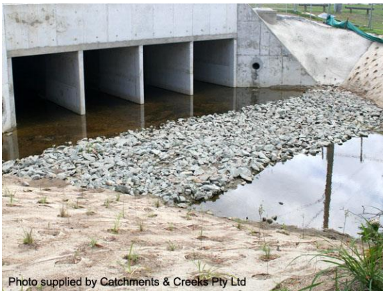
Culvert outlet scour control (Qld)
