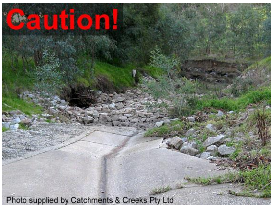
Rock downstream of a concrete drain
