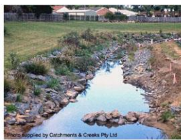
Photo 2 – Rock stabilisation with plants introduced at time of rock placement
