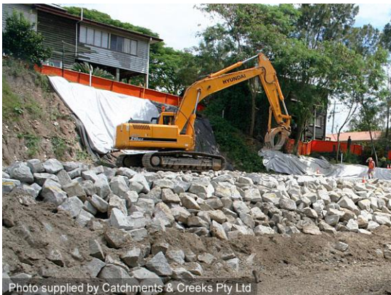
Rock placement over filter cloth (Qld)
