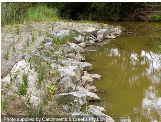
Vegetated rock stabilisation of bank (Qld)
