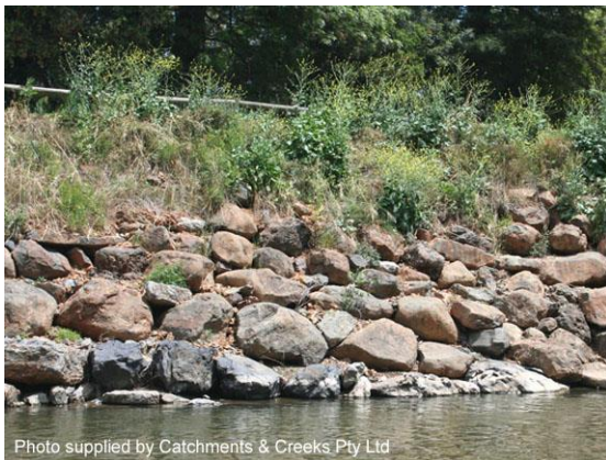
Partial vegetated bank stabilisation (NSW)
