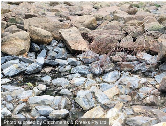
Rock filter layer (blue) under surface rock
