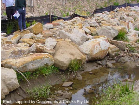
Larger rocks forming toe protection (NSW)
