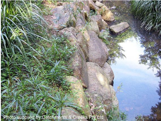
Stacked boulder wall (Qld)
