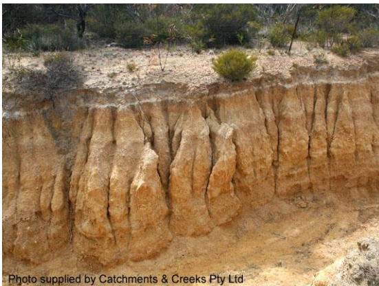
Fluting erosion in a dispersive soil (SA)
