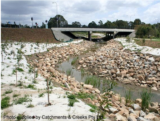
Rock-lined bank stabilisation (Qld)
