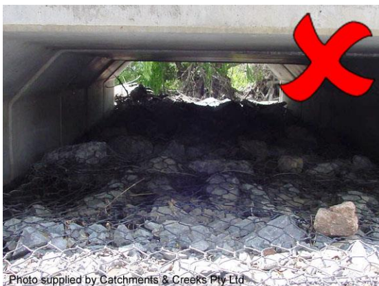
Rock mattress placed on culvert bed
