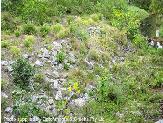
Planted rock-stabilised creek bank (Qld)
