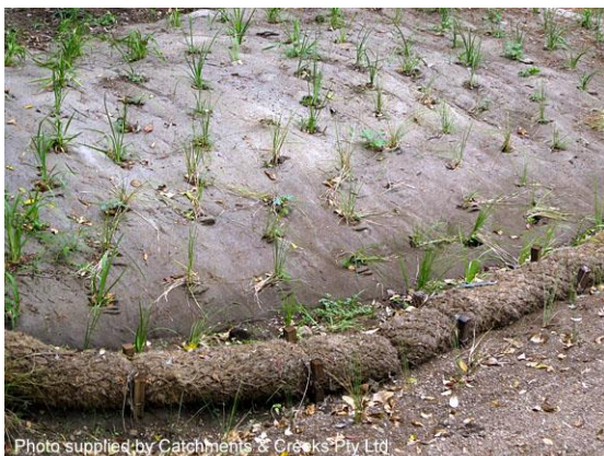
Coir 'geo-log' temporary toe protection
