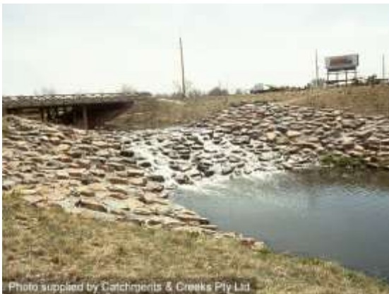
Curved weir crest on a drop structure
