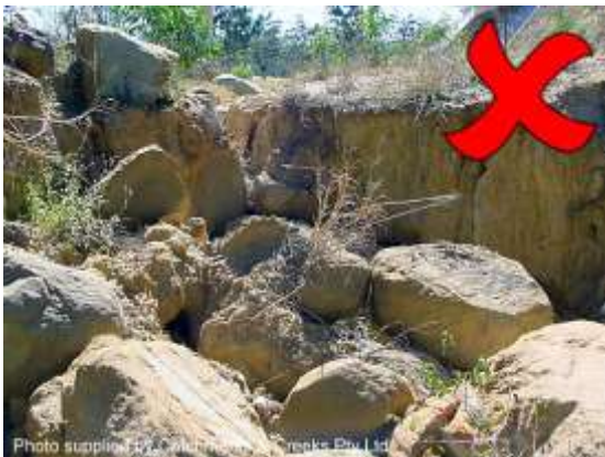
Gully chute formed on a dispersive soil
