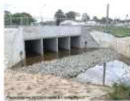
Photo 2 – Rock pad outlet structure at end of a multi-cell box culvert.
