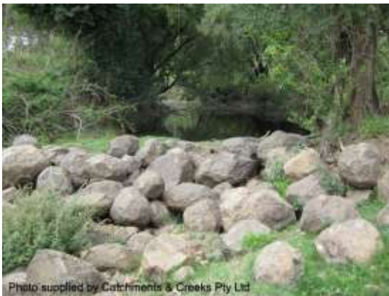
Rock weir made from round natural stone
