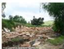
Photo 2 – Rock-lined gully chute
