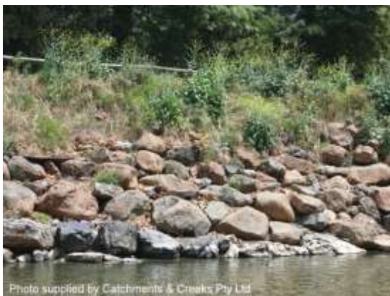
Partial vegetated bank stabilisation (NSW)
