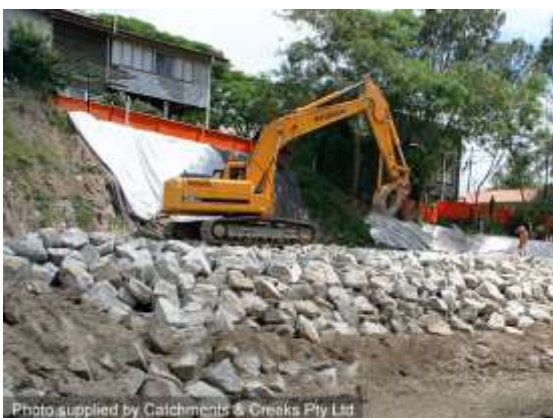
Rock placement over filter cloth (Qld)
