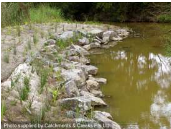
Vegetated rock stabilisation of bank (Qld)
