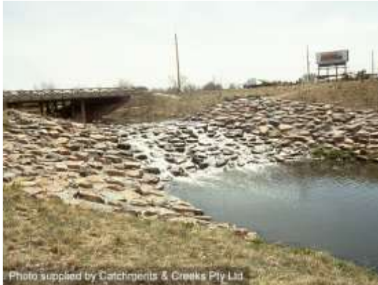
Grouted rock drop structure (USA)
