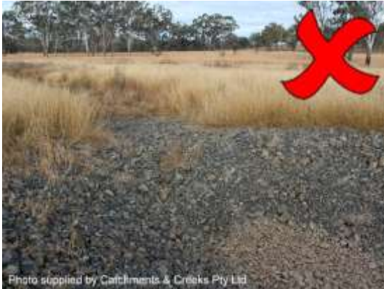
Gully chute formed from small rocks
