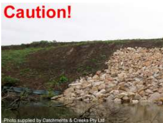
Photo supplied by Catchments & Creeks Pty Ltd Rock downstream of a 'smooth' bank
