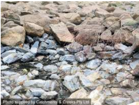
Rock filter layer (blue) under surface rock
