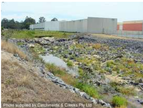
Energy dissipation basin for a chute
