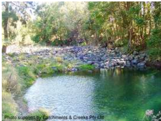
Pool downstream of a rock ramp (NSW)
