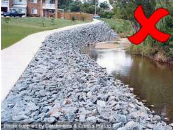
Rock placement without planting
