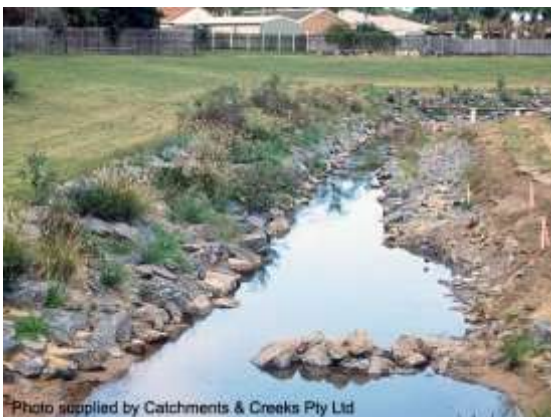
Vegetated rock stabilisation (Qld)
