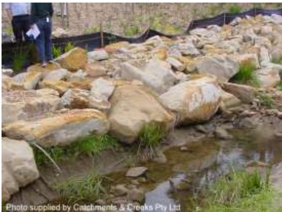
Larger rocks forming toe protection (NSW)
