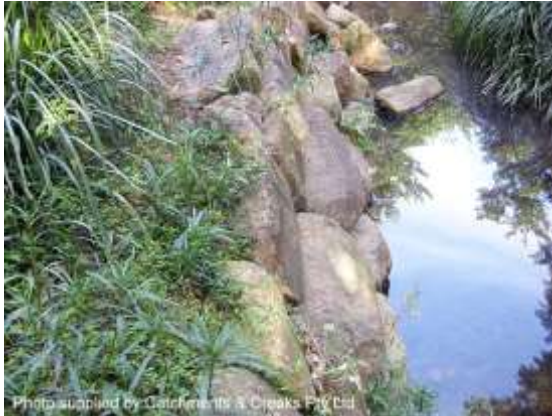
Stacked boulder wall (Qld)
