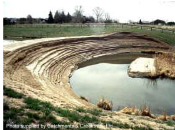
Grade control structure with curved crest
