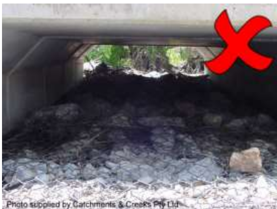
Rock mattress placed on culvert bed
