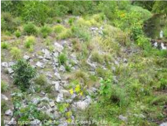
Planted rock-stabilised creek bank (Qld)
