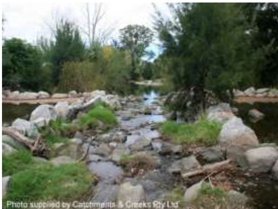
Looking 'down' a rock ramp fishway (NSW)
