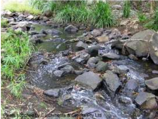
Constructed riffle in a clay-based creek
