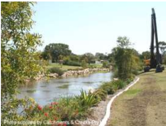
Waterway maintenance (Qld)
