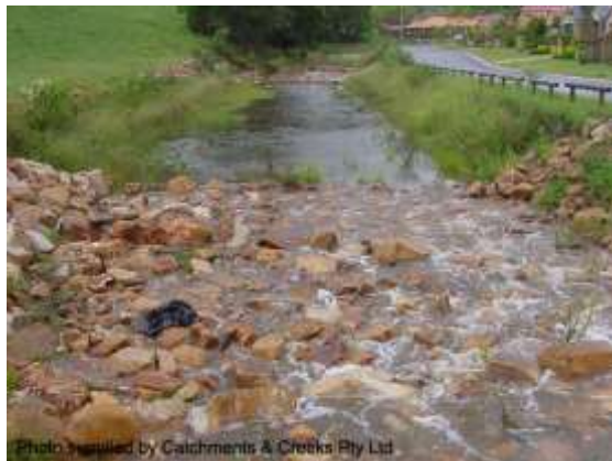
Constructed riffle (Qld)
