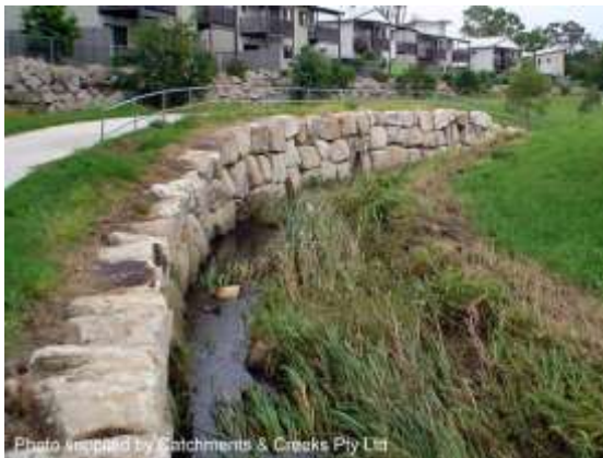
Stacked boulder wall (Qld)
