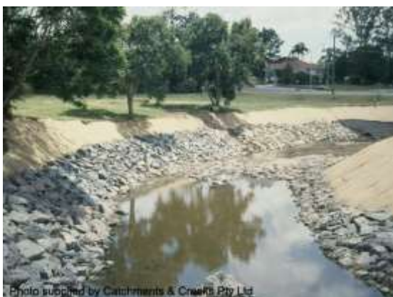
Rock stabilisation on channel bend (Qld)
