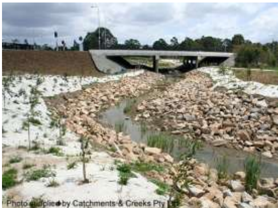
Rock-lined bank stabilisation (Qld)
