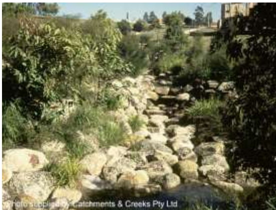
Grouted rock gully chute (Qld)
