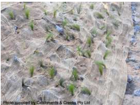
Planted rock covered with jute mesh
