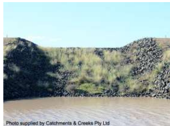
Dam spillway with flat, straight weir crest
