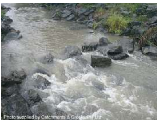
Rock sitting high with exposed edges
