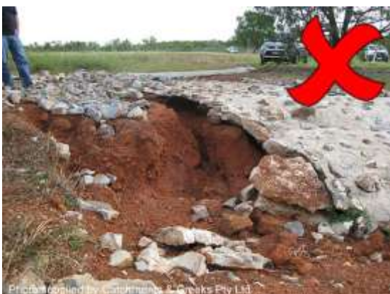
Grouted rock placed on dispersive soil
