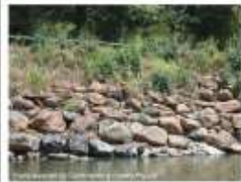
Photo 1 – Lower bank rock stabilisation with voids filled with small rocks
