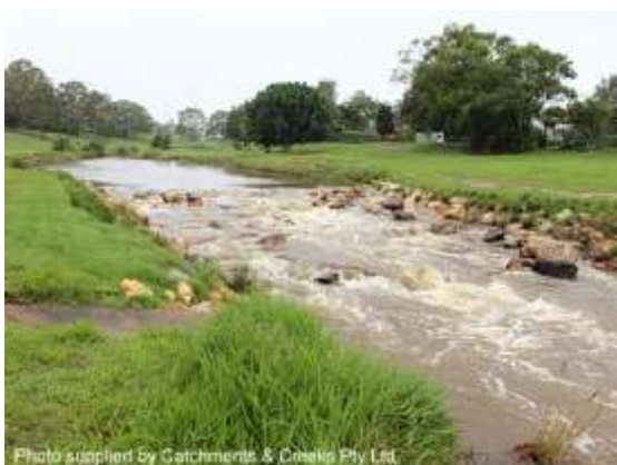
Constructed waterway riffle (Qld)
