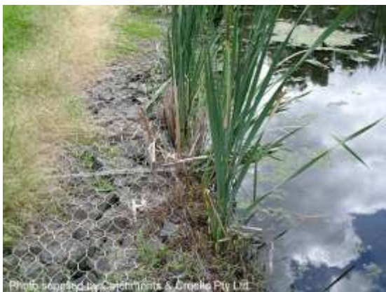
Gabion-lined waterway bank (NSW)
