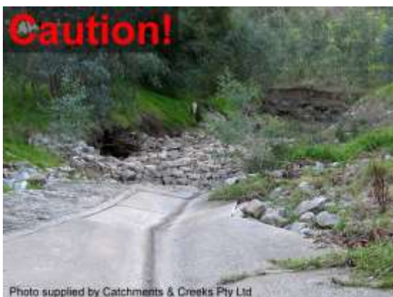
Photo supplied by Catchments & Creeks Pty Ltd Rock downstream of a concrete drain
