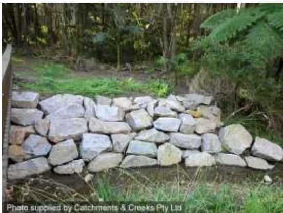
Stacked boulder wall adjacent a footbridge
