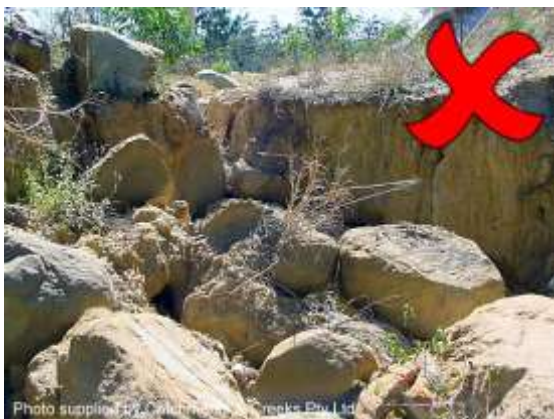
Collapsed dispersive soil bank
