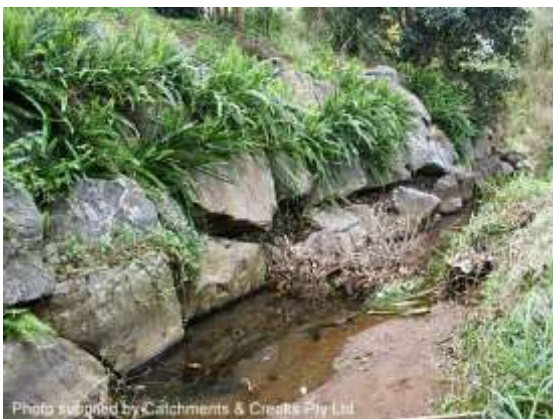
Stacked boulder wall (Qld)
