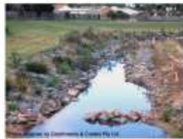
Photo 2 – Rock stabilisation with plants introduced at time of rock placement
