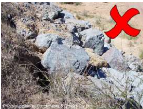
Erosion under rocks on a dispersive soil
