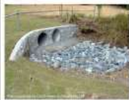
Photo 1 – Rock pad outlet structure at end of a dual stormwater pipe outlet.
