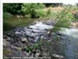
Photo 1 – Rock-lined waterway chute
