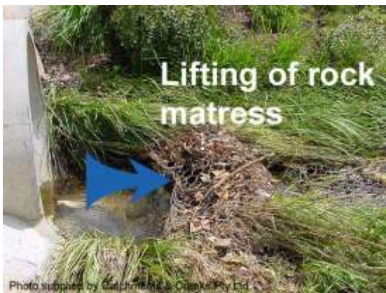
Lifting of rock mattress (Qld)
