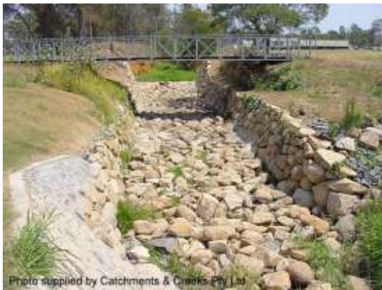
Grouted rock gully chute (Qld)
