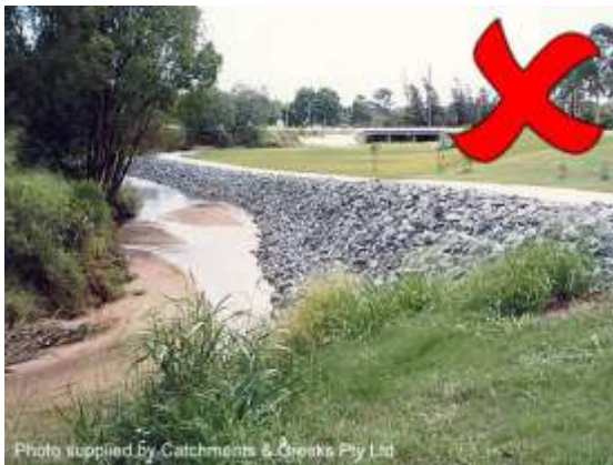
Rock placement without planting
