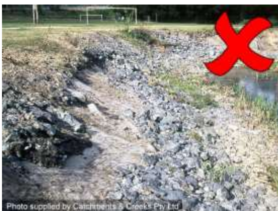
Rocks displaced down filter cloth
