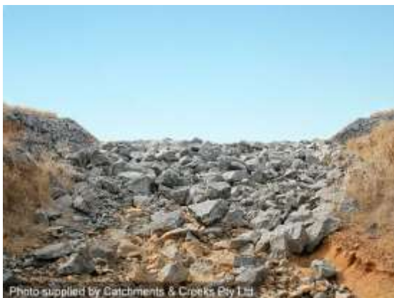
Looking upstream to crest of rock chute
