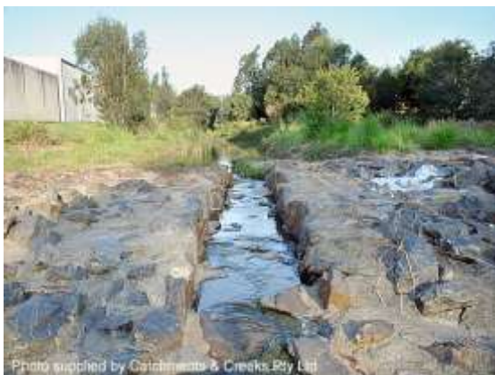
Low-flow channel set in grouted rock
