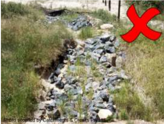
Batter chute placed on a dispersive soil
