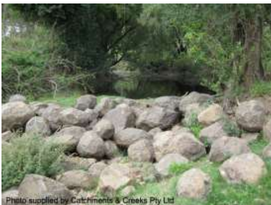
Gully chute formed from round rocks
