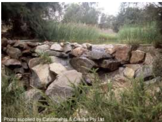
Grouted rock wetland outflow weir (Qld)
