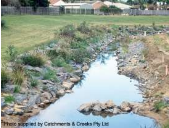
Vegetated rock stabilisation works
