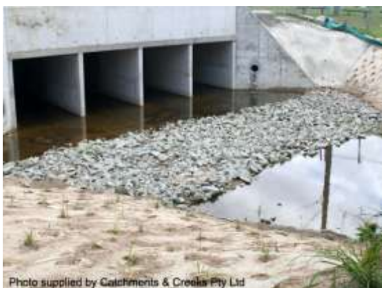
Culvert outlet scour control (Qld)
