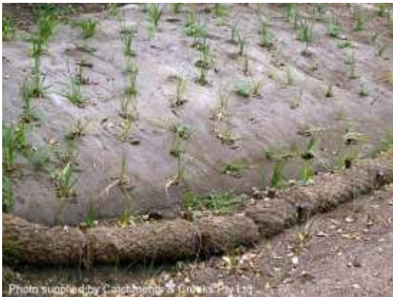
Coir 'geo-log' temporary toe protection
