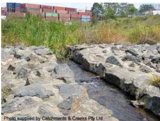
Low-flow channel set in grouted rock
