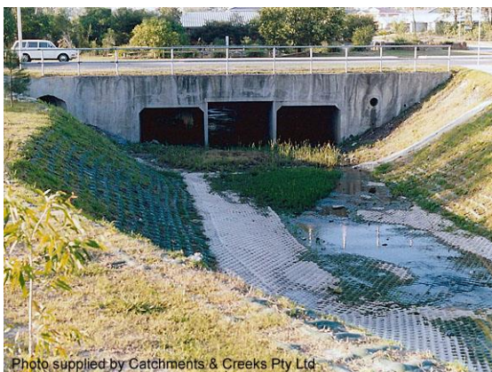
Excessive 'hardening' of the waterway
