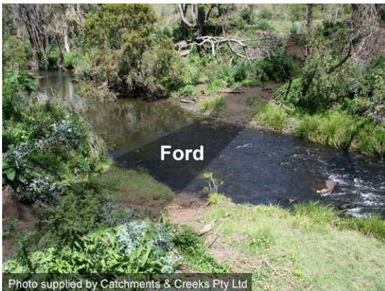
Ford crossing over a rock riffle (Qld)
