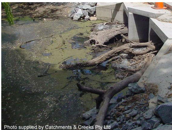
Flood debris caught on roughness units
