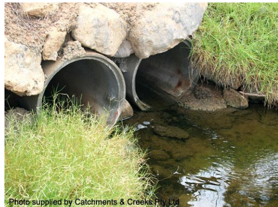
Twin pipe culvert
