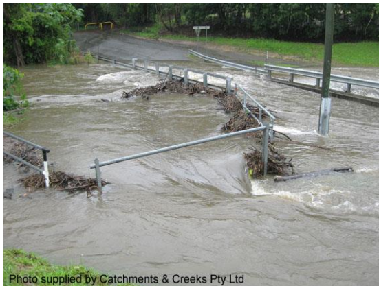
Drowned-out culvert structure (Qld)
