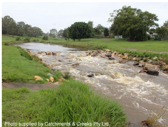
Constructed rock riffle (Qld)
