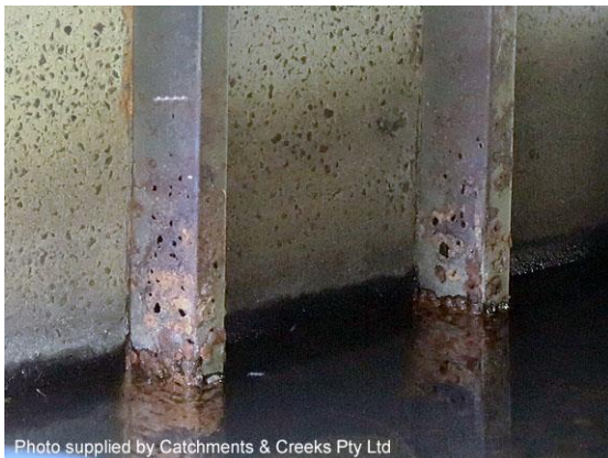
Rusted steel baffles 13 years later
