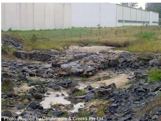
Damaged rock chute
