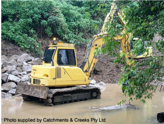
Placement of scour protection (Qld)
