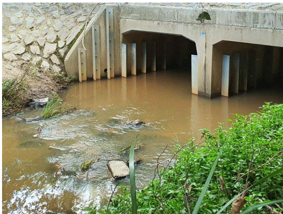
Box culvert with baffles (Qld)
