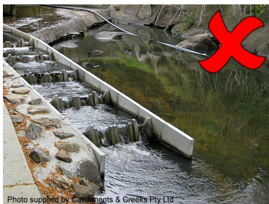
Poor location of a fishway outlet
