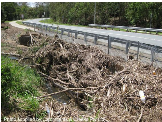
Full debris blockage of culvert entrance
