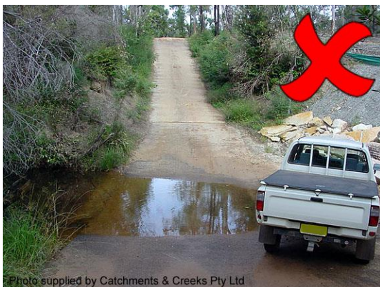
Concrete crossing of sand -based creek
