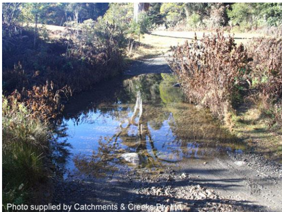
Ford crossing of a gravel -based creek
