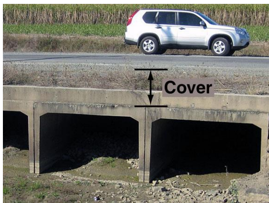
Road base cover over a box culvert (Qld)
