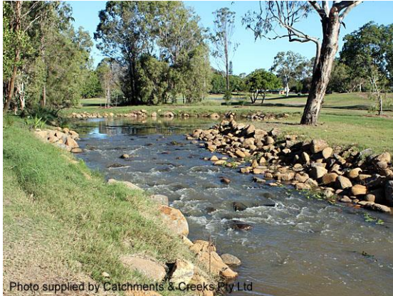
Constructed rock ramp/riffle/chute (Qld)
