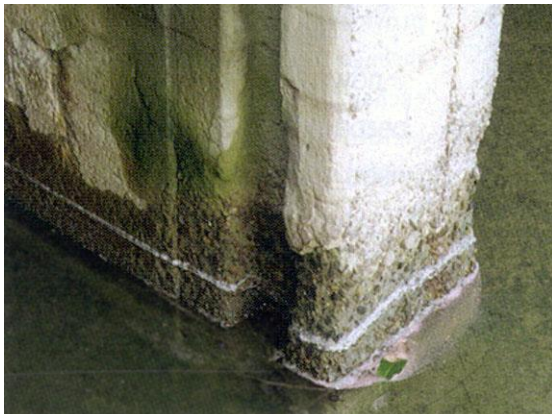
Damage to culvert by acidic waters
