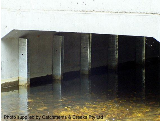
Recently-installed galvanised steel baffles
