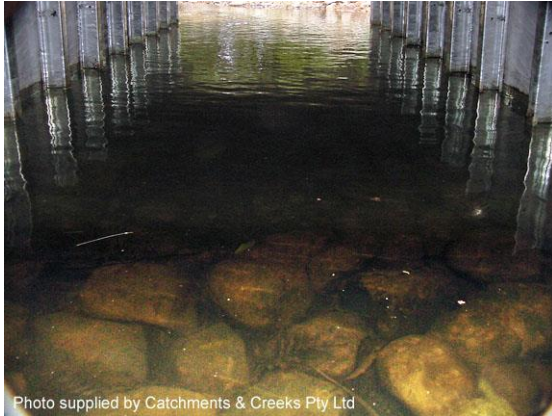
Introduced bed roughness (NSW)
