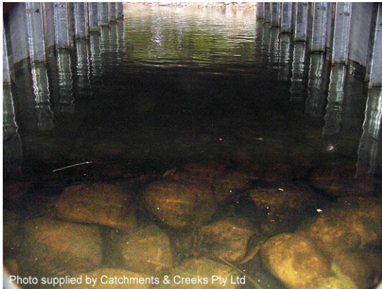
Artificial culvert-bed roughness (NSW)
