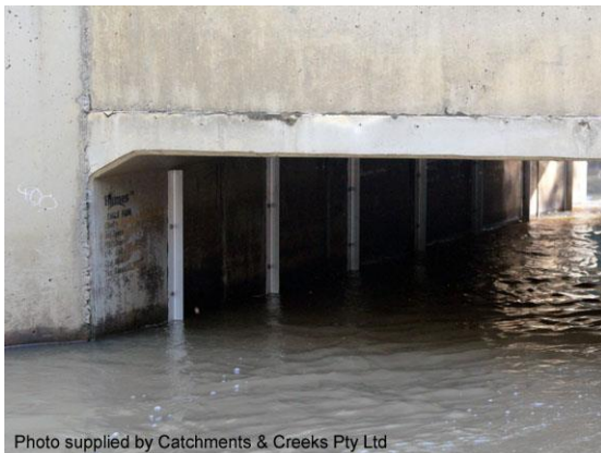
Box culvert with experimental baffles
