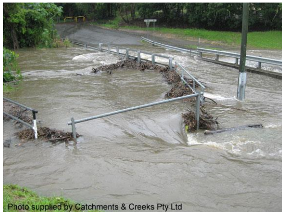
Floodwater overtopping a culvert (Qld)
