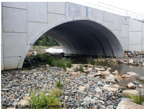
Low-flow channel under an arch (NSW)
