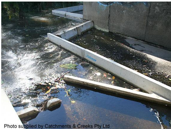
Baffles used to direct flows in the fishway
