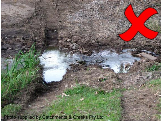
Ford crossing of a clay -based creek
