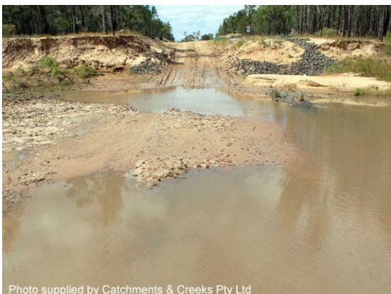
Ford crossing of a sand-based creek (Qld)
