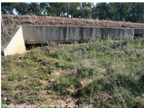
Near-full sediment blockage of a culvert
