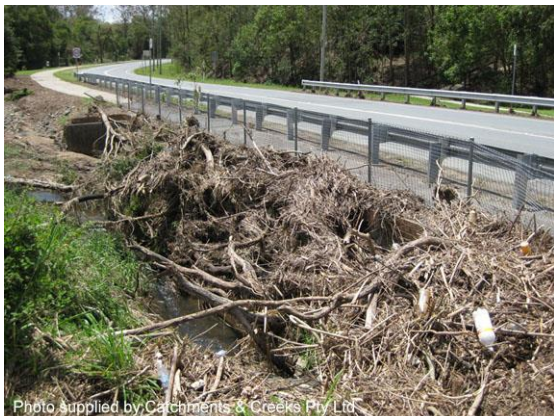
Full debris blockage of a culvert (Qld)
