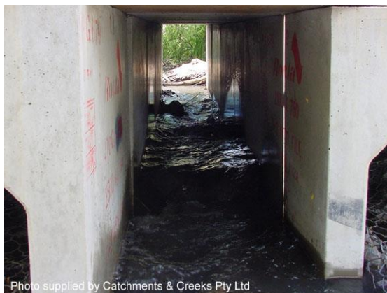
Low flows directed into central cell
