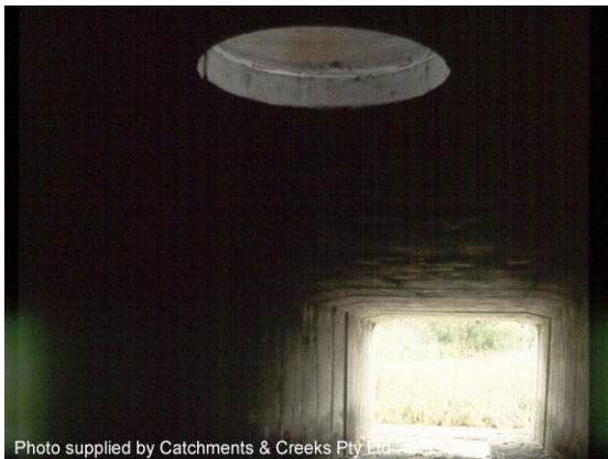
Skylight placed in a box culvert (Qld)
