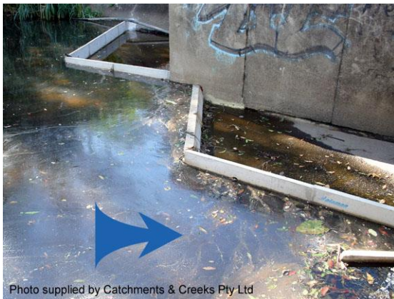
Controlling the passage of low flows
