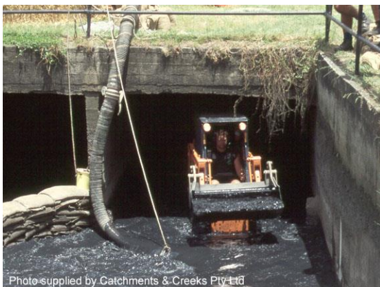
Culvert de-silting
