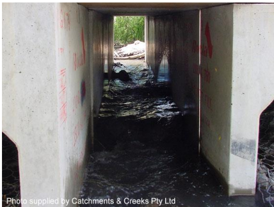
Low flows directed into central cell
