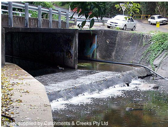
Potential fish barrier at culvert exit
