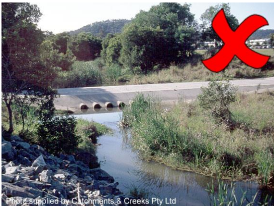
Causeway crossing of a clay-based creek
