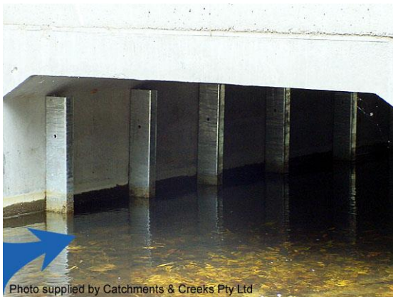
Sidewall baffles (NSW)
