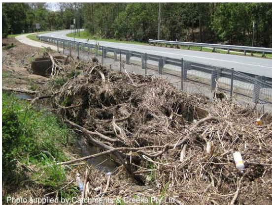
Flood debris blockage of a culvert (Qld)
