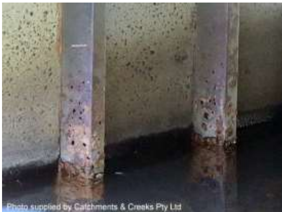
Rusted steel baffles 13 years later
