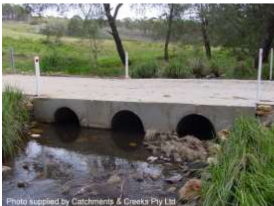
Pipe culvert on a rural property driveway
