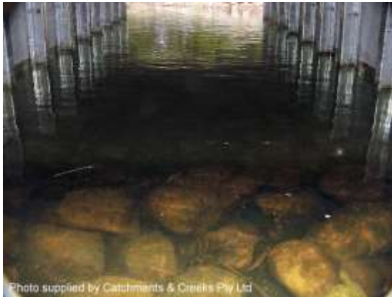
Artificial culvert-bed roughness (NSW)
