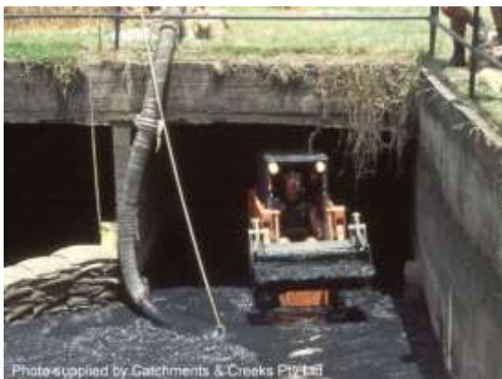
Culvert de-silting
