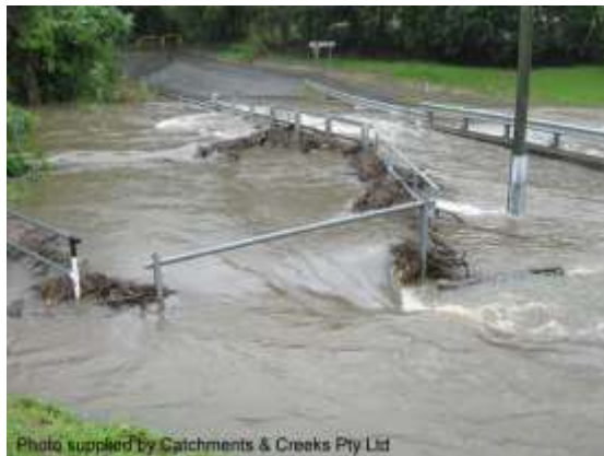
Drowned-out culvert structure (Q1d)
