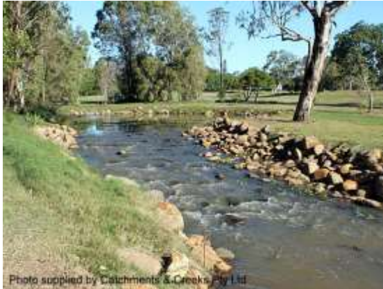
Constructed rock ramp/riffle/chute (Qld)
