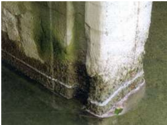
Damage to culvert by acidic waters
