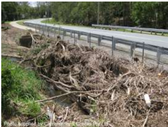
Flood debris blockage of a culvert (Qld)
