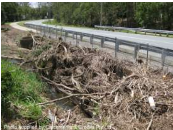
Full debris blockage of culvert entrance
