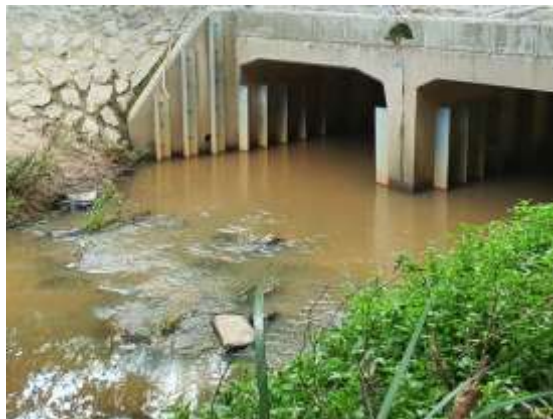
Box culvert with baffles (Qld)
