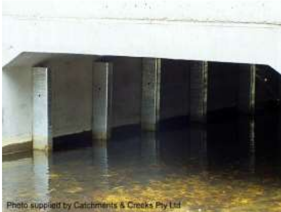
Recently-installed galvanised steel baffles
