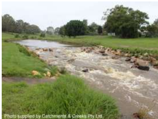
Constructed rock riffle (Qld)
