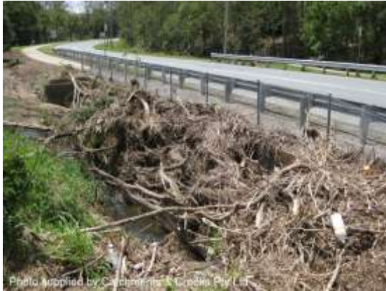
Full debris blockage of a culvert (Qld)
