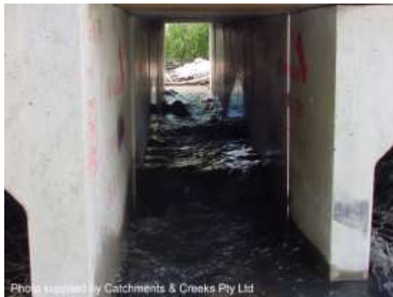
Low flows directed into central cell
