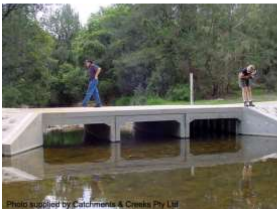
Recessed culvert (NSW)
