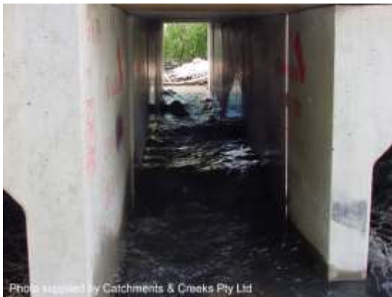
Low flows directed into central cell
