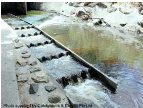
Mechanical fishway outside a culvert
