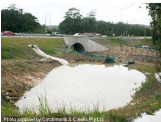
Sediment basins linked to new road works
