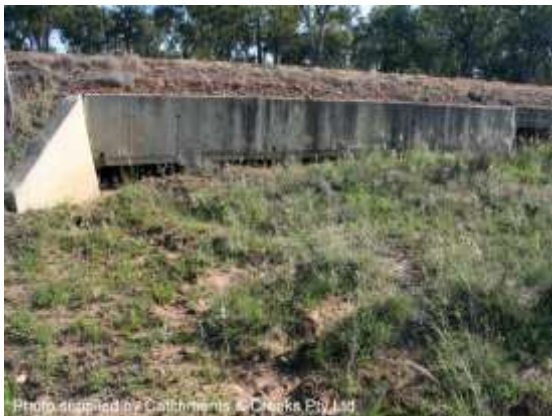
Near-full sediment blockage of a culvert
