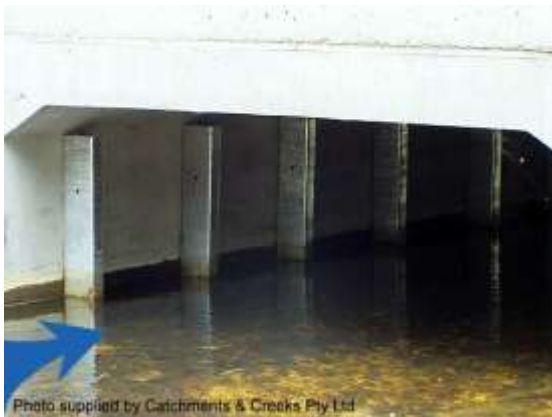
Sidewall baffles (NSW)
