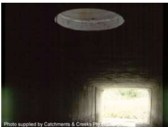
Skylight in the roof of a box culvert (Qld)
