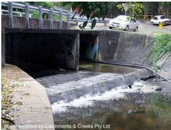
Potential fish barrier at culvert exit
