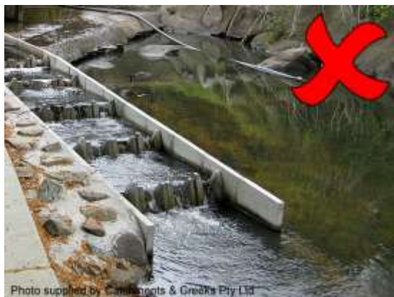
Poor location of a fishway outlet
