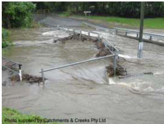
Floodwater overtopping a culvert (Qld)
