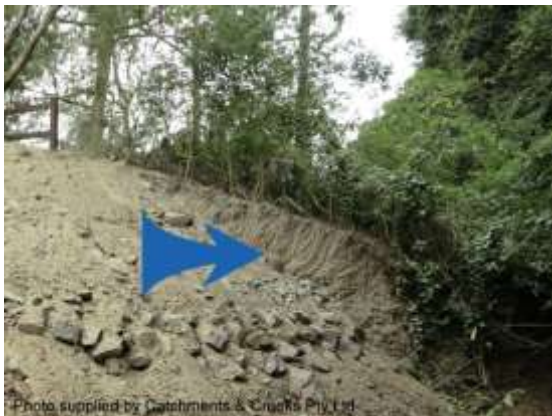
Discontinuity in bank profile post works
