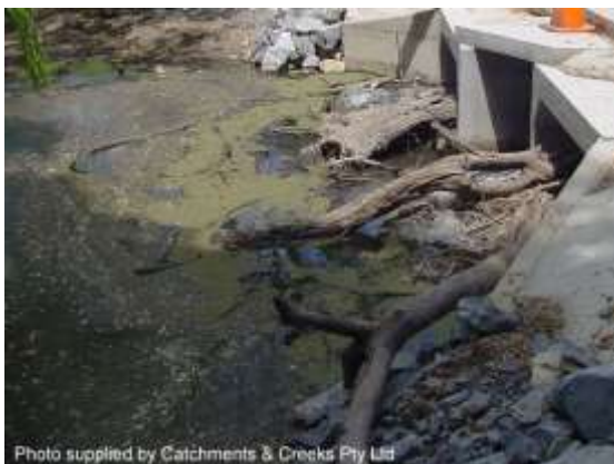
Flood debris caught on roughness units
