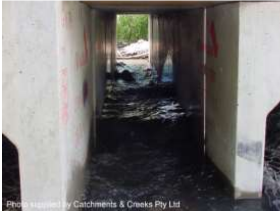
Dedicated low-flow fishway in a culvert
