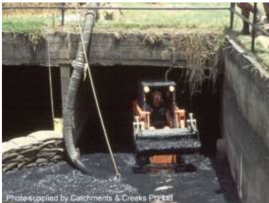
De-silting operation (Qld)
