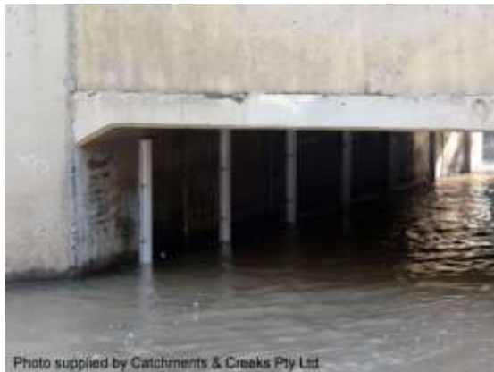
Box culvert with experimental baffles
