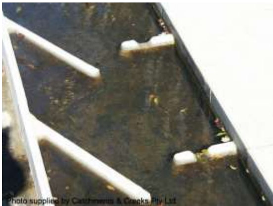
Mechanical fishway in a culvert (Qld)
