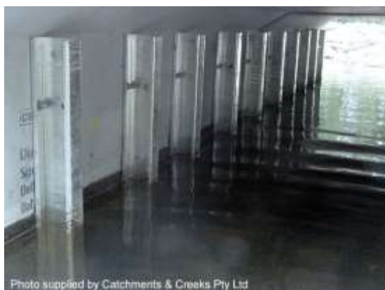
Sidewall baffles (NSW)
