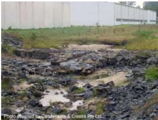
Damaged rock chute
