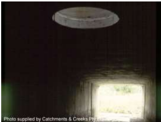
Skylight placed in a box culvert (Qld)
