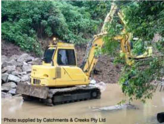
Placement of scour protection (Qld)
