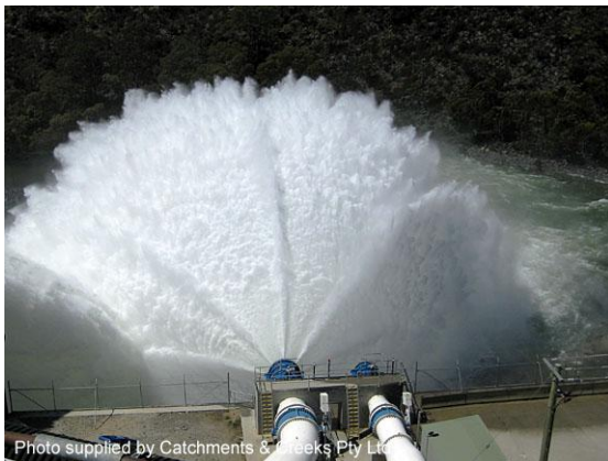
Water supply dam outlet structure
