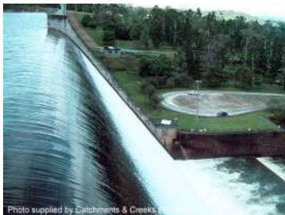
Critical flow at the crest of a dam spillway
