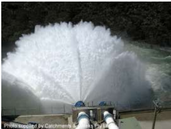
Water supply dam outlet structure
