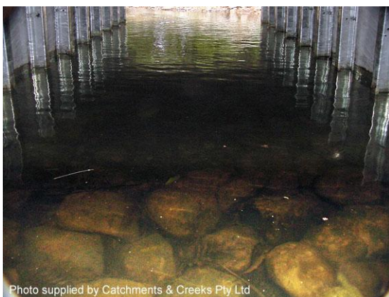
Placement of loose rock (NSW)
