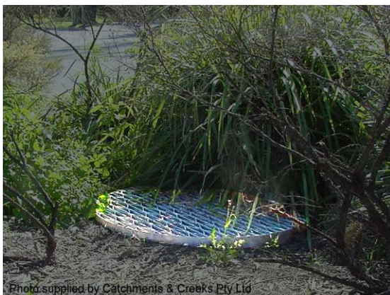
Skylights placed within the median (Qld)
