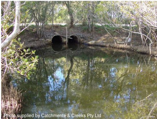
Outlet scour hole (pool) on a tidal culvert
