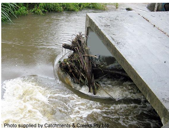
Example of a low level of debris blockage
