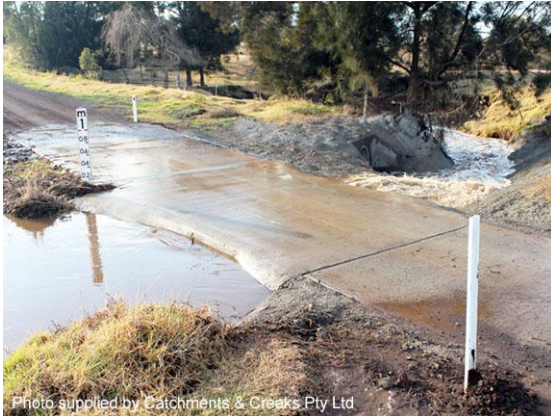
Inlet control (looking downstream, Qld)
