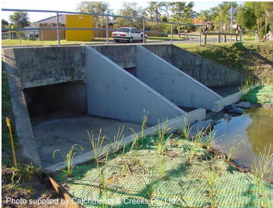
Culvert with sediment control weirs (Q1d)
