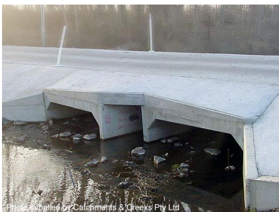
Gravel bed within a culvert (NSW)
