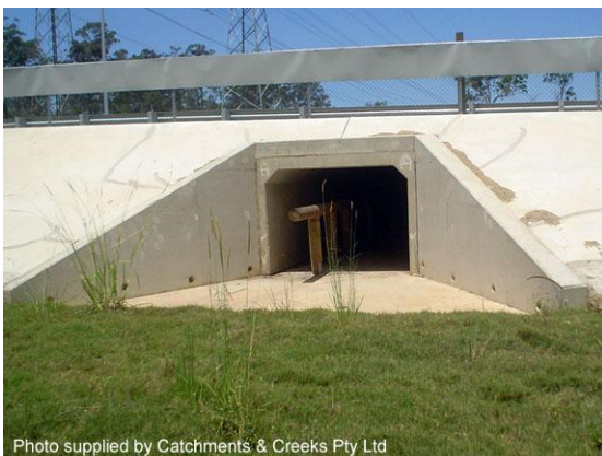
Floodplain culvert (Qld)
