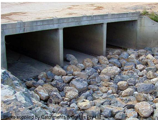
Culvert outlet with rock pad (NSW)
