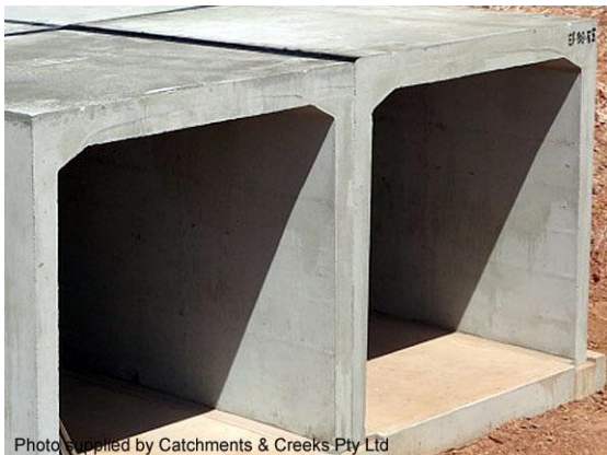
Smooth concrete surface (NT)
