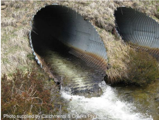
Culvert discharge with very low tailwater
