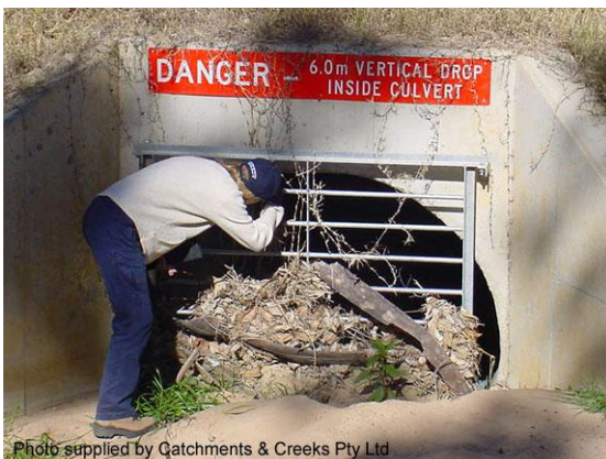
Inspection of an inlet safety screen (Qld)
