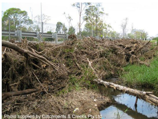
Culvert fully blocked by flood debris (Qld)
