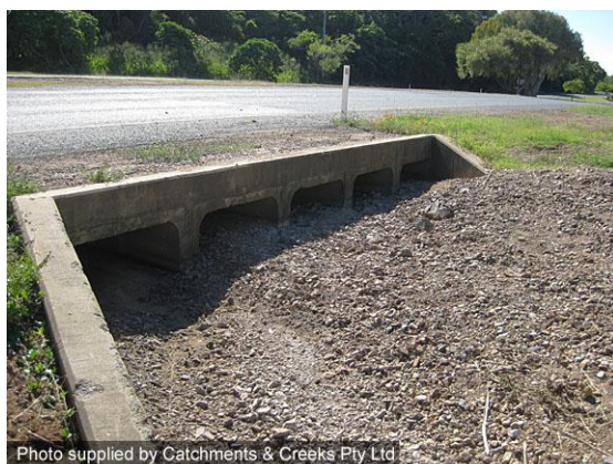
Sediment blockage (Qld)
