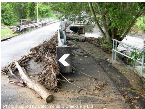
Debris blockage of traffic barrier (Qld)
