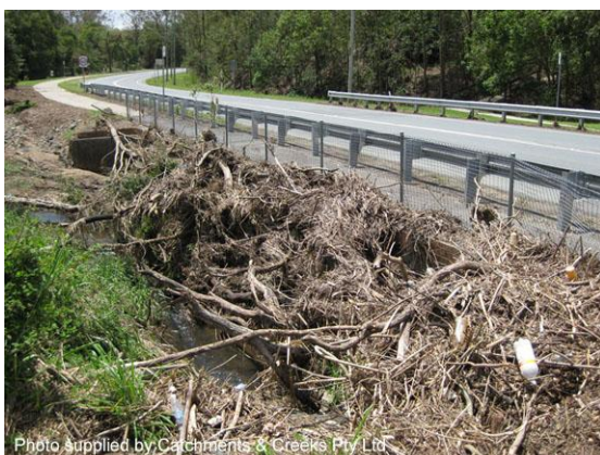
Severe debris blockage of a culvert (Qld)
