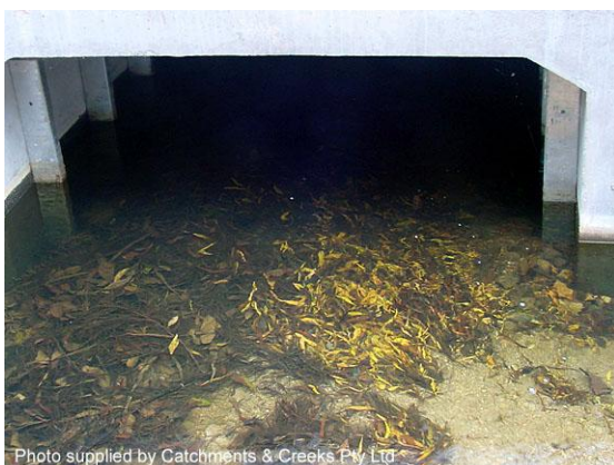
Natural deposition of bed sand (NSW)
