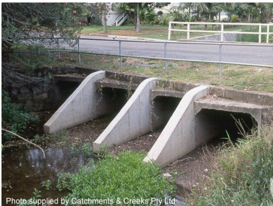
Debris deflection walls, 1995 (Qld)
