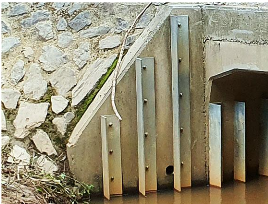
Baffles placed on a culvert wingwall (Qld)
