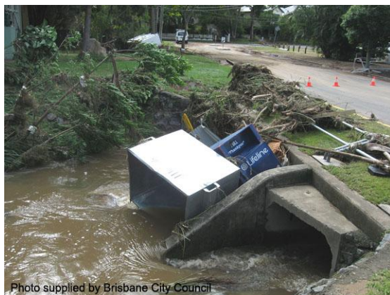
Blockage by industrial waste bins (Qld)
