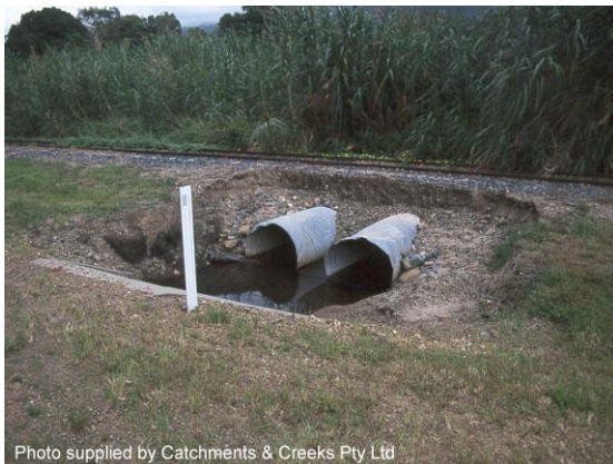
Severe inlet erosion on cane field railway
