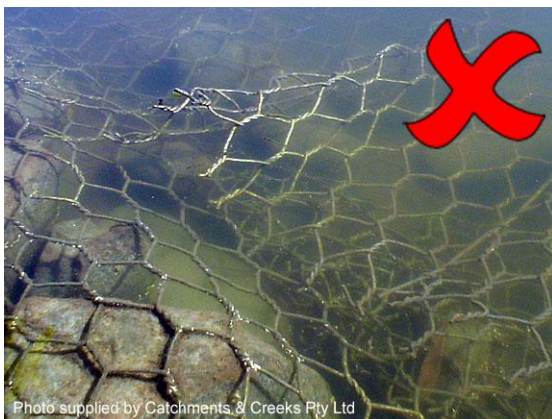
Damaged wire mesh
