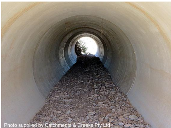
Natural deposition of bed material (NSW)
