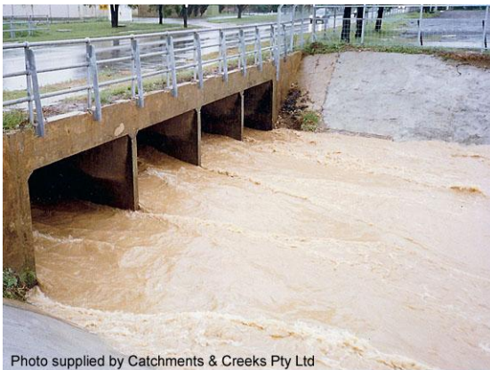
Culvert discharge with low tailwater (NSW)
