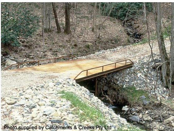
Small steel bridge (USA)
