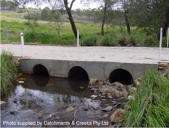
Inlet flush with a straight headwall (NSW)
