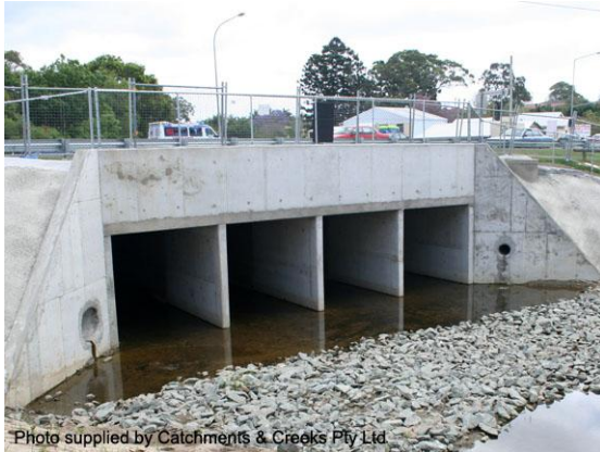
Box culvert with deep deck (Qld)
