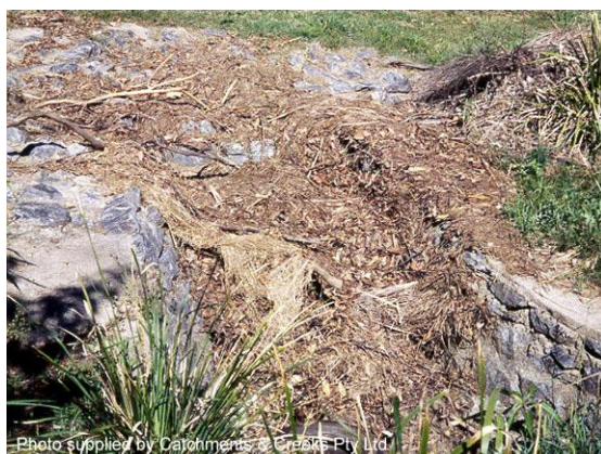
A fully blocked inlet screen (Qld)
