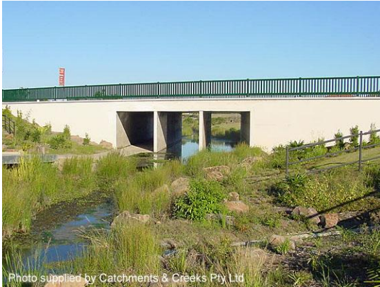
Flush or straight headwall (Qld)
