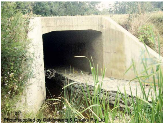
Single cell culvert (Qld)
