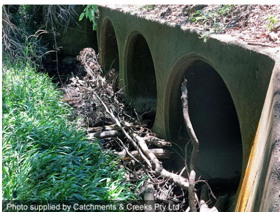
Debris blockage (Qld)
