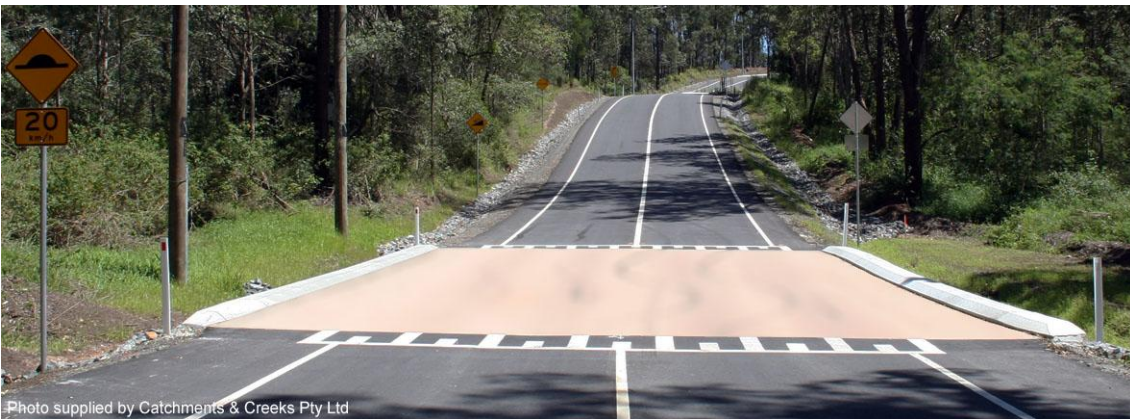
Traffic calming speed bump (Qld)
