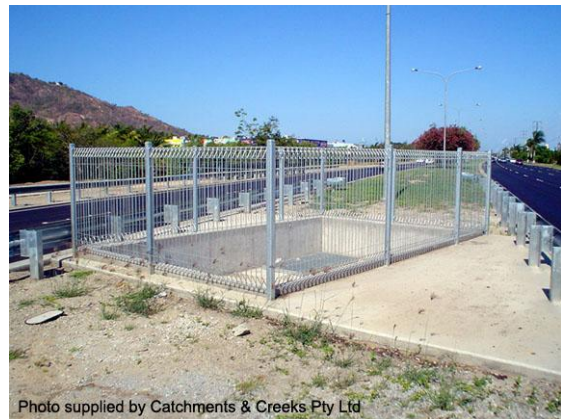
Skylights placed within the median (Qld)
