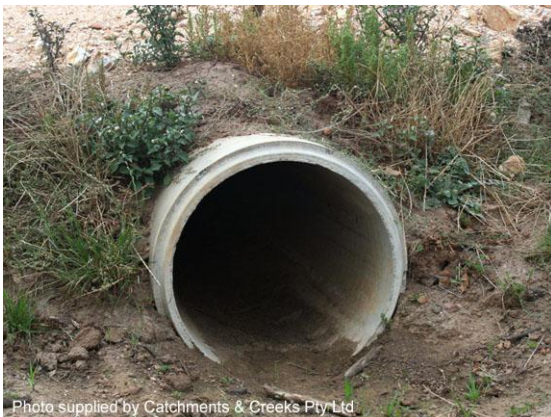
Projected pipe inlet (SA)
