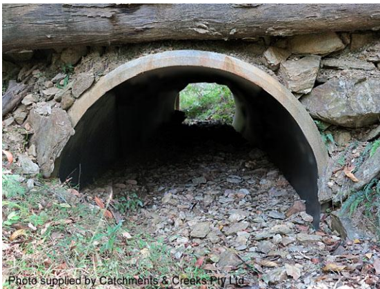
Small private culvert without headwall
