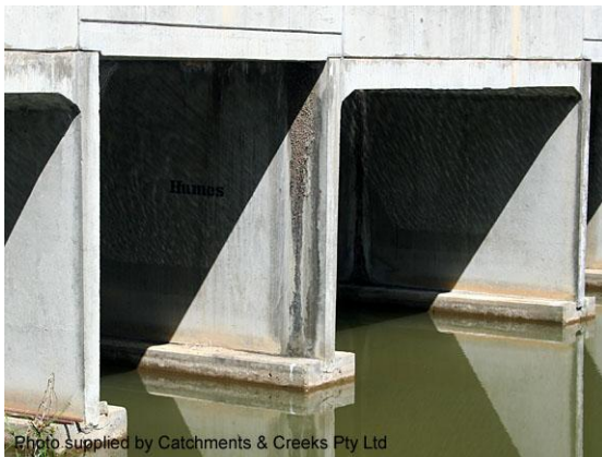
Pre-cast box culvert with bridging slab
