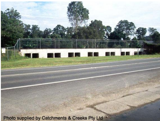
Floodplain culvert adjacent a bridge (Qld)
