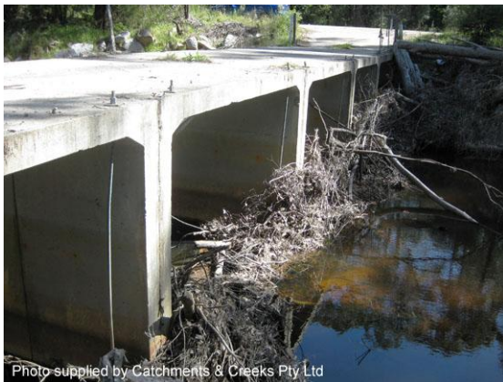
Rural, multi-cell box culvert (NSW)
