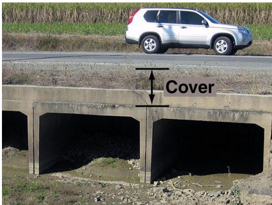
Roadbase cover over a box culvert (Qld)
