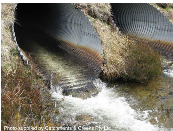
Elevated pipe culvert (NSW)
