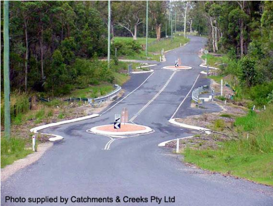
Traffic calming on a rural road (Qld)
