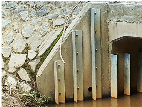
Baffles placed on wingwalls (Qld)
