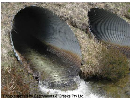
Corrugated pipe culvert (NSW)
