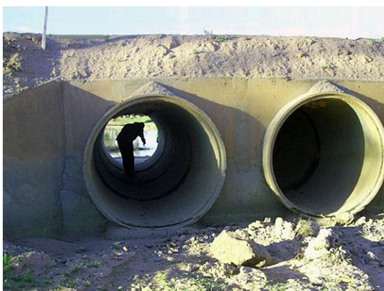
Post-flood culvert inspection (Qld)
