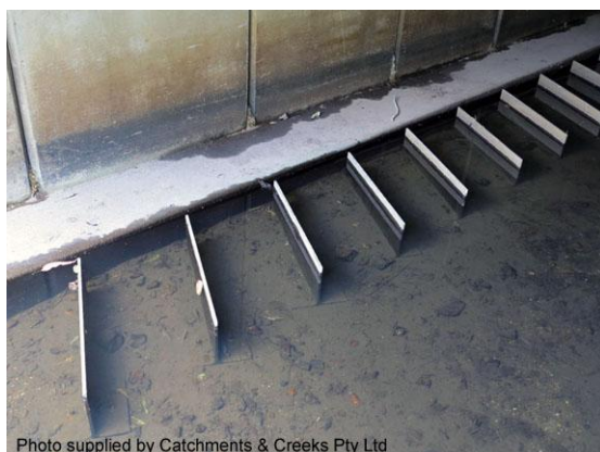
Baffles attached to the terrestrial pathway
