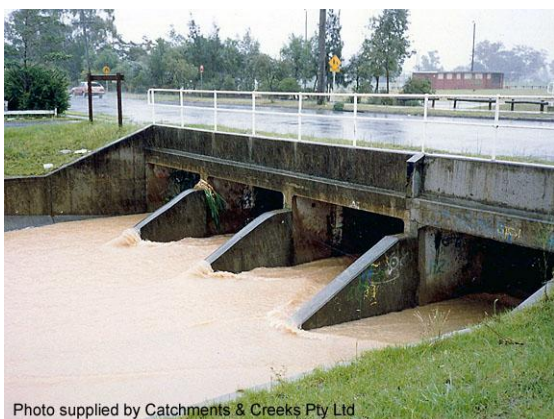
Debris deflection walls (NSW)
