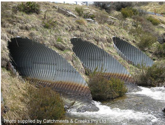
Corrugated pipe culvert (NSW)
