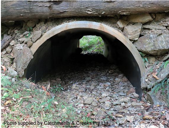
Simple arch crossing (Qld)
