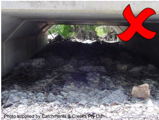
Rock mattress placed on culvert bed
