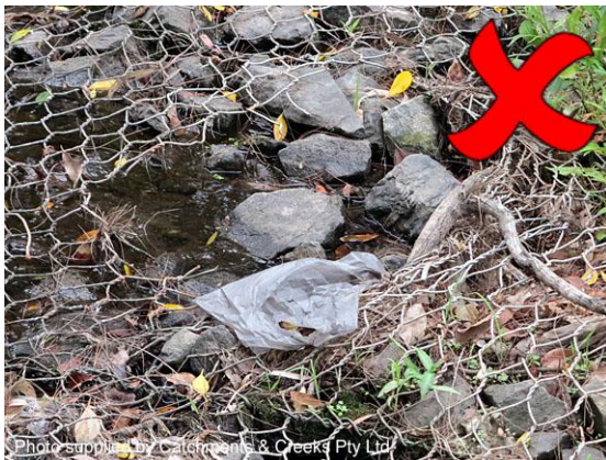
Wire mesh ripped open
