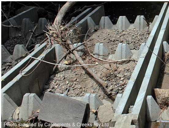
Sediment deposition within a fishway
