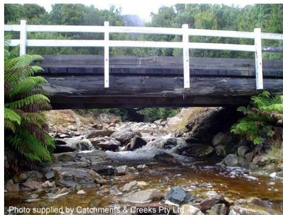
Single span log bridge (Tas)
