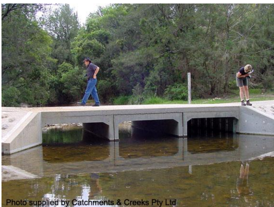
Recessed culvert without aprons (NSW)
