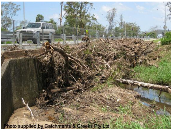
100% debris blockage (Qld)
