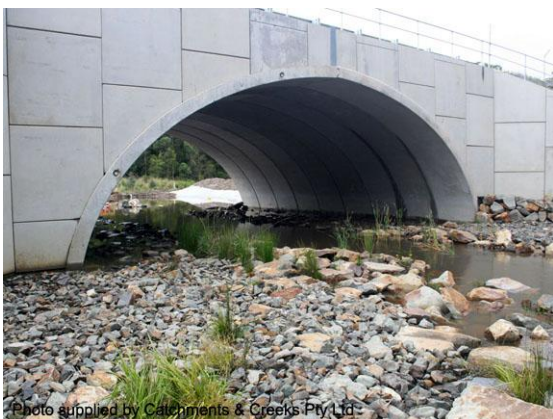
Arch bridge (NSW)
