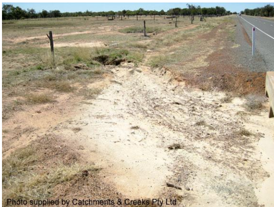
Early stage of upstream gully erosion
