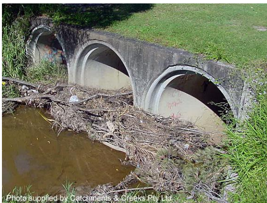
Medium level of debris blockage
