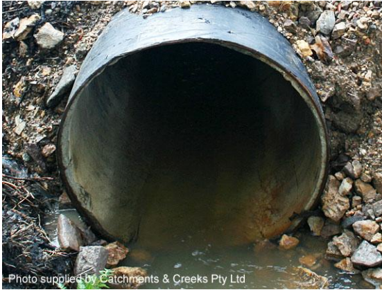
Projected pipe inlet (Qld)
