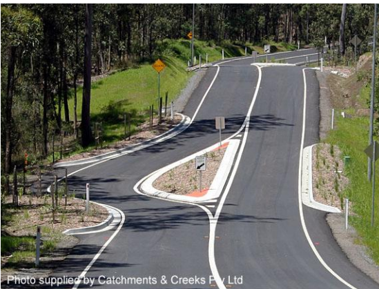
Traffic calming on a back road (Qld)
