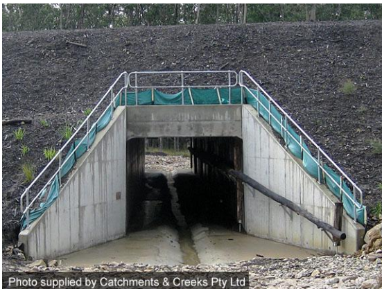
Floodplain culvert (NSW)
