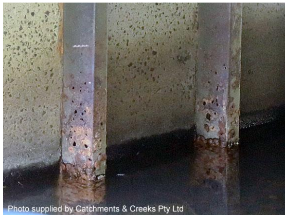
Rusted galvanised steel baffles (NSW)
