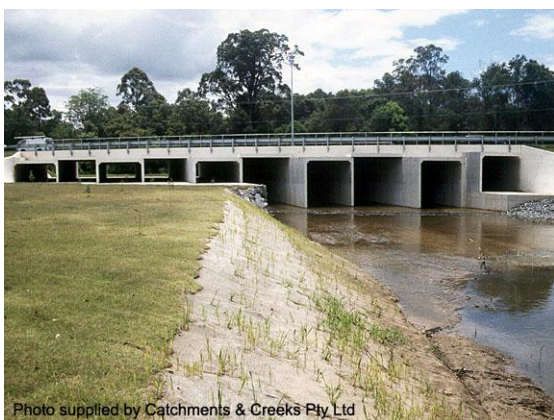
Multi-purpose culvert with wet & dry cells
