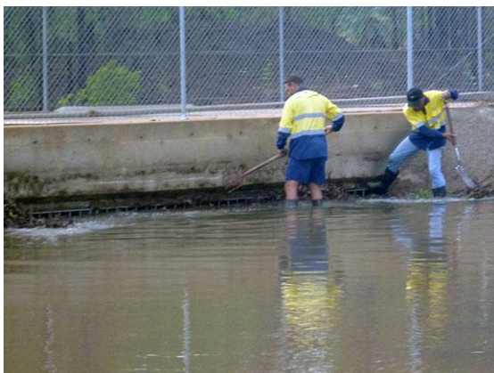
Post-flood screen clearing (NT)
