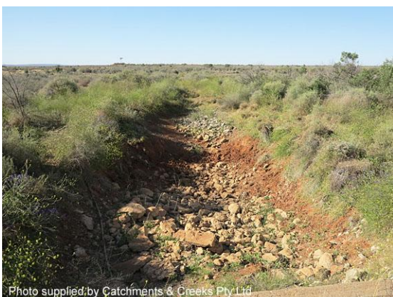
Looking downstream from a culvert (Qld)
