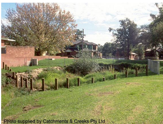
Safety poles (NSW)
