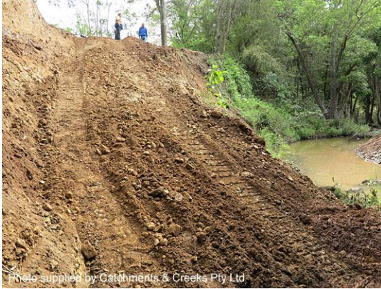
Temporary access ramp (Qld)
