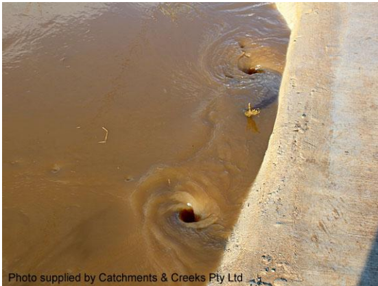
Inlet control (drowned inlet with vortices)
