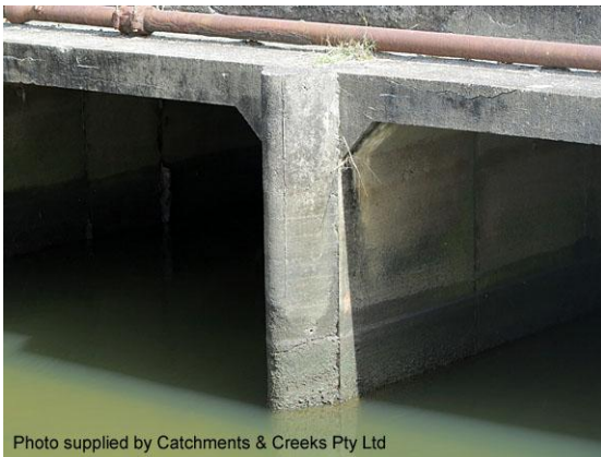
Rounded box culvert leg (Qld)
