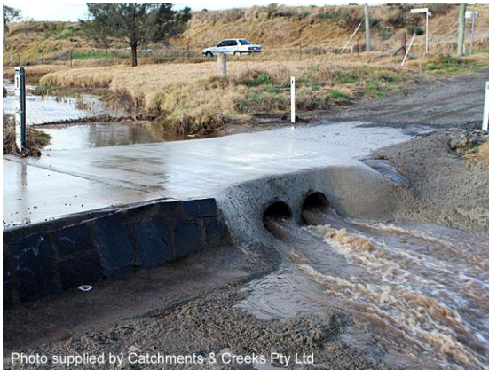
Inlet control (looking upstream, Qld)
