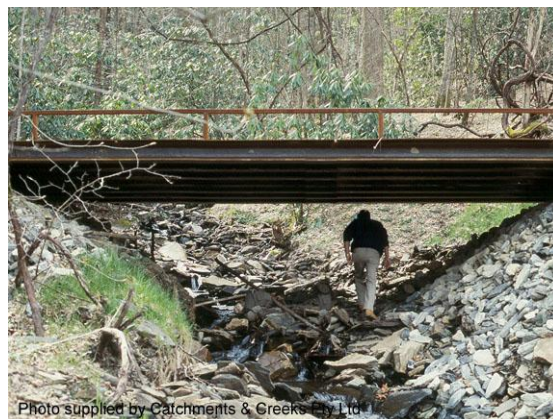
Small steel bridge (USA)
