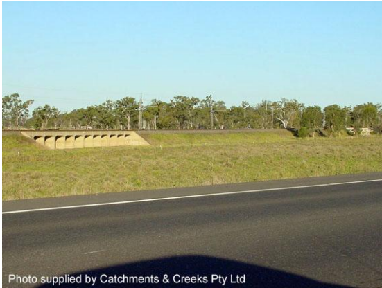
Floodplain culvert (bridge on far right)
