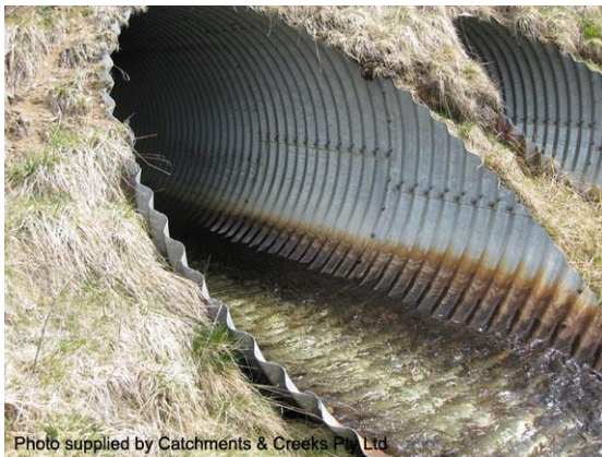
Corrugated pipe culvert (NSW)
