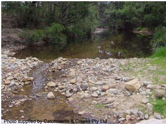
Constructed upstream riffle (2001)
