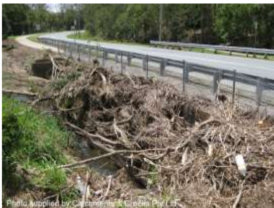
Severe debris blockage of a culvert (Qld)
