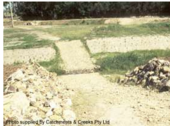
Access ramp (Qld)
