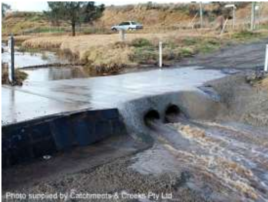
Inlet control (looking upstream, Qld)
