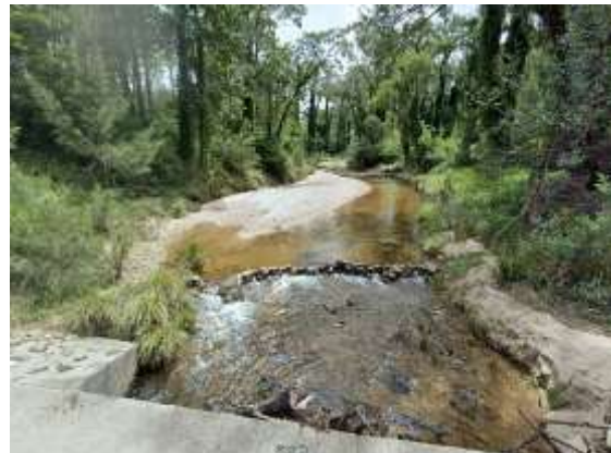
Inlet riffle washed away (2022)
