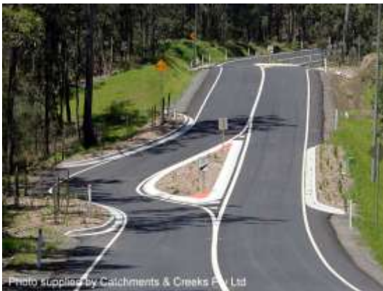
Traffic calming on a back road (Qld)
