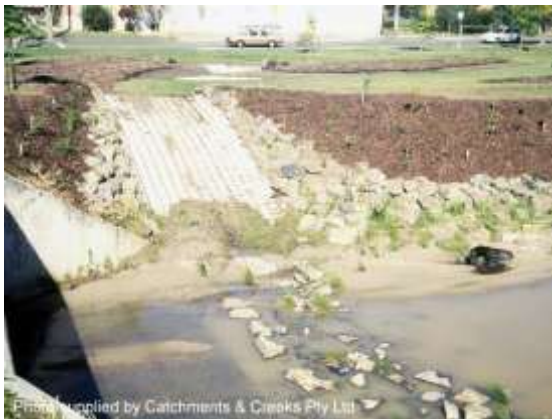
Recently installed ramp (1997)
