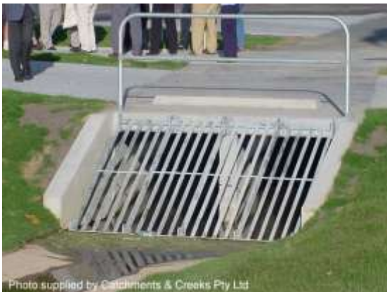
45-degree inlet screen (Qld)
