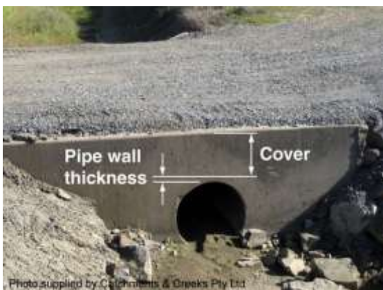
Small pipe culvert on a gravel road (Qld)
