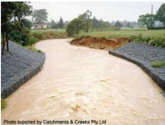
Outlet jetting during high tailwater (NSW)
