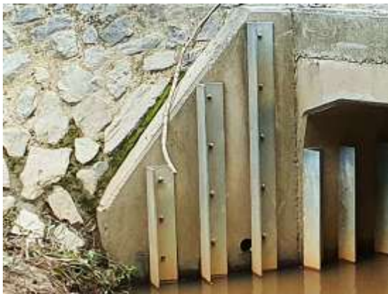
Baffles placed on wingwalls (Qld)
