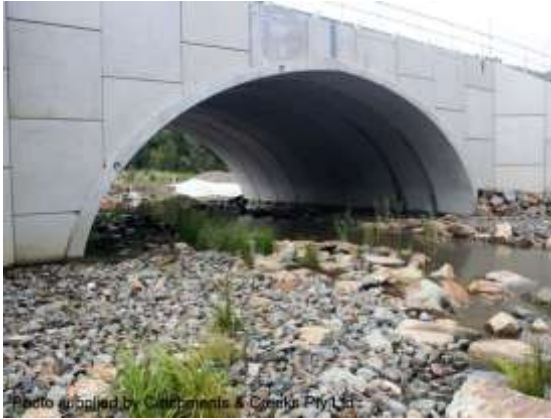
Arch bridge (NSW)
