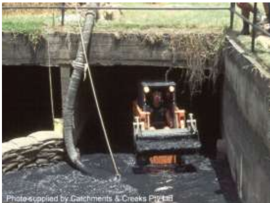
De-silting a long culvert
