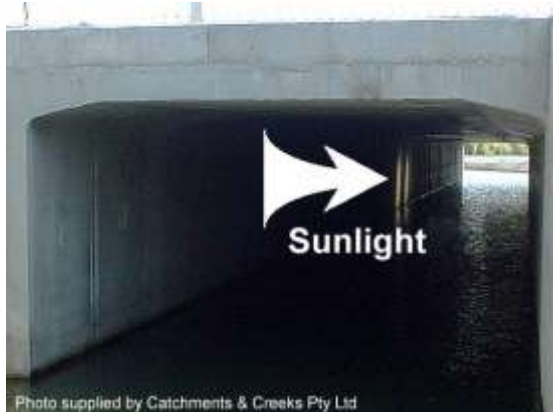
Light entering the culvert (Qld)
