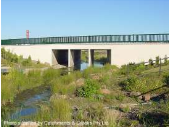
Flush or straight headwall (Qld)
