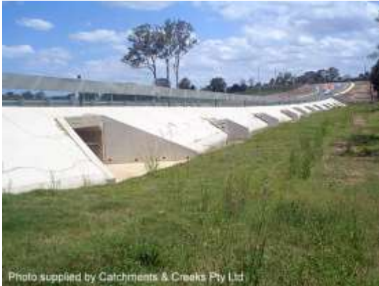
Floodplain culvert with well-spaced cells
