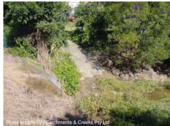
Same access ramp shown left in 2003
