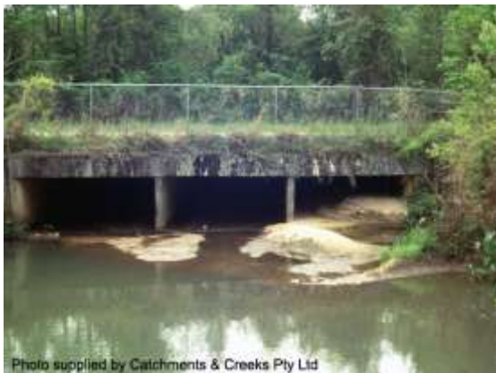
Sediment deposition (USA)
