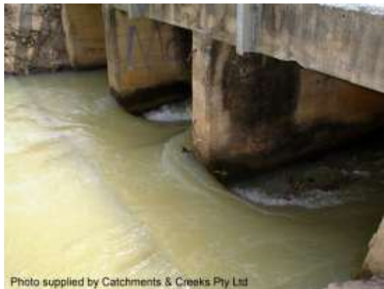
Inlet of a multi-cell box culvert (Qld)
