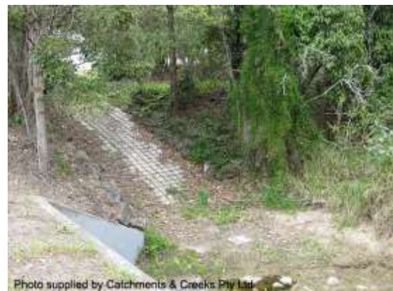
Same access ramp in 2014
