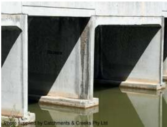
Pre-cast box culvert with bridging slab
