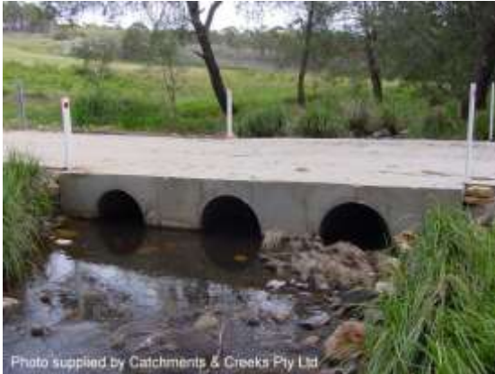
Inlet flush with a straight headwall (NSW)
