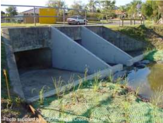
Culvert with sediment control weirs (Qld)
