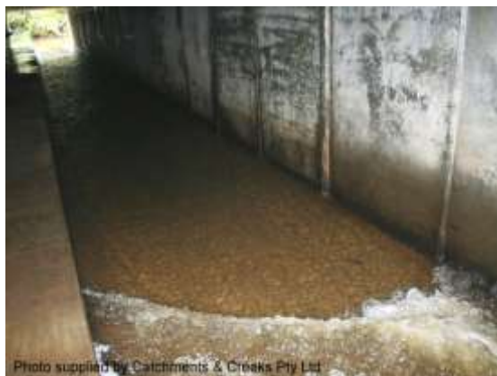
Supercritical flow within a culvert (Qld)
