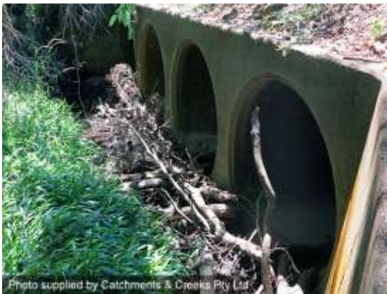
Debris blockage (Qld)
