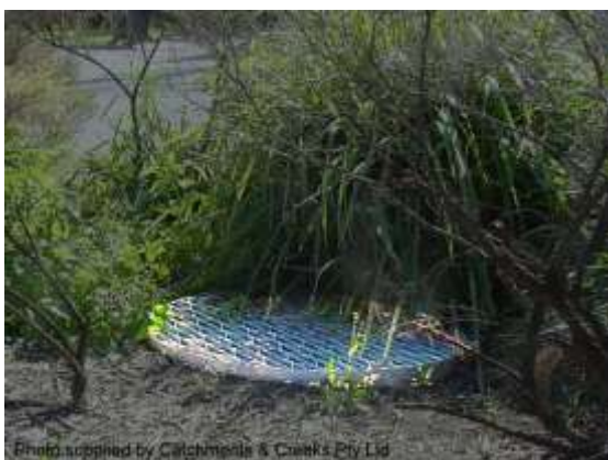
Skylights placed within the median (Qld)
