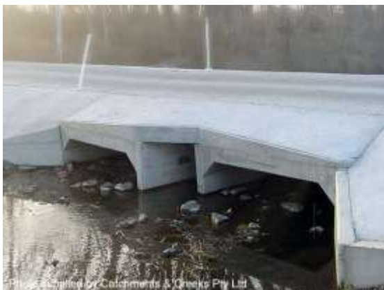
Gravel bed within a culvert (NSW)
