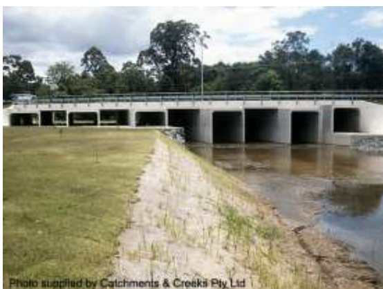
Multi-purpose culvert with wet & dry cells
