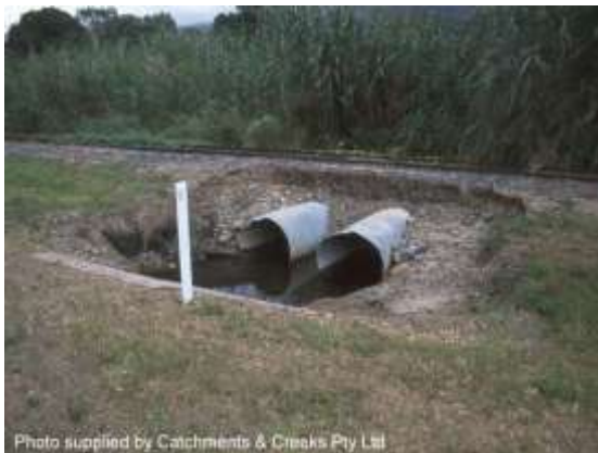
Severe inlet erosion on cane field railway
