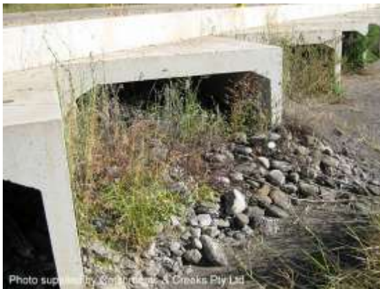
Culvert placed over a gravel-based creek
