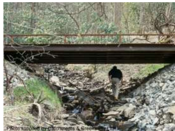
Small steel bridge (USA)
