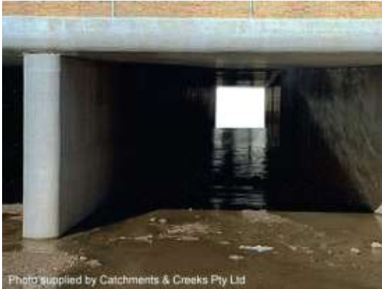
Rounded face of a box culvert leg (NSW)
