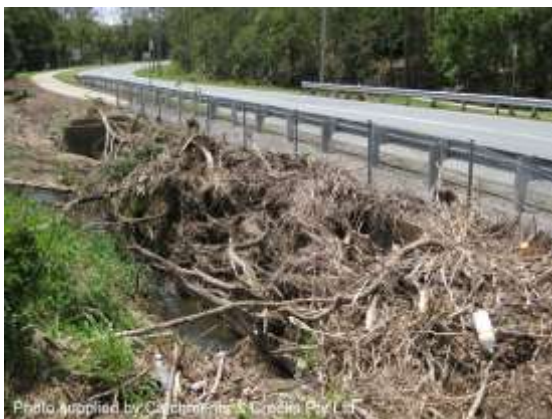
High level of debris blockage
