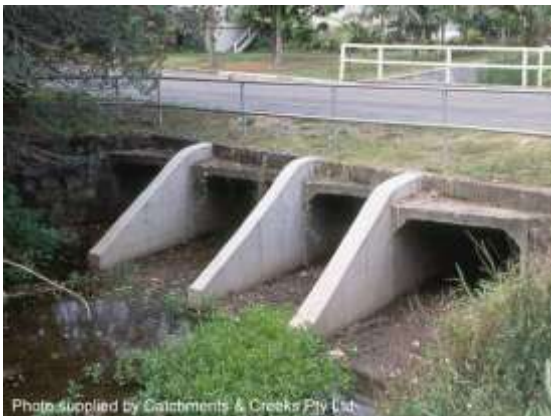
Debris deflection walls, 1995 (Qld)
