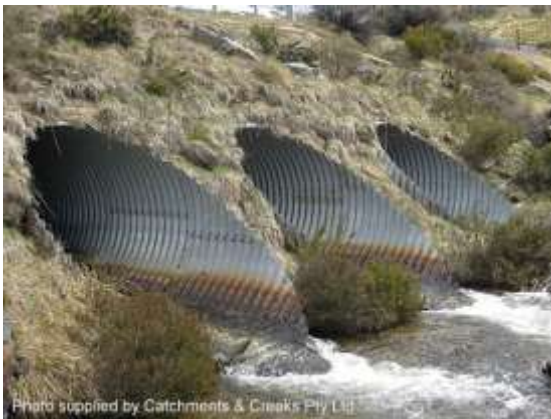
Corrugated pipe culvert (NSW)
