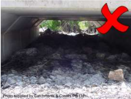
Rock mattress placed on culvert bed
