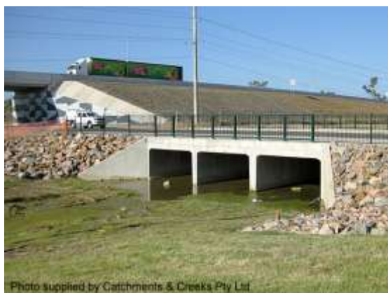
Box culvert (Qld)
