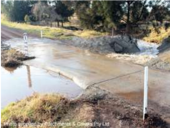
Inlet control (looking downstream, Qld)
