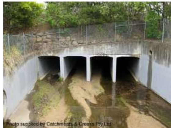
Open roof section within a long culvert
