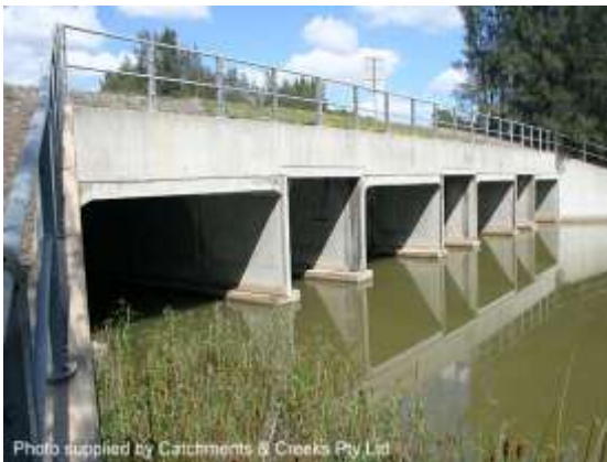
Multi-cell culvert with flat bed (NSW)
