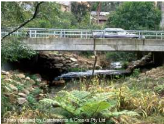
Single span concrete bridge (NSW)
