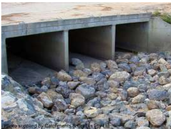
Culvert outlet with rock pad (NSW)
