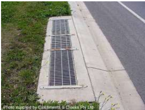
Skylight installed into the grass verge
