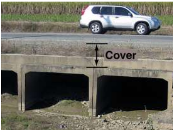
Roadbase cover over a box culvert (Qld)
