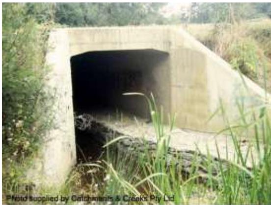
Single cell culvert (Qld)
