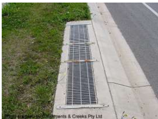
Skylights placed in footpath verge (Qld)
