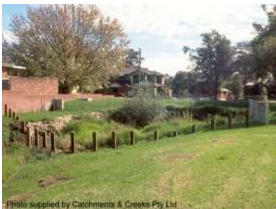
Safety poles (NSW)
