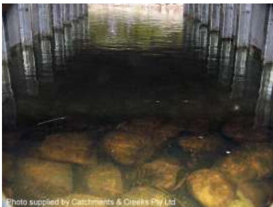
Placement of loose rock (NSW)
