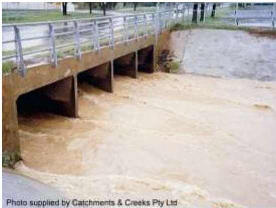
Culvert discharge with low tailwater (NSW)
