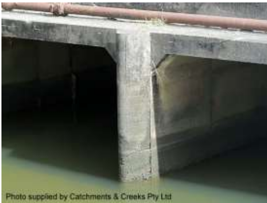
Rounded box culvert leg (Qld)
