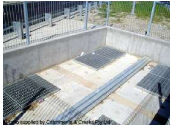
Skylights placed within the median (Qld)
