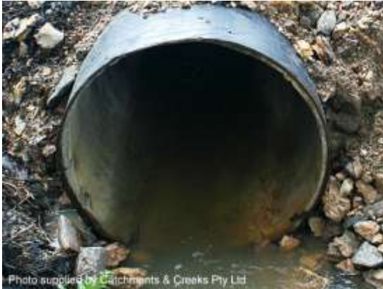
Projected pipe inlet (Qld)
