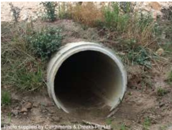
Projected pipe inlet (SA)
