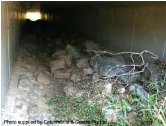
Rocks deposited in a low-flow channel
