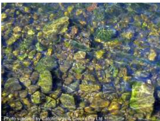
Loose rock placement (SA)
