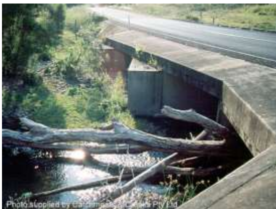
Trapped woody flood debris (Qld)
