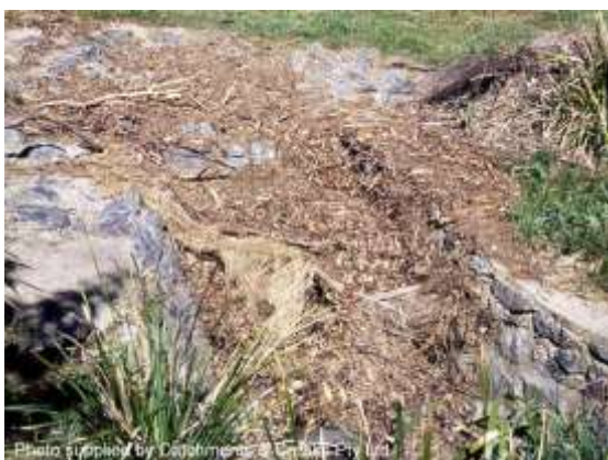
A fully blocked inlet screen (Qld)
