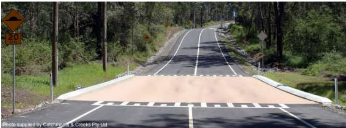
Traffic calming speed bump (Qld)
