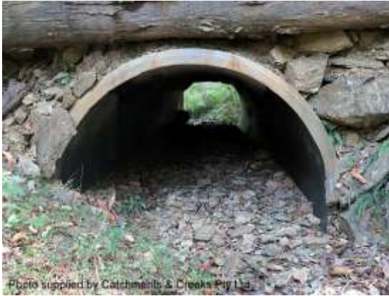
Simple arch crossing (Qld)
