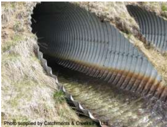
Corrugated pipe culvert (NSW)
