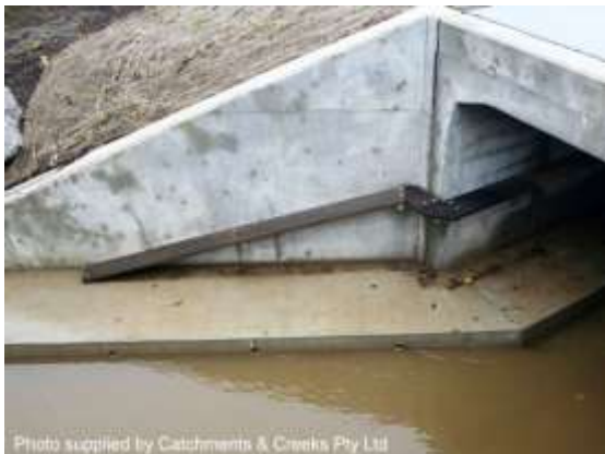
Access ramps (Qld)
