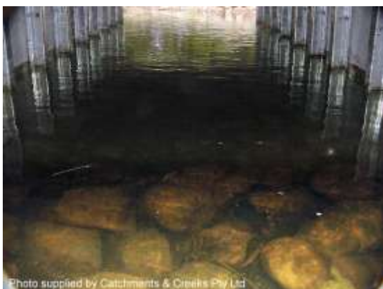
Rock placement (NSW)
