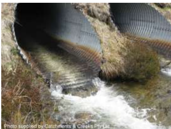
Elevated pipe culvert (NSW)
