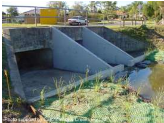
Culvert with sediment control weirs (Q1d)
