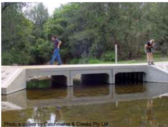
Recessed culvert without aprons (NSW)
