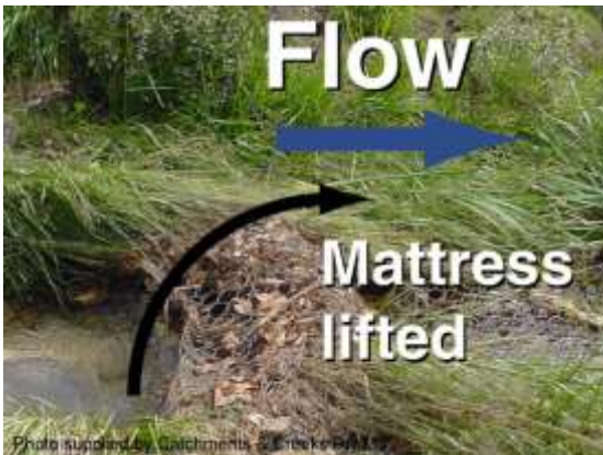
Lifting of rock mattress (Qld)
