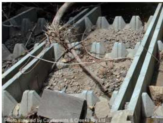
Sediment deposition within a fishway
