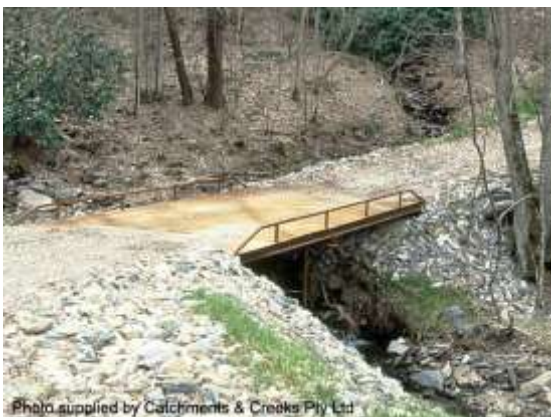
Small steel bridge (USA)
