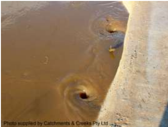
Inlet control (drowned inlet with vortices)
