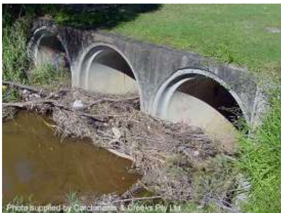
Medium level of debris blockage
