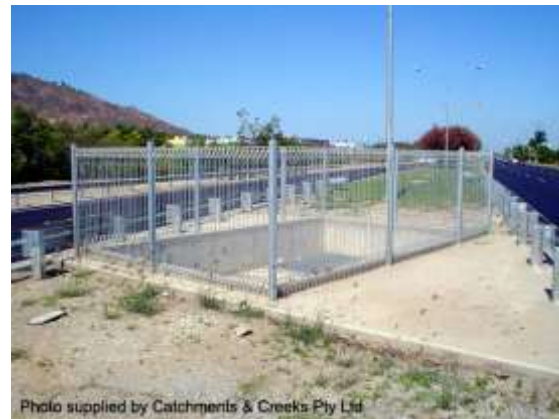
Skylights placed within the median (Qld)
