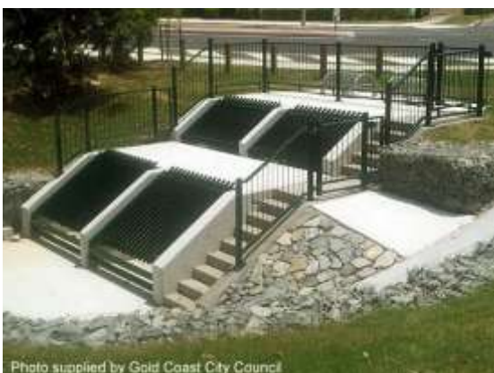
Complex inlet screen (Gold Coast, Qld)
