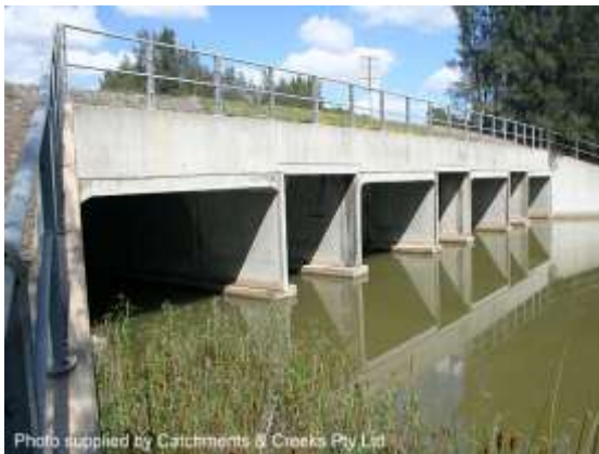
Culvert with multiple wet cells (NSW)
