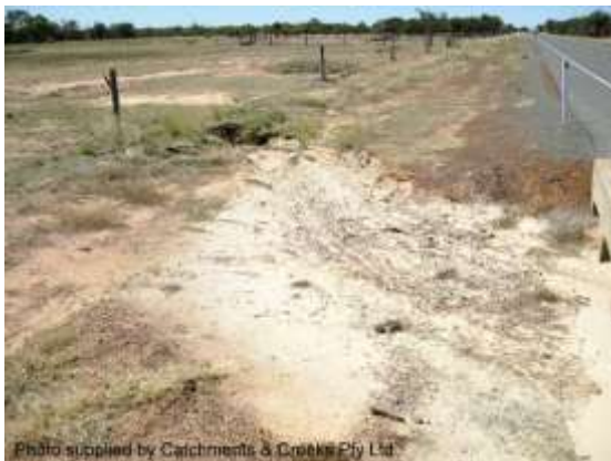
Early stage of upstream gully erosion
