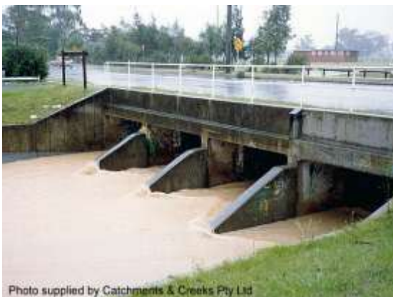
Debris deflection walls (NSW)
