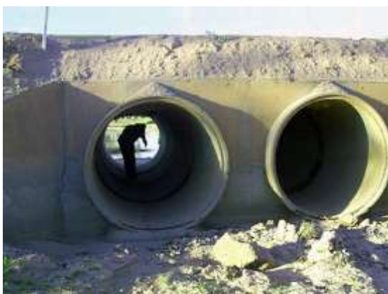
Post-flood culvert inspection (Qld)
