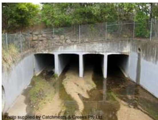
Open roof section within a long culvert
