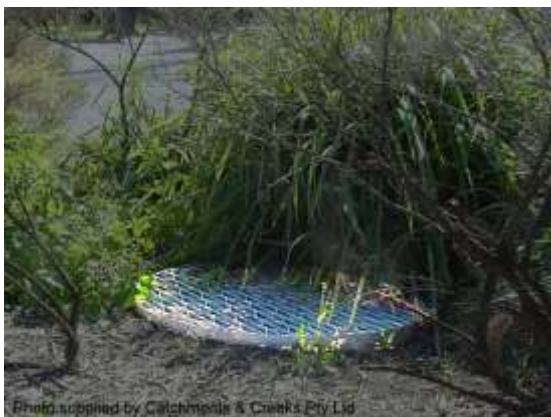
Skylights installed in a raised median (Qld)
