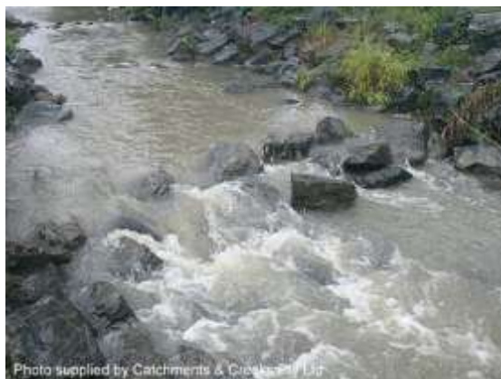
Constructed pool-riffle system (Qld)
