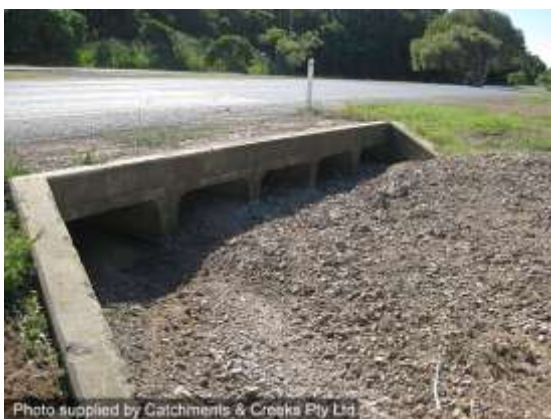
Sediment blockage (Qld)
