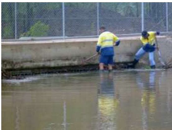
Post-flood screen clearing (NT)
