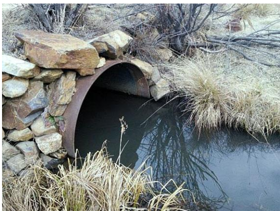
Recessed culvert on Bogong Creek, ACT
