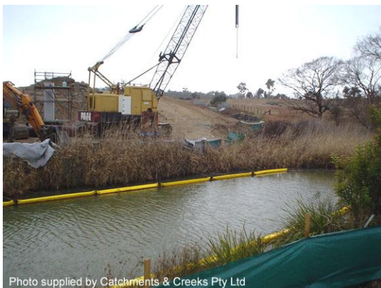
Instream flow-diversion silt curtain (NSW)
