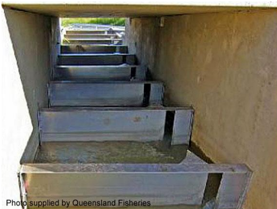
Slotted weir-type baffle (Tim Marsden)
