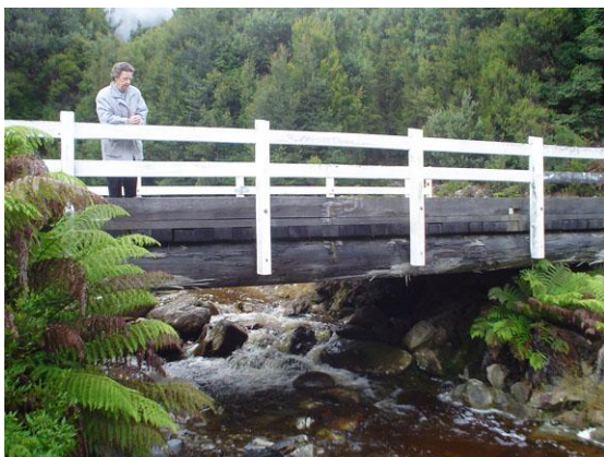
Timber bridge near Montezuma Falls, Tas.
