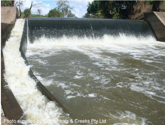
Fish ladder adjacent to a weir (Qld)
