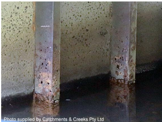
Rusted galvanised steel baffles (NSW)
