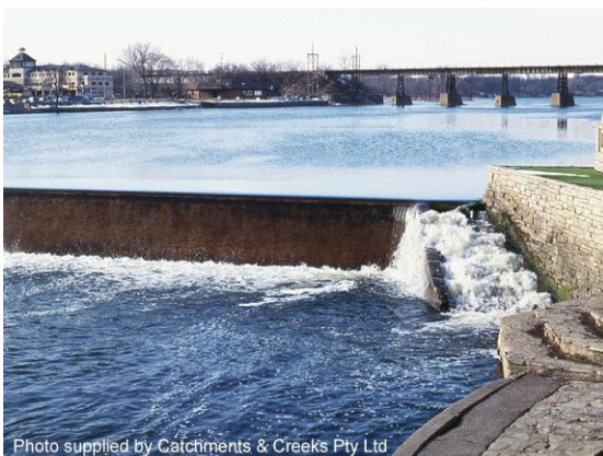
Fish ladder on a river weir (USA)
