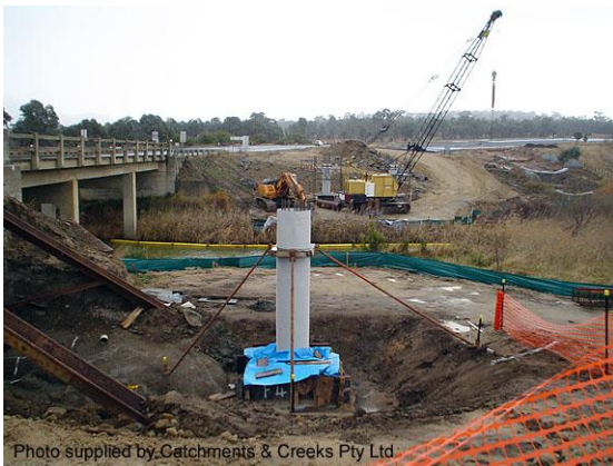
Bridge construction (NSW)
