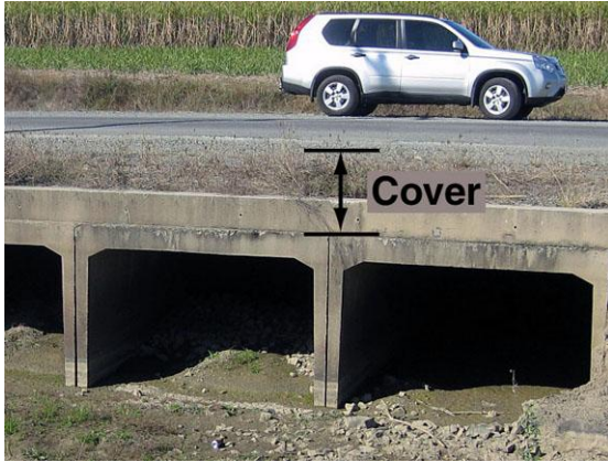
Roadbase cover over a box culvert
