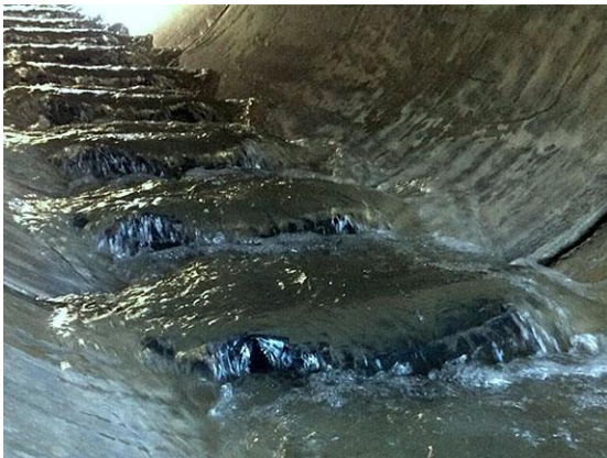
Flexible weir floor baffle (USA)
