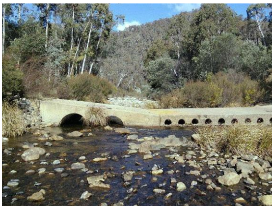
Burkes Creek Road crossing, ACT
