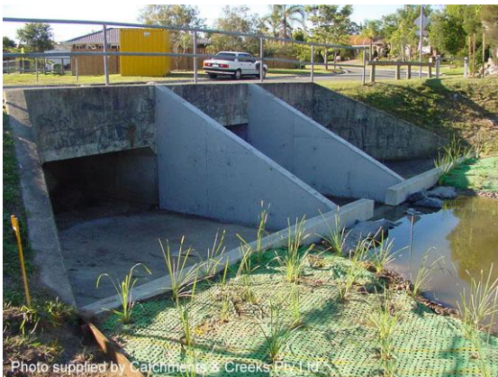
Culvert with sediment control weirs (Qld)
