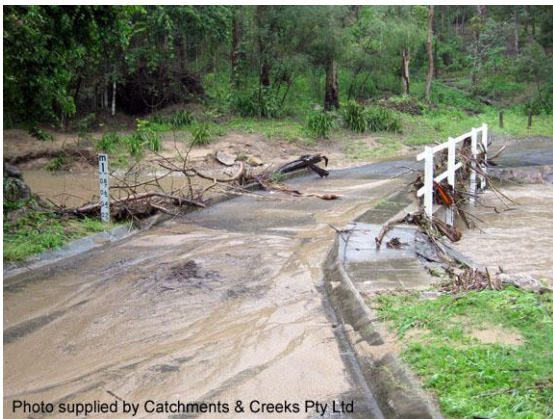
Flood damage to waterway crossing (Qld)
