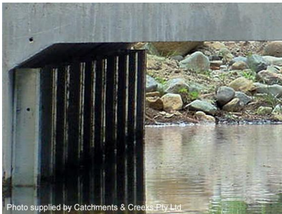
Sidewall baffles (NSW)
