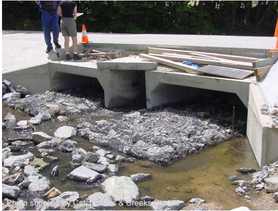
Culvert reconstruction (NSW)
