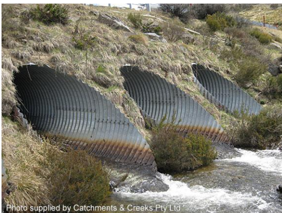
Corrugated pipe culvert (NSW)
