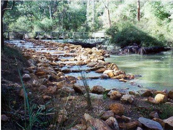
Apex Weir Fishway, Margaret River, WA
