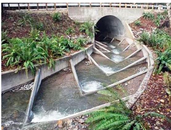
Chevron baffles at culvert inlet
