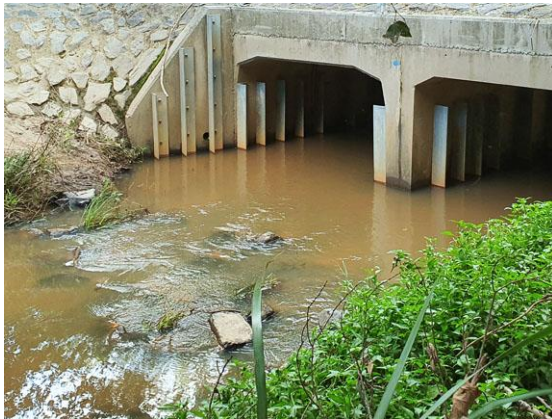
Box culvert with baffles
