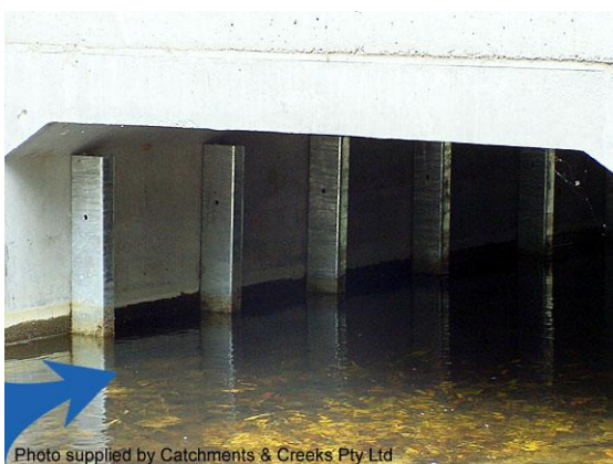
Sidewall baffles
