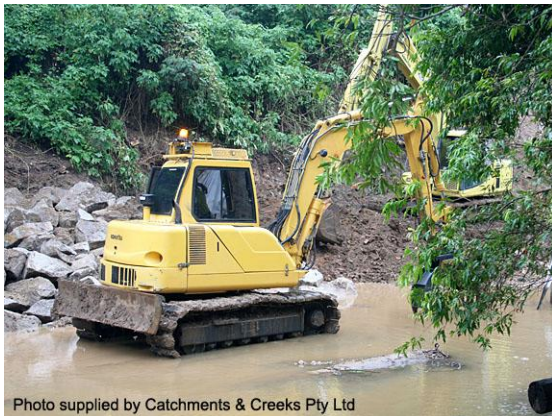
Placement of scour protection
