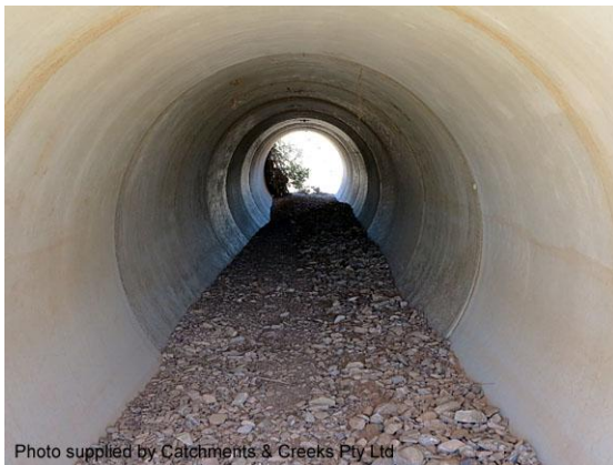
Deposition of sediments in a pipe culvert
