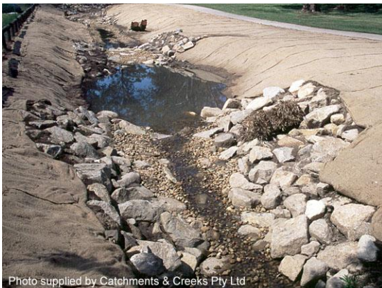
Constructed pool-riffle system (Qld)
