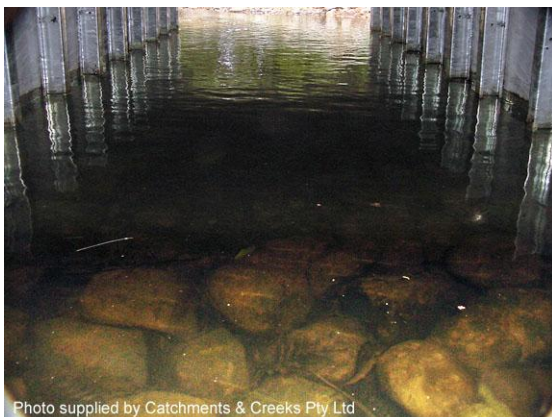
Introduced bed roughness rock
