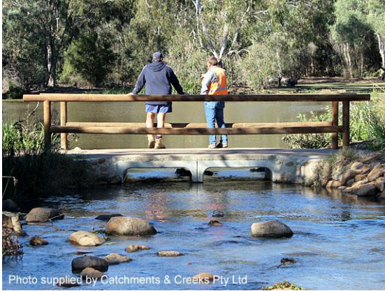
Fishway bypass around a fish barrier
