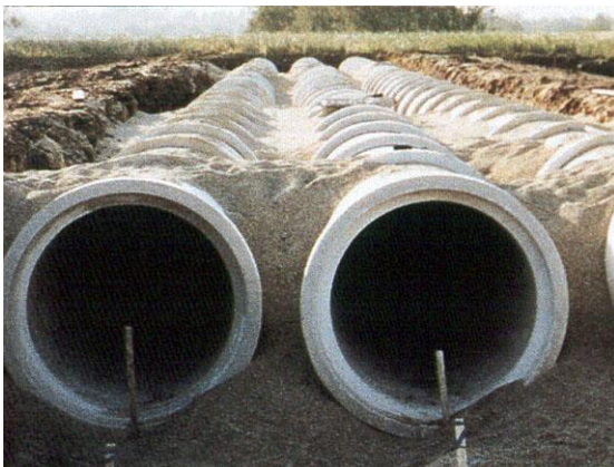
Installation of a long pipe culvert
