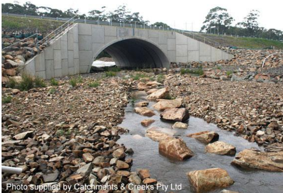
Arch bridge construction (NSW)
