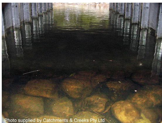
Introduced bed roughness rocks
