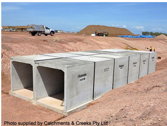
Culvert construction (NT)
