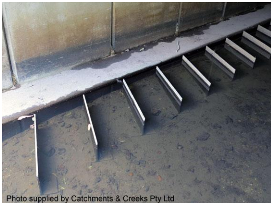
Baffles attached to the terrestrial pathway
