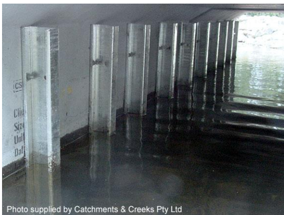
Sidewall baffles (NSW)
