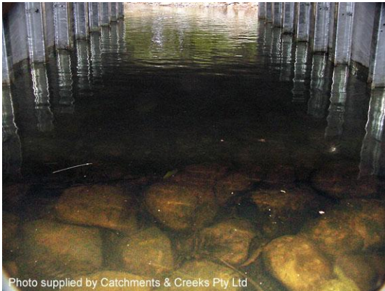
Artificial culvert-bed roughness
