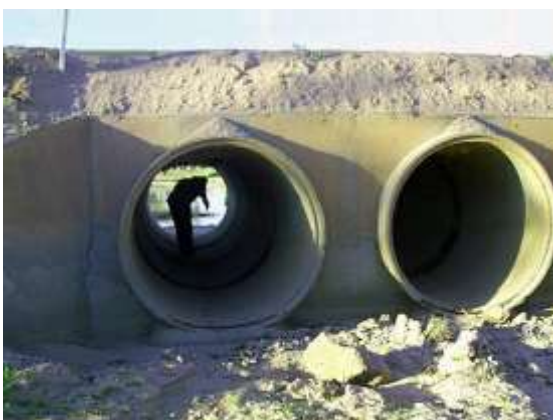
Culvert inspection (Qld)
