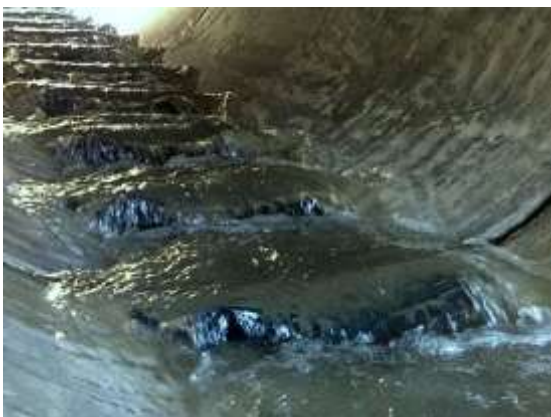
Flexible weir floor baffle (USA)
