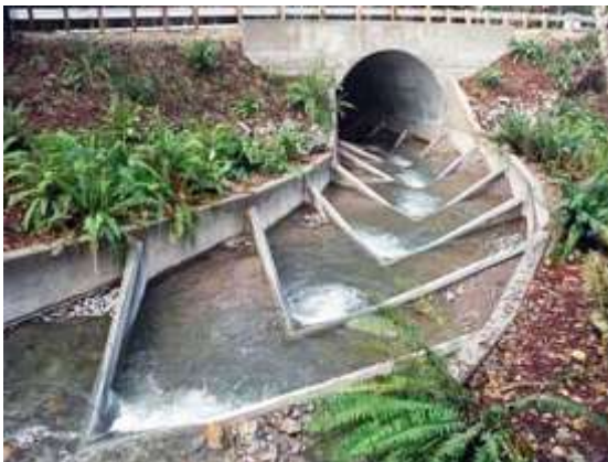
Chevron baffles at culvert inlet
