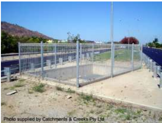
Sunken skylight placed in a road median
