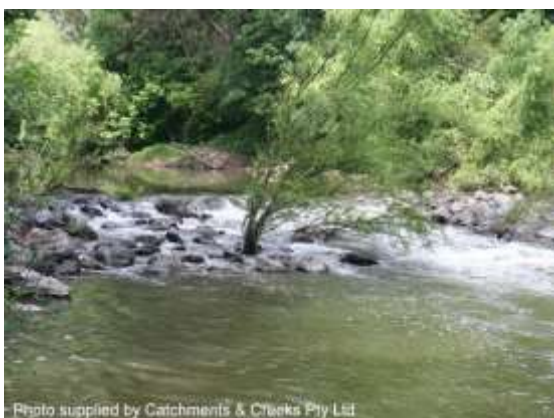
Constructed rock ramp/chute (NSW)
