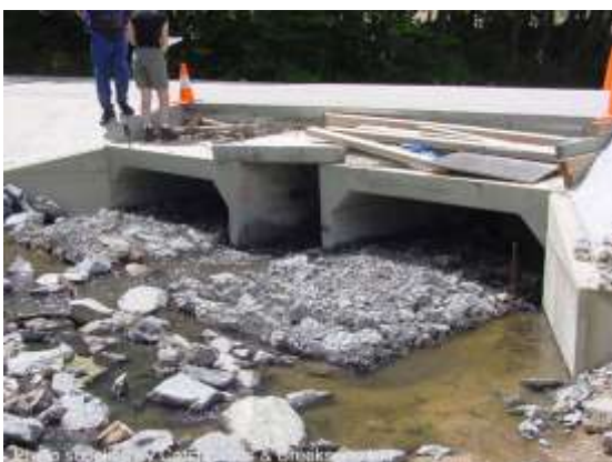
Culvert construction (NSW)
