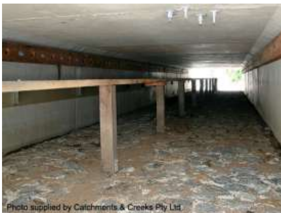
Lizard runs and roughened culvert bed
