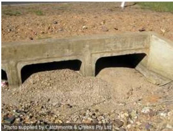
Sediment flow through a culvert (Qld)
