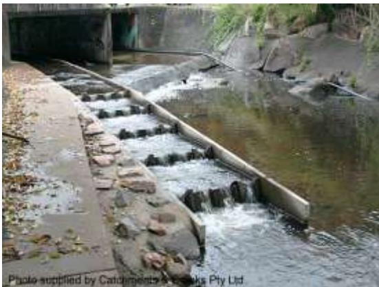
Constructed fishway (Qld)
