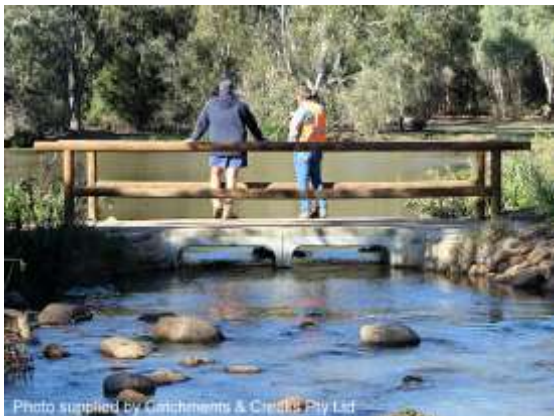
Fishway bypass around a fish barrier
