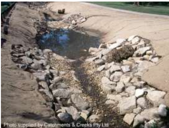
Constructed pool-riffle system (Qld)
