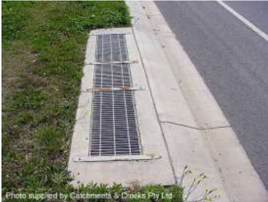
Example of a skylight ('light grid')
