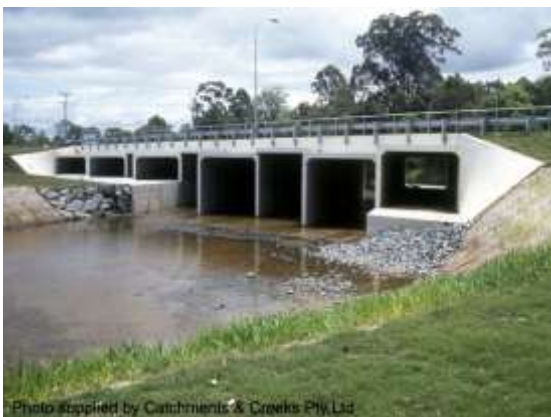
Multi-cell box culvert
