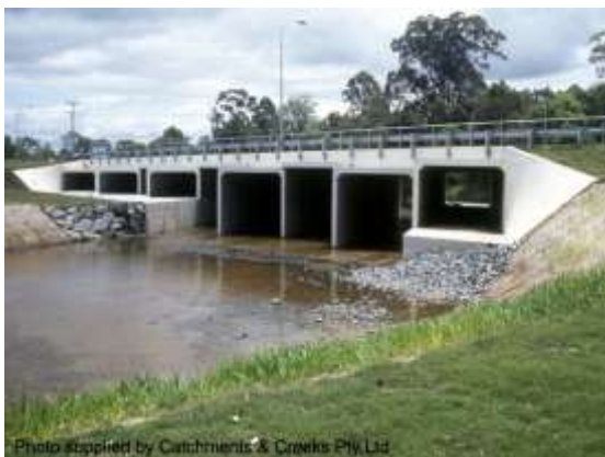
Multi-cell box culvert with wet & dry cells
