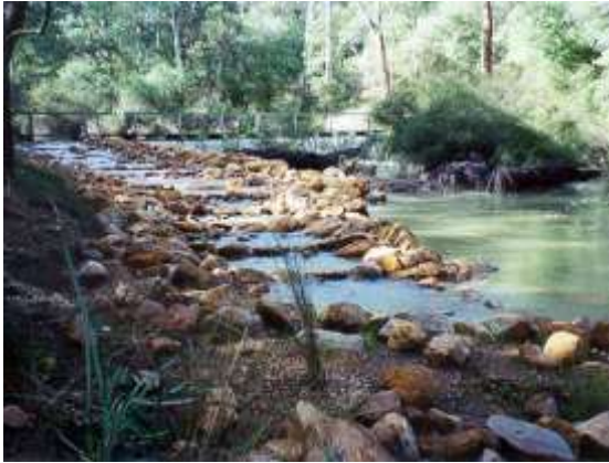
Apex Weir Fishway, Margaret River, WA
