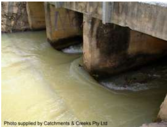
Flow separation at culvert inlet (Qld)
