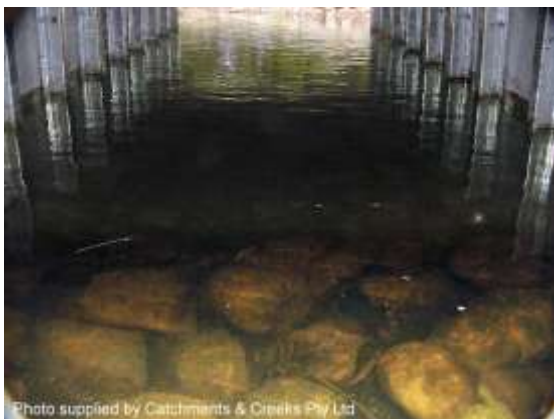
Artificial culvert-bed roughness
