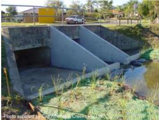
Culvert with sediment control weirs (Qld)
