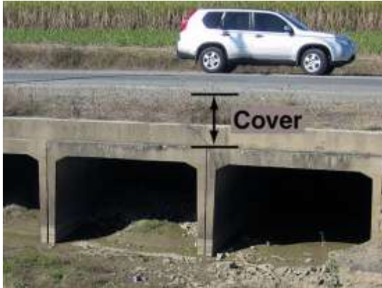
Roadbase cover over a box culvert
