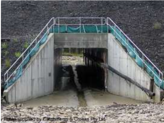
Fauna tunnel (NSW)
