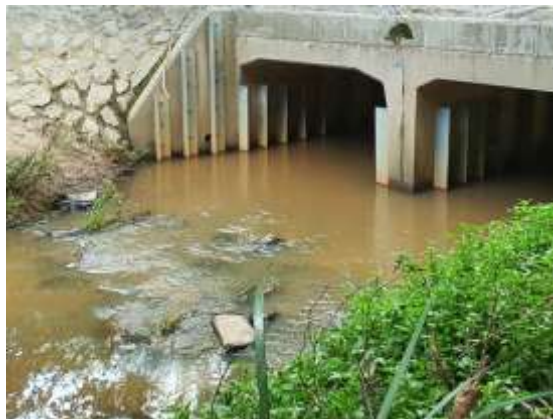
Box culvert with baffles
