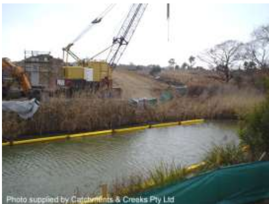
Instream flow-diversion silt curtain (NSW)
