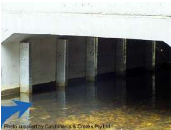
Sidewall baffles
