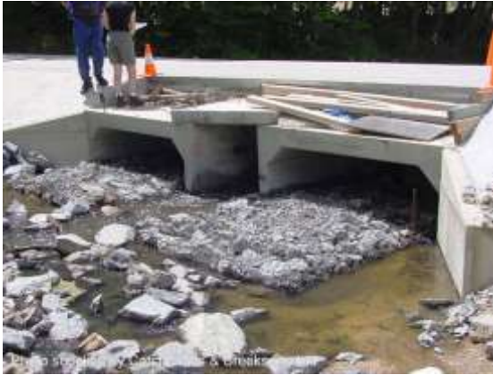
Culvert reconstruction (NSW)
