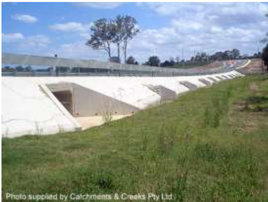
Floodplain culverts (Qld)
