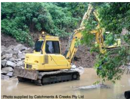
Placement of scour protection
