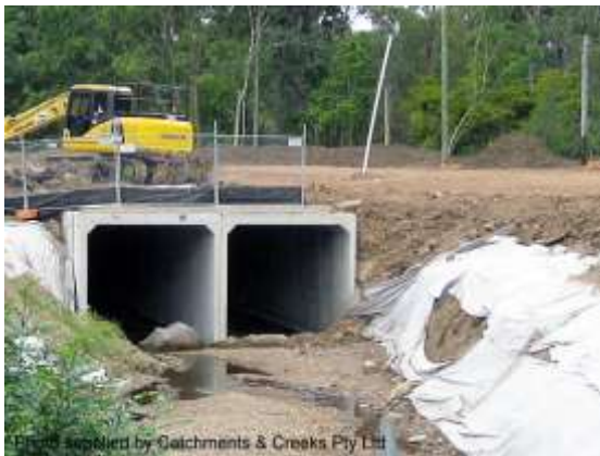
Culvert construction during low flows
