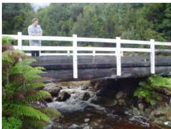
Timber bridge near Montezuma Falls, Tas.
