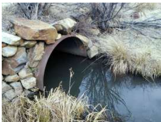
Recessed culvert on Bogong Creek, ACT
