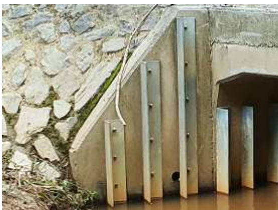
Baffles placed on a culvert wingwall (Qld)
