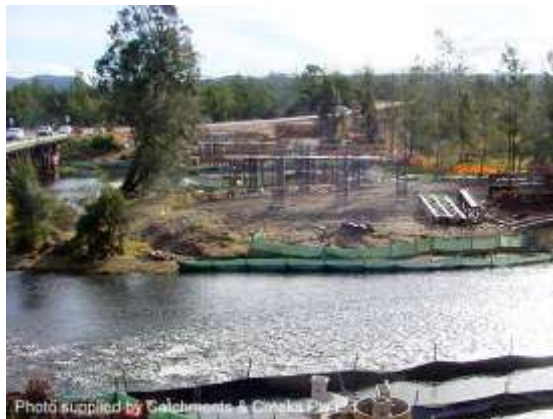
Bridge construction, Nepean River, NSW
