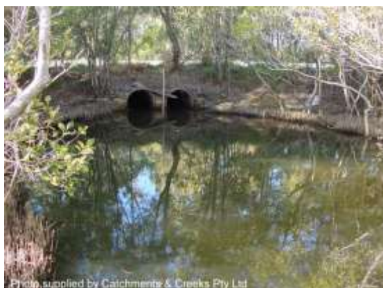
Tidal culvert (Brunswick Heads, NSW)
