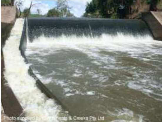
Fish ladder adjacent to a weir (Qld)
