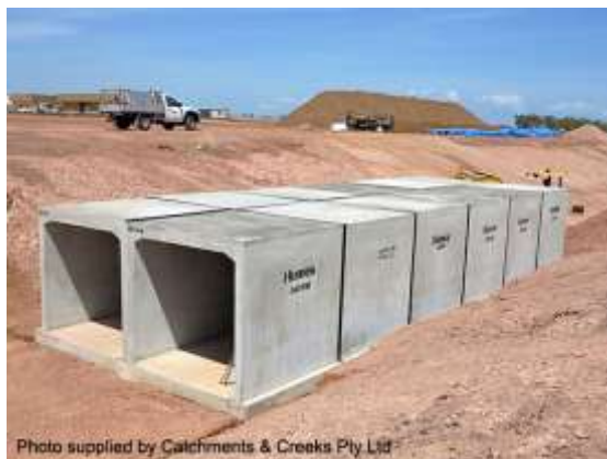
Culvert construction (NT)
