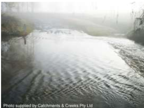
Smooth-turbulent flow over a road (NSW)
