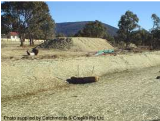
Long-term stockpile (bridge works, NSW)
