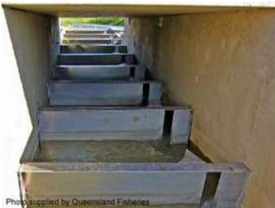
Slotted weir-type baffle (Tim Marsden)
