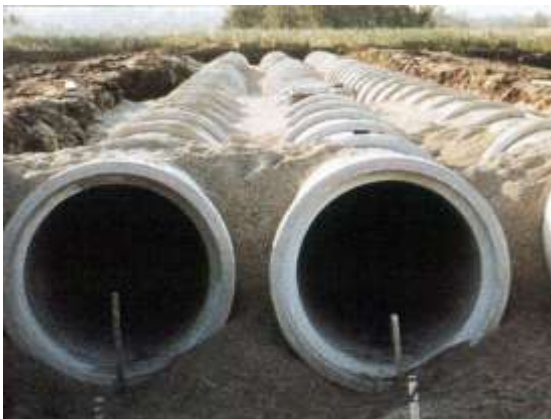
Installation of a long pipe culvert
