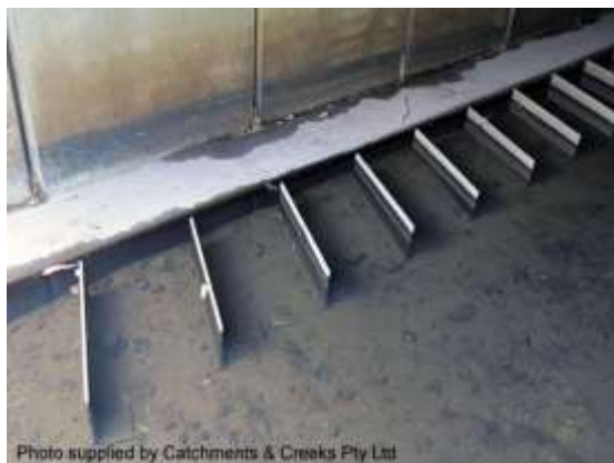
Baffles attached to the terrestrial pathway
