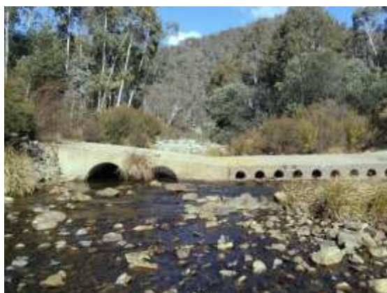
Burkes Creek Road crossing, ACT
