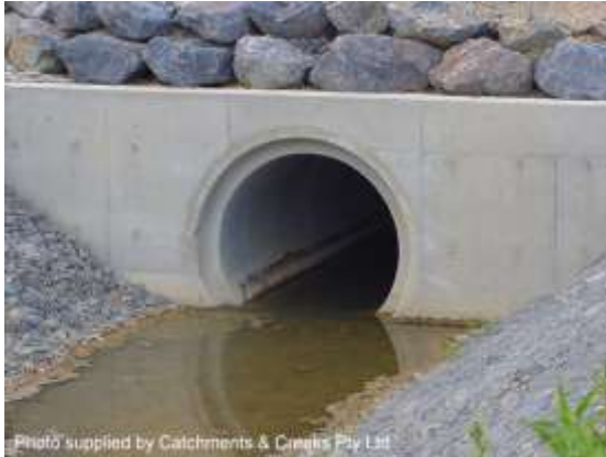
Single cell pipe culvert
