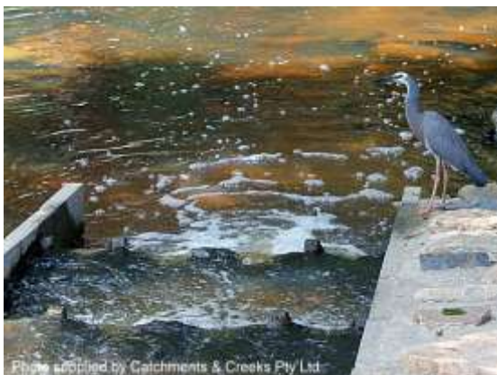
Inlet of the fishway (outlet of water flow)
