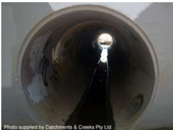
Single cell (barrel) of a pipe culvert
