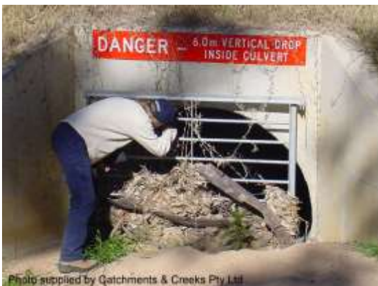
Inspection of an inlet safety screen (Qld)
