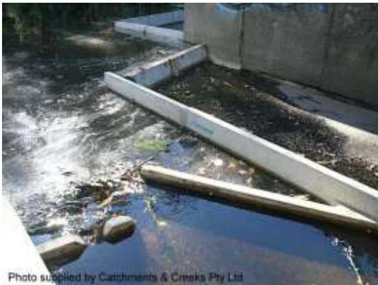
Upstream end of fishway (Qld)
