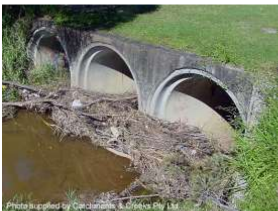
Medium level of debris blockage
