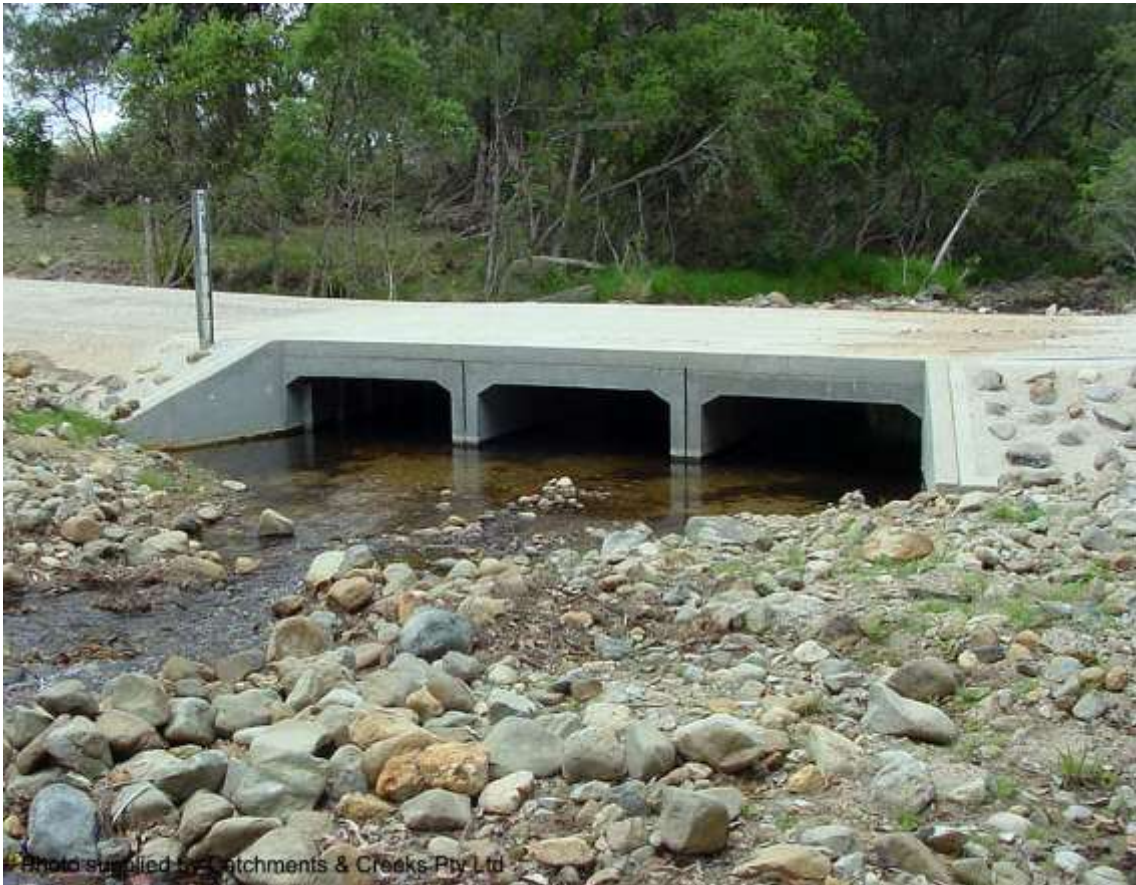
Replacement culvert, Ewingar, NSW (2001)
