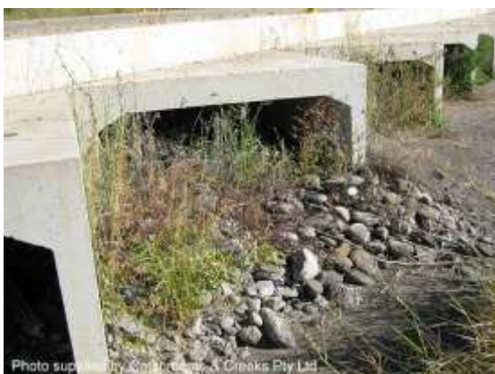
Deposition of natural bed gravel (Qld)
