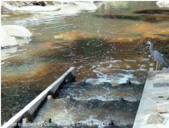
Downstream end of fishway (Qld)
