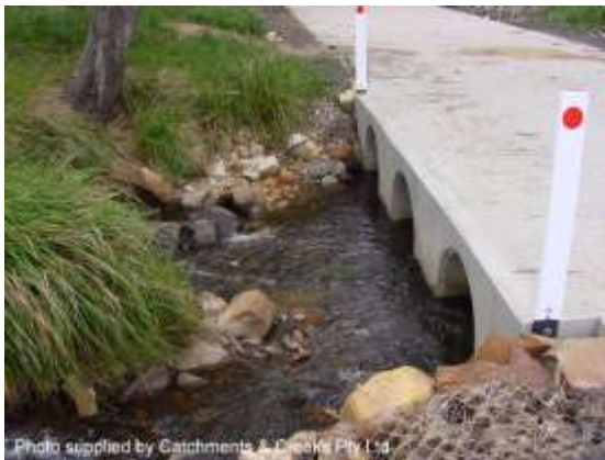
Outlet of the new culvert (NSW)
