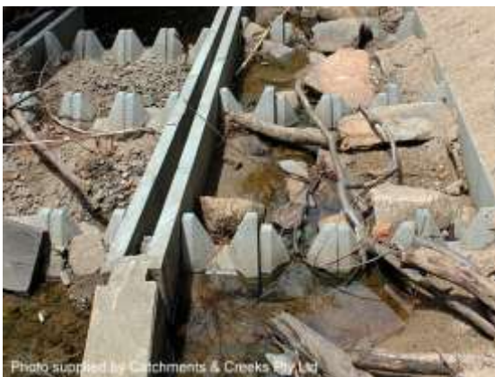
Sediment and boulders in a fishway
