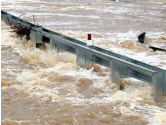
Floodwater passing under a guardrail
