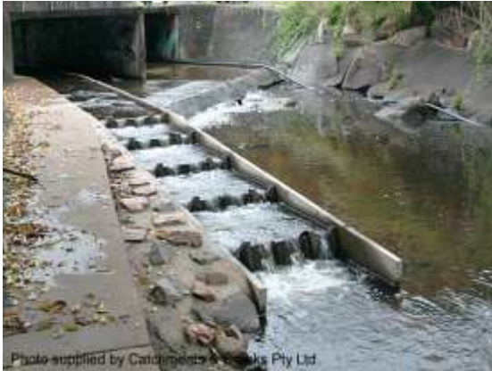
Pre-cast concrete fishway (Qld)
