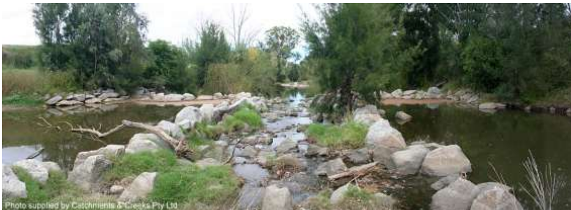
Rock ramp fishway looking downstream from the top of the fishway (Tamworth, NSW)
