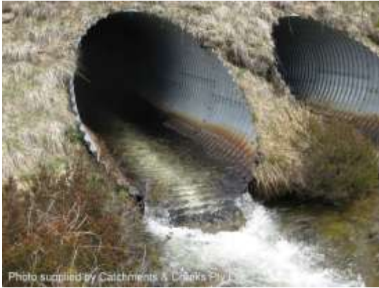
Culvert with drop-outlet
