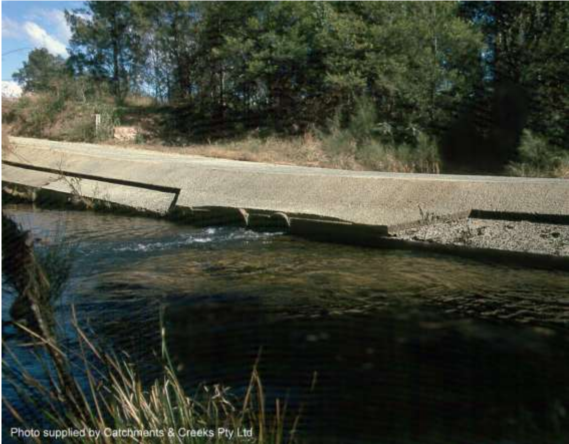
Old Ewingar Creek culvert, Ewingar, NSW (2000)
