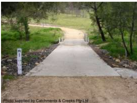
New culvert crossing (NSW)
