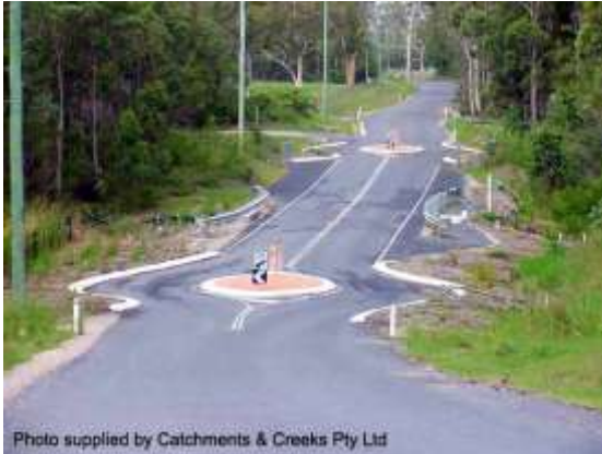
Traffic calming on a rural road (Qld)
