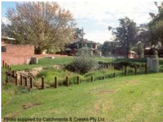
Safety poles (NSW)
