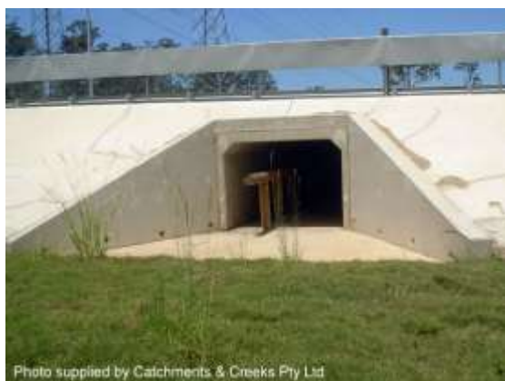
Fauna culvert (Qld)
