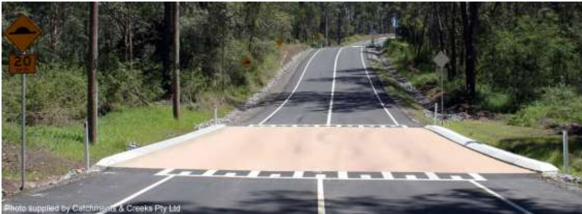
Traffic calming speed bump (Qld)
