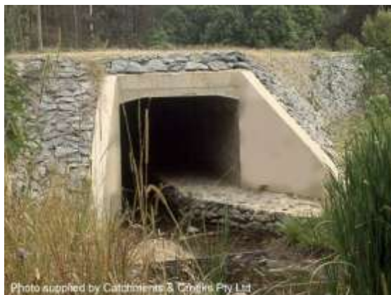
Single cell waterway culvert (Qld)
