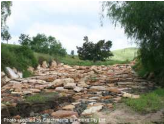
Rock chute stabilising gully erosion (Qld)
