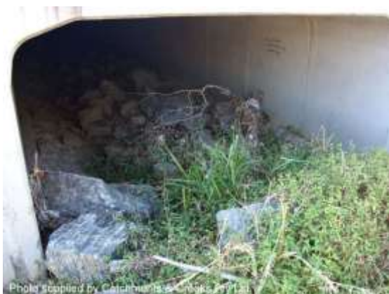
Deposition of large rocks at culvert inlet
