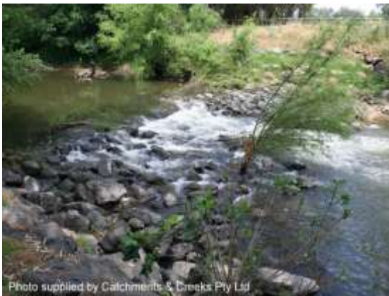
Constructed riffle (NSW)
