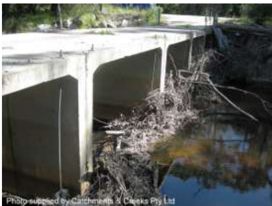
Rural, multi-cell box culvert (NSW)
