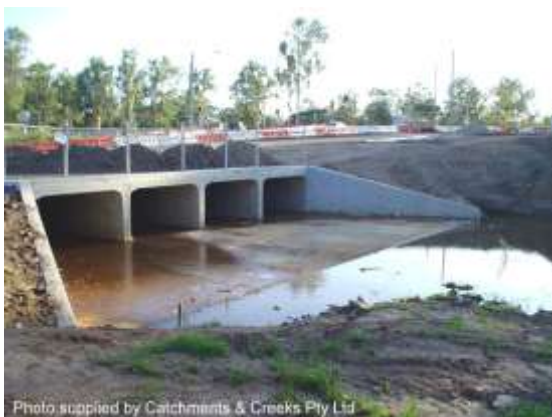
Concrete apron at culvert inlet
