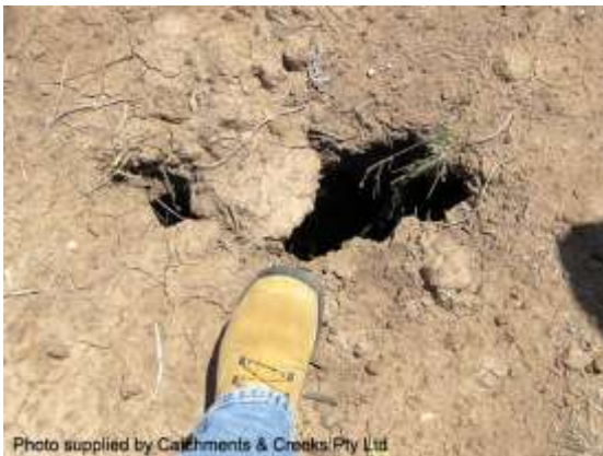
Deep rilling and tunnel erosion (Qld)
