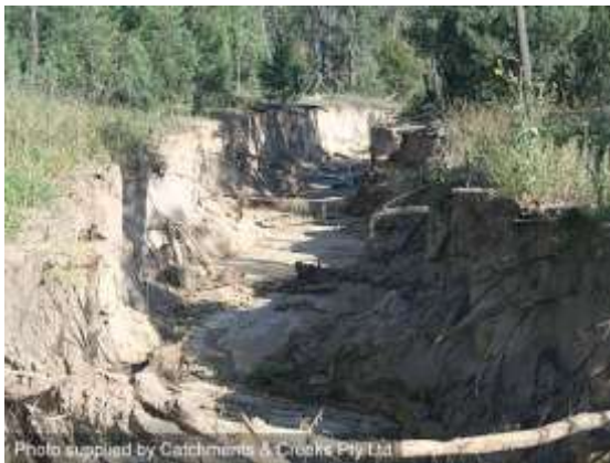
Gully erosion through a sandy soil (Qld)
