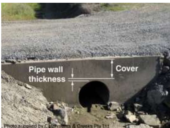
Small pipe culvert on a gravel road
