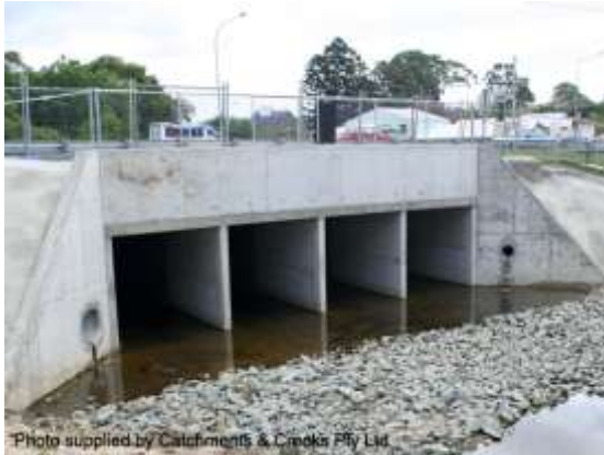
Box culvert with deep deck (Qld)
