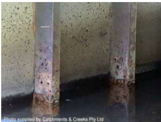
Rusted sidewall baffles (NSW)
