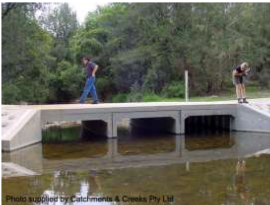
Backwater passing through a culvert
