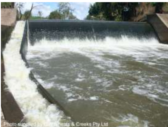
Fish ladder adjacent to a weir (Qld)
