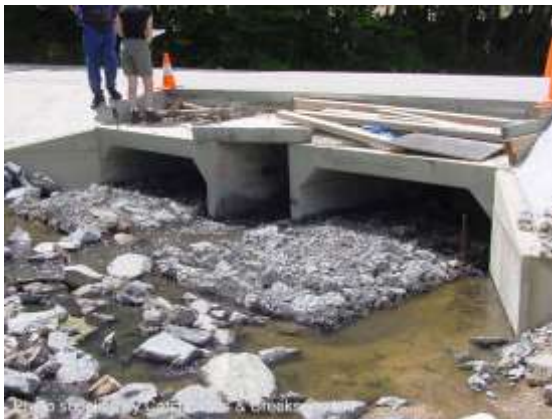
New culvert during construction (NSW)
