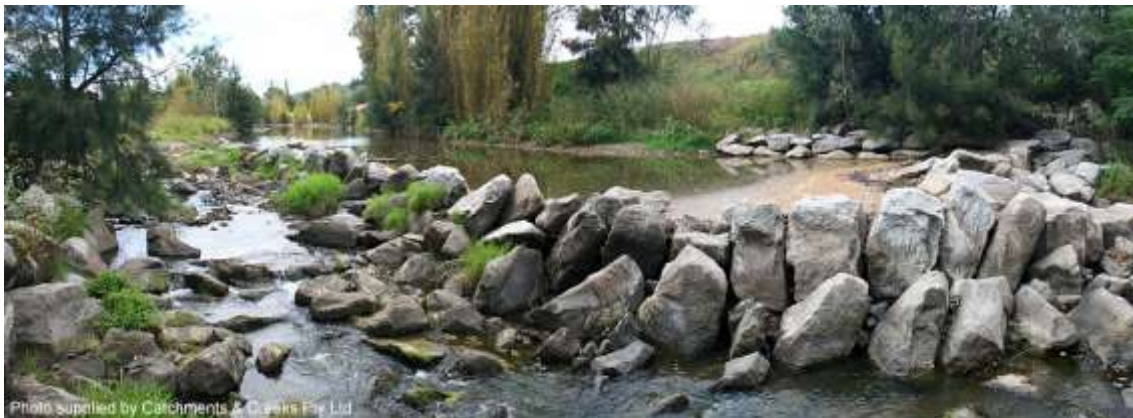
Rock ramp fishway looking upstream from the base of the fishway (Tamworth, NSW)
