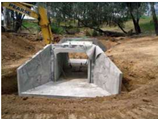
Culvert with wingwalls under construction
