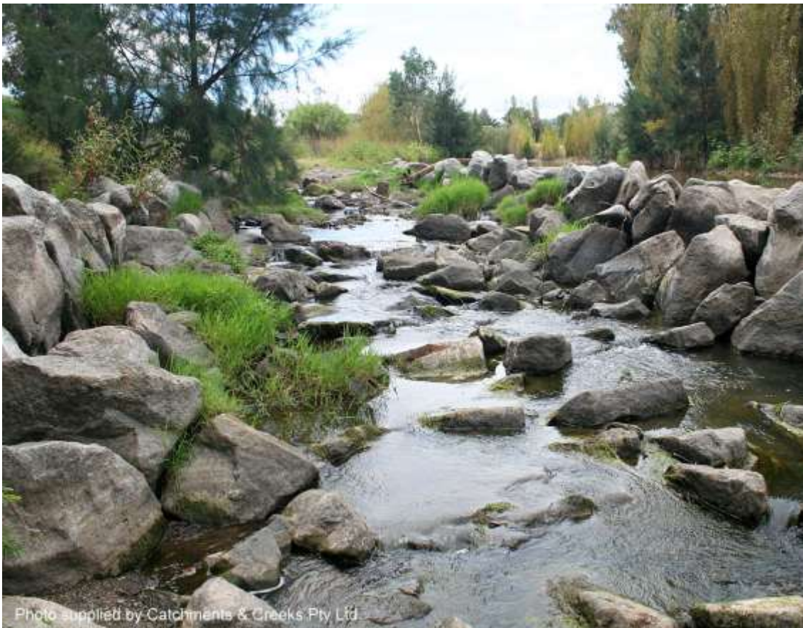
Constructed rock ramp (fishway) in Tamworth, NSW
