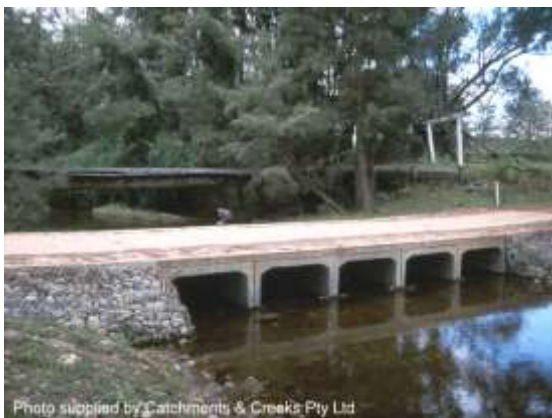
Recessed box culvert
