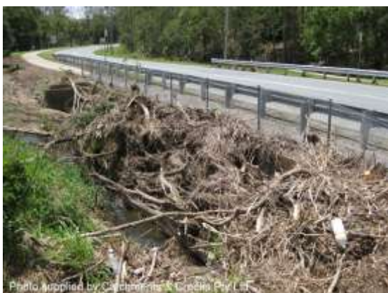
High level of debris blockage
