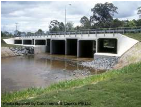
A culvert containing both wet and dry cells
