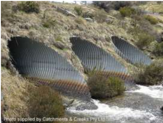
Corrugated pipe culvert (NSW)
