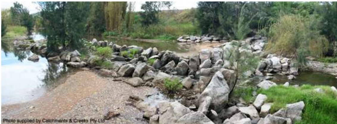
Rock ramp fishway viewed from the right bank (Tamworth, NSW)
