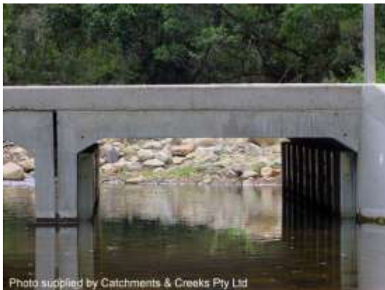
Countersunk box culvert
