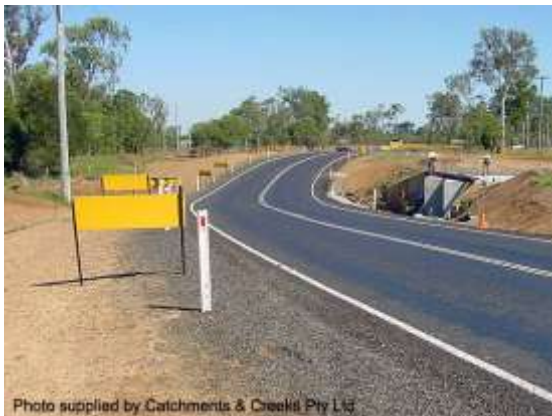
Culvert upgrade as part of road works
