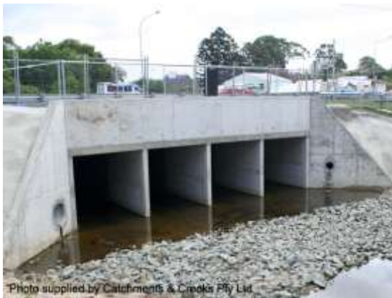
Multi-cell box culvert
