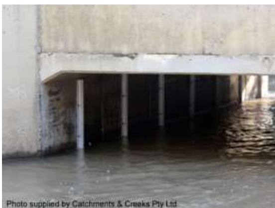
Introduced sidewall baffles (Qld)
