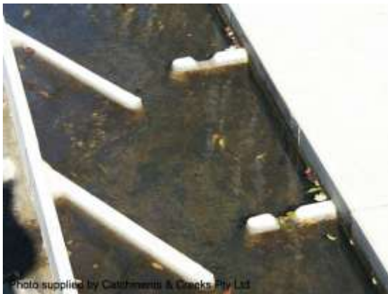
Floor baffles in the fishway (Qld)
