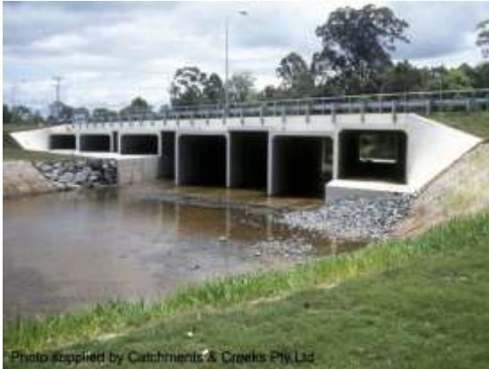
A culvert containing both wet and dry cells
