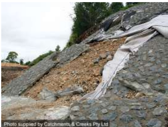
Flood damage to grouted stone-pitching
