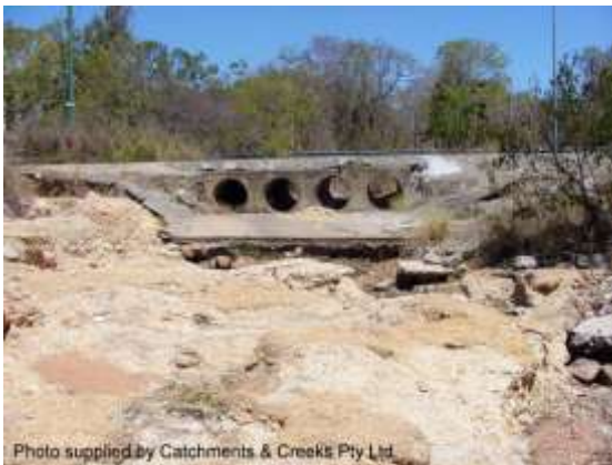
Culvert with elevated apron
