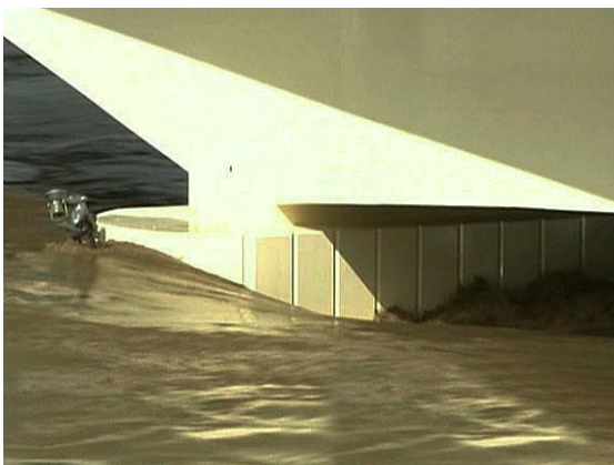
Subcritical flow around a bridge pier
