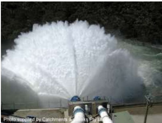
Water supply dam outlet structure
