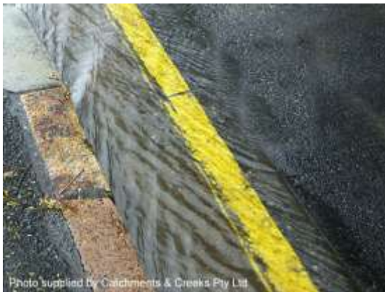
Photo supplied by Catchments & Creeks Pty Ltd Supercritical kerb flow
