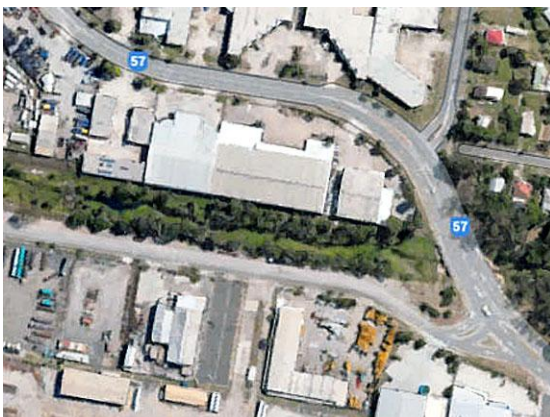
A relocated waterway channel (Q1d)
