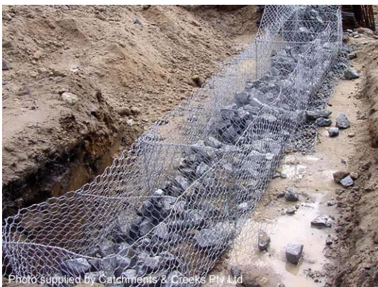
Gabions (during construction)
