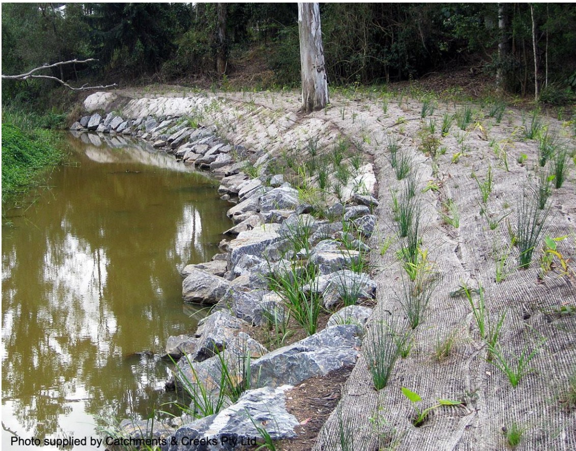
Vegetated rock placement, Kedron Brook, upstream of Ferny Way, Brisbane, Qld
