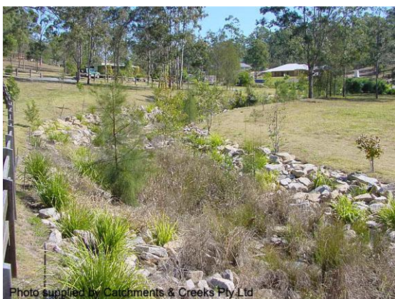
A newly-constructed drainage channel
