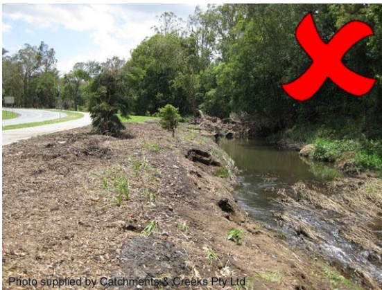
Excessive weed removal
