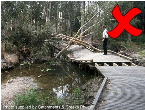
failed boardwalk crossing a creek
