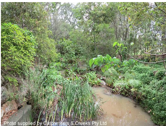
Fully constructed drainage channel (Qld)
