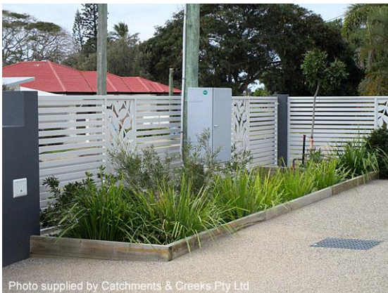
Stormwater retention basin (Qld)
