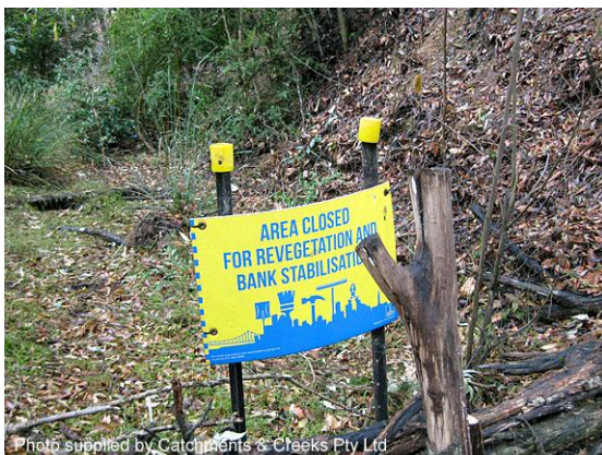
Access to bush regeneration site (Qld)
