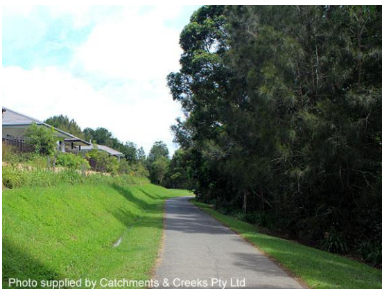
Benched floodway (Qld)
