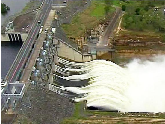
Flood-control dam (Qld)
