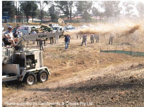
Straw mulcher with bitumen spray
