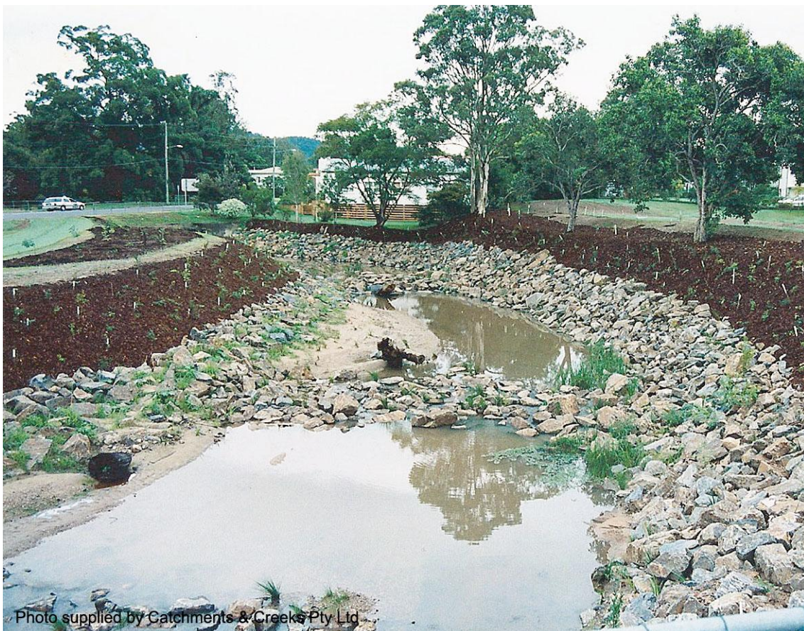
Channel expansion for drainage improvement and flood mitigation works (1997)
