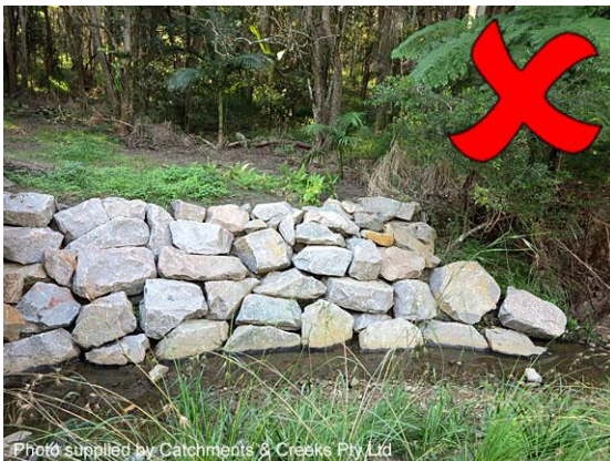
Open-void rock work can attract weeds
