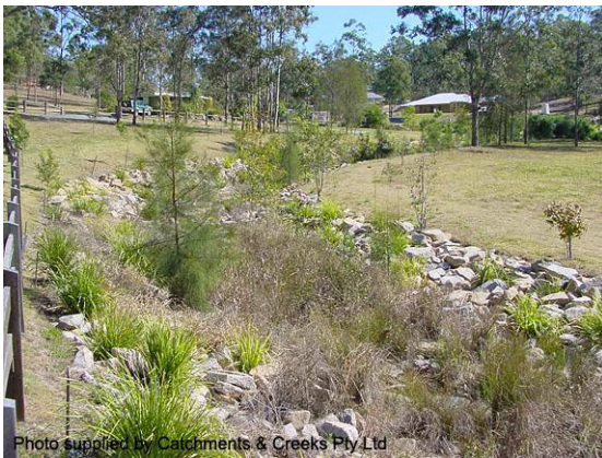
Constructed drainage channel (Qld)
