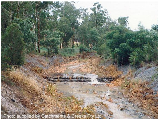
Weed control of rock mattresses (Qld)
