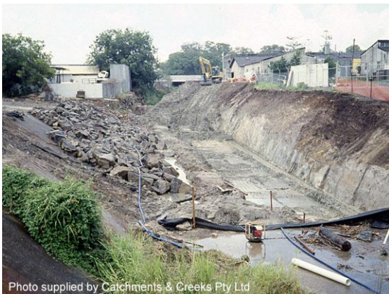
Channel expansion (Qld)
