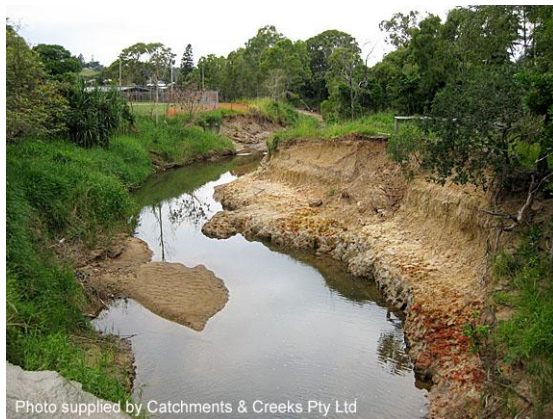
Bed and bank scour (Qld)
