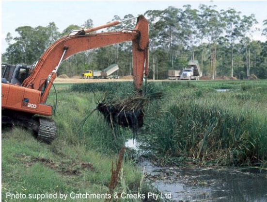
Channel maintenance (Qld)
