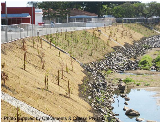
Rehabilitation of an eroded creek bank
