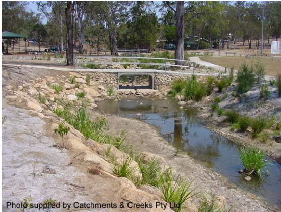
Constructed drainage channel (Qld)
