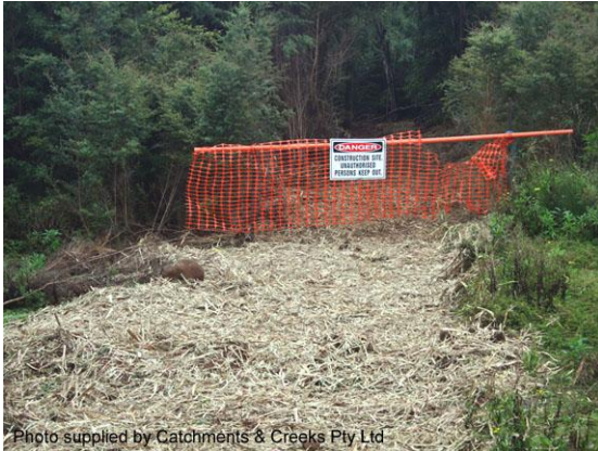
Restoration of a site access pathway
