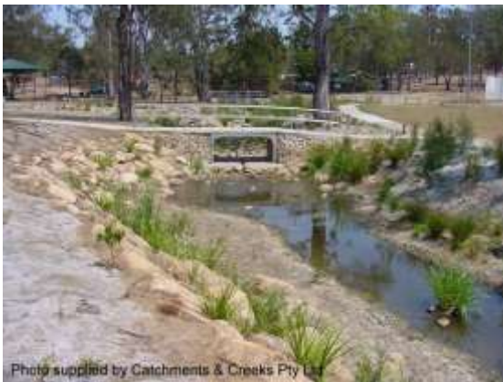
Constructed drainage channel (Qld)
