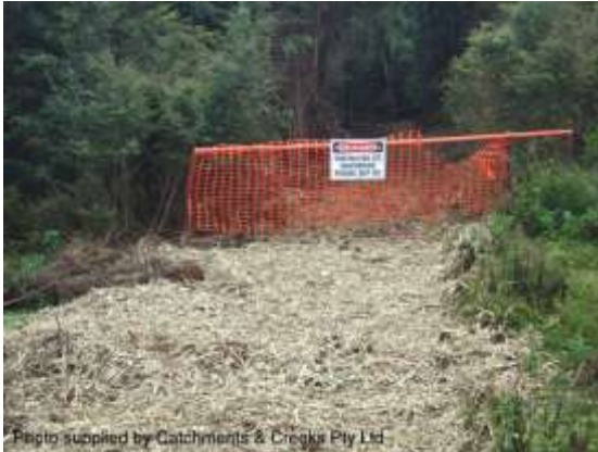
Restoration of a site access pathway
