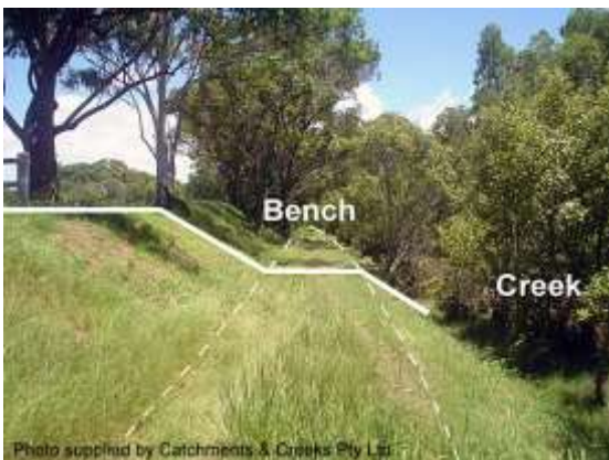
Benching a waterway bank (Qld)
