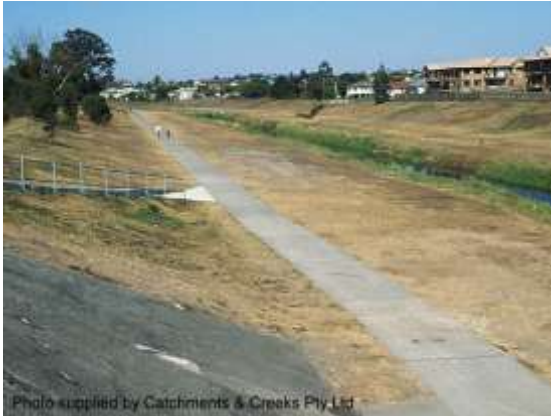
A section of widened channel (Qld)
