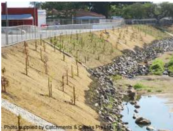
Rehabilitation of an eroded creek bank
