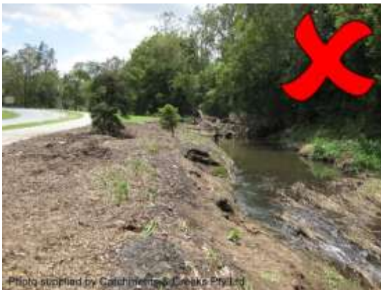
Excessive weed removal
