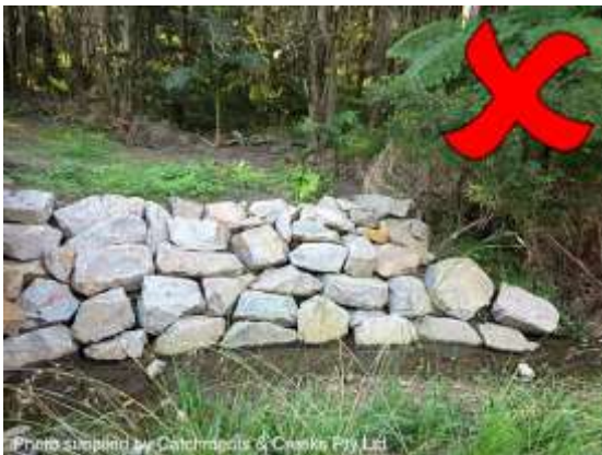
Open-void rock work can attract weeds
