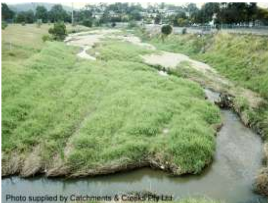
Sediment deposition in a widened channel
