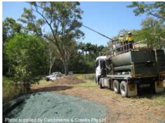
Hydromulcher (Bonded Fibre Matrix)
