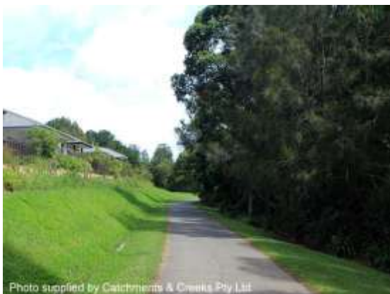
Benched floodway (Qld)
