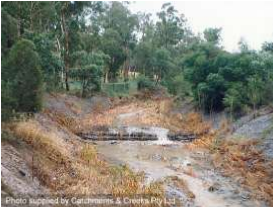
Weed control of rock mattresses (Qld)
