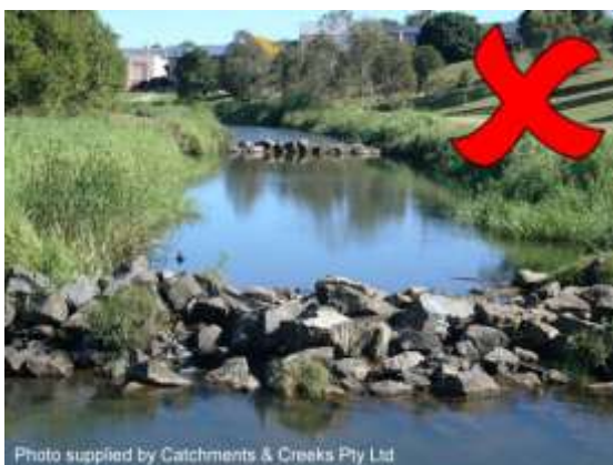
Problematic rock riffles (weirs)
