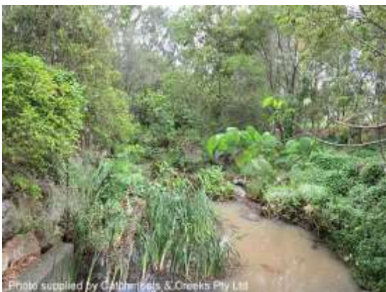
Fully constructed drainage channel (Qld)
