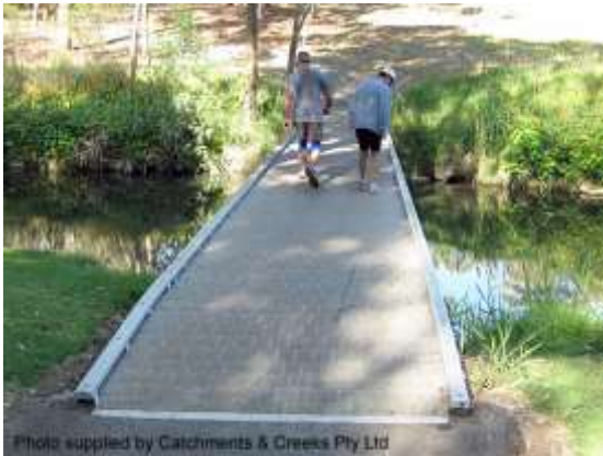
Low-level footbridge (SA)
