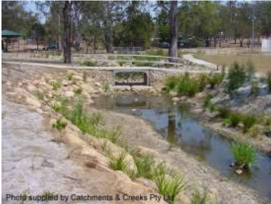
Constructed drainage channel (Qld)
