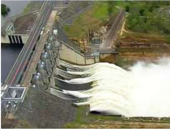
Flood-control dam (Qld)
