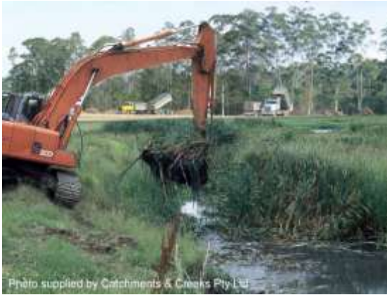
Channel maintenance (Qld)
