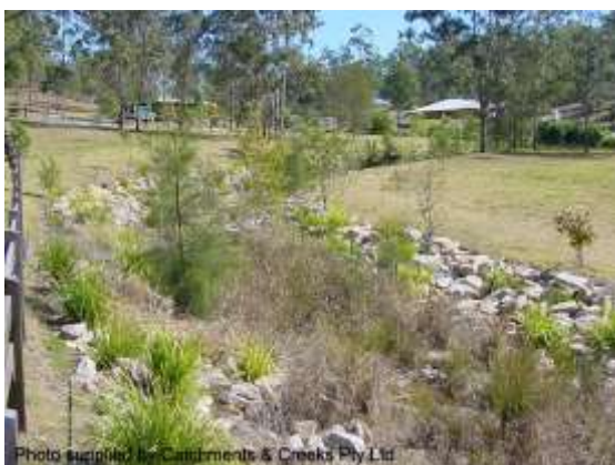
A newly-constructed drainage channel
