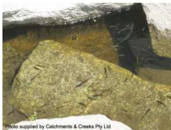
Open voids in rocks below water level
