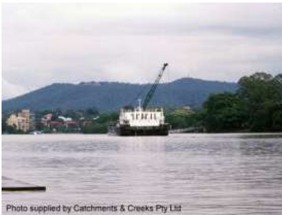
River dredging (Qld)
