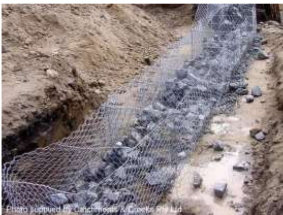
Gabions (during construction)
