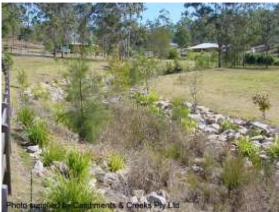
Constructed drainage channel (Qld)
