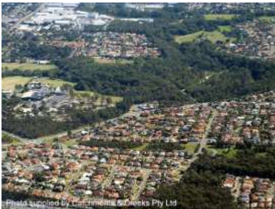
A modified drainage catchment (Qld)
