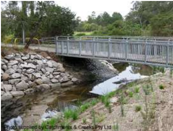
High-level footbridge (Qld)
