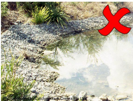
A rock mattress-lined sediment pond!
