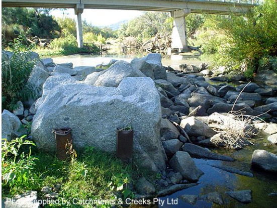
Habitats formed by placement of boulders
