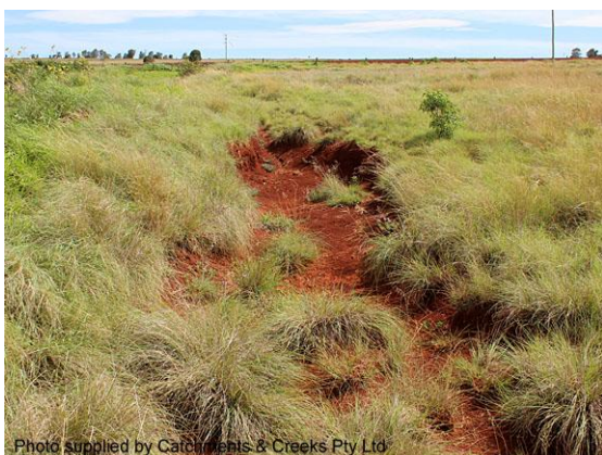
Scour along an overland flow path (Qld)
