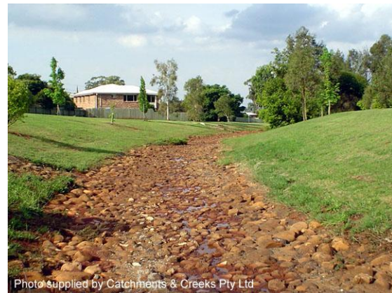
Grouted rock low-flow (Qld)
