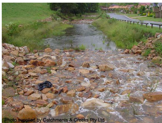
Constructed riffle (Qld)
