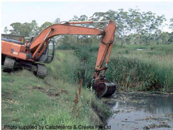
Channel maintenance (de-silting)
