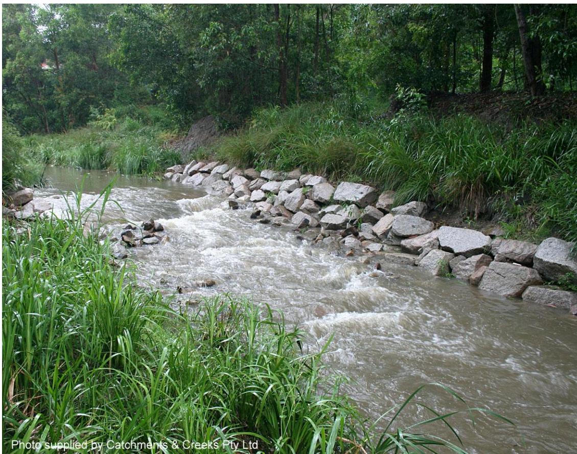
Constructed riffle (Qld)
