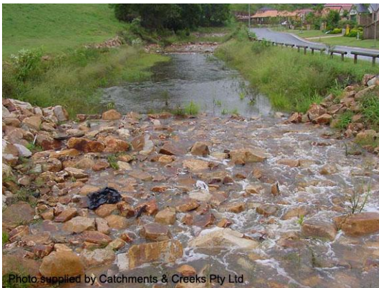
Constructed rock riffle (Qld)
