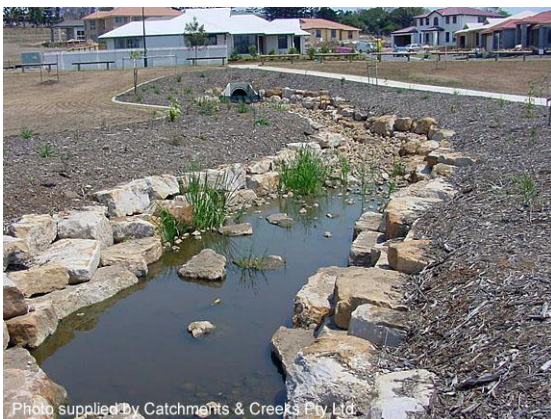
Rock-lined low-flow channel (Qld)
