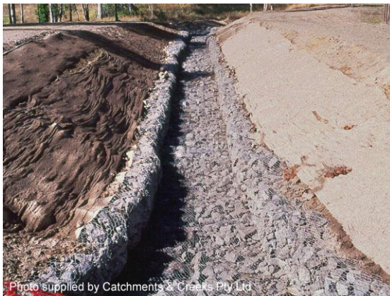
Gabion-lined low-flow channel (Qld)
