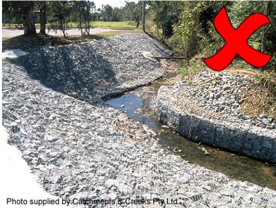
Rock mattress lined channel (Qld)
