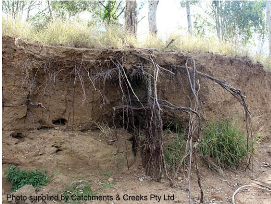
Bank undercutting (Qld)
