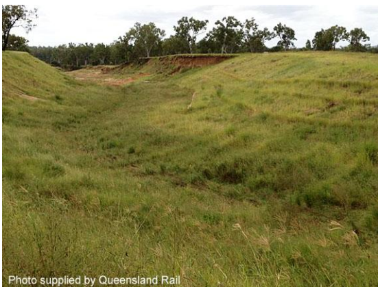
Gully stabilisation with vetiver grass (Qld)
