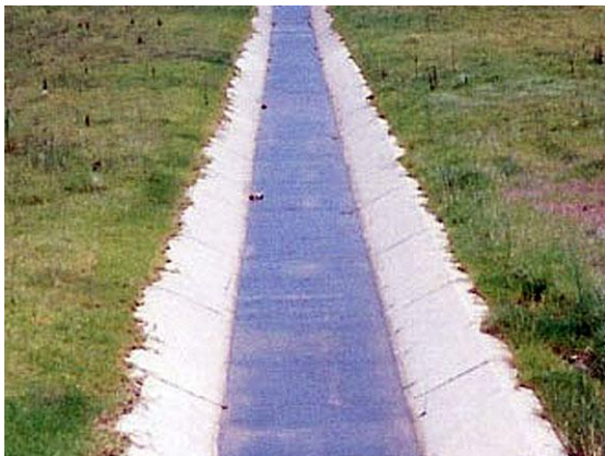
Concrete-lined low-flow channel (NSW)
