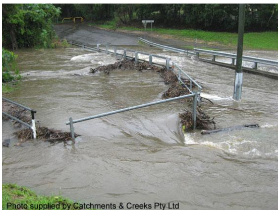
Backwater effects of a culvert crossing
