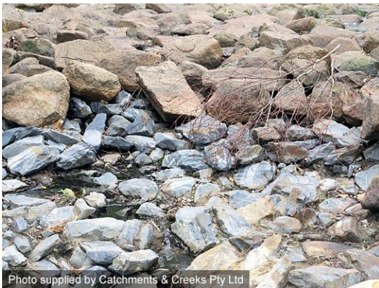
Rock filter layer (blue) under surface rock
