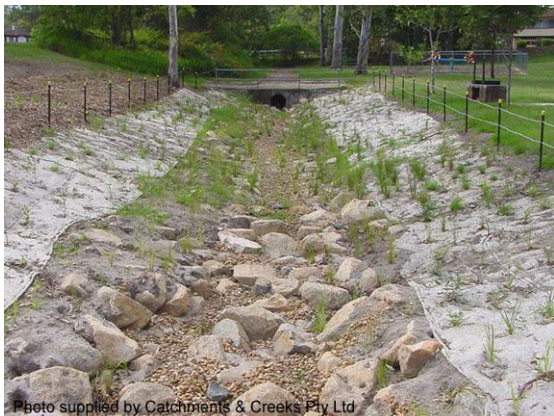
Vegetated drainage channel in 2001 (Qld)
