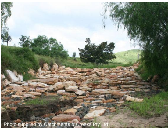
Non-fish-friendly drop structure (Qld)
