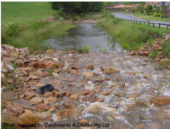
Constructed riffle (Qld)
