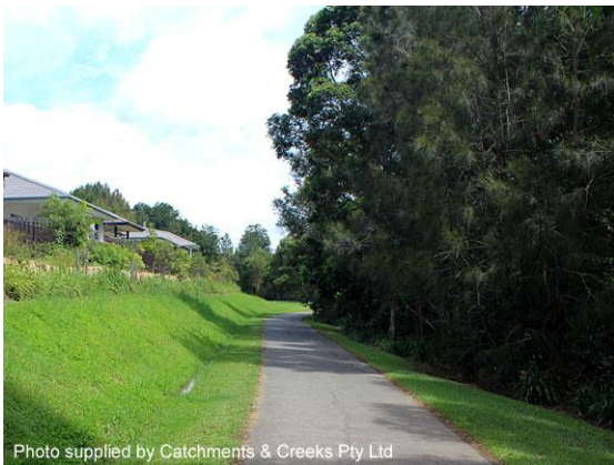
Constructed floodway (Qld)
