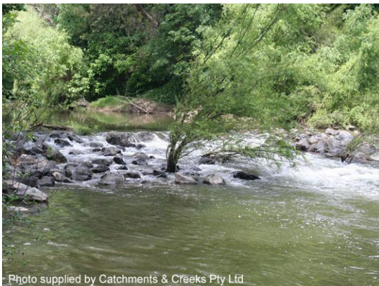
Constructed rock ramp/chute (NSW)
