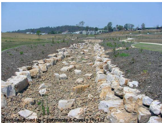
Rock-lined low-flow channel (Qld)
