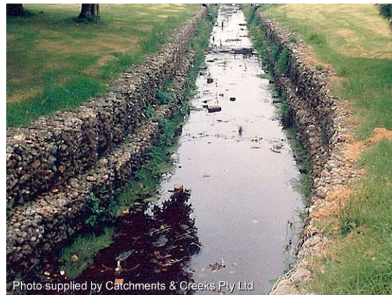
Gabion-lined low-flow channel (NSW)
