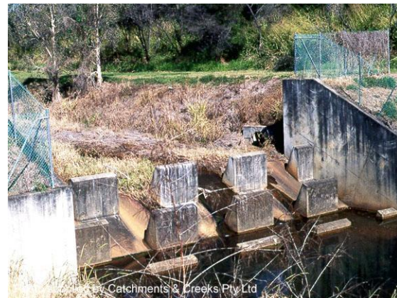
Baffled drop structures (Qld)
