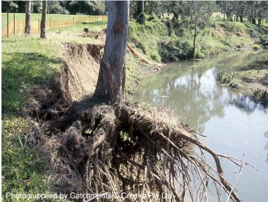
Exposed tree roots (Qld)
