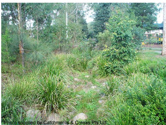
The above drainage channel in 2005
