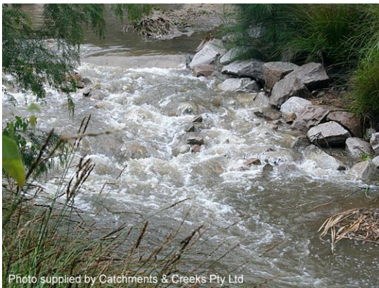
Constructed rock chute (Qld)
