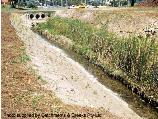
Maintenance of a drainage channel
