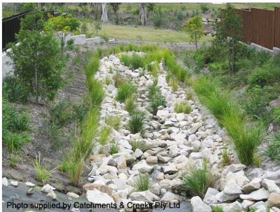
Rock-lined low-flow channel (Qld)
