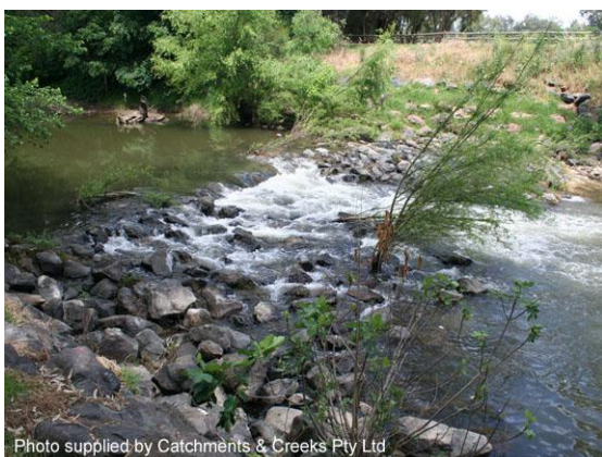
Constructed riffle (NSW)
