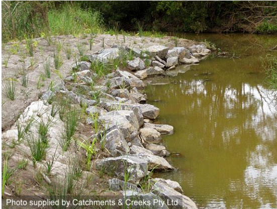
Vegetated rock stabilisation of bank (Qld)
