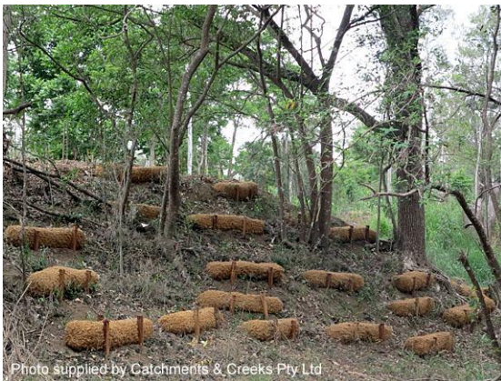
Geo logs used on a steep creek bank
