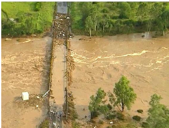
Flow conditions just below the bridge deck
