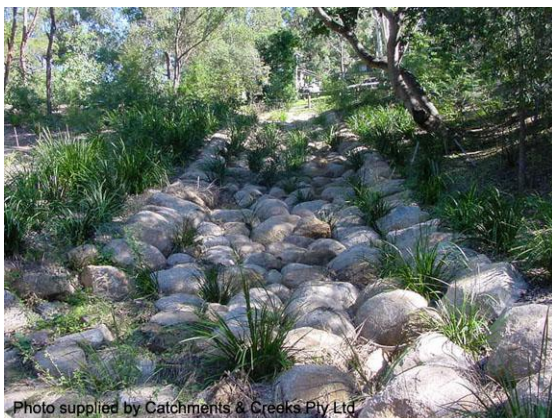
Partially-vegetated batter chute (Qld)
