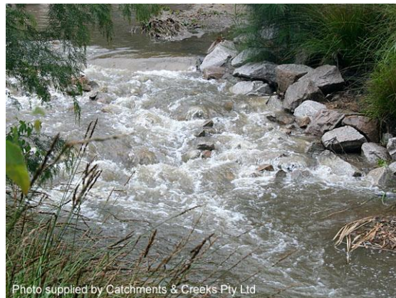
Constructed rock chute (Qld)
