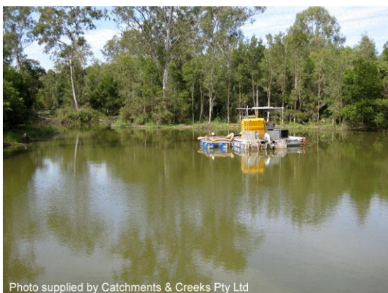
Lake maintenance (dredging)
