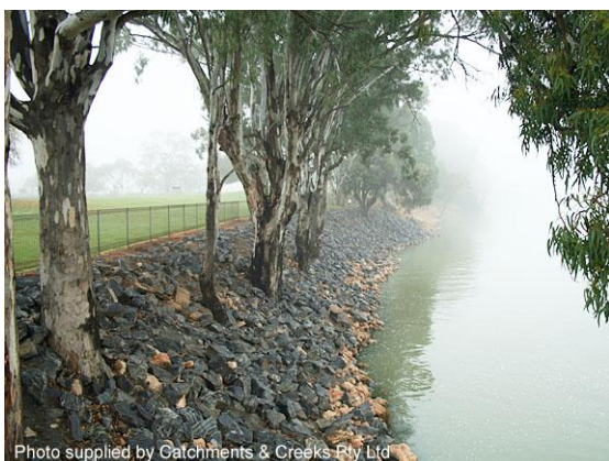
Rock stabilisation of a river bank (NSW)
