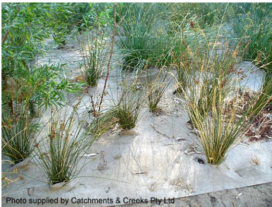
Jute erosion control blanket (SA)
