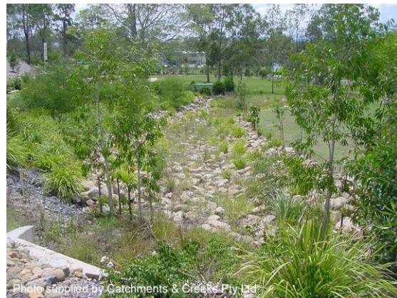
Rock-lined low-flow channel (Qld)
