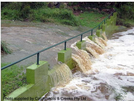
Vertical drop structure (Qld)
