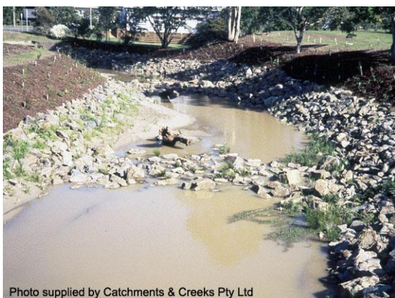
Constructed rock riffle (Qld)
