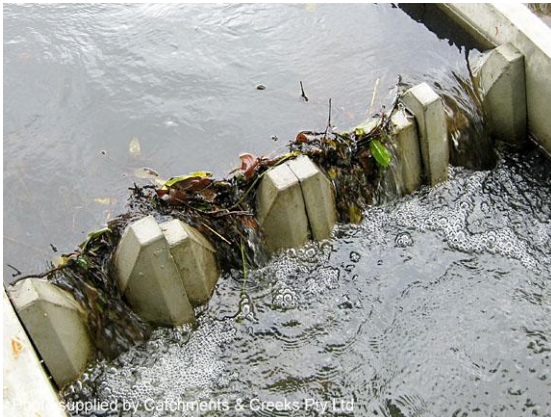
Debris blockage of fishway (Qld)
