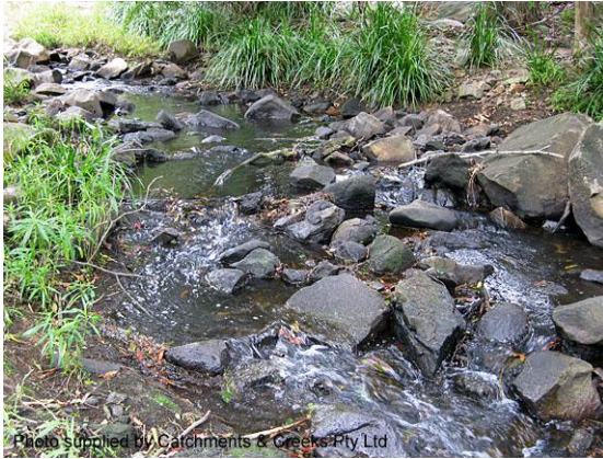
Constructed riffle in a clay-based creek
