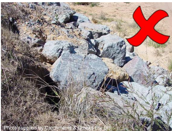
Erosion under rocks on a dispersive soil
