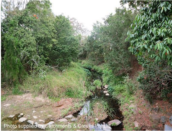
Earth-lined low-flow channel (Qld)
