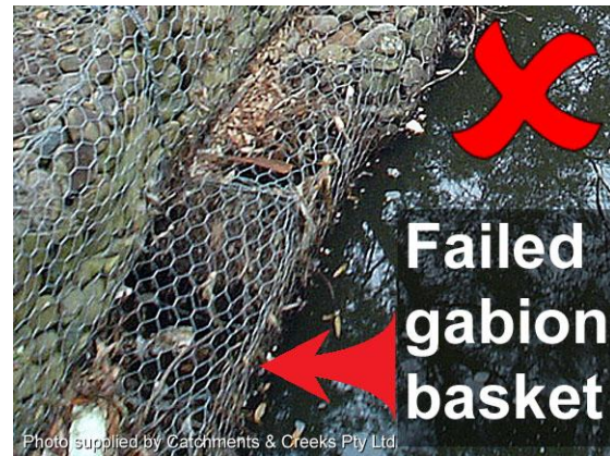
Failed basket in adjacent channel image
