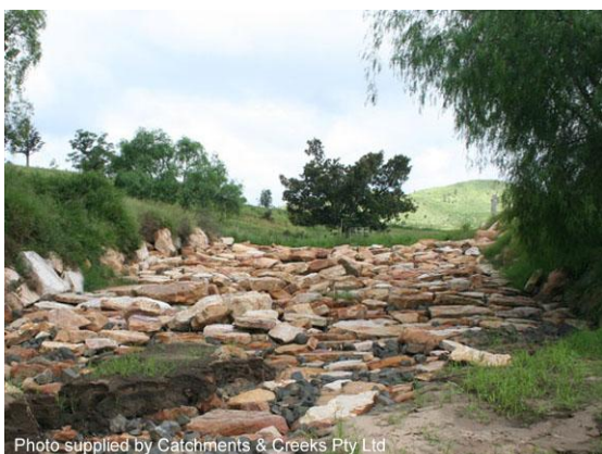
Rock chute stabilising gully erosion (Qld)
