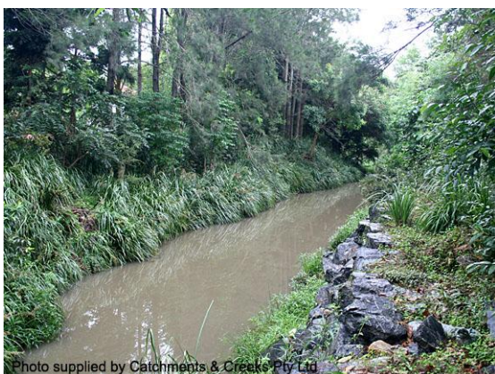
Fully established creek bank (2010)
