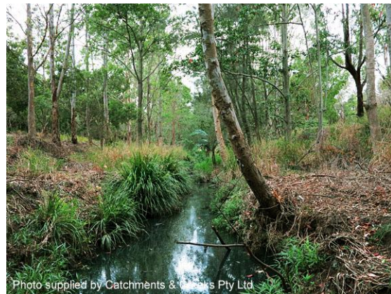
Earth-lined low-flow channel (Qld)
