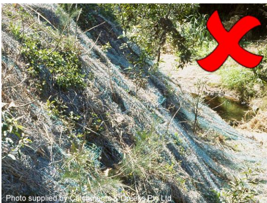
Plastic-reinforced erosion control mat
