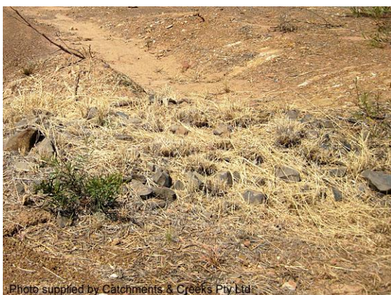
Recessed rock check dams (NT)
