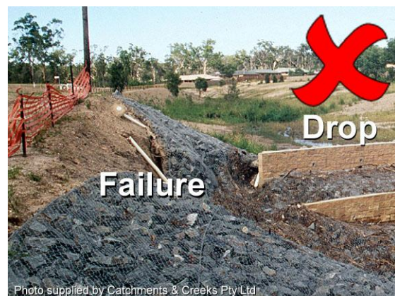
Open channel drop structure (Qld)
