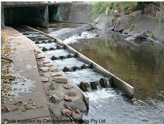
Constructed fishway (Qld)
