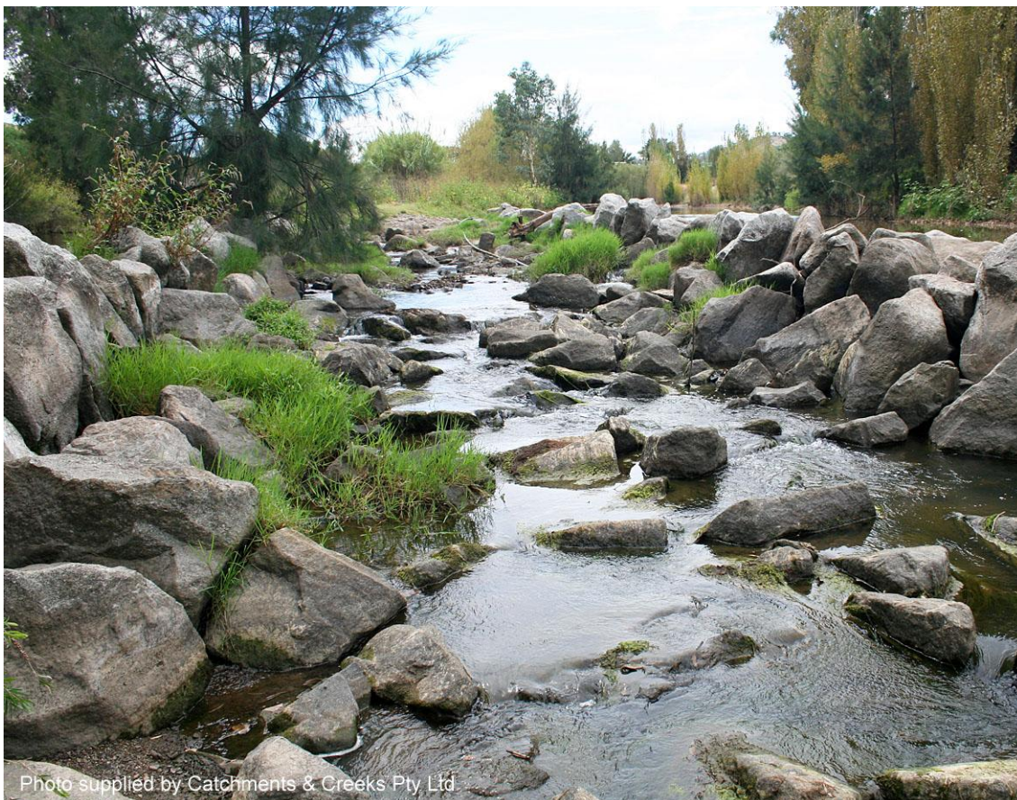
Constructed rock ramp (fishway) in Tamworth, NSW
