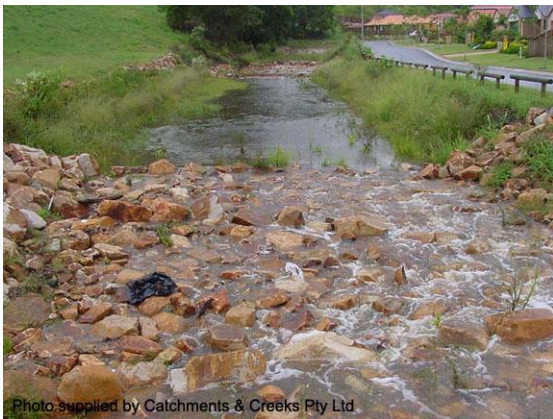
Constructed riffle (Qld)
