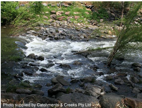
Constructed rock chute (NSW)
