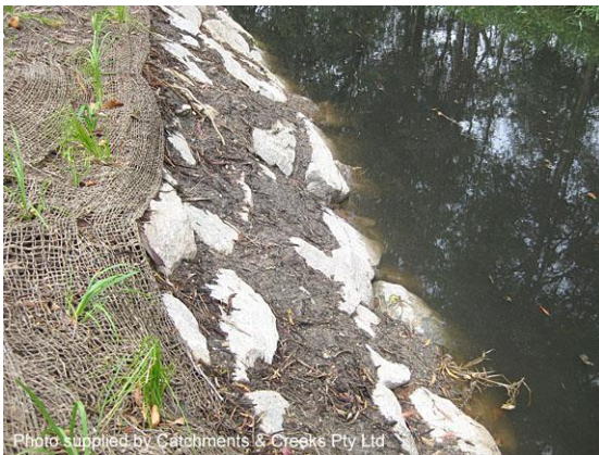
Voids filled with soil ready for planting
