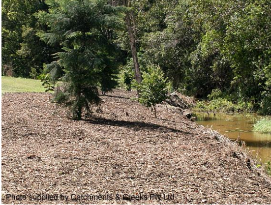
Loose mulch applied to a creek bank
