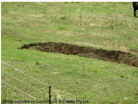
Lateral bank erosion (NSW)
