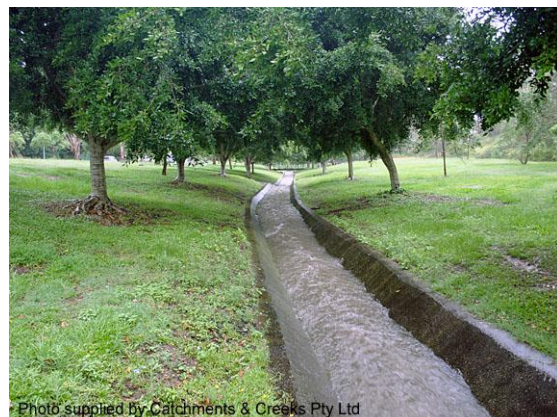
Concrete low-flow channel (Qld)
