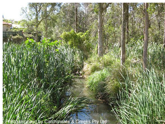
Vegetated low-flow channel (Qld)
