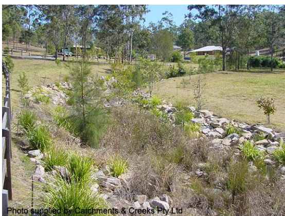
Vegetated drainage channel (Qld)
