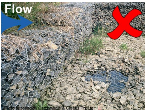
Open channel drop structure (NSW)
