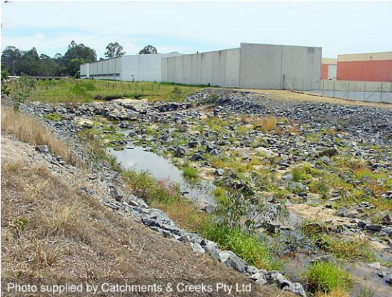
Energy dissipation basin at base of chute
