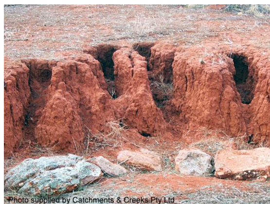
Erosion of a dispersive soil (NSW)
