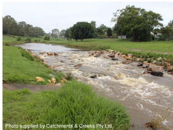
Constructed riffle (Qld)
