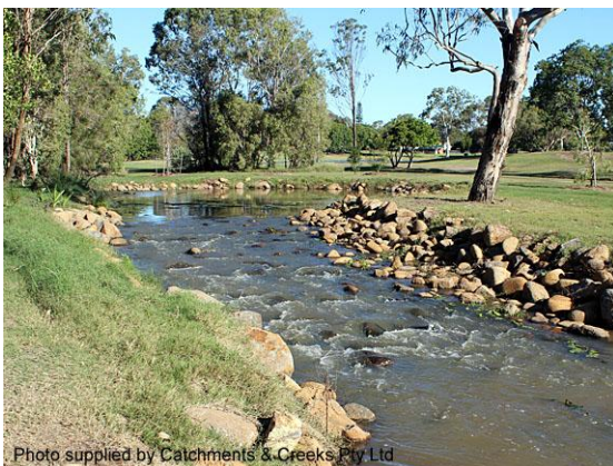
Fish-friendly rock ramp (Qld)
