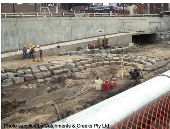
Channel construction (USA)
