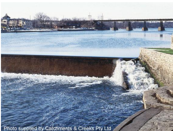
Fish ladder on a river weir (USA)
