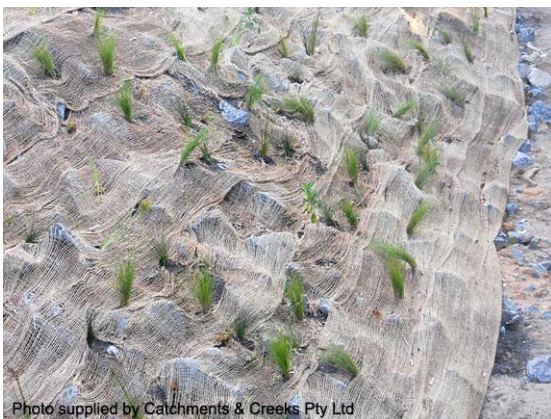
Planted rock covered with jute mesh
