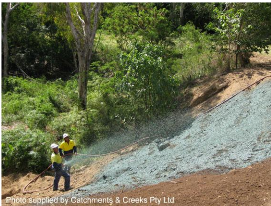
Hydraulically-applied blanket (Qld)
