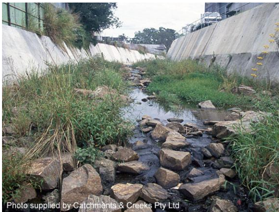
Rocks grouted to concrete floor of drain
