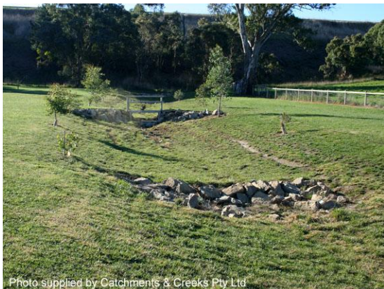
Recessed rock check dams (SA)
