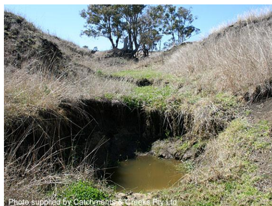
Scour along an overland flow path (Qld)
