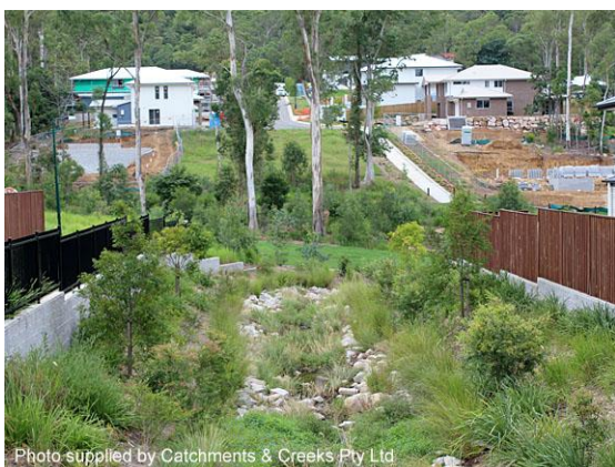
Vegetated drainage channel (Qld)
