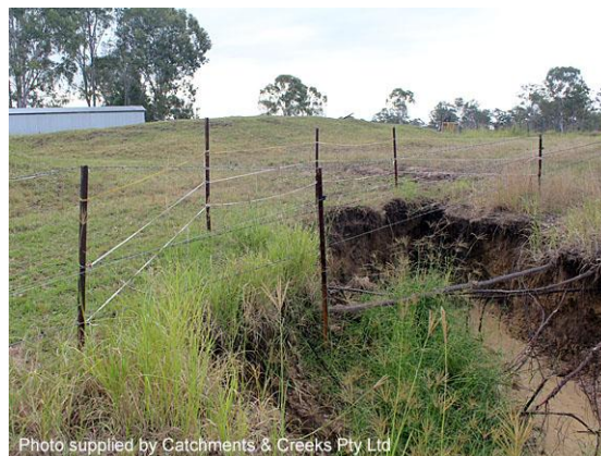
Erosion downstream of a farm dam (Qld)
