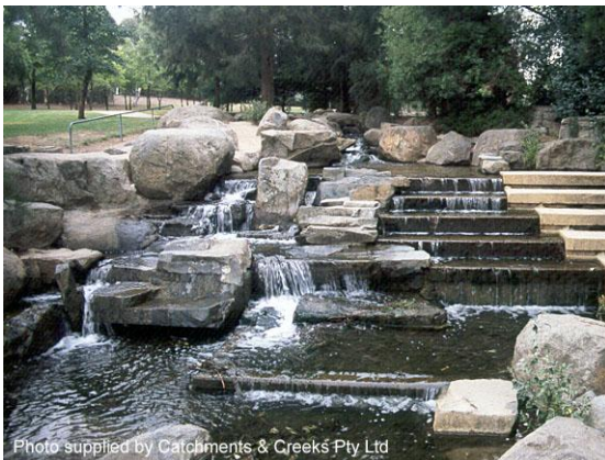
Stepped drop structure (ACT)
