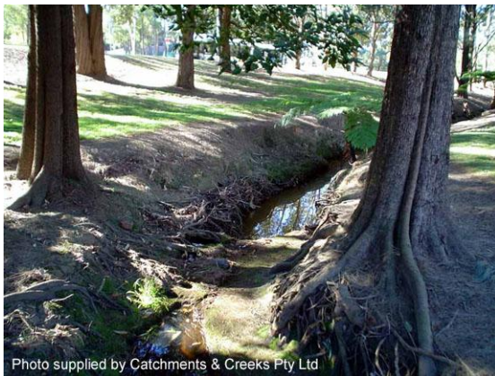
Earth-lined low-flow channel (Qld)
