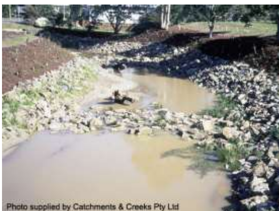
Photo supplied by Catchments & Creeks Pty Ltd Constructed rock riffle (Qld)
