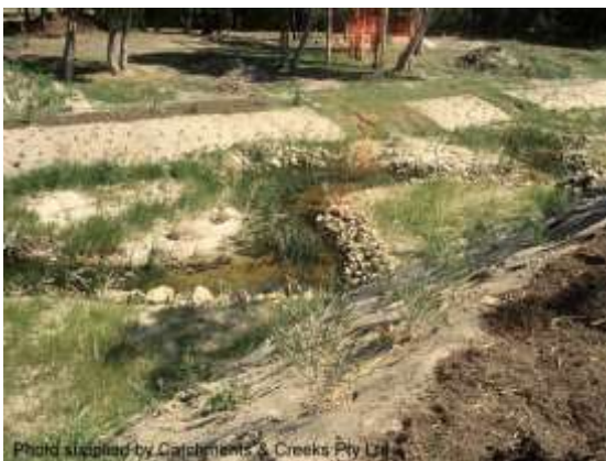
Meandering low-flow channel (Qld)
