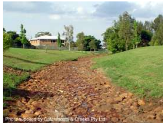
Grouted rock low-flow (Qld)
