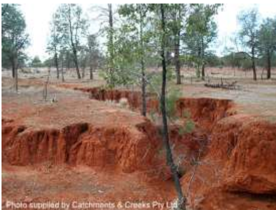
Erosion of a dispersive soil (NSW)
