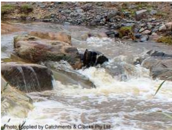
Constructed rock riffle (Qld)
