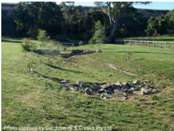
Photo supplied by Catchments & Creeks Pty Ltd Recessed rock check dams (SA)
