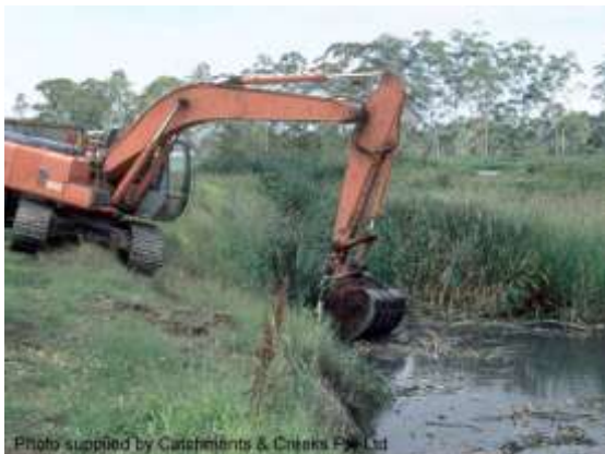
Channel maintenance (de-silting)
