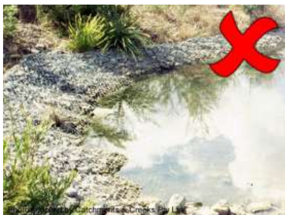
A rock mattress-lined sediment pond!
