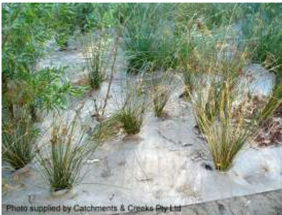
Jute erosion control blanket (SA)
