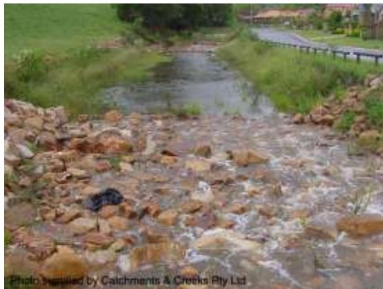
Constructed riffle (Qld)
