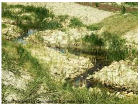
Meandering low-flow channel (Qld)
