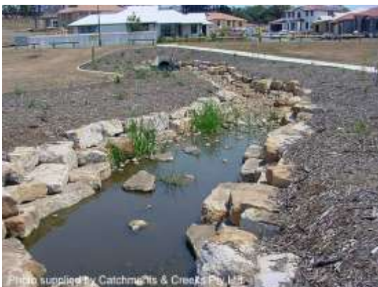
Rock-lined low-flow channel (Qld)
