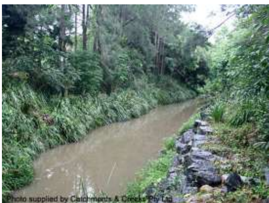
Fully established creek bank (2010)
