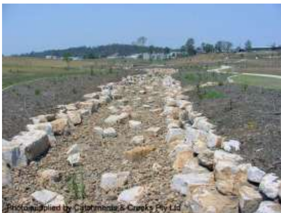
Rock-lined low-flow channel (Qld)
