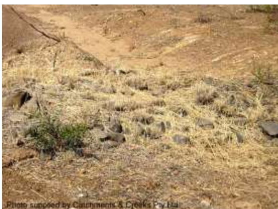
Photo supplied by Catchments & Creeks Pty Ltd Recessed rock check dams (NT)
