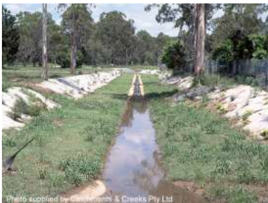
Concrete low-flow channel (Qld)
