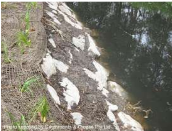
Voids filled with soil prior to planting (Qld)
