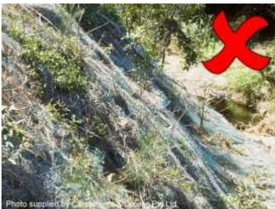
Plastic-reinforced erosion control mat
