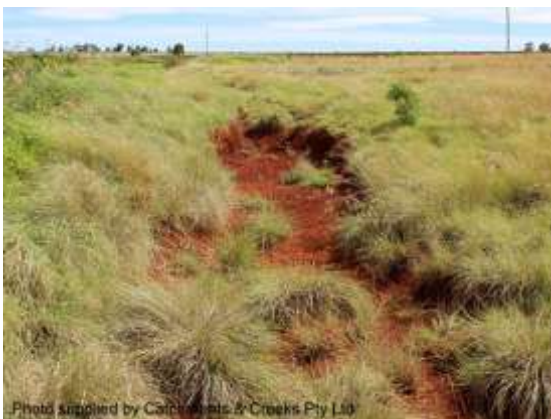
Scour along an overland flow path (Qld)
