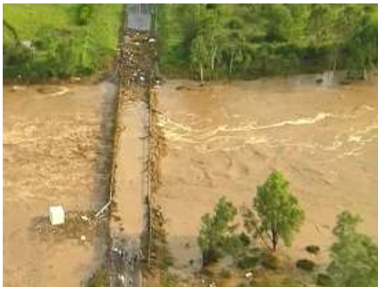
Flow conditions just below the bridge deck
