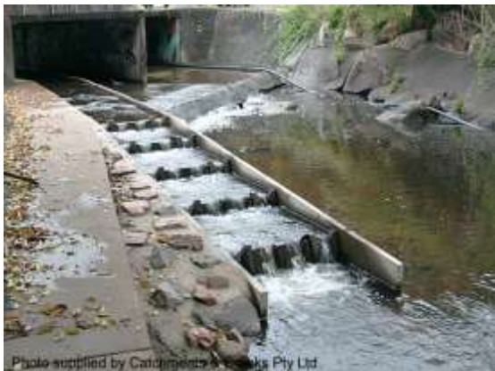
Precast concrete fishway (Qld)
