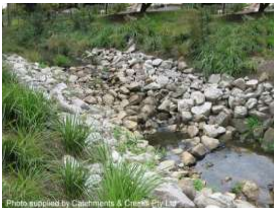
Pool-riffle in a narrow channel (Qld)
