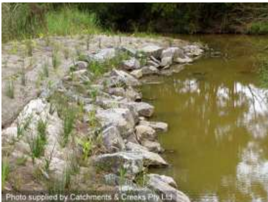
Vegetated rock stabilisation (Qld)
