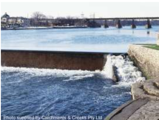
Fish ladder on a river weir (USA)
