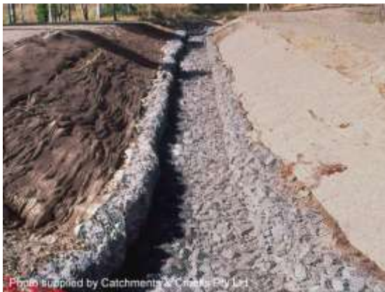
Gabion-lined low-flow channel (Qld)
