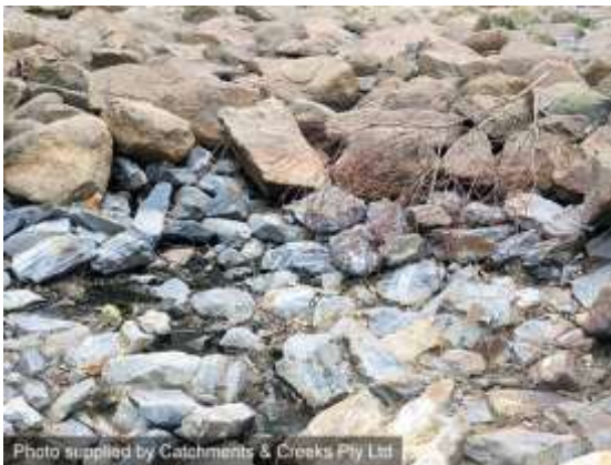
Rock filter layer (blue) under surface rock
