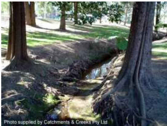
Earth-lined low-flow channel (Qld)
