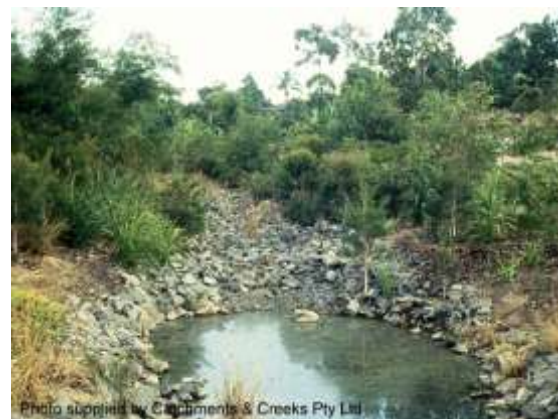
Example of constructed plunge pool
