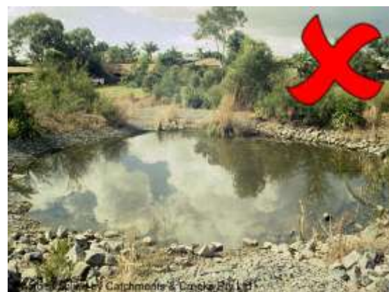
Mattress-lined in-stream pond (Qld)
