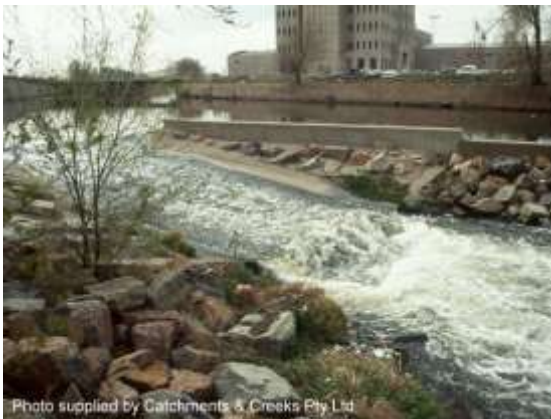
Inclined drop structure (USA)
