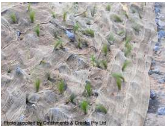
Planted rock covered with jute mesh
