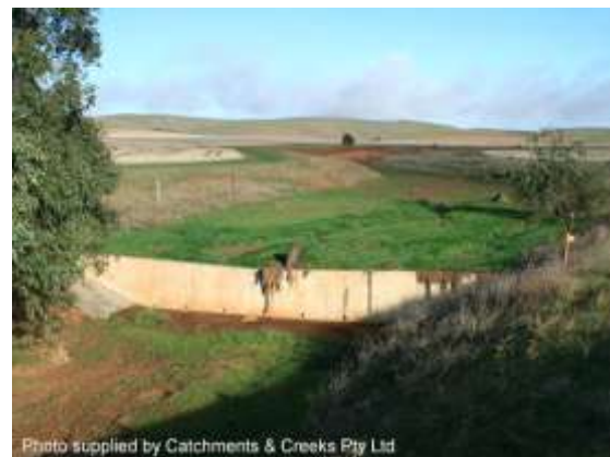
Vertical drop structure (SA)
