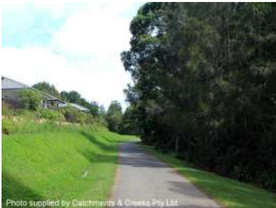
Maintenance berm (Qld)
