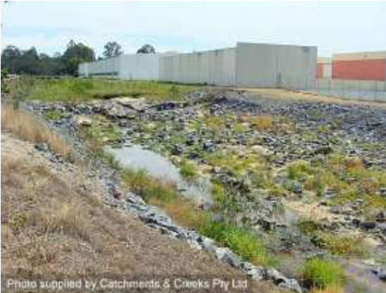
Energy dissipation basin at base of chute
