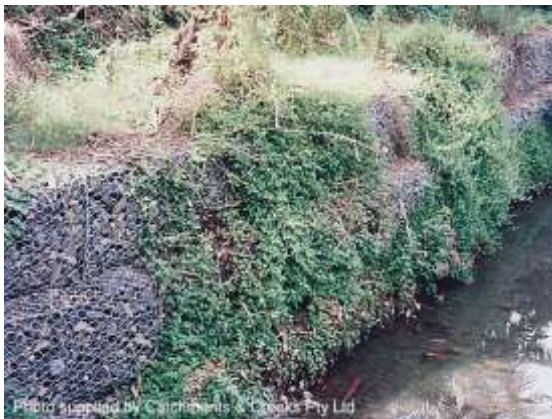
Vines begin to cover gabions (NSW)
