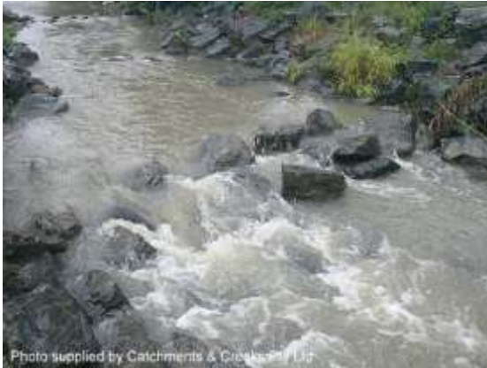
Rock sitting high with exposed edges
