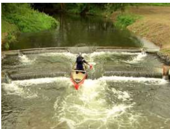
Concrete weirs (UK)
