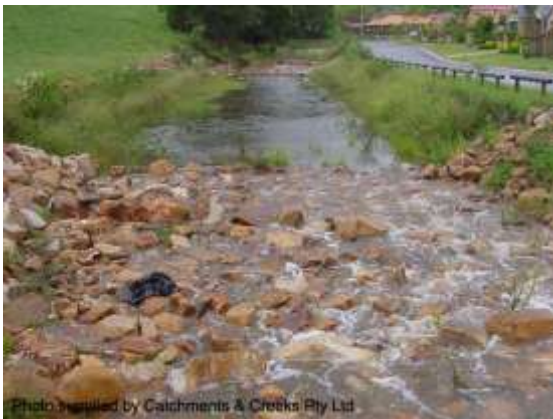
Constructed riffle (Qld)
