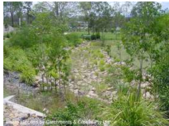
Rock-lined low-flow channel (Qld)
