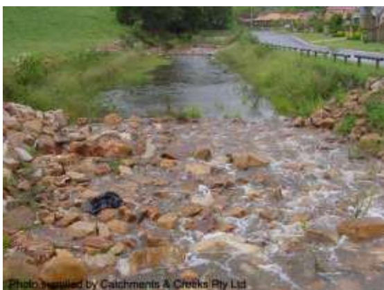
Constructed rock riffle (Qld)
