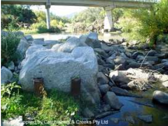
Habitats formed by placement of boulders
