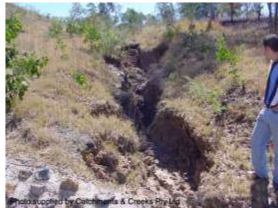
Lateral bank erosion (Qld)
