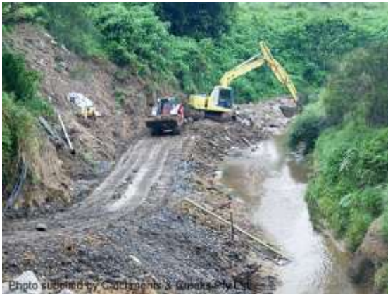
Equipment access (Qld)
