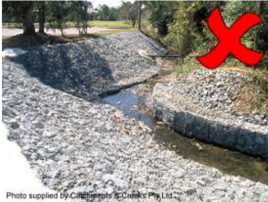
Rock mattress lined channel (Qld)
