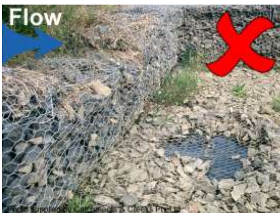
Open channel drop structure (NSW)
