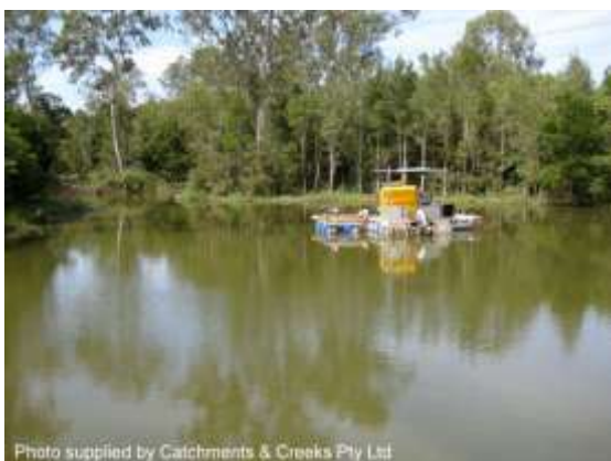
Lake maintenance (dredging)
