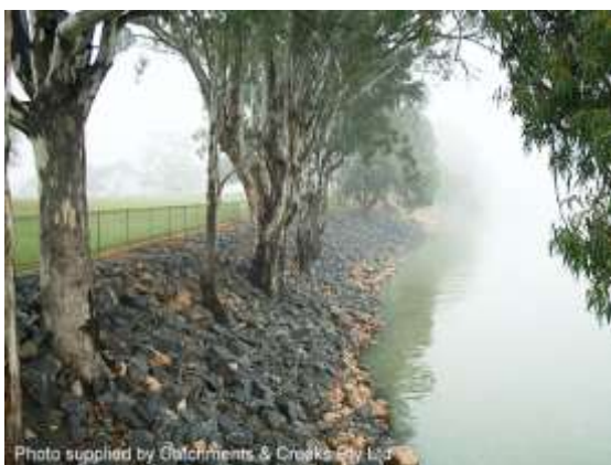
Rock stabilisation of a river bank (NSW)
