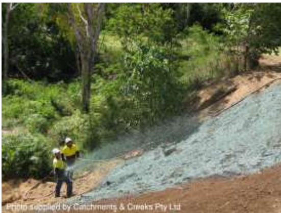
Hydraulically-applied blanket (Qld)
