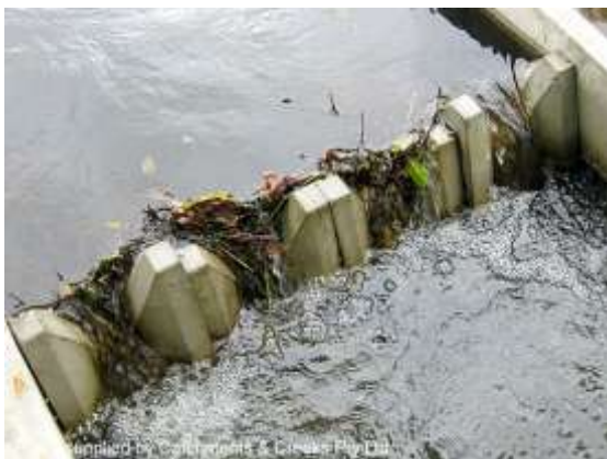
Debris blockage of fishway (Qld)
