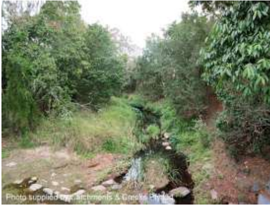
Earth-lined low-flow channel (Qld)
