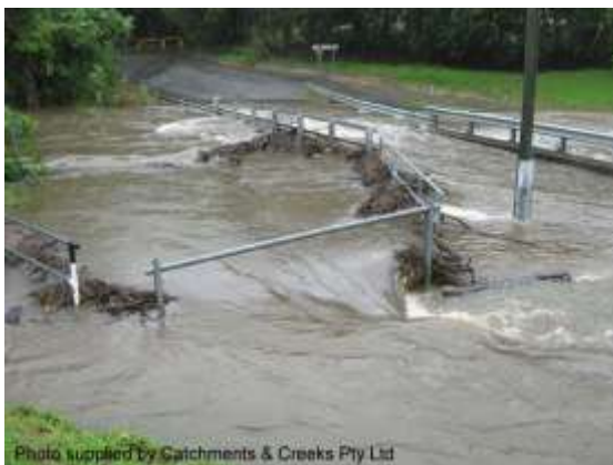
Backwater effects of a culvert crossing
