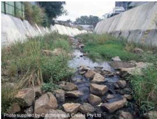
Rocks grouted to concrete floor of drain
