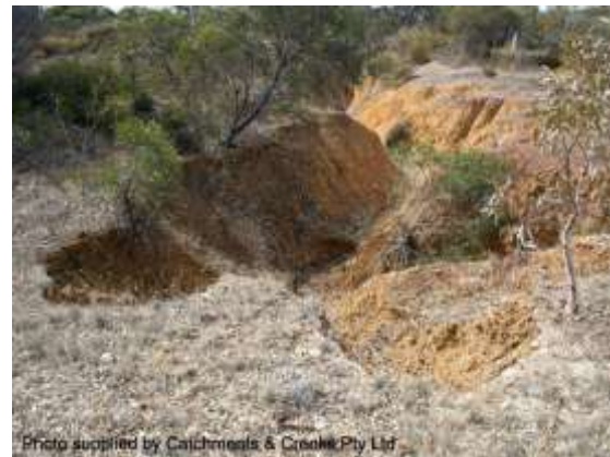
Lateral bank erosion (SA)
