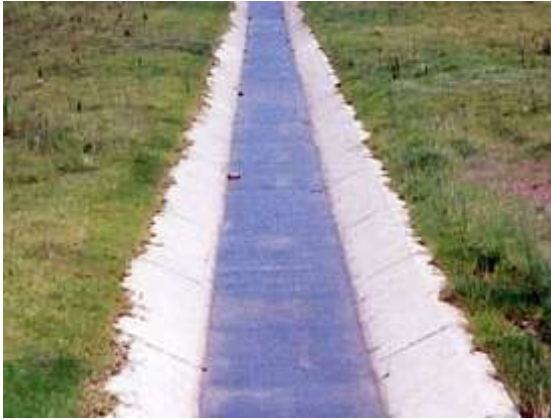
Concrete-lined low-flow channel (NSW)
