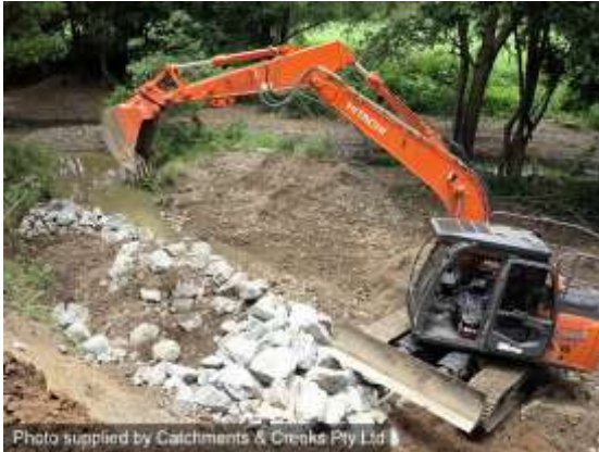
Bank stabilisation with rock (Qld)
