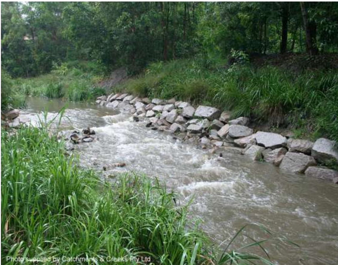
Constructed riffle (Qld)
