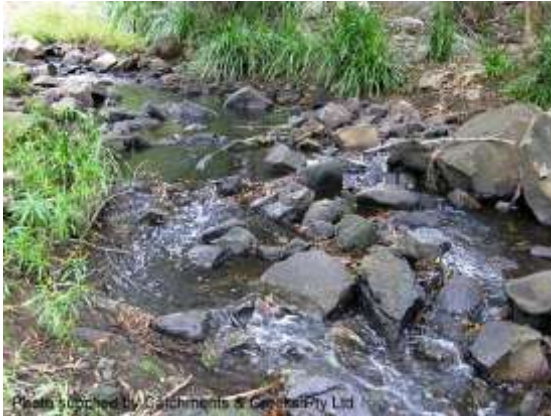
Constructed riffle in a clay-based creek
