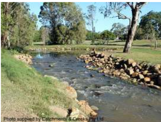
Fish-friendly rock ramp (Qld)
