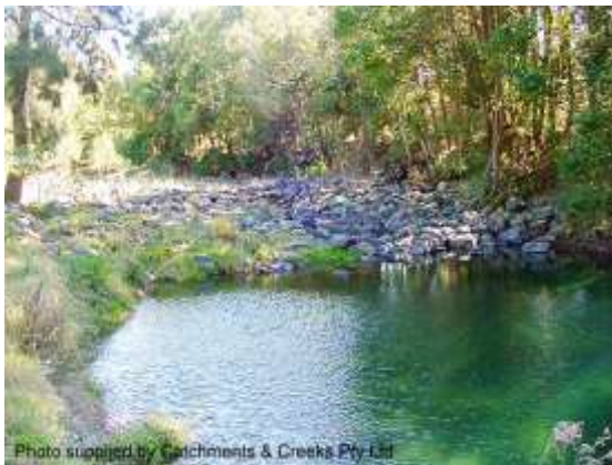
Pool downstream of a rock ramp (NSW)
