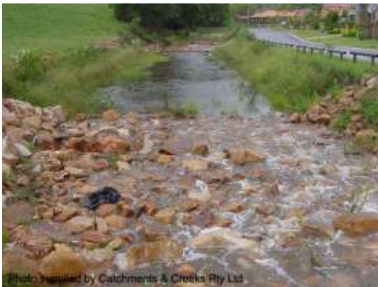
Constructed riffle (Qld)
