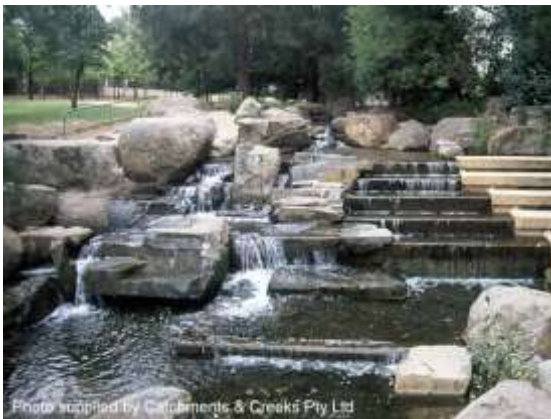
Stepped drop structure (ACT)
