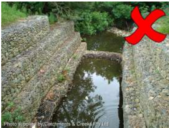
Gabion-lined channel (NSW)
