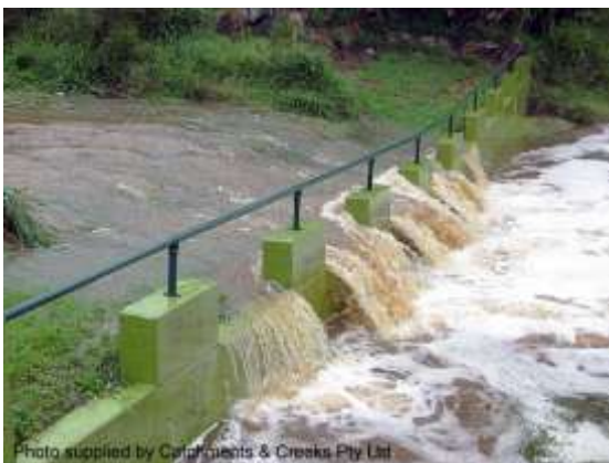
Vertical drop structure (Qld)
