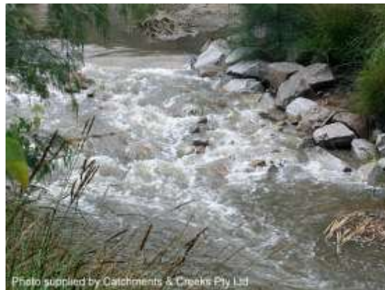
Constructed rock chute (Qld)
