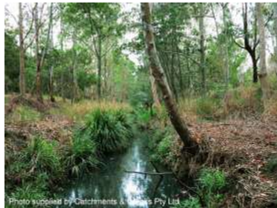
Earth-lined low-flow channel (Qld)
