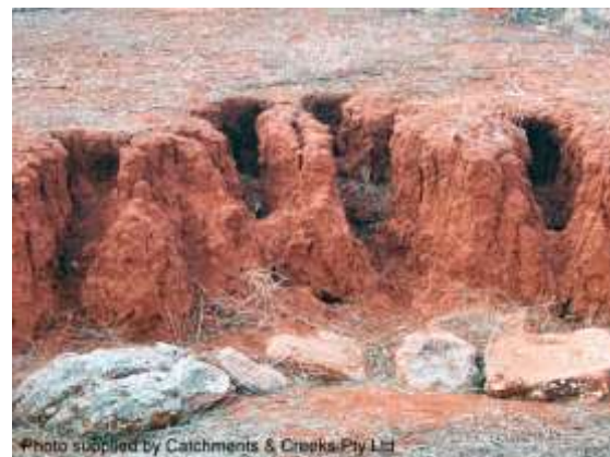
Erosion of a dispersive soil (NSW)
