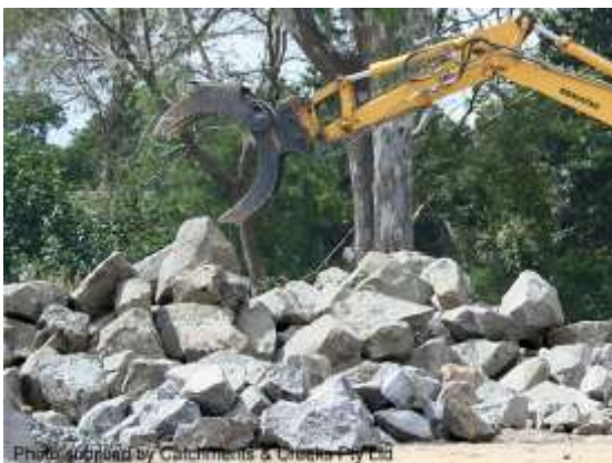
Large fractured rock (Qld)
