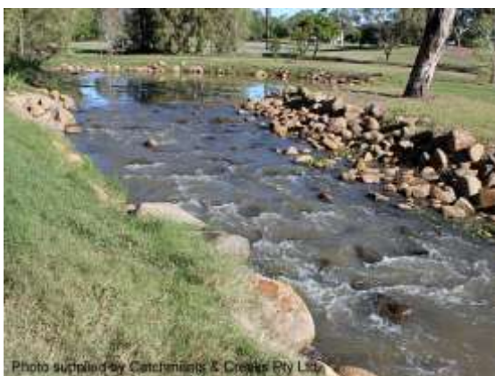
Rock ramp fishway (Qld)
