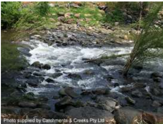
Constructed rock chute (NSW)
