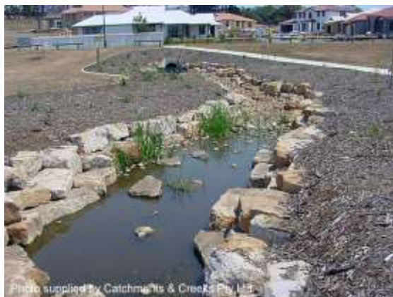
Rock-lined low-flow channel (Qld)
