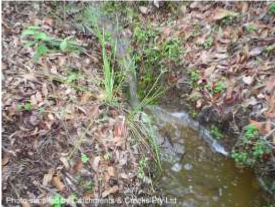
Scour along an overland flow path (Qld)
