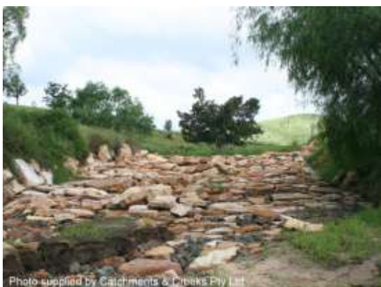
Rock chute stabilising gully erosion (Qld)
