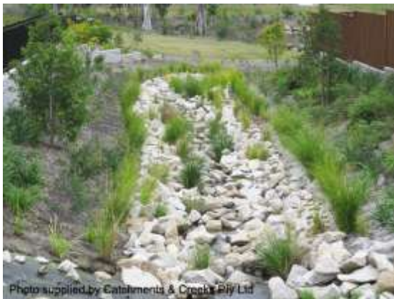
Rock-lined low-flow channel (Qld)
