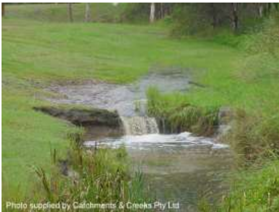
Formation of a scour hole (Qld)
