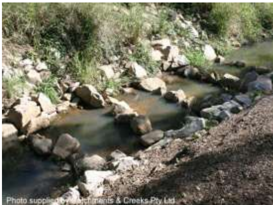
Ridge rock ramp (Qld)
