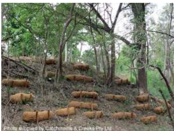
Geo logs used on a steep creek bank
