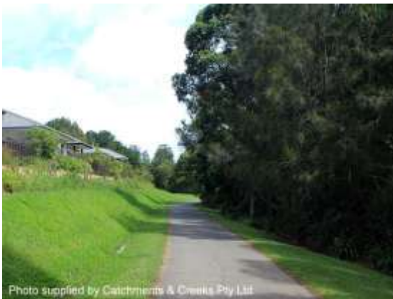
Constructed floodway (Qld)
