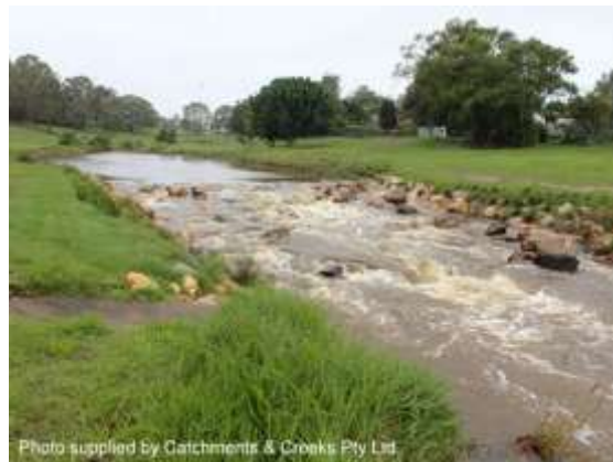
Constructed riffle (Qld)
