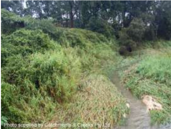
Grasses flattened by floodwater (Qld)
