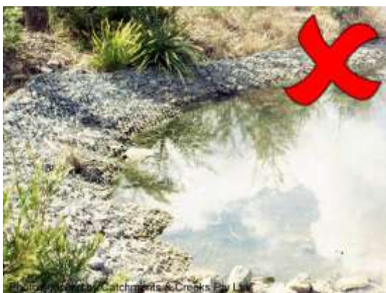
Mattress-lined sediment pond (Qld)
