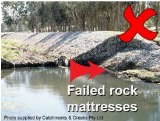
Open channel drop structure (Qld)
