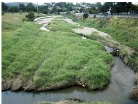
Sedimentation problems in a wide channel
