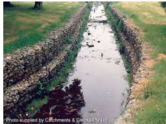
Gabion-lined low-flow channel (NSW)
