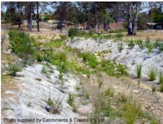
Drainage channel (Qld)
