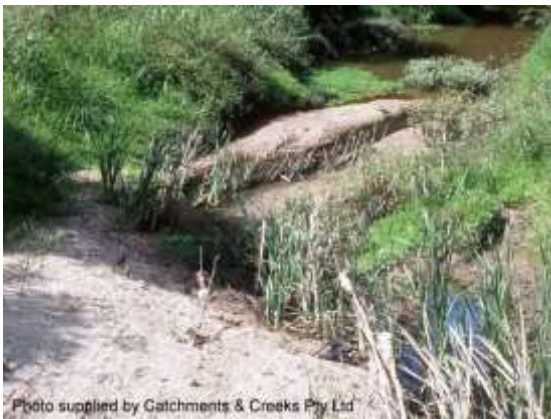
Unnatural sediment in an urban creek
