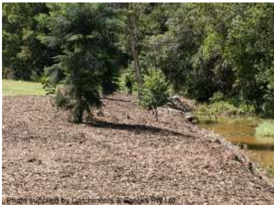
Loose mulch applied to a creek bank
