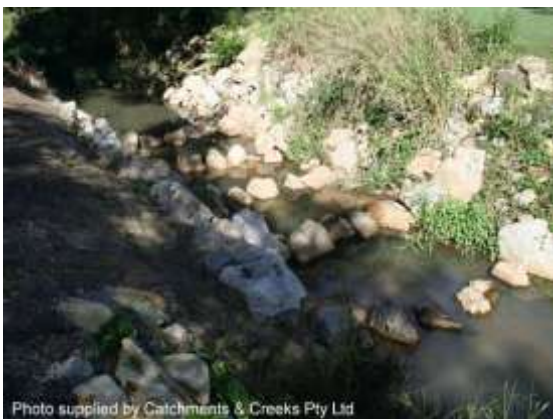
Ridge rock ramp (Qld)
