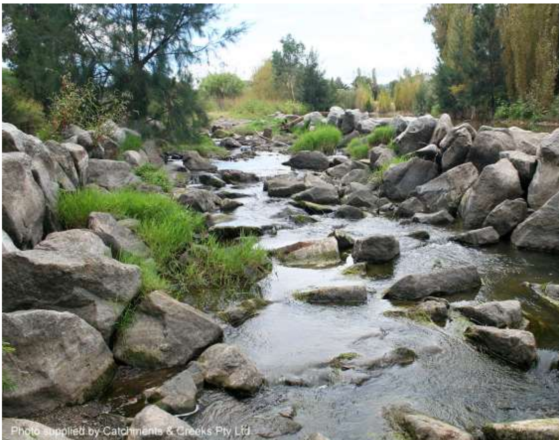
Constructed rock ramp (fishway) in Tamworth, NSW
