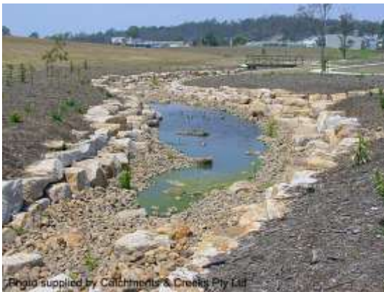
Constructed pool (Qld)
