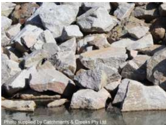
Fractured rock (Qld)
