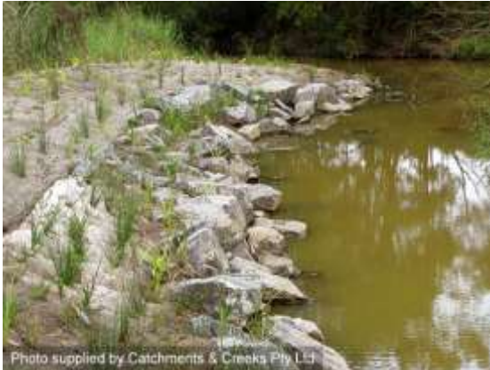
Vegetated rock stabilisation of bank (Qld)
