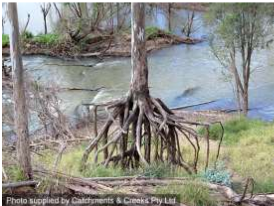
Exposure of roots by severe bank erosion
