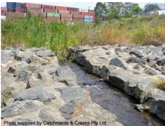
Low-flow channel set in grouted rock
