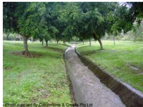
Concrete low-flow channel (Qld)
