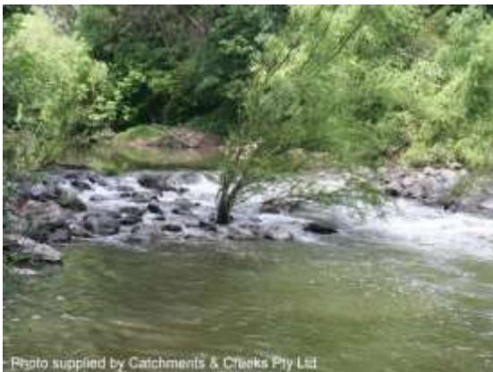
Constructed rock ramp/chute (NSW)
