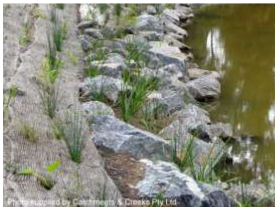
Newly placed and vegetated rock (Qld)
