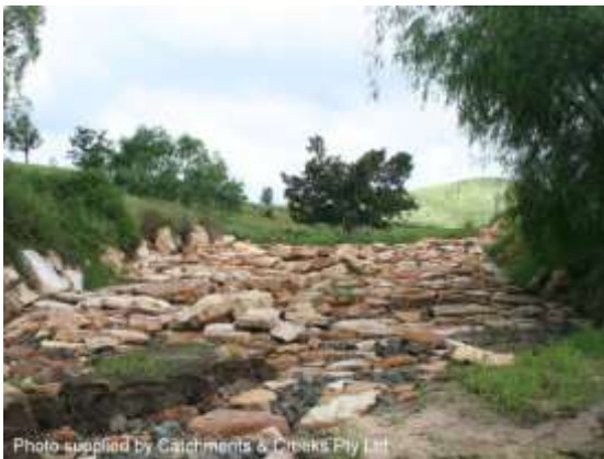
Non-fish-friendly drop structure (Qld)
