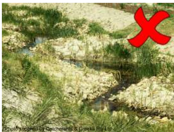
Meandering low-flow channel
