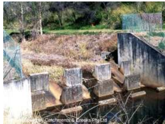
Baffled drop structures (Qld)
