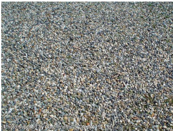
Initial placement of gravel and soil
