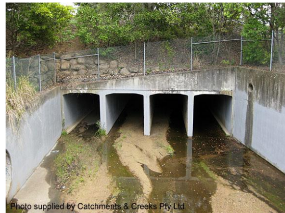
Open roof section within a long culvert
