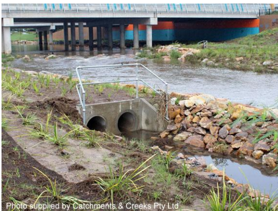
Recessed stormwater outlet with water quality treatment swale (Qld)
