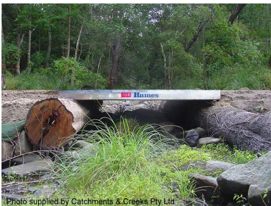
Small bridge formed from a 'bridging slab'
