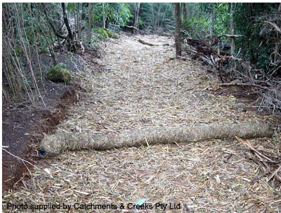
A closed track cover in mulch (Qld)
