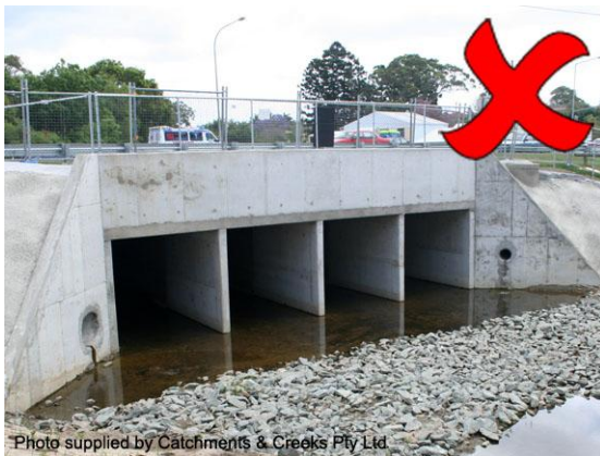
Maximum height culverts should be used
