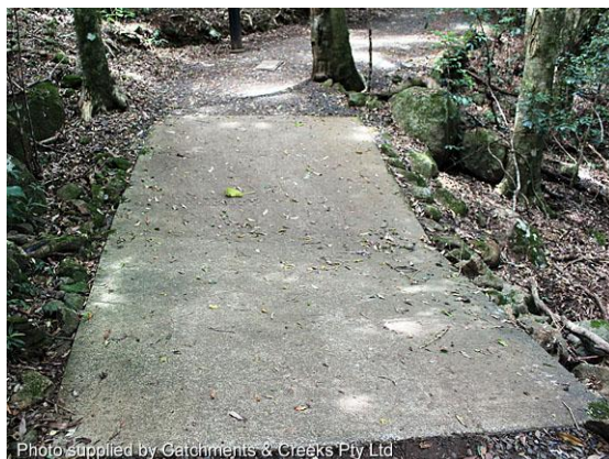
Concrete cross drain on a walking track
