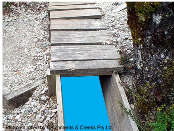
Timber cross drain (Tas)
