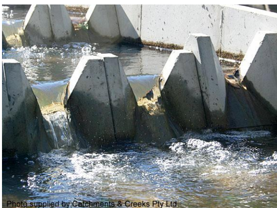
Block-ramp fishway (Walaman)
