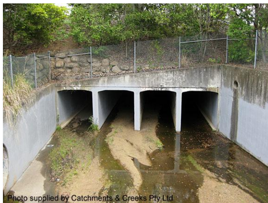
Open roof section within a long culvert
