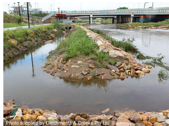
Recessed stormwater outlet with water quality treatment swale (Qld)
