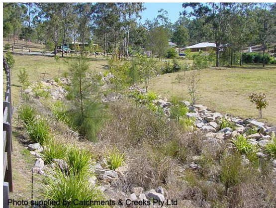
New drainage channel (Qld)
