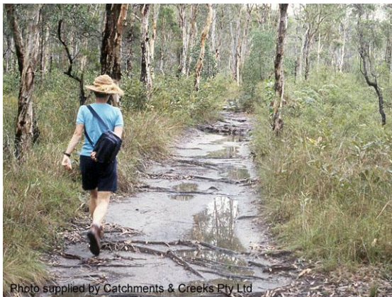
Walking track with exposed tree roots
