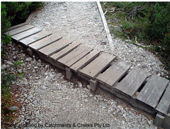
Timber cross drain (Tas)
