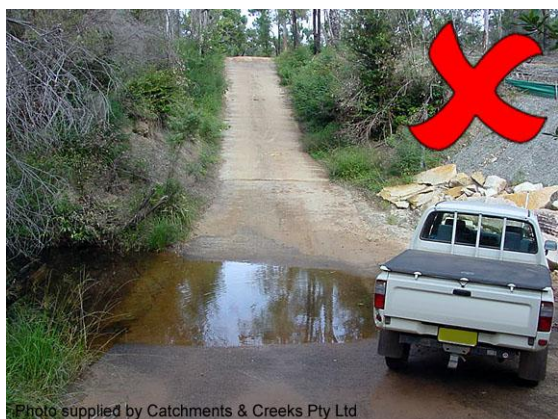
Concrete-lined ford crossing
