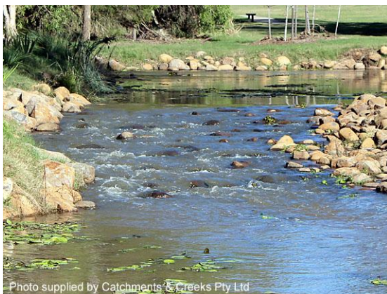
Rock chute (rock ramp) drop structure
