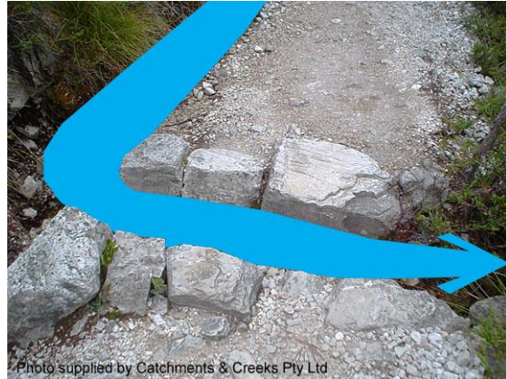
Stone cross drain (Tas)
