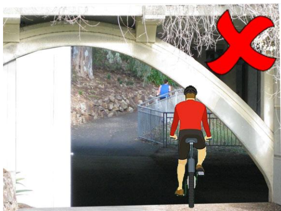
Insufficient head room below the arch
