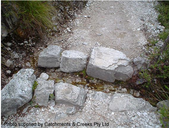
Stone cross drain (Tas)
