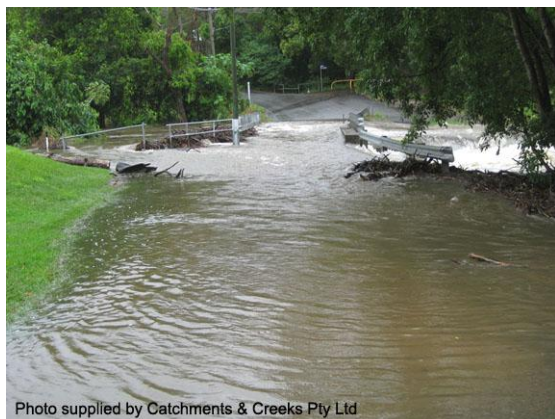
Flood overtopping road culvert (Qld)
