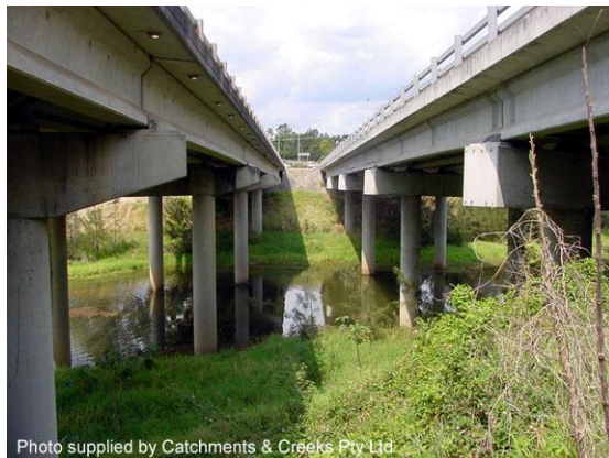
Twin bridges with good light penetration
