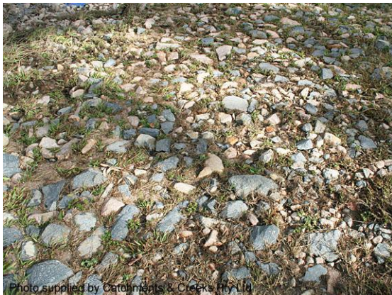
A stabilised gravel-grass surface (NSW)
