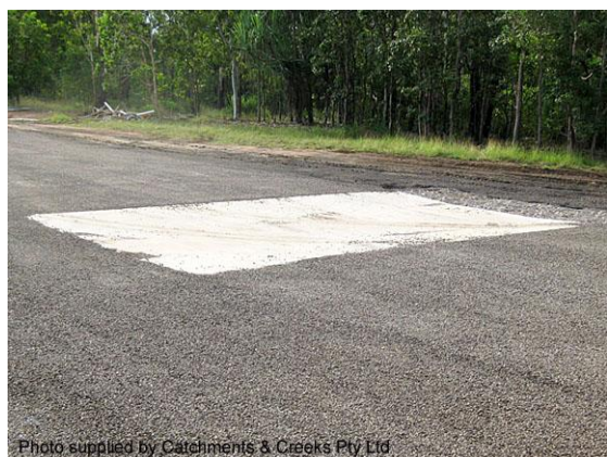
Crossing of a drainage swale (NT)
