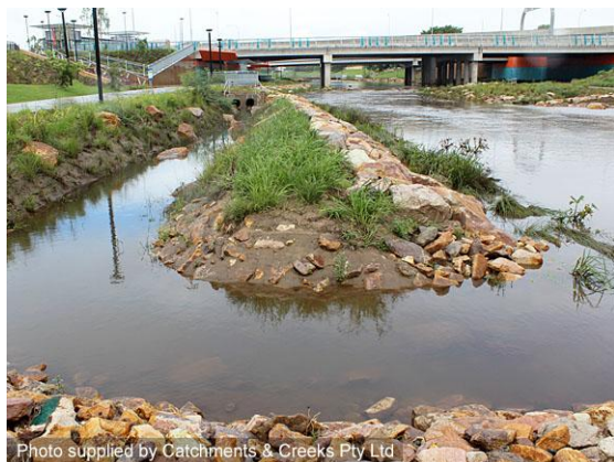
Recessed stormwater treatment channel
