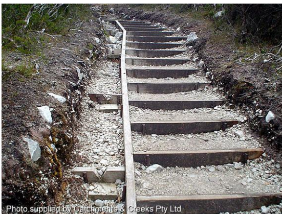
Timber steps and drain (Tas)
