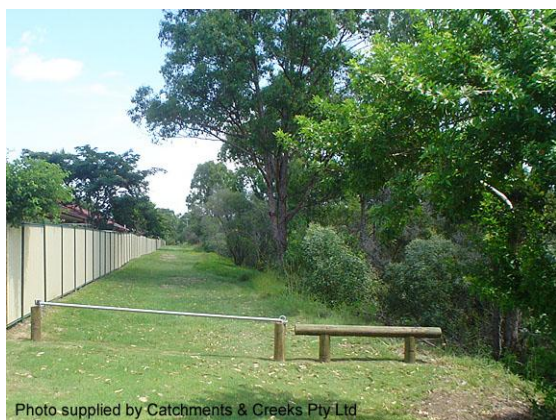
Fire trail and maintenance berm (Qld)
