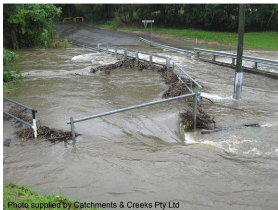
Floodwater overtop a road culvert
