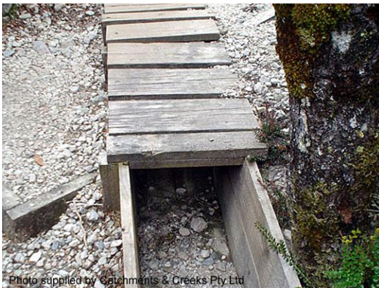
Timber cross drain (Tas)
