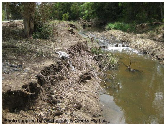
Bank erosion following weed removal
