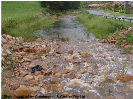
Constructed riffle (Qld)
