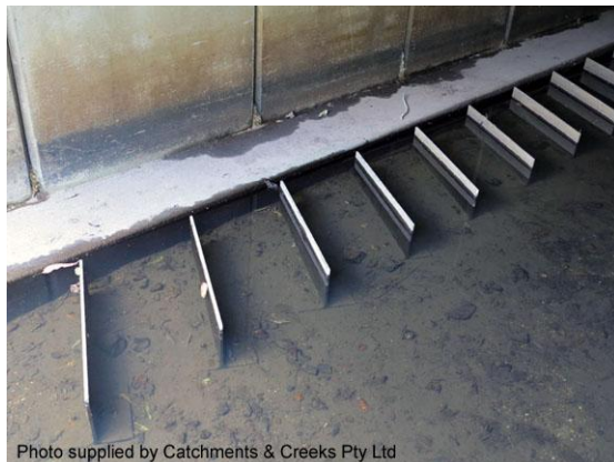
Baffles attached to the terrestrial pathway
