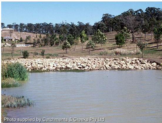
Rock chute inlet upstream of a lake
