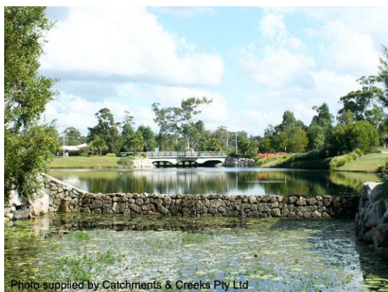
Downstream control weir (Qld)
