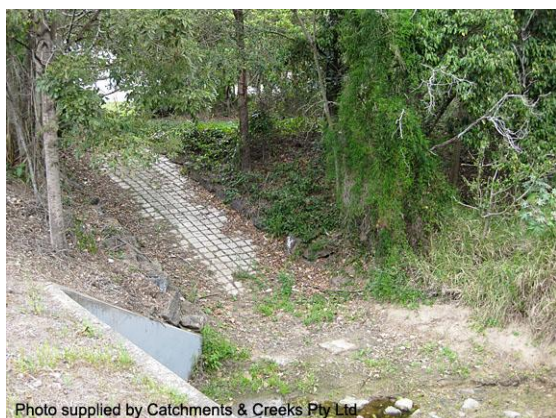
Maintenance access ramp (Qld)
