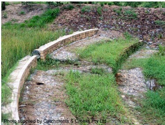
Stepped rock-mattress drop structure (Qld)
