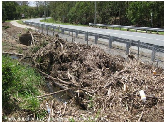
Debris blockage of culvert entrance
