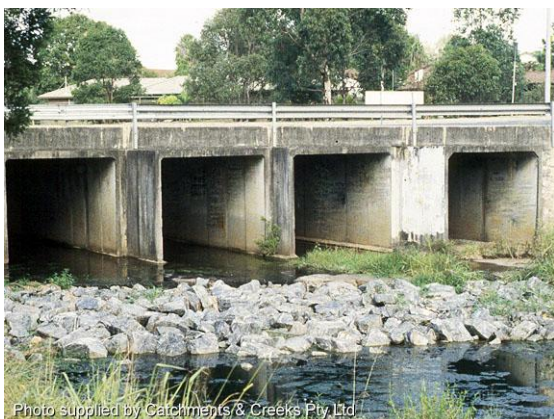
Rock pad outlet protection (Qld)
