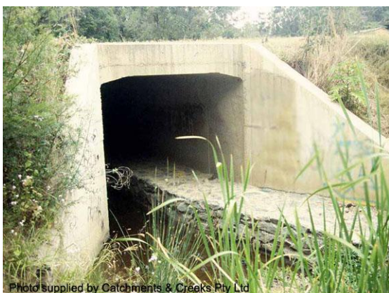
Terrestrial passage through culvert (Qld)
