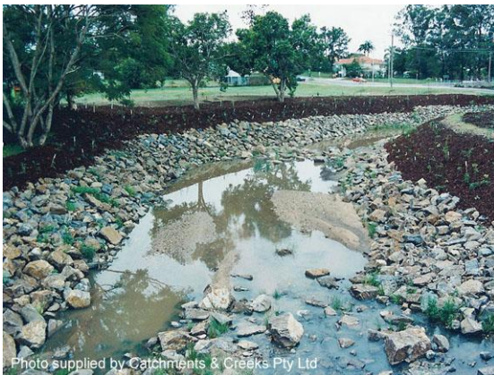
Rock placement on a channel bend (Qld)
