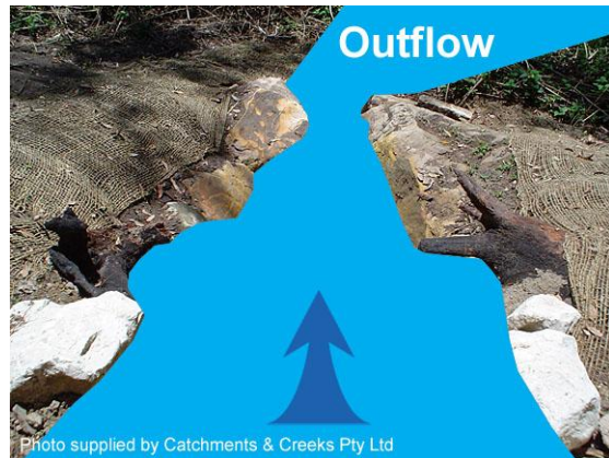
Discharge end of a cross bank (NSW)
