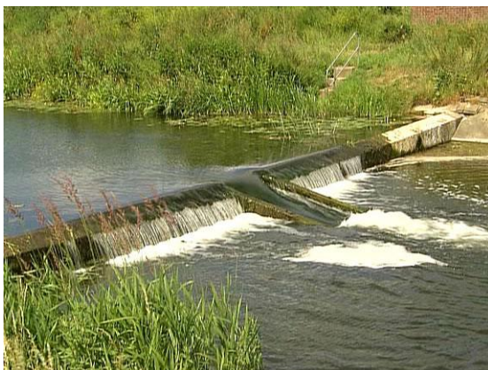
Non-fish-friendly grade control structure
