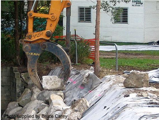
Example of 'placed rock' (Qld)
