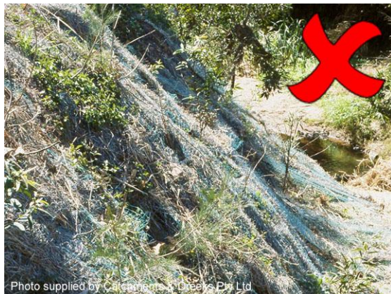
Plastic-reinforced erosion control mat
