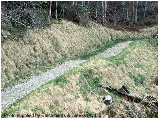
Cross banks on a gravel access road
