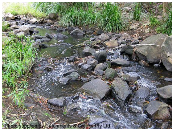
Constructed riffle (Qld)
