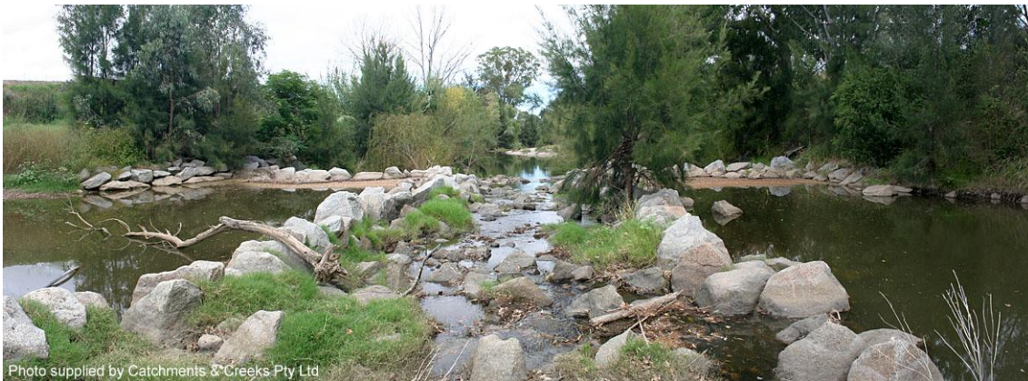
4. Rock ramp located within a rock weir (Tamworth, NSW)
