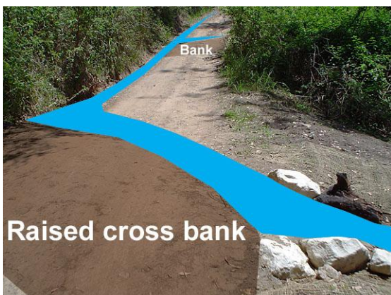
Dirt access road with cross bank (NSW)
