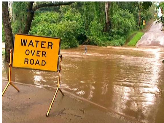
Closure of a waterway crossing (Qld)
