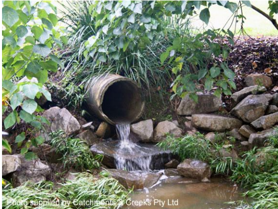
Stormwater outlet into a creek (Qld)
