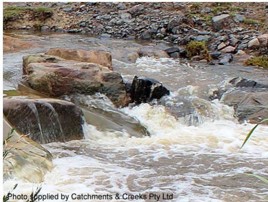
Constructed rock riffle (Qld)
