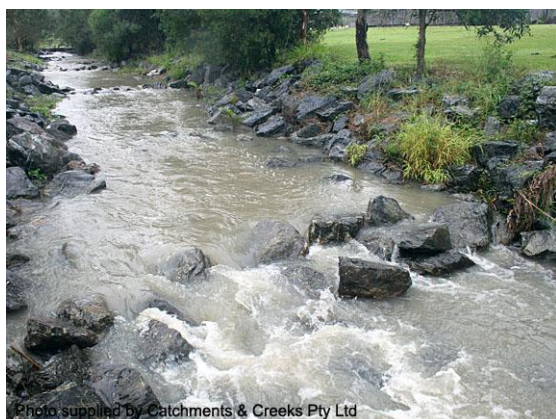
Constructed pool-riffle sequence (Qld)
