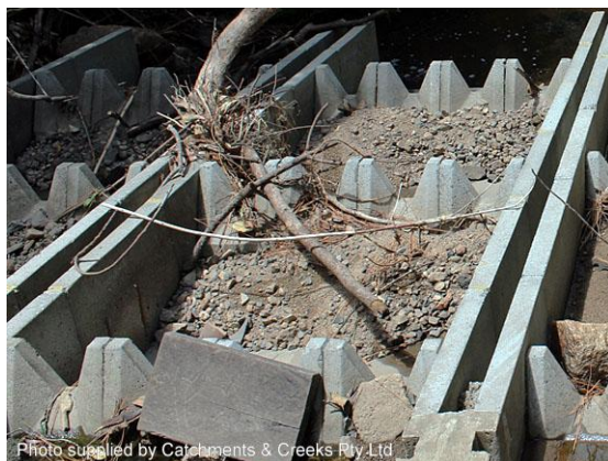
Sediment deposition within a fishway
