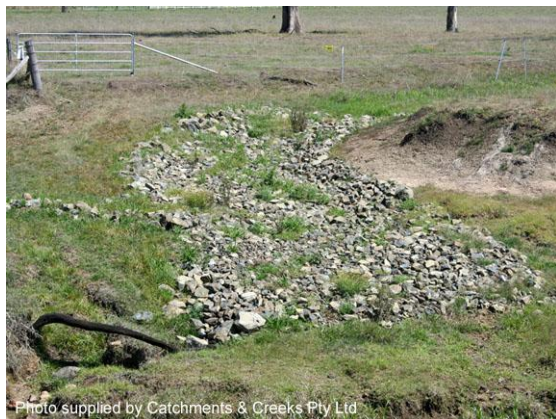
Stabilised stock access ramp (Qld)
