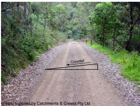
Dirt road with infall drainage
