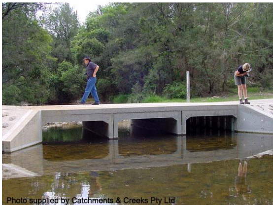
Culvert with sunken invert (NSW)
