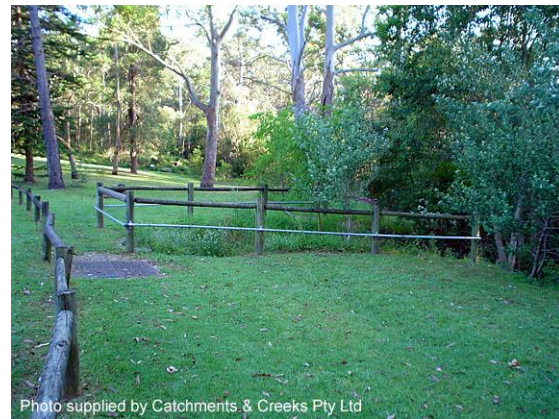
Recessed stormwater outlet (NSW)
