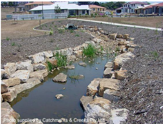
Recently constructed storm drain (2000)
