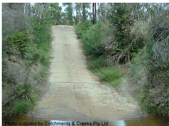
Permanent road access (NSW)
