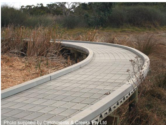
Boardwalk formed from recycled goods
