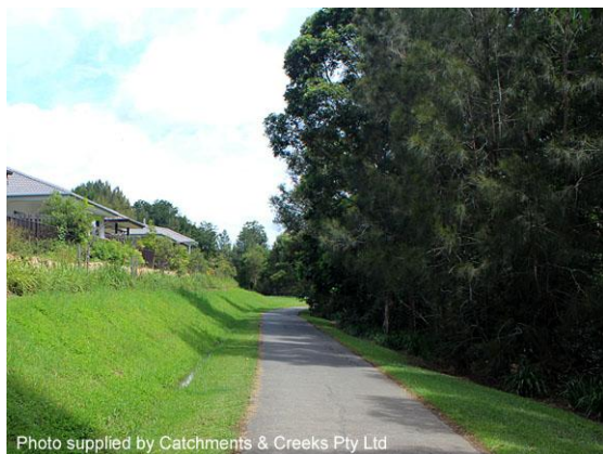
Benched floodway (Qld)
