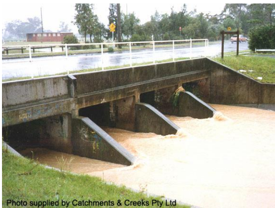
Debris deflector walls (NSW)
