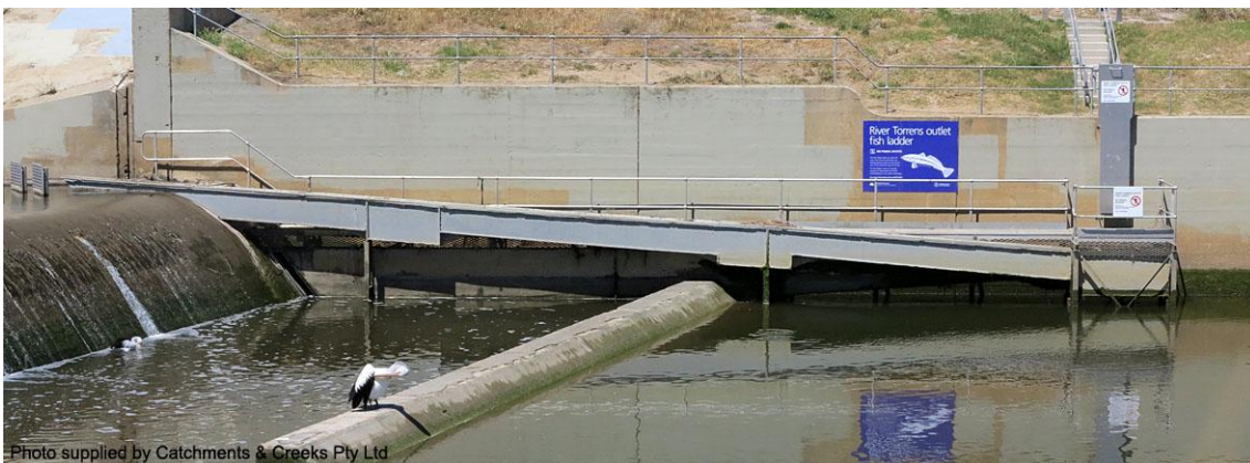
5. Torrens River outlet weir fishway (SA)
