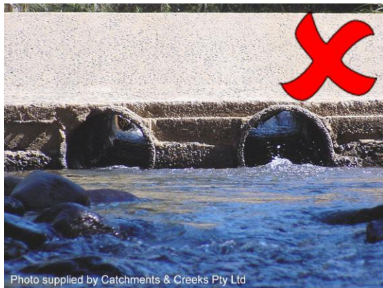
High-velocity, low-flow pipes
