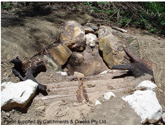
Discharge end of a cross bank (NSW)
