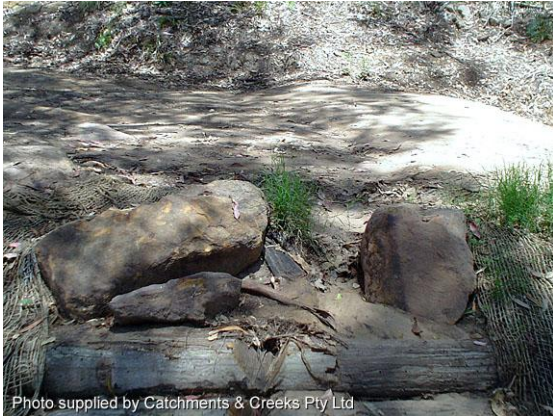
Discharge end of a cross bank (NSW)
