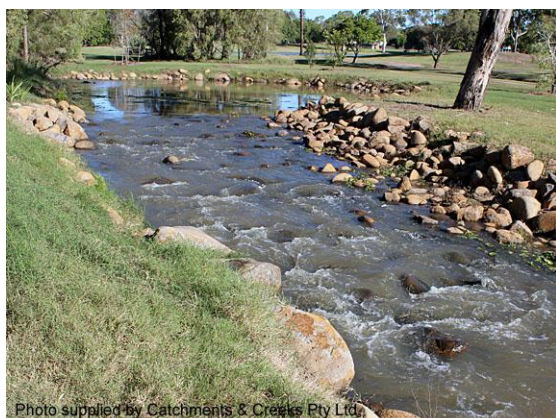
Constructed riffle (Qld)
