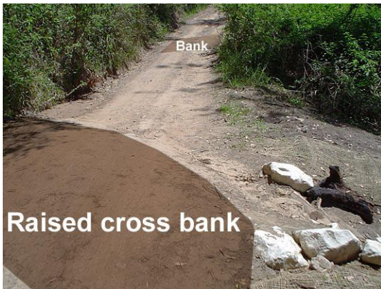
Dirt access road with cross bank (NSW)
