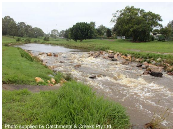
Constructed pool-riffle (Qld)
