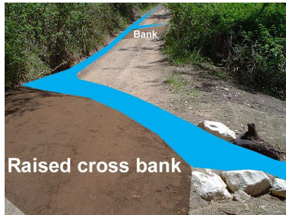
Dirt access road with cross bank (NSW)
