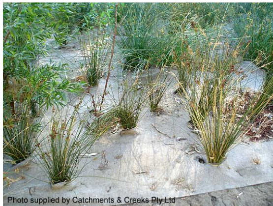
Jute erosion control blanket (SA)
