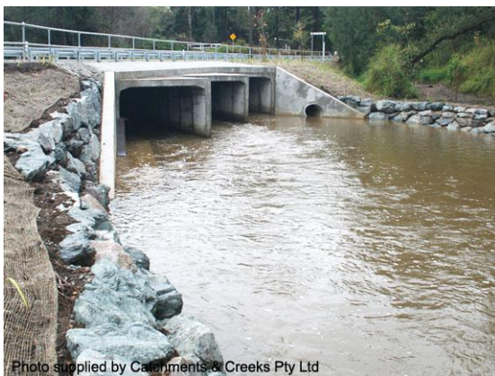
Box culvert (Qld)
