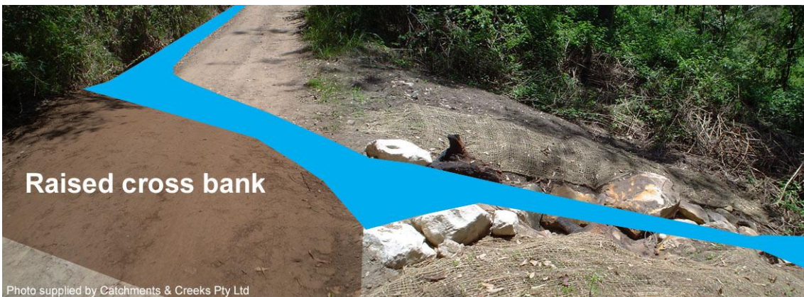
Outfall cross bank, which releases the flow down a stabilised rock-lined chute (NSW)
