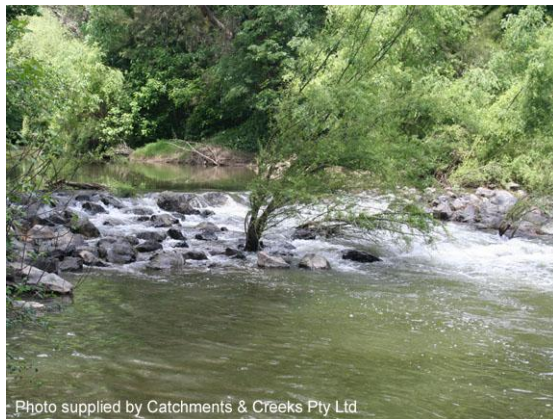
Constructed rock ramp/chute (NSW)
