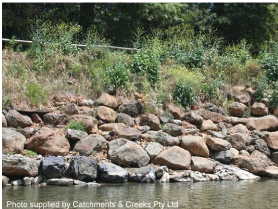
Partial vegetated bank stabilisation (NSW)
