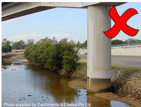
Bridge piers placed near a stream bank
