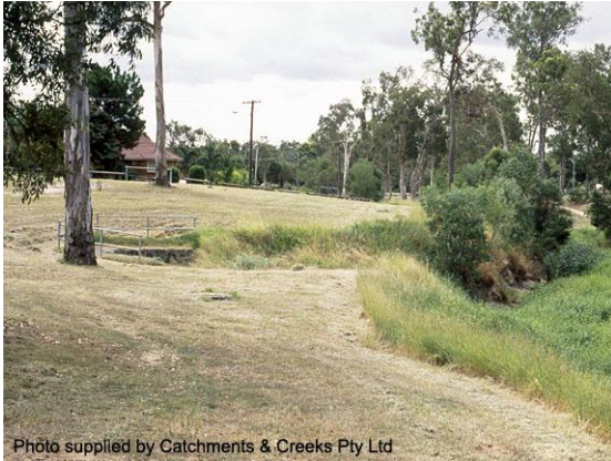
Recessed stormwater outlet (Qld)
