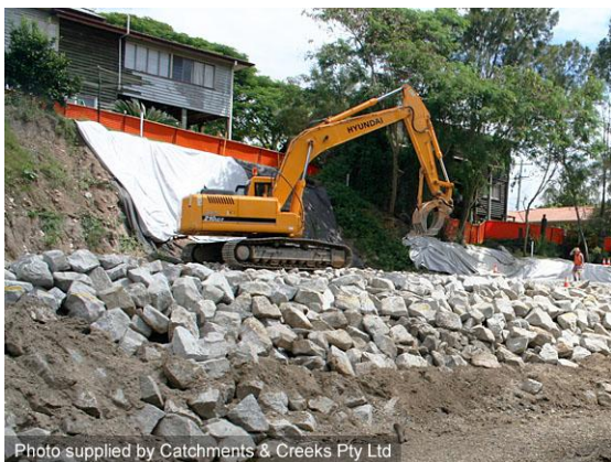
Rock placement over filter cloth (Qld)
