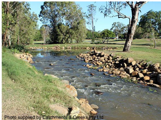
Constructed pool-riffle (Qld)
