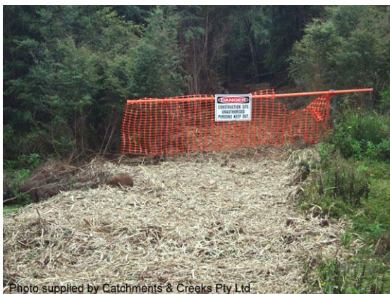
Straw mulch placed on a walking track
