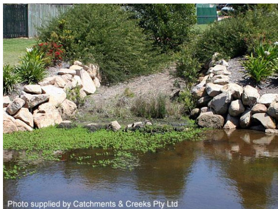
Maintenance access to the waterway
