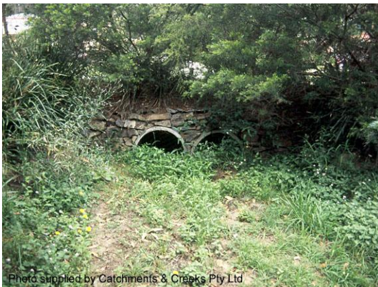
Recessed stormwater outlet (Qld)
