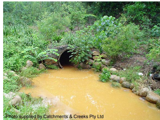
Recessed stormwater outlet (Qld)
