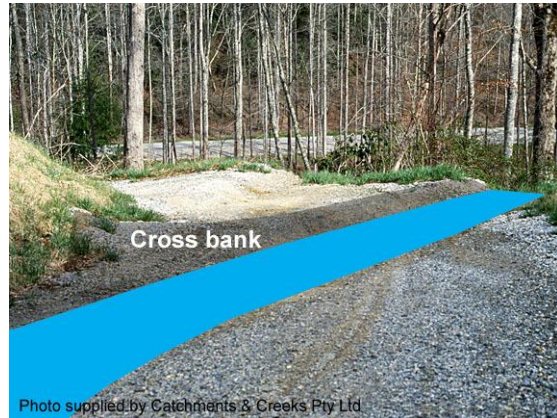
Gravel access road with cross bank
