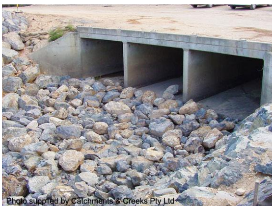
Thin deck box culvert (NSW)
