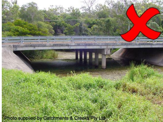
Bridge with minimal 'dry' passage
