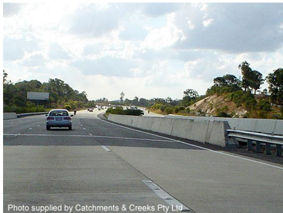
Low-noise asphalt placed over the bridge
