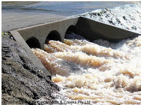
Excessive flow velocities (Qld)
