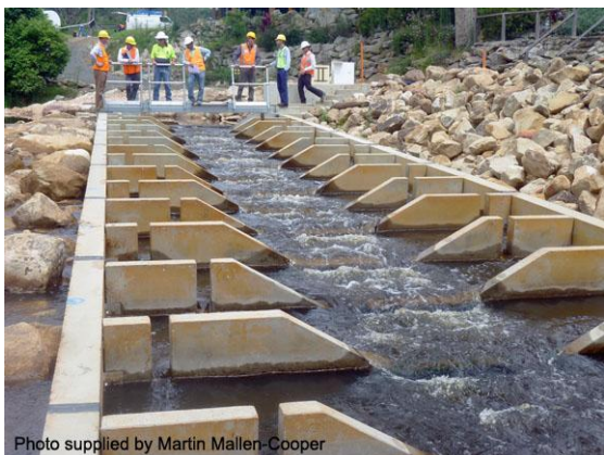
Baffled fishway (NSW)
