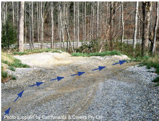
Cross bank drainage (USA)
