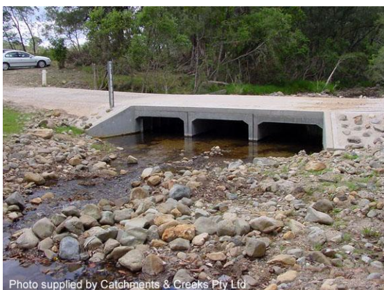
Fish friendly rural culvert (NSW)
