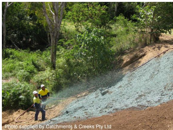
Hydraulically-applied blanket (Qld)
