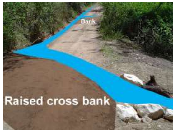
Dirt access road with cross bank (NSW)
