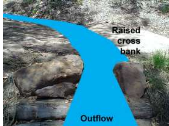
Discharge end of a cross bank (NSW)
