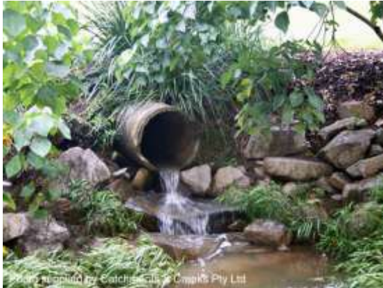
Stormwater outlet into a creek (Qld)
