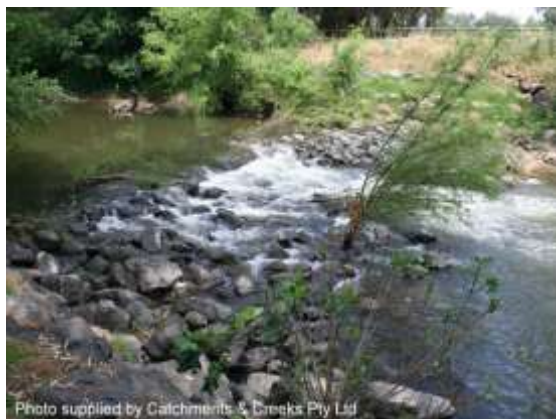
Constructed riffle (NSW)
