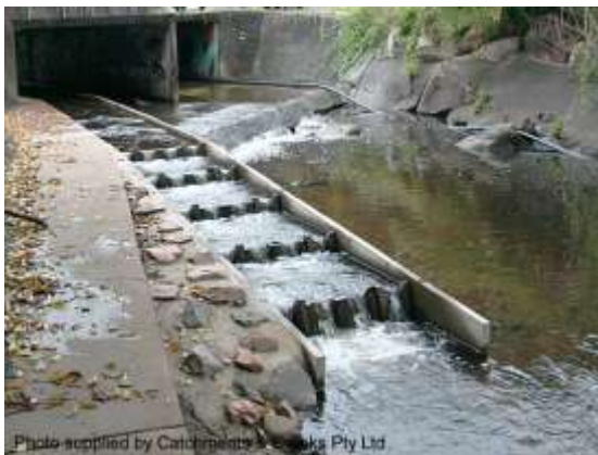
Constructed fishway (Qld)
