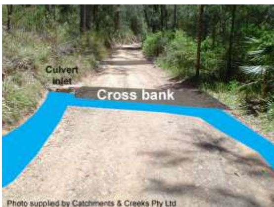
Combined cross bank and cross drain
