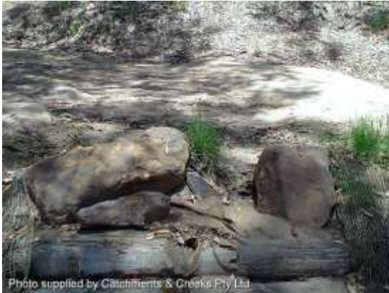
Discharge end of a cross bank (NSW)
