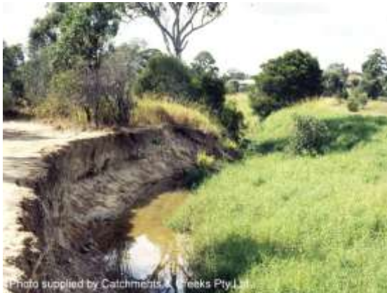
Erosion along a shaded north bank (Qld)
