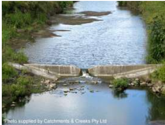
Small town water supply weir (Qld)
