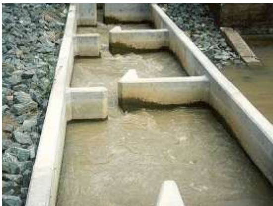
Vertical slot fishway
