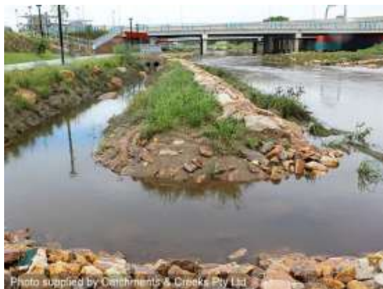
Recessed stormwater treatment channel
