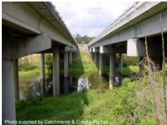
Twin bridges with good light penetration
