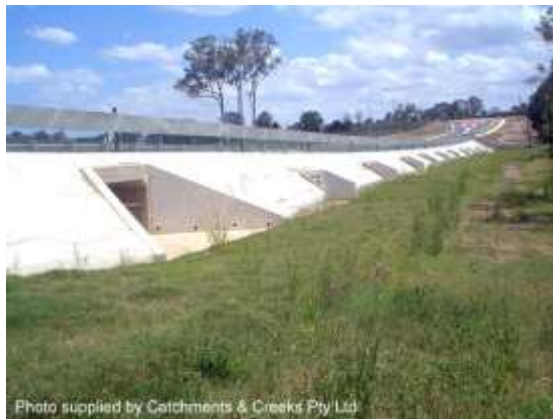
Floodplain culverts (Qld)
