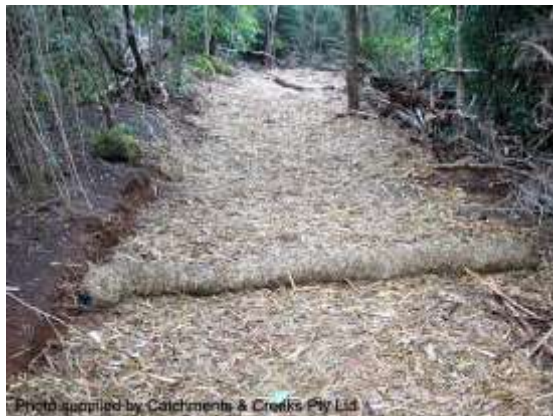
Photo supplied by Catchments & Creeks Pty Ltd A closed track cover in mulch (Qld)
