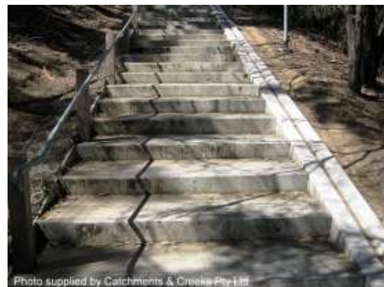
Concrete stair (SA)
