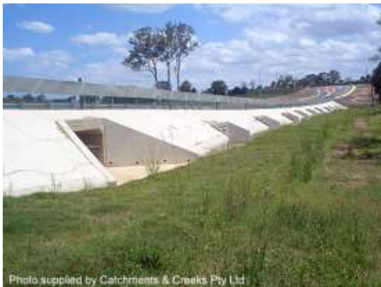
Floodplain culvert (Qld)
