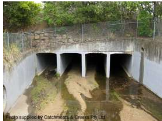
Open roof section within a long culvert
