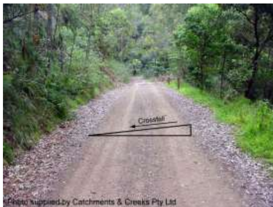
Infall trail drainage
