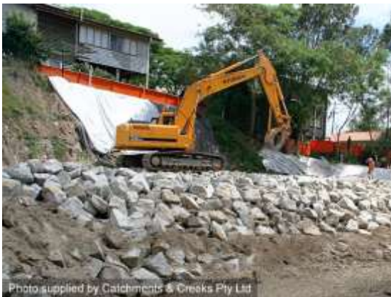
Rock placement over filter cloth (Qld)
