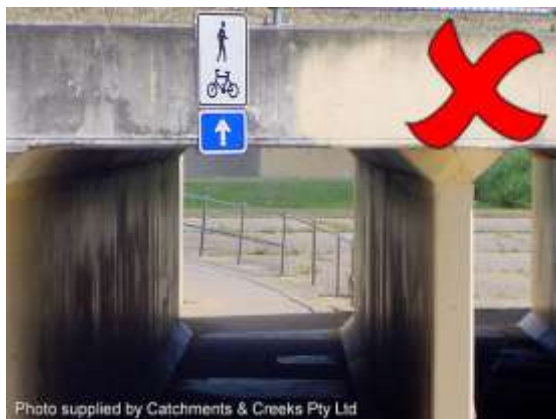
Photo supplied by Catchments & Creeks Pty Ltd Limited line-of-sight at tunnel exit
