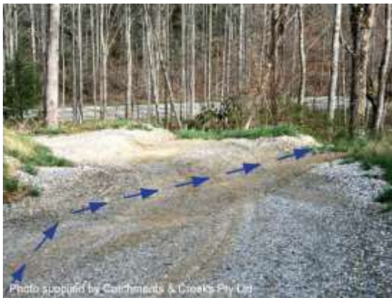
Cross bank drainage (USA)
