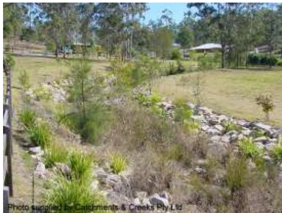
New drainage channel (Qld)
