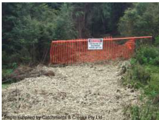
Fire trail closed for rehabilitation (Qld)
