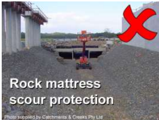
Hard engineering scour protection
