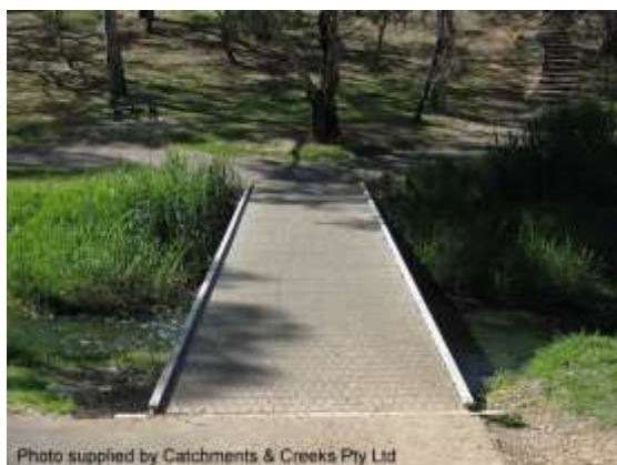
Low-level footbridge without railings (SA)
