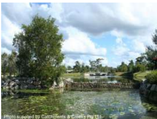
Rock weir downstream of a lake
