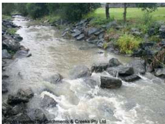
Constructed pool-riffle sequence (Qld)
