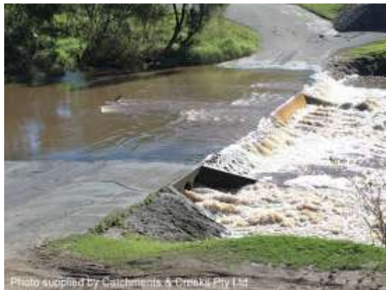
Stream flow just overtopping a causeway
