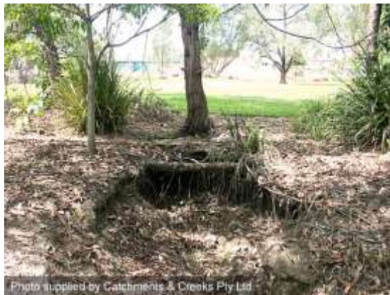
Stormwater-induced lateral bank erosion
