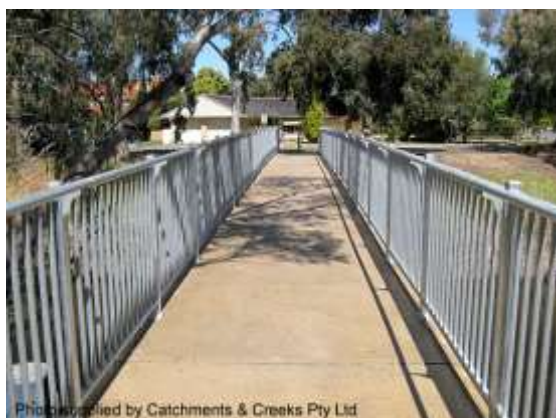
High-level footbridge (SA)
