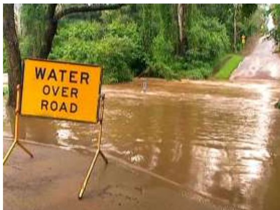
Closure of a waterway crossing (Qld)
