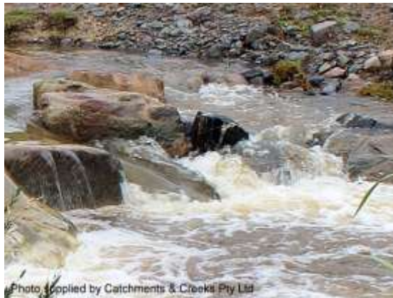
Constructed rock riffle (Qld)
