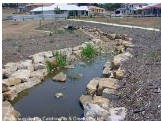
Recently constructed storm drain (2000)
