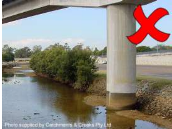
Bridge piers placed near a stream bank
