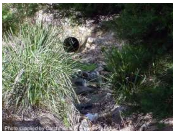
Shading of a storm drain (Qld)
