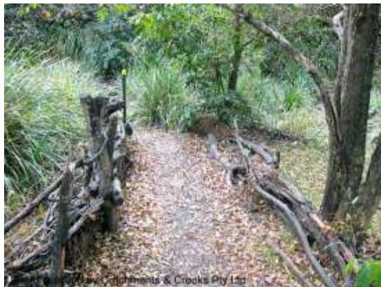
Controlling pedestrian movement (Qld)
