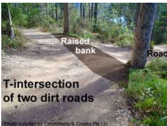
T-junction with cross bank (NSW)
