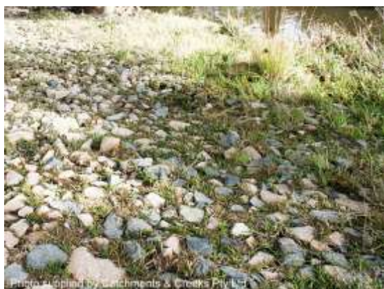
Photo supplied by Catchments & Creeks Pty Ltd Gravel-grass access road (NSW)
