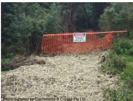
Straw mulch placed on a walking track
