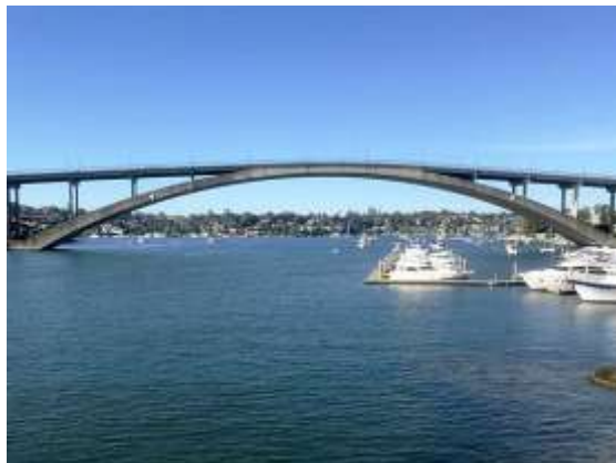
Gladesville Bridge, Sydney, NSW
