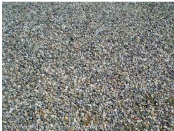
Initial placement of gravel and soil
