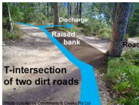
T-junction with cross bank (NSW)
