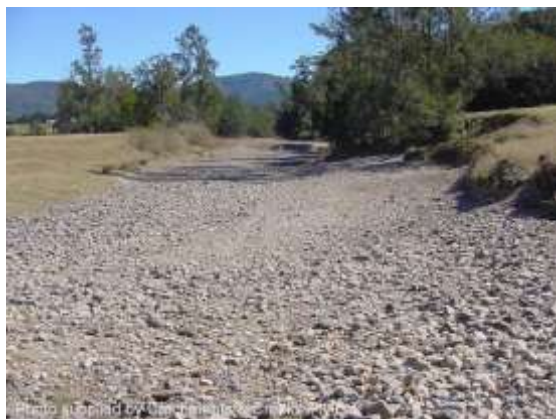
Bed gravel upstream of a causeway
