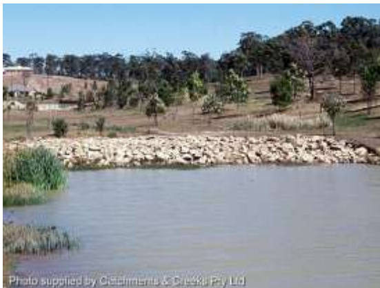
Rock chute inlet upstream of a lake
