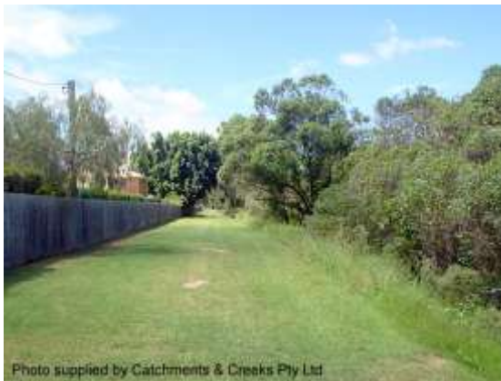
Outfall drainage of a fire trail (Qld)
