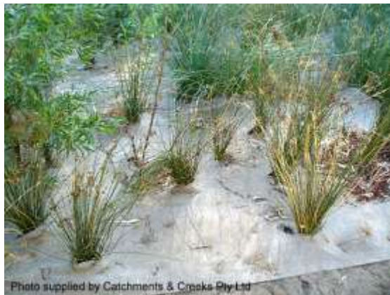
Jute erosion control blanket (SA)
