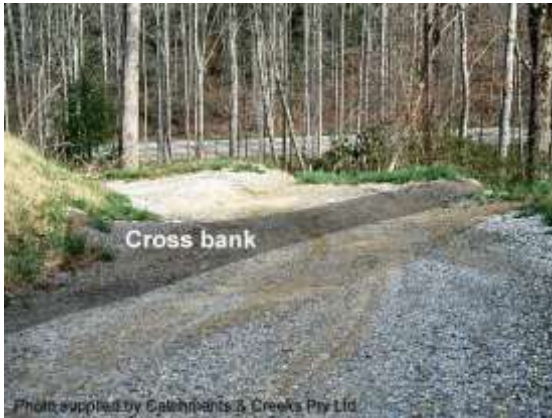
Gravel access road (USA)
