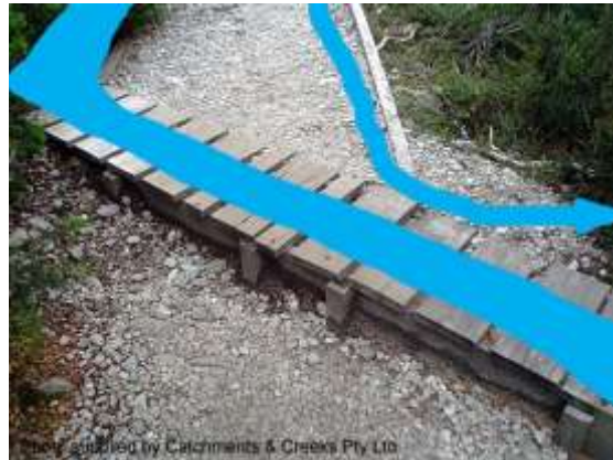
Timber cross drain (Tas)
