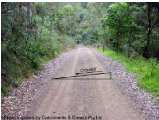
Dirt road with infall drainage
