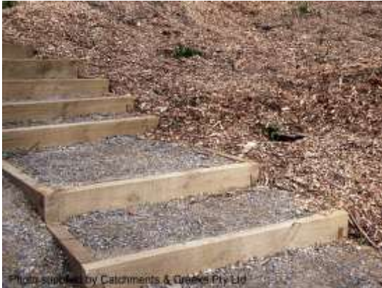
Timber steps (Qld)
