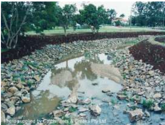
Rock placement on a channel bend (Qld)
