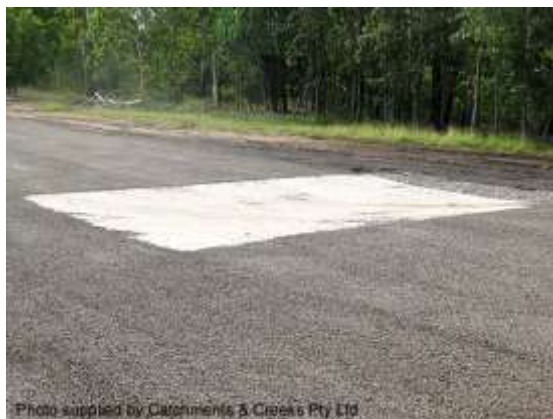
Crossing of a drainage swale (NT)
