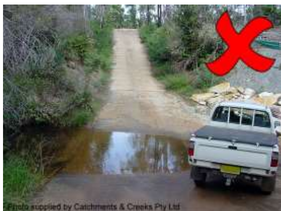
Concrete-lined ford crossing
