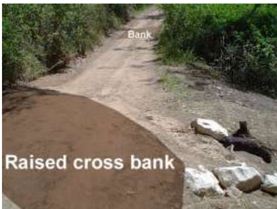
Dirt access road with cross bank (NSW)
