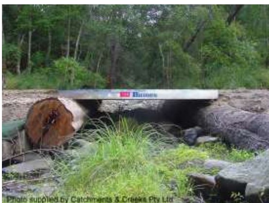
Small bridge formed from a 'bridging slab'
