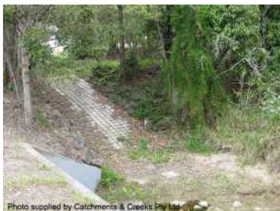
Maintenance access ramp (Qld)
