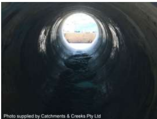
Very dark culvert
