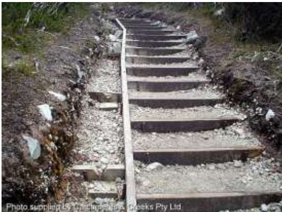
Timber steps and drain (Tas)
