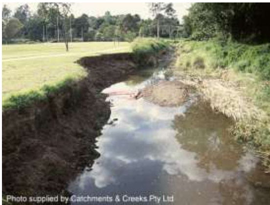
Erosion along a shaded north bank (Qld)
