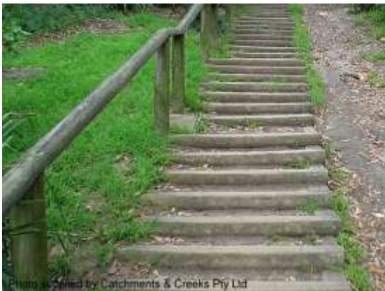
Timber steps (NSW)
