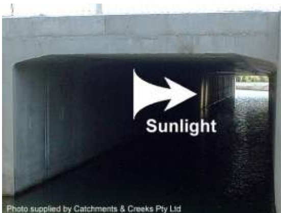
Light entering the culvert (Qld)
