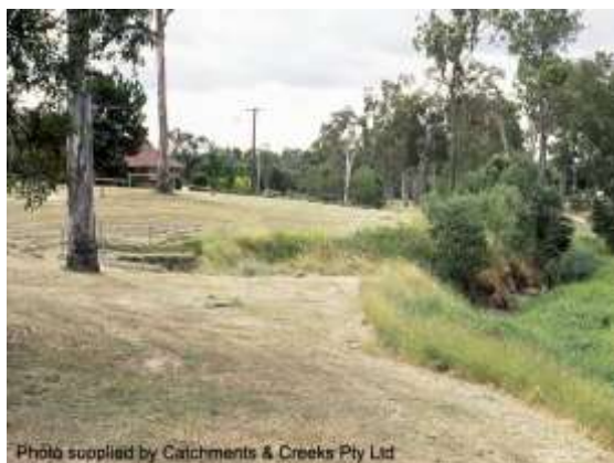
Recessed stormwater outlet (Qld)
