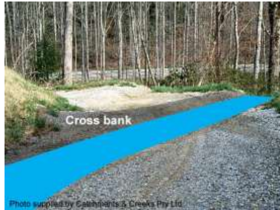
Gravel access road with cross bank
