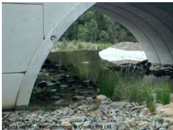
Terrestrial pathway under an arch (NSW)
