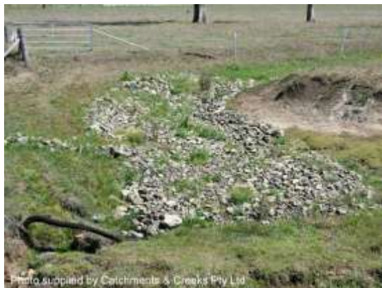
Stabilised stock access ramp (Qld)
