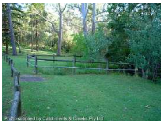
Recessed stormwater outlet (NSW)
