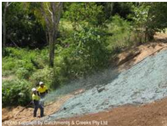
Hydraulically-applied blanket (Qld)
