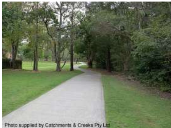
Floodway adjacent to riparian zone
