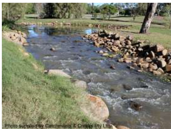
Constructed riffle (Qld)
