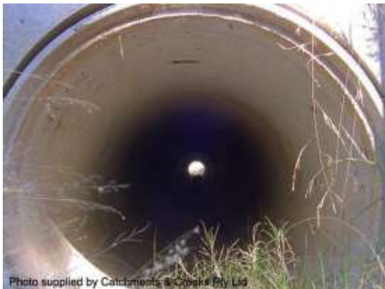
A long, smooth-wall culvert
