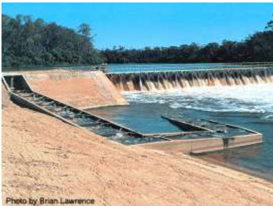
2. Fishway bypass fishway (SA)
