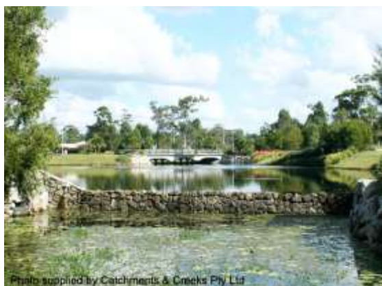
Downstream control weir (Qld)
