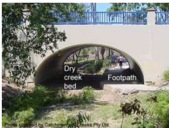
Arch bridge over ephemeral creek (Qld)
