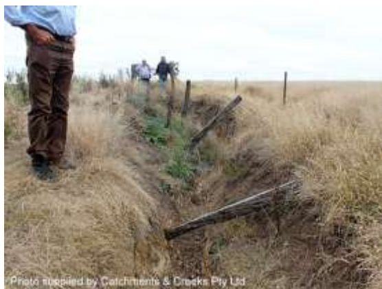
Gully erosion along a fence line (Qld)
