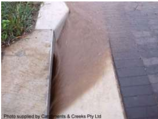
Turbid stormwater runoff
