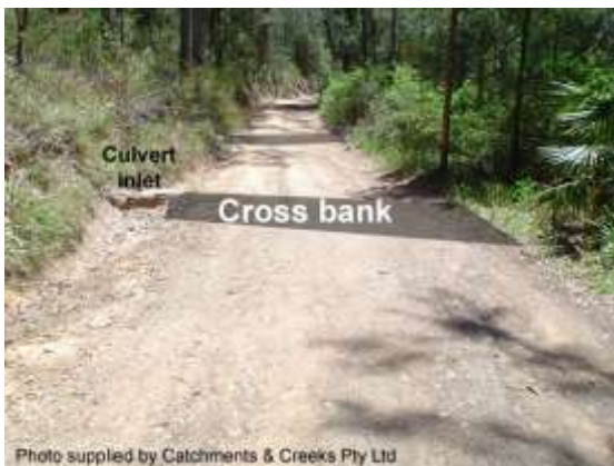
Cross banks and culvert drain (NSW)
