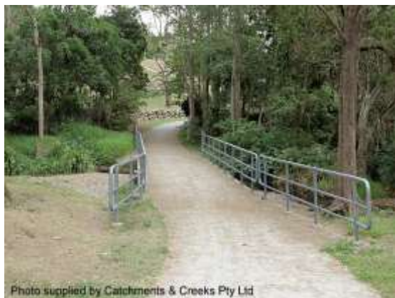
Low-level footbridge with railings (Qld)
