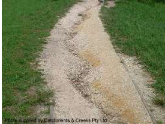
Photo supplied by Catchments & Creeks Pty Ltd Rill erosion on a walking track (NSW)
