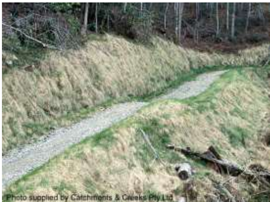
Cross banks on a gravel access road
