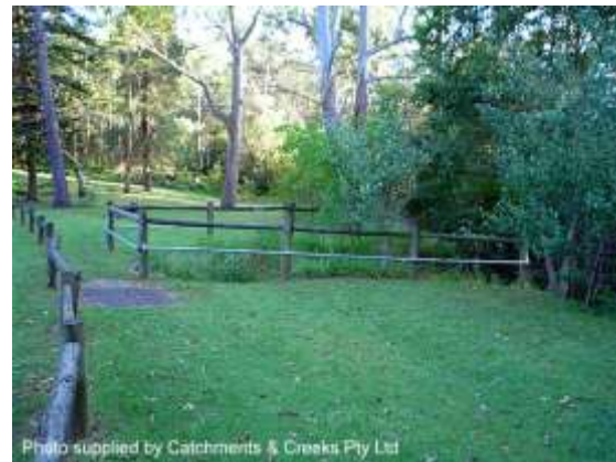
Recessed stormwater outlet (NSW)
