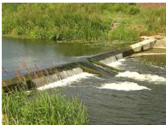
Non-fish-friendly grade control structure
