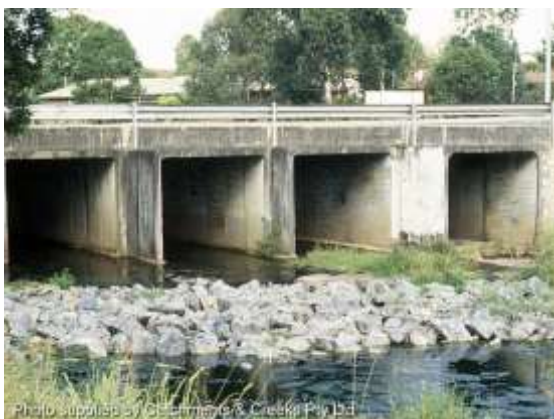
Rock pad outlet protection (Qld)
