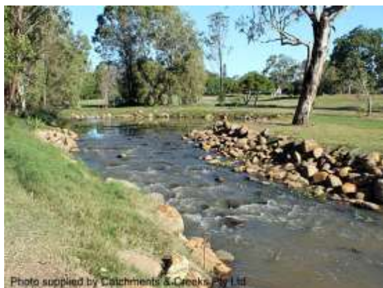
Constructed pool-riffle (Qld)
