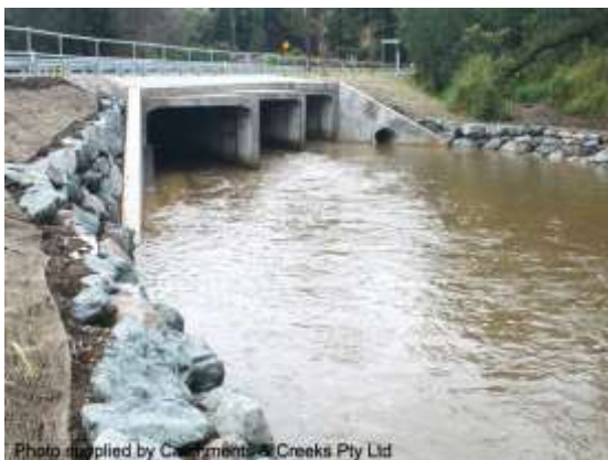
Box culvert (Qld)
