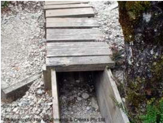
Timber cross drain (Tas)
