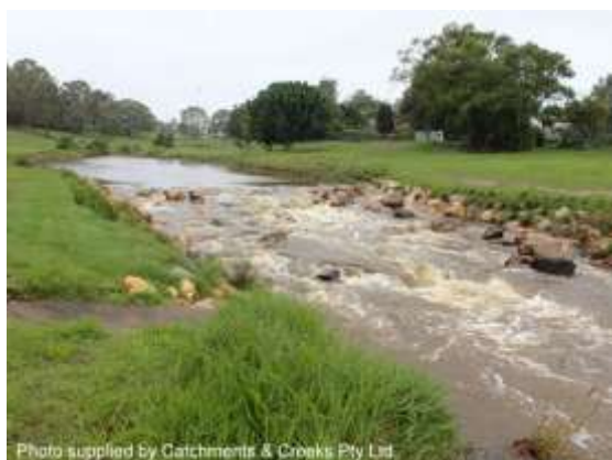
Constructed pool-riffle (Qld)
