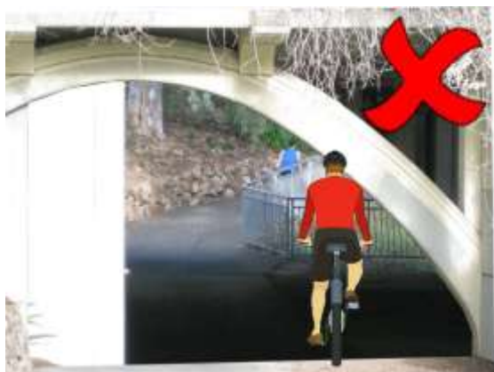
Insufficient head room below the arch
