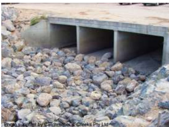
Thin deck box culvert (NSW)
