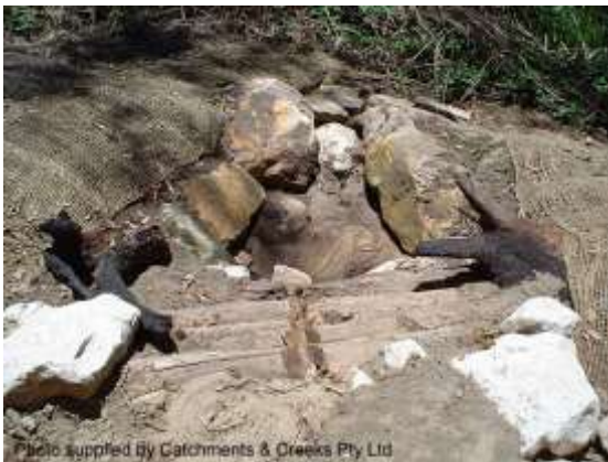
Discharge end of a cross bank (NSW)
