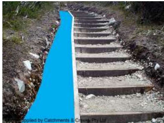
Timber steps and drain (Tas)
