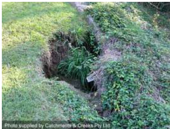
Tunnel erosion adjacent a creek (Qld)
