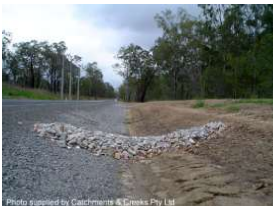
Rock check dam (Qld)
