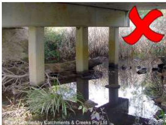
Piers located within the waterway
