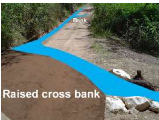
Dirt access road with cross bank (NSW)
