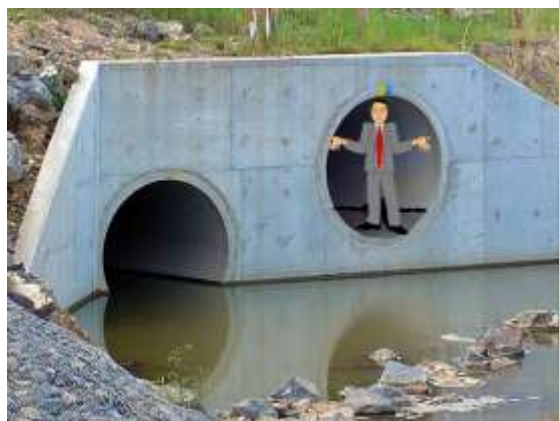
A 'dry' cell not connected to dry land
