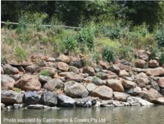
Partial vegetated bank stabilisation (NSW)
