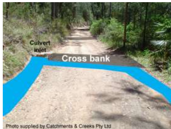
Cross banks and culvert drain (NSW)
