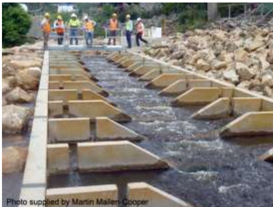
Baffled fishway (NSW)
