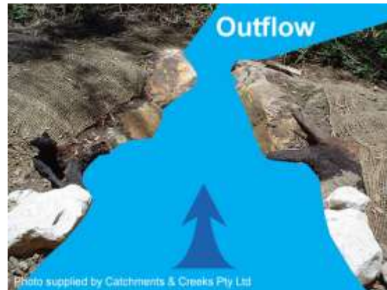
Discharge end of a cross bank (NSW)
