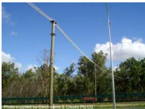
Rope bridge (Qld)
