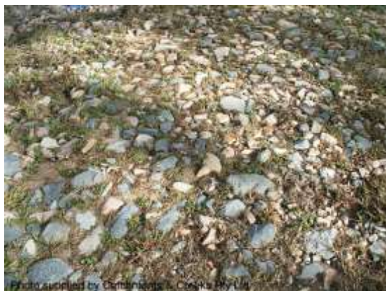
Photo supplied by Catchments & Creeks Pty Ltd A stabilised gravel-grass surface (NSW)
