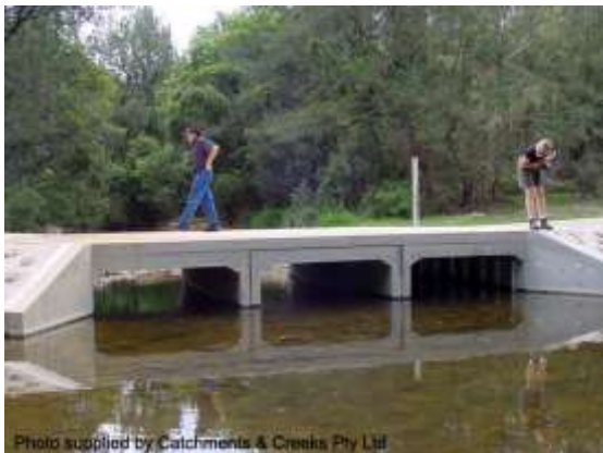
Culvert with sunken invert (NSW)
