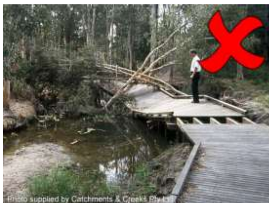
Flood damage to creek boardwalk
