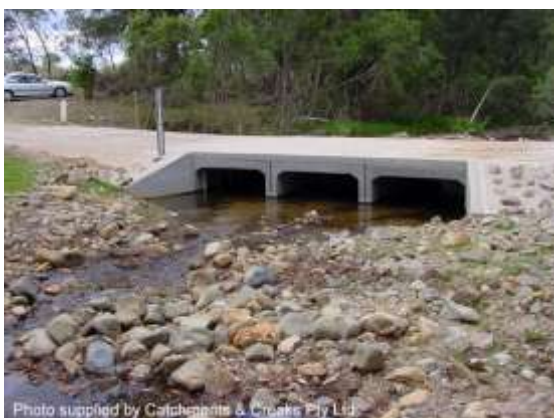
Fish friendly rural culvert (NSW)
