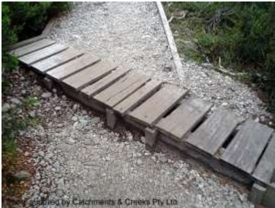
Timber cross drain (Tas)
