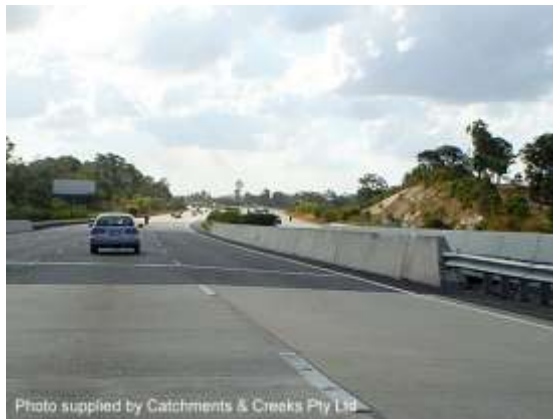
Low-noise asphalt placed over the bridge
