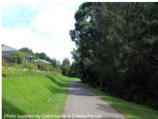
Benched floodway (Qld)
