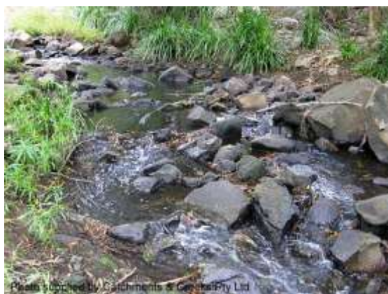
Photo supplied by Catchments & Creeks Pty Ltd Constructed riffle (Qld)
