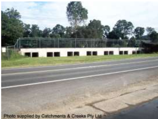
Floodplain culvert (Qld)
