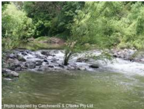
Constructed rock ramp/chute (NSW)
