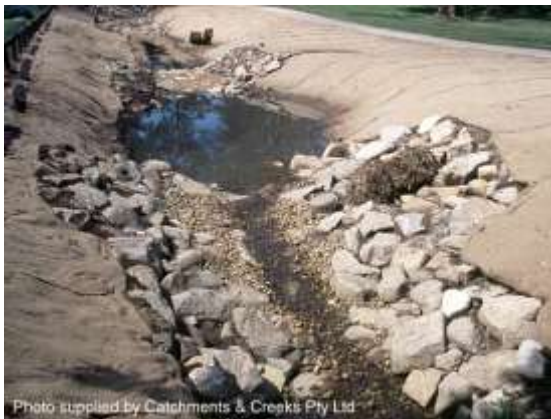
Constructed pool-riffle system (Qld)
