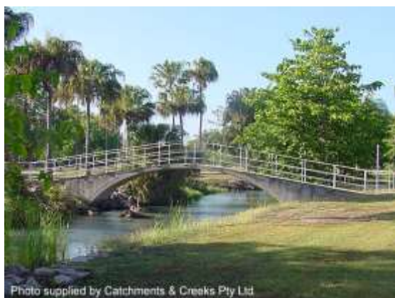
Arched footbridge (Qld)
