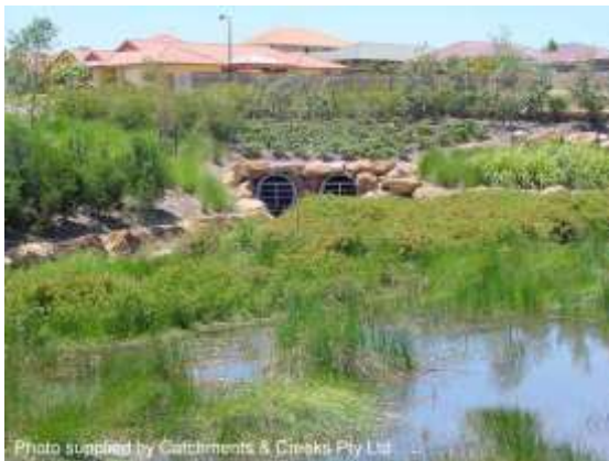
Stormwater treatment wetland (Qld)
