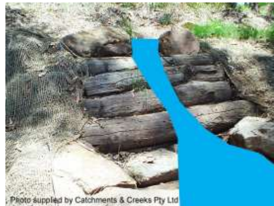
Discharge from a cross bank (NSW)
