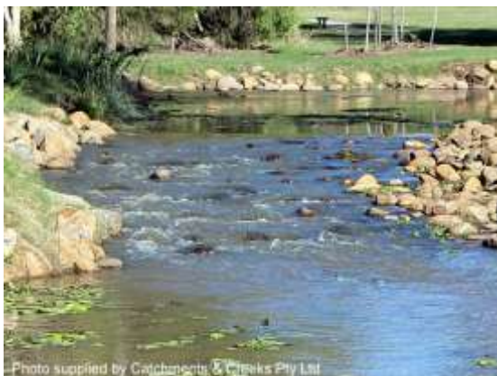
Rock chute (rock ramp) drop structure
