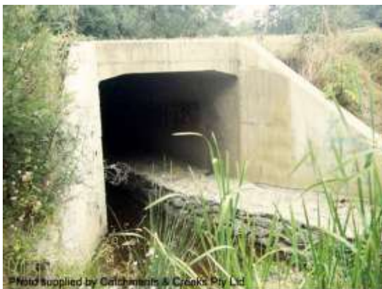
Terrestrial passage through culvert (Qld)
