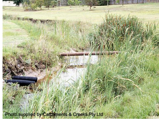
Sewer pipe crossing (1997)
