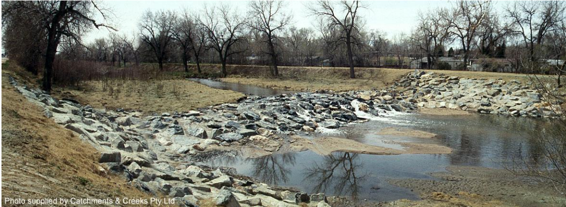
Grouted rock drop structure, Denver (1995)
