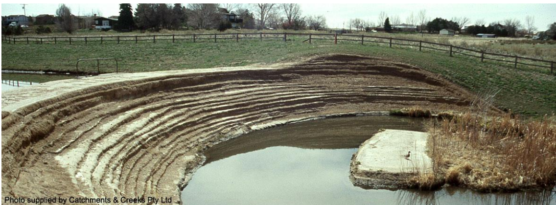
Rolled soil-cement drop structure, Denver (1995)
