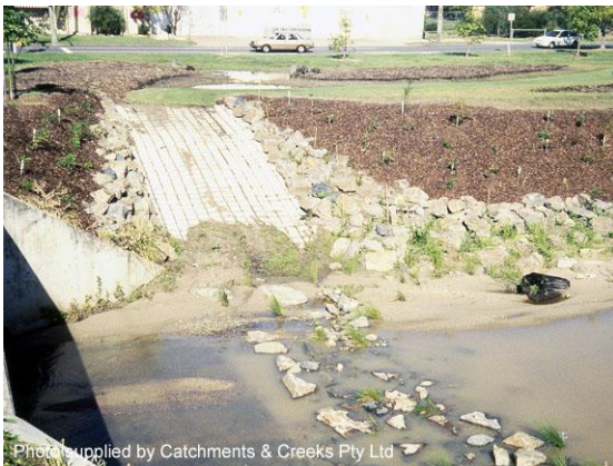
Maintenance access ramp (1997)
