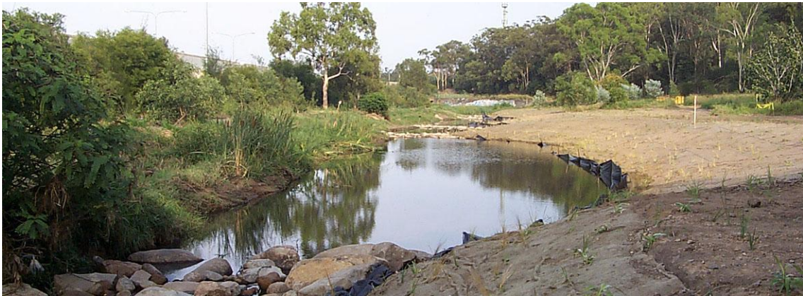
Looking downstream to culvert (2001)
