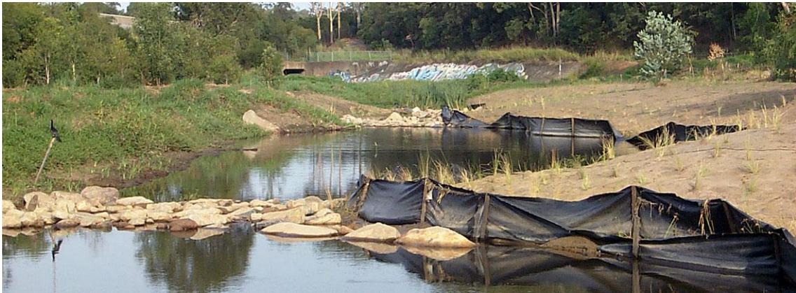
Looking downstream to culvert (2001)
