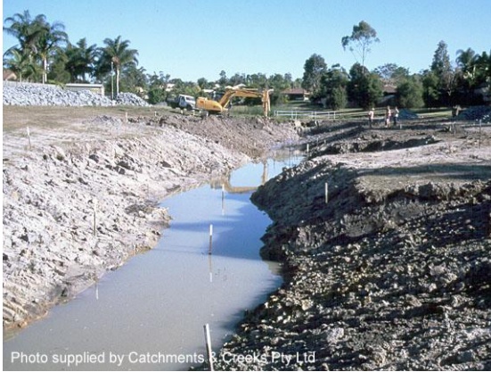
Looking u/s, construction phase (1999)
