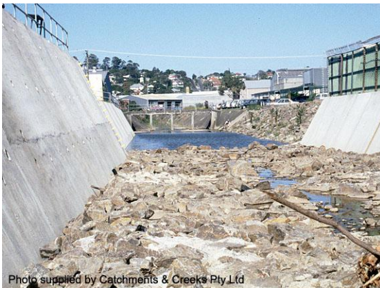
Grouted rock bed on concrete channel
