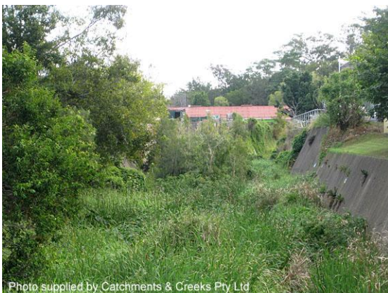
Looking upstream from footbridge (2014)
