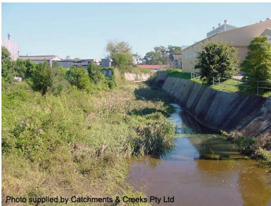
Looking upstream Magura St (2003)
