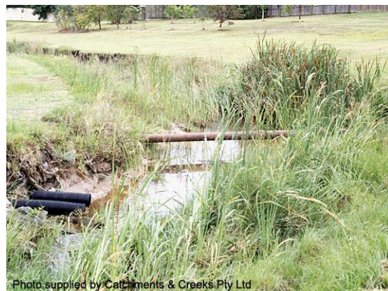
Exposed Ag-pipe & sewer crossing (1997)
