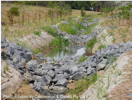
Pool-riffle system (looking upstream)
