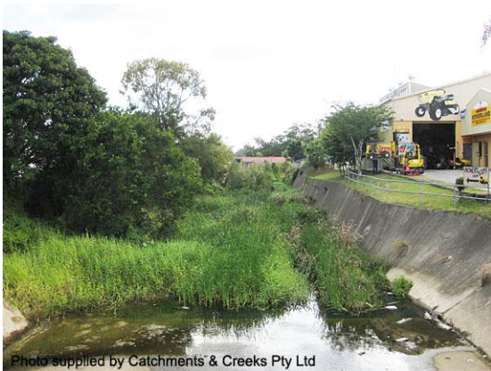
Looking upstream Magura St (2014)
