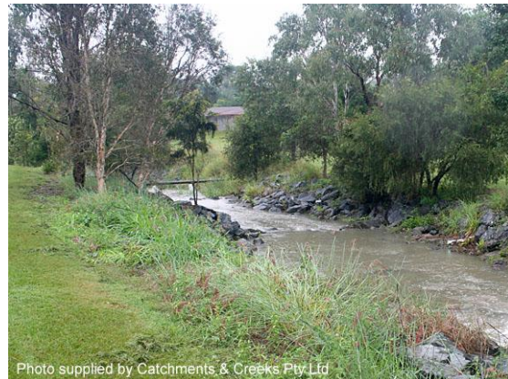
Sewer pipe crossing (2010)
