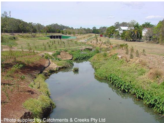
Following first stage of works (2001)
