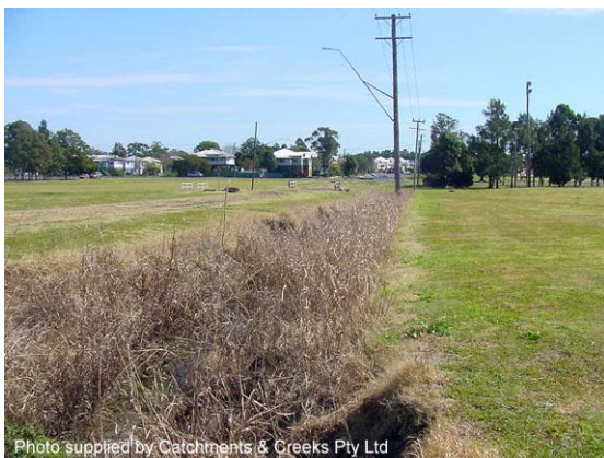
Pre-works site conditions (2003)
