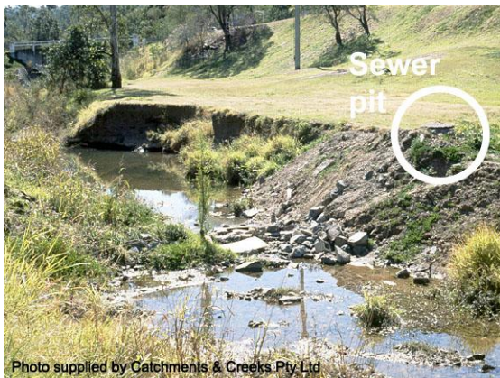
Looking u/s towards Moggill Rd (1991)
