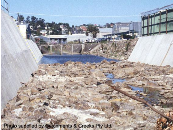
Looking d/s to Magura St footbridge
