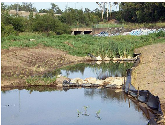
Looking downstream to culvert (2001)
