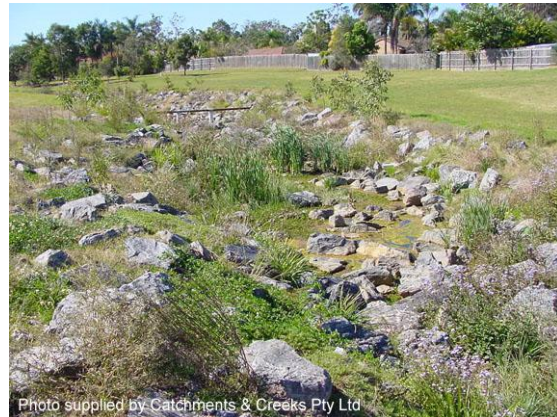
Sewer pipe crossing (2000)
