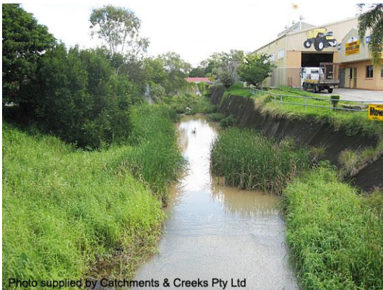
Looking upstream Magura St (2011)
