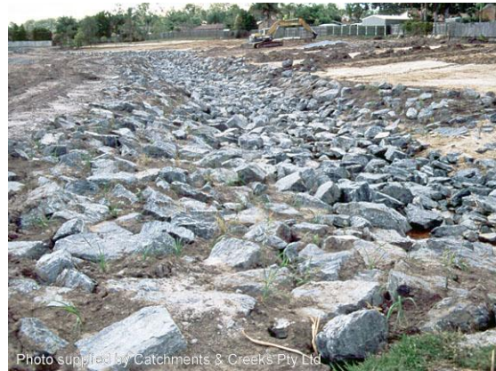
Sewer pipe crossing (1999)
