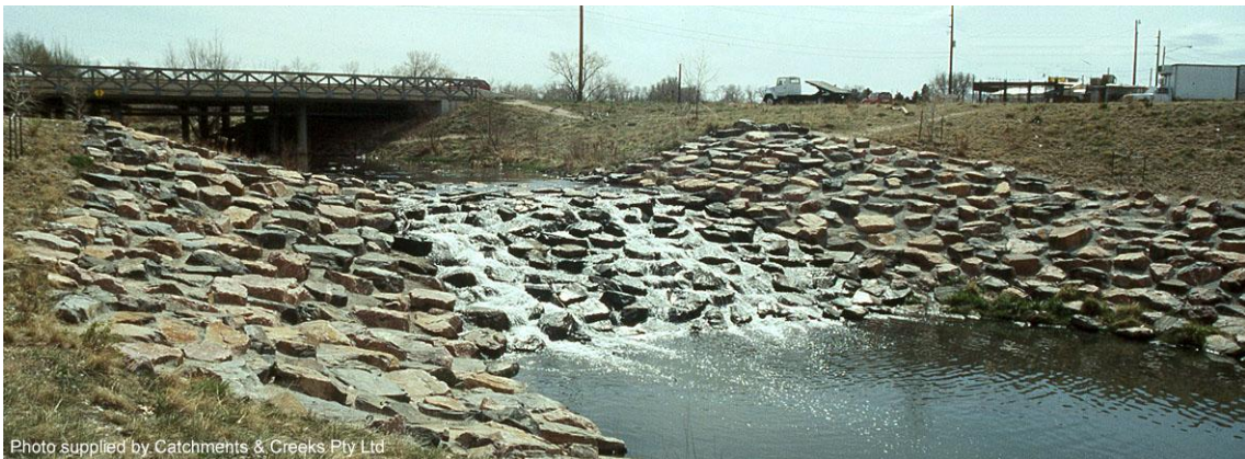
Grouted boulder drop structure, Denver (1995)
