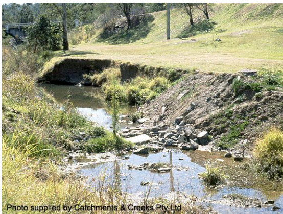
Protection of sewer with rubble (1991)
