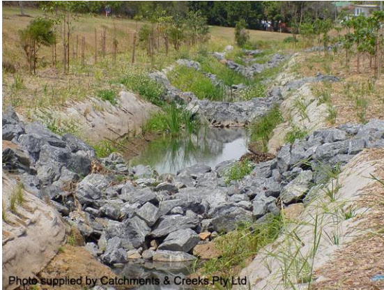
Constructed pool-riffle system (2001)
