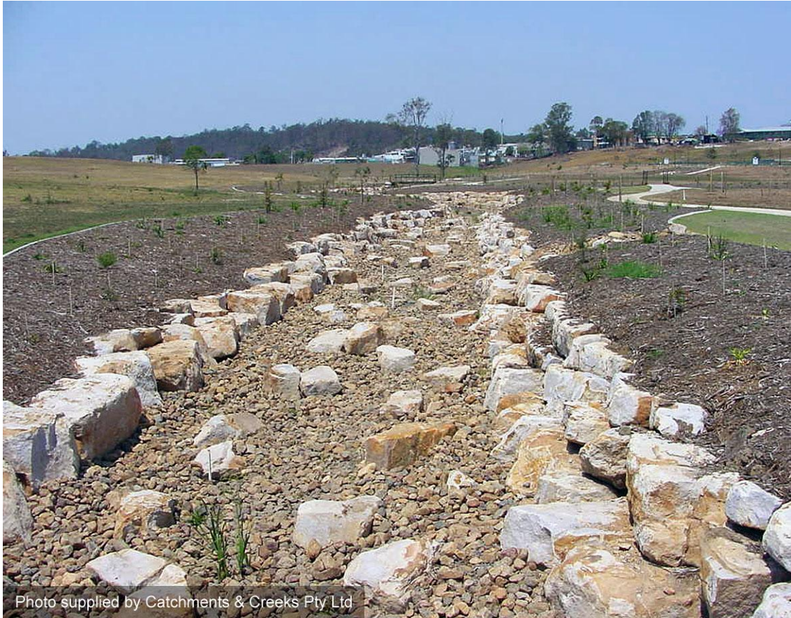
Constructed waterway looking downstream from the Sinnamon Road culvert (2000)
