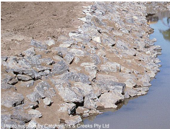
Soil-filled voids ready for planting (1999)
