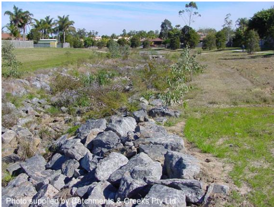
Looking upstream to footbridge (2000)
