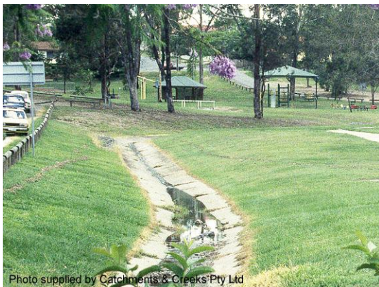
Original concrete drain (1998)
