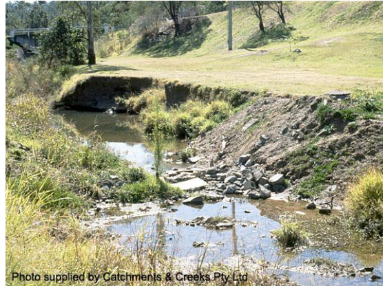
Looking u/s towards Moggill Rd (1991)
