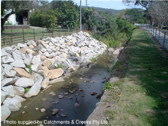
Upstream end of works (2005)
