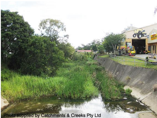
Looking upstream Magura St (2014)
