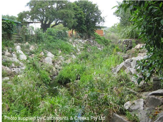
Upstream end of works (2012)
