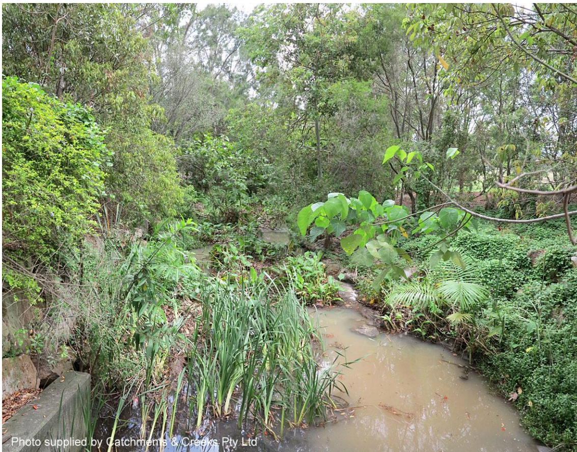
Looking downstream from Sinnamon Road culvert (2014)
