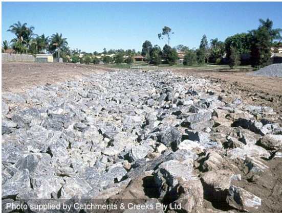
Looking upstream to footbridge (1999)
