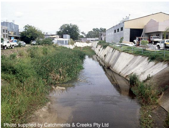
Looking upstream Magura St (1999)
