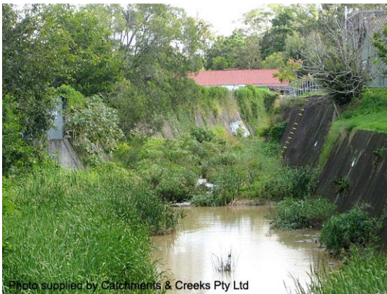
Looking upstream from footbridge (2011)
