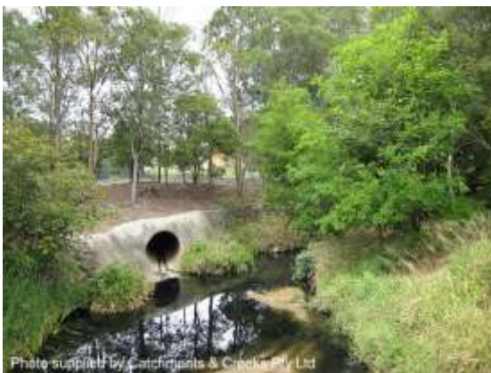
Looking upstream Pickering St (2014)
