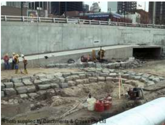
Construction of a weir (1995)
