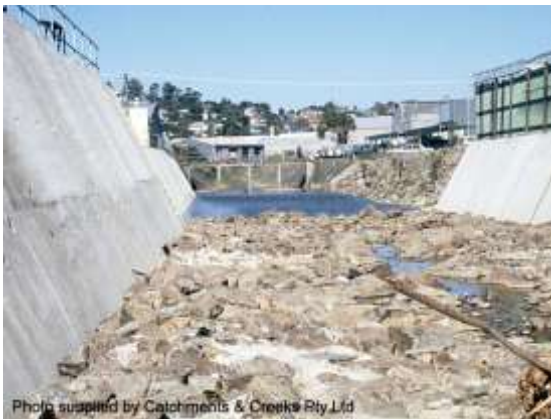
Grouted rock bed on concrete channel
