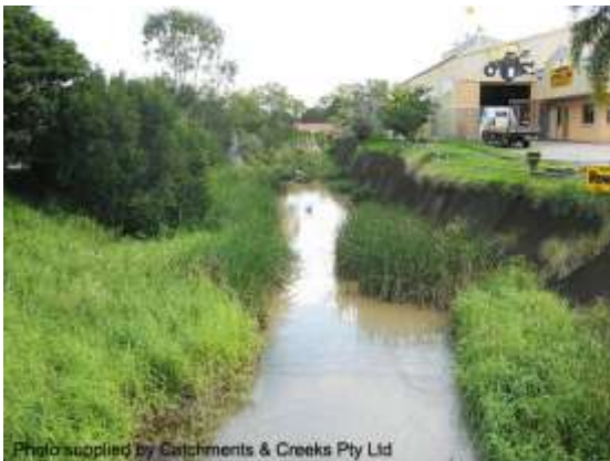
Looking upstream Magura St (2011)
