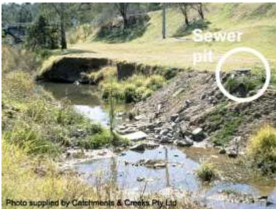
Looking u/s towards Moggill Rd (1991)
