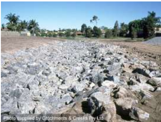
Looking upstream to footbridge (1999)
