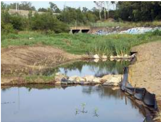
Looking downstream to culvert (2001)
