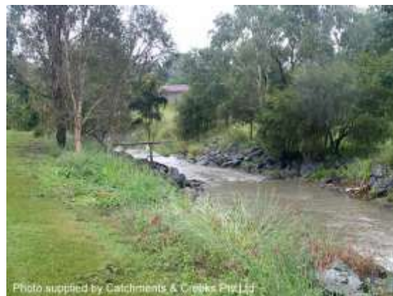
Sewer pipe crossing (2010)
