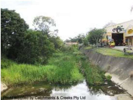
Looking upstream Magura St (2014)
