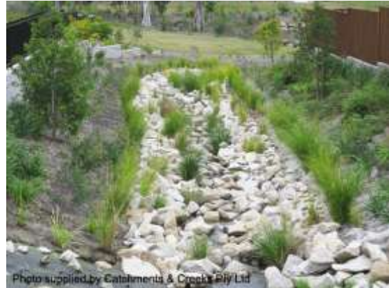
Looking d/s from Settlement Rd (2012)
