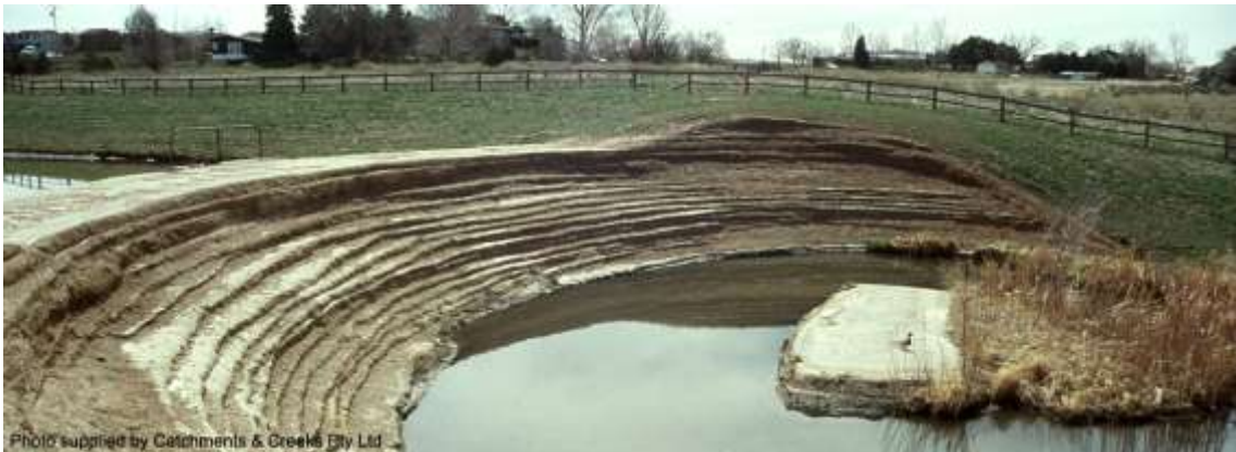
Rolled soil-cement drop structure, Denver (1995)
