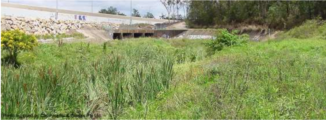
Looking downstream to culvert (2000)
