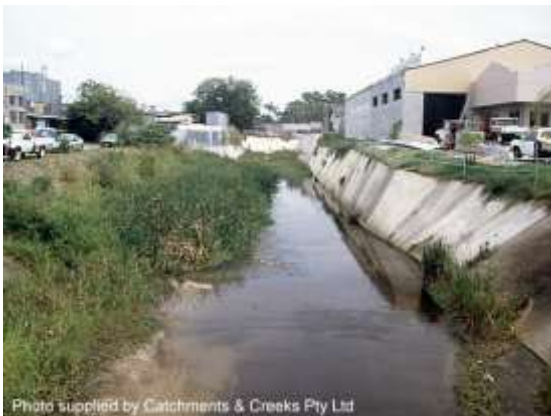
Looking upstream Magura St (1999)
