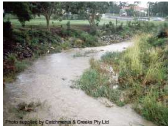
Looking downstream Pickering St (1998)
