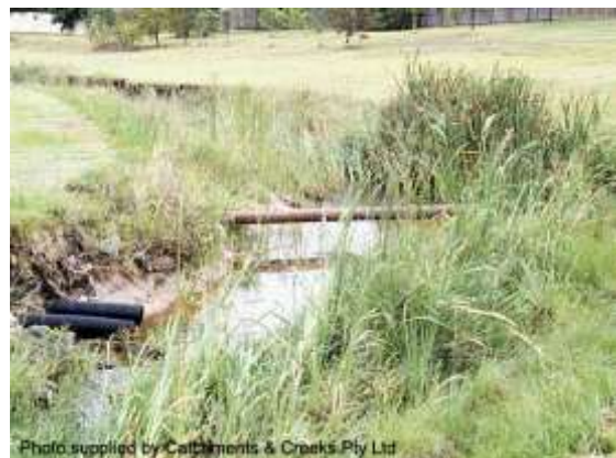
Exposed Ag-pipe & sewer crossing (1997)
