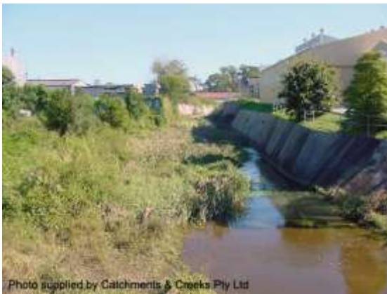
Looking upstream Magura St (2003)
