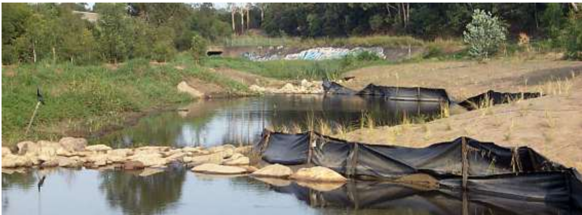
Looking downstream to culvert (2001)
