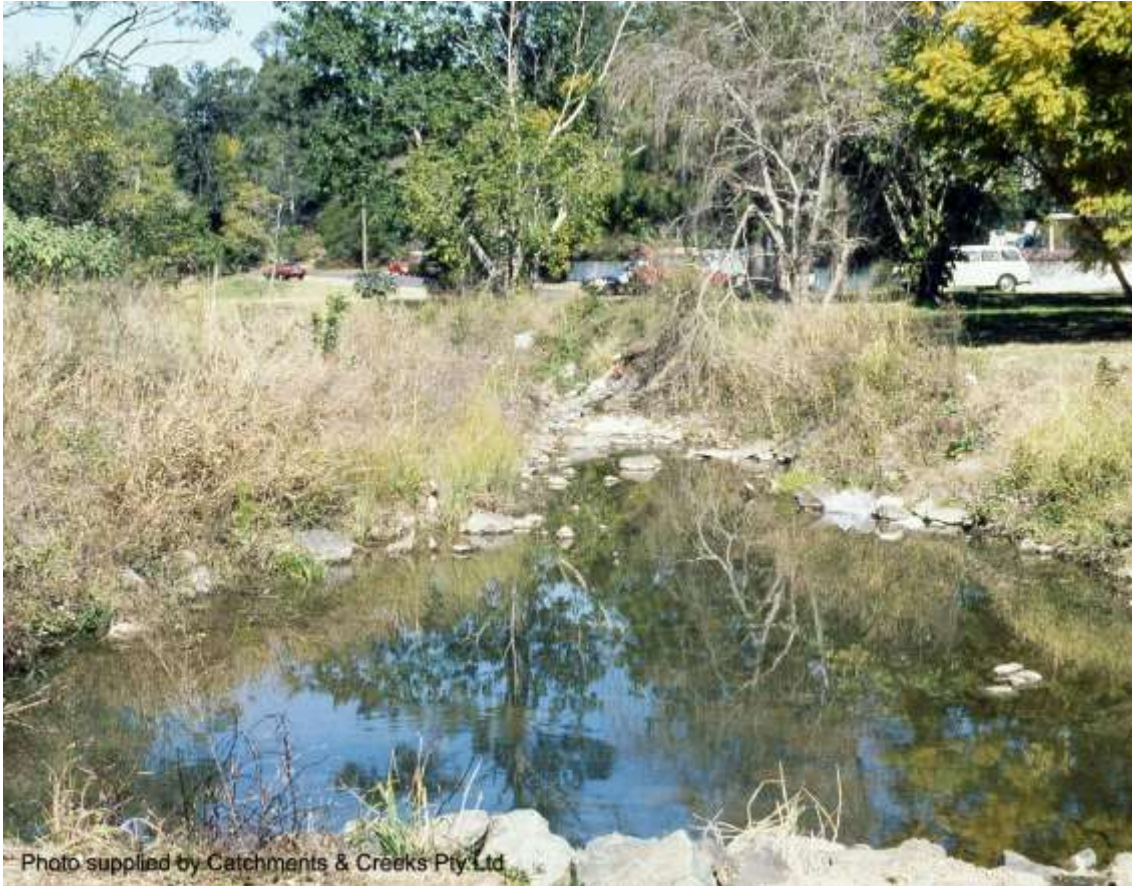
Looking downstream from the Moggill Road culvert (1991)
