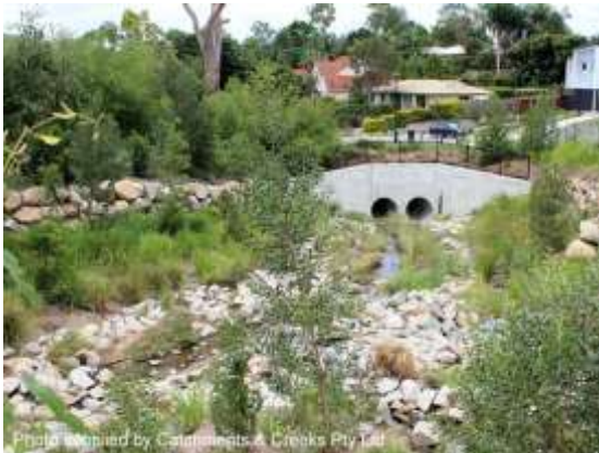
Modified creek channel u/s of Tilquin St
