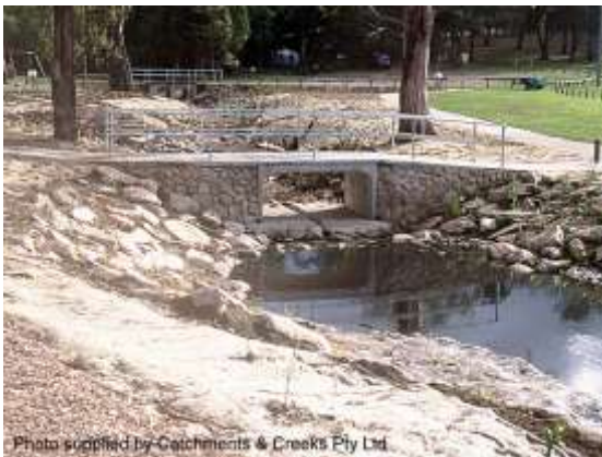
New footbridge (d/s of junction, 2000)
