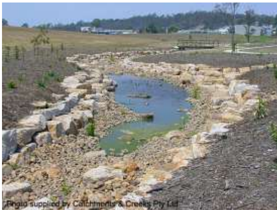
Looking downstream to footbridge (2000)
