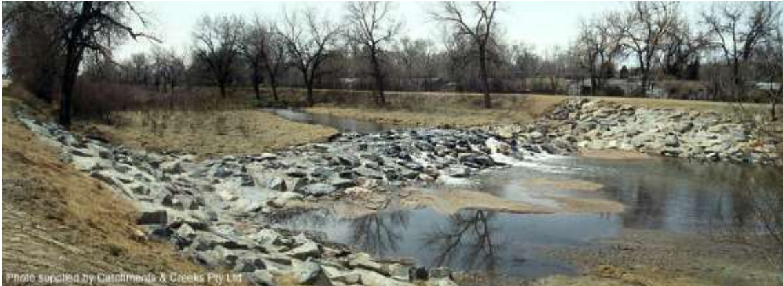
Grouted rock drop structure, Denver (1995)
