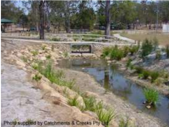
Looking u/s to footbridge (2000)
