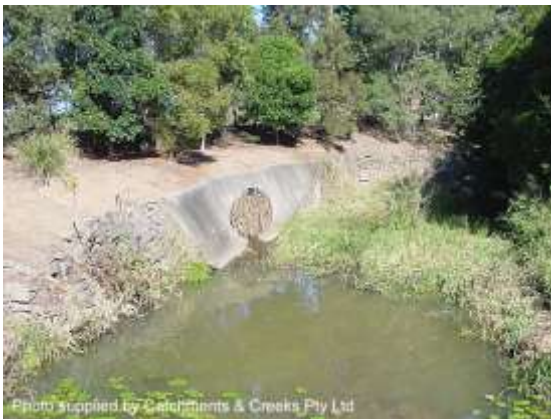
Looking upstream Pickering St (2003)
