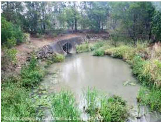
Looking upstream Pickering St (2007)
