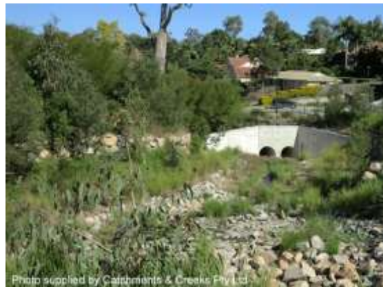
Looking d/s to Tilquin St (May 2013)
