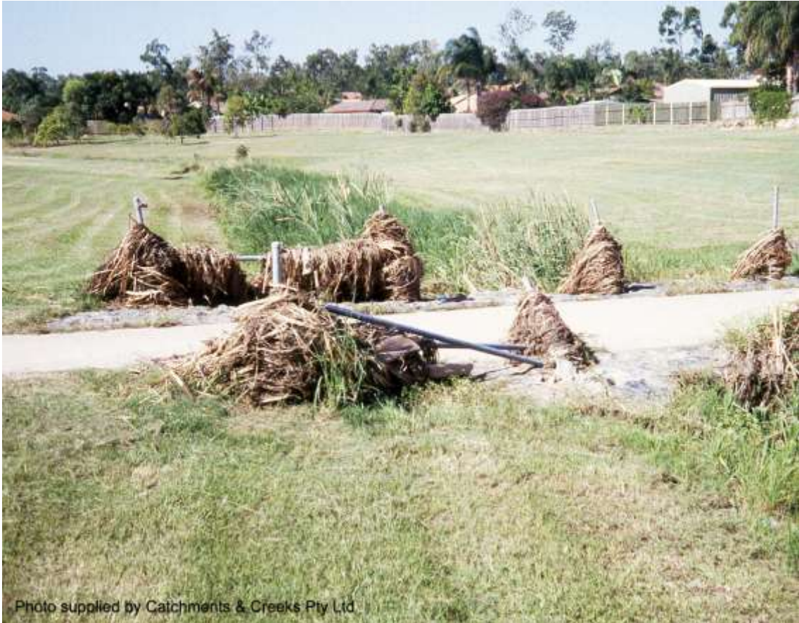
Looking downstream towards the footbridge (1997)
