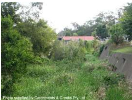
Looking upstream from footbridge (2014)
