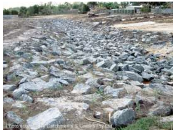
Sewer pipe crossing (1999)
