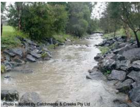
Looking upstream to footbridge (2010)
