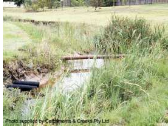
Sewer pipe crossing (1997)
