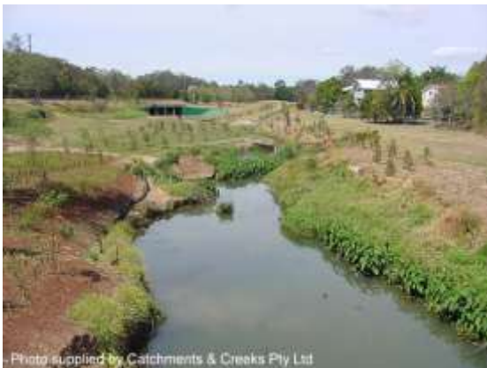
Following first stage of works (2001)
