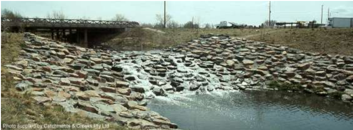
Grouted boulder drop structure, Denver (1995)
