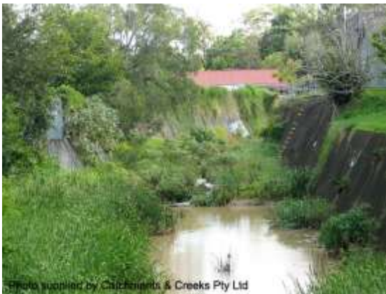
Looking upstream from footbridge (2011)
