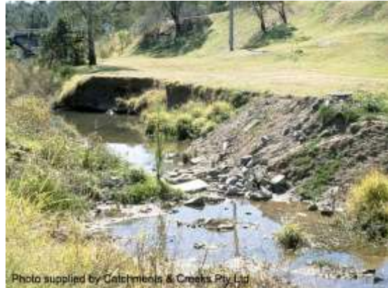
Looking u/s towards Moggill Rd (1991)
