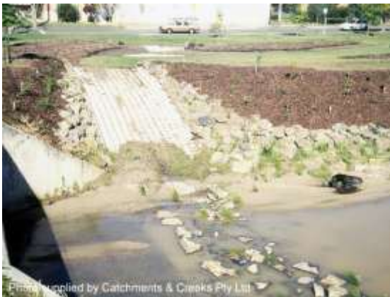
Maintenance access ramp (1997)
