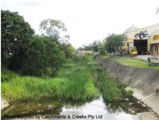
Looking upstream Magura St (2014)
