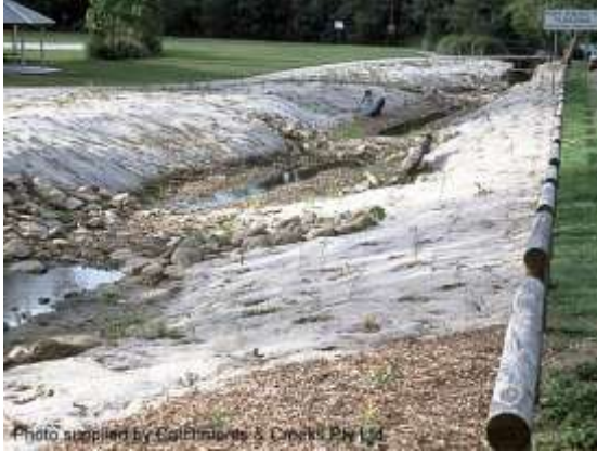
Pool-riffle system (2000)
