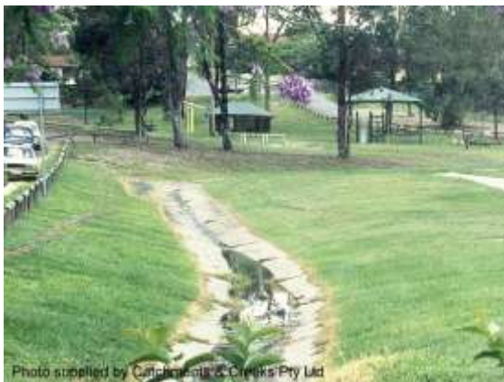
Original concrete drain (1998)
