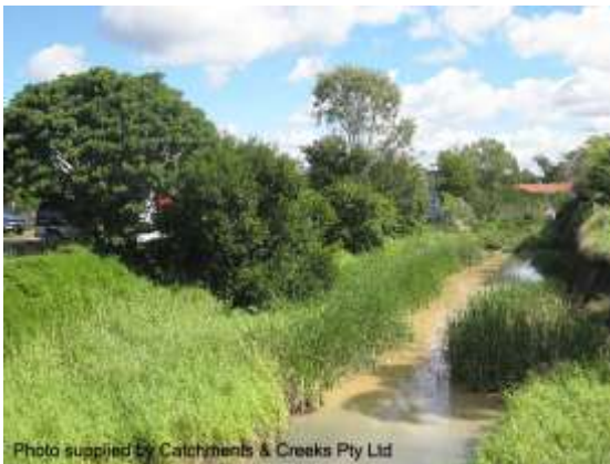
Looking upstream Magura St (2011)
