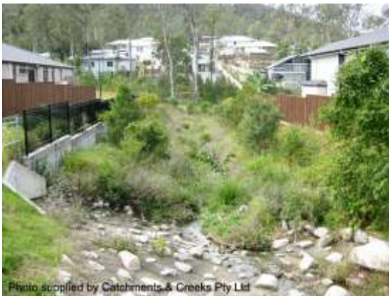
Looking d/s from Settlement Rd (2014)
