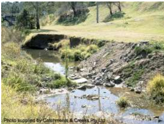
Protection of sewer with rubble (1991)
