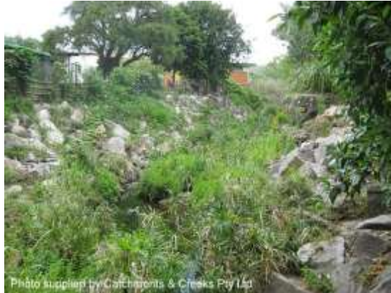
Upstream end of works (2012)
