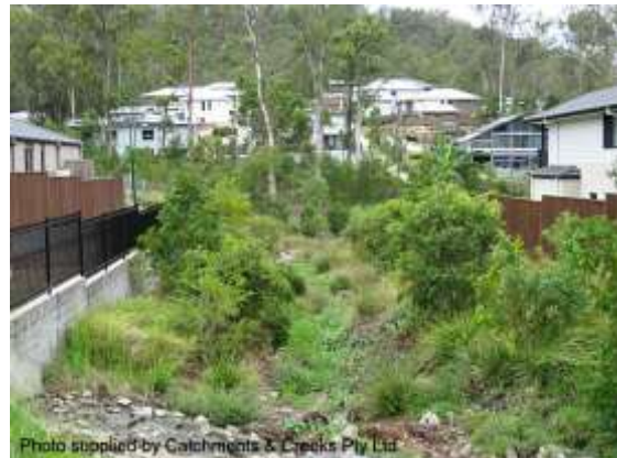
Looking d/s from Settlement Rd (2014)
