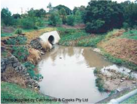
Looking upstream Pickering St (1997)
