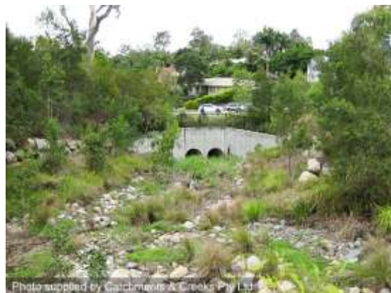
Looking d/s to Tilquin St (2014)
