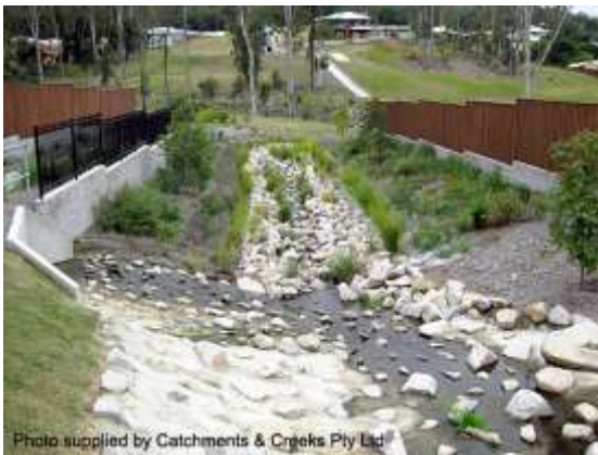
Constructed drainage channel
