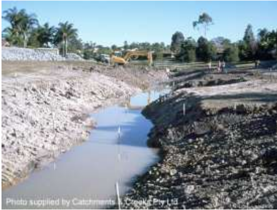
Looking u/s, construction phase (1999)
