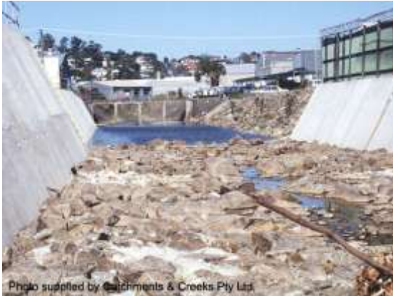
Looking d/s to Magura St footbridge
