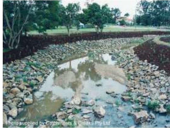
Looking downstream Pickering St (1997)
