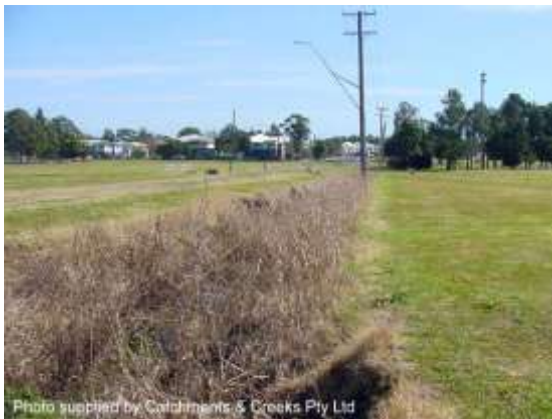
Pre-works site conditions (2003)
