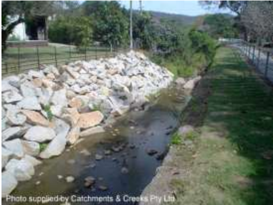
Upstream end of works (2005)
