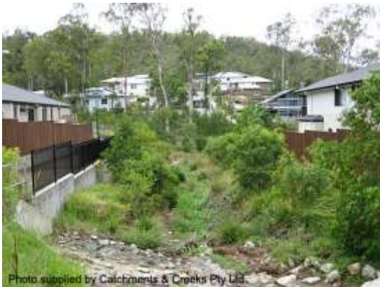
Looking d/s from Settlement Rd (2014)
