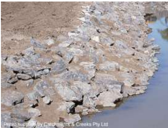
Soil-filled voids ready for planting (1999)
