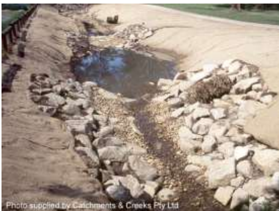
Pool-riffle system (2000)
