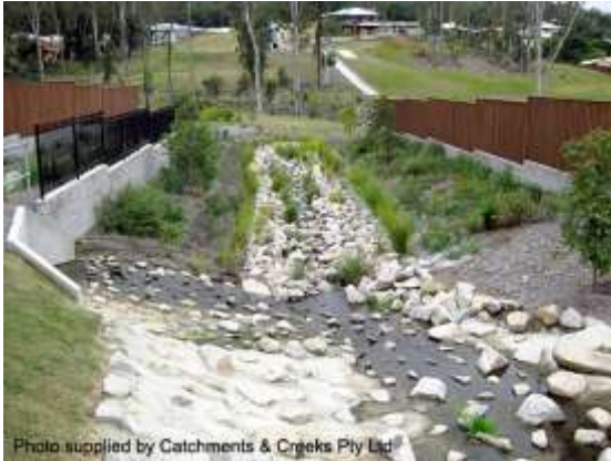
Looking d/s from Settlement Rd (2012)
