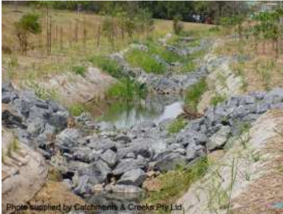
Constructed pool-riffle system (2001)
