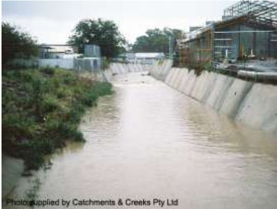
Looking upstream Magura St (1998)
