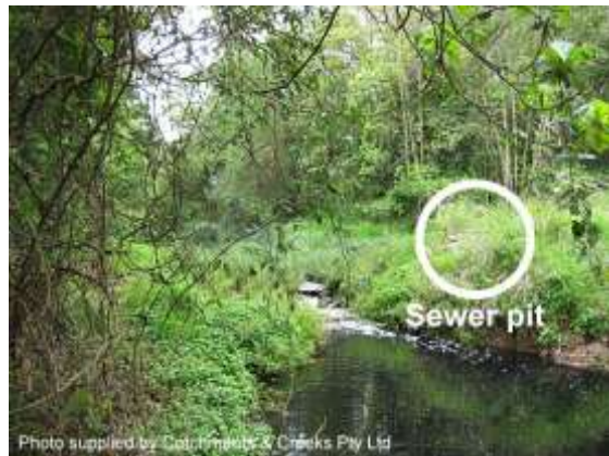
Looking u/s towards Moggill Rd (2014)
