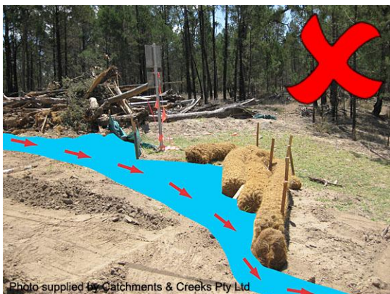
Stormwater runoff bypasses sediment trap
