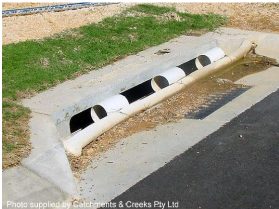
Sag-type kerb inlet sediment trap
