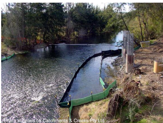
Sediment fence isolation barrier
