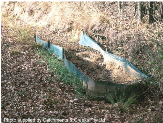
U-shaped sediment trap
