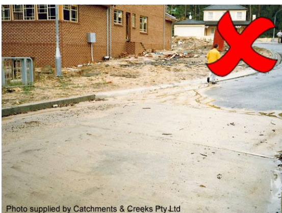
Sediment deposition on a roadway
