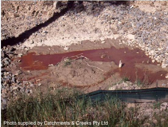
Acidic runoff draining into a pond
