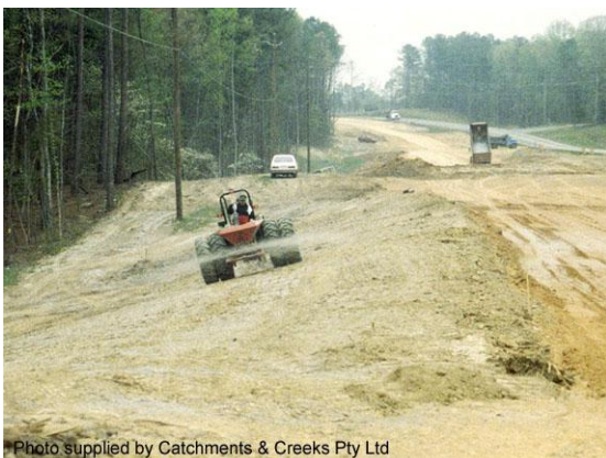
Slope being prepared for revegetation
