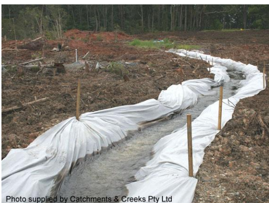
Temporary drain lined with filter cloth
