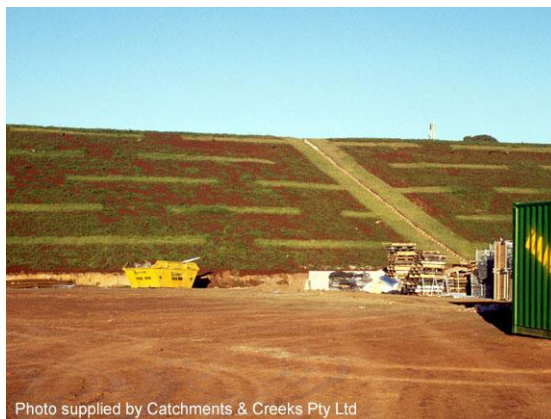
Turf filter strips on a steep slope
