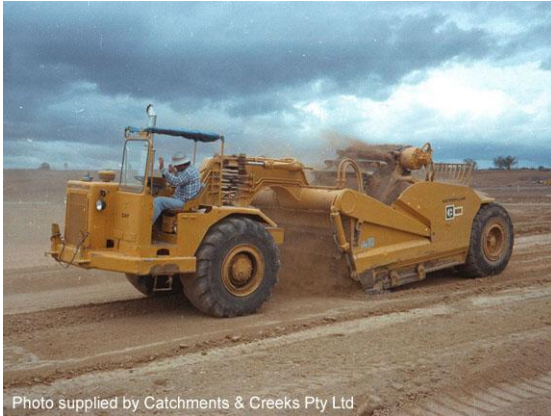
Scraper stripping soil
