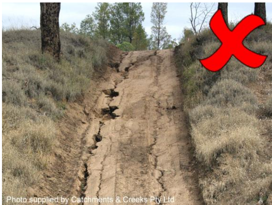
Drainage damage to an access road
