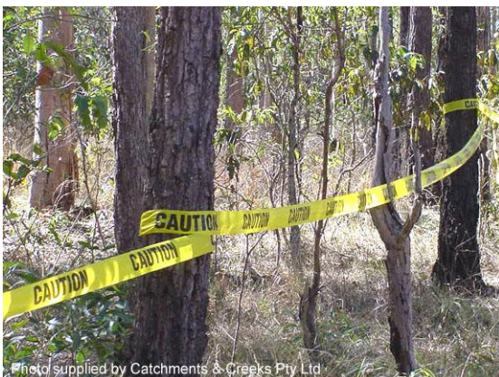
Marking the limits of planned land clearing
