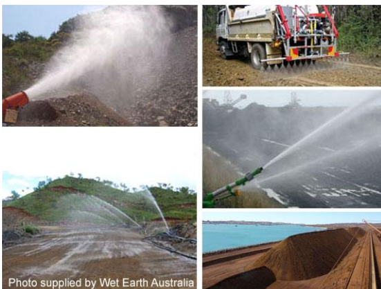
Use of dust control soil binders
