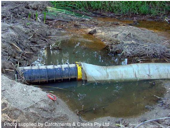
Filter tube attached to an embankment
