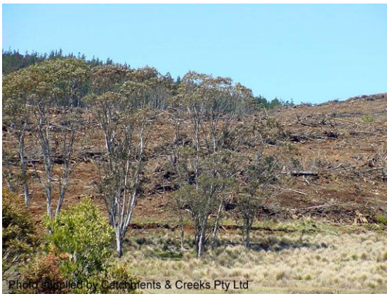
Tree clearing with minimal soil disturbance
