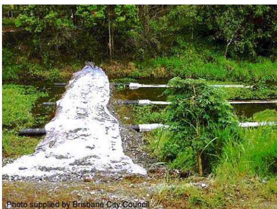
In-stream rock filter dam with filter tubes
