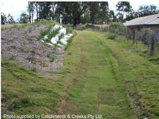
Wide, shallow, grass-lined drain
