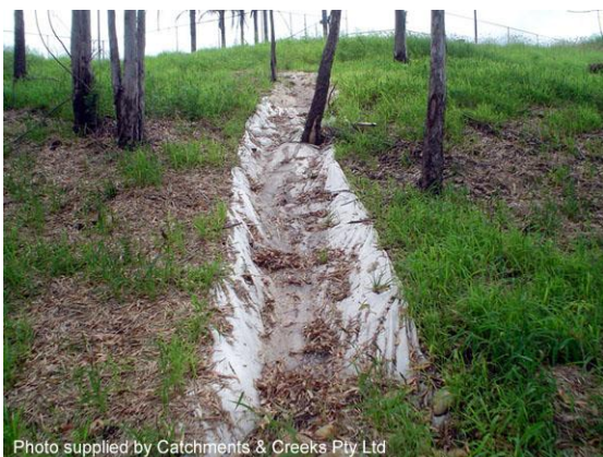
Batter chute lined with filter cloth
