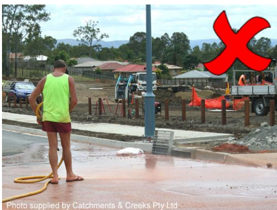
Inappropriate clean-up procedure
