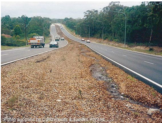
Loose mulch displaced by a storm
