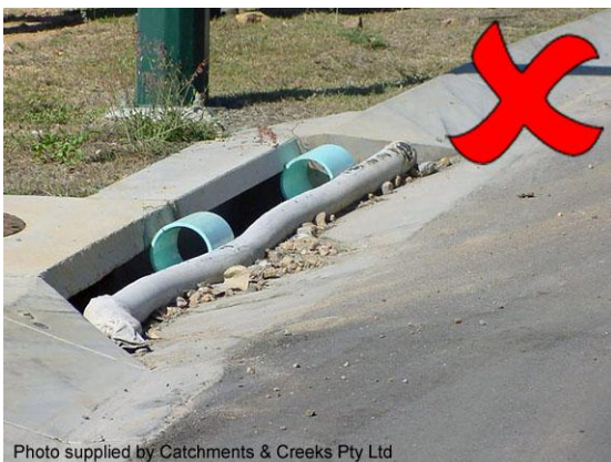
Fully blocked on-grade gully inlet
