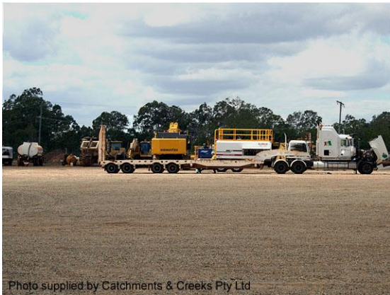
Gravelled work compound
