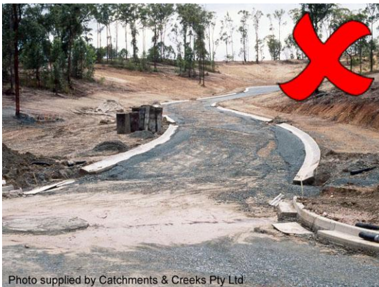
Site with limited drainage & erosion control
