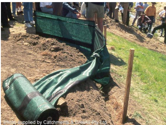
Installation of a sediment fence
