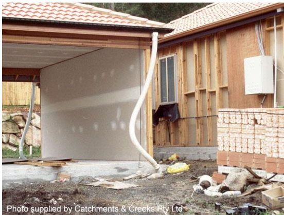
Temporary roof water connection
