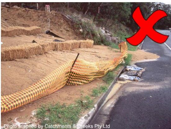
Failed sediment control measures
