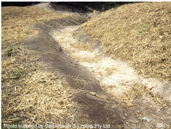
Loss of mulch by concentrated storm flow
