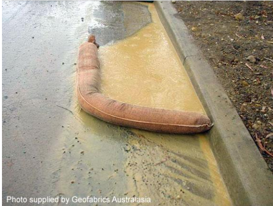
Sand-filled filter sock
