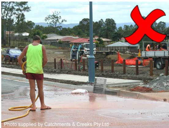
Poor maintenance practice
