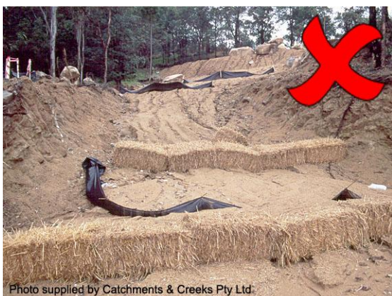
Failed sediment traps on a steep ramp
