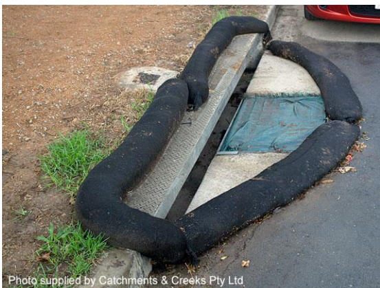
Sag inlet sediment trap
