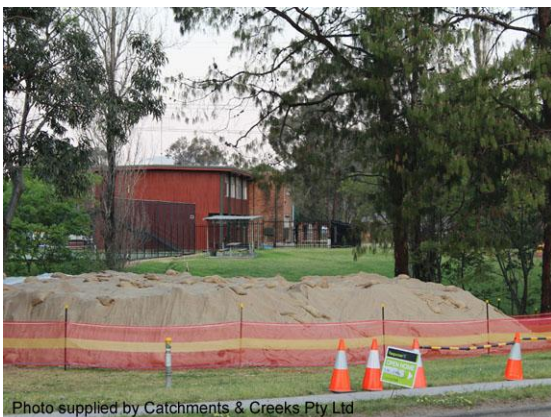
Stockpile covered with jute blankets
