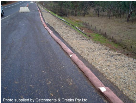
Temporary flow diversion system
