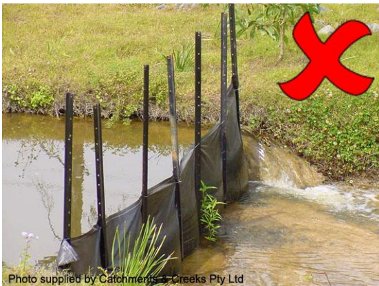
Poorly-designed sediment trap
