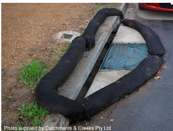
Sag-type kerb inlet protection
