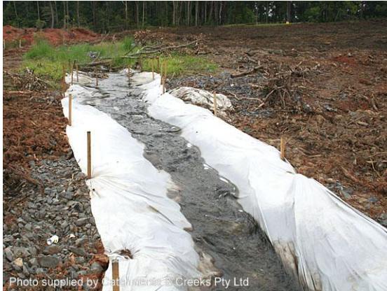
Control of 'clean' run-on water
