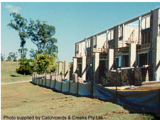
Sediment fence adjacent to a building site
