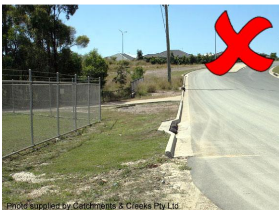
Sediment simply flows off the roadway
