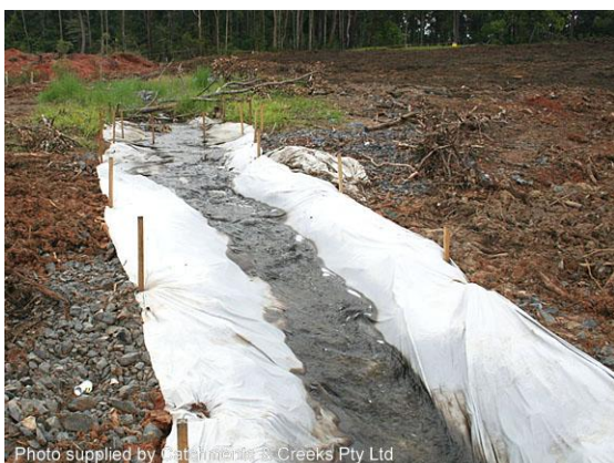
Diversion of 'clean' run-on water
