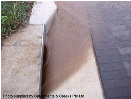
Poor runoff water quality
