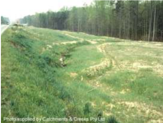
Temporary grassing of active road works
