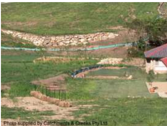
Straw bales diverting stormwater runoff
