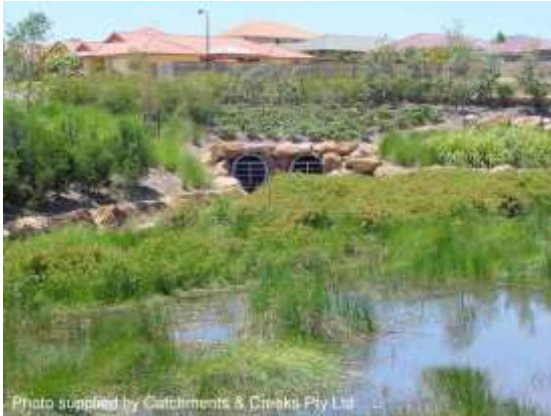
Stormwater treatment wetland
