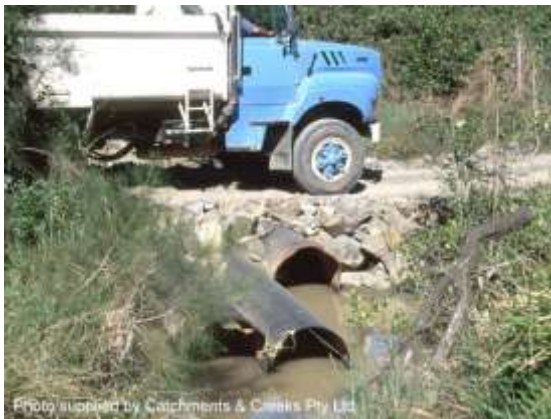
Temporary culvert crossing
