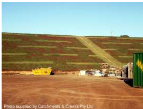
Turf filter strips on a steep slope
