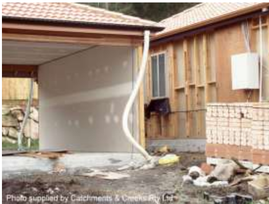
Temporary roof water connection
