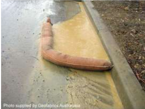
Sand-filled filter sock
