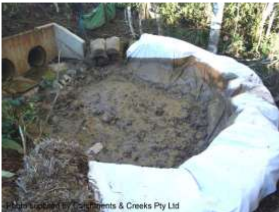
Straw bale sediment trap on a steep slope
