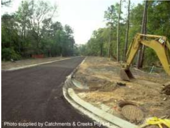
New subdivision with retained vegetation
