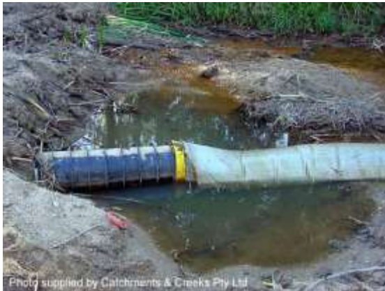
Filter tube attached to an embankment
