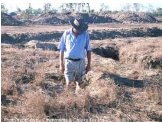
Tunnelling within a dispersive soil
