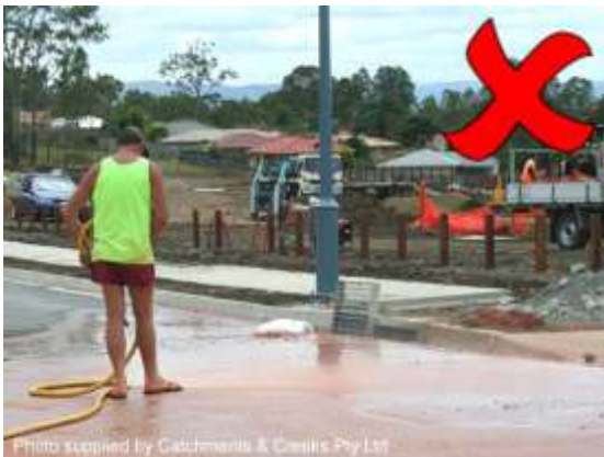
Poor maintenance practice
