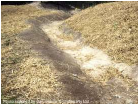
Loss of mulch by concentrated storm flow
