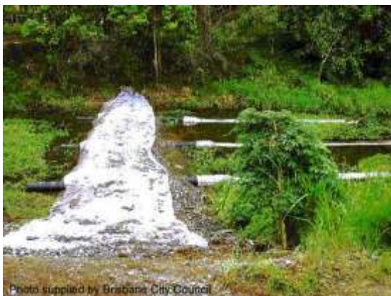
Instream rock filter dam with filter tubes
