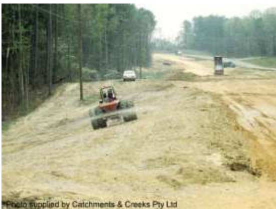
Slope being prepared for revegetation
