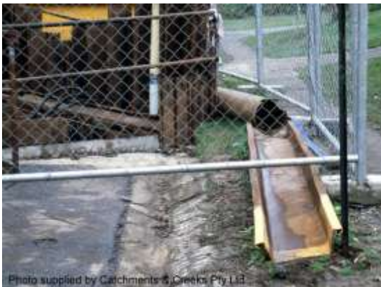
Stormwater diverted around a pit
