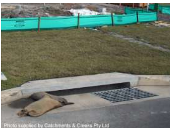
On-grade kerb inlet sediment trap
