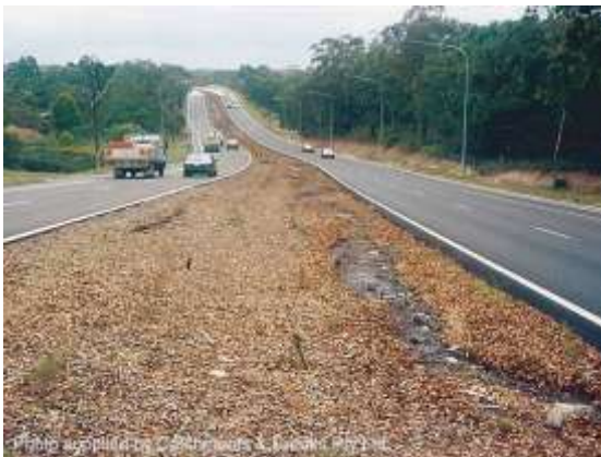
Loose mulch displaced by a storm
