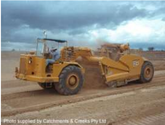
Scraper stripping soil
