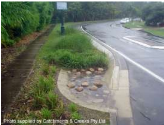
Roadside biofiltration cell
