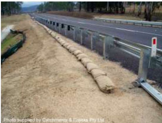
Road runoff diverted away from a slope
