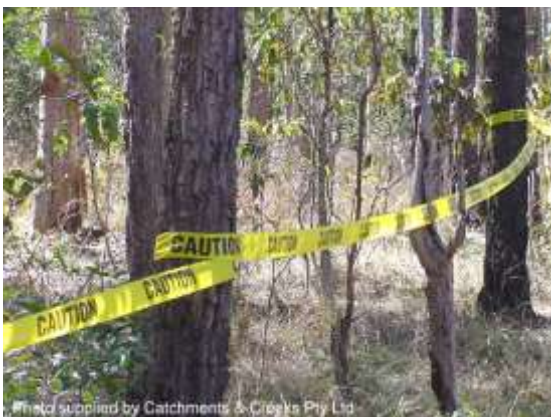
Marking the limits of planned land clearing
