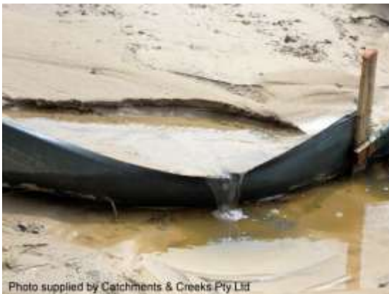
Sediment fence with settled sediment
