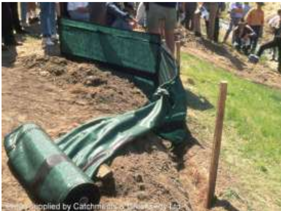
Installation of a sediment fence
