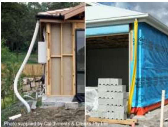
Temporary downpipes
