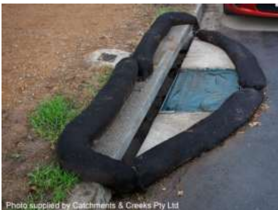
Sag-type kerb inlet protection
