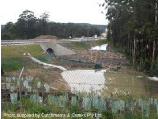
Post-construction sediment basins
