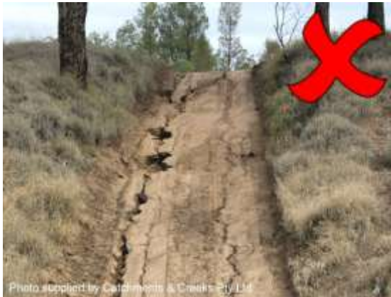
Drainage damage to an access road
