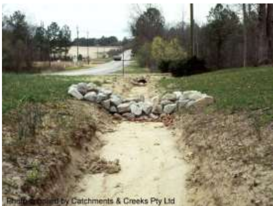
Rock check dam
