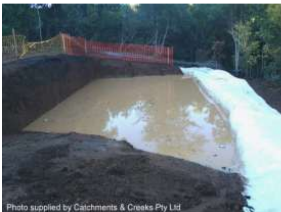
Basin full and ready to overflow
