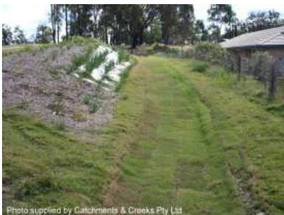
Wide, shallow, grass-lined drain
