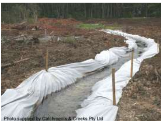
Temporary drain lined with filter cloth
