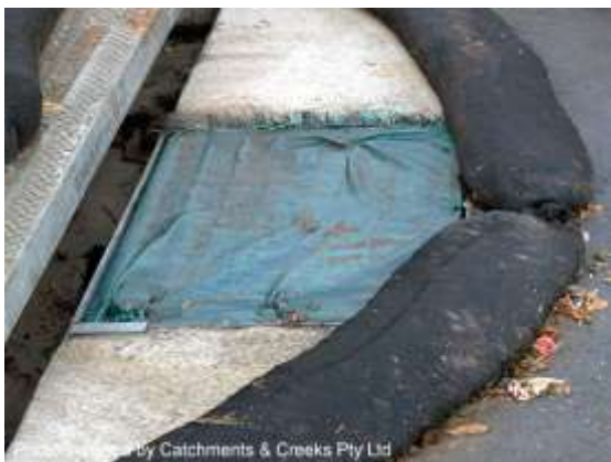
Inappropriate use of fabrics
