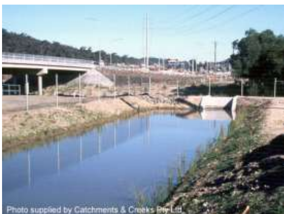
Type D sediment basin
