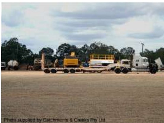
Gravelled work compound
