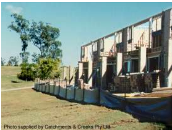
Sediment fence adjacent to a building site
