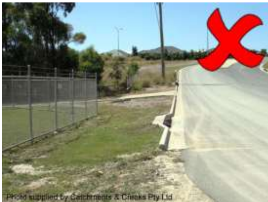
Sediment simply flows off the roadway
