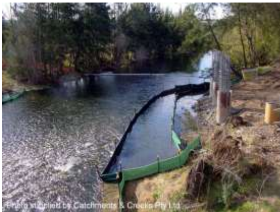
Sediment fence isolation barrier
