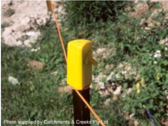
Safety cap on a support stake
