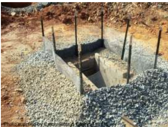
Mesh and aggregate drop inlet protection
