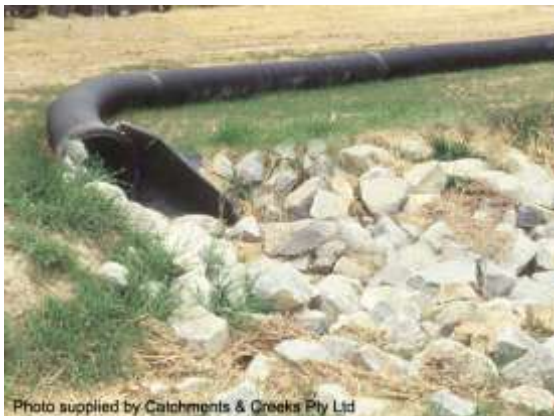
Diversion drain outlet structure
