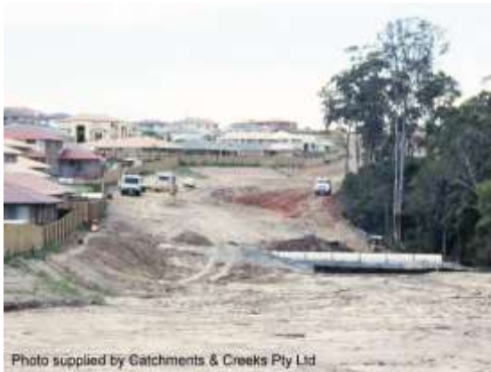
Early installation of stormwater pipe
