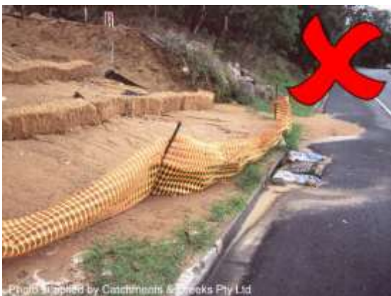
Failed sediment control measures
