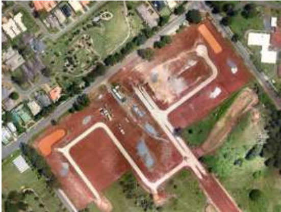
Construction site with sediment basins
