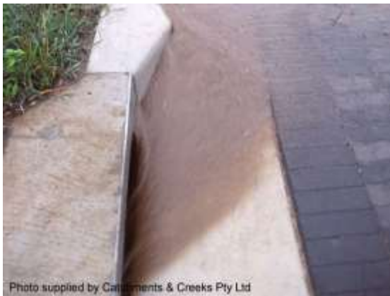
Poor runoff water quality
