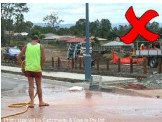
Inappropriate clean-up procedure
