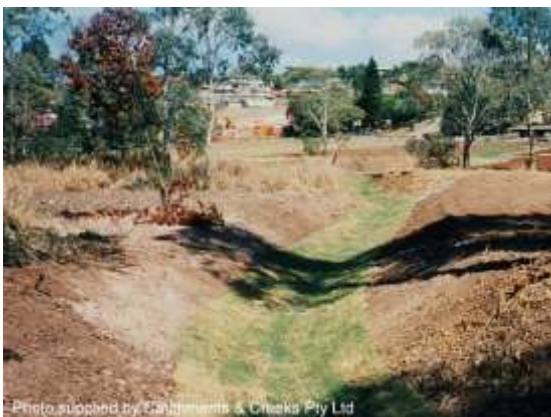
Early establishment of a diversion drain
