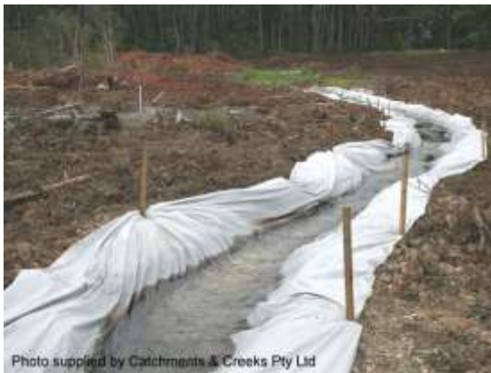
'Clean' water diversion drain
