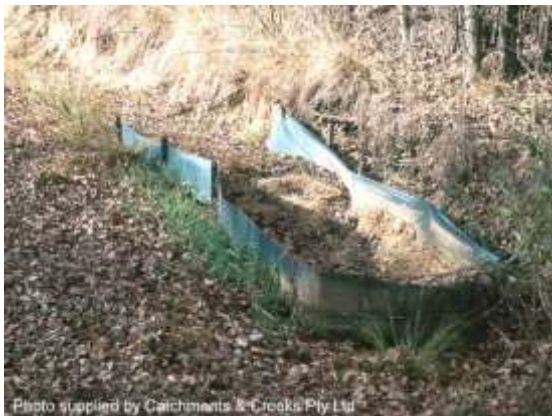
U-shaped sediment trap
