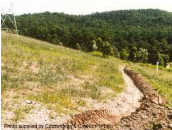
Unlined catch drain
