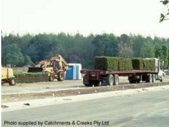
Delivery of turf to a construction site
