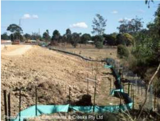
Sediment fence with regular 'returns'
