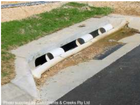
Sag-type kerb inlet sediment trap
