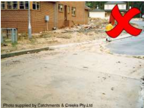
Sediment deposition on a roadway
