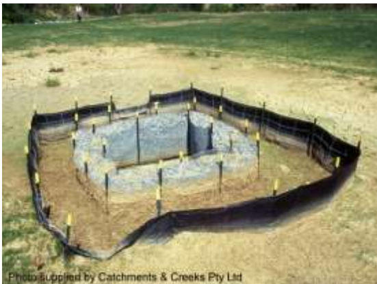
Sediment weir surrounding a field inlet
