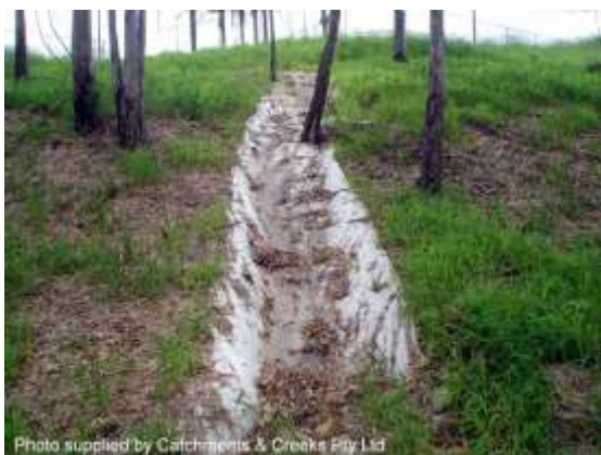
Batter chute lined with filter cloth
