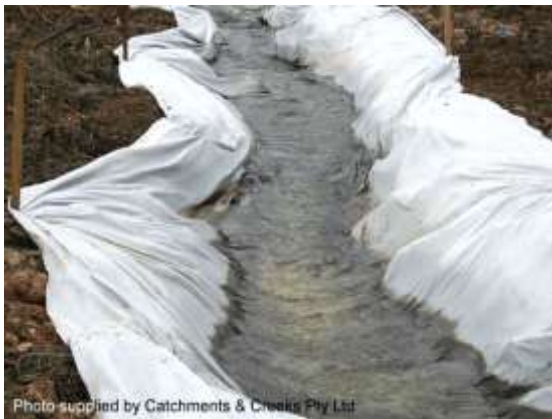
Temporary 'clean' water diversion drain
