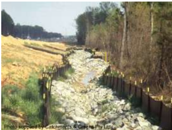
Protection of permanent storm drain
