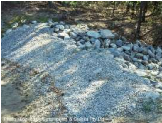
Rock filter dam with aggregate filter
