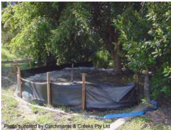
Off-stream filter pond
