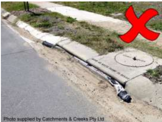
Sediment trap blocking inflows
