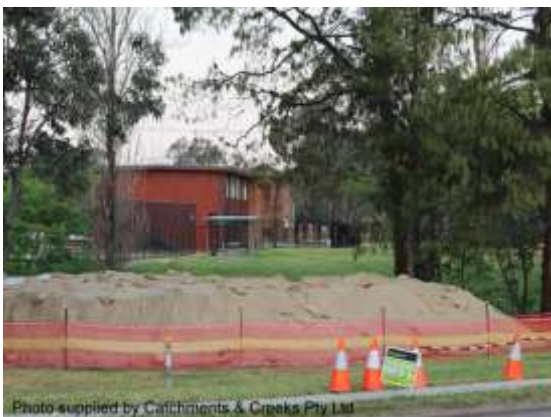
Stockpile covered with jute blankets
