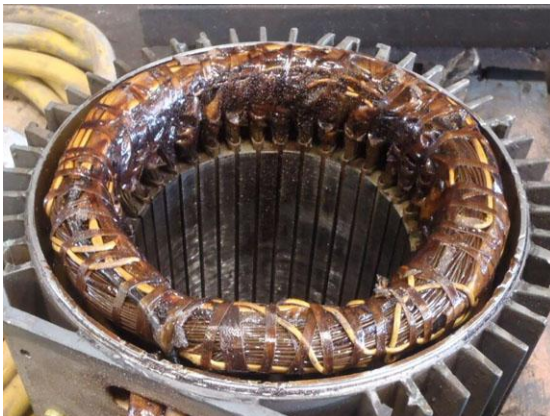
Burnt wiring of an electric motor
