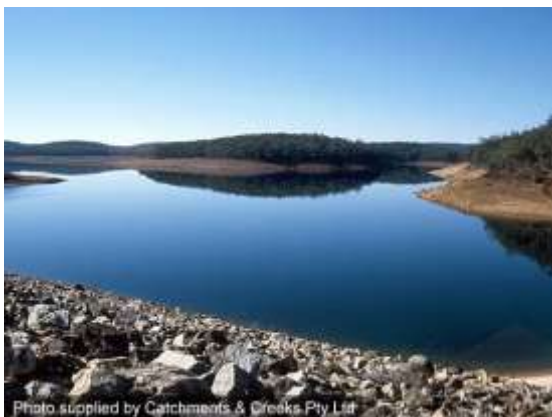
Water supply dam
