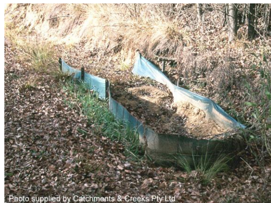
U-shaped sediment trap on steep slope
