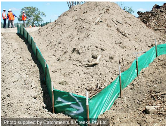
Sediment fence (Type 3)
