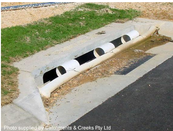
Sag inlet sediment trap
