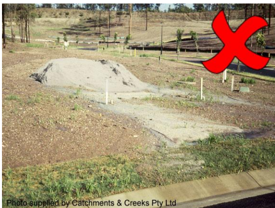
Stockpile locate on an overland flow path
