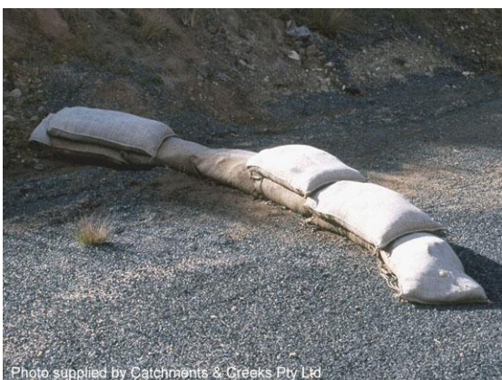
Sandbag sediment trap
