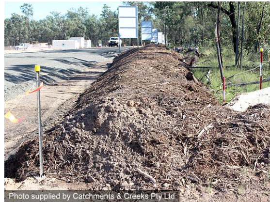
Mulch berm sediment barrier
