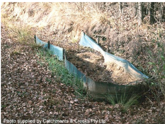
U-shaped sediment trap in steep drain
