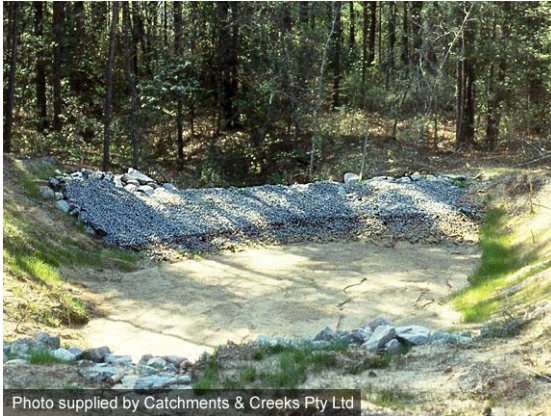
Rock filter dam with aggregate filter
