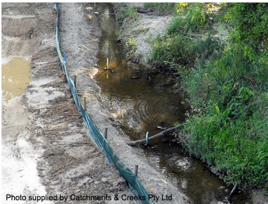
Sediment fence isolation barrier
