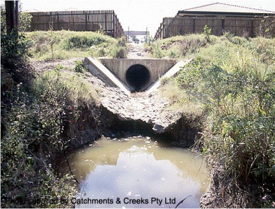
Pipe outlet pre-construction
