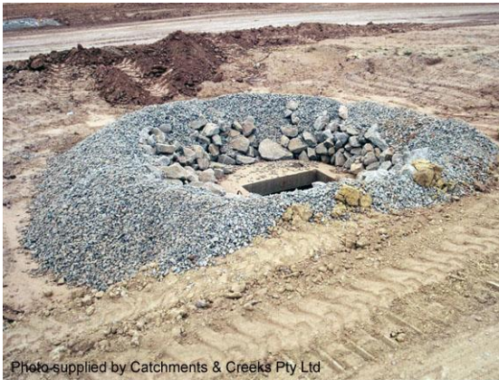
Rock & aggregate drop inlet protection
