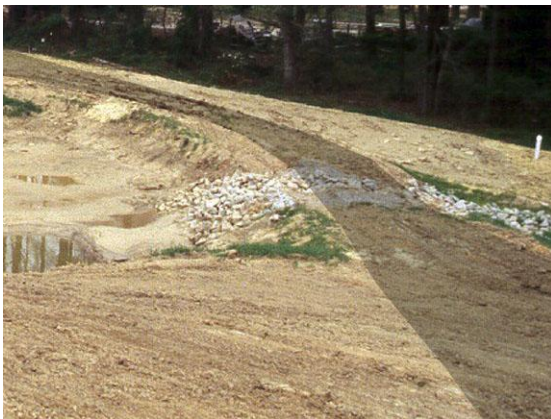
Access road crosses between SB-1 & SB-2
