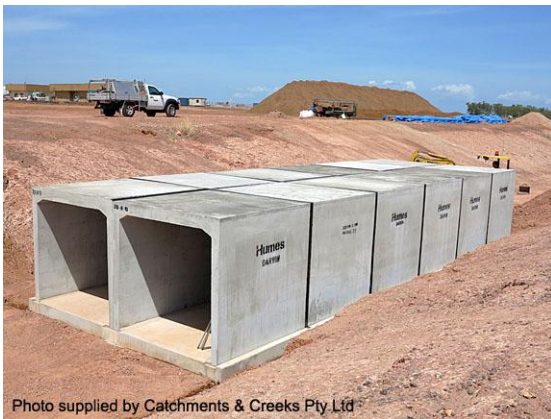
Culvert construction in a dry channel
