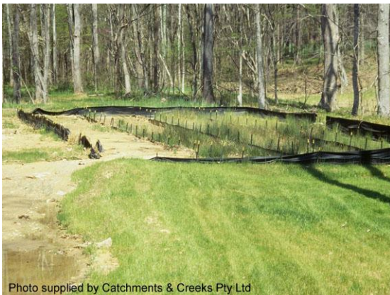
Coarse sediment trap
