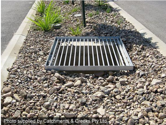
Field inlet located within median strip
