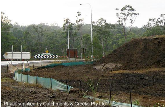
Topsoil stockpile
