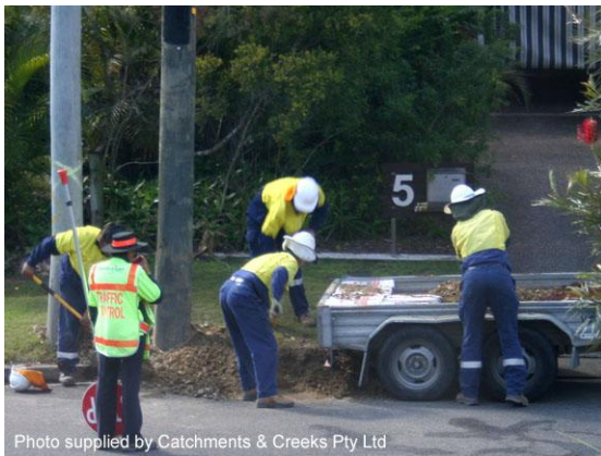
Replacement of telegraph pole
