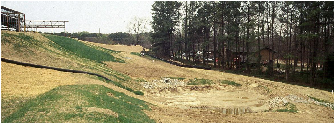
Photo 1: Looking south towards sediment basin 1 and western access road (1995)
