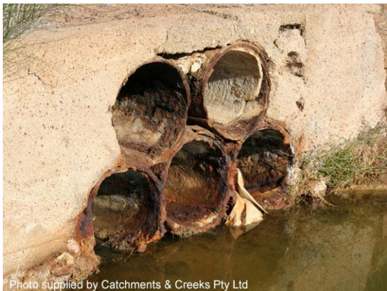
Culvert damaged by acidic water
