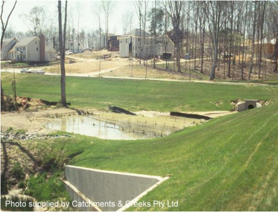
Coarse sediment trap
