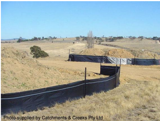
Sediment control down-slope of stockpile
