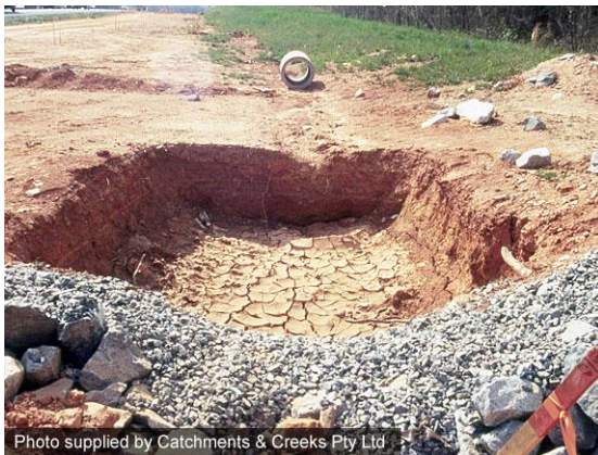
Excavated sediment sump
