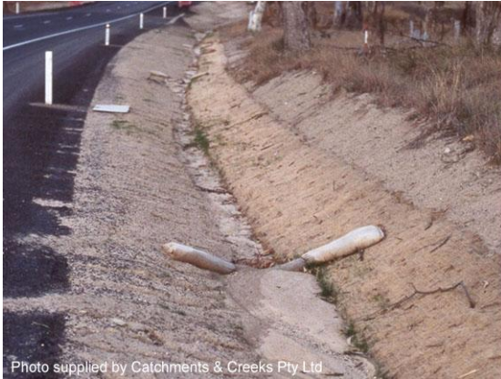
Check dam sediment trap
