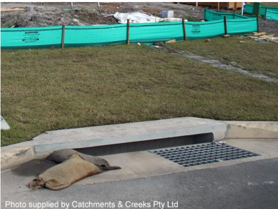
'On-grade' kerb inlet sediment trap
