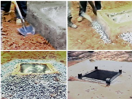
Excavated drop inlet protection
