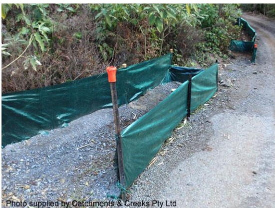
U-shaped sediment trap on mild slope
