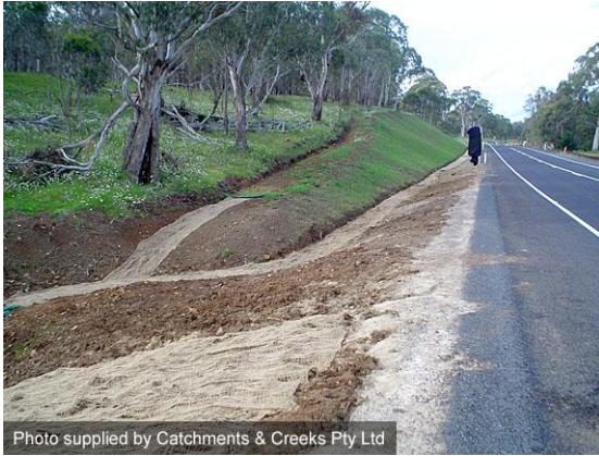
Catch drain and table drain
