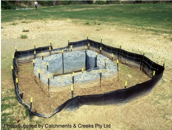
Sediment weir (field inlet protection)
