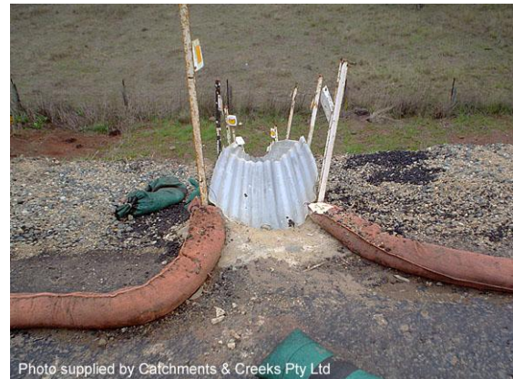
Concrete water seal at chute inlet
