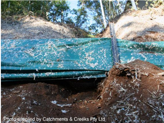
Storm undermines a sediment fence
