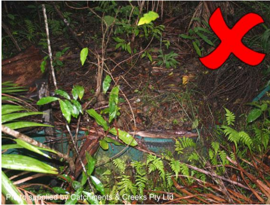
Sediment fence located in bushland
