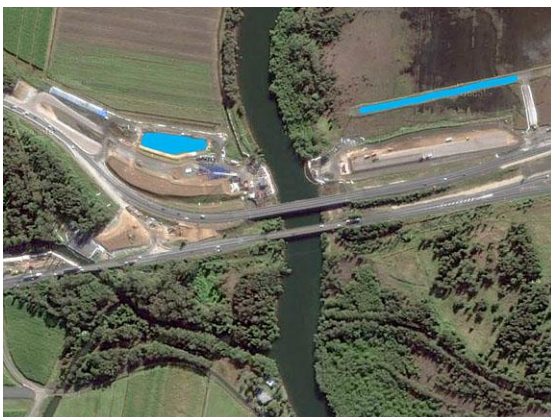
Complex road construction
