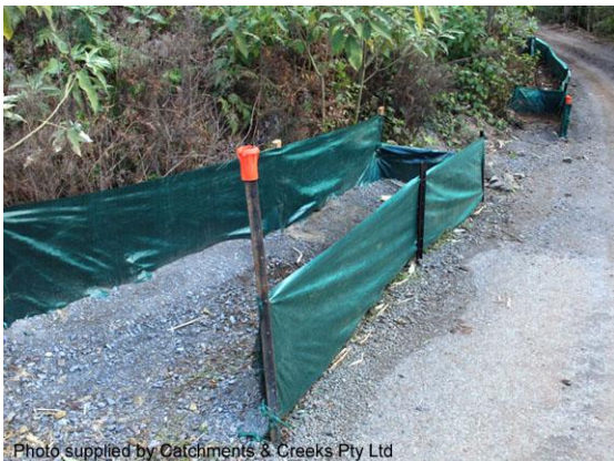
U-shaped sediment trap
