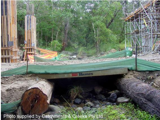
Temporary access construction bridge
