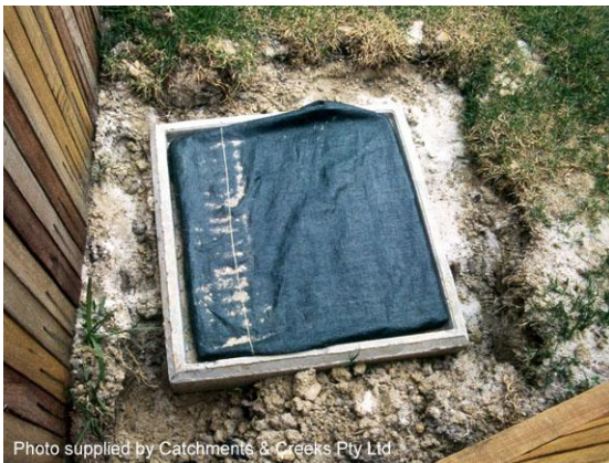
Fabric wrap inlet protection
