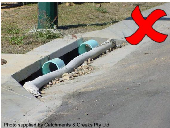
Inappropriate on-grade inlet control
