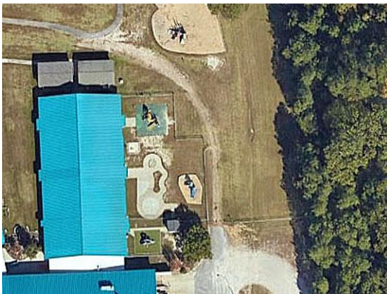
Replacement of sealed road with dirt road
