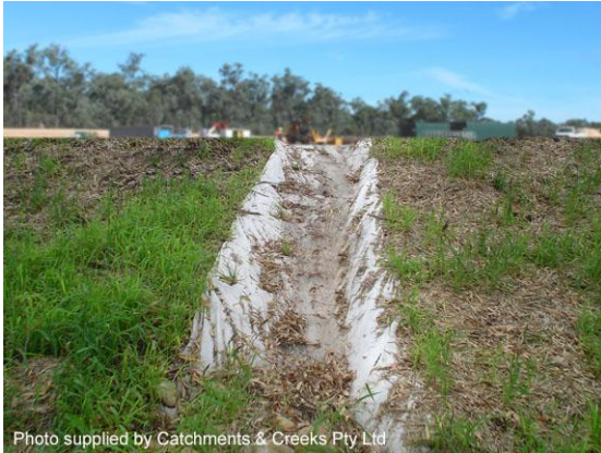
Filter cloth lined batter chute
