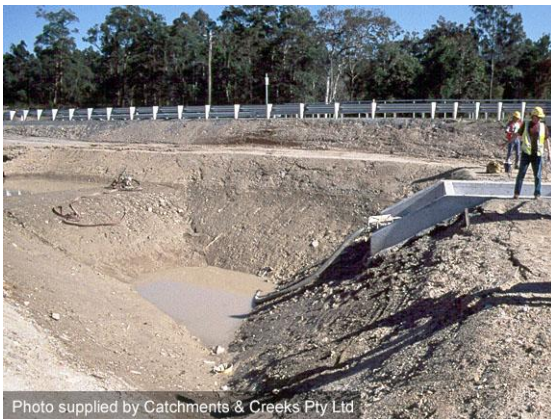
Sediment basins (Type 1 sediment trap)
