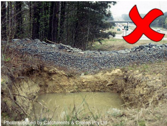
Excavated sediment trap and RFD
