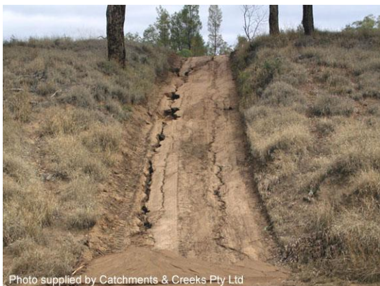
Access road located along a flow path
