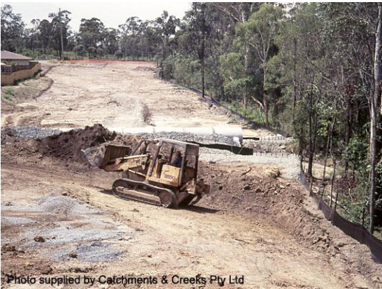
Excavating a sediment basin
