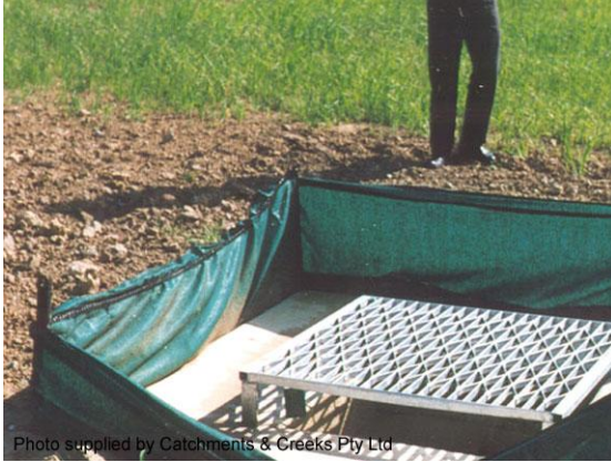
Fabric drop inlet protection
