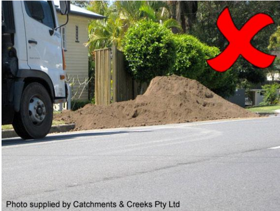
Topsoil stockpile placed on public roadway
