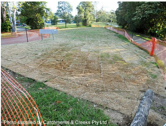
Turfing of overbank disturbance
