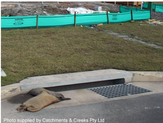
On-grade kerb inlet sediment trap
