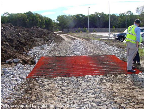
Temporary construction access road
