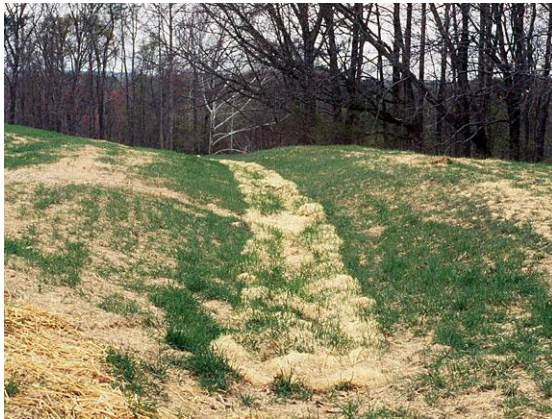
Erosion control mat (Hodge Rd, 1995)
