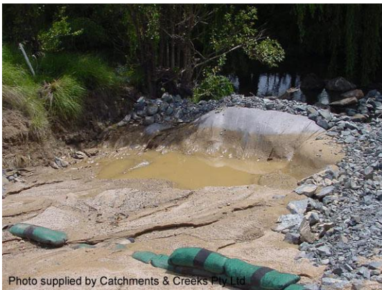
Rock filter dam (Type 2)
