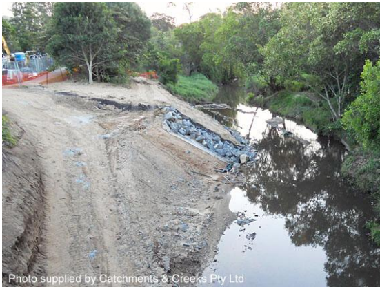
Upstream rock stabilisation
