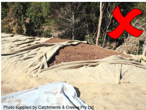
Blankets displaced by wind
