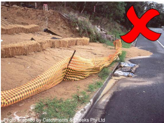
Sediment deposited off the site
