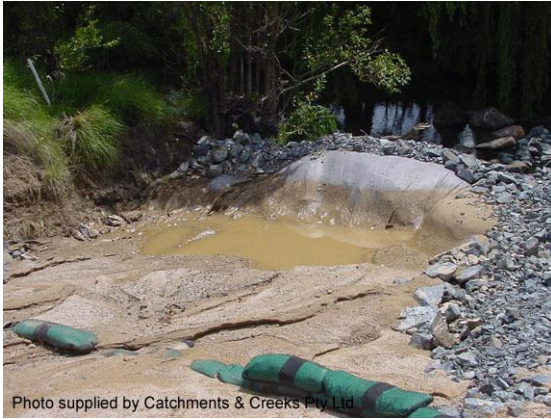
Rock filter dam (Type 2 sediment trap)
