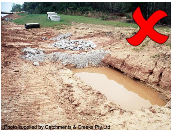
Sediment sump formed in dispersive soil
