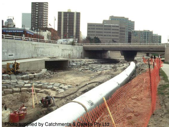
Instream works with piped-flow bypass
