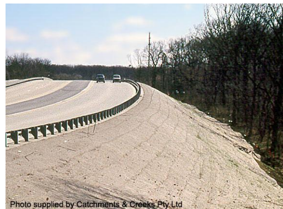
Erosion control blankets
