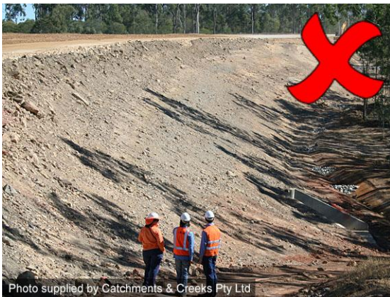
Fully exposed road batter
