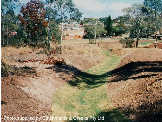
Turf lined diversion drain
