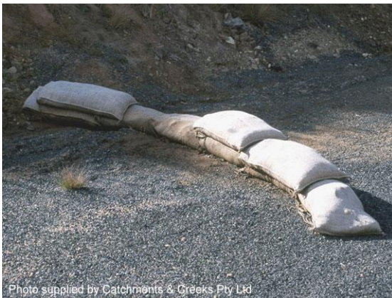
Check dam sediment trap
