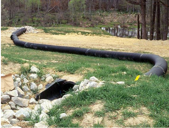
Slope drain (Hodge Road site, 1995)
