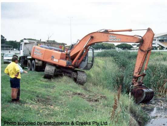
De-silting of a stormwater drain
