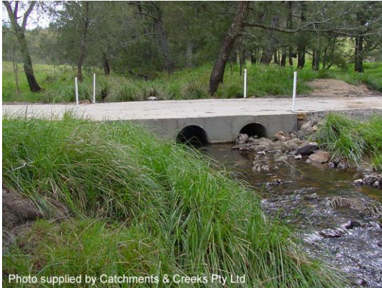
Private driveway crossing of a creek
