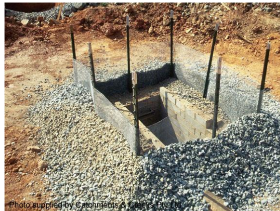
Mesh & aggregate drop inlet sediment trap
