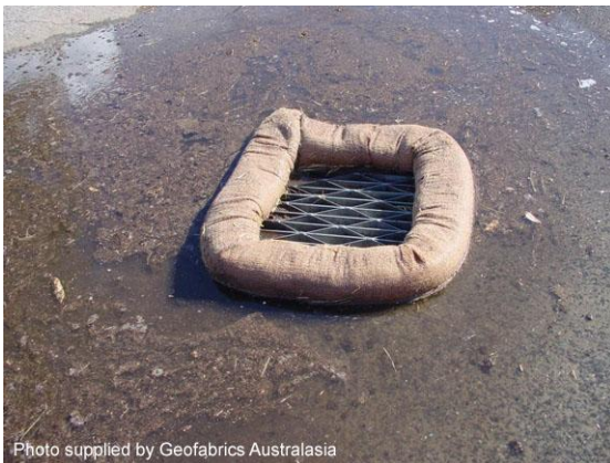
Filter sock drop inlet protection
