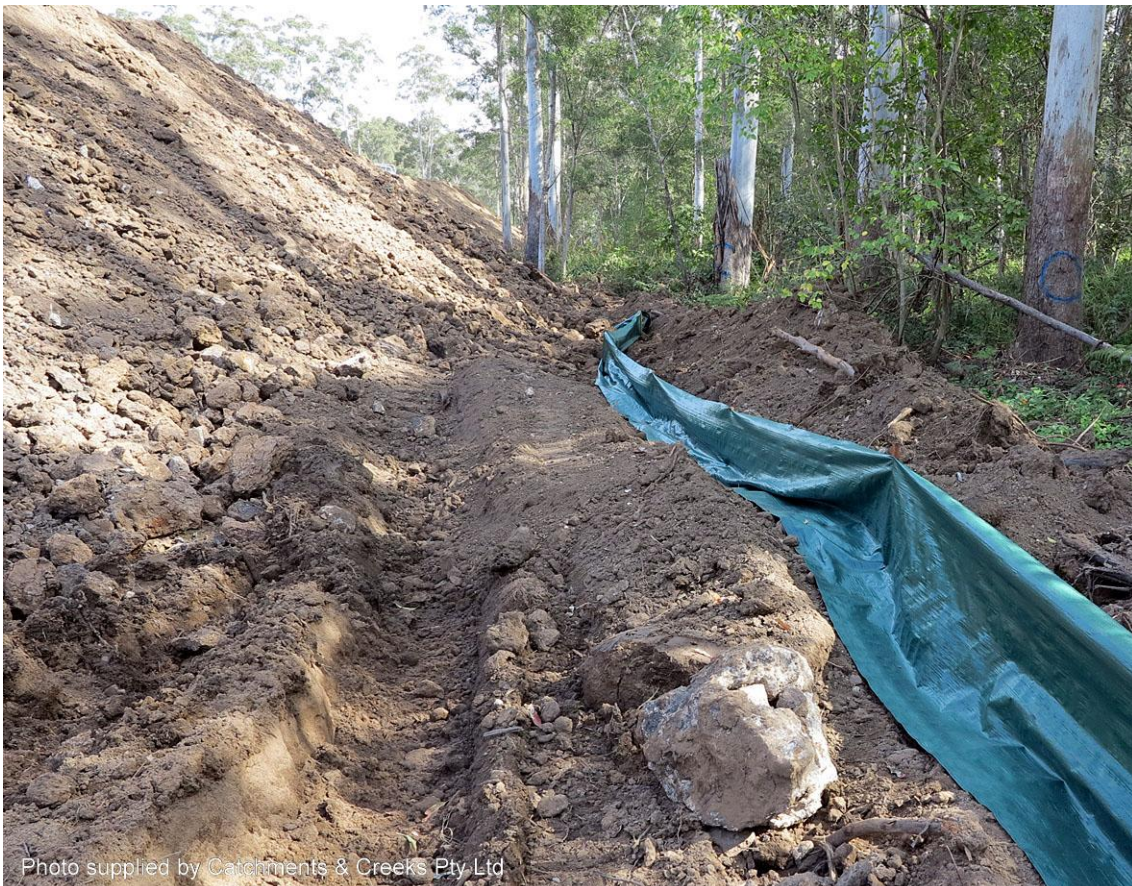
Figure 3 – The problem of filling up to the edge of a ‘protected’ riparian zone
