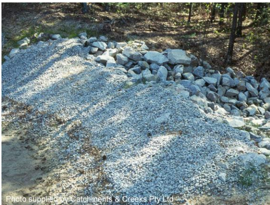
Rock filter dam with aggregate filter
