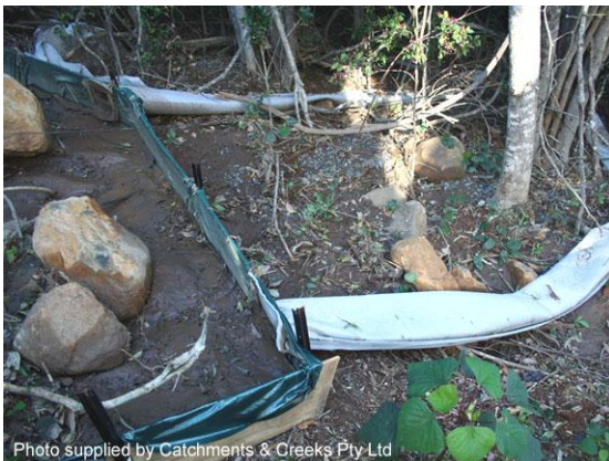
Filter tube dam sediment trap
