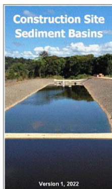
Construction Site Sediment Basins
