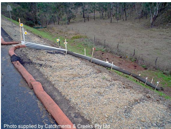
Corrugated iron batter chute
