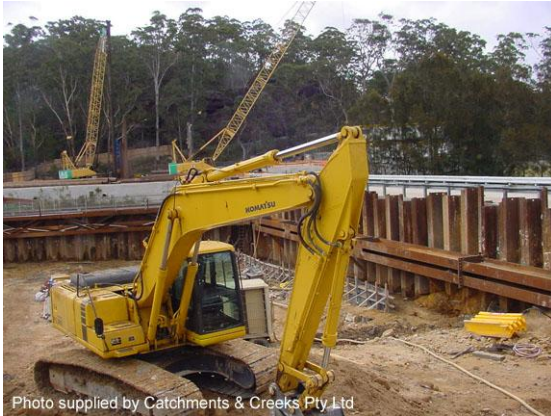
Sheet piling isolation barrier
