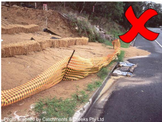
Site entry located on an overland flow path
