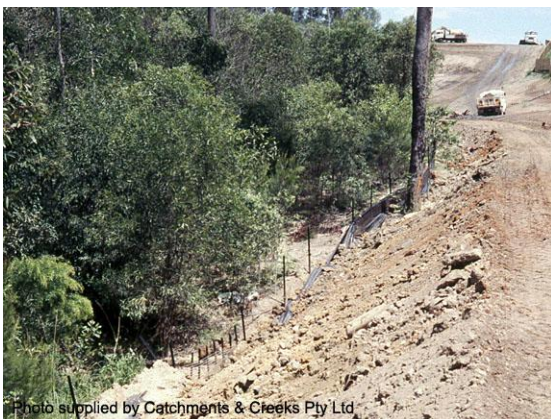
Spill-through weir outlet structure
