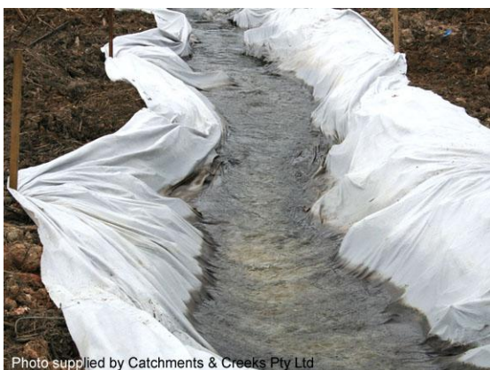
Filter cloth anchored with timber stakes
