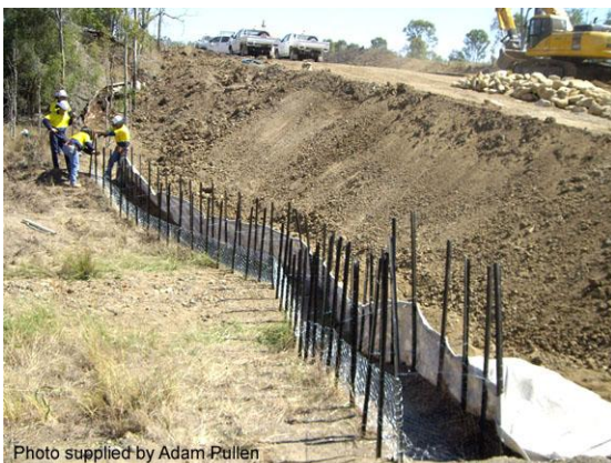
Construction of a sediment weir
