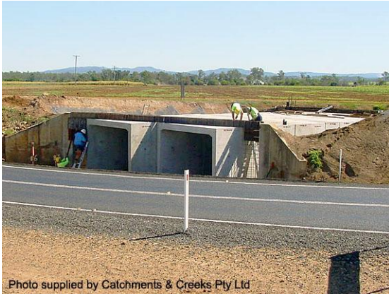
Culvert construction
