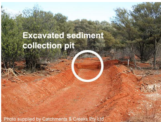
Excavated sediment trap
