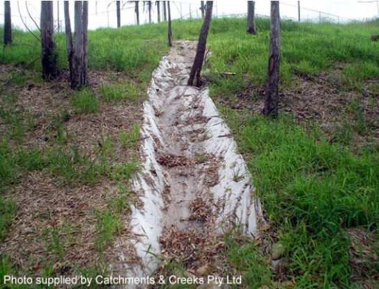
Geotextile lined drainage chute
