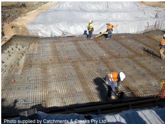
Construction of a culvert base slab (Qld)
