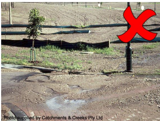
Inappropriate use of sediment fences
