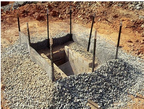
Mesh & aggregate drop inlet trap (1995)
