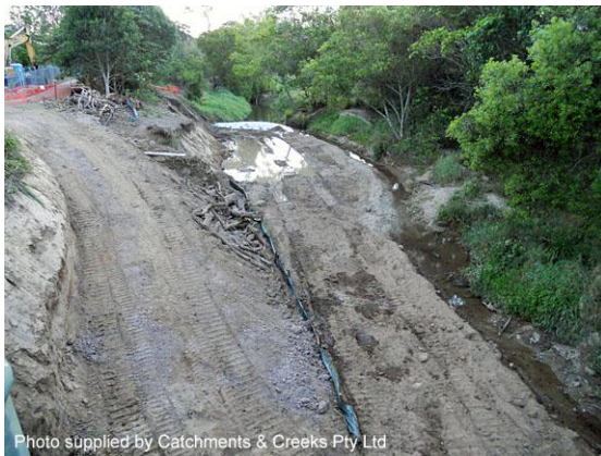
Isolation of the work area
