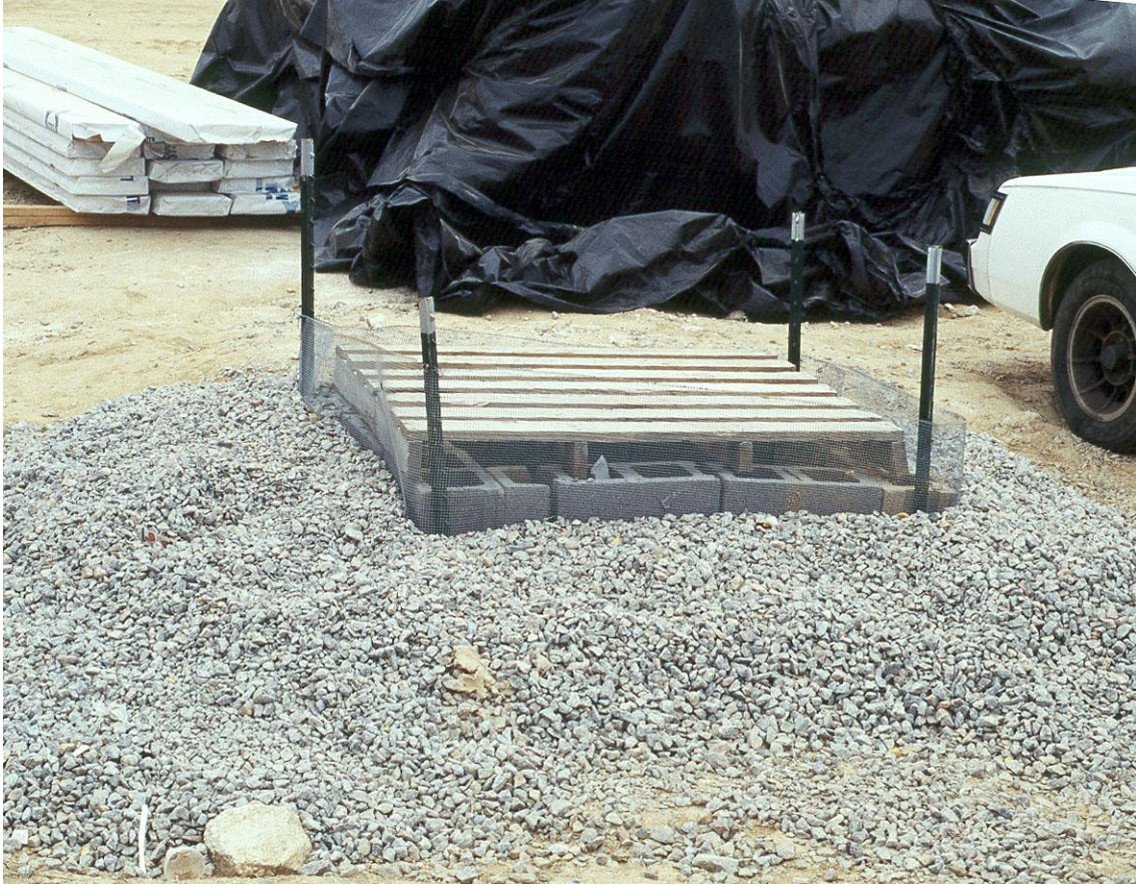
Figure 22 – Block & Aggregate Drop Inlet Protection (Hodge Road School, 1995)
