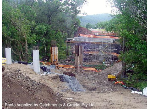
Bridge construction (Qld)
