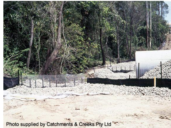
Rock filter dam outlet structure
