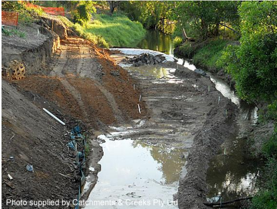
Reconstruction of the eroded bank
