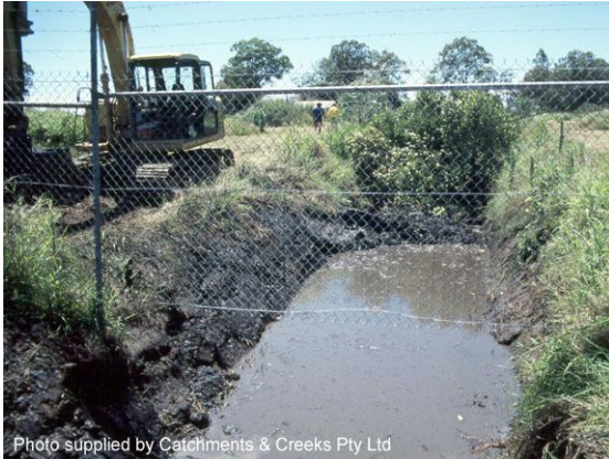
De-silting a storm drain outlet (Qld)
