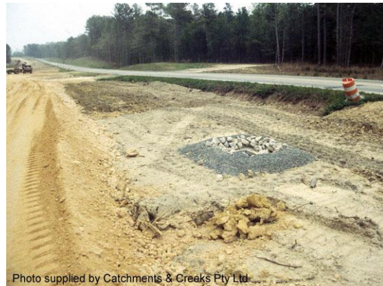
Rock & aggregate drop inlet sediment trap
