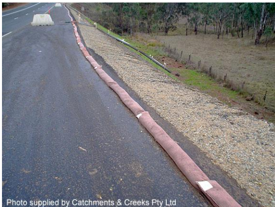
Temporary flow diversion berm
