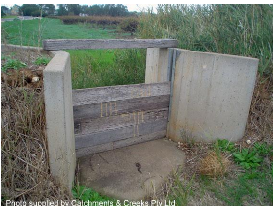
'Stop-board' outlet control system (SA)
