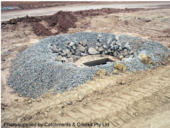
Rock & aggregate drop inlet sediment trap
