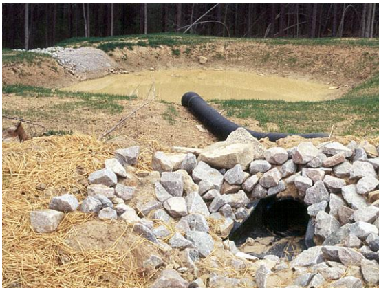
Slope drain pipe entrance (1995)
