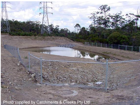
Fenced sediment basin adjacent to a creek
