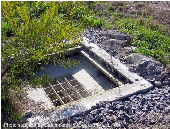
Block & aggregate drop inlet protection
