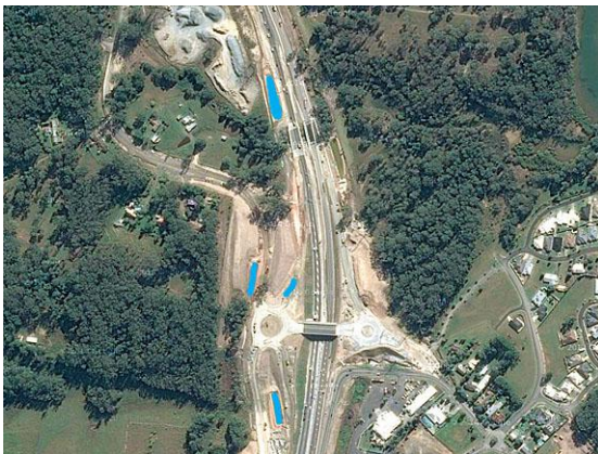
Complex construction site (NSW)
