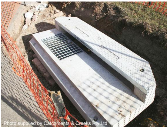
Replacement of roadside stormwater pit
