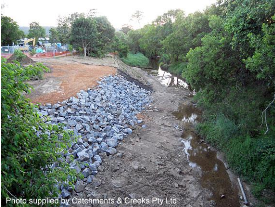
Downstream rock stabilisation
