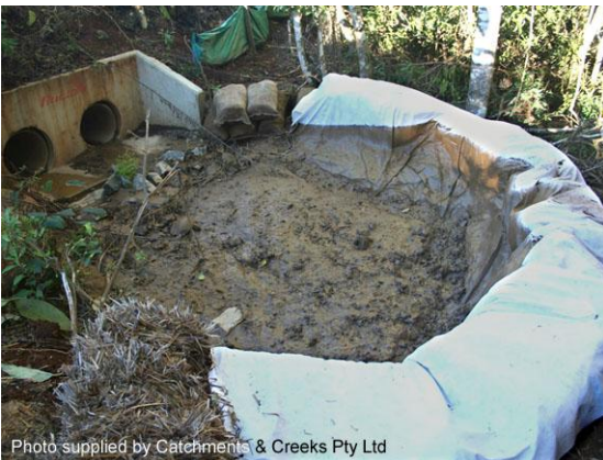
Straw bale barrier
