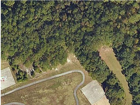
Rehabilitated sediment basin SB-4 (2022)
