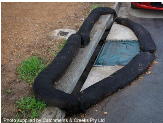
Sag inlet protection (Supplementary)
