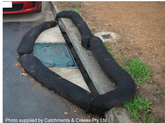
'Sag' kerb inlet sediment trap
