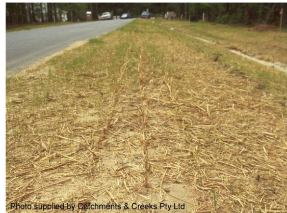
Crimped straw mulch
