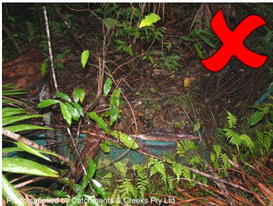
Sediment fence located in bushland
