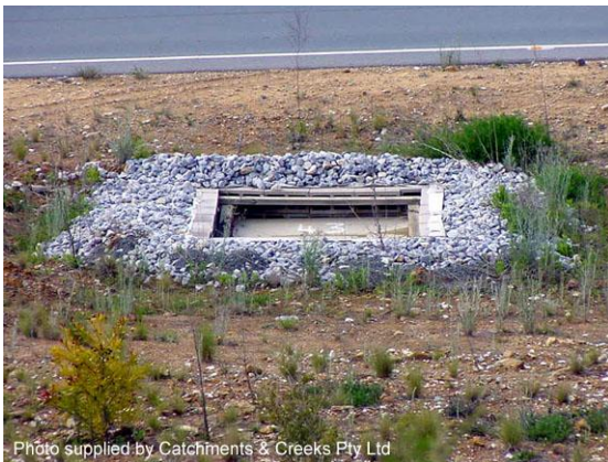
Block & aggregate drop inlet sediment trap
