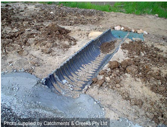
Temporary half-pipe batter chute
