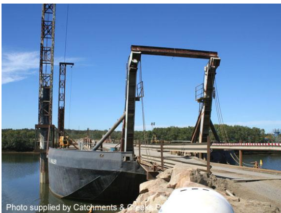
Barge crossing of a tidal inlet
