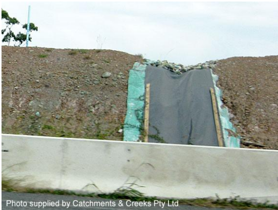
Temporary plastic sheet batter chute
