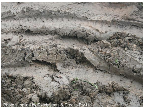
Mud generated around a site office
