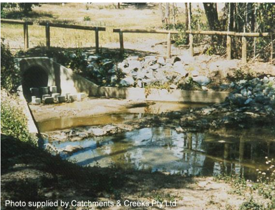
Excavated sediment trap
