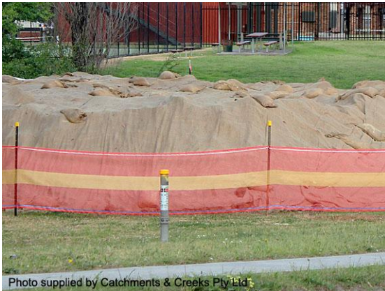
Long-term stockpile covered with jute
