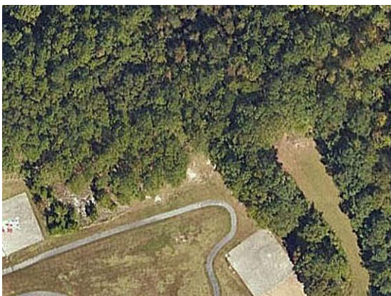
Rehabilitation of sediment basin, SB-4
