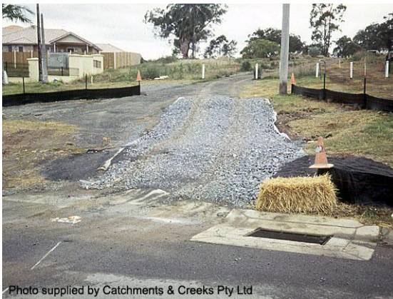
Rock pad with flow diversion berm
