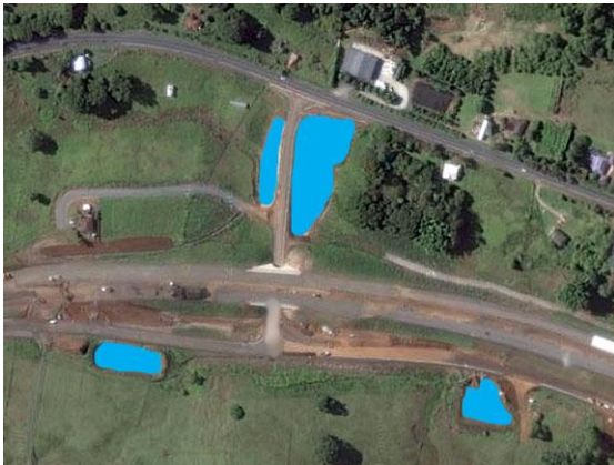
Sediment basins on road construction
