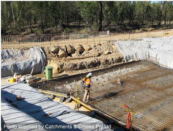
Construction of a culvert base slab
