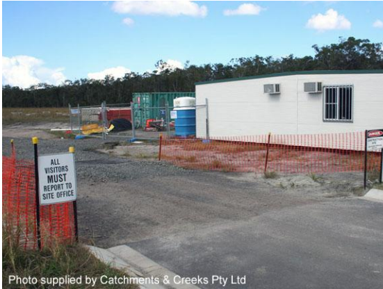
Site entry and office
