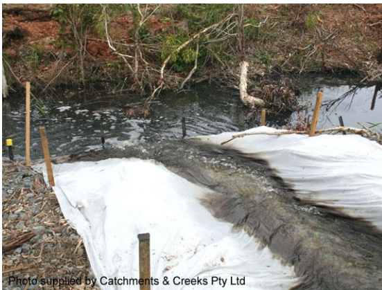
Release of clean water into a drain
