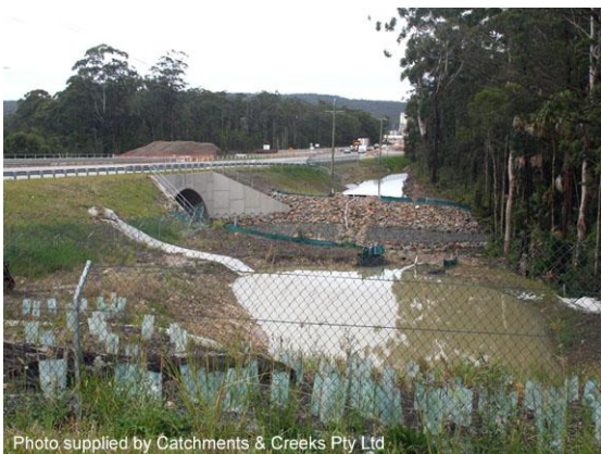
Basins retained for stormwater treatment
