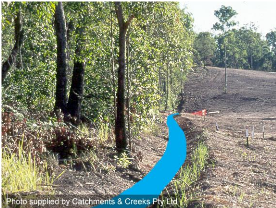
Flow diversion using a catch drain
