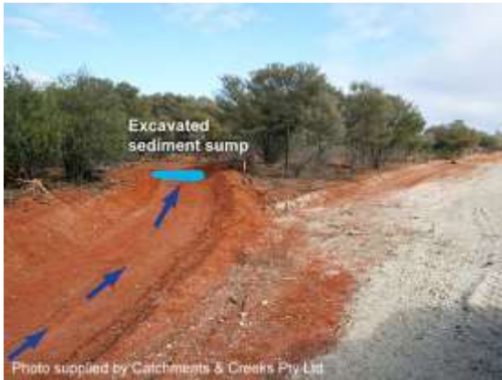
Excavated sediment trap/sump
