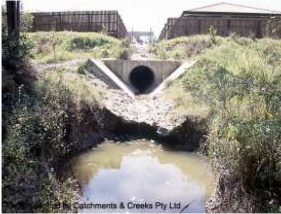
Pipe outlet pre-construction
