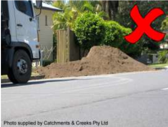
Topsoil stockpile placed on public roadway
