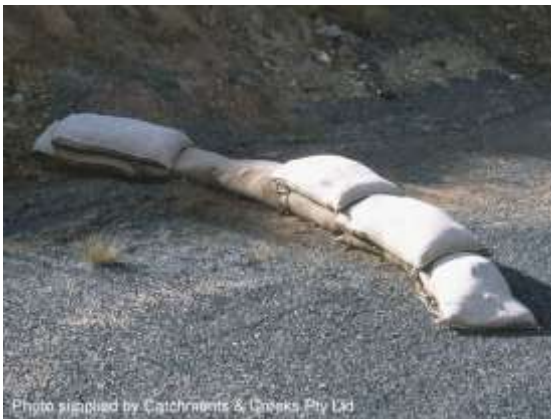
Sandbag sediment trap
