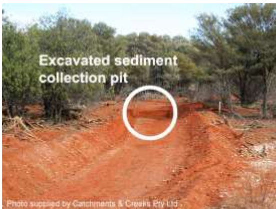
Excavated sediment trap
