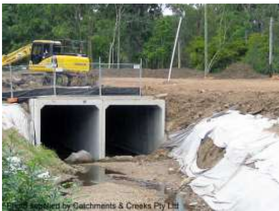
Culvert construction (Qld)
