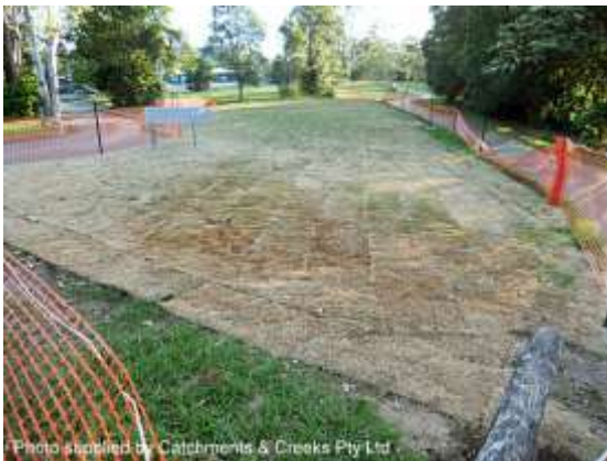
Turfing of overbank disturbance
