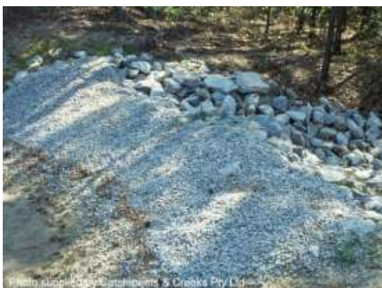
Rock filter dam with aggregate filter
