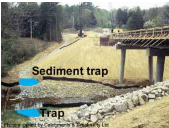
Rock filter dams (Type 2 sediment trap)
