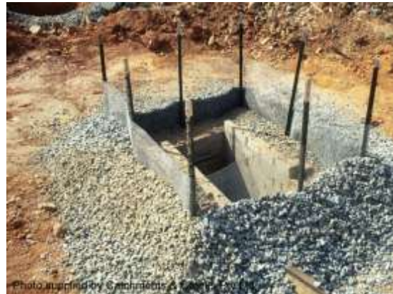
Mesh & aggregate drop inlet sediment trap
