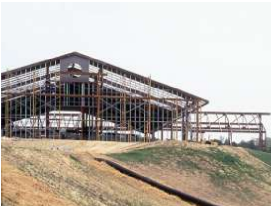
Framing of school building (1995)
