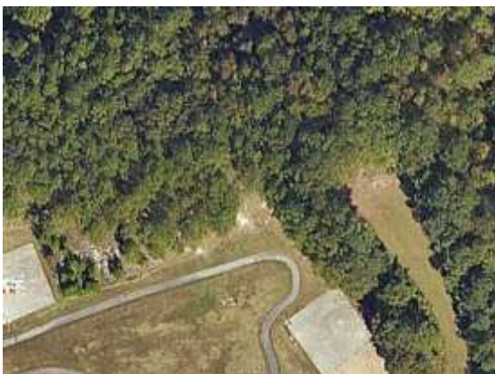
Rehabilitation of sediment basin, SB-4
