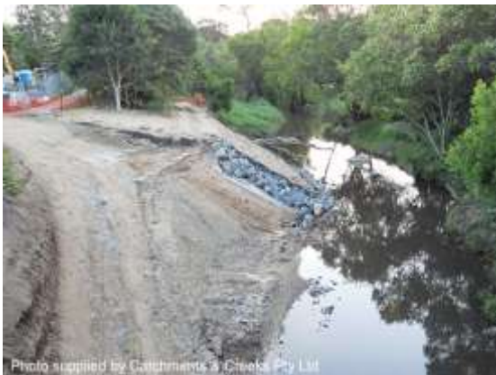
Upstream rock stabilisation
