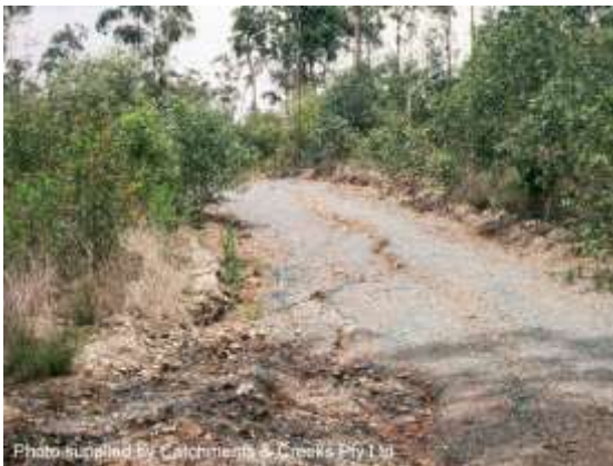
Temporary access road
