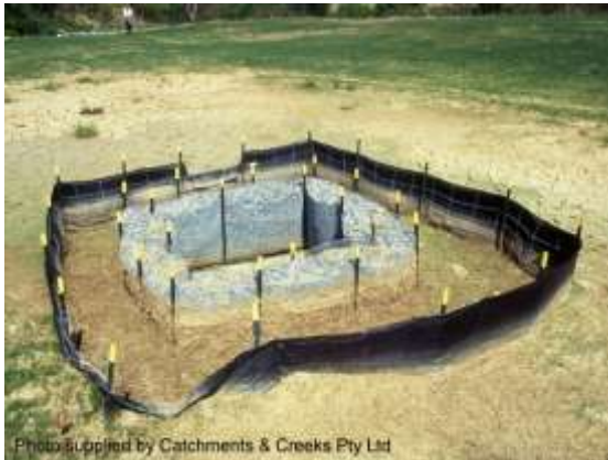
Sediment weir (field inlet protection)
