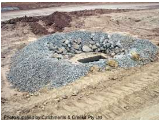
Rock & aggregate drop inlet protection
