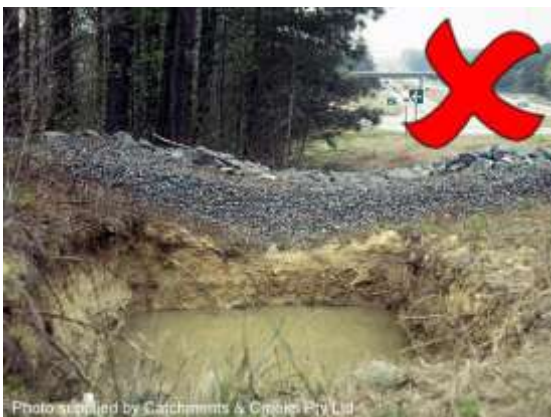
Excavated sediment trap and RFD
