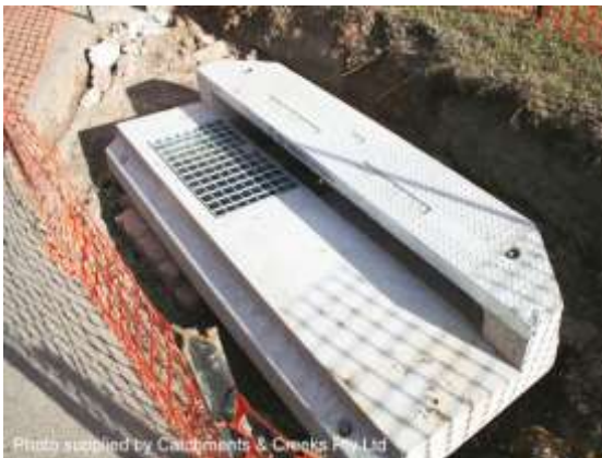
Replacement of roadside stormwater pit
