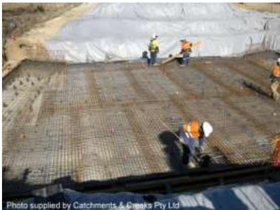
Construction of a culvert base slab (Qld)
