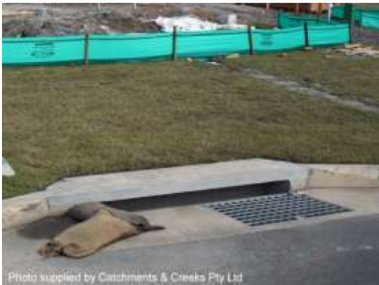
'On-grade' kerb inlet sediment trap
