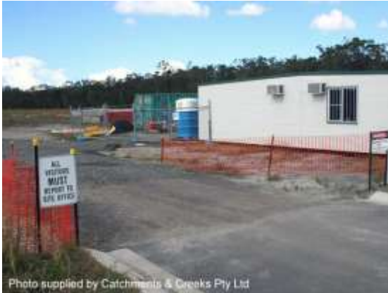
Site entry and office
