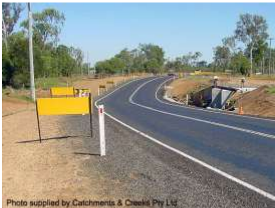
Temporary bypass road
