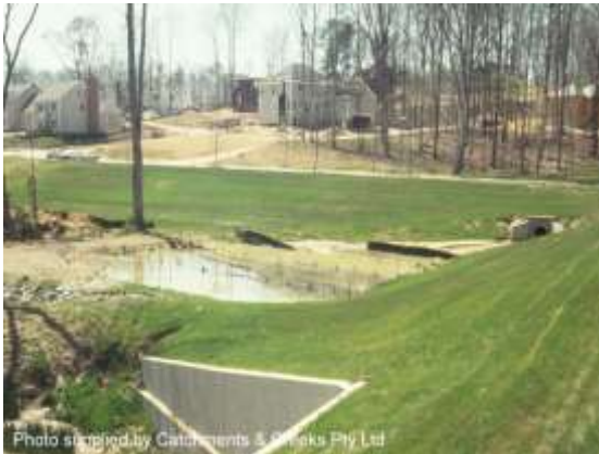
Coarse sediment trap
