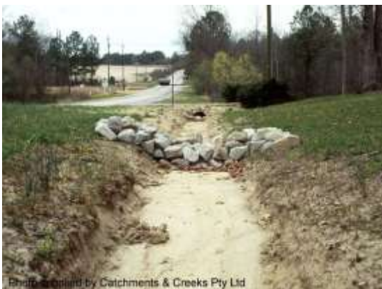
Rock check dam
