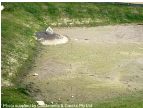
Type C sediment basin with grassed banks
