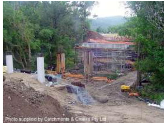
Bridge construction (Qld)
