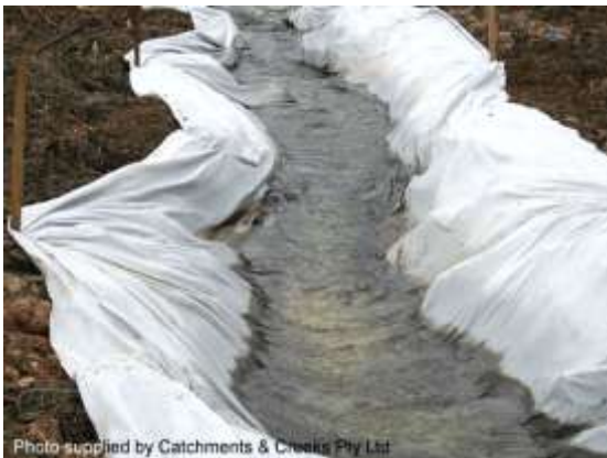
Filter cloth anchored with timber stakes
