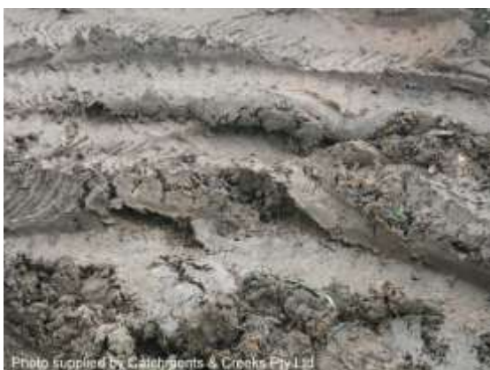
Mud generated around a site office
