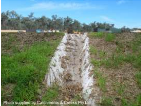
Filter cloth lined batter chute
