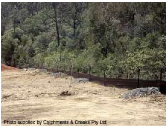
Check dams adjacent a sediment fence
