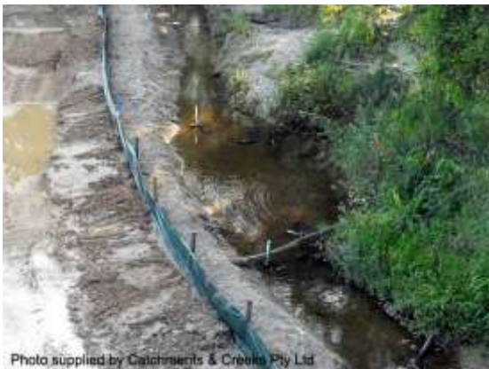
Sediment fence isolation barrier
