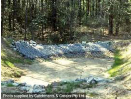
Rock filter dam with aggregate filter
