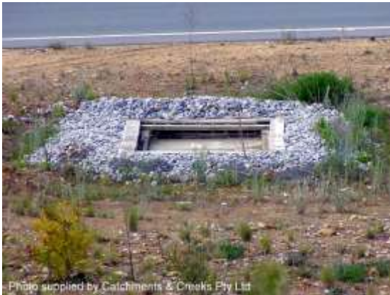
Block & aggregate drop inlet sediment trap
