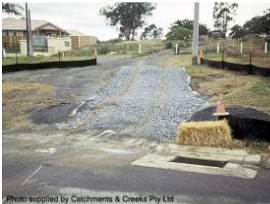
Rock pad with flow diversion berm
