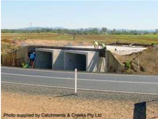
Culvert construction
