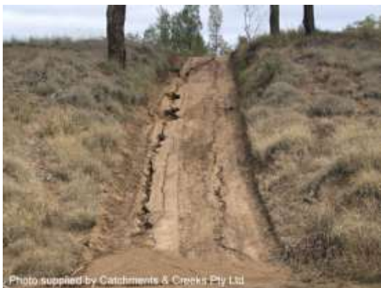
Access road located along a flow path
