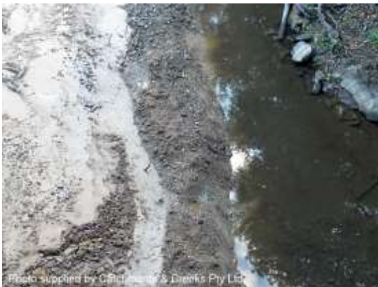
Flow diversion berm
