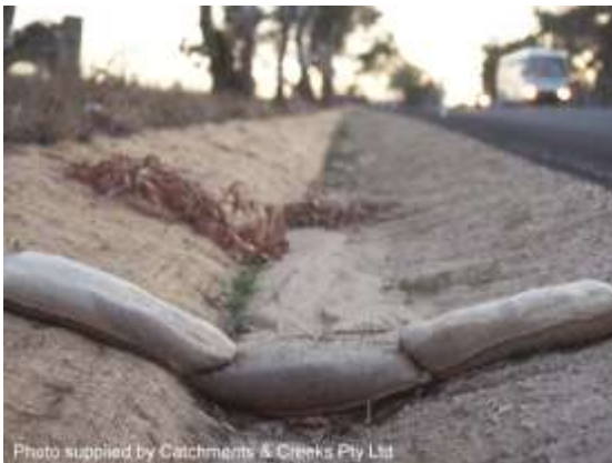
Sandbag check dam
