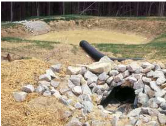
Slope drain pipe entrance (1995)
