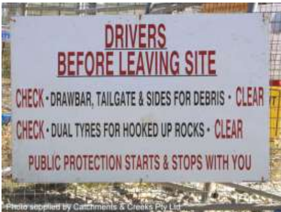
Control of rocks carried from rock pads
