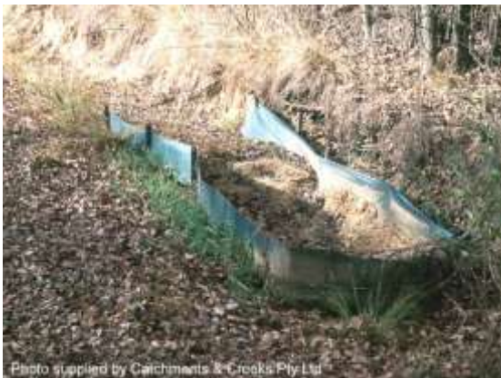
U-shaped sediment trap in steep drain
