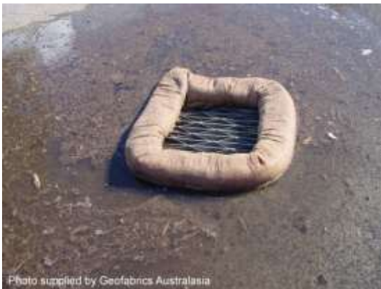
Filter sock drop inlet protection
