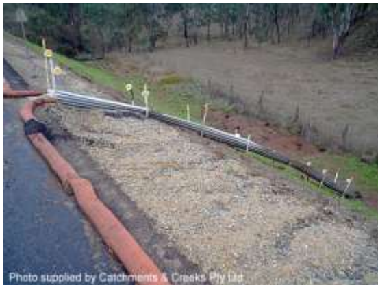
Corrugated iron batter chute
