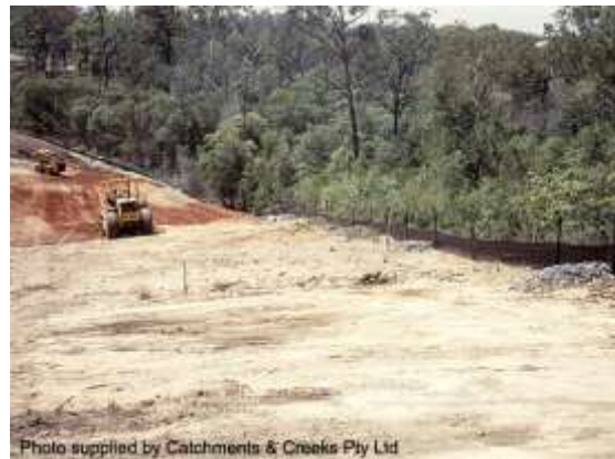
Sediment fence with rock check dams
