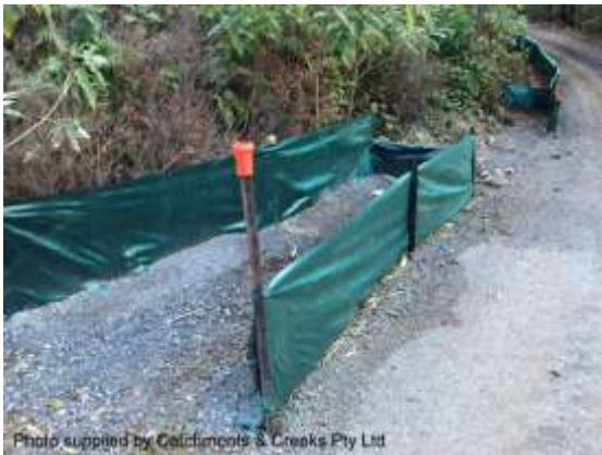
U-shaped sediment trap on mild slope
