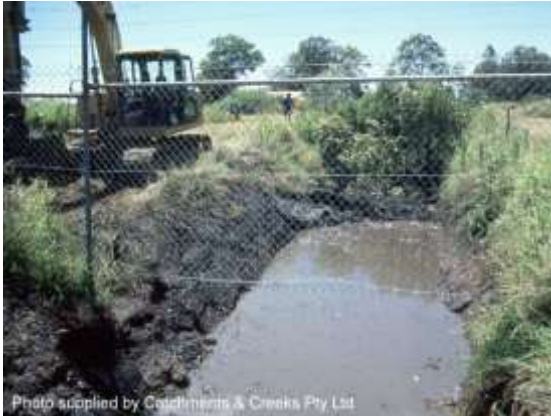
De-silting a storm drain outlet (Qld)
