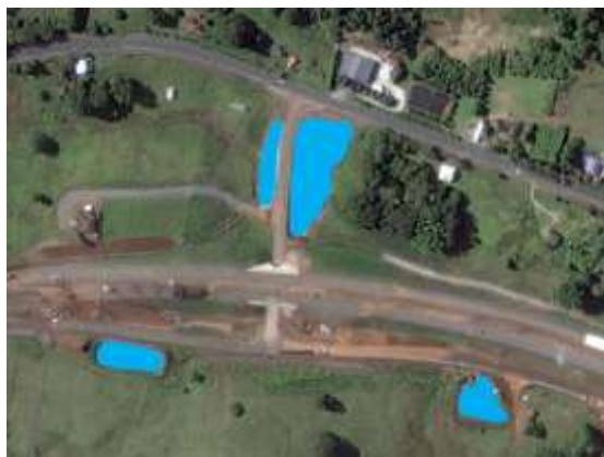
Sediment basins on road construction
