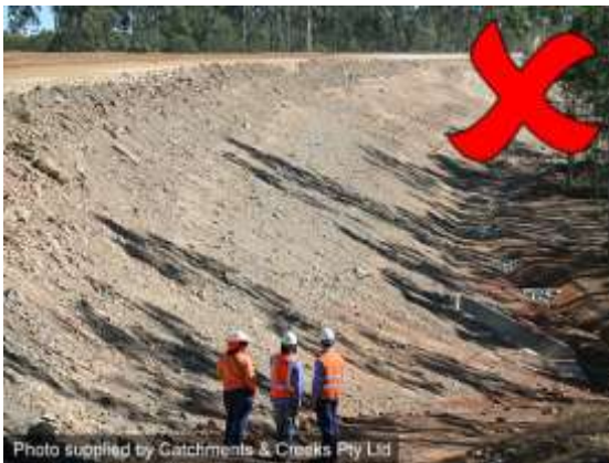
Fully exposed road batter
