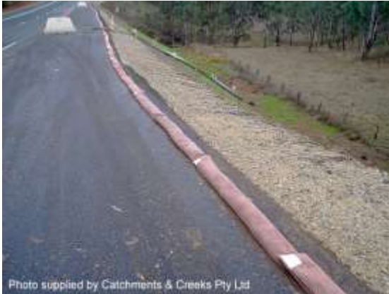
Temporary flow diversion berm
