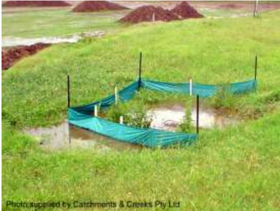
Sediment fence (Type 3 sediment trap)
