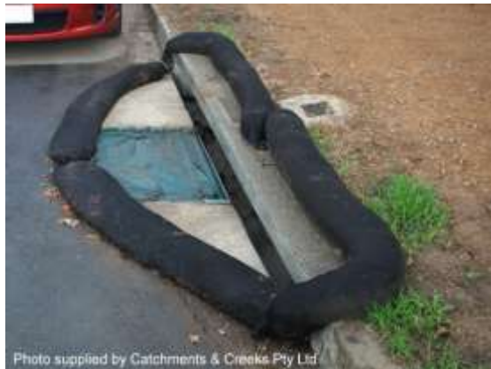
'Sag' kerb inlet sediment trap
