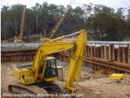
Sheet piling isolation barrier
