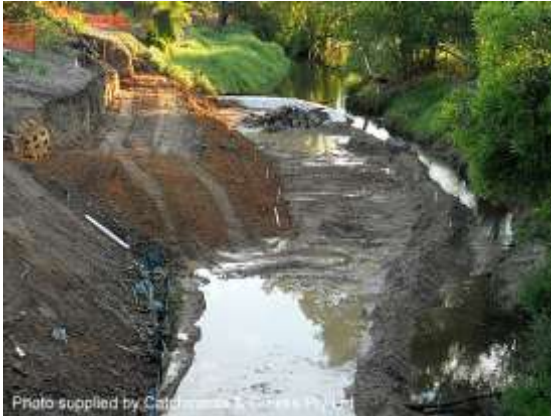
Reconstruction of the eroded bank
