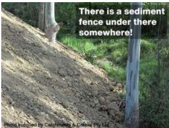
Buried trees and sediment fence
