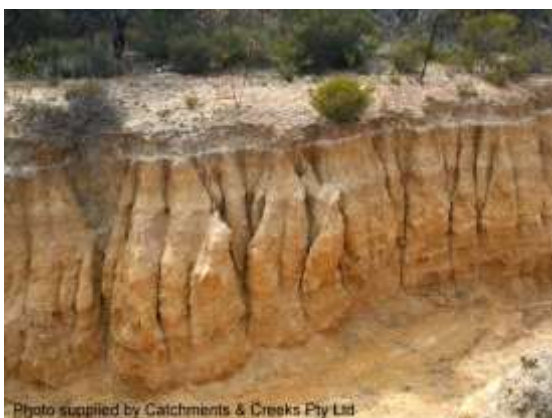
'Fluting' erosion within a dispersive soil
