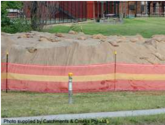
Long-term stockpile covered with jute
