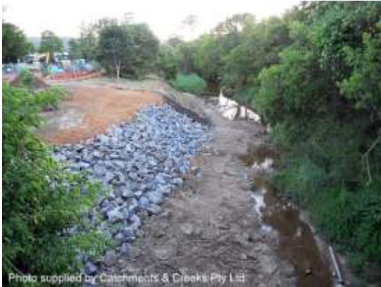
Downstream rock stabilisation
