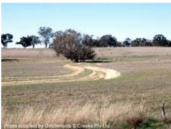
Large catch drain
