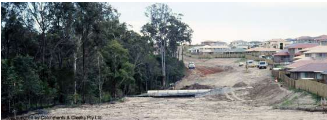
Road construction corridor viewed from the eastern end of the project
