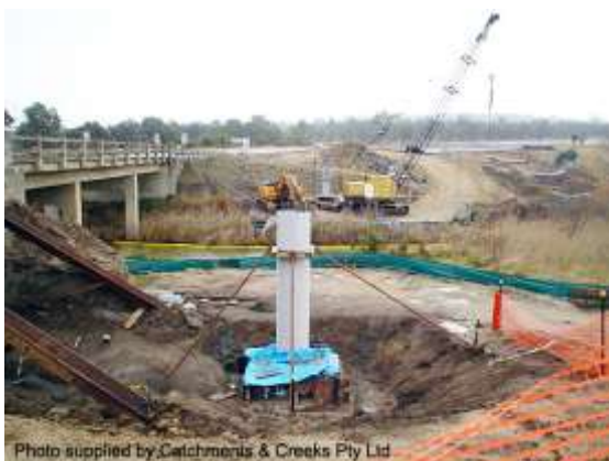
Bridge construction (NSW)
