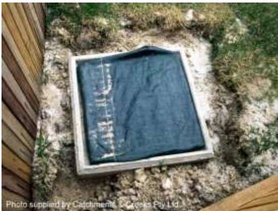
Fabric wrap inlet protection
