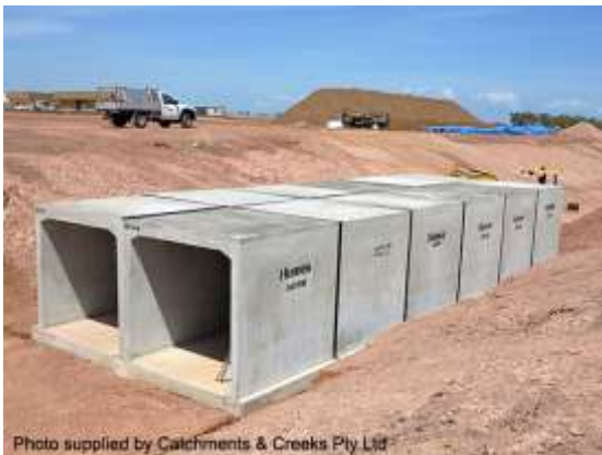
Culvert construction in a dry channel
