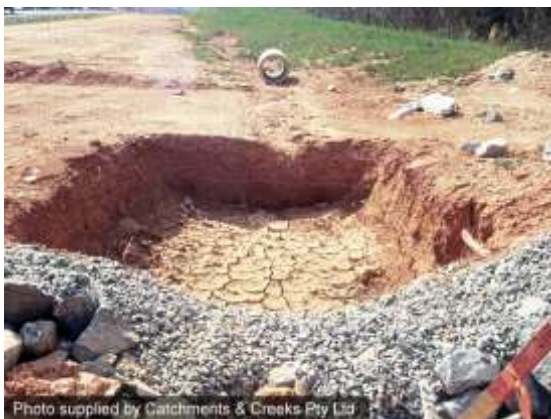
Excavated sediment sump
