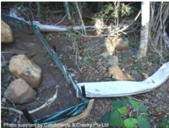
Filter tube dam sediment trap
