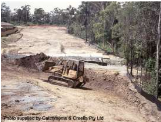
Excavating a sediment basin
