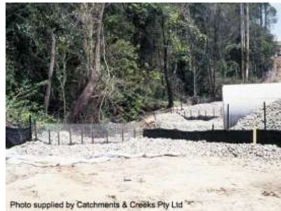
Rock filter dam outlet structure
