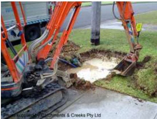
Emergency repair to broken pipeline
