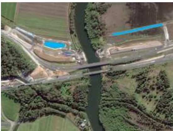
Complex road construction
