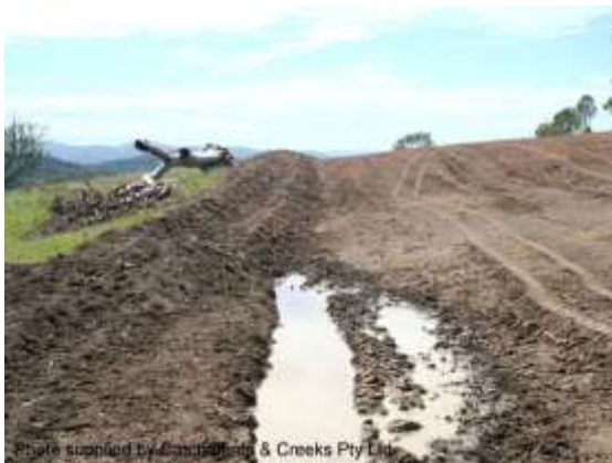
Flow diversion bank
