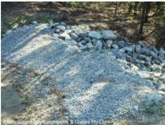
Rock filter dam with aggregate filter
