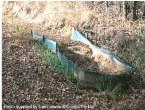
U-shaped sediment trap on steep slope
