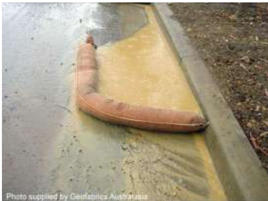
Sand-filled filter sock
