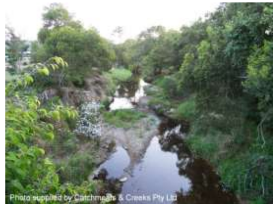
Erosion visible on the left bank, 2012
