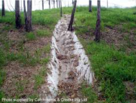
Geotextile lined drainage chute
