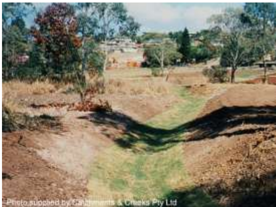
Turf lined diversion drain
