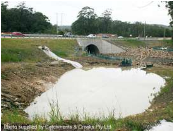
Sediment basins (Type 1 sediment trap)
