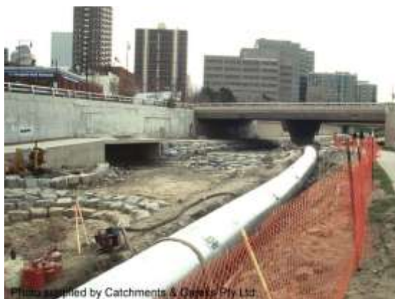
Instream works with piped-flow bypass
