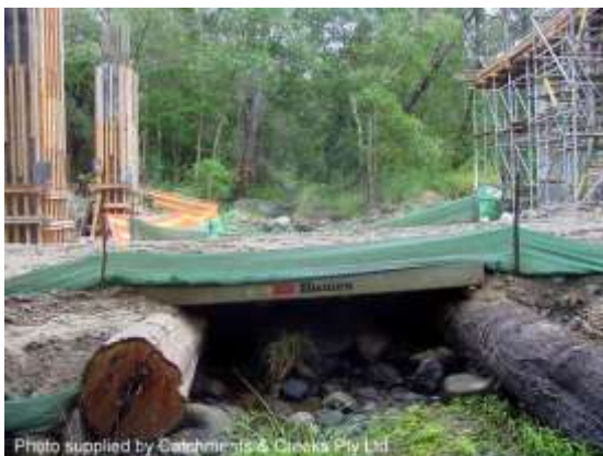
Temporary stream crossing
