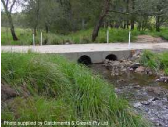
Private driveway crossing of a creek
