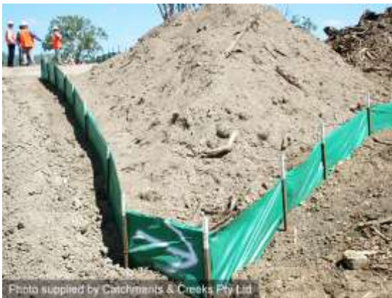
Sediment fence (Type 3)
