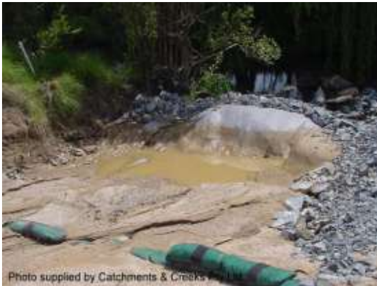
Rock filter dam (Type 2 sediment trap)
