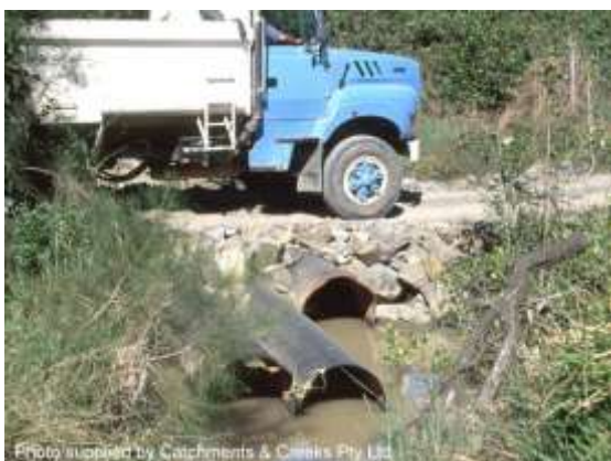
Temporary pipe culvert
