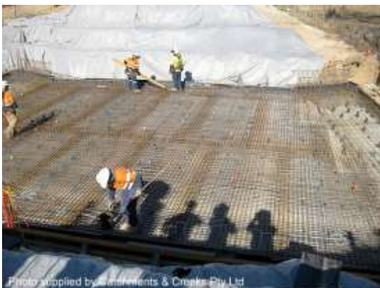
Construction of a culvert base slab
