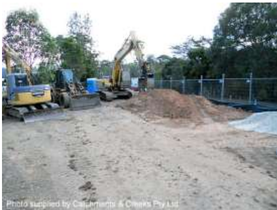
Site office and stockpile area
