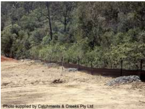
Sediment fence with rock check dams
