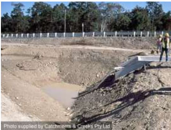
Sediment basins (Type 1 sediment trap)
