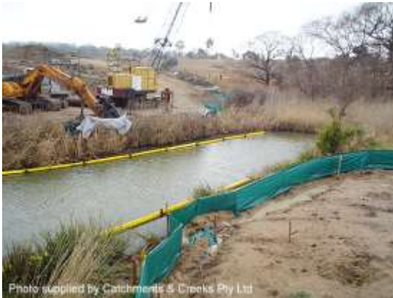
Sediment fence (Type 3 sediment trap)
