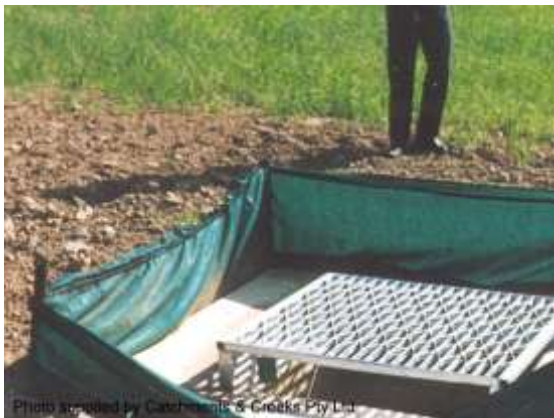
Fabric drop inlet protection
