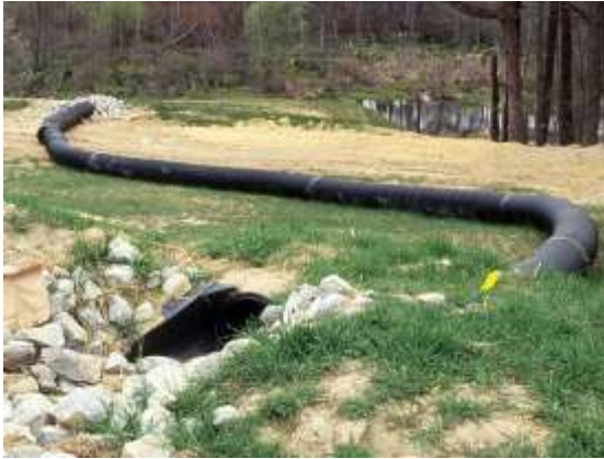
Slope drain (Hodge Road site, 1995)
