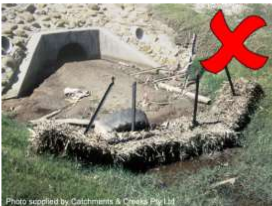
Inappropriate choice of sediment trap
