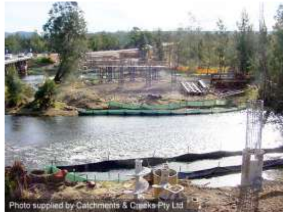
Bridge construction (NSW)
