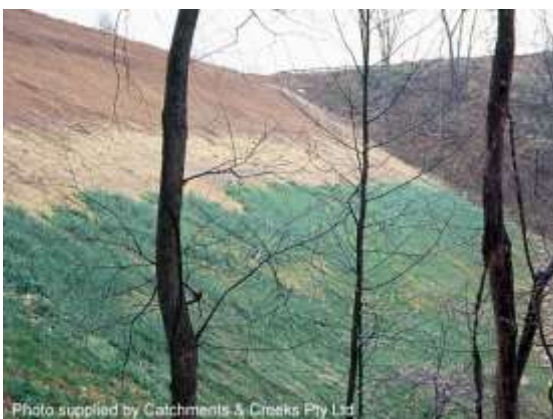
Progressive batter revegetation
