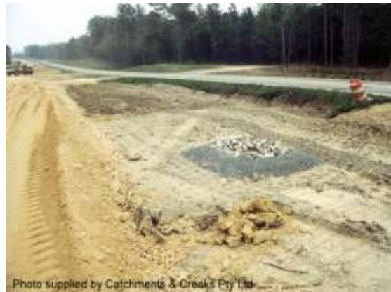
Rock & aggregate drop inlet sediment trap
