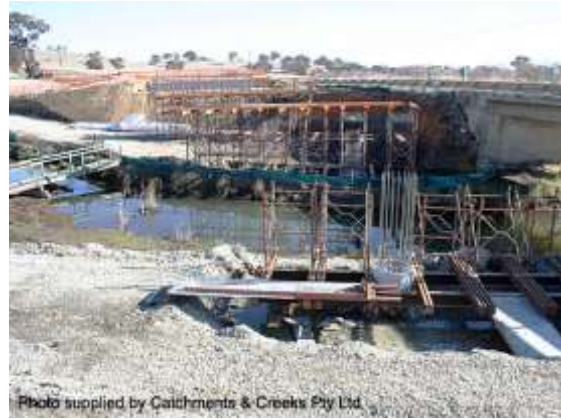
Bridge construction (NSW)
