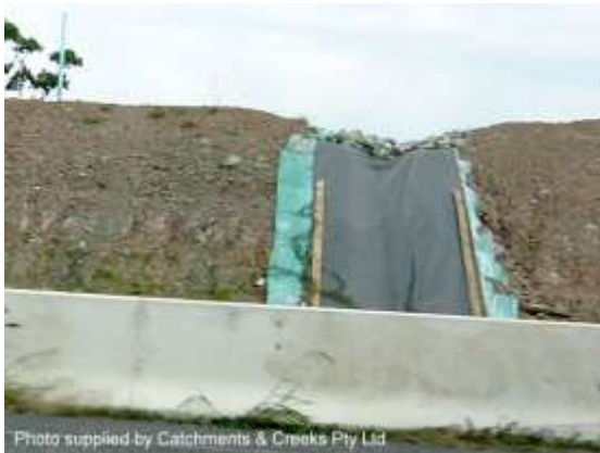
Temporary plastic sheet batter chute
