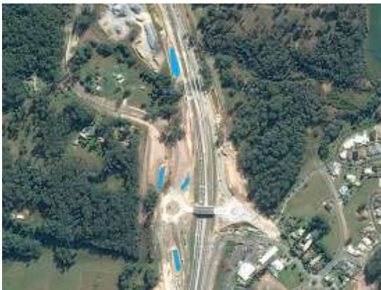
Complex construction site (NSW)
