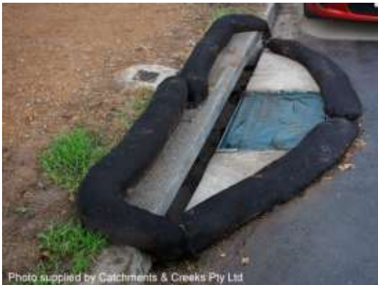
Sag inlet protection (Supplementary)
