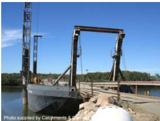
Barge crossing of a tidal inlet
