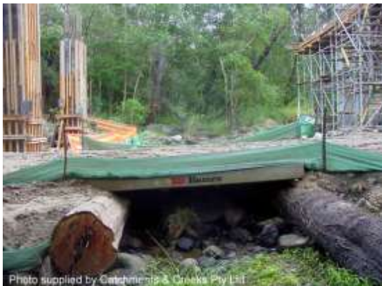
Temporary access construction bridge
