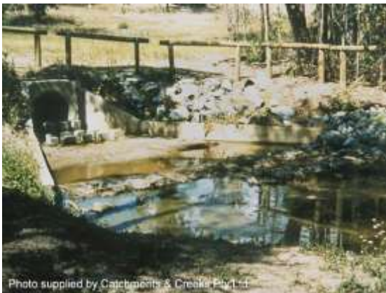
Excavated sediment trap
