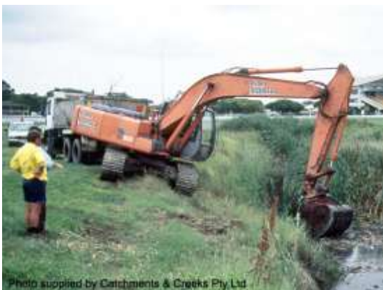
De-silting of a stormwater drain
