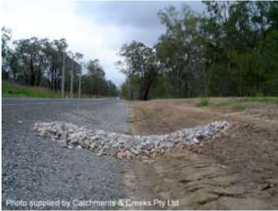
Rock check dam
