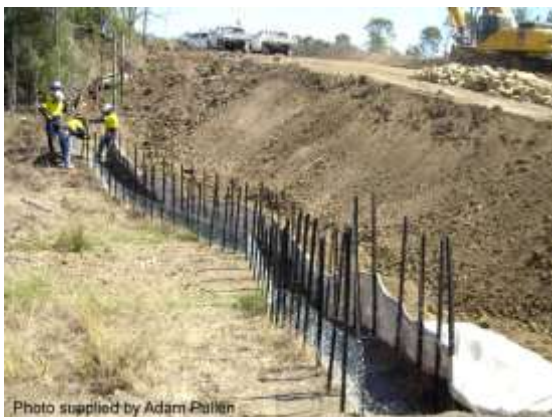
Construction of a sediment weir
