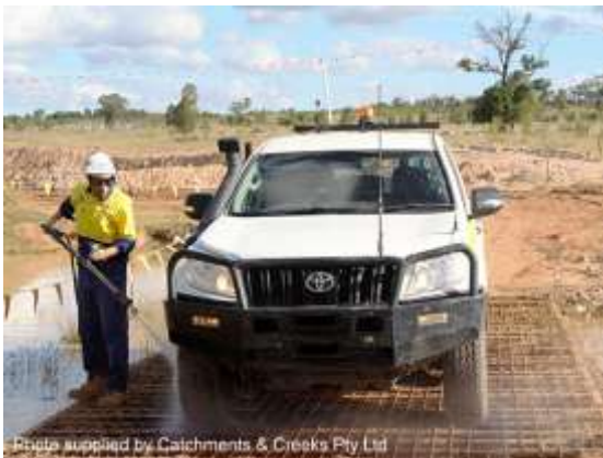
Vehicle wash-down area
