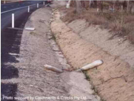
Check dam sediment trap
