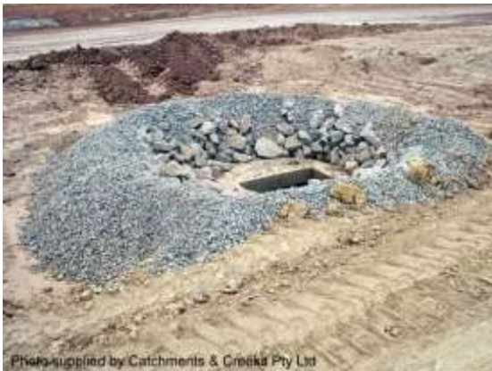
Rock & aggregate drop inlet sediment trap
