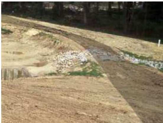
Access road crosses between SB-1 & SB-2
