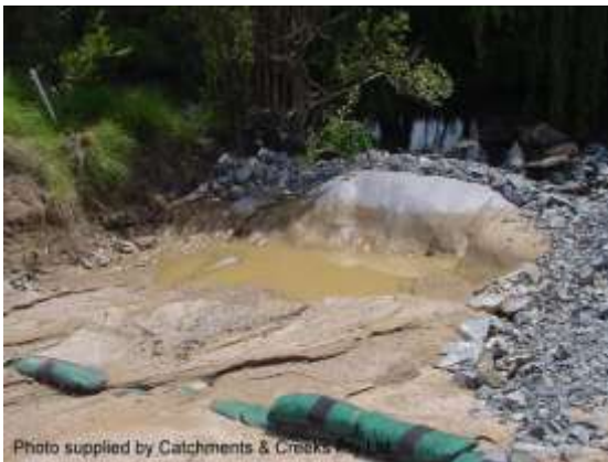
Rock filter dam (Type 2)
