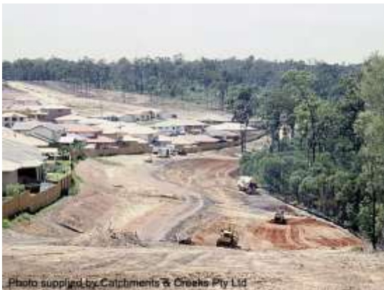
Topsoil cleared from road reserve
