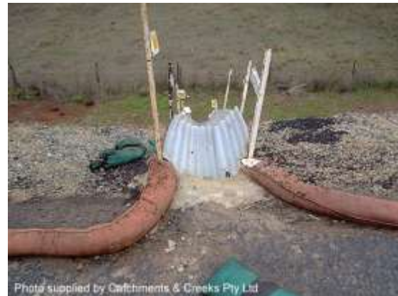
Concrete water seal at chute inlet
