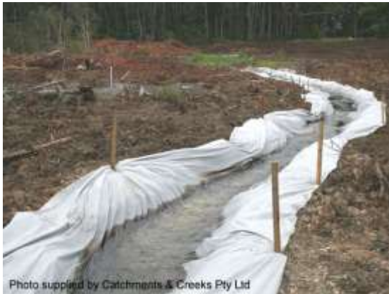
Diversion of clean water through a site
