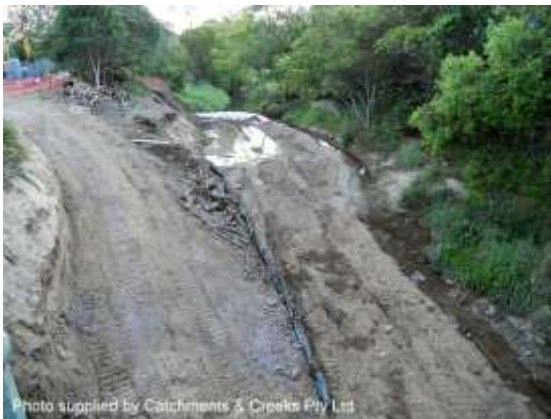
Isolation of the work area
