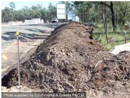
Mulch berm sediment barrier
