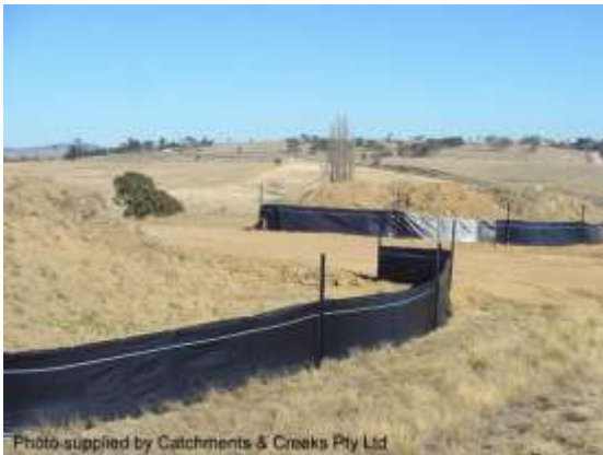
Sediment control down-slope of stockpile
