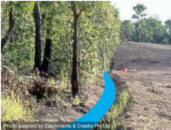
Flow diversion using a catch drain
