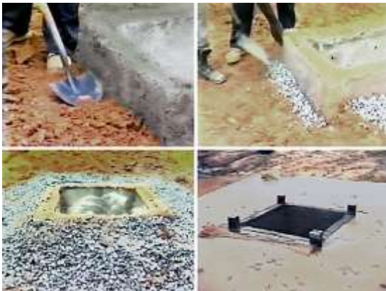
Excavated drop inlet protection
