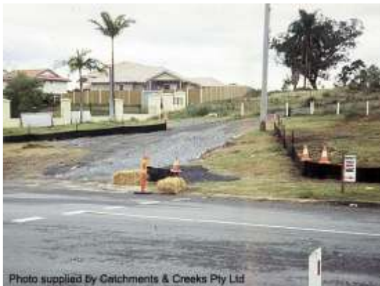
Heavy vehicle site entry point
