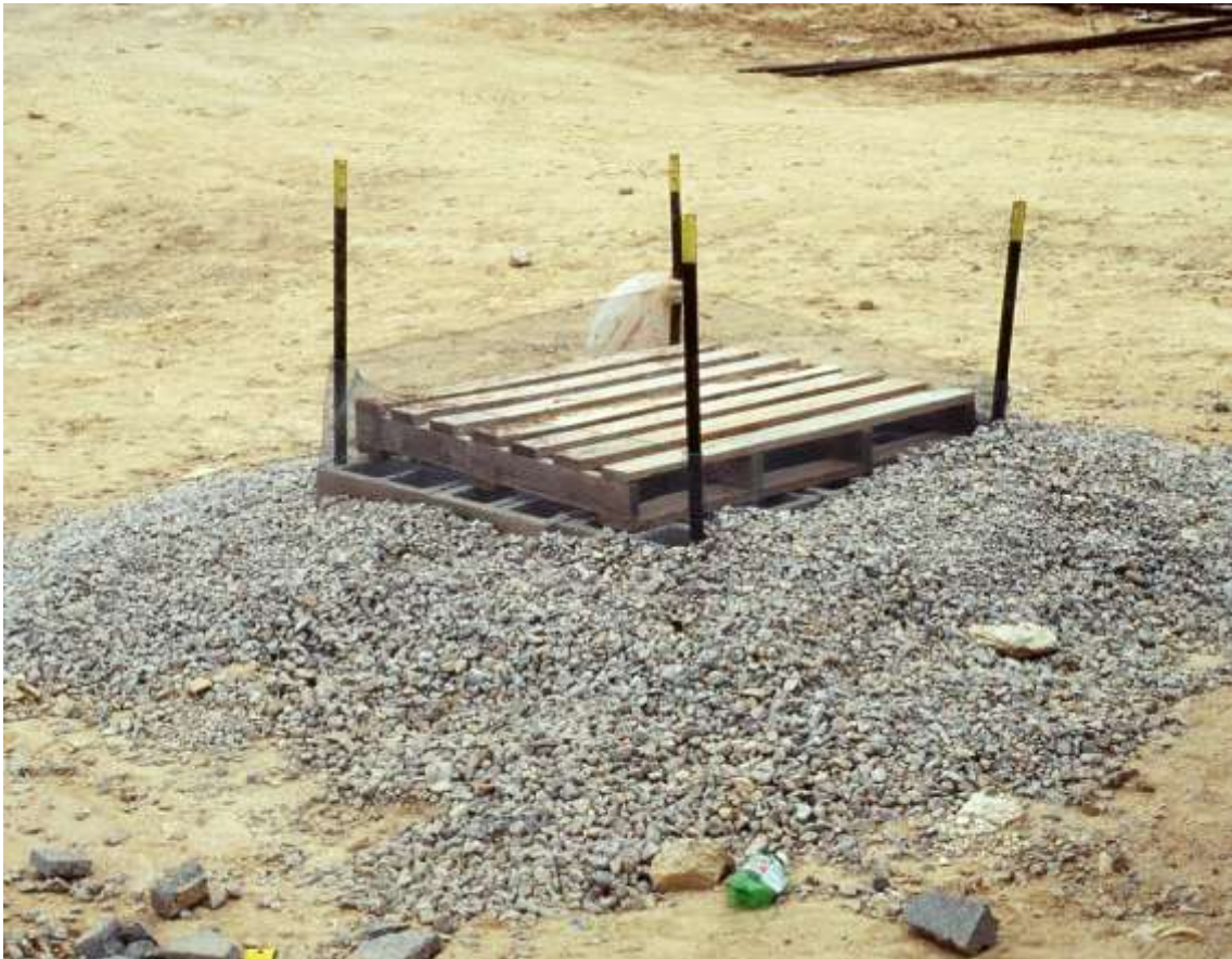
Figure 23 – Block & Aggregate Drop Inlet Protection (Hodge Road School, 1995)
