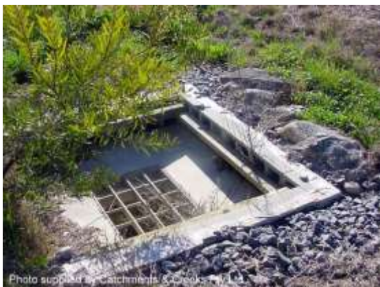
Block & aggregate drop inlet protection
