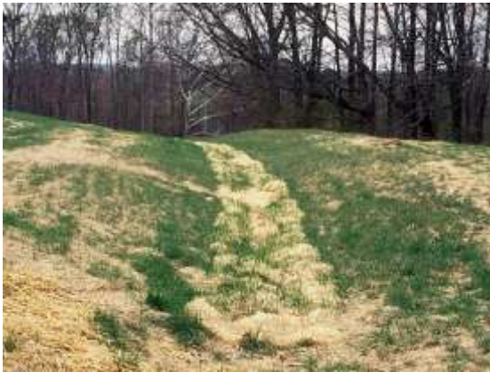
Erosion control mat (Hodge Rd, 1995)
