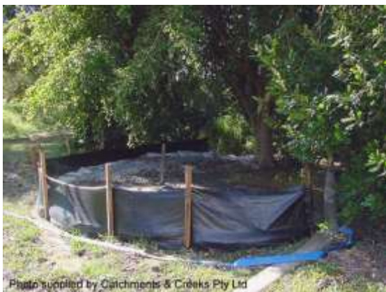
De-watering filter pond (Qld)
