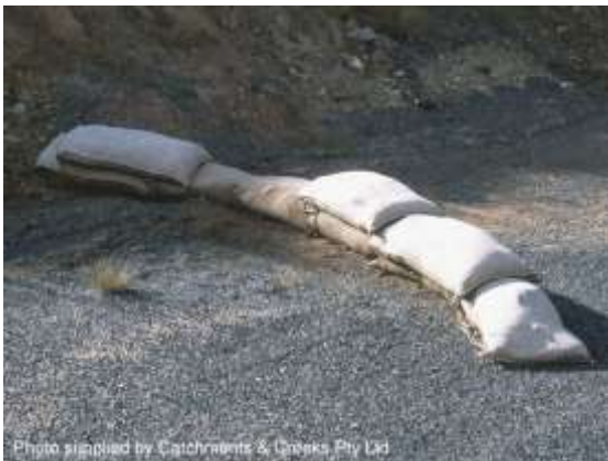
Check dam sediment trap
