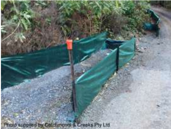
U-shaped sediment trap
