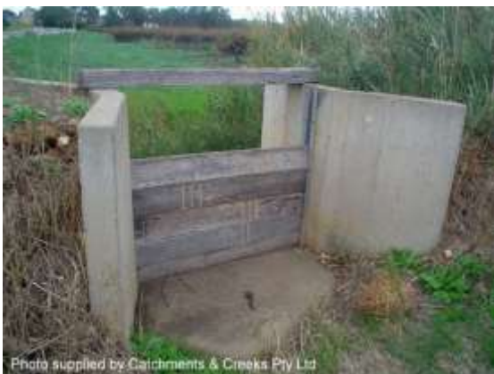
'Stop-board' outlet control system (SA)
