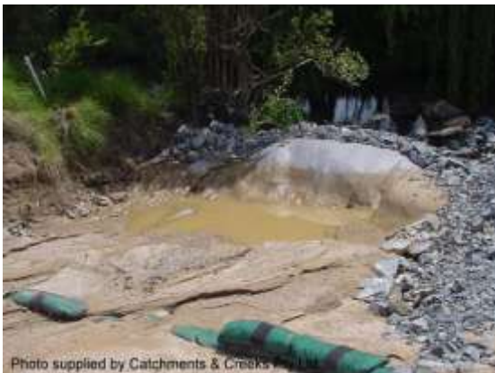
Rock filter dam with geotextile filter
