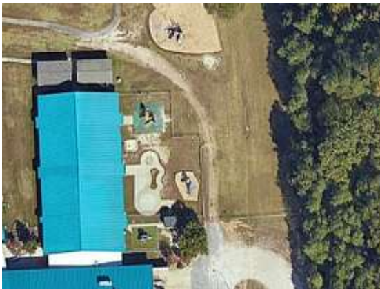
Replacement of sealed road with dirt road
