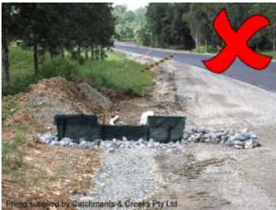
Inappropriate installation
