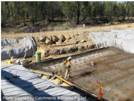
Construction of a culvert base slab
