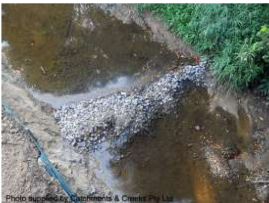
Rock filter dam
