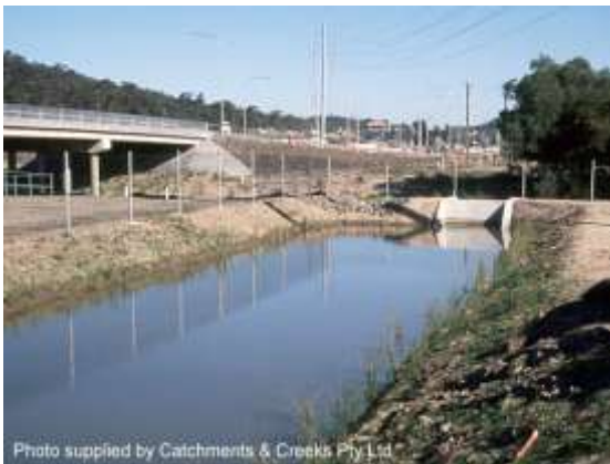
Sediment basin (Type 1 sediment trap)
