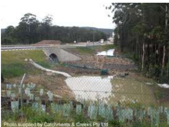
Basins retained for stormwater treatment
