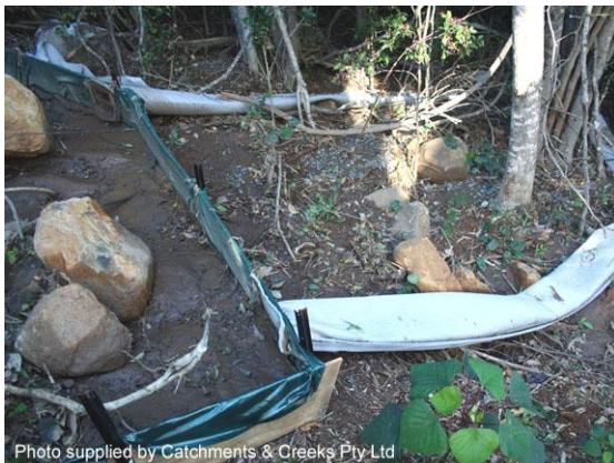
Filter tube dam sediment trap
