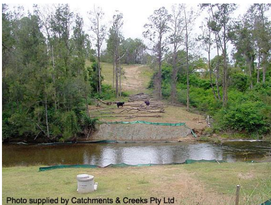
Rehabilitation of pipeline RoW
