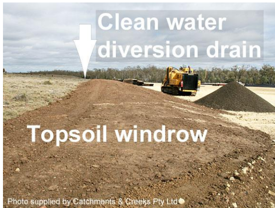
Topsoil windrow diversion drain
