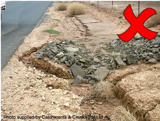
Rock check dam placed on dispersive soil
