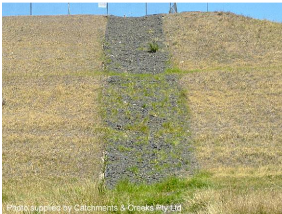
Rock-lined batter chute
