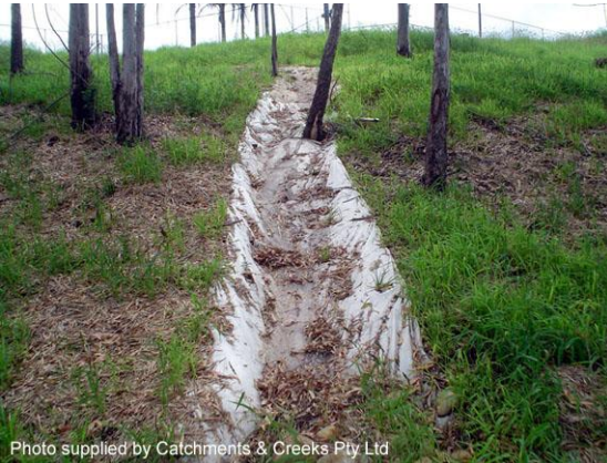
Geotextile lined drainage chute
