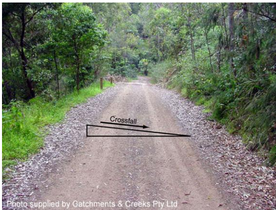
Dirt road with in-fall drainage
