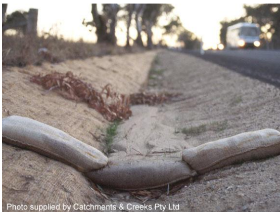
Sandbag check dam
