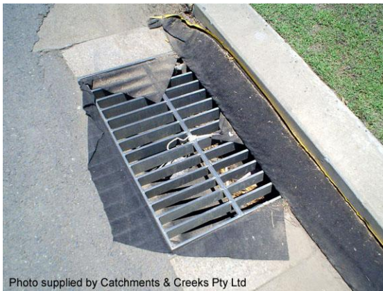
Gully bag sediment trap
