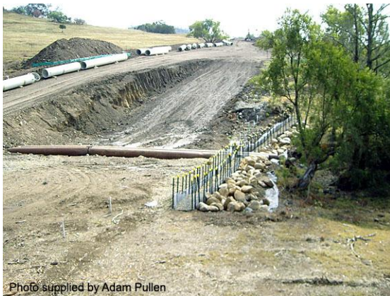
Sediment controls at waterway crossing
