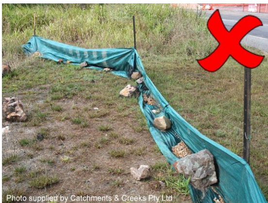
Toe of fabric incorrectly anchored
