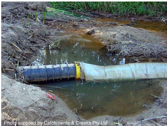
Filter tube attached to an embankment
