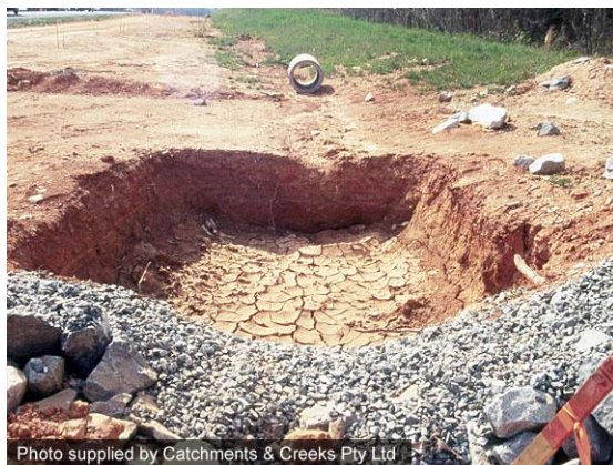
Excavated sediment sump
