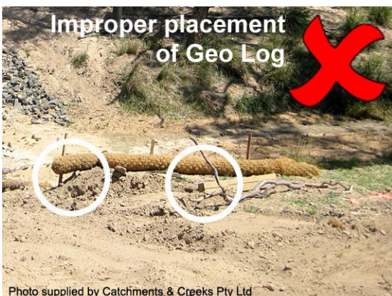
Flow allowed to pass under geo log
