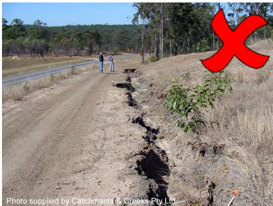
Catch drain cut into a dispersive soil
