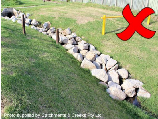
Newly established rock chute
