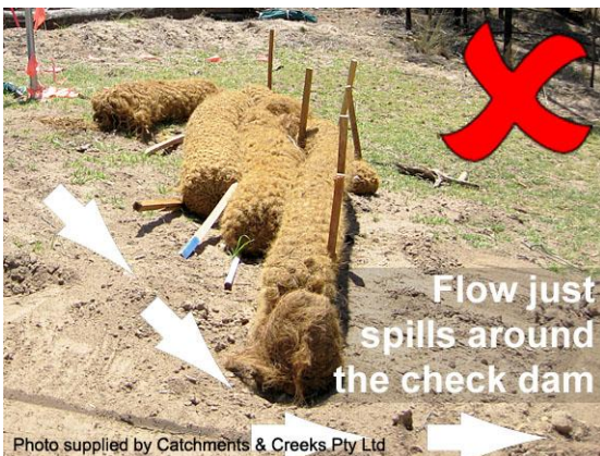
Flow allowed to pass around geo logs
