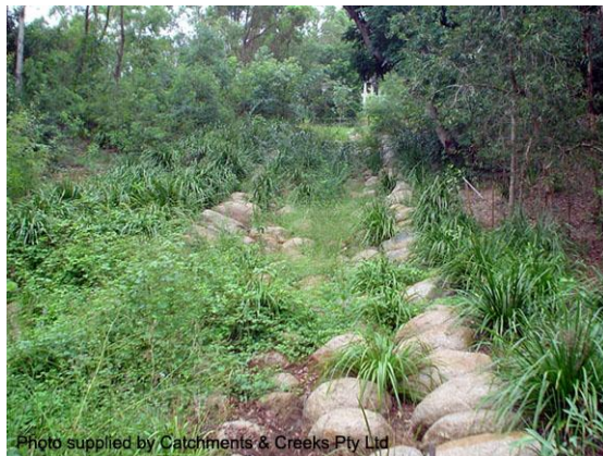
Vegetated rock-lined batter chute
