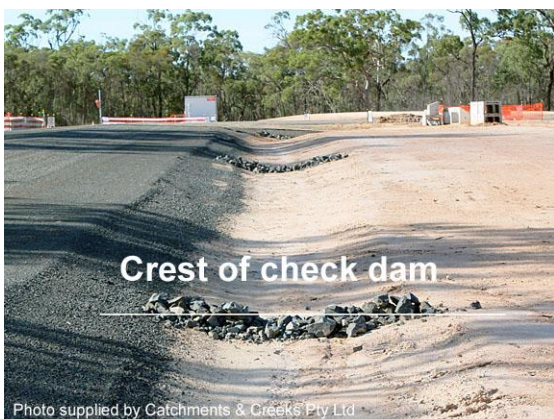
Rock check dam
