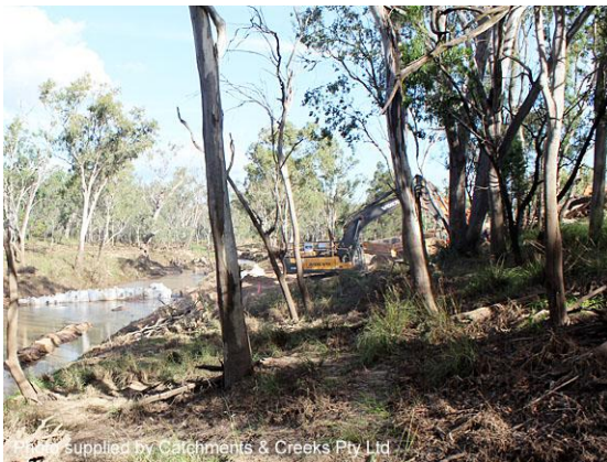
Land clearing adjacent to a crossing
