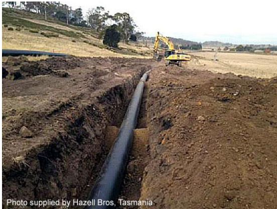
Installation of an irrigation pipeline
