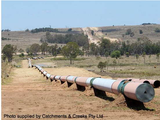
Pipeline prior to trenching
