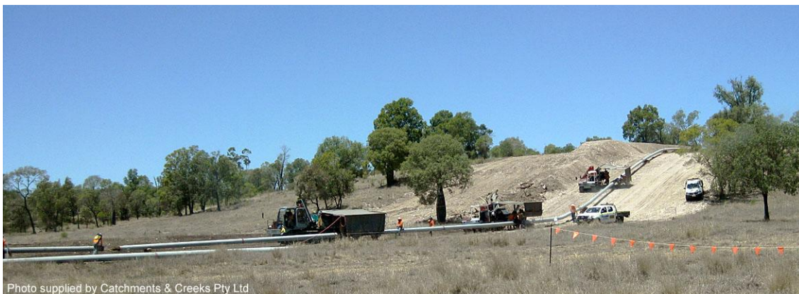
Pipe preparation prior to trenching
