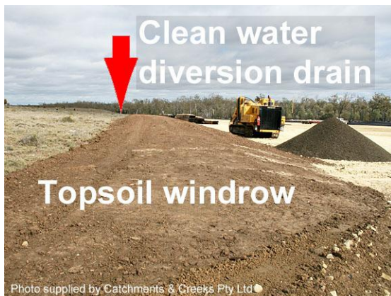
Topsoil windrow flow diversion bank
