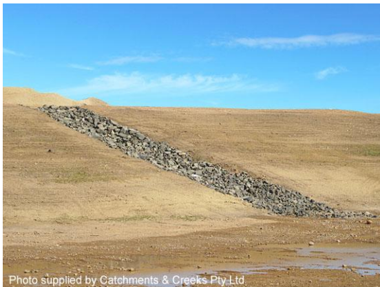
Rock-lined batter chute
