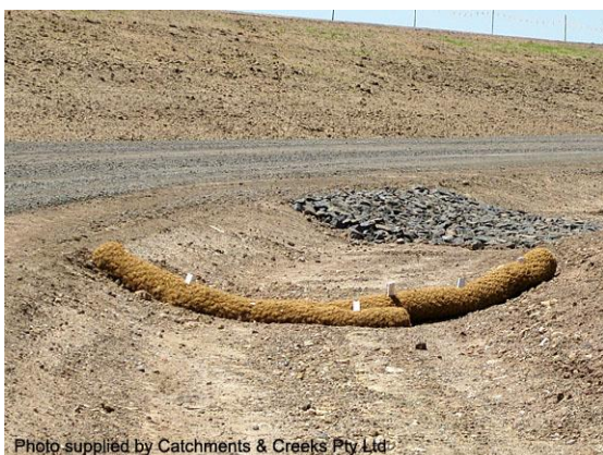
Geo log check dam
