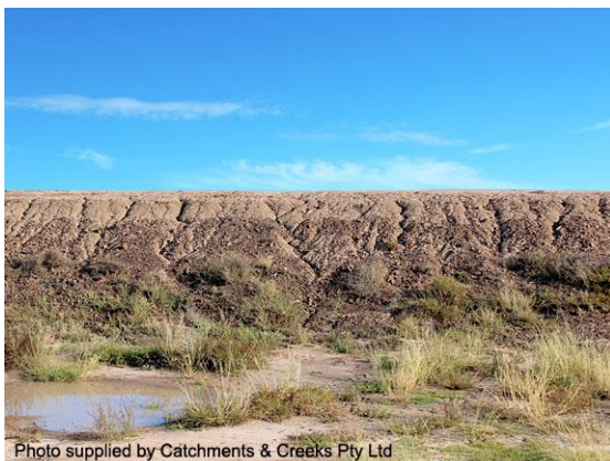
Rilling that extends to top of bank
