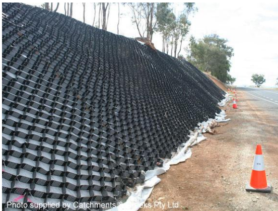
Installation on road batter
