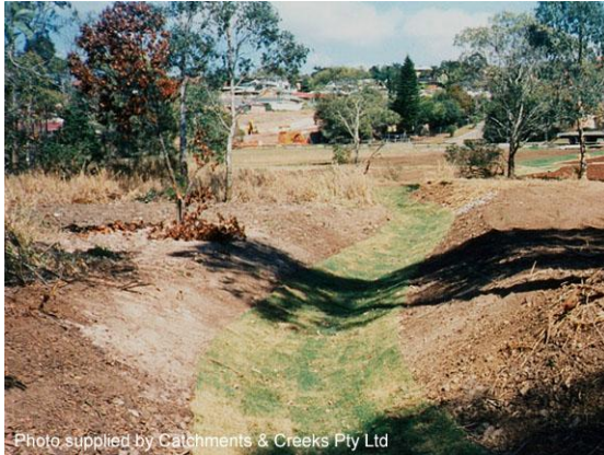
Turf lined diversion drain
