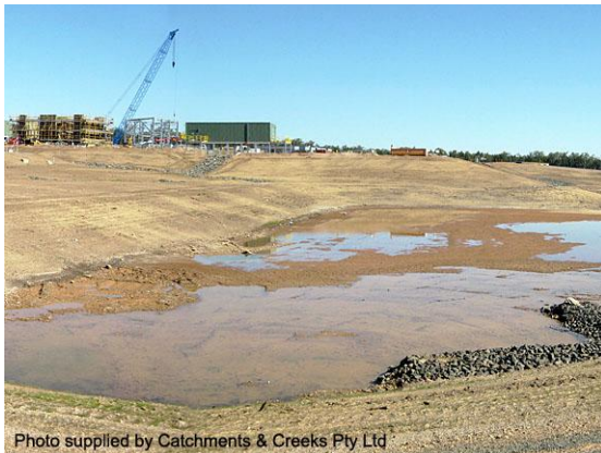
Sediment basin at a gas processing plant
