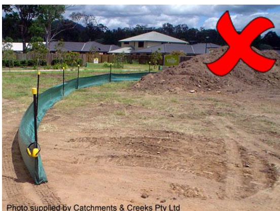
Post placed on wrong side of fence
