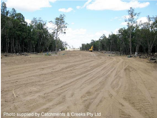
Cleared pipeline RoW
