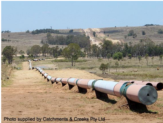
Assembled pipeline prior to trenching
