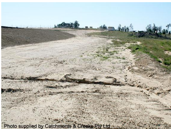
Rill erosion across an access track
