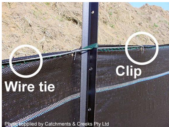
Sediment fence with top wire
