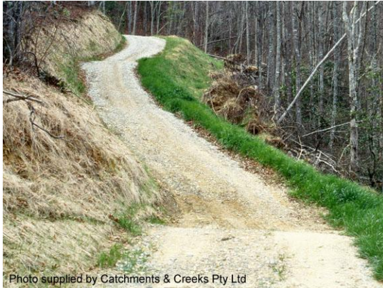
Permanent maintenance access road
