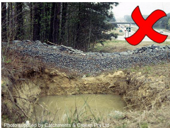
Excavated sediment trap
