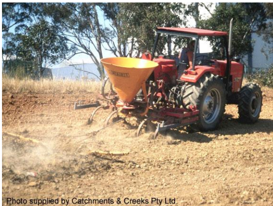
Seeding road batter
