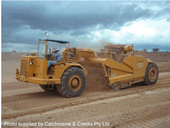
Scraper stripping soil
