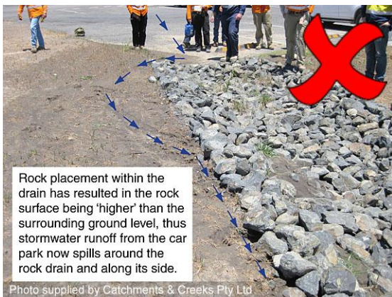
Rock sits above adjacent ground
