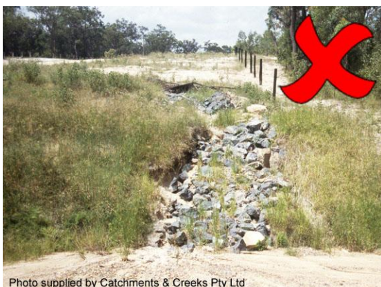
Batter chute placed on a dispersive soil
