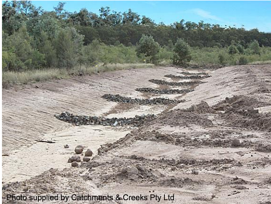
Check dam sediment trap
