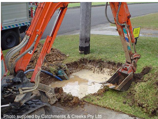
Pipe trench de-watering
