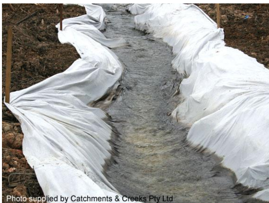
Temporary diversion drain
