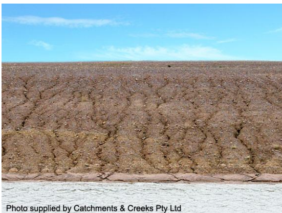
Severe rilling known as 'fluting'
