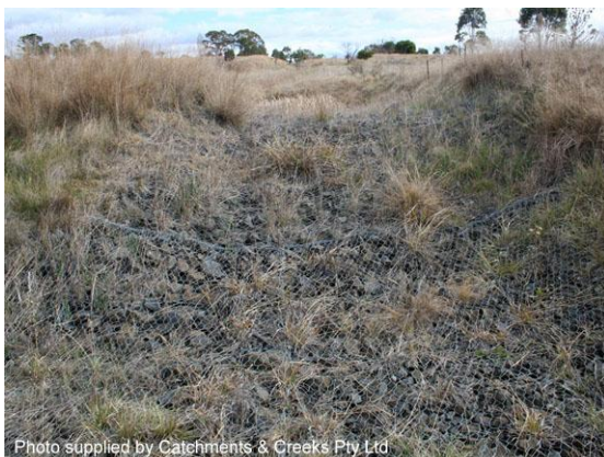
Rock mattress-lined basin spillway
