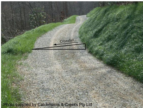
Gravel road with out-fall drainage
