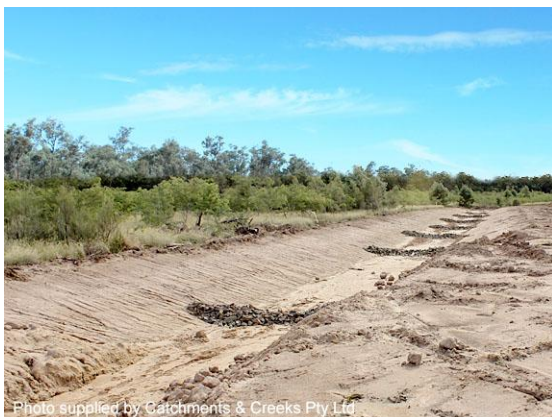
Rock check dams
