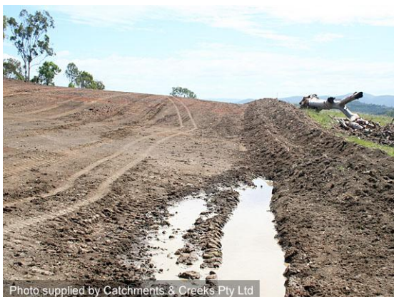
Flow diversion topsoil windrow
