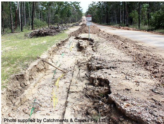
Erosion along a slaking soil trench
