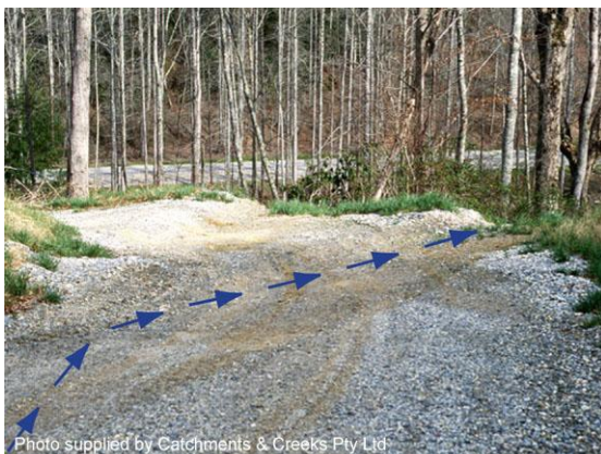
Cross bank drainage
