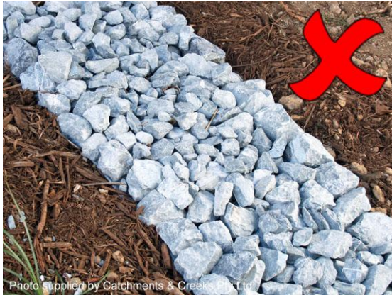
Rock-lined stormwater drain
