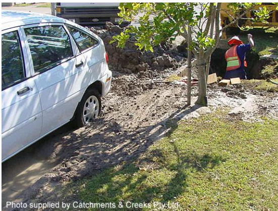
Repairing a pressure pipe failure
