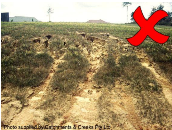
Erosion of recently seeded surface
