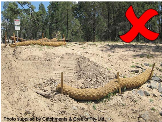
Geo log placed on steep slope
