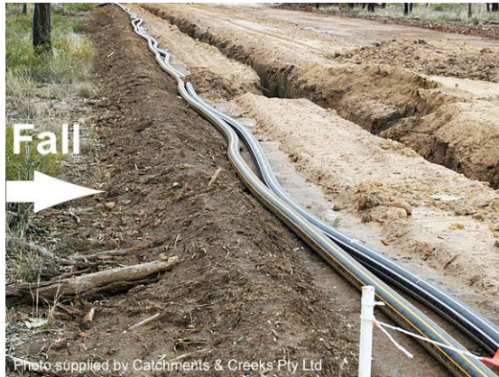
Topsoil windrow up-slope of trench
