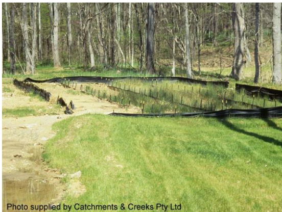
Coarse sediment trap
