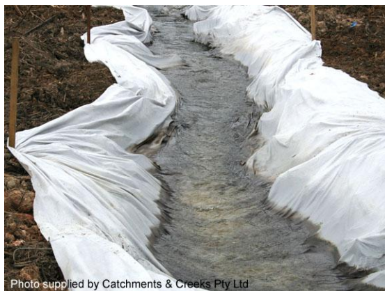
Filter cloth anchored with timber stakes
