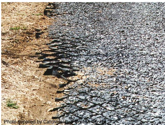
Gravelled car park
