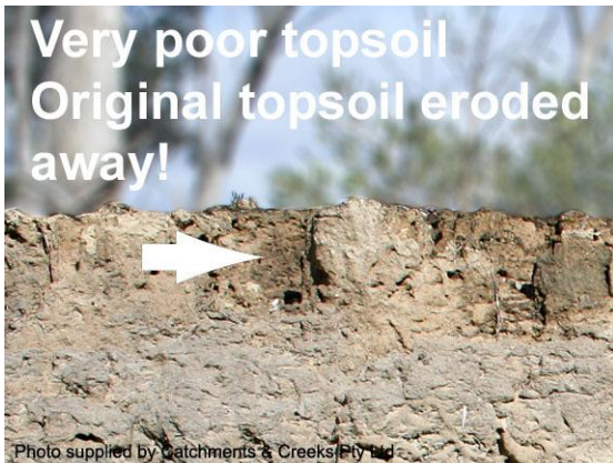
Poor quality topsoil
