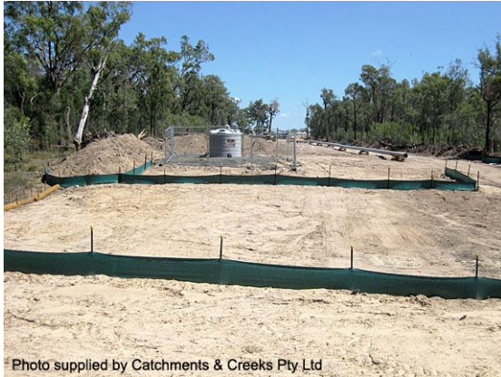
ESC measures on a pipeline RoW
