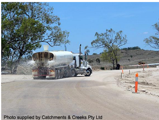
Water truck used for dust control
