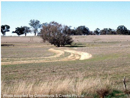
Flow diversion drain
