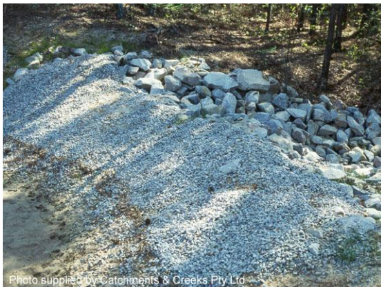
Rock filter dam with aggregate filter
