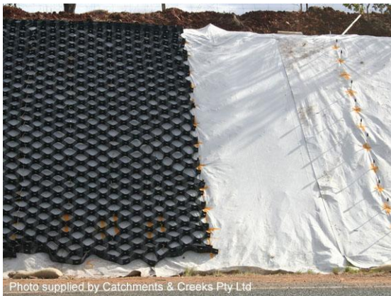
Installation on road batter
