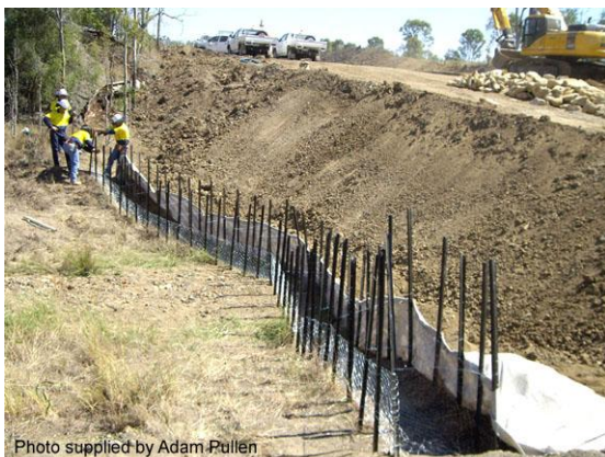
Construction of a sediment weir
