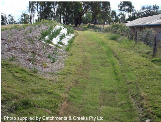
Wide, shallow, grass-lined drain
