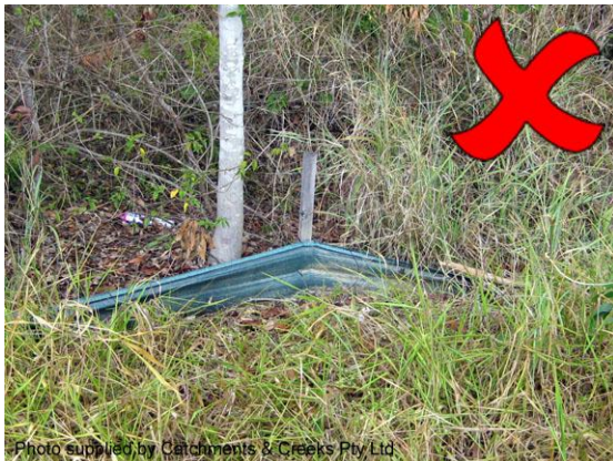
Sediment fence not removed after use
