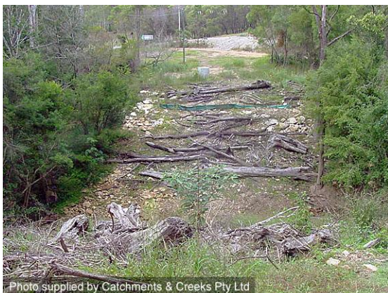
Placement of tree debris over RoW
