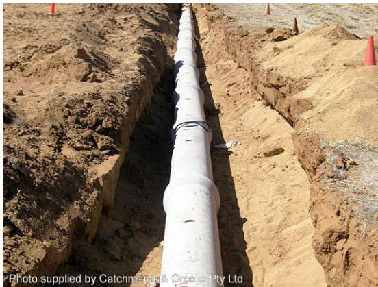
Installation of a stormwater pipeline
