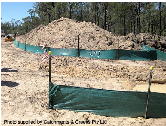
Sediment trap on pipeline RoW
