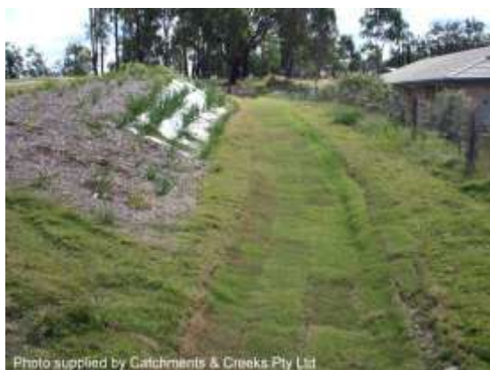
Wide, shallow, grass-lined drain
