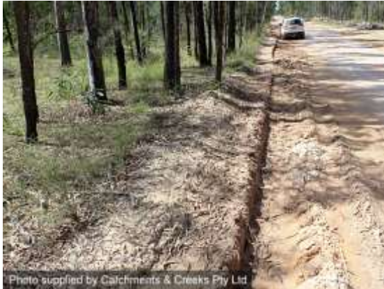
Sunken access road
