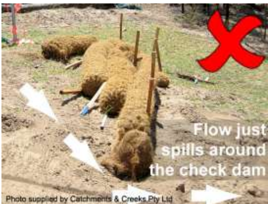
Flow allowed to pass around geo logs
