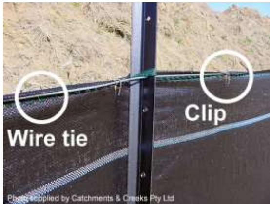
Sediment fence with top wire
