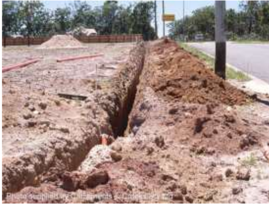
Domestic pipe installation
