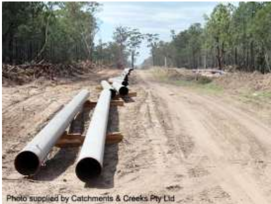
Pipeline installation project
