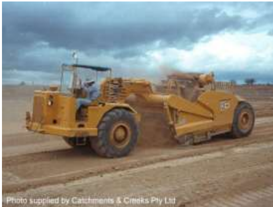
Scraper stripping soil
