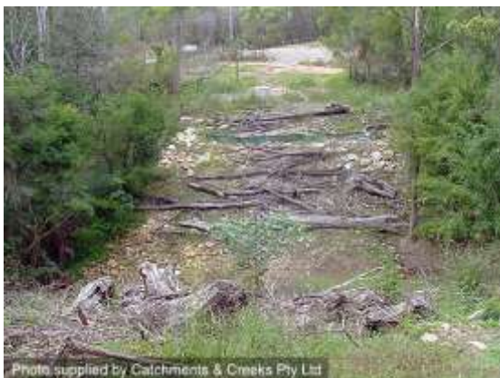
Placement of tree debris over RoW
