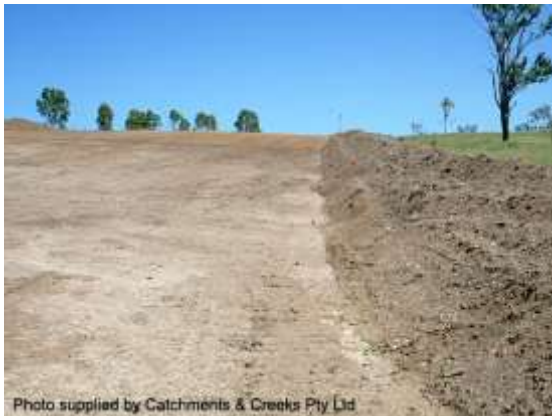
Topsoil windrow down-slope of RoW
