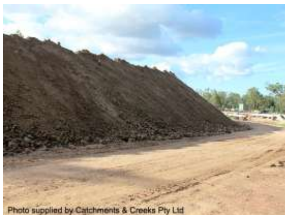
Topsoil stockpile
