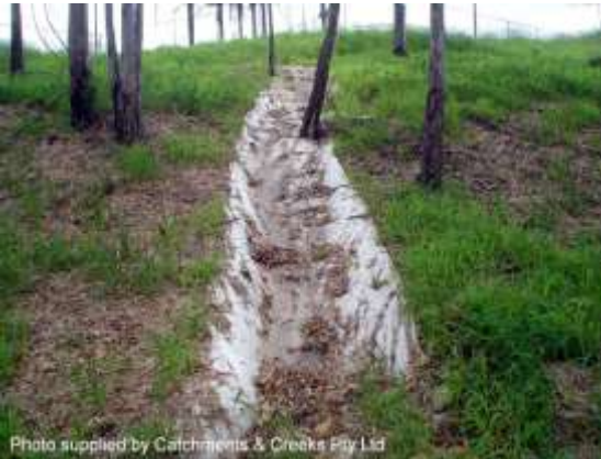
Geotextile lined drainage chute
