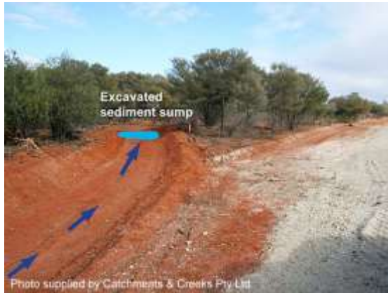
Excavated sediment sump
