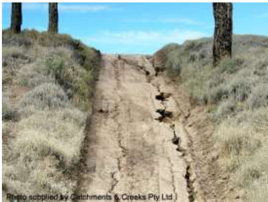
Steep, dispersive soil access track
