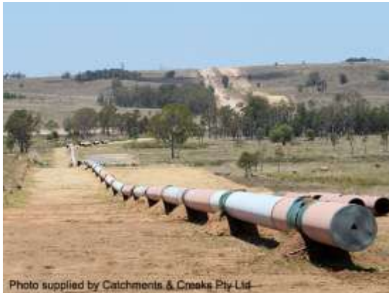
Assembled pipeline prior to trenching
