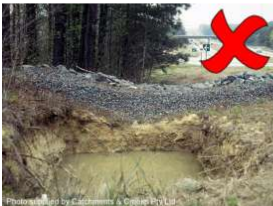
Excavated sediment trap
