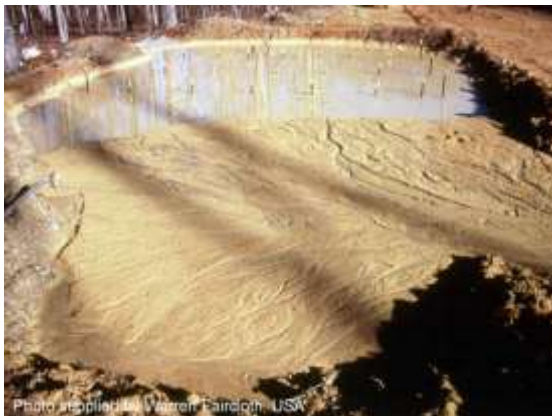
Sediment retained in a sediment trap
