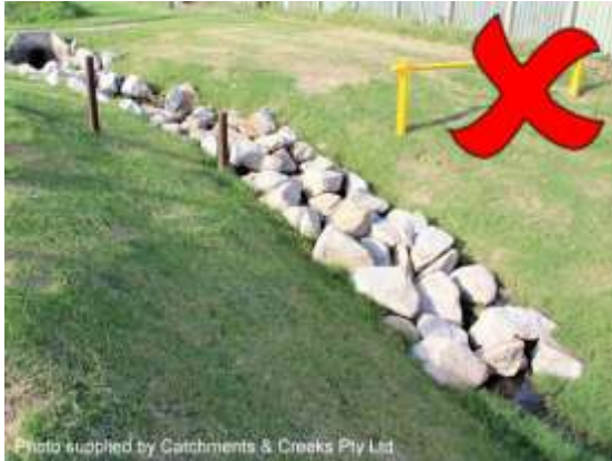
Newly established rock chute
