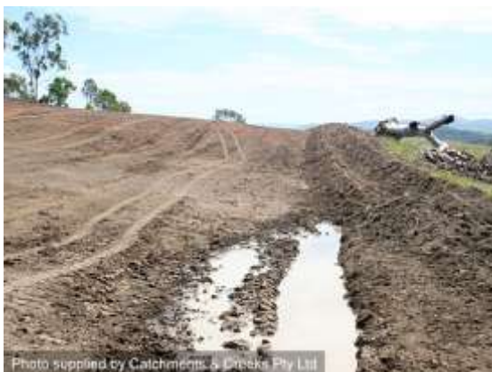
Flow diversion topsoil windrow
