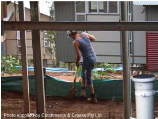
Maintenance of control measures
