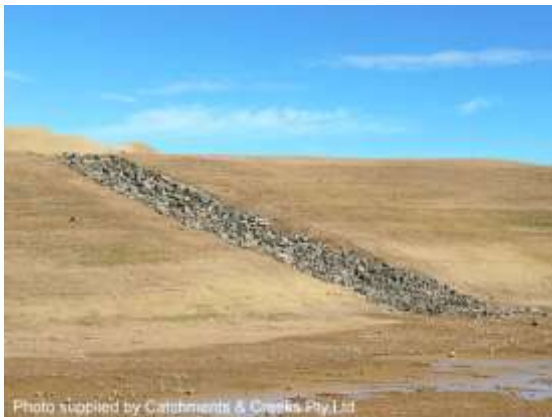
Rock-lined batter chute
