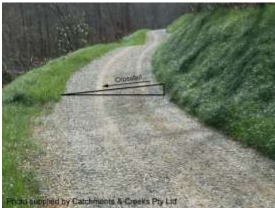
Gravel road with out-fall drainage
