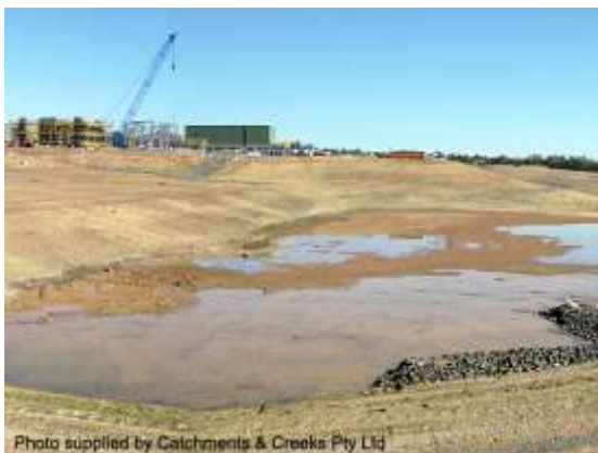
Sediment basin at a gas processing plant
