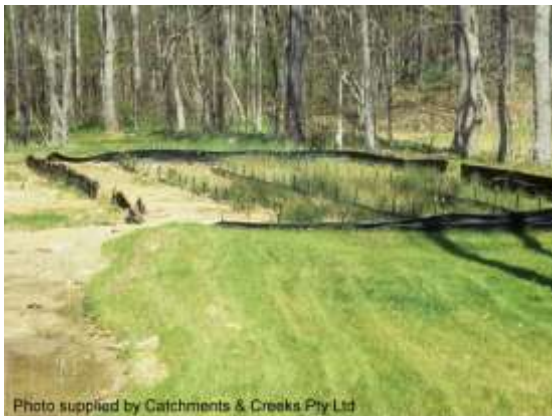
Coarse sediment trap
