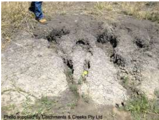
Deep rilling and tunnel erosion
