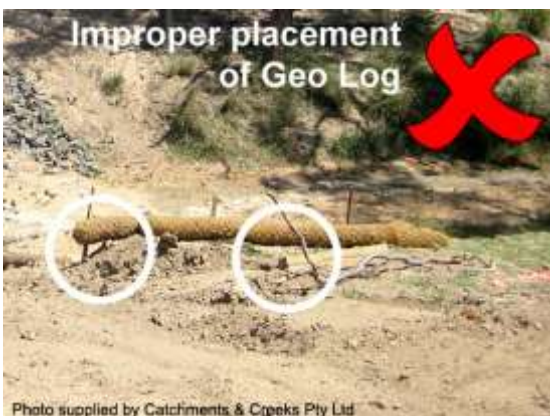
Flow allowed to pass under geo log
