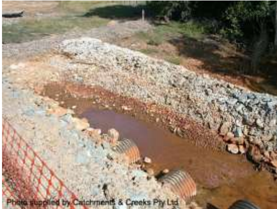
Rock filter dam with aggregate filter
