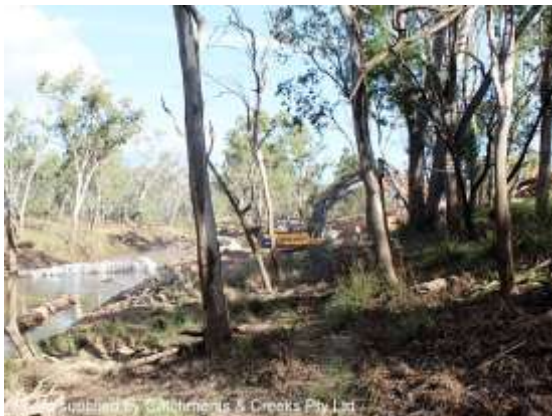
Land clearing adjacent to a crossing
