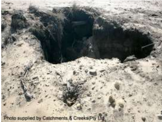
Entrance to tunnel erosion
