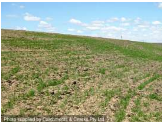
Grass establishment on embankment
