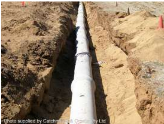
Installation of a stormwater pipeline
