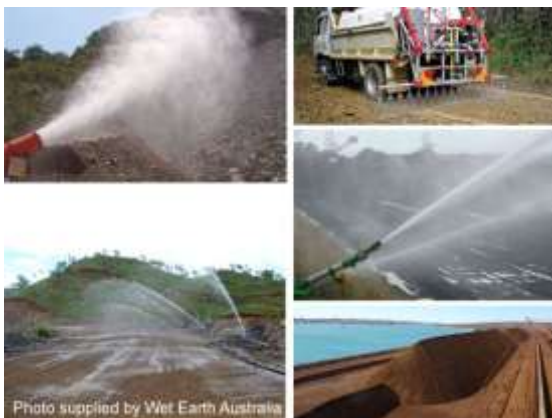
Application of soil binders
