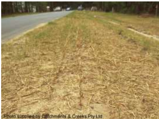
Straw mulching of road shoulder
