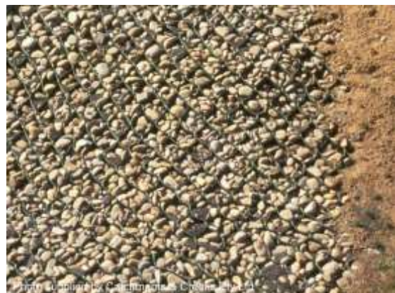
Gravelled batter slope
