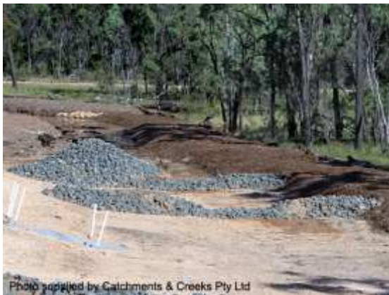
Velocity control check dams
