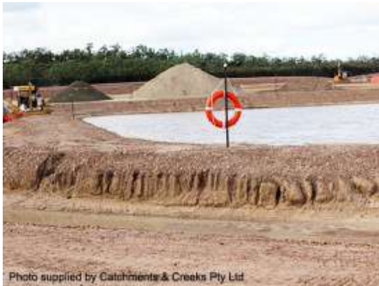
'Wet' type sediment basin
