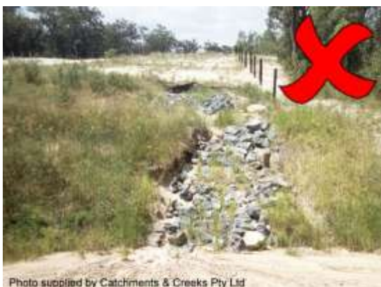
Batter chute placed on a dispersive soil
