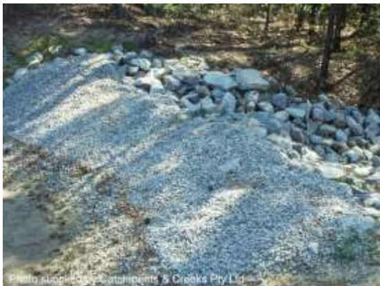
Rock filter dam with aggregate filter
