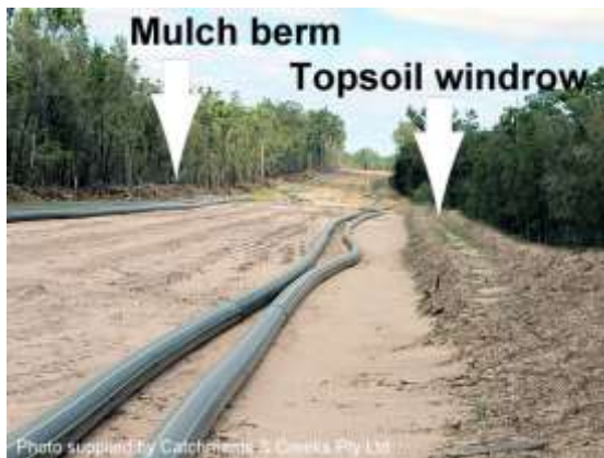
Pipeline prior to trenching
