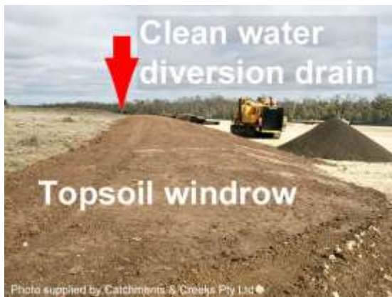
Topsoil windrow flow diversion bank
