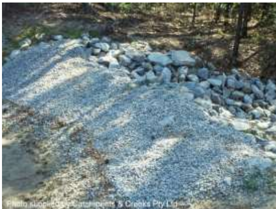
Rock filter dam - aggregate filter
