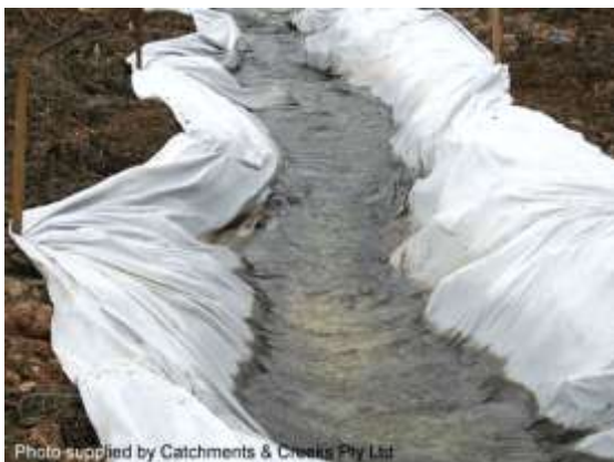
Temporary diversion drain
