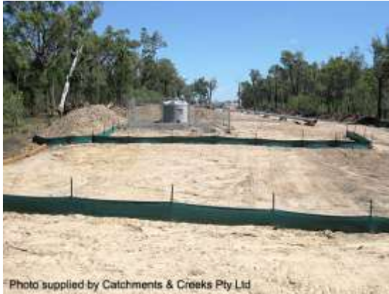
ESC measures on a pipeline RoW
