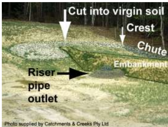
Spillway formed within virgin soil
