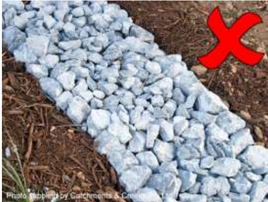
Rock-lined stormwater drain
