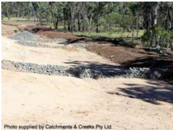
Velocity control check dams
