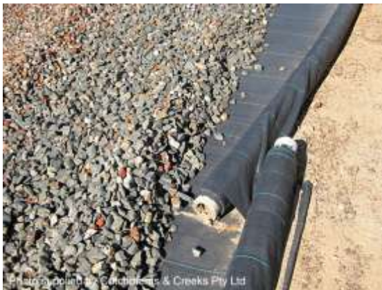
Placement of gravel over geotextile
