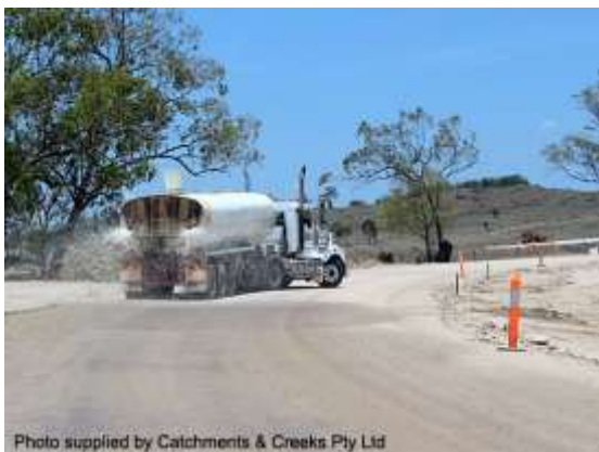
Water truck used for dust control
