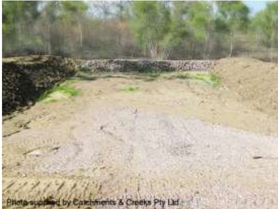
Rock filter dam
