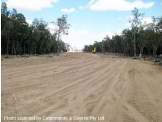
Cleared pipeline RoW
