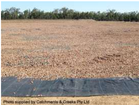
Gravelling of processing plant site
