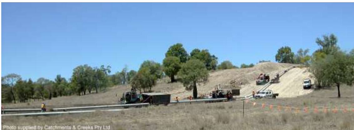
Pipe preparation prior to trenching
