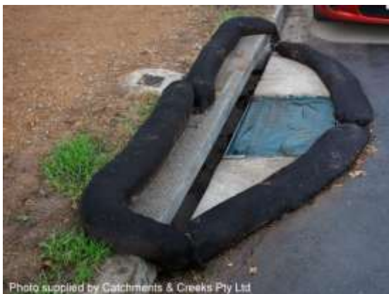
Sag-type kerb inlet protection
