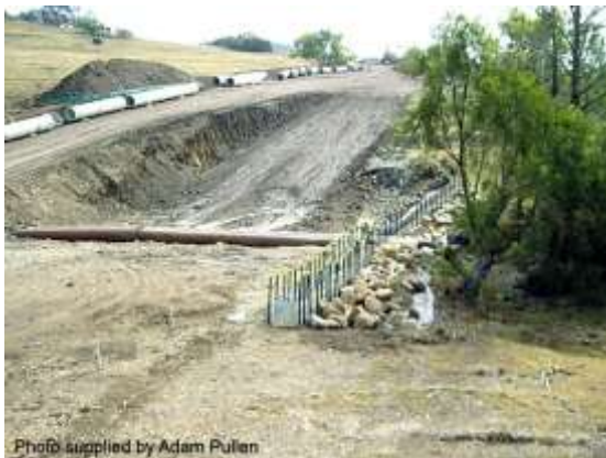
Sediment controls at waterway crossing
