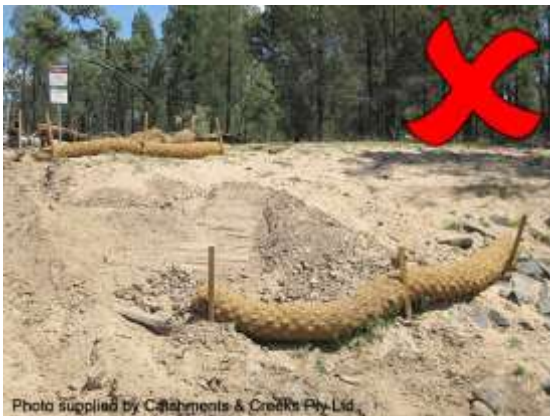
Geo log placed on steep slope
