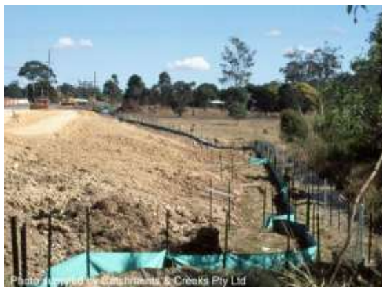
Placement of regular ‘returns’
