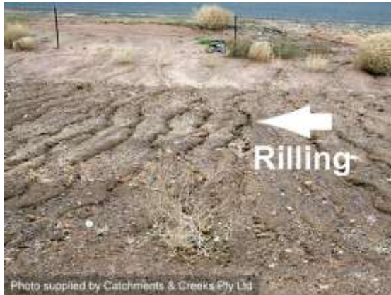
Sheet and rill erosion
