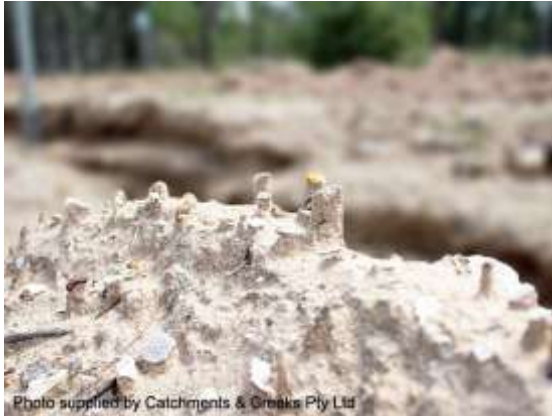
Evidence of raindrop impact erosion
