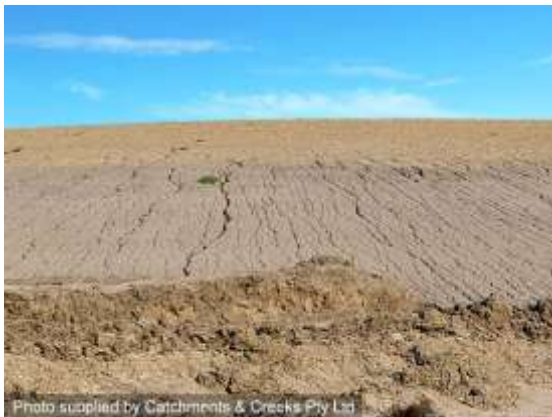
Rilling limited to a single band of soil
