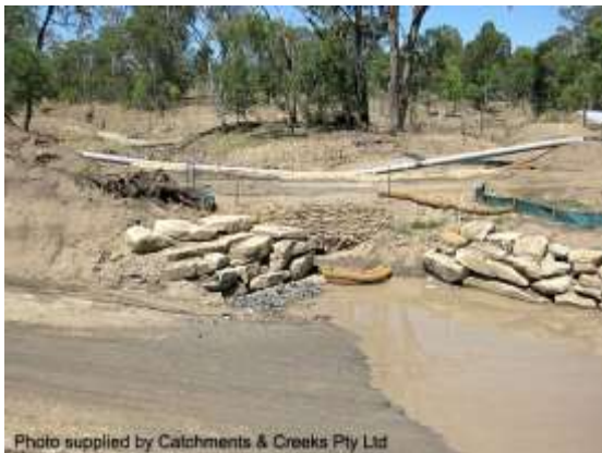
Pipeline crossing of a waterway
