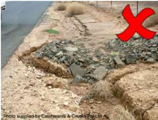
Rock check dam placed on dispersive soil
