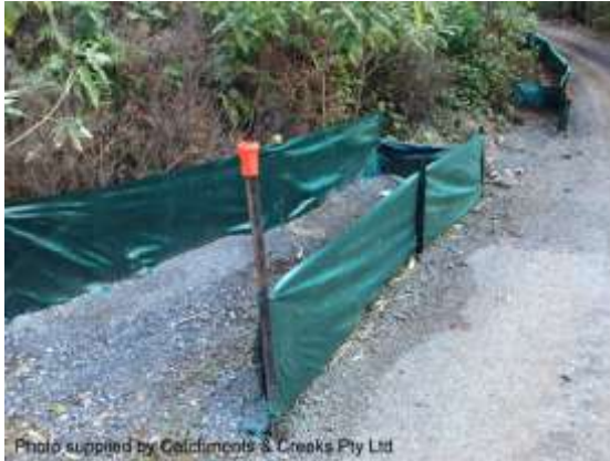
U-shaped sediment trap
