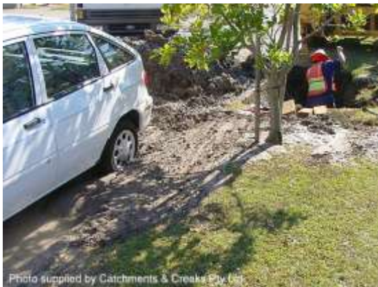
Repairing a pressure pipe failure
