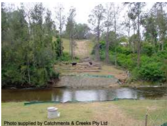
Rehabilitation of pipeline RoW
