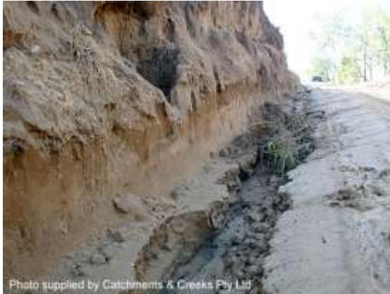
Deep rilling within a sandy soil
