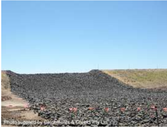
Spillway with well-defined weir profile
