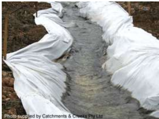
Filter cloth anchored with timber stakes
