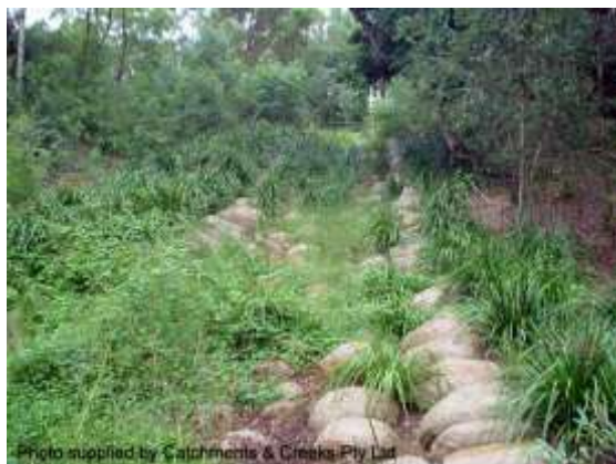
Vegetated rock-lined batter chute
