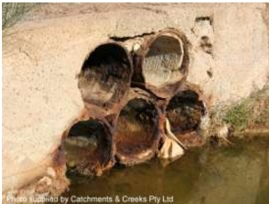
Culvert damaged by acidic water
