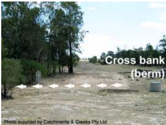
Cross drainage within pipeline RoW
