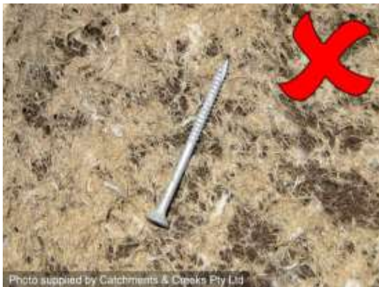
Wood screws used to anchor a blanket
