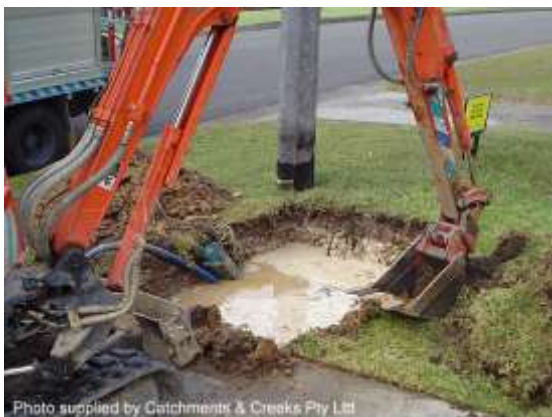
Pipe trench de-watering
