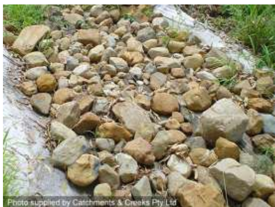
Rock-lined drainage channel
