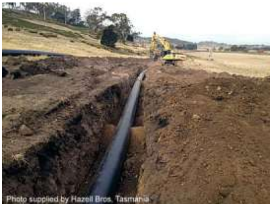
Installation of an irrigation pipeline
