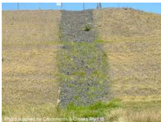
Rock-lined batter chute
