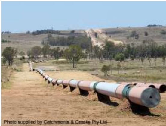
Pipeline prior to trenching
