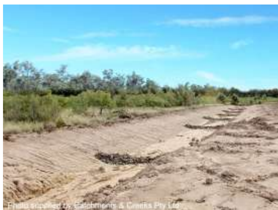
Rock check dams
