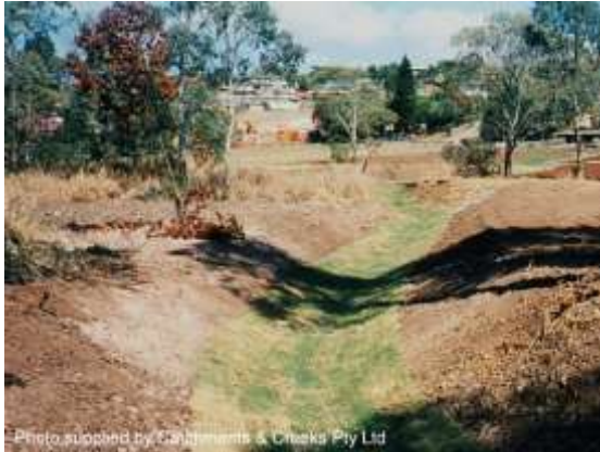
Turf lined diversion drain
