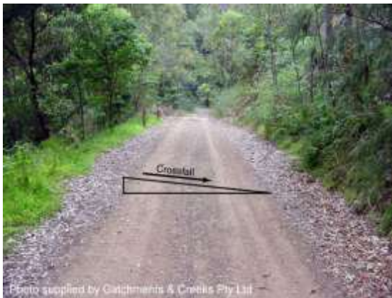
Dirt road with in-fall drainage
