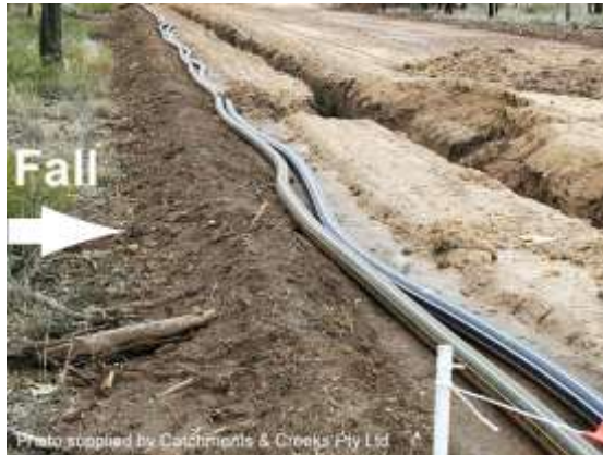
Topsoil windrow up-slope of trench
