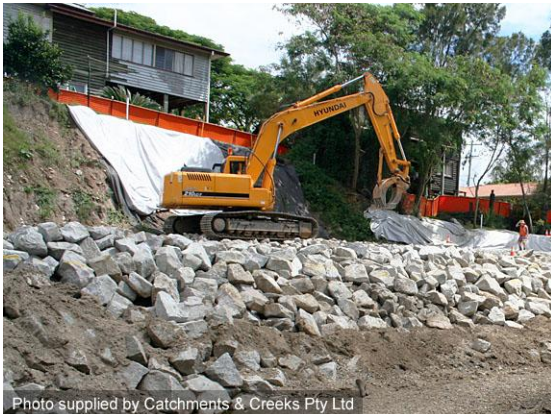
Rock placement over filter cloth
