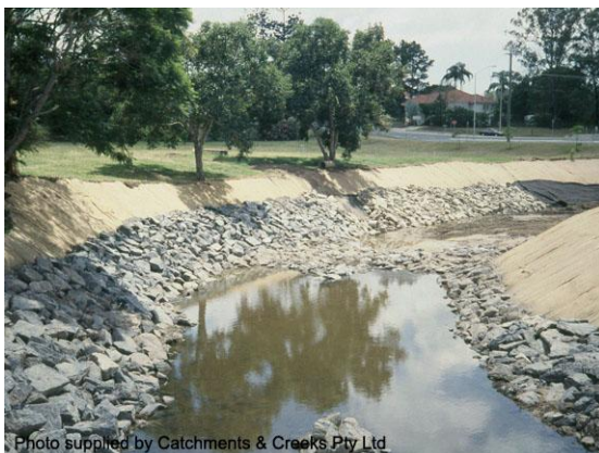
Rock stabilisation on channel bend
