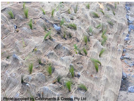
Planted rock covered with jute mesh
