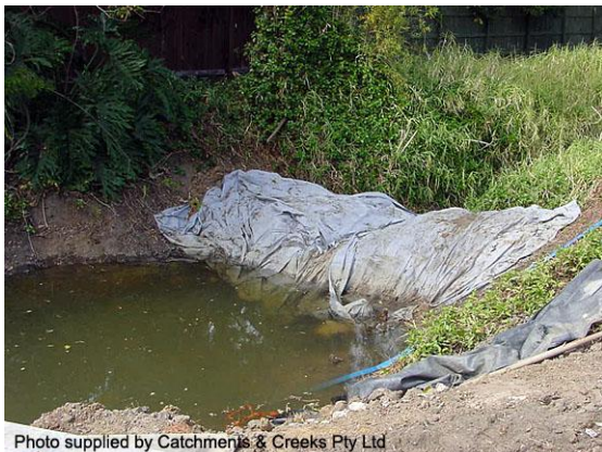
Instream rock filter dam
