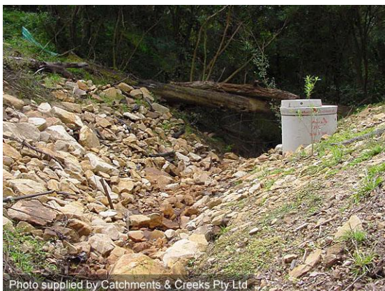
Rock-lining adjacent to an access pit
