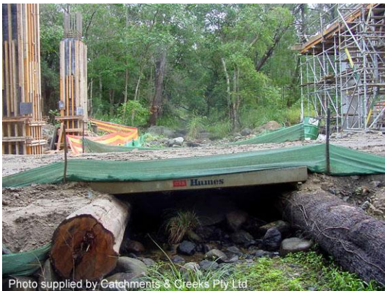
Temporary bridge crossing
