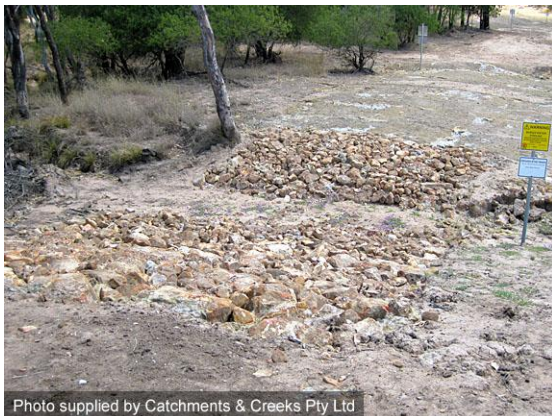
Rock stabilisation above pipeline
