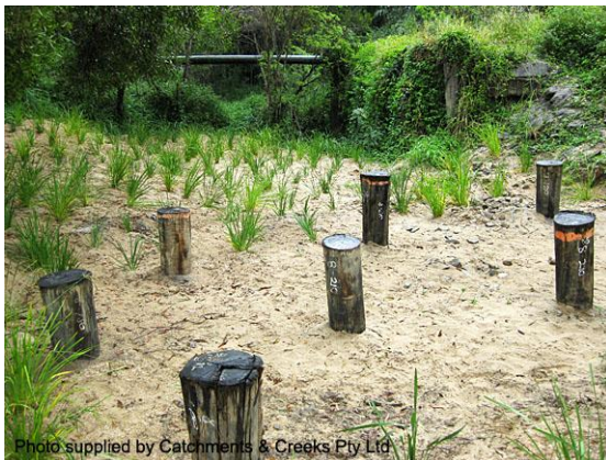
Pile field in sand-based waterway
