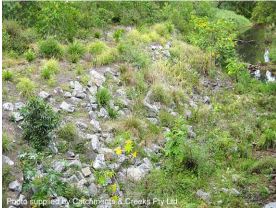
Planted rock-stabilised creek bank
