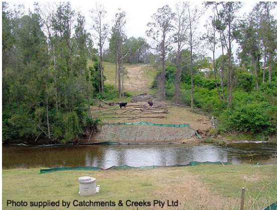
Rehabilitated pipeline crossing
