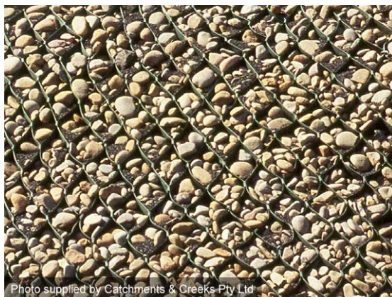
Cellular confinement system stabilisation
