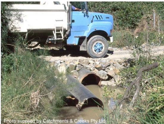
Temporary culvert crossing
