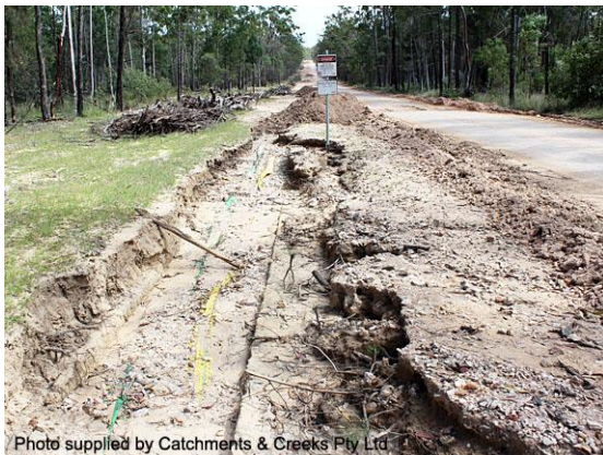
Erosion along the pipeline RoW
