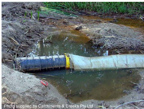
Filter tube connected to ribbed pipe
