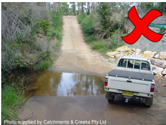
Concrete sealed 'ford' crossing
