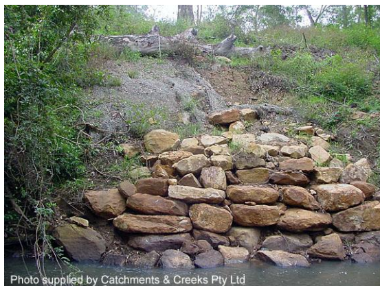
Non-vegetated rock stabilisation
