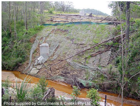
Non-vegetated rock stabilisation
