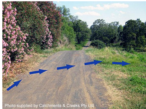
Cross bank placed at top of descent
