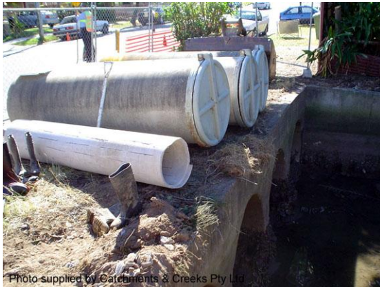
Floodgates prior to their installation
