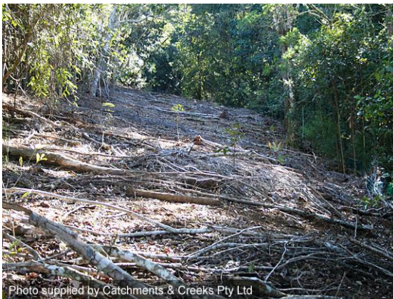
Placement of woody debris
