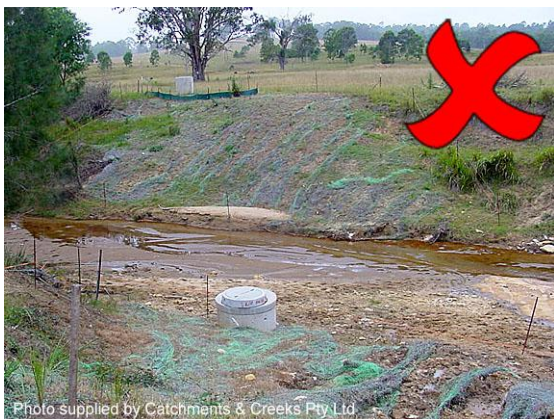
Use of synthetic reinforced mats
