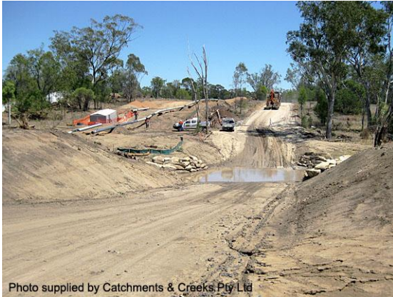
Vehicle access across a waterway
