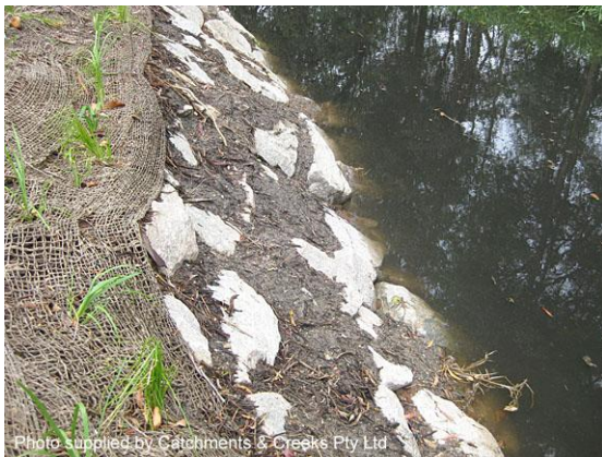
Voids filled with soil ready for planting
