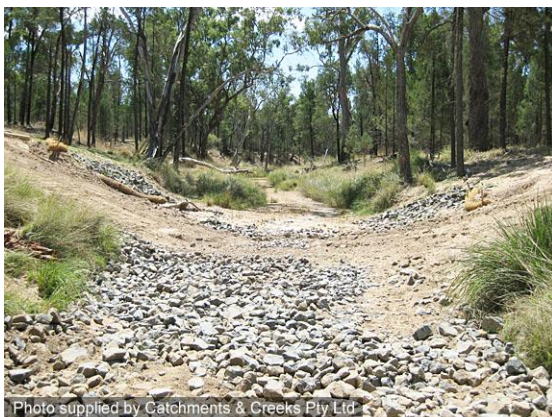
Rock-stabilised vehicle crossing
