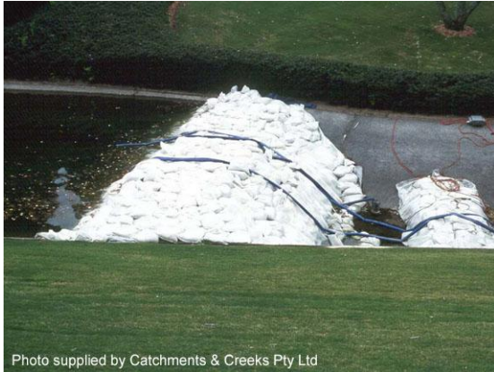
Sandbag cofferdam in concrete drain
