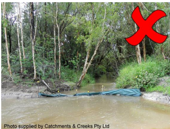
Inappropriate instream sediment control
