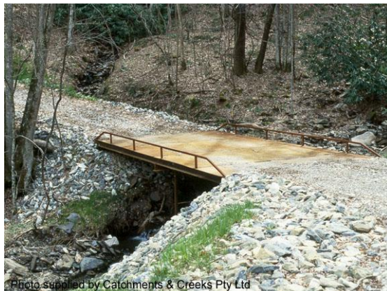
Permanent maintenance access bridge
