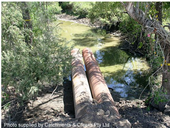
Gravity bypass pipe (flume) system
