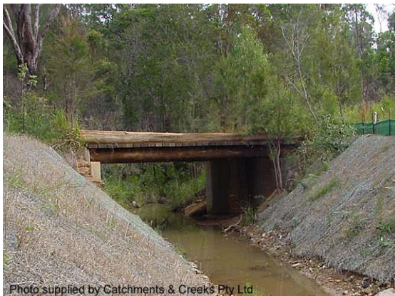
Permanent maintenance access bridge
