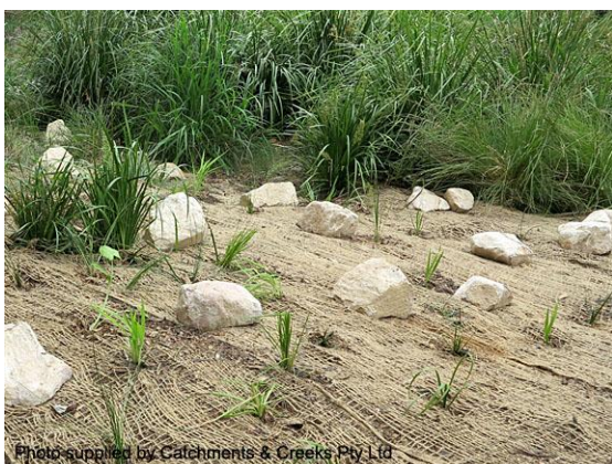
Erosion control jute mesh
