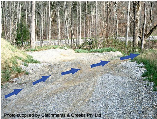
Flows diverted off access track
