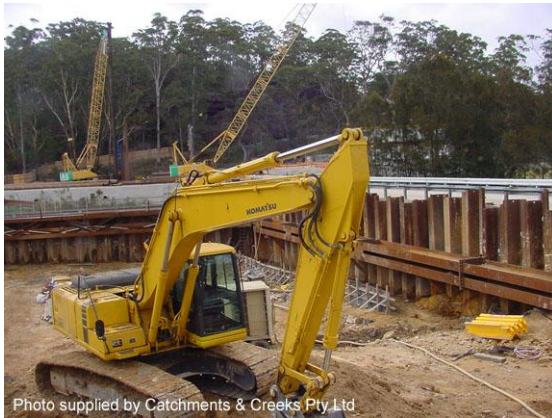
Sheet piling isolation barrier
