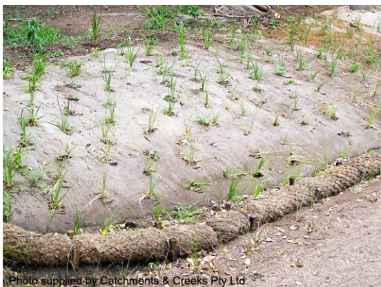
Coir geo-log temporary toe protection
