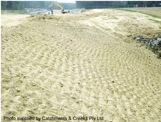
Roughened earth batter
