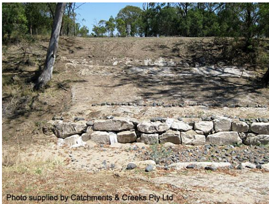
Rock-stabilised pipe crossing
