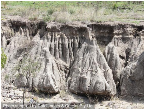
Unstable gully banks (fluting erosion)
