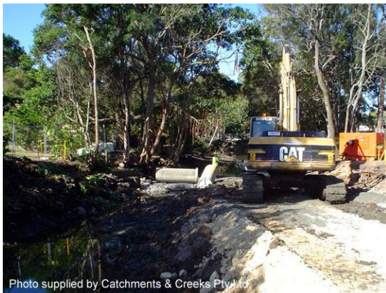
Construction of a cofferdam
