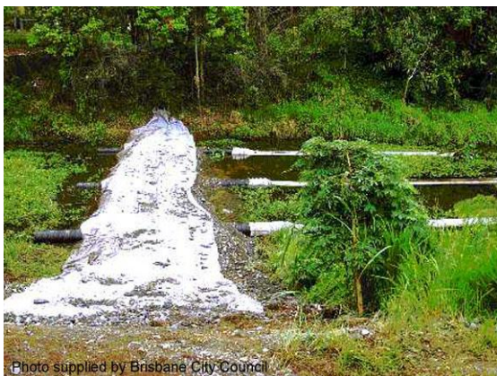
Rock filter dam with filter tubes
