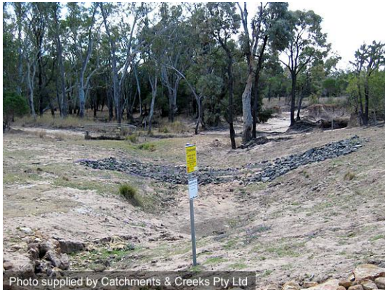
Rock-stabilised vehicle crossing
