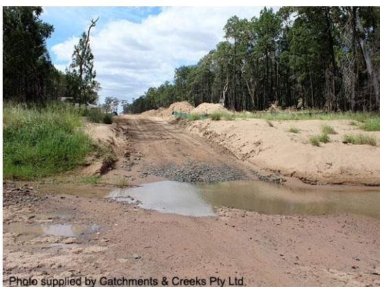
Crossing of a sand-based watercourse
