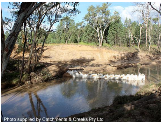
Construction of a pipeline crossing
