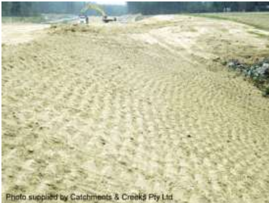
Roughened earth batter
