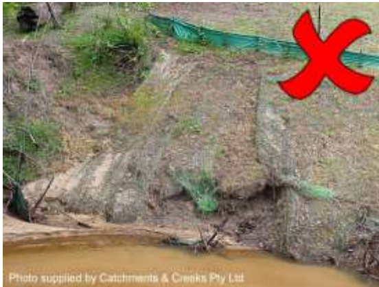
Erosion along toe of bank
