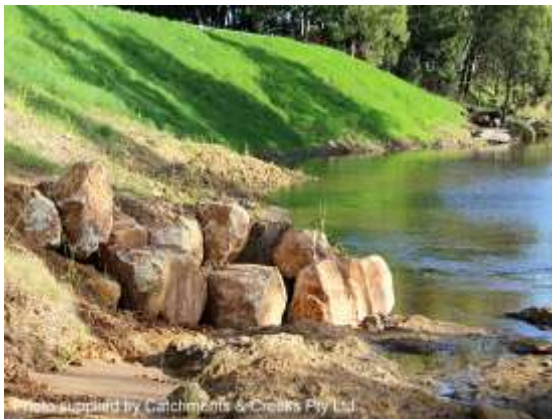
Rock flow control groyne
