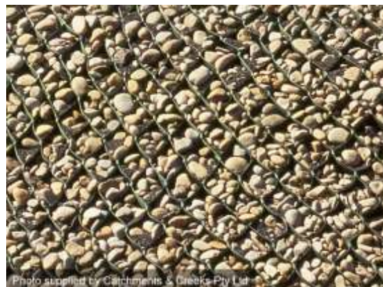
Cellular confinement system stabilisation
