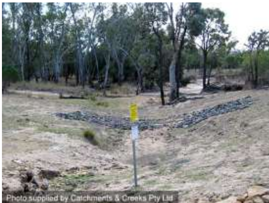
Rock-stabilised vehicle crossing
