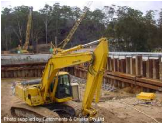
Sheet piling isolation barrier
