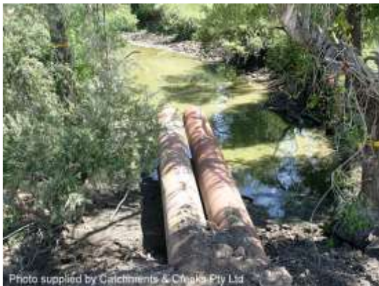
Gravity bypass pipe (flume) system
