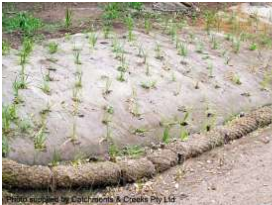
Coir geo-log temporary toe protection
