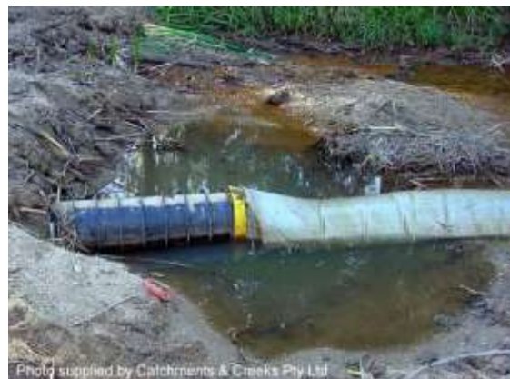
Filter tube connected to ribbed pipe
