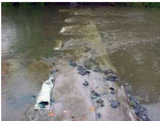
Elevated stream flows at work site
