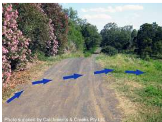
Cross bank placed at top of descent
