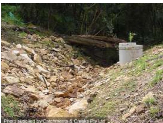
Rock-lining adjacent to an access pit
