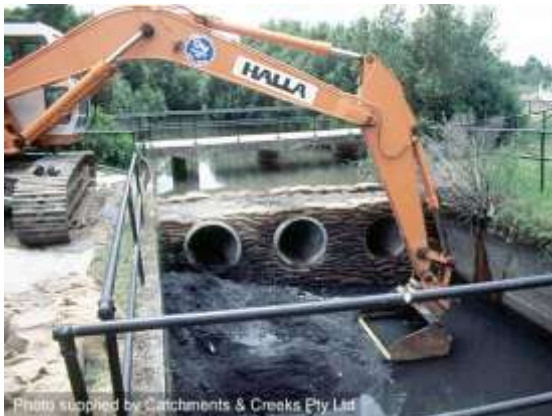
Works within a tidal waterway
