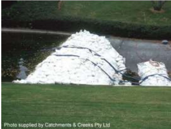
Sandbag cofferdam in concrete drain
