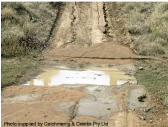
Boggy drainage line crossing
