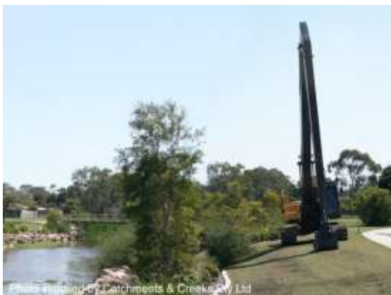
Long reach excavator
