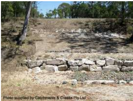
Rock-stabilised pipe crossing
