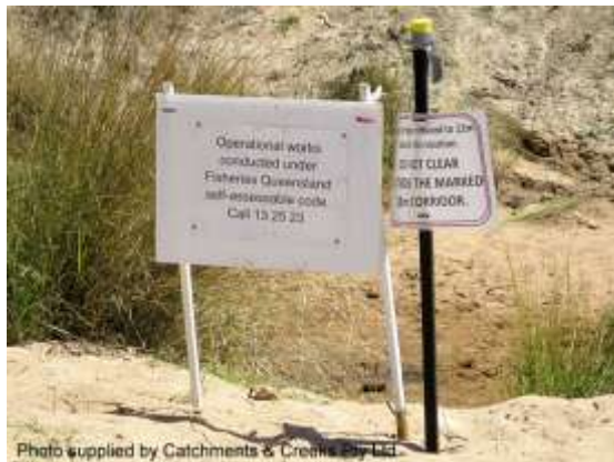
Signage at in-stream works
