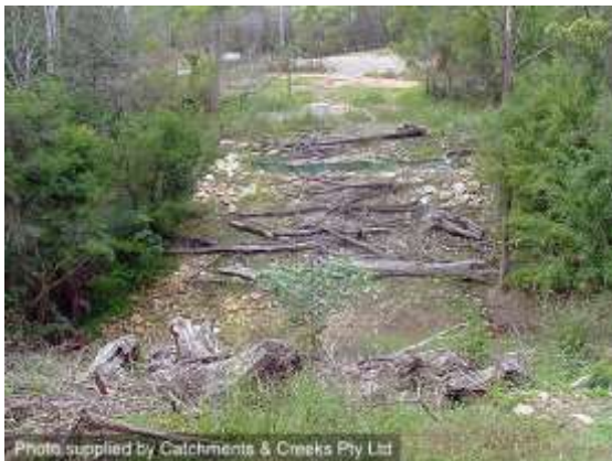
Bank stabilisation measures
