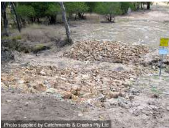
Rock stabilisation above pipeline
