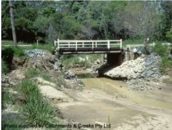
Timber bridge prior to 1996 flood
