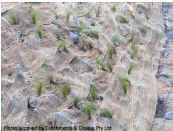
Planted rock covered with jute mesh
