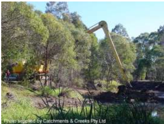
Use of a long-reach excavator
