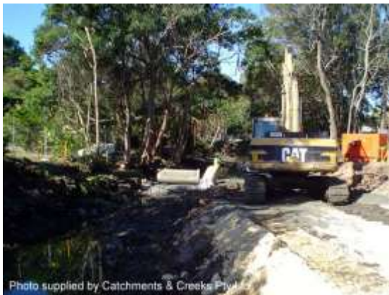
Construction of a cofferdam
