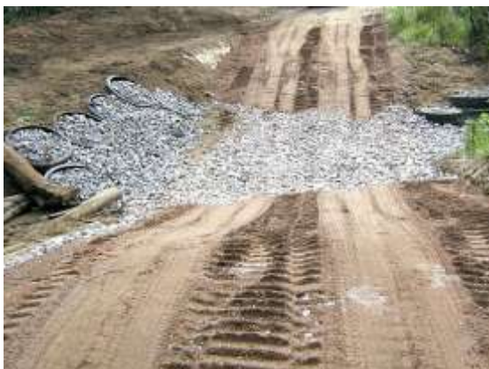
Ecoflex 'E-pave' stabilisation system
