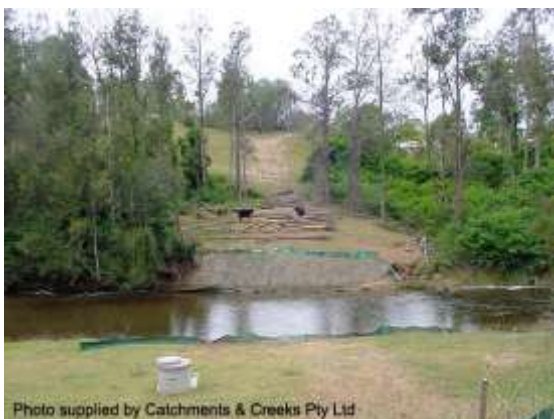
Rehabilitated pipeline crossing
