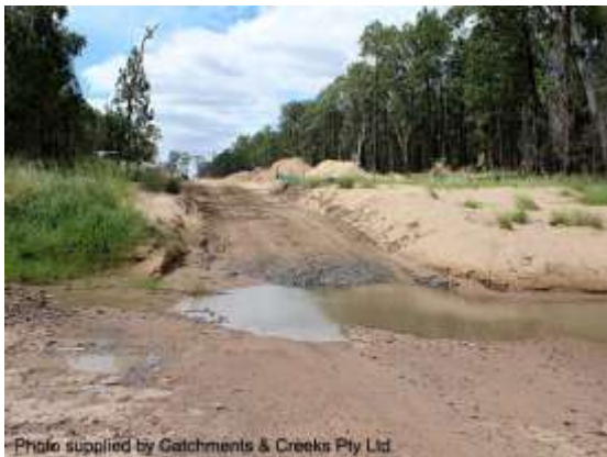
Crossing of a sand-based watercourse
