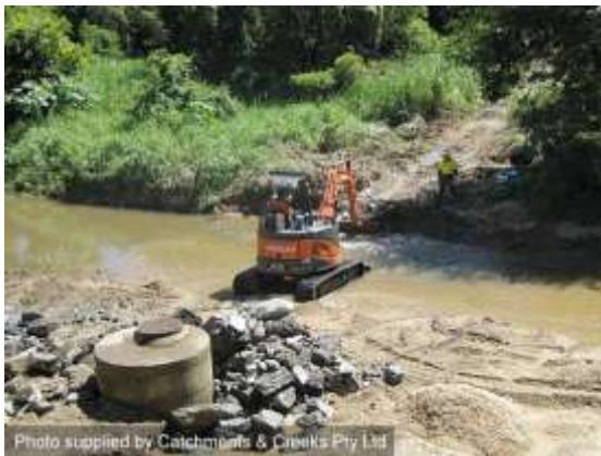
Works within a sandy waterway
