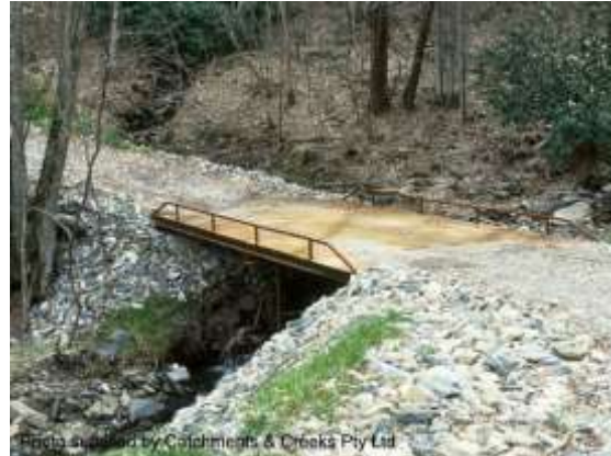
Permanent maintenance access bridge
