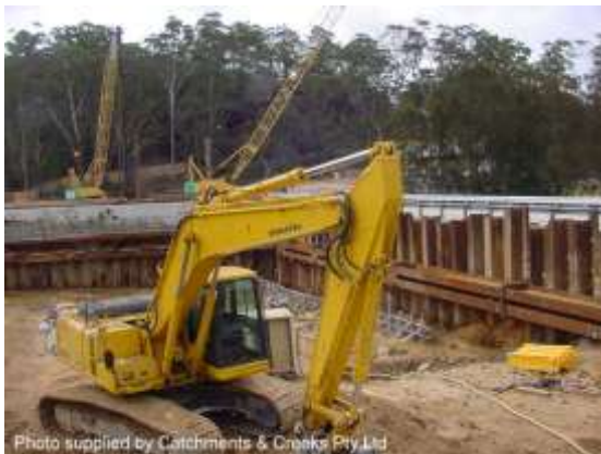
Use of sheet piling isolation barrier
