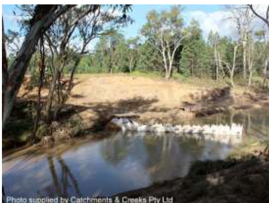
Construction of a pipeline crossing
