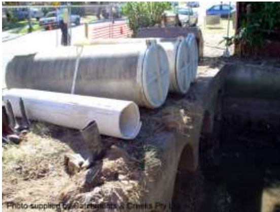
Floodgates prior to their installation
