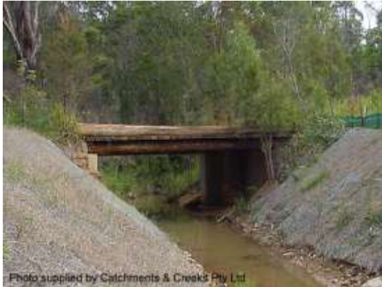
Permanent maintenance access bridge
