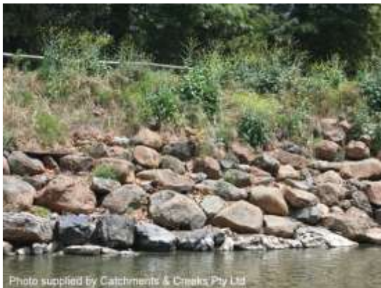
Partial vegetated bank stabilisation
