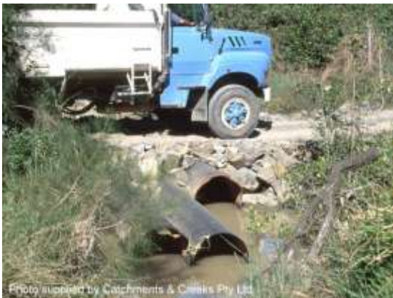
Temporary culvert crossing
