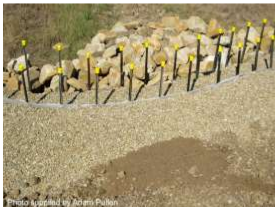
Sediment control weir
