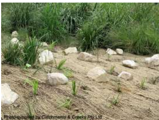
Erosion control jute mesh
