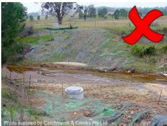
Use of synthetic reinforced mats
