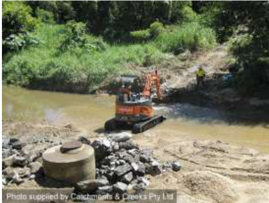
Instream construction works
