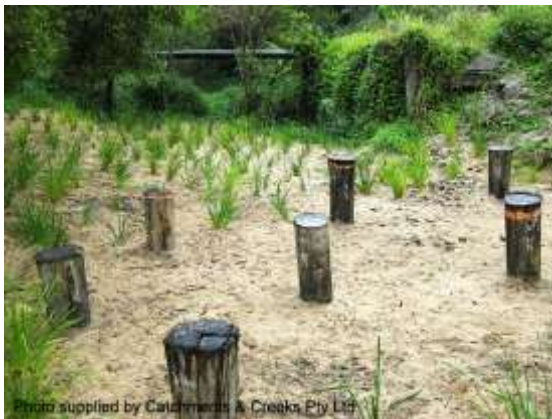
Pile field in sand-based waterway
