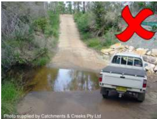
Concrete sealed 'ford' crossing
