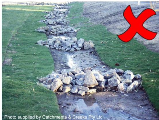
Flows forced to pass around check dams
