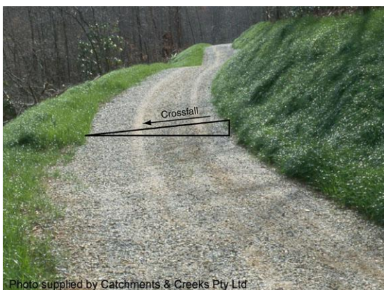
Gravel road with out-fall drainage
