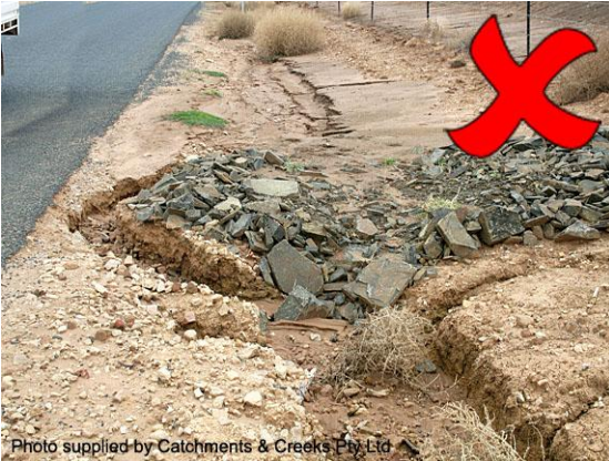
Rock check dam placed on dispersive soil
