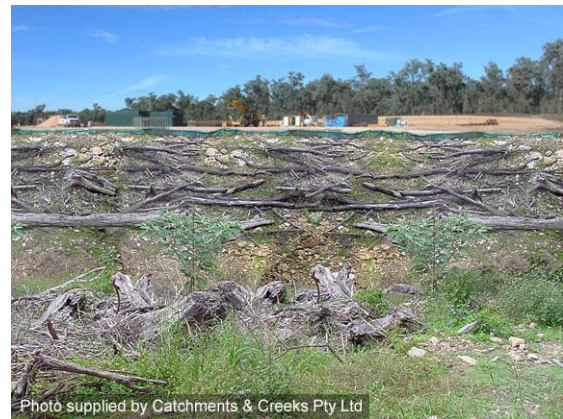
Brushwood used to stabilise a batter
