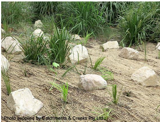
Jute mesh anchored with rocks
