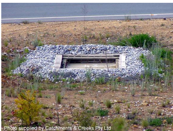
Block & aggregate drop inlet protection
