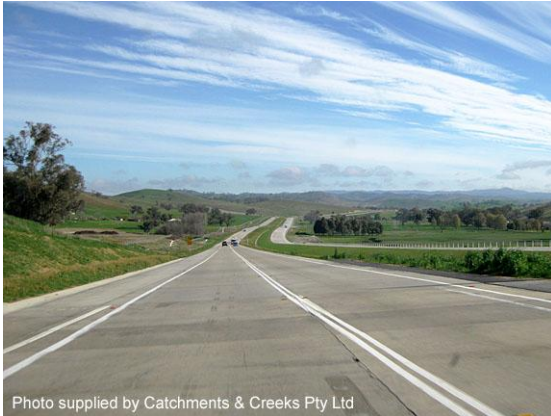
Major arterial roadway
