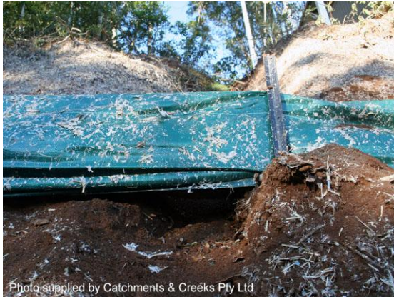
Storm undermines a sediment fence
