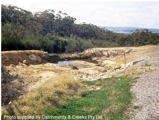
Type-2 sediment trap (1994)
