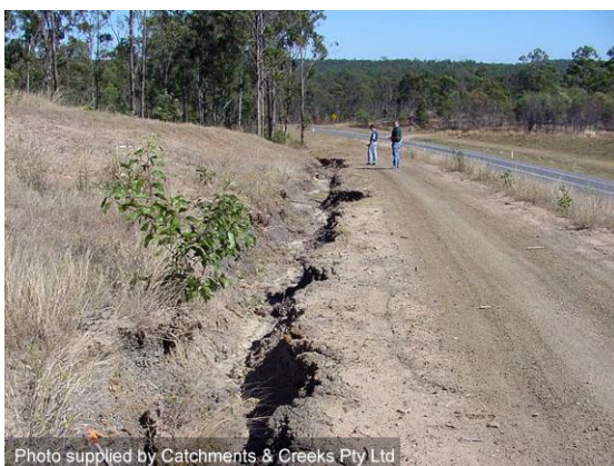
Bench cut into a dispersive soil
