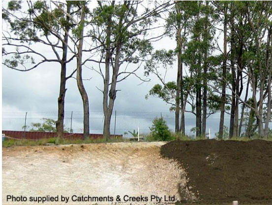
Topsoil placement
