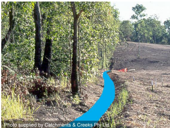
Catch drain used to divert run-on water
