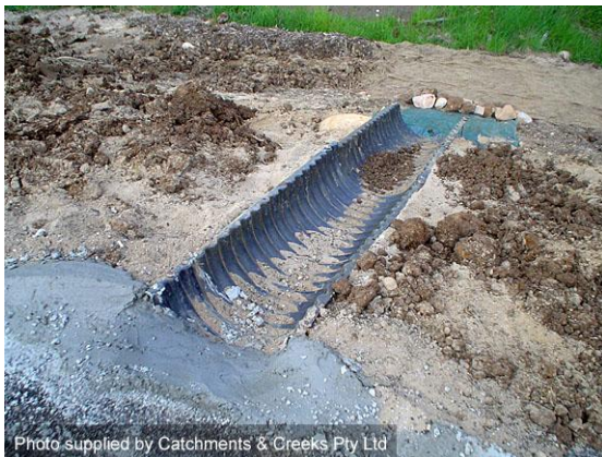
Temporary half-pipe batter chute
