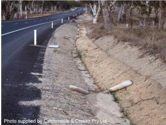
Sandbag check dams
