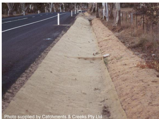
Fine jute mat over seeded soil
