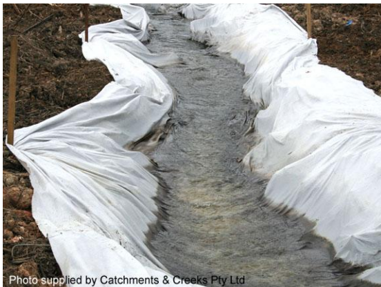
Filter cloth anchored with timber stakes
