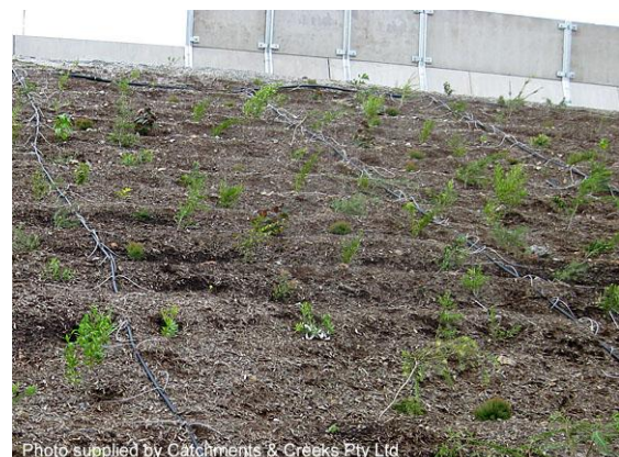
Revegetated stair-stepped batter
