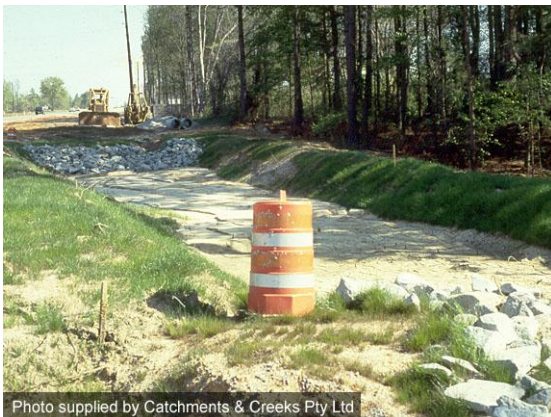
Rock filter dam
