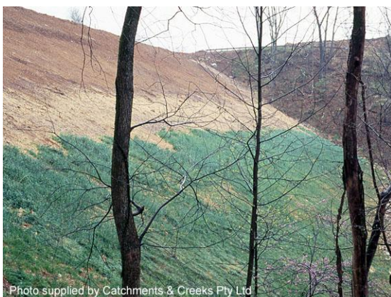
Progressive batter revegetation
