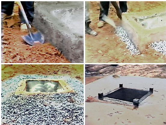
Excavated drop inlet protection
