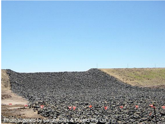
Spillway with well-defined weir profile
