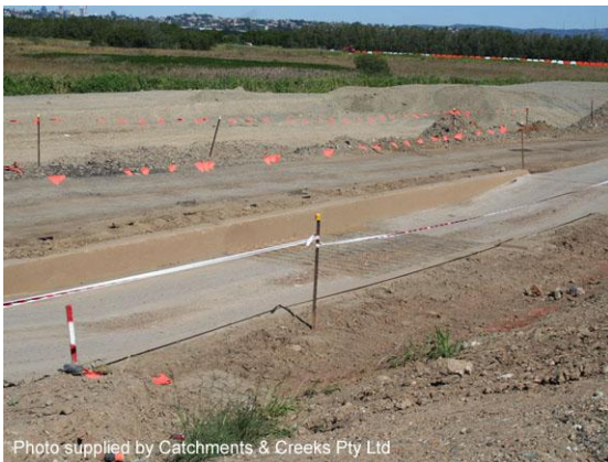
Drained wash bay (vibration grid)
