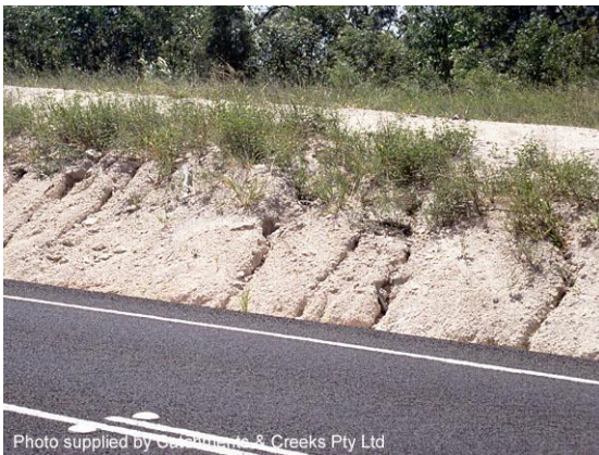
Rill erosion on a cut batter
