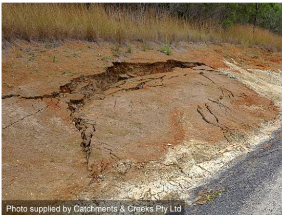
Bank slumping on a cut batter
