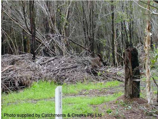
Brushwood barrier sediment trap
