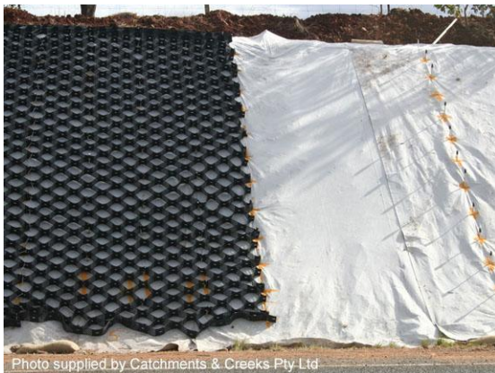
Installation on road batter
