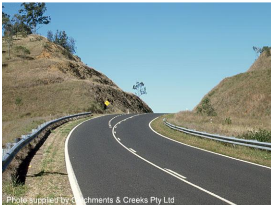
Benched road batters
