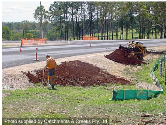
Replacement of topsoil
