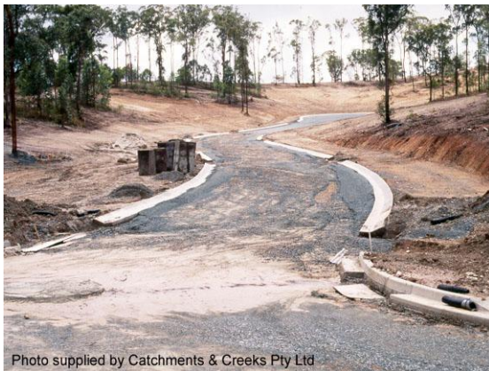
Storm damage to pavement road base
