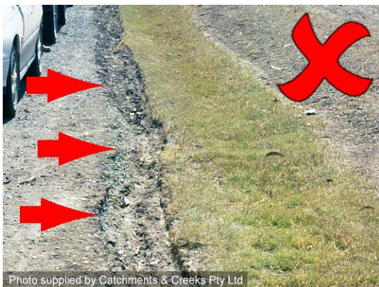
Rilling along the edge of turf
