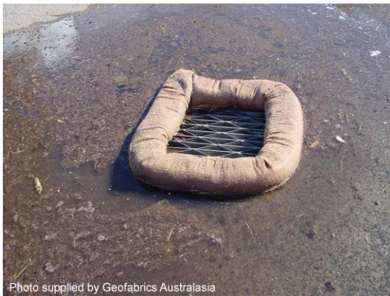
Filter sock drop inlet protection
