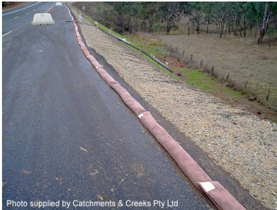
Temporary flow diversion berm
