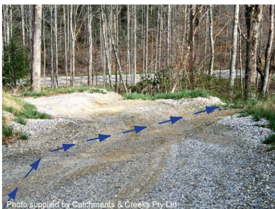
Cross bank drainage
