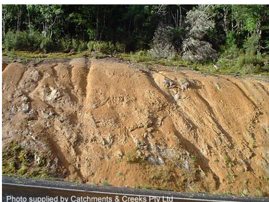
Rilling that extends to top of bank
