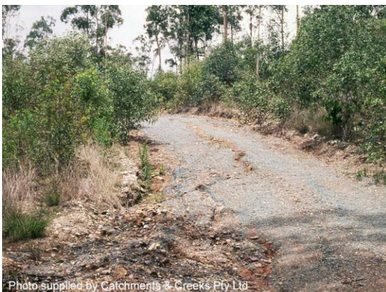
Damage to construction access road
