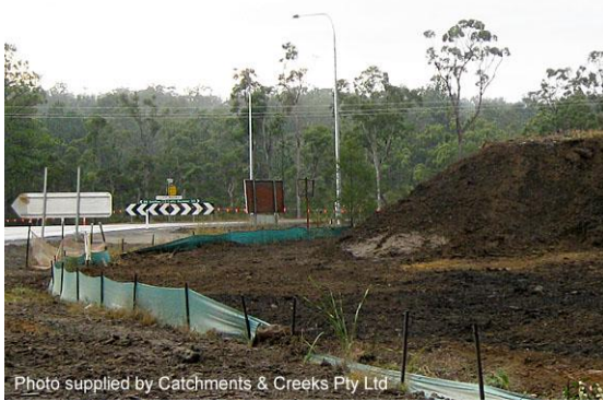
Stockpile placed up-slope of road works
