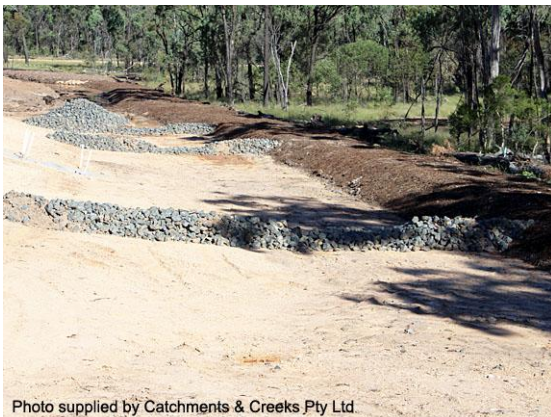
Velocity control check dams
