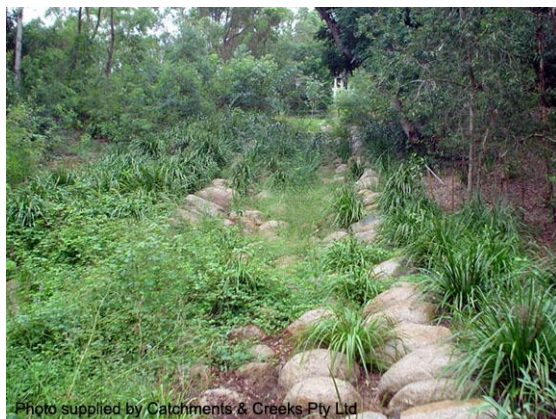
Vegetated rock-lined batter chute
