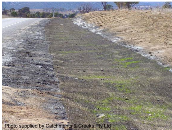
Jute mesh with bitumen seal
