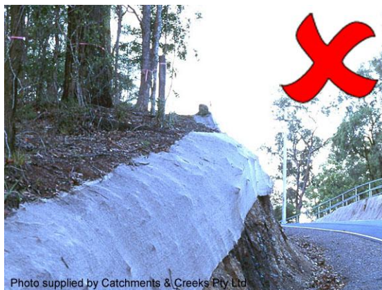
Blanket stretched over irregular ground
