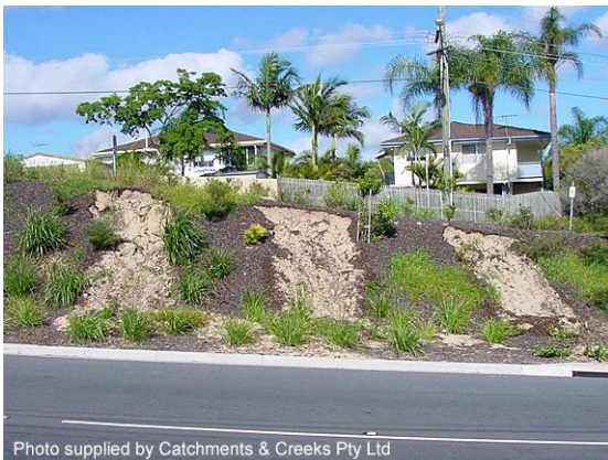
Storm damage to road batter
