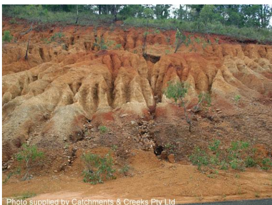
Erosion of an exposed dispersive soil
