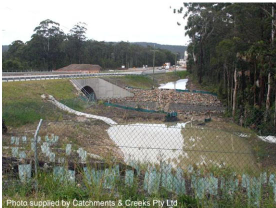
Basins retained for stormwater treatment
