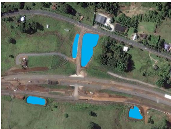
Sediment basins on road construction
