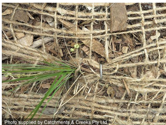
Jute mesh anchoring loose mulch
