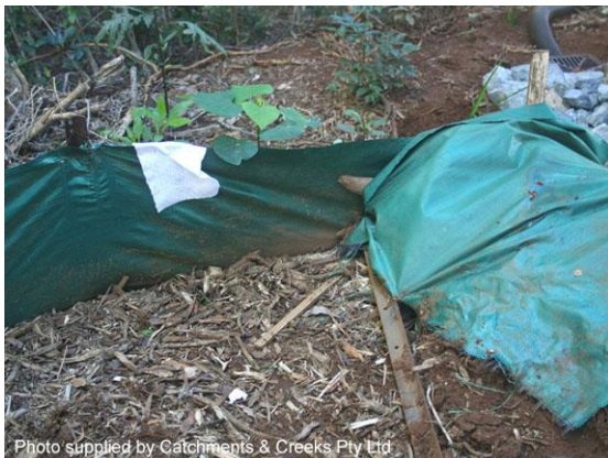
Damaged fence tagged for repair
