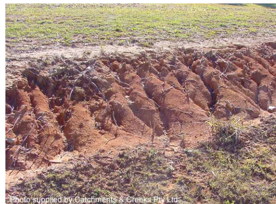
Fluting of the exposed dispersive soil
