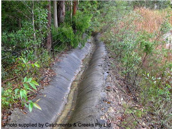
Permanent catch drain
