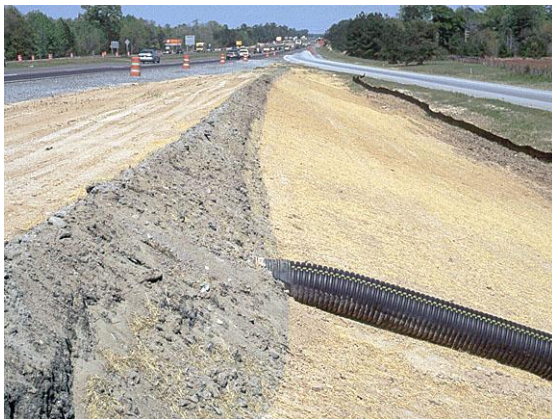
Topsoil flow diversion bank
