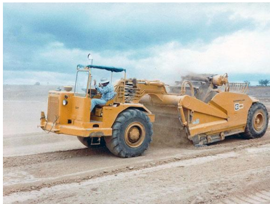
Topsoil stripping
