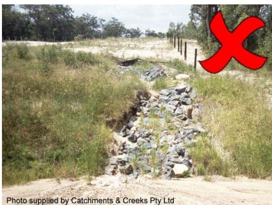
Batter chute placed on a dispersive soil
