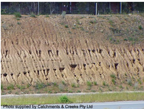
A form of rilling known as 'fluting'
