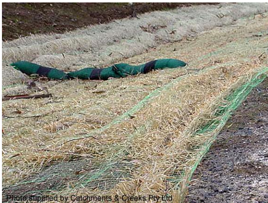
Temporary erosion control mat
