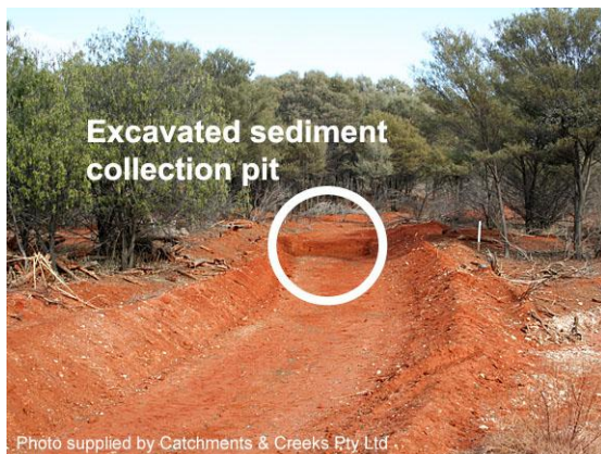
Excavated sediment sump
