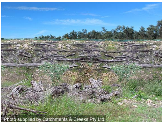
Woody debris placed along a fill batter
