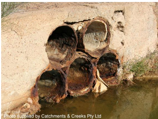
Culvert damaged by acidic water
