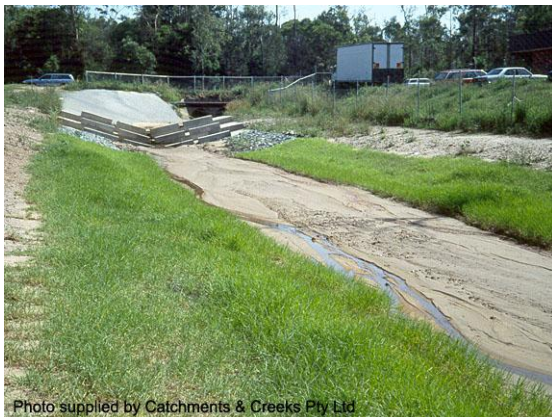
Deposition of sediment in a storm drain
