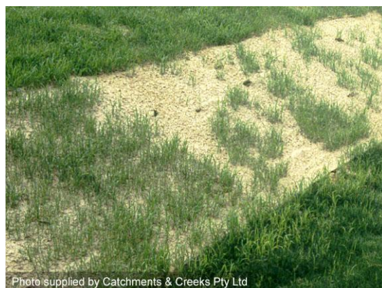
Grass establishing on a thick blanket
