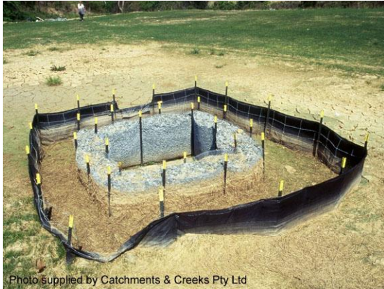
Sediment weir (field inlet protection)
