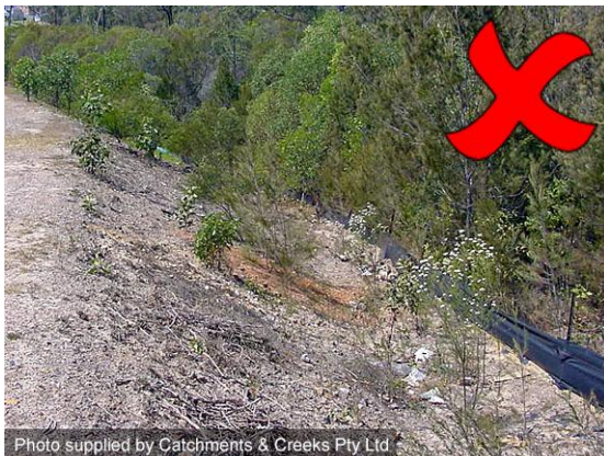
Poor veg growth on heavily-compacted soil
