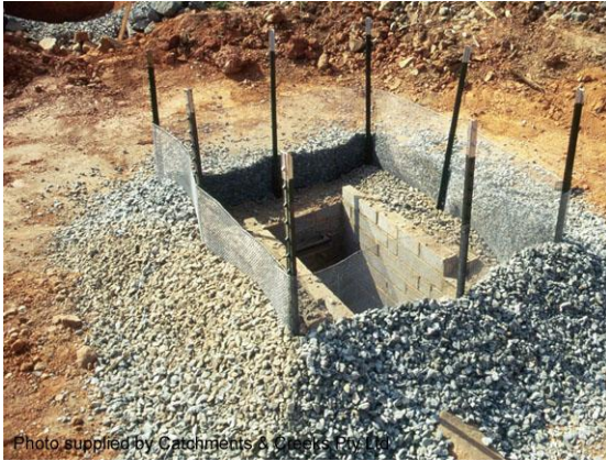
Mesh & aggregate drop inlet protection
