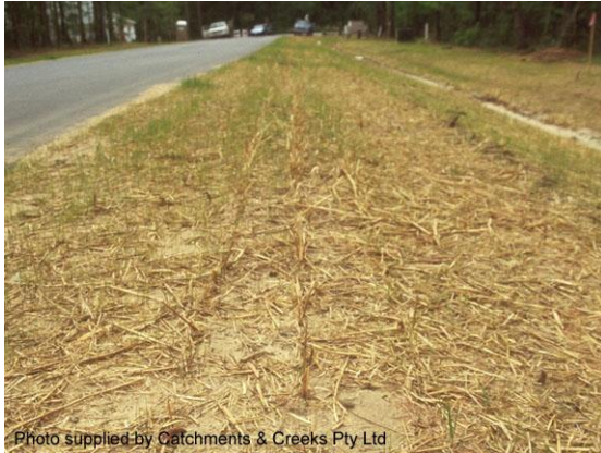
Straw mulching of road shoulder
