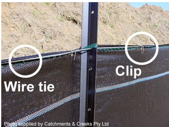
Sediment fence with top wire
