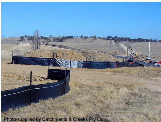
Sediment control down-slope of stockpile
