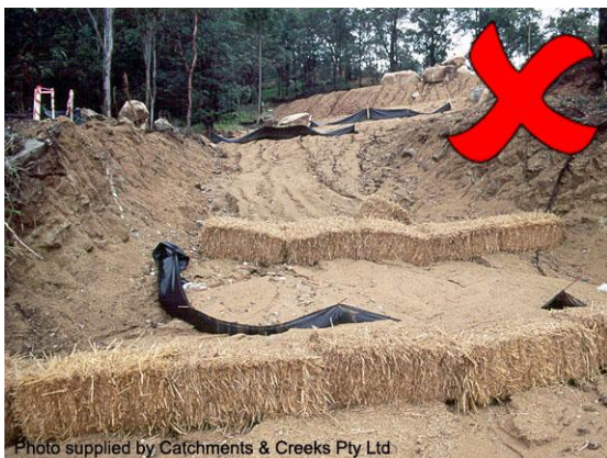
Sediment traps placed on site access
