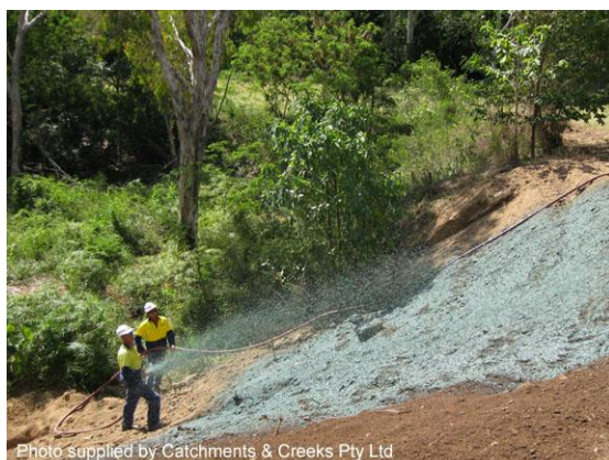
Bonded fibre matrix
