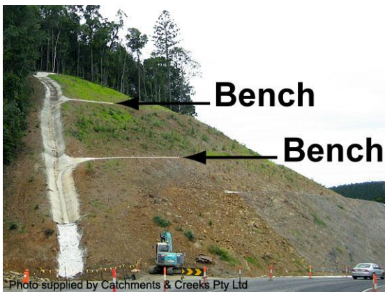
Benched cut batter
