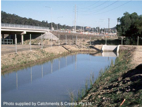
Stormwater treatment pond
