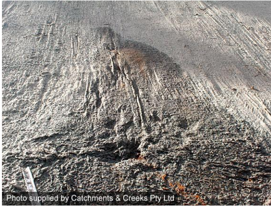
Spring water visible on jute blanket
