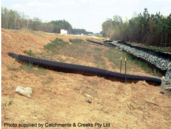
Temporary and permanent road drainage
