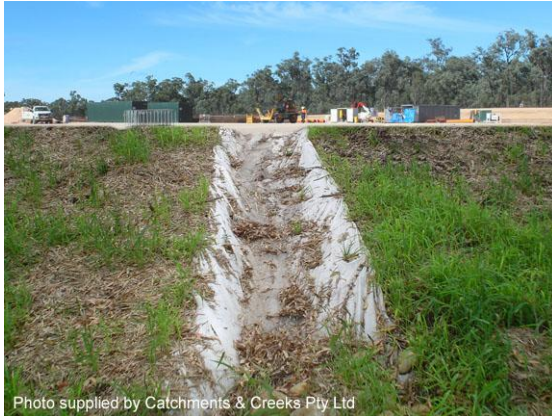
Filter cloth lined batter chute
