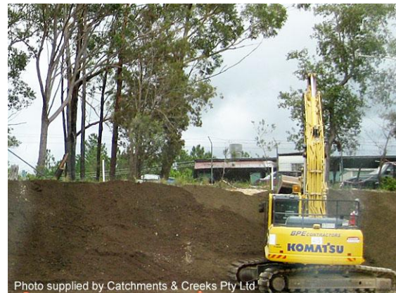
Placement of topsoil
