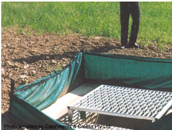
Fabric drop inlet protection
