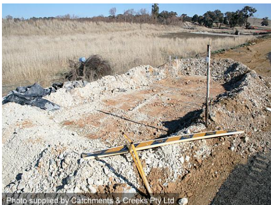
Concrete truck wash-out point
