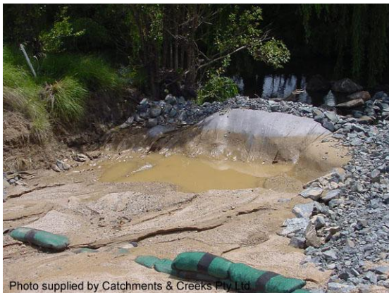
Rock filter dam – geotextile filter
