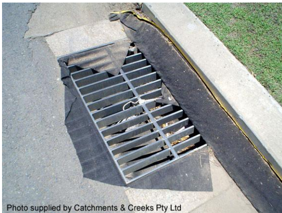
Gully bag sediment trap
