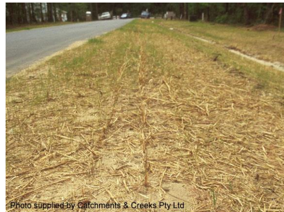
Crimped straw mulch
