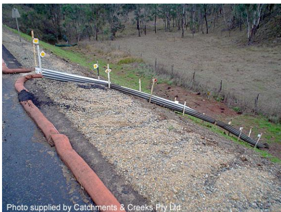
Corrugated iron batter chute
