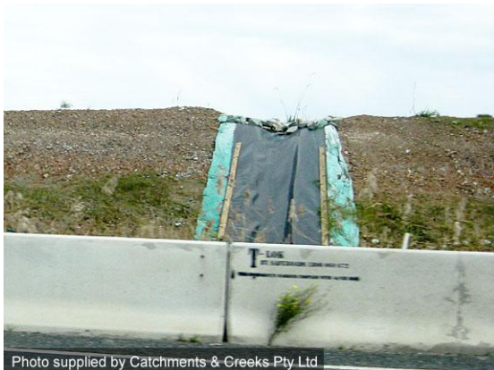
Temporary batter chute
