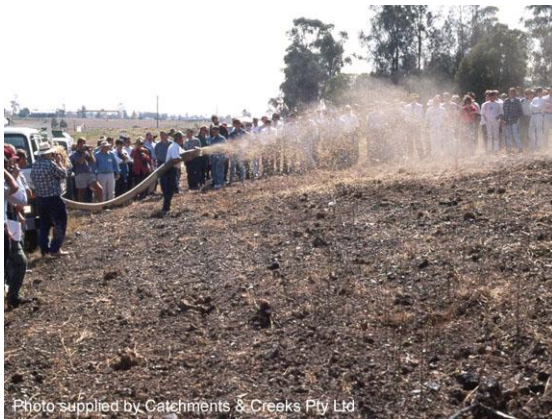
Straw mulching of a road batter
