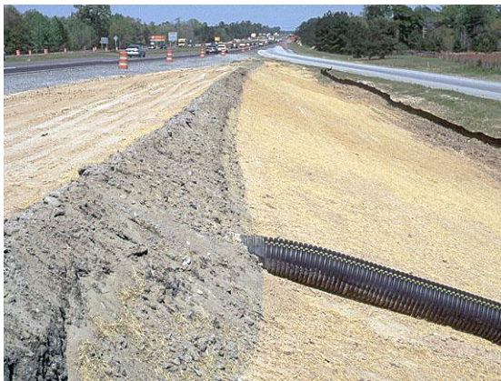
Flow control berm at pipe inlet
