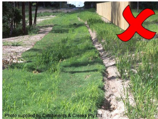
Rilling along the edge of turf
