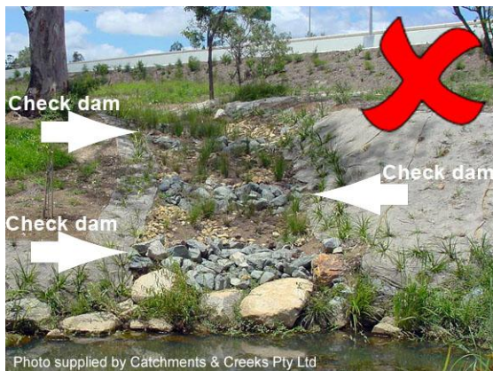
Check dams placed on a batter chute
