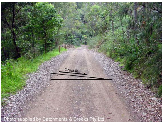
Dirt road with in-fall drainage
