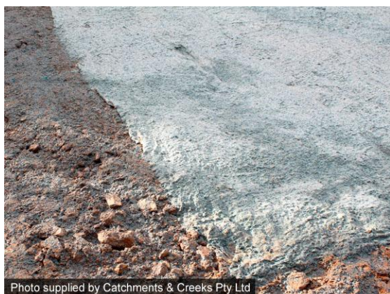
Thick blanket seeded with BFM
