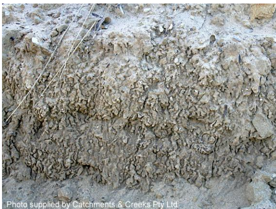
Bank not exposed to direct rainfall
