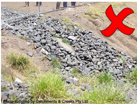
Rocks slipping down batter chute
