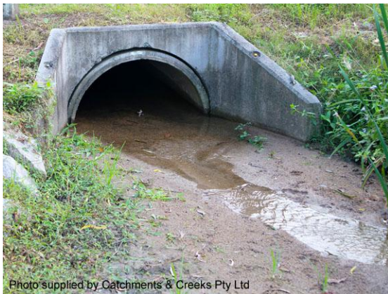
Sedimentation of drainage pipe
