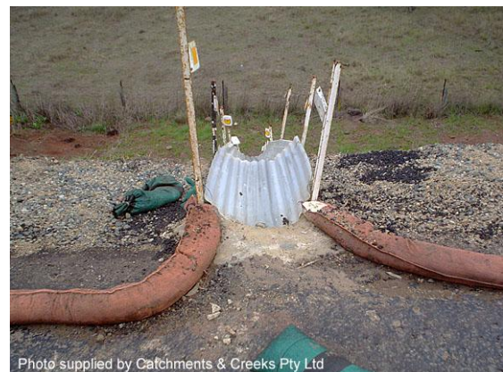
Concrete water seal at chute inlet
