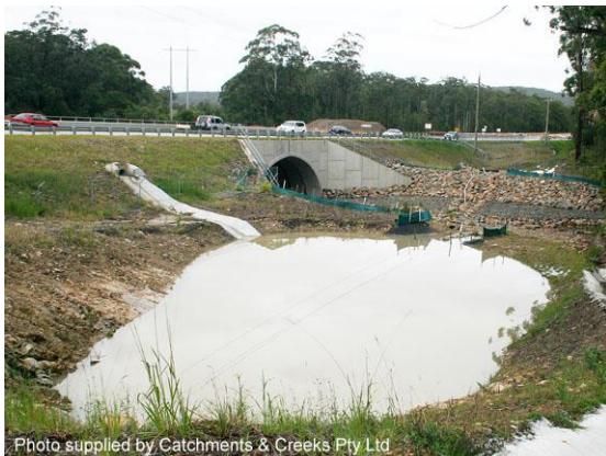
Stormwater treatment pond (2009)
