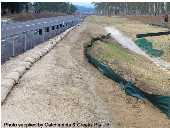
Sandbags used to divert road runoff
