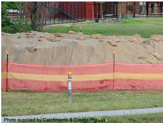
Long-term stockpile covered with jute
