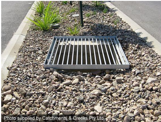
Field inlet located within median strip
