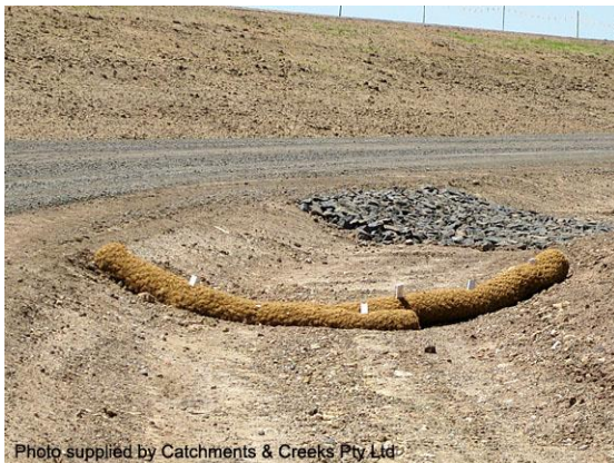
Geo-log check dam
