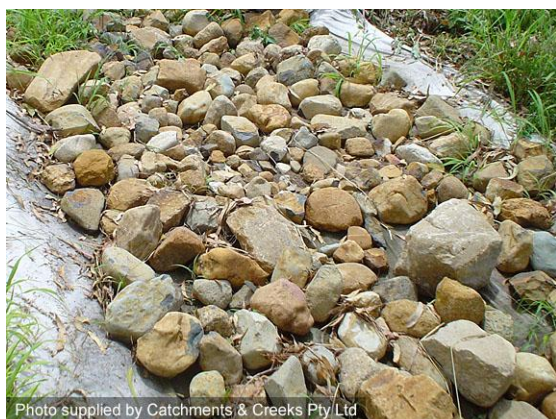
Rock-lined drainage channel
