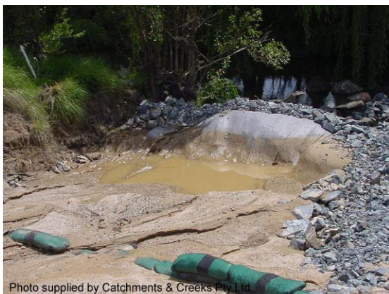
Type-2 sediment trap
