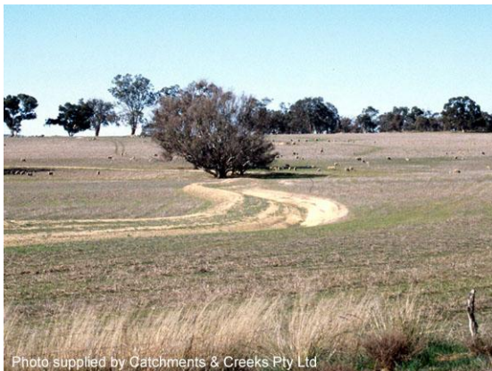
Flow diversion channel
