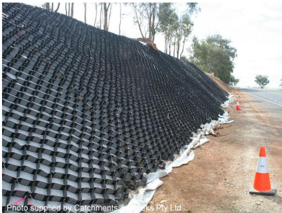
Installation on road batter
