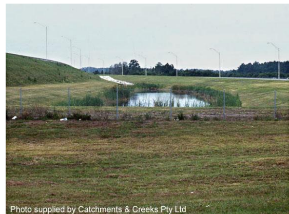
Stormwater treatment pond
