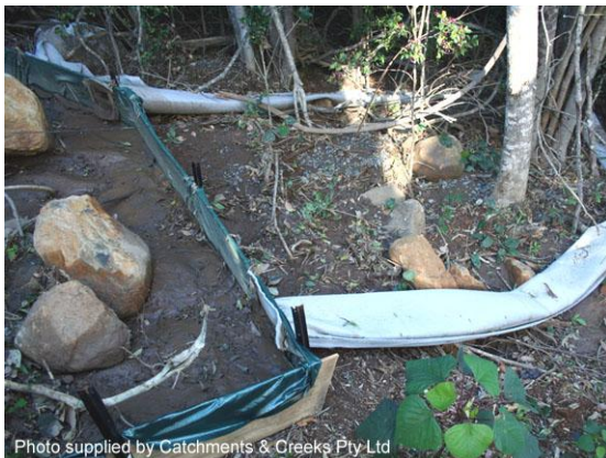
Filter tube dam sediment trap
