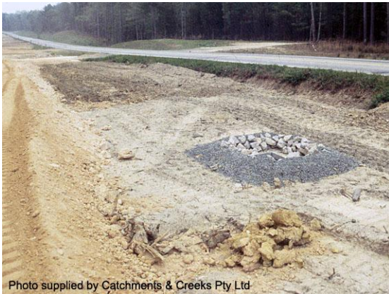
Rock & aggregate drop inlet protection
