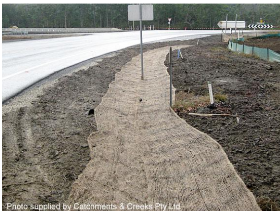
Jute mesh channel lining
