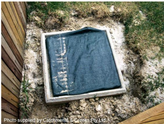
Fabric wrap inlet protection
