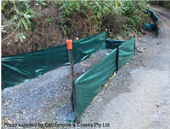
U-shaped sediment trap
