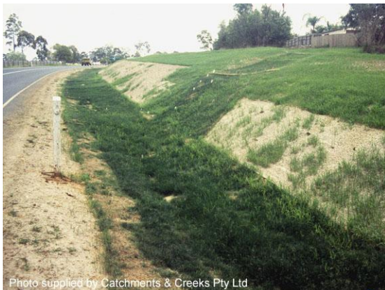
Jute blankets placed on dispersive soil
