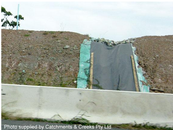
Temporary plastic sheet batter chute
