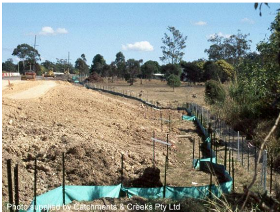
Placement of regular ‘returns’
