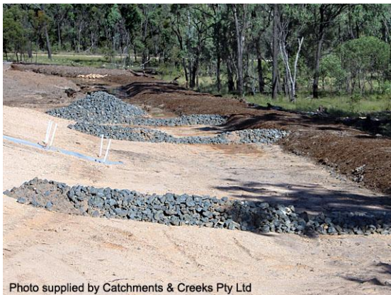
Velocity control check dams
