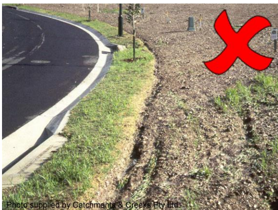
Rilling along the edge of turf
