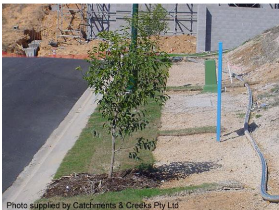
Placement of lateral turf strips
