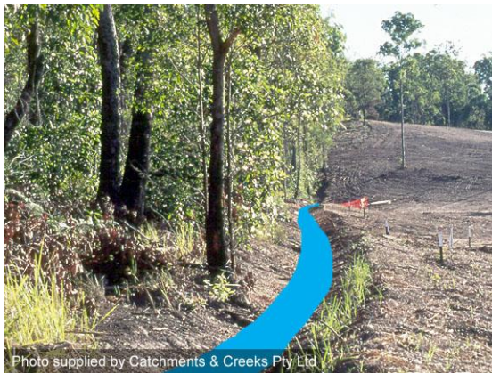
Flow diversion using a catch drain
