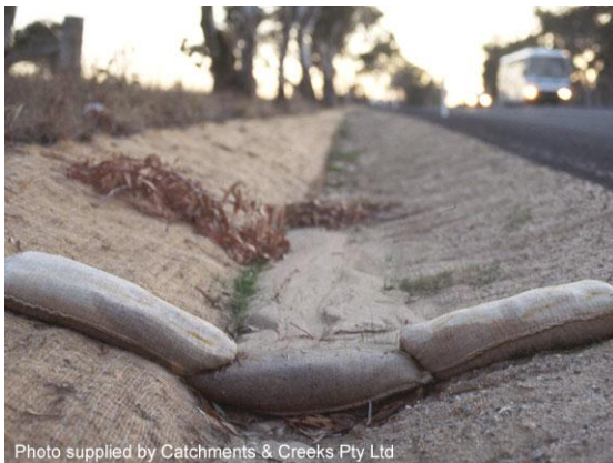
Sandbag check dam
