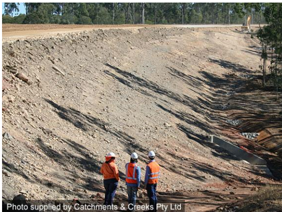
Road batter awaiting stabilisation
