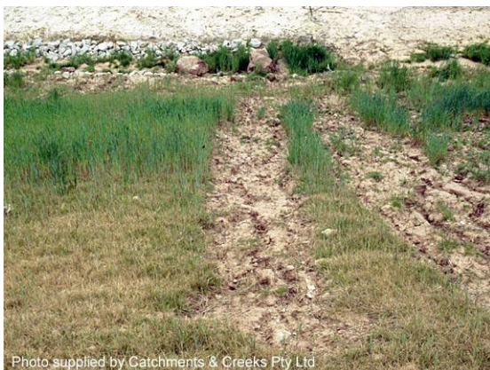
Rill erosion on newly formed fill batter
