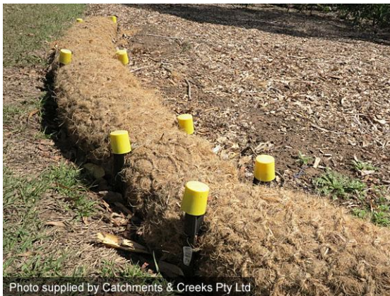
Geo log flow diversion
