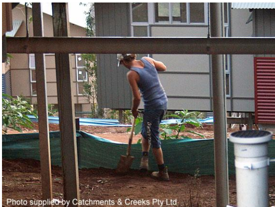
Maintenance of control measures
