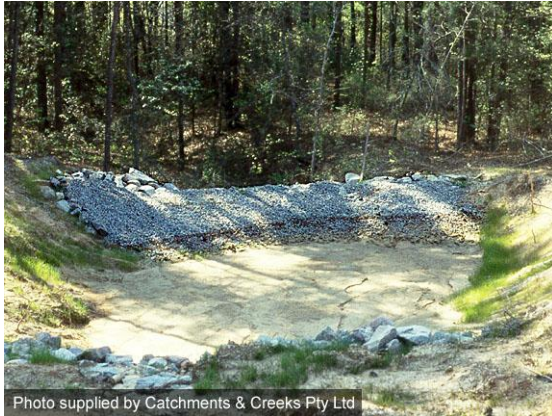
Rock filter dam – aggregate filter
