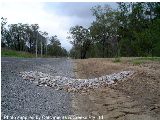
Rock check dam
