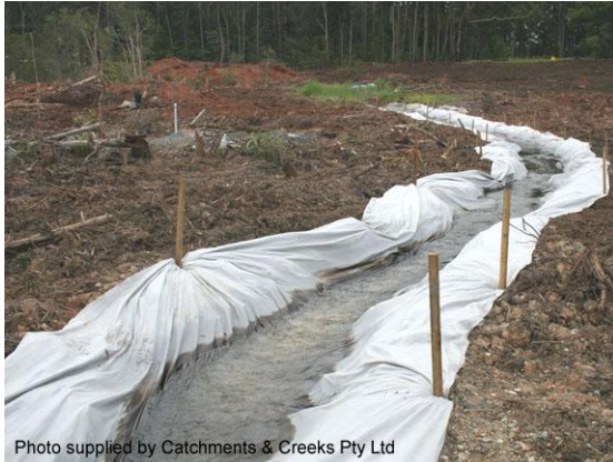
Clean water flow diversion
