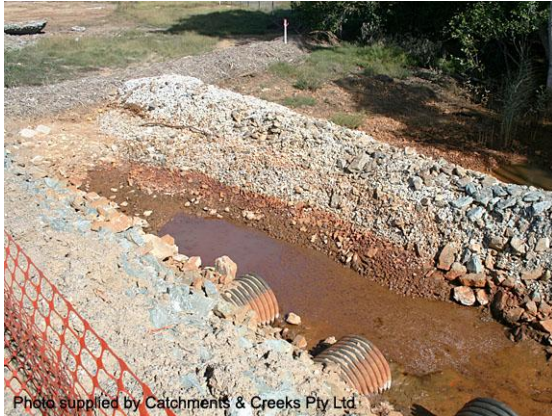
Rock filter dam with aggregate filter
