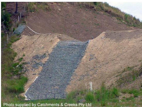
Mattress-lined sediment basin spillway
