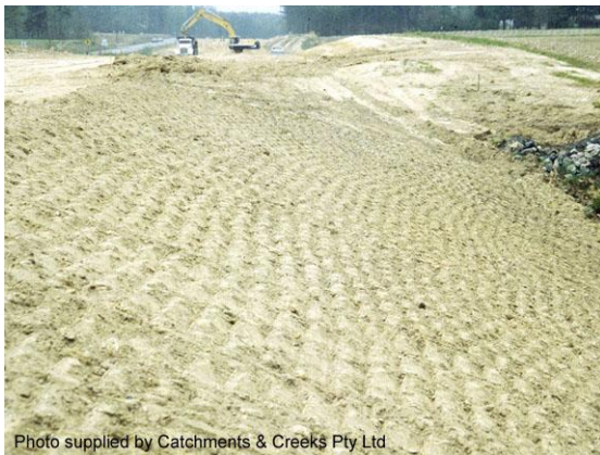
Roughened earth batter
