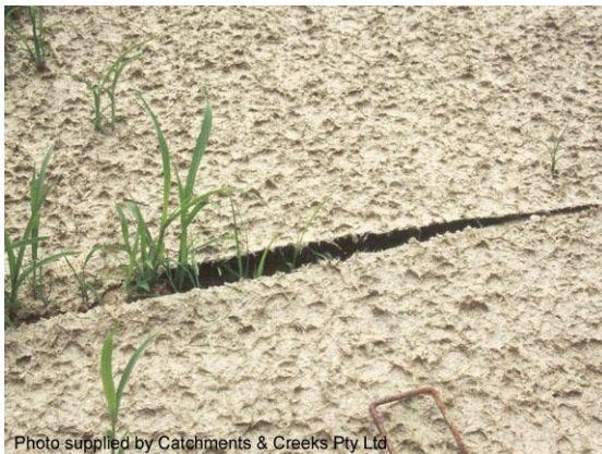
Soil erosion occurring under blanket
