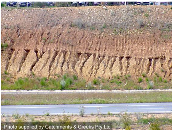
Rilling limited to a given soil horizon
