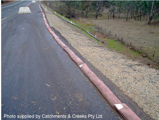
Filter sock flow diversion berm
