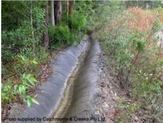
Permanent catch drain
