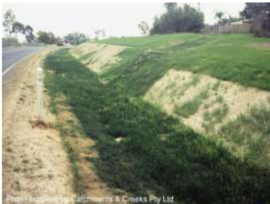
Jute blankets placed on dispersive soil
