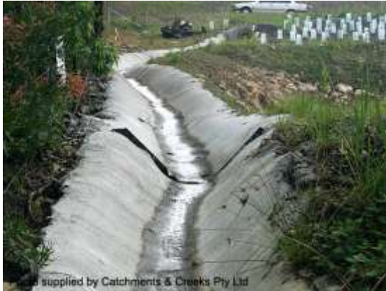
Concrete-lined catch drain
