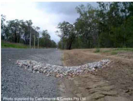
Rock check dam
