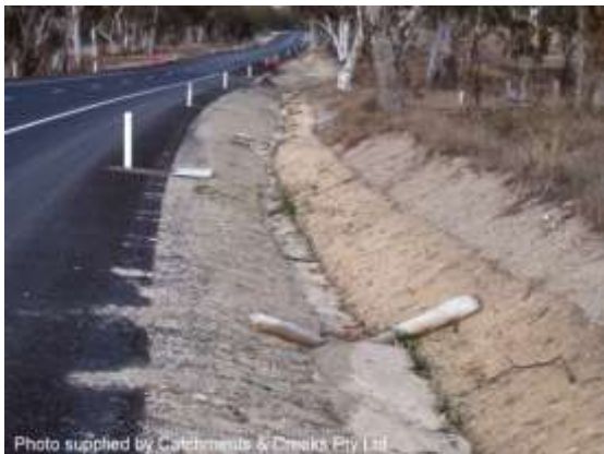
Sandbag check dams
