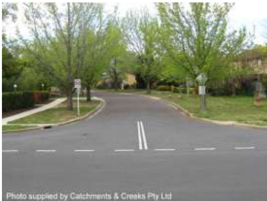
Sealed urban road
