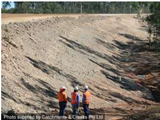
Road batter awaiting stabilisation
