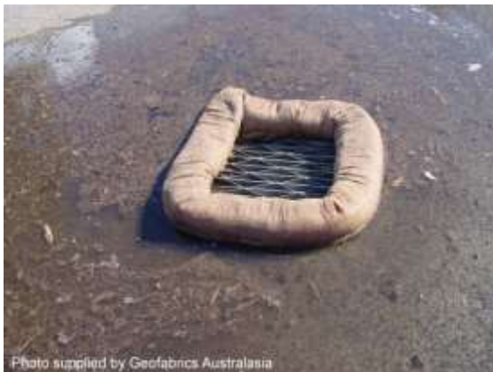
Filter sock drop inlet protection
