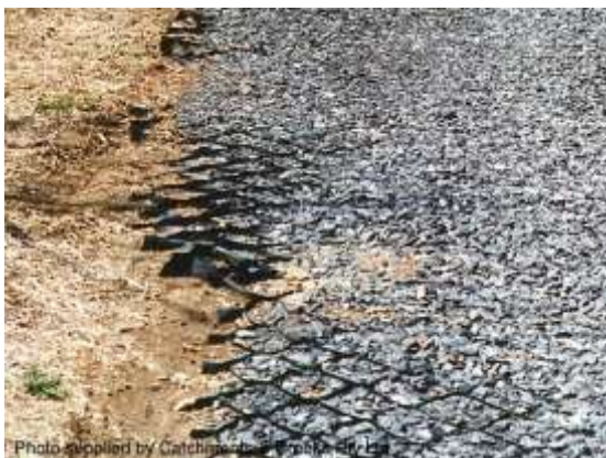
Gravelled car park
