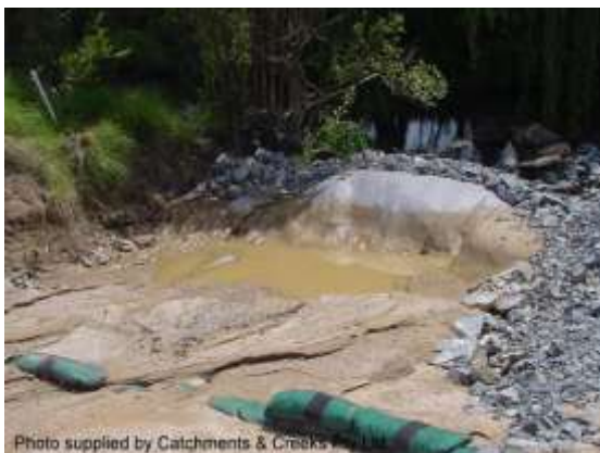
Type-2 sediment trap
