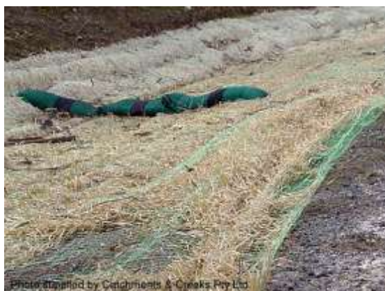
Non UV-stabilised synthetic composite mat
