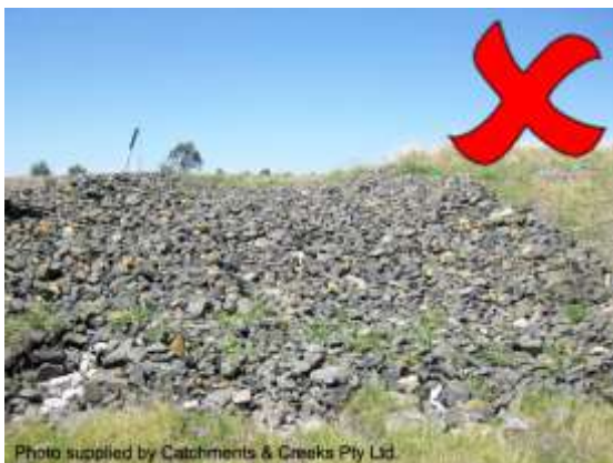
Inadequate rock size
