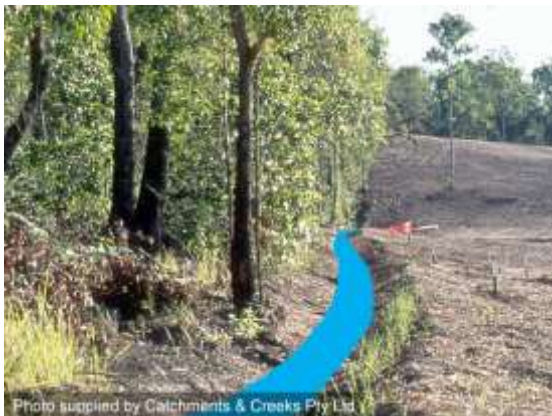
Catch drain used to divert run-on water
