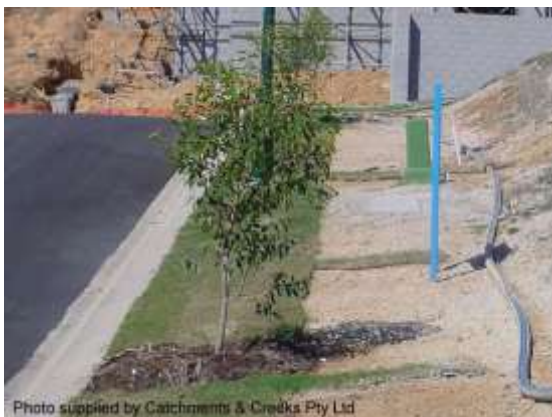
Placement of lateral turf strips
