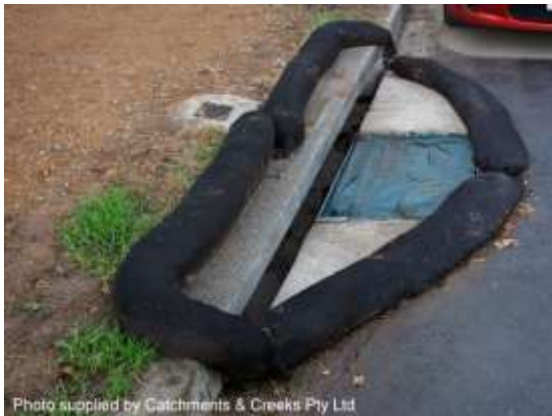
Kerb inlet protection (supplementary)
