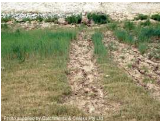
Rill erosion on newly formed fill batter
