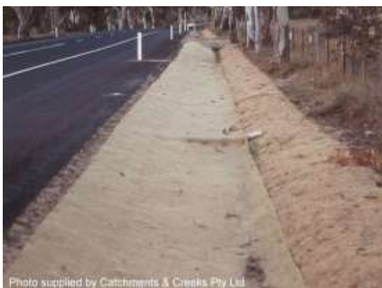
Jute erosion control mat
