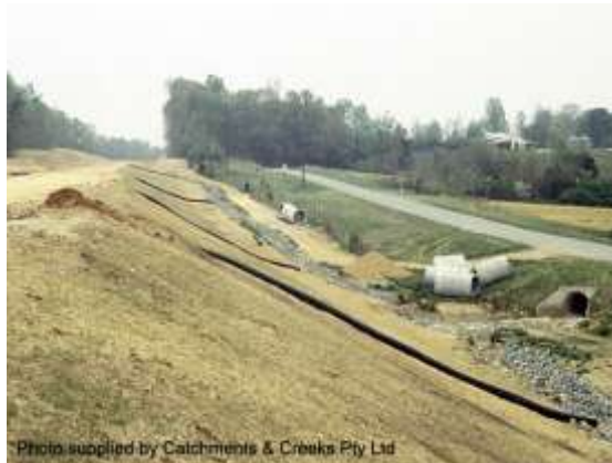
Slope drains
