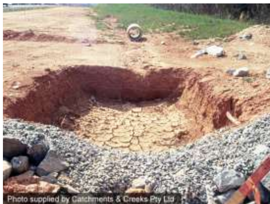
Excavated sediment sump
