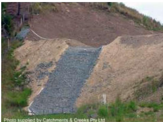
Mattress-lined sediment basin spillway
