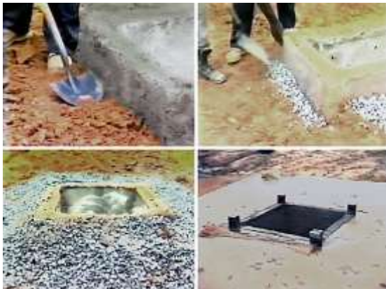
Excavated drop inlet protection
