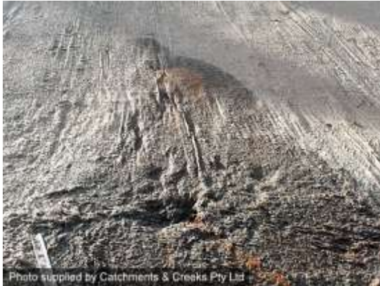
Spring water visible on jute blanket
