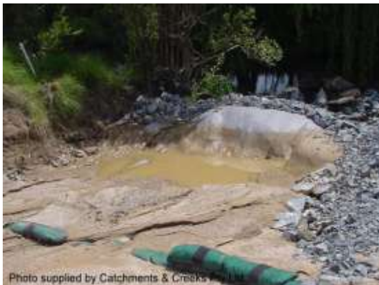
Rock filter dam – geotextile filter
