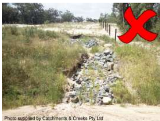
Batter chute placed on a dispersive soil
