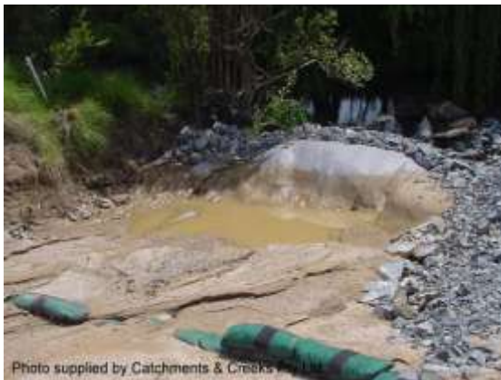
Rock filter dam (Type-2)
