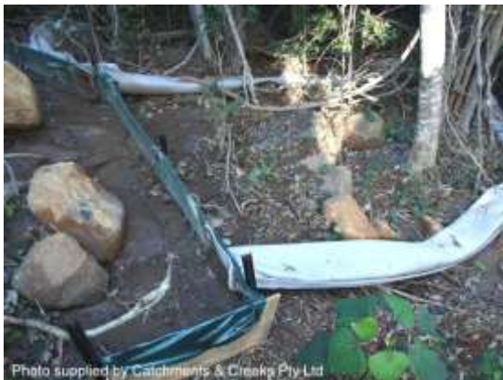
Filter tube dam sediment trap
