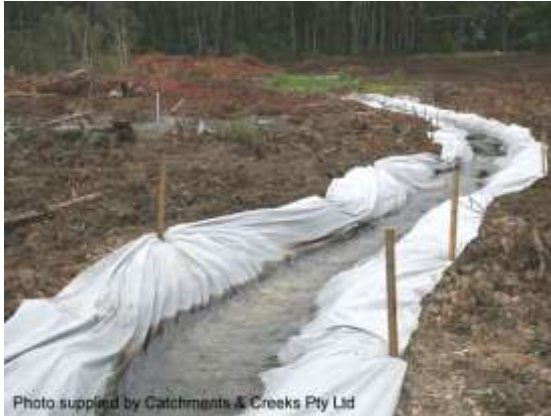
Clean water flow diversion
