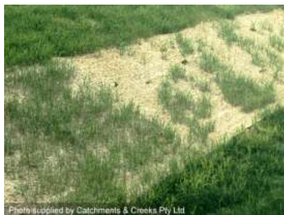
Grass establishing on a thick blanket
