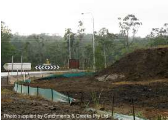
Stockpile placed up-slope of road works
