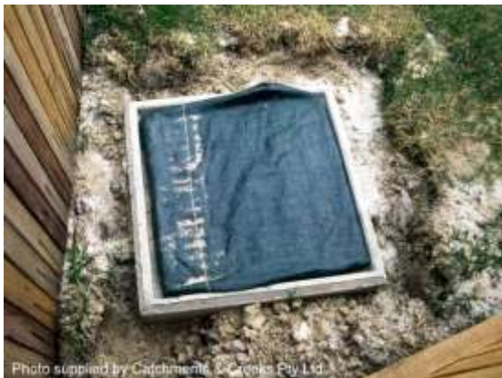
Fabric wrap inlet protection
