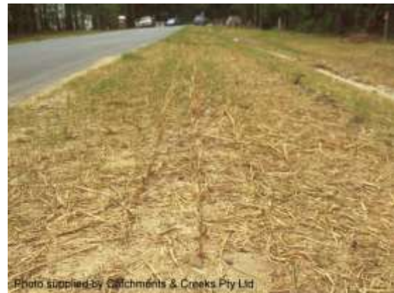
Crimped straw mulch
