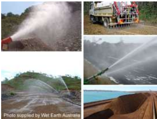
Application of soil binders
