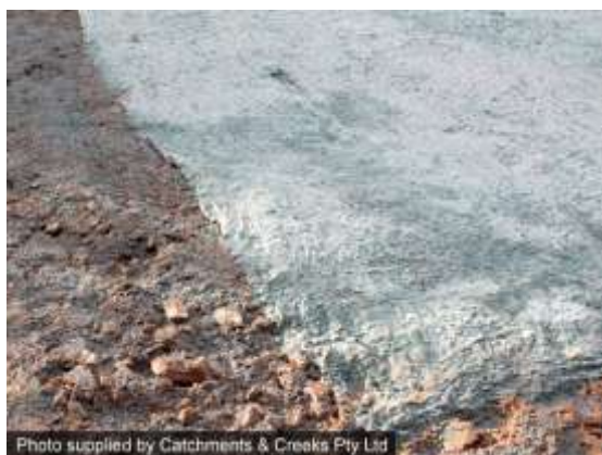
Thick blanket seeded with BFM
