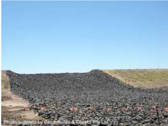
Spillway with well-defined weir profile
