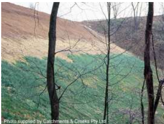
Progressive batter revegetation
