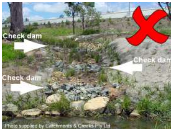
Check dams placed on a batter chute
