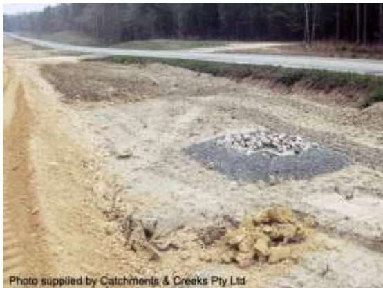
Rock & aggregate drop inlet protection
