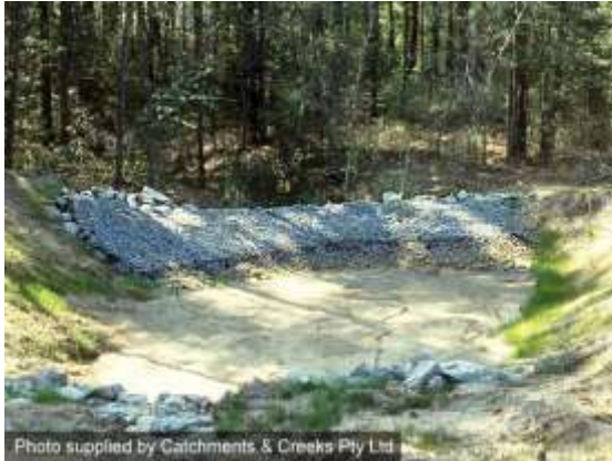
Rock filter dam – aggregate filter
