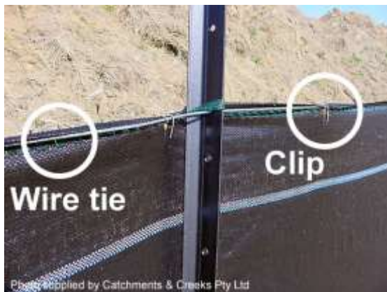
Sediment fence with top wire
