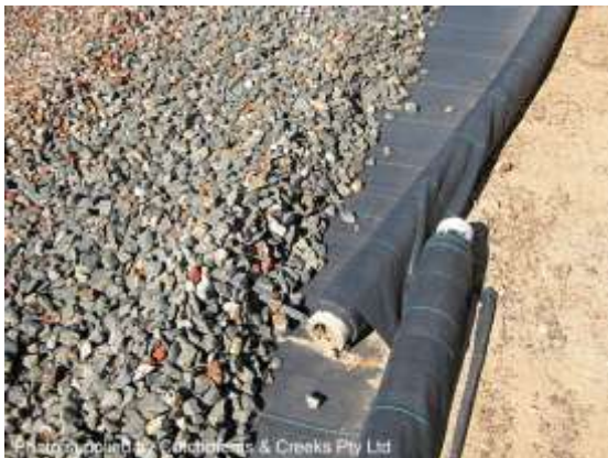
Placement of gravel over geotextile
