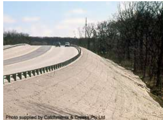
Erosion control blankets
