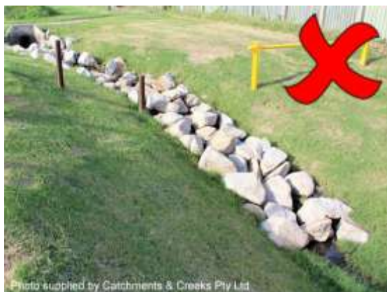
Newly established rock chute
