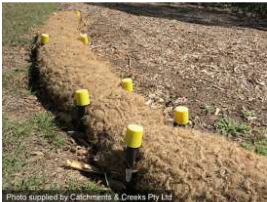
Geo log flow diversion
