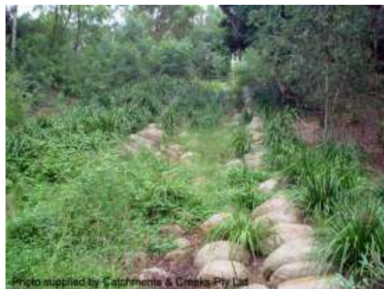
Vegetated rock-lined batter chute
