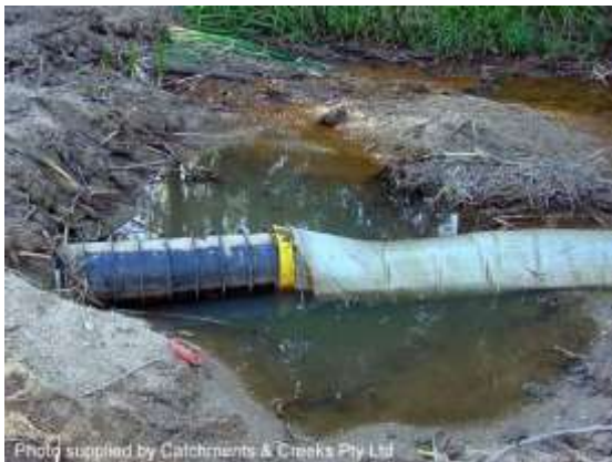
Filter tube attached to an embankment
