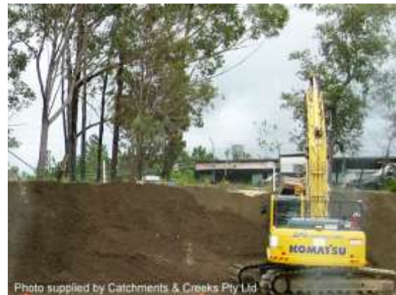
Placement of topsoil
