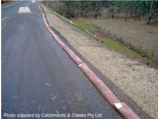
Filter sock flow diversion berm
