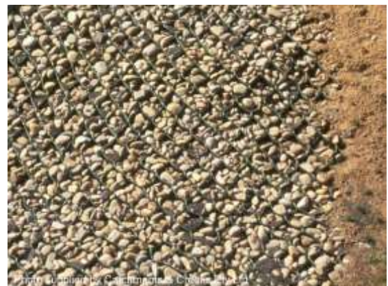
Gravelled batter slope
