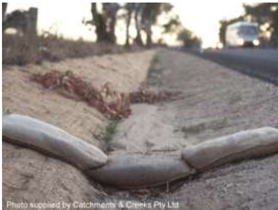
Sandbag check dam
