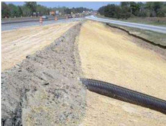
Topsoil flow diversion bank
