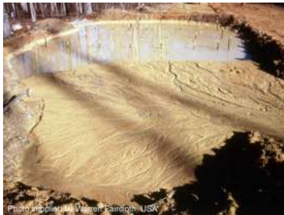
Sediment retained in a basin
