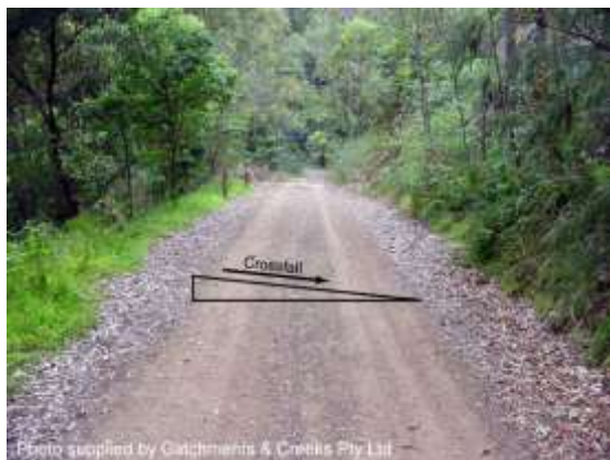
Dirt road with in-fall drainage
