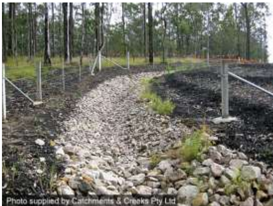
Rock-lined catch drain
