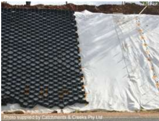
Installation on road batter
