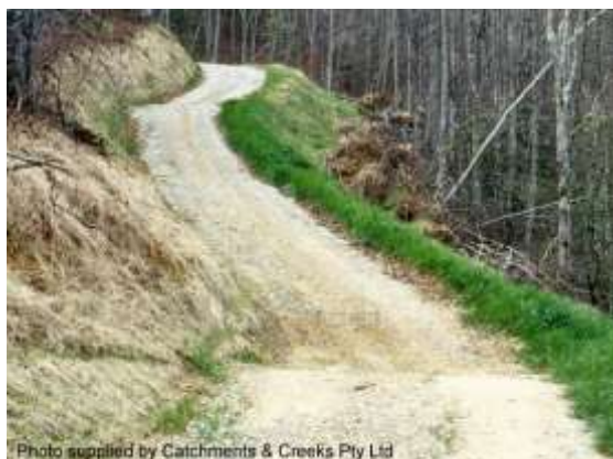
Permanent maintenance access road
