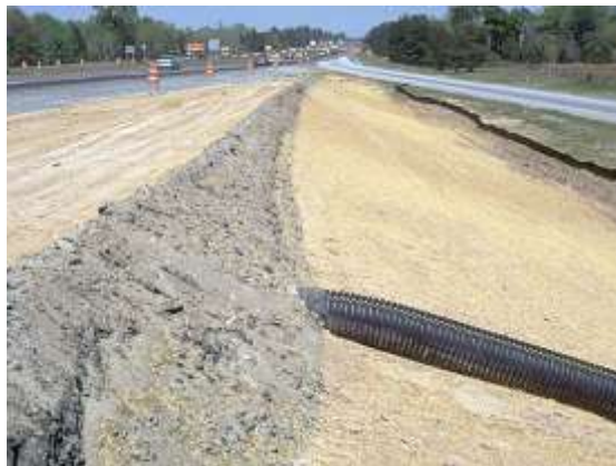
Flow control berm at pipe inlet
