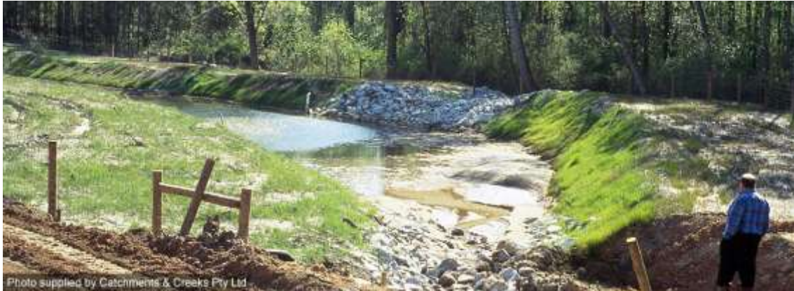
US example of a major Type-2 sediment trap with rock filter dam outlet system (1995)
