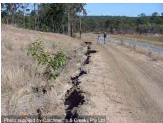
Bench cut into a dispersive soil
