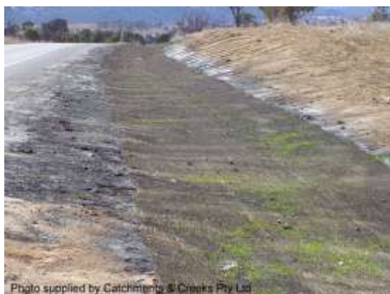
Jute mesh with bitumen seal
