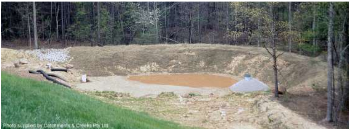
Type-C sediment basin with riser pipe outlet (1995)
