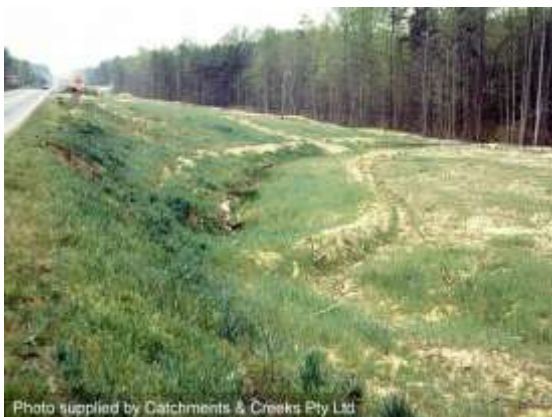
Full vegetation clearing
