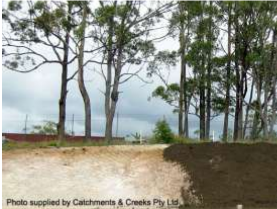
Topsoil placement
