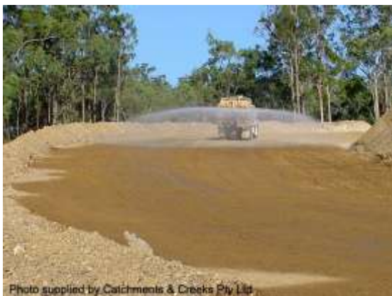
Water truck used for dust control
