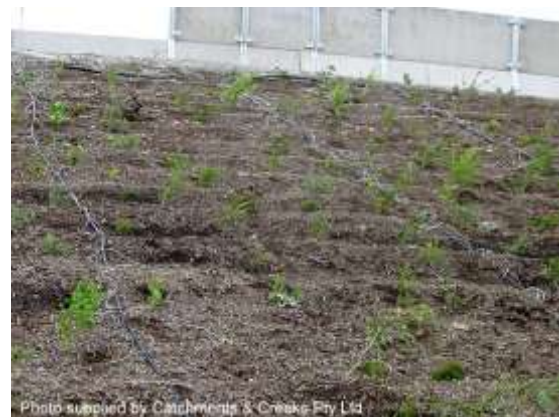
Revegetated stair-stepped batter
