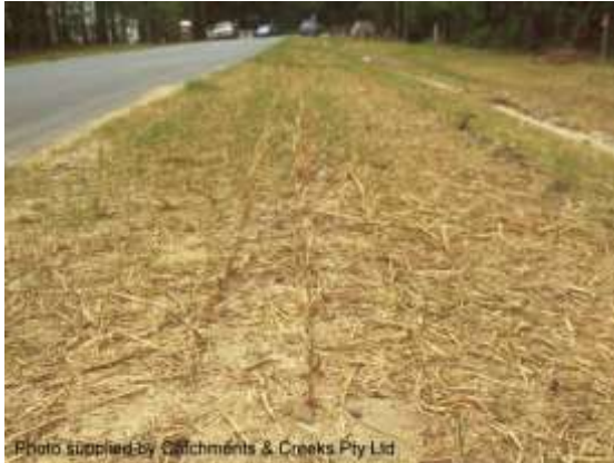
Straw mulching of road shoulder
