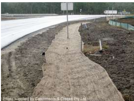
Jute mesh channel lining
