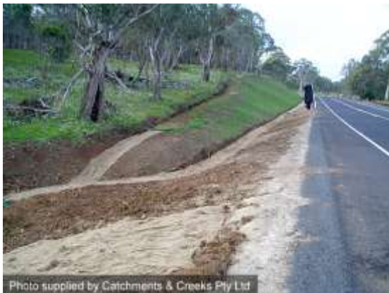
Flow diversion drains
