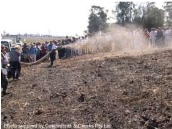
Straw mulching of a road batter
