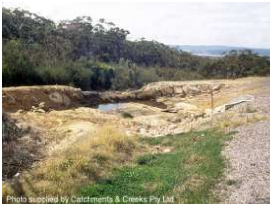
Type-2 sediment trap (1994)
