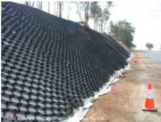
Installation on road batter
