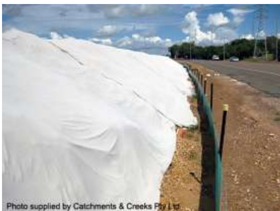
Covering of long-term soil stockpile
