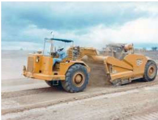
Topsoil stripping
