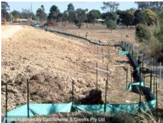
Sediment fence (Type-3)
