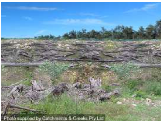
Woody debris placed along a fill batter
