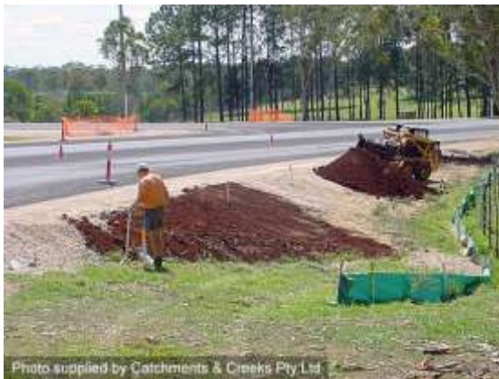
Replacement of topsoil
