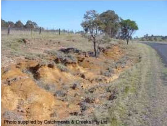
Erosion of a dispersive soil
