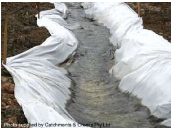
Filter cloth anchored with timber stakes
