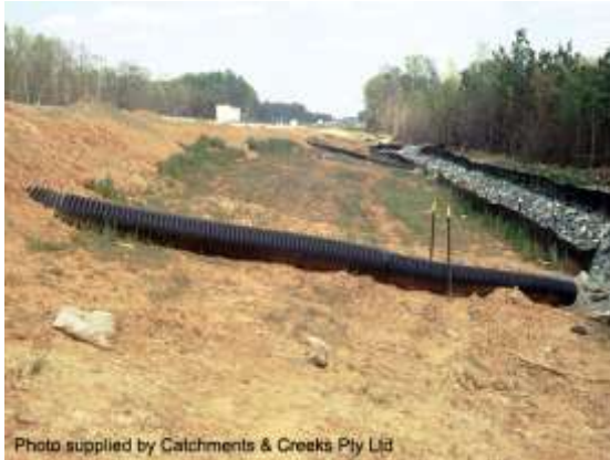
Temporary and permanent road drainage
