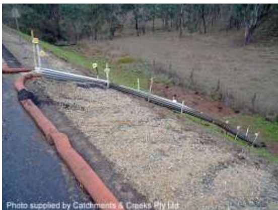
Corrugated iron batter chute
