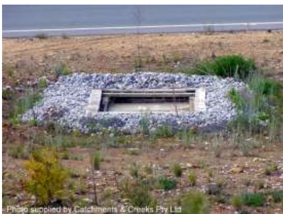
Block & aggregate drop inlet protection
