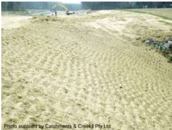
Roughened earth batter
