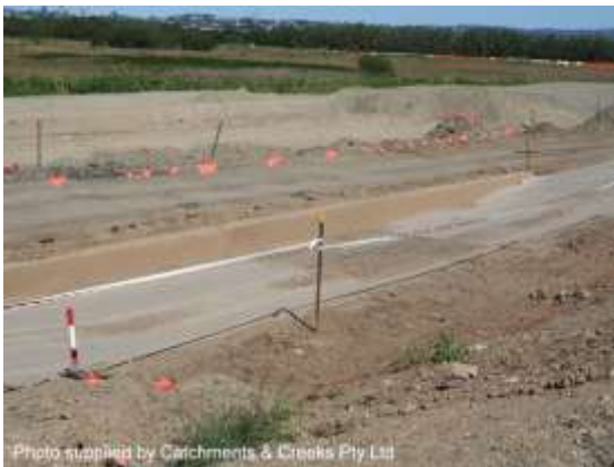
Drained wash bay (vibration grid)
