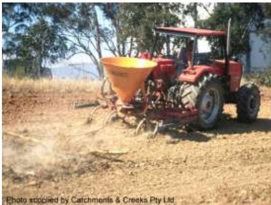
Seeding road batter
