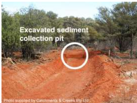
Excavated sediment sump
