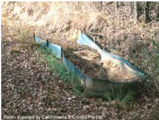
U-shaped sediment trap in steep drain
