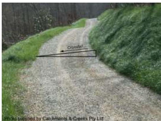
Gravel road with out-fall drainage
