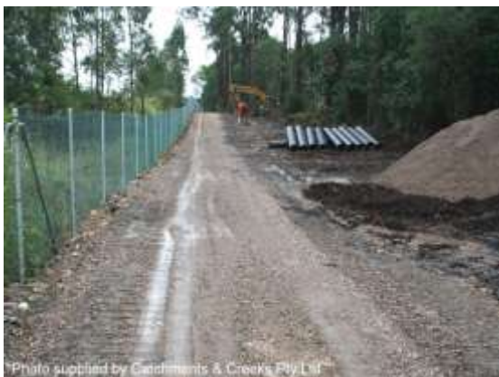
Unsealed construction access road
