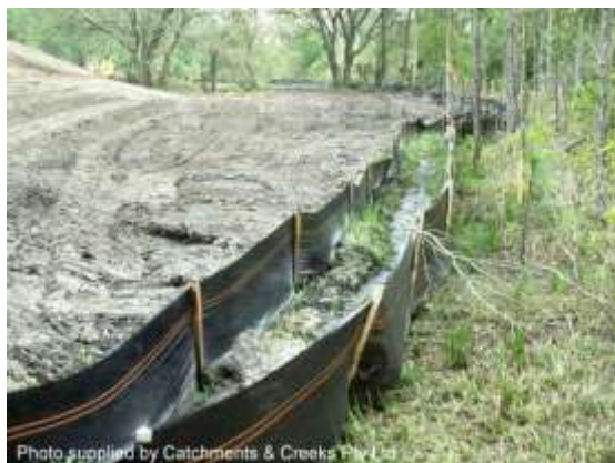
Double sediment fence
