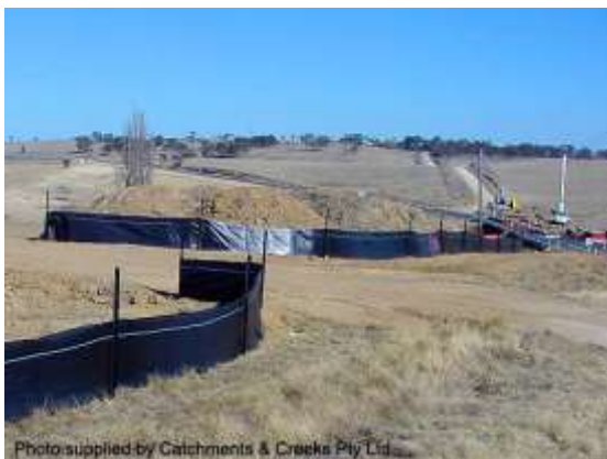
Sediment control down-slope of stockpile
