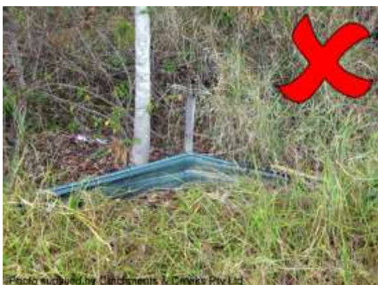
Sediment fence not removed after use
