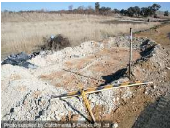
Concrete truck wash-out point
