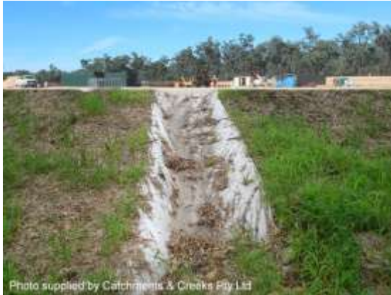
Filter cloth lined batter chute
