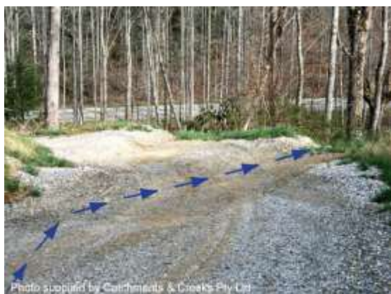
Cross bank drainage
