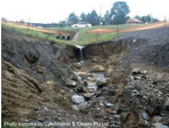
Gully erosion
