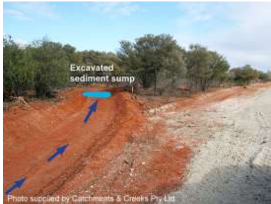
Excavated sediment sump
