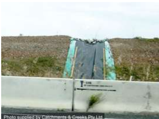
Temporary batter chute
