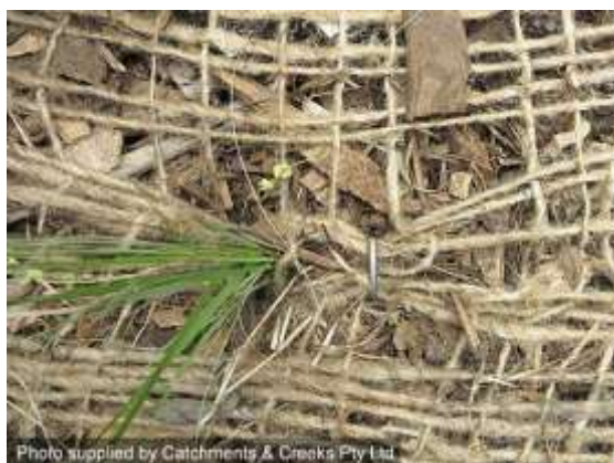
Jute mesh anchoring loose mulch
