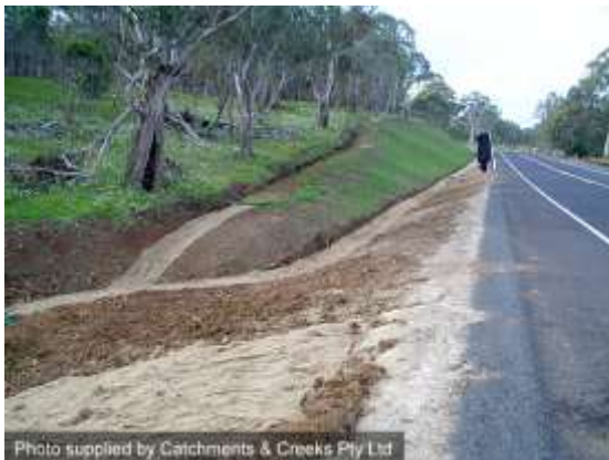
Catch drain and table drain
