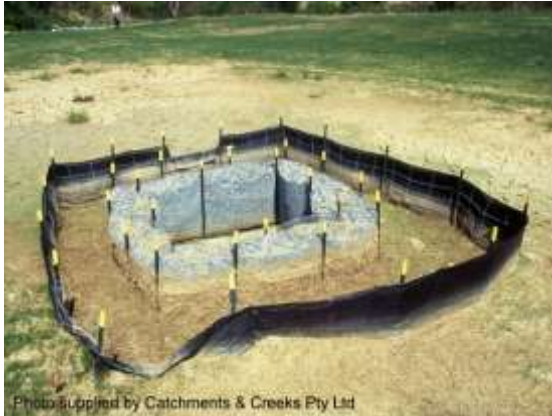
Sediment weir (field inlet protection)
