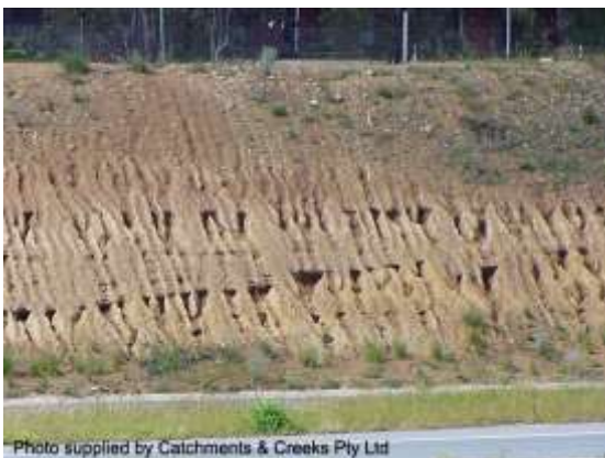
A form of rilling known as 'fluting'
