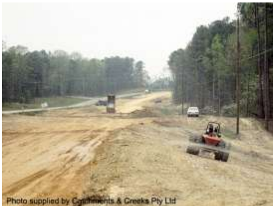
Amelioration of subsoils
