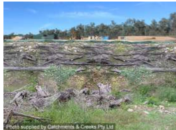
Brushwood used to stabilise a batter
