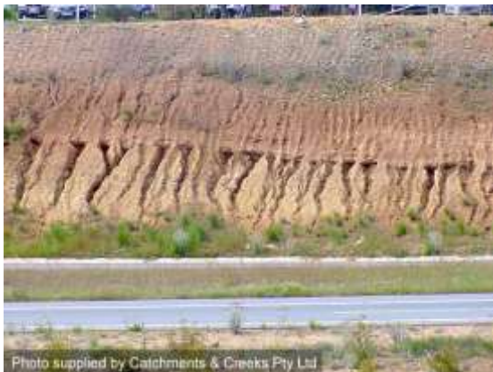
Rilling limited to a given soil horizon
