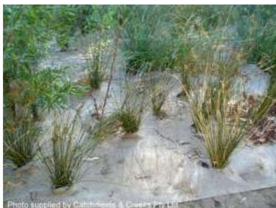
Tube stock planted into a thick blanket
