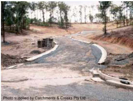
Storm damage to pavement road base
