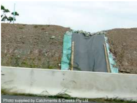
Temporary plastic sheet batter chute
