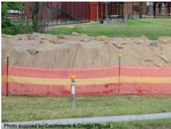
Long-term stockpile covered with jute
