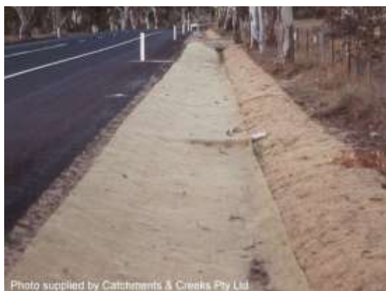
Fine jute mat over seeded soil
