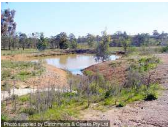
Post-construction farm dam
