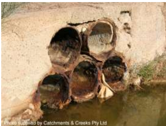
Culvert damaged by acidic water
