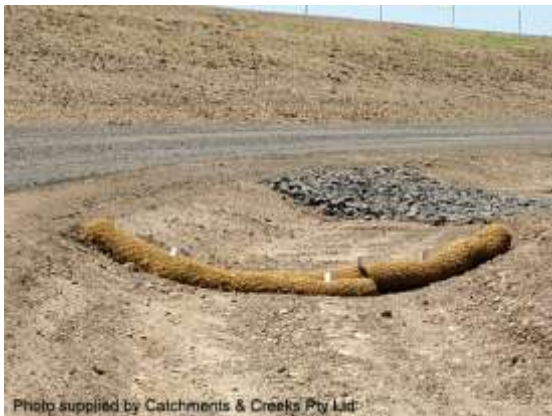
Geo-log check dam
