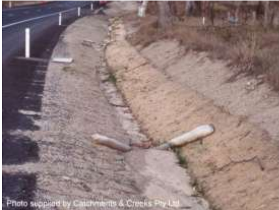
Check dam sediment trap
