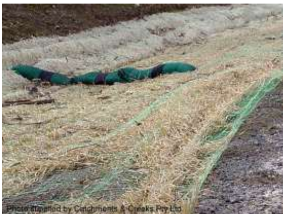
Temporary erosion control mat
