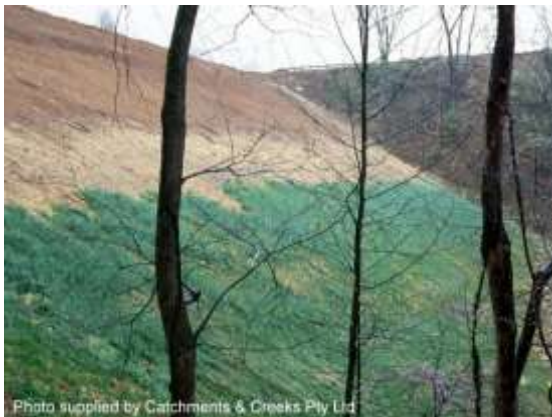
Staged revegetation of road batter
