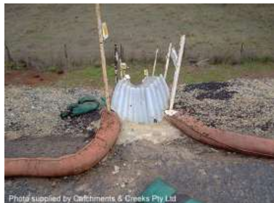
Concrete water seal at chute inlet
