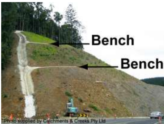
Benched cut batter
