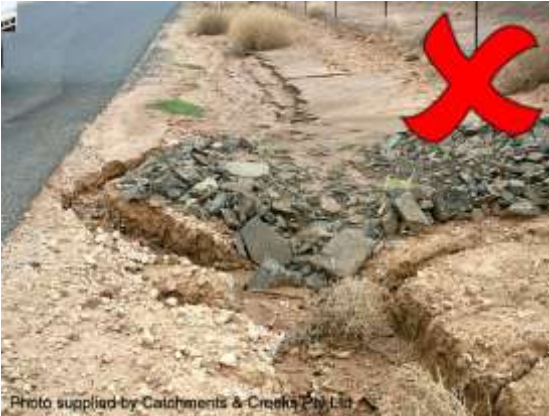
Rock check dam placed on dispersive soil
