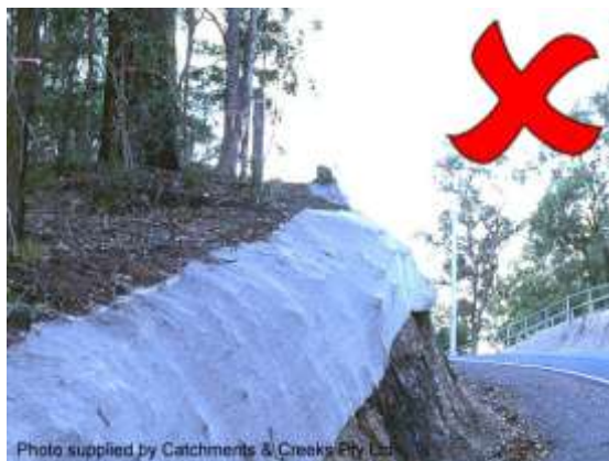
Blanket stretched over irregular ground
