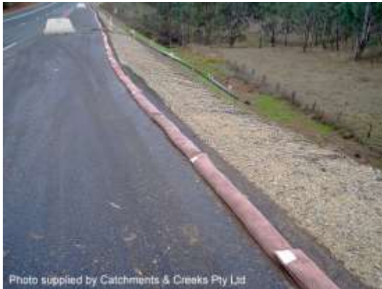
Temporary flow diversion berm
