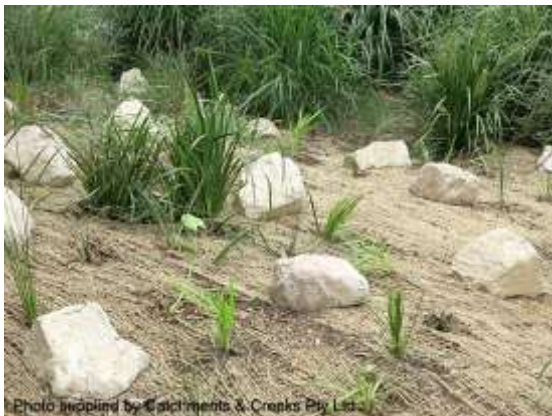
Jute mesh anchored with rocks
