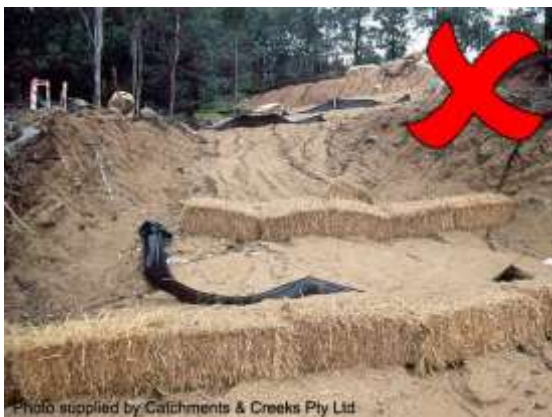
Sediment traps placed on site access
