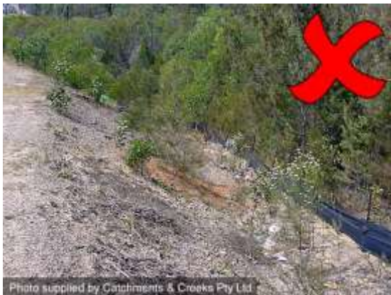
Poor veg growth on heavily-compacted soil
