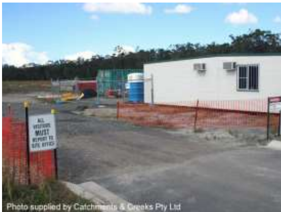
Site entry and office
