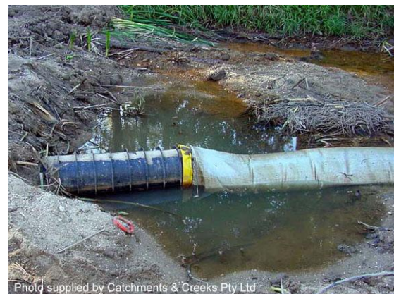
Filter tube connected to ribbed pipe
