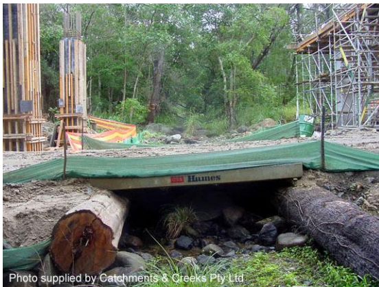
Temporary access construction bridge
