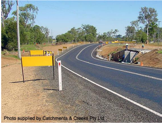
Temporary bypass road
