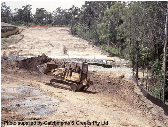
Excavating a sediment basin
