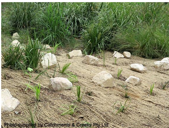
Jute mesh with additional rock anchors
