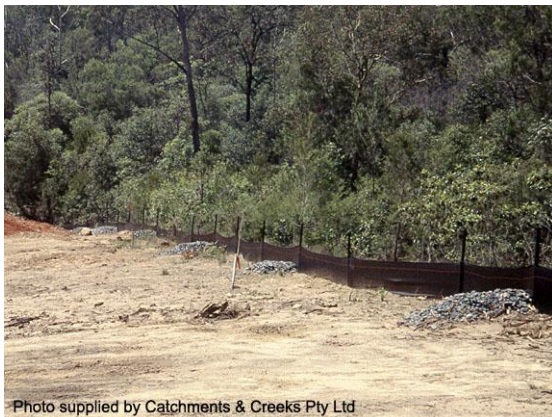
Sediment fence with rock check dams
