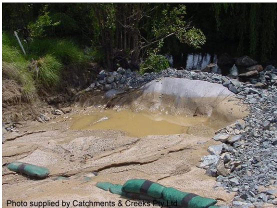
Rock filter dam (Type-2 sediment trap)
