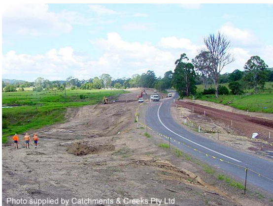
Road construction works
