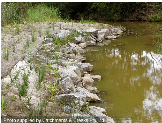
Vegetated rock stabilisation of bank
