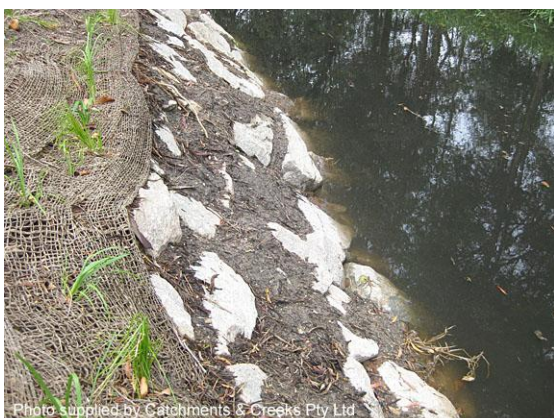
Voids filled with topsoil ready for planting
