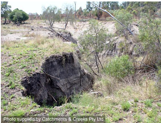
Lateral bank erosion
