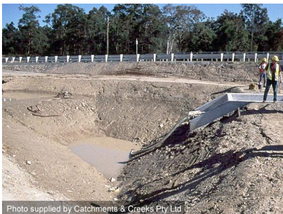
Sediment basins (Type-1 sediment trap)
