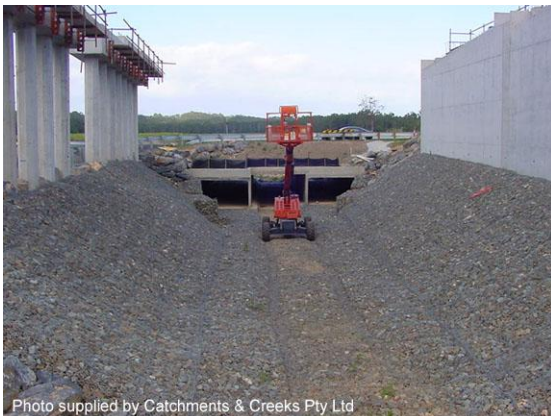
Non-vegetated rock mattresses
