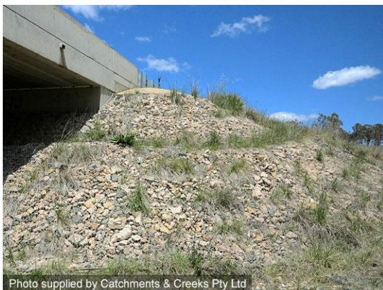
Vegetated rock mattresses
