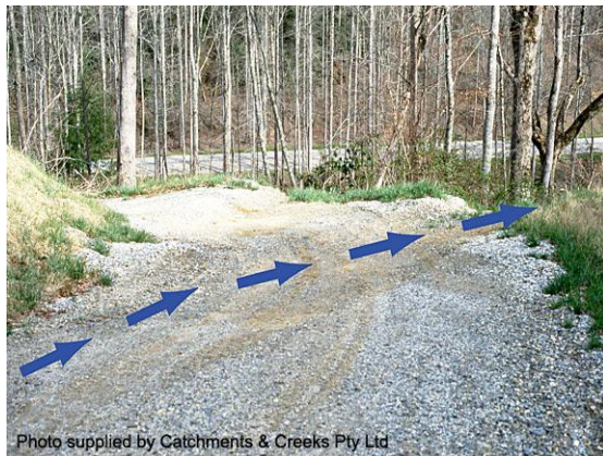
Flows diverted off access track
