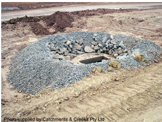
Rock & aggregate drop inlet sediment trap
