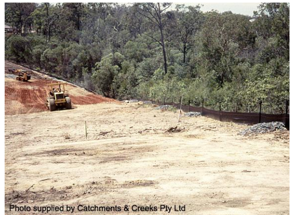
Sediment fence with rock check dams
