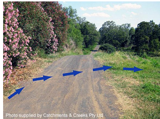
Cross bank placed at top of descent
