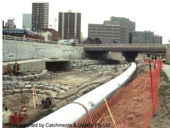
Instream works with piped-flow bypass
