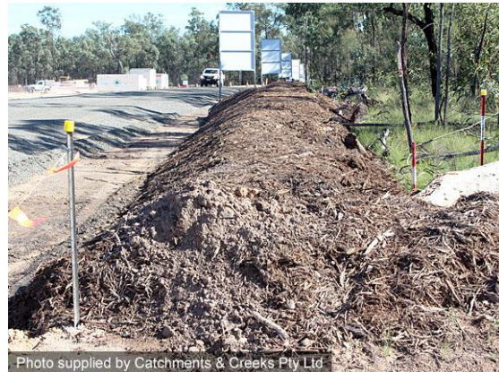
Mulch berm sediment barrier
