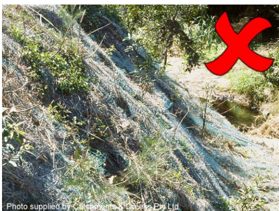
Synthetic reinforced erosion control mat
