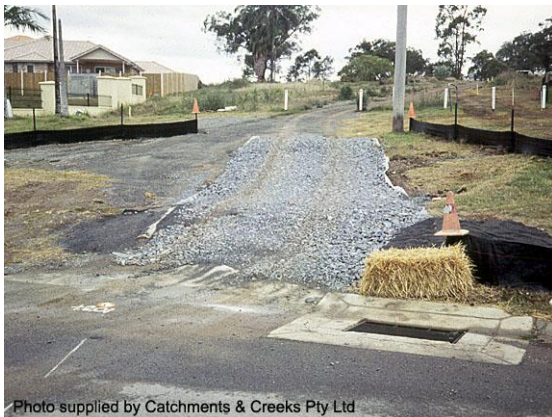
Rock pad with flow diversion berm
