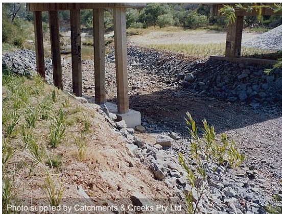
Rock stabilisation of bed and banks
