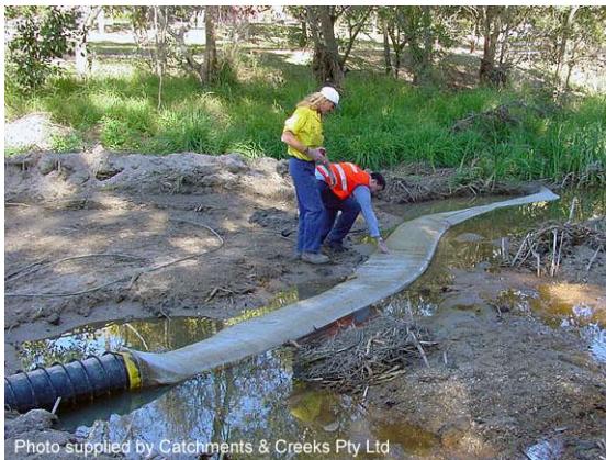
Instream sediment control system
