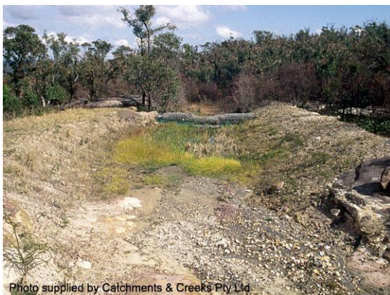
Type-2 sediment trap (1994)
