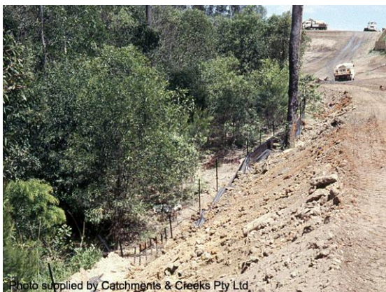
Spill-through weir outlet structure
