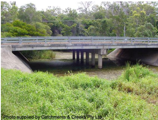
Concrete abutments
