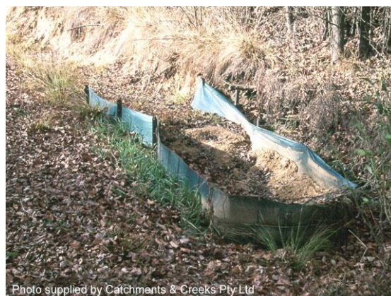
U-shaped sediment trap on steep slope
