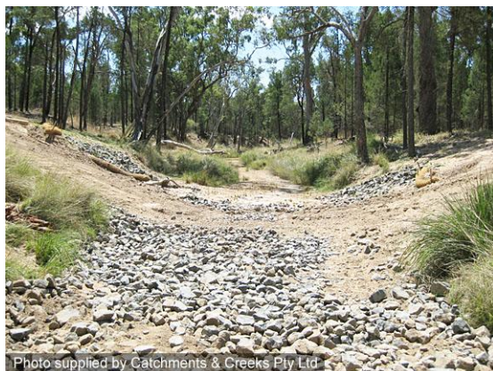
Rock-stabilised vehicle crossing
