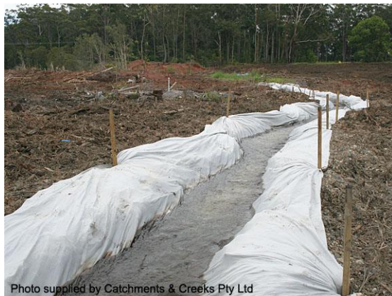
Clean water cross-drainage system
