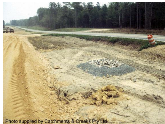
Rock & aggregate drop inlet sediment trap
