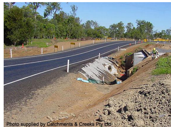
Example of a temporary bypass road
