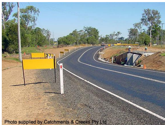
Temporary bypass road
