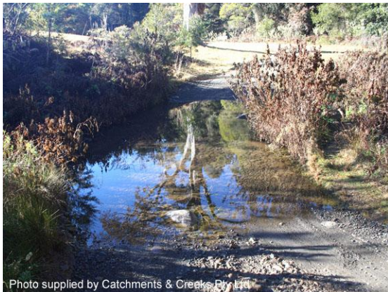
Ford crossing of alluvial stream
