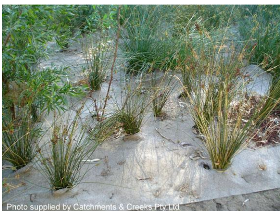
Jute erosion control blanket
