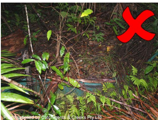
Sediment fence located in bushland
