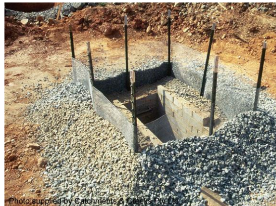
Mesh & aggregate drop inlet sediment trap
