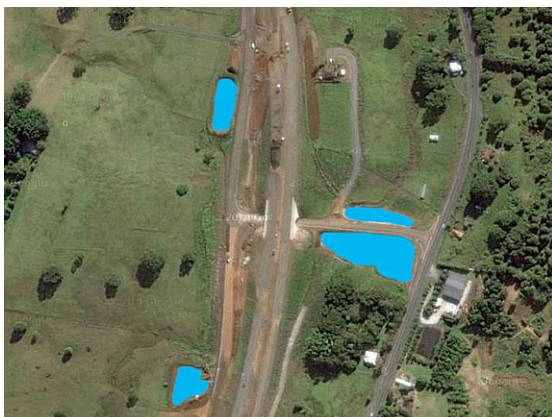
Rural road construction
