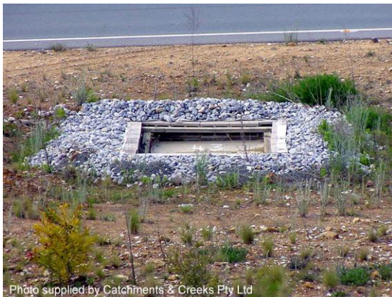
Block & aggregate drop inlet sediment trap
