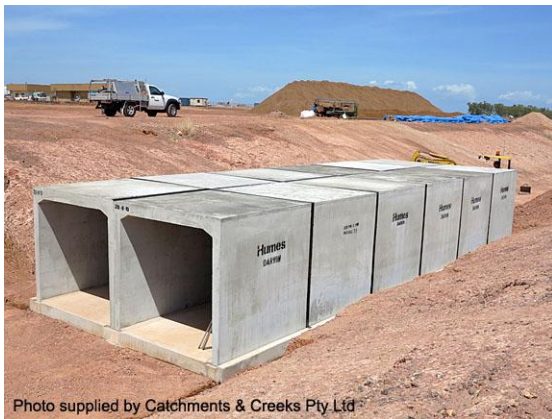
Culvert construction in a dry channel
