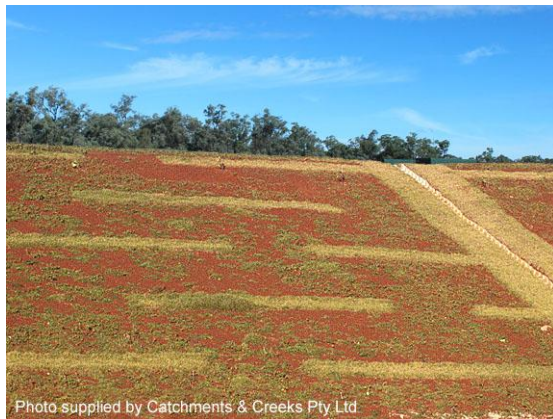
Turf filter strips placed along the contour
