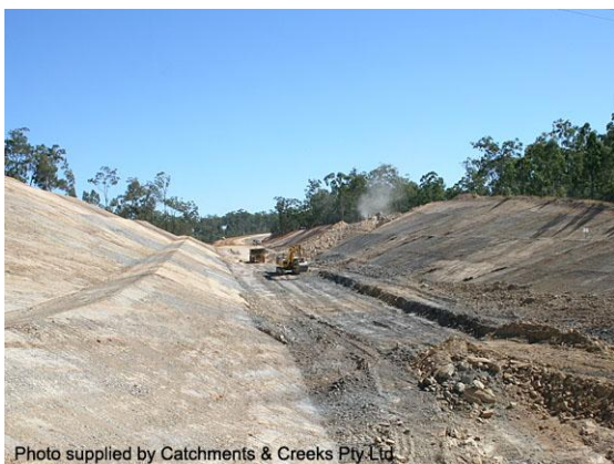
Road construction works
