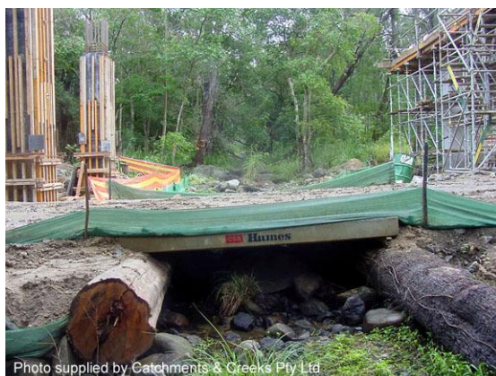
Temporary stream crossing
