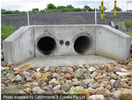
Minor culvert crossing
