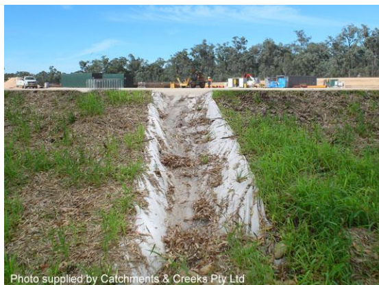
Temporary batter chute
