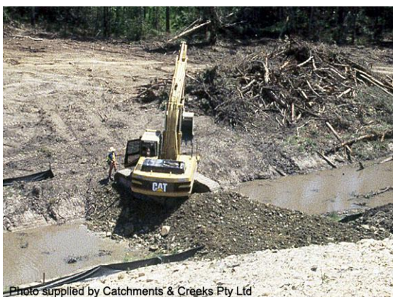
Cofferdam construction
