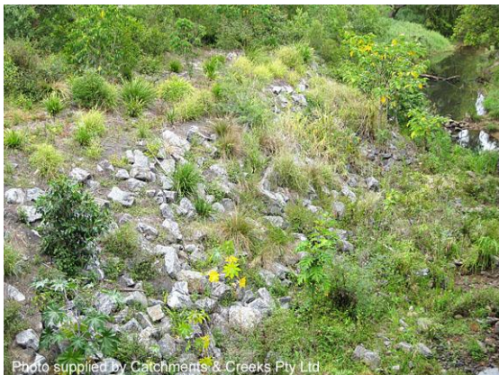
Planted rock-stabilised creek bank
