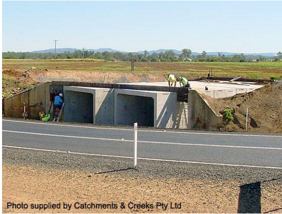
Culvert construction
