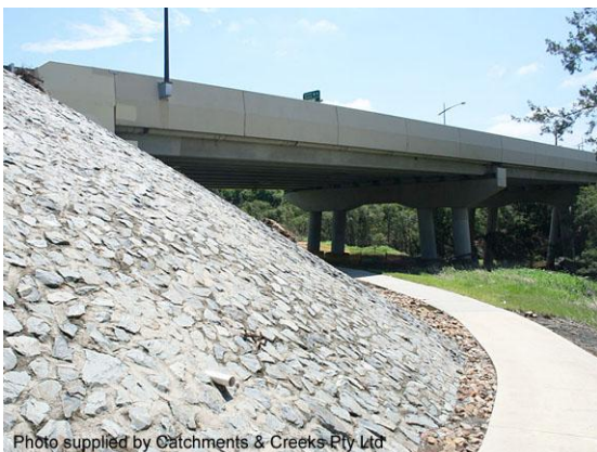
Grouted stone pitched abutment
