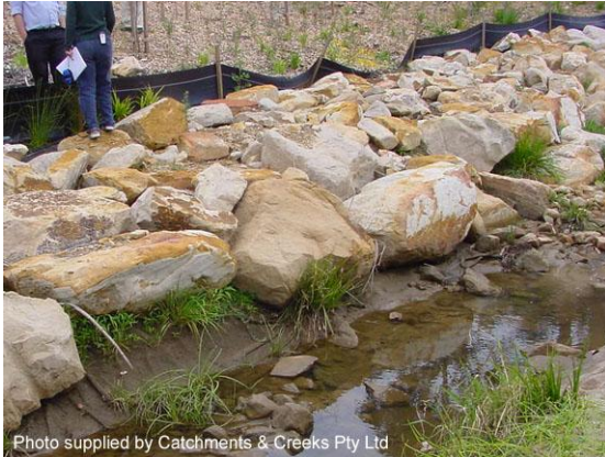
Larger rocks forming toe protection
