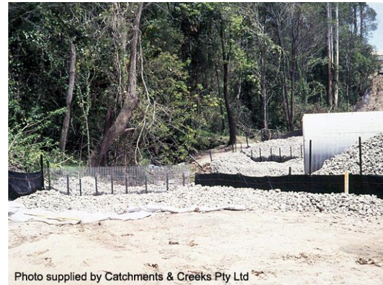
Rock filter dam outlet structure
