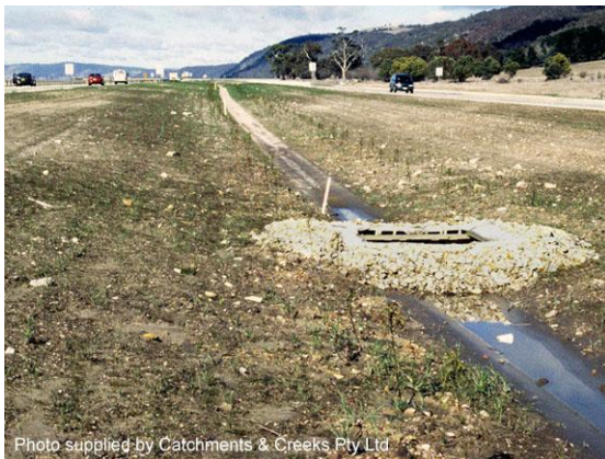
Drop inlet sediment trap
