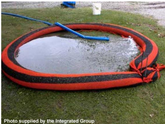
Compost-filled filter sock/berm
