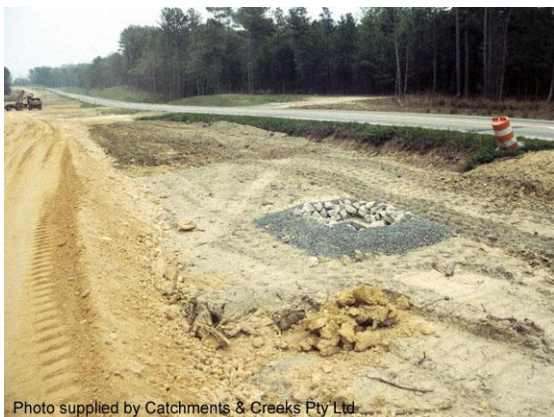
Type-2 drop inlet sediment trap
