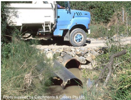
Temporary pipe culvert
