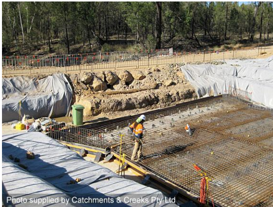
Construction of a culvert base slab
