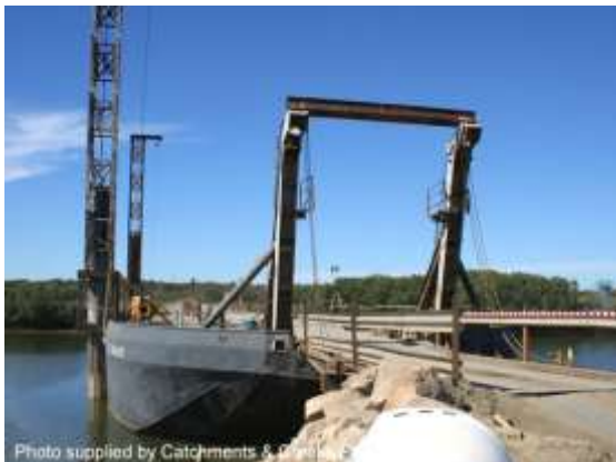
Barge crossing of tidal inlet
