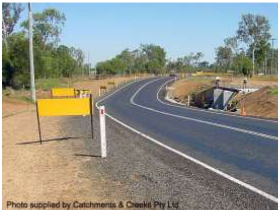
Temporary bypass road
