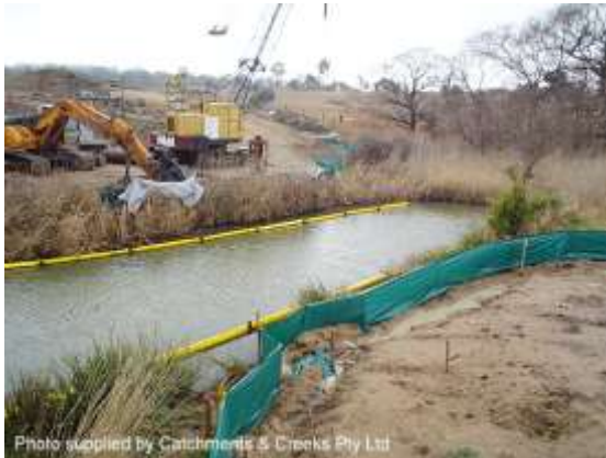
Sediment fence (Type-3 sediment trap)
