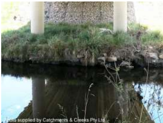
Vegetated rock stabilisation
