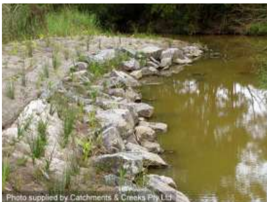
Vegetated rock stabilisation of bank
