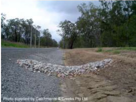
Velocity control check dam
