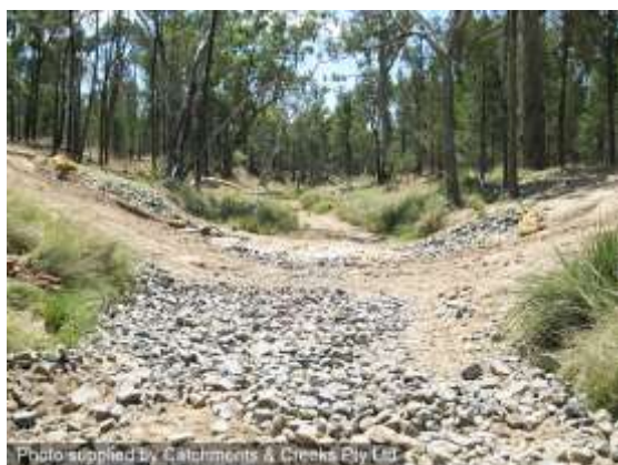
Rock-stabilised vehicle crossing
