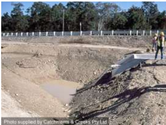
Sediment basins (Type-1 sediment trap)
