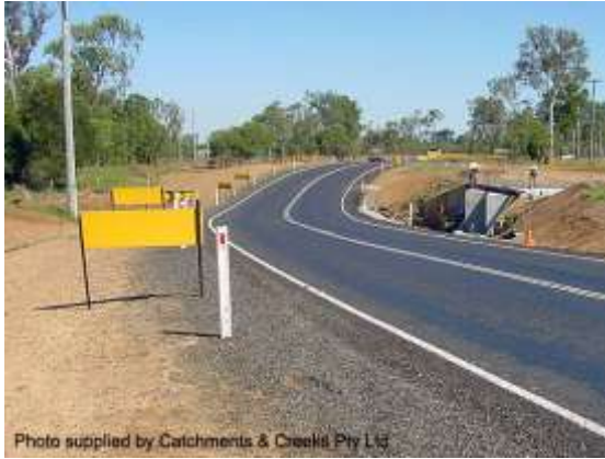
Temporary bypass road
