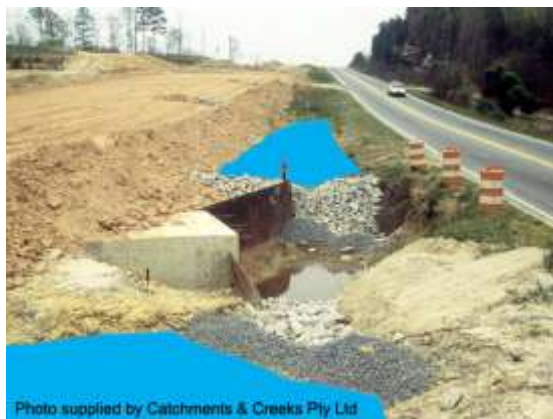
Culvert construction
