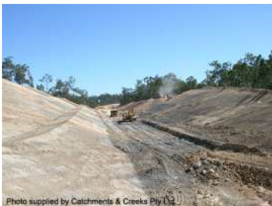
Road construction works
