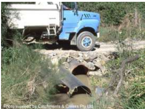
Temporary pipe culvert
