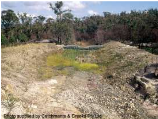
Type-2 sediment trap (1994)
