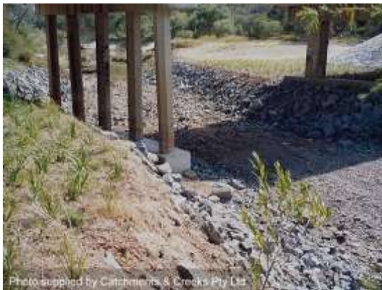
Rock stabilisation of bed and banks
