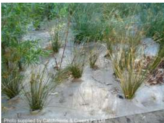
Jute erosion control blanket
