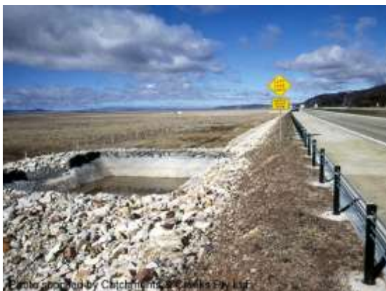
Roadside pollution containment pond
