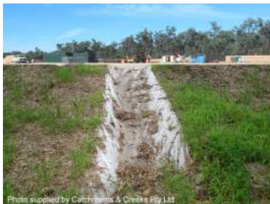
Temporary batter chute
