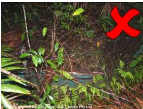
Sediment fence located in bushland
