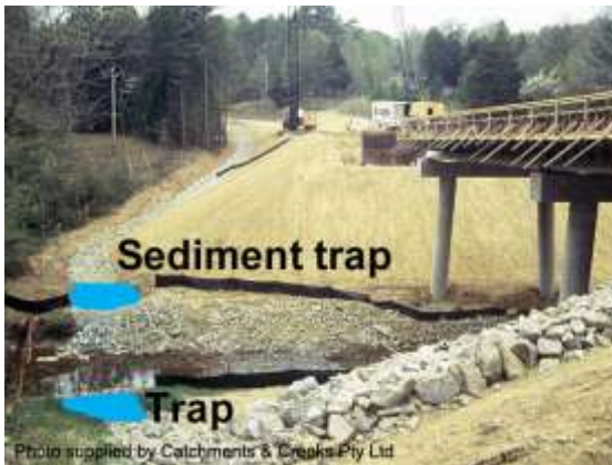
Rock filter dams (Type-2 sediment trap)
