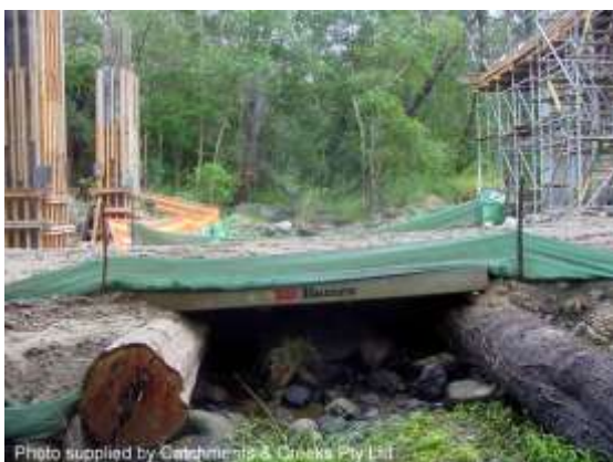
Temporary access construction bridge
