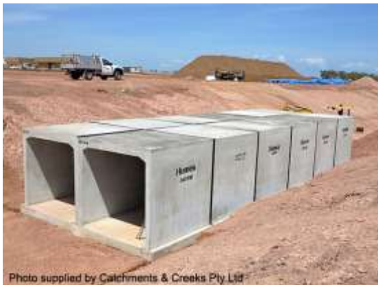
Culvert construction in a dry channel
