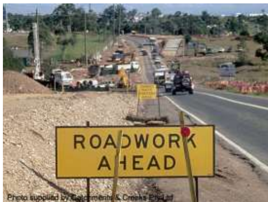
Duplication of an existing roadway
