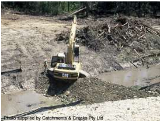
Cofferdam construction
