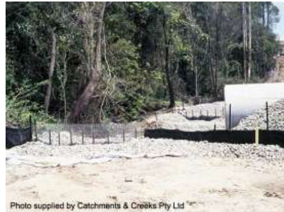
Rock filter dam outlet structure
