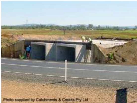
Culvert construction
