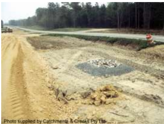
Type-2 drop inlet sediment trap
