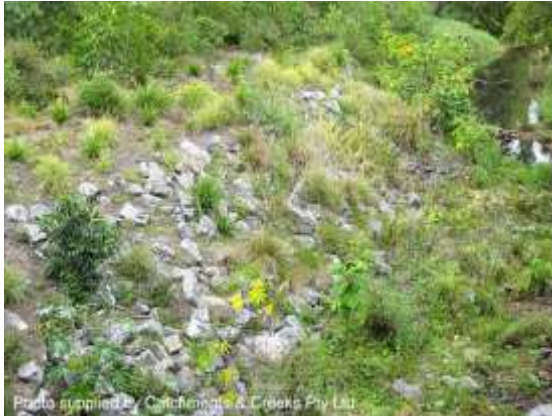
Planted rock-stabilised creek bank
