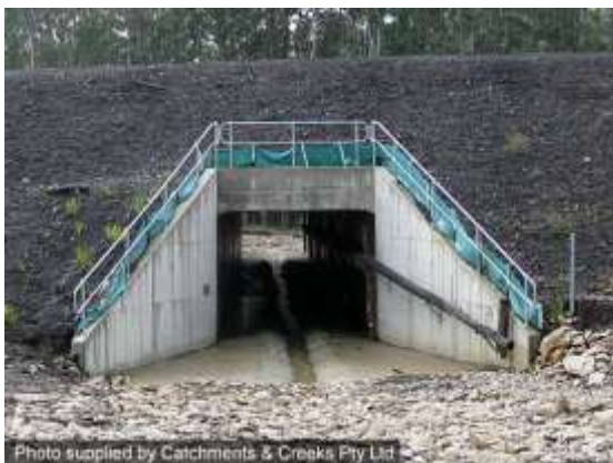
Fauna passage culverts
