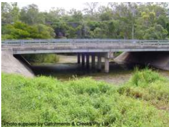
Concrete abutments
