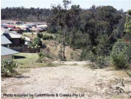
Road reserve prior to road works
