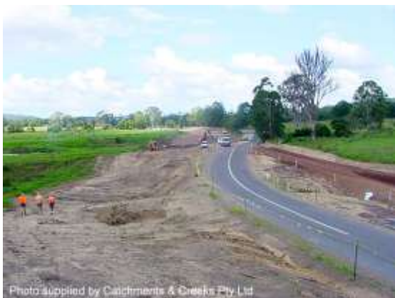
Road construction works
