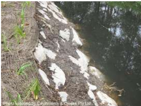
Voids filled with topsoil ready for planting
