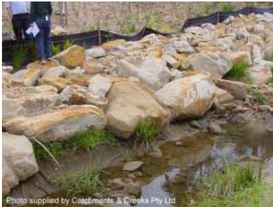
Larger rocks forming toe protection
