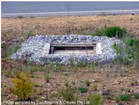
Block & aggregate drop inlet sediment trap
