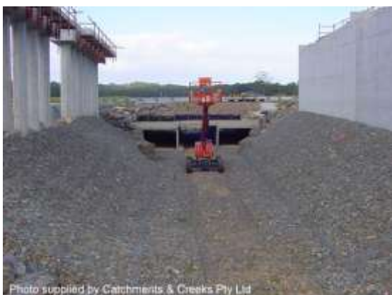
Non-vegetated rock mattresses
