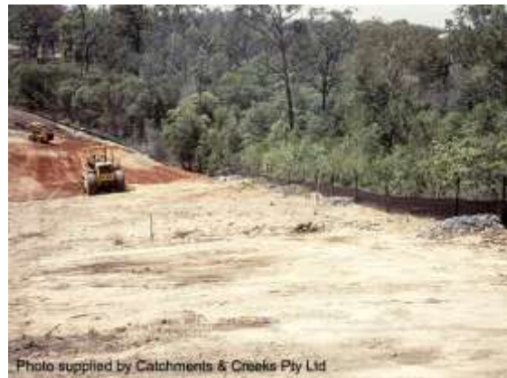
Sediment fence with rock check dams
