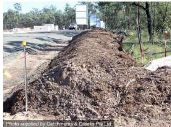
Mulch berm sediment barrier
