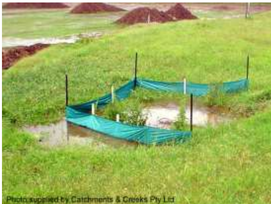
Sediment fence (Type-3 sediment trap)
