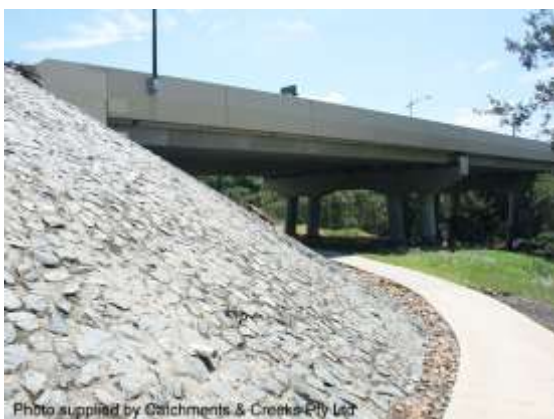
Grouted stone pitched abutment
