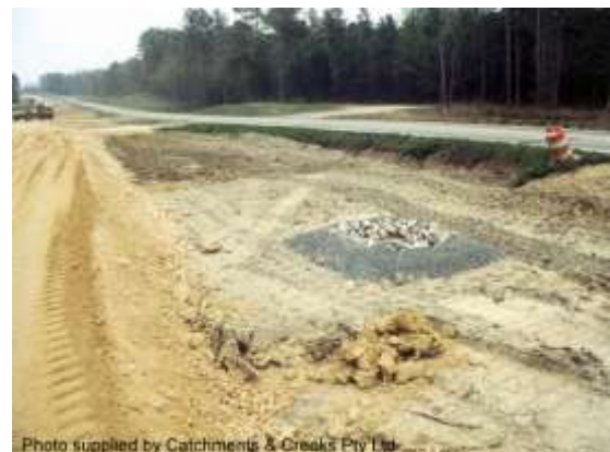
Rock & aggregate drop inlet sediment trap
