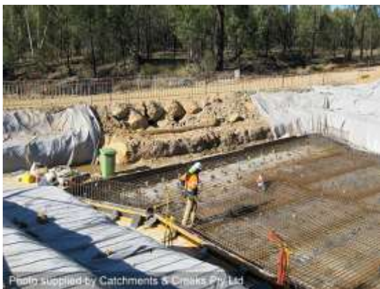
Construction of a culvert base slab
