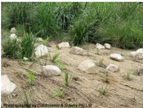
Jute mesh with additional rock anchors
