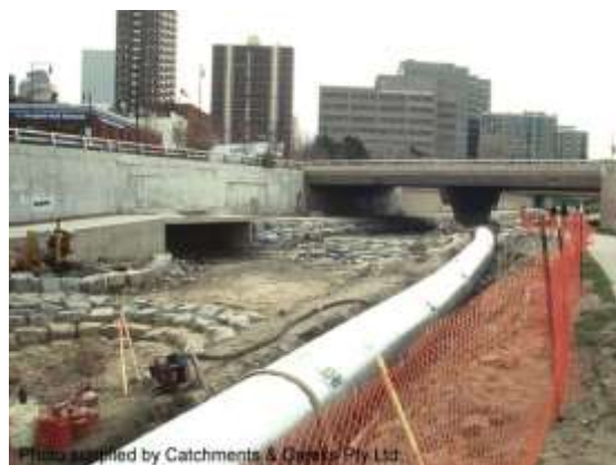
Instream works with piped-flow bypass
