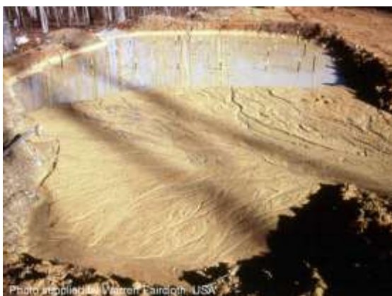
Sediment retained in a sediment trap
