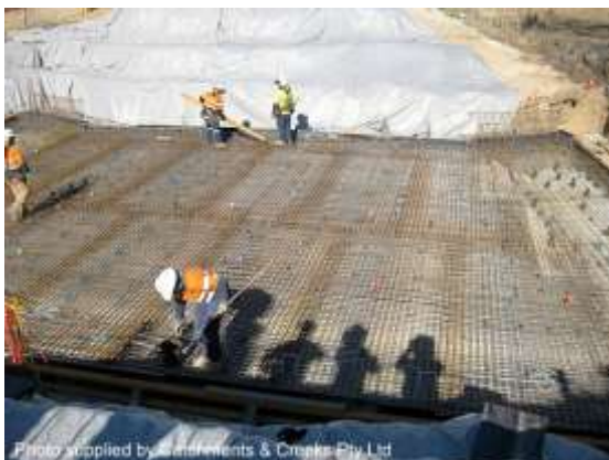
Construction of a culvert base slab
