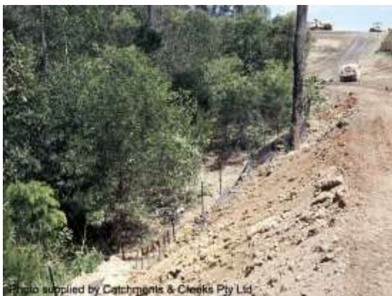
Spill-through weir outlet structure
