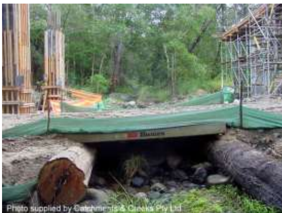
Temporary stream crossing
