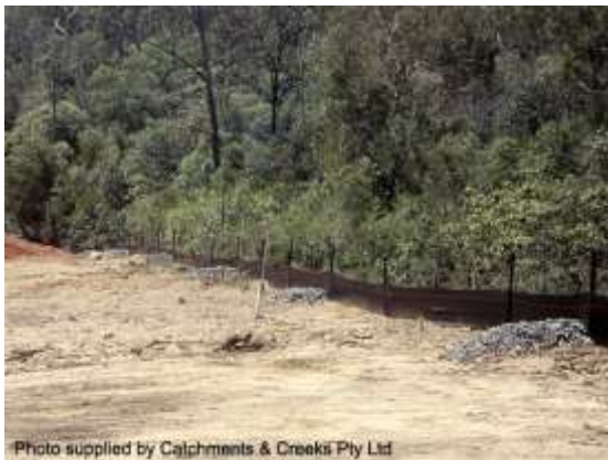
Check dams adjacent to a sediment fence
