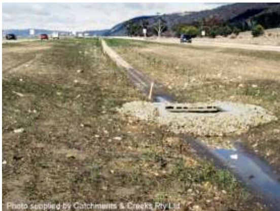
Drop inlet sediment trap
