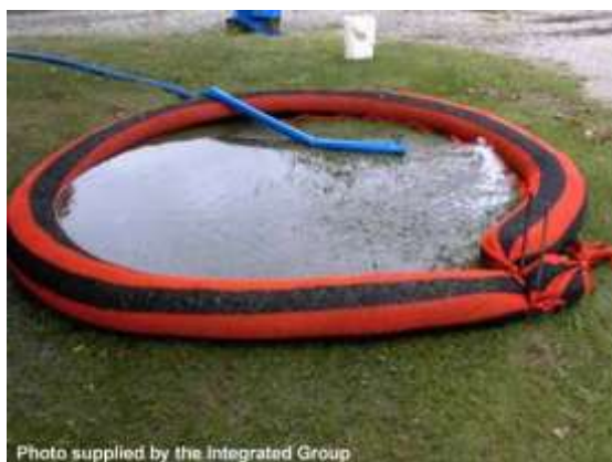
Compost-filled filter sock/berm
