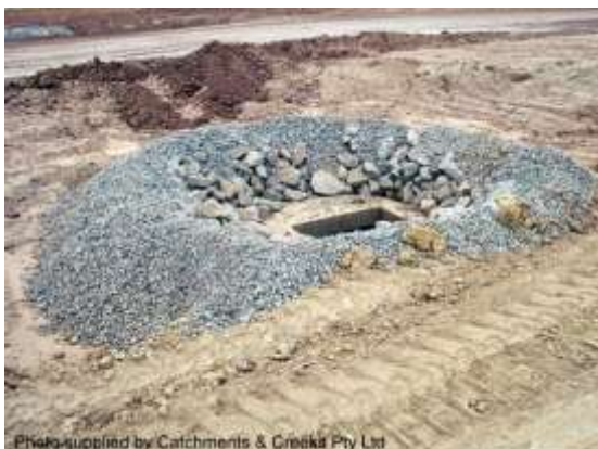
Rock & aggregate drop inlet sediment trap
