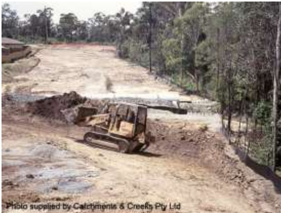
Excavating a sediment basin
