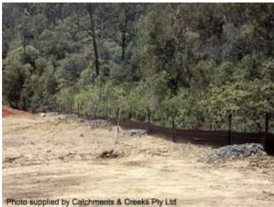
Sediment fence with rock check dams
