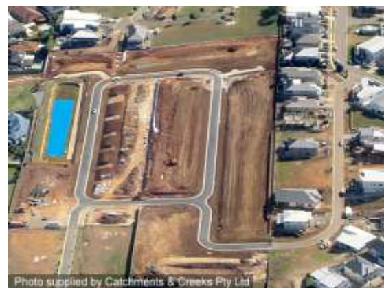
Residential road construction
