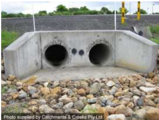
Minor culvert crossing
