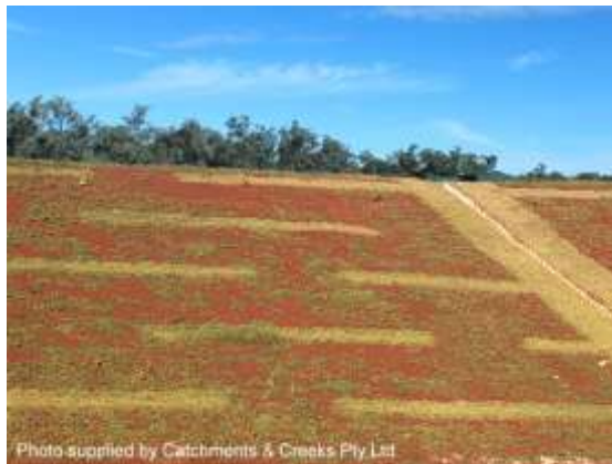
Turf filter strips placed along the contour
