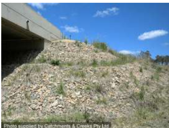
Vegetated rock mattresses
