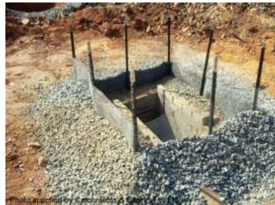
Mesh & aggregate drop inlet sediment trap
