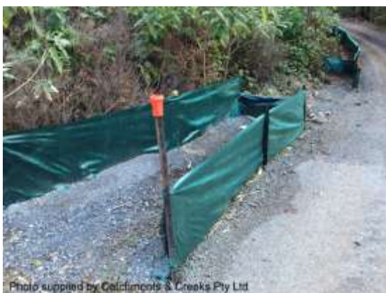
U-shaped sediment trap on mild slope
