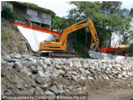
Rock placement over filter cloth
