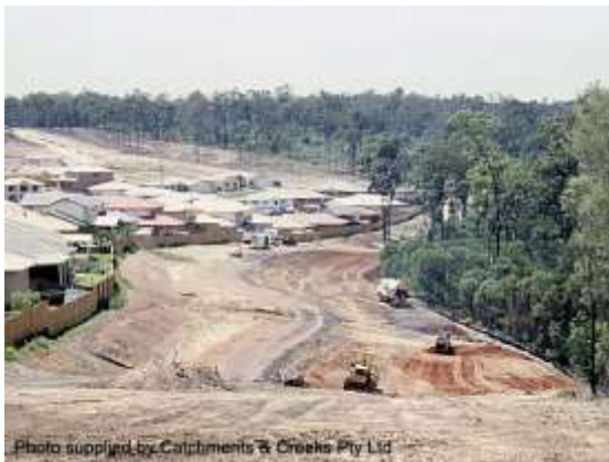
Topsoil cleared from road reserve
