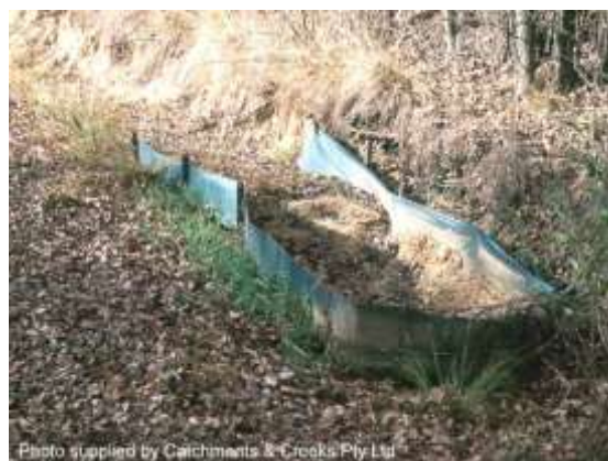
U-shaped sediment trap on steep slope
