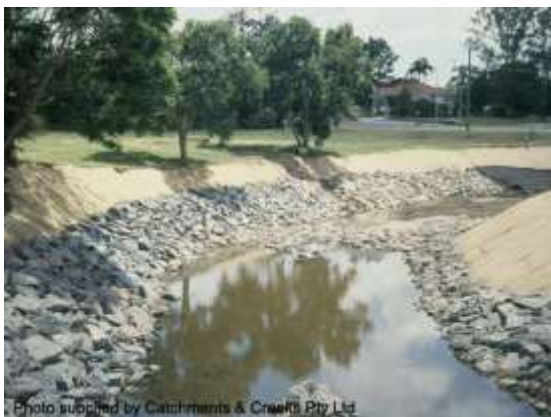
Rock stabilisation on channel bend
