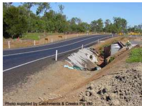
Example of a temporary bypass road
