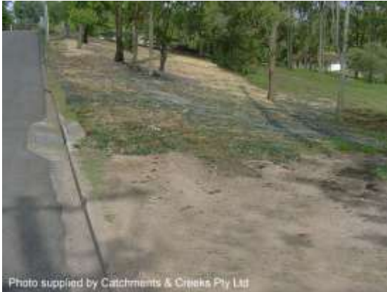
Compacted clay soil (2003)
