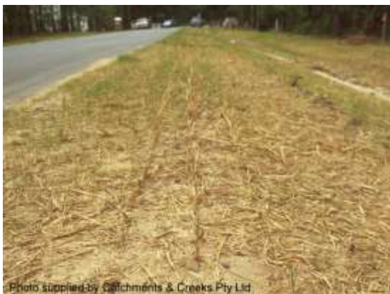
Crimped straw mulch (USA)
