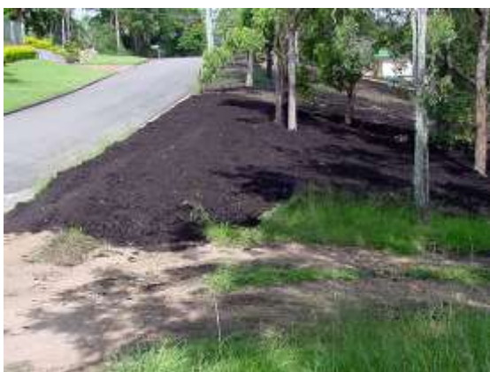
Mulch treatment of a compacted soil (Qld)
