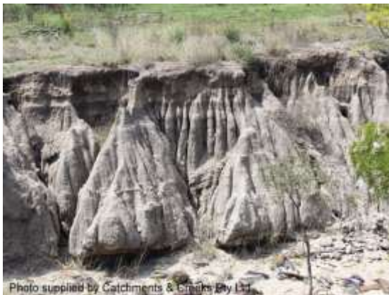
Dispersive soil bank erosion (Qld)
