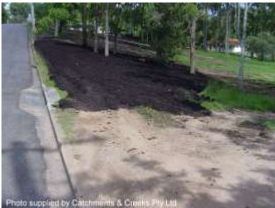
Placement of treated mulch (2003)
