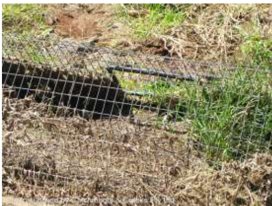
A-frame, wire mesh, leaky weir (Qld)
