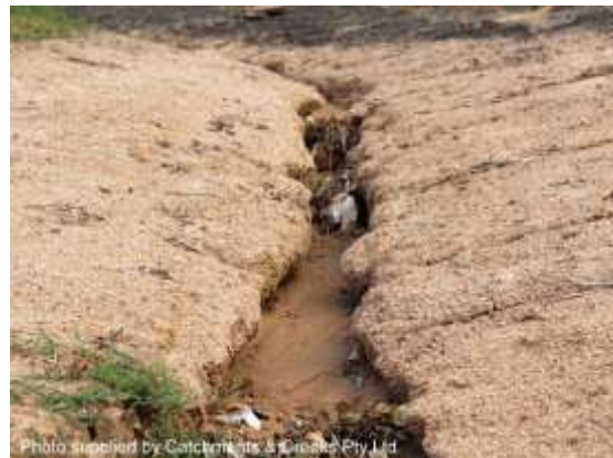
Invert rill erosion (Qld)
