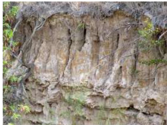
Creek bank erosion (Qld)
