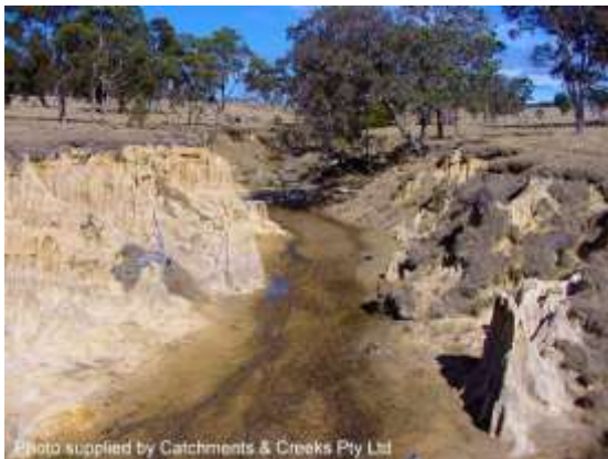
Dispersive soil creek erosion (NSW)
