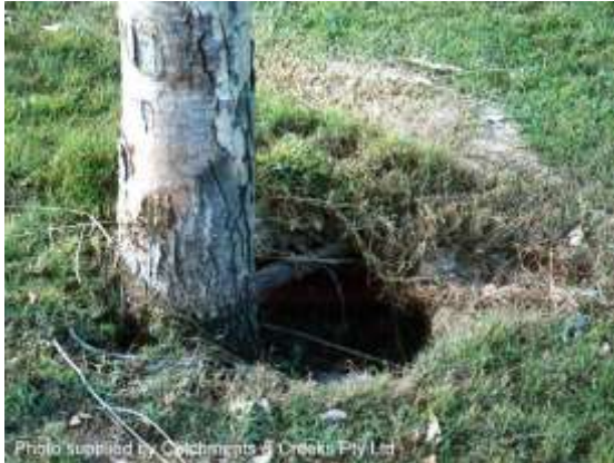
Flood-induced soil scour
