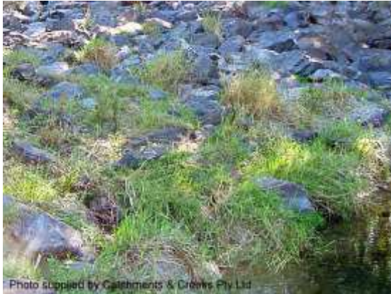
Vegetated rock placement (NSW)
