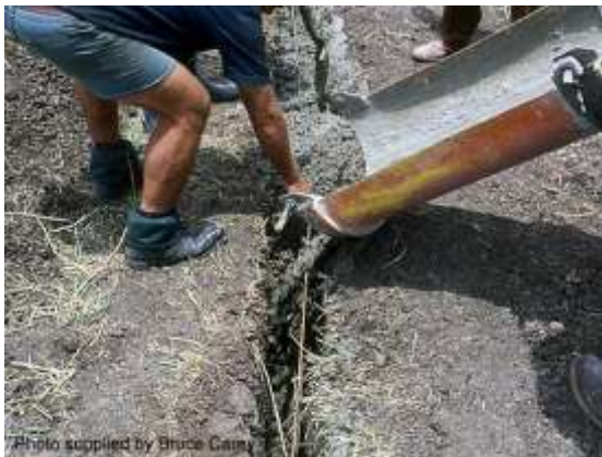
Poring concrete into cut-off trench
