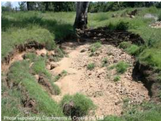
Erosion downstream of a floodplain tree
